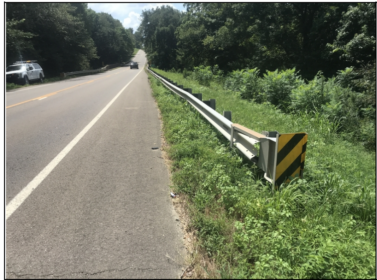
Northwest approach guardrail with damage to the end terminal and the guardrail.
