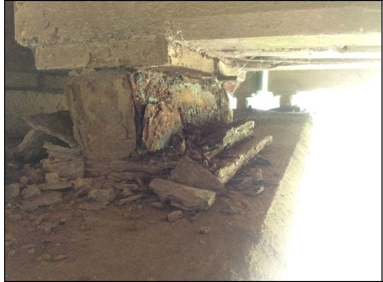
Span #3, bearing #2, over bent #3- Severe corrosion / section loss. Photo #2.
