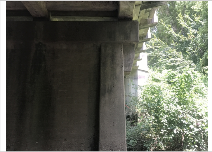
Bent #3 Column # vertical cracks in the edge of the column.
