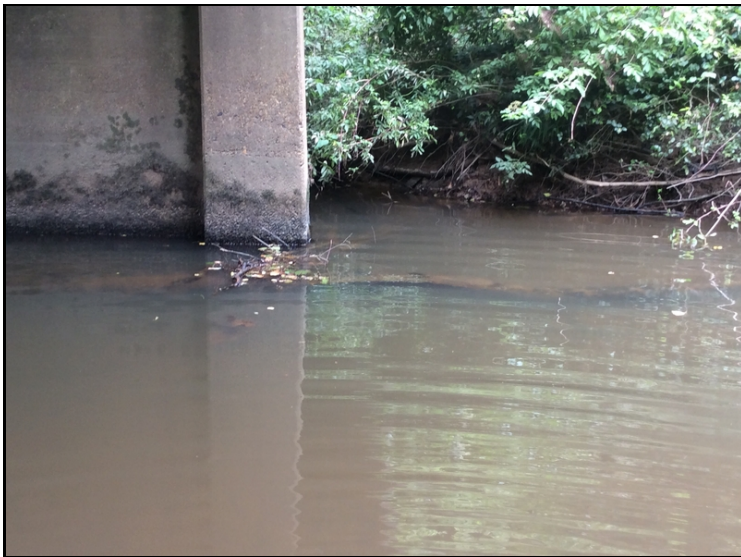
Bent #3, column #2-Drift.
