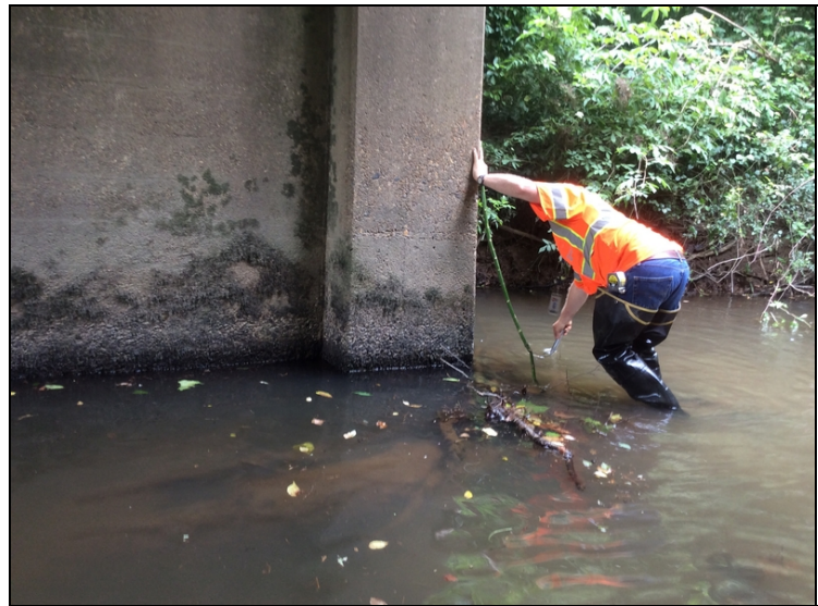
Scour hole at column #2 of bent #3.
