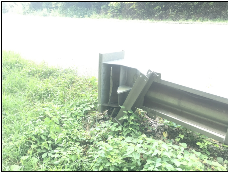
Southeast approach guardrail end terminal with a broke post.
