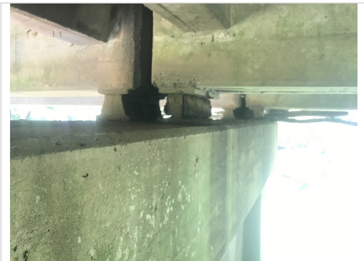
Bent #2 bearings with active corrosion and layers of flaking rust.
