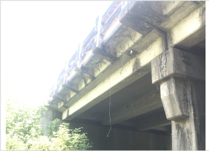
Span #3 Lt spalling with exposed reinforcing steel on the undersurface of the deck and on the rail post undersurface.
