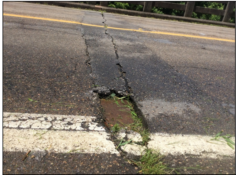
Bent #2 expansion joint-Pothole in asphalt driving surface.
