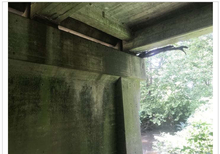
The backface of bent #2 cap has a shallow 8" spall with exposed reinforcing steel on the right side.
