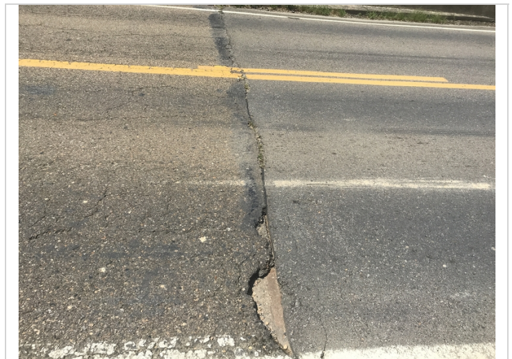
Abutment #2 wearing surface over the expansion joint.
