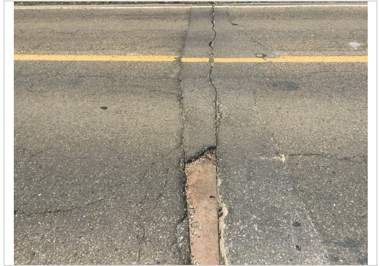
Bent #2 wearing surface over the expansion joint.
