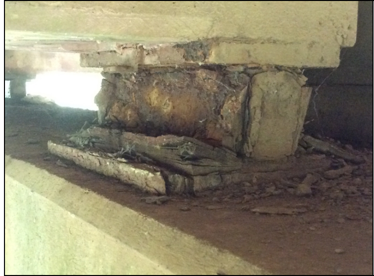
Span #3, bearing #3, over bent #3- Severe corrosion / section loss.
