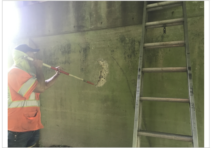
Backface of bent #2 pier wall has a 16" delaminated/spall under girder #2.
