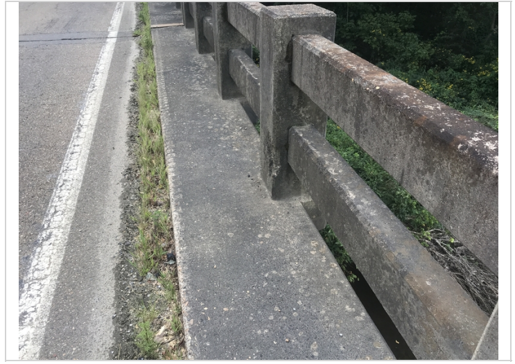
Left bridge rail with spalling.
