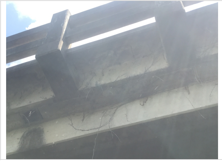
Span #2 Lt spalling under the concrete curb.
