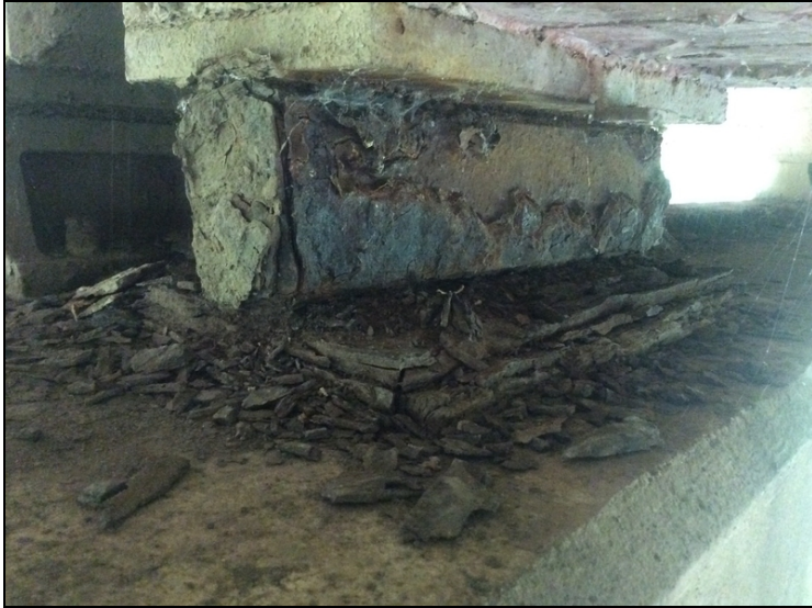
Span #1, bearing #2 over bent #2- Severe corrosion / section loss.
