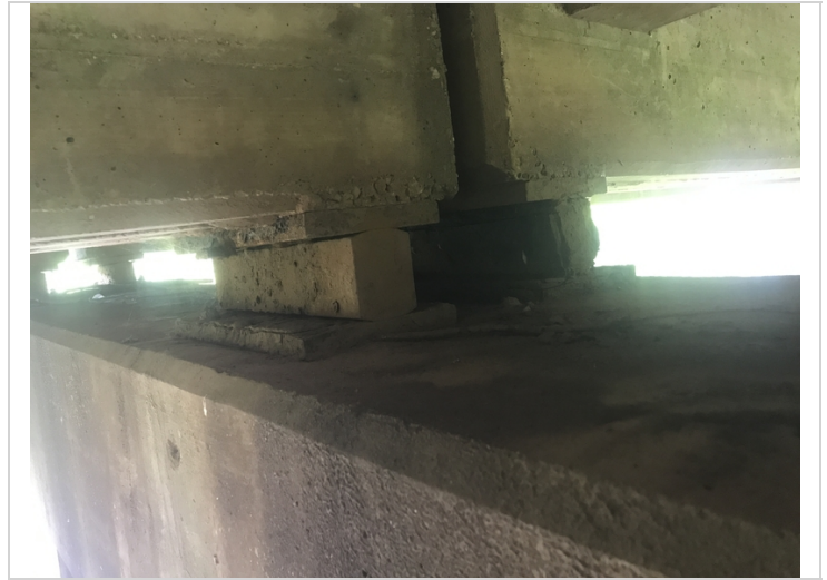
Bent # 3 bearings with active corrosion and layers of flaking rust.
