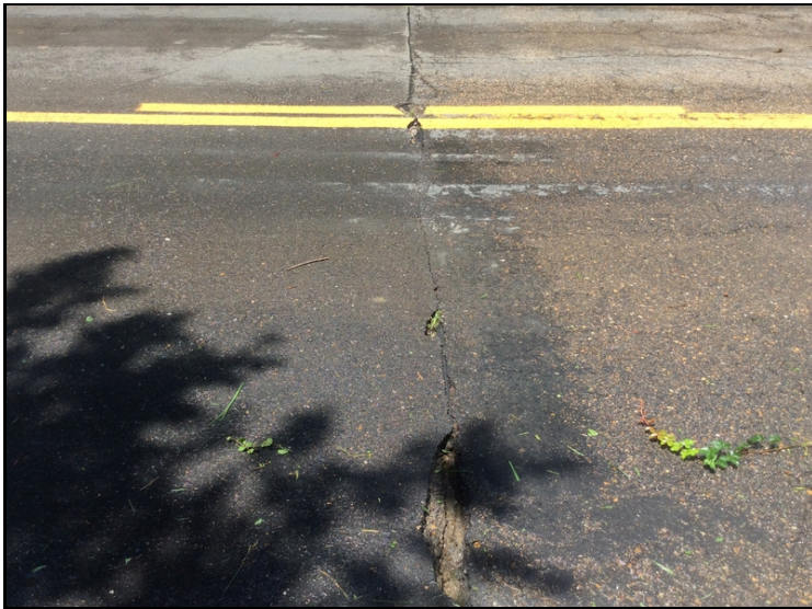
Pothole forming over abutment #1 expansion joint.
