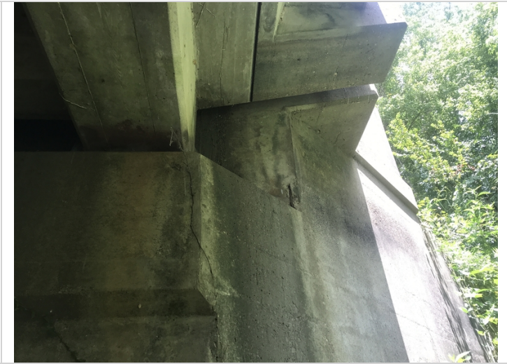
Abutment #2 Rt shallow spalling with exposed reinforcing steel at the wing wall juncture.
