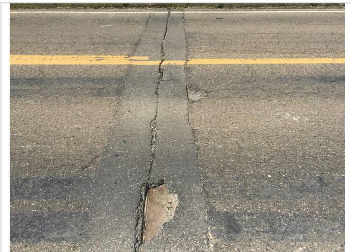
Bent #3 wearing surface over the expansion joint.
