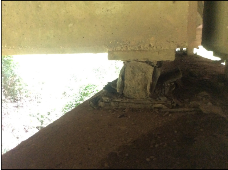
Span #3, bearing #2-Severe corrosion / section loss.
