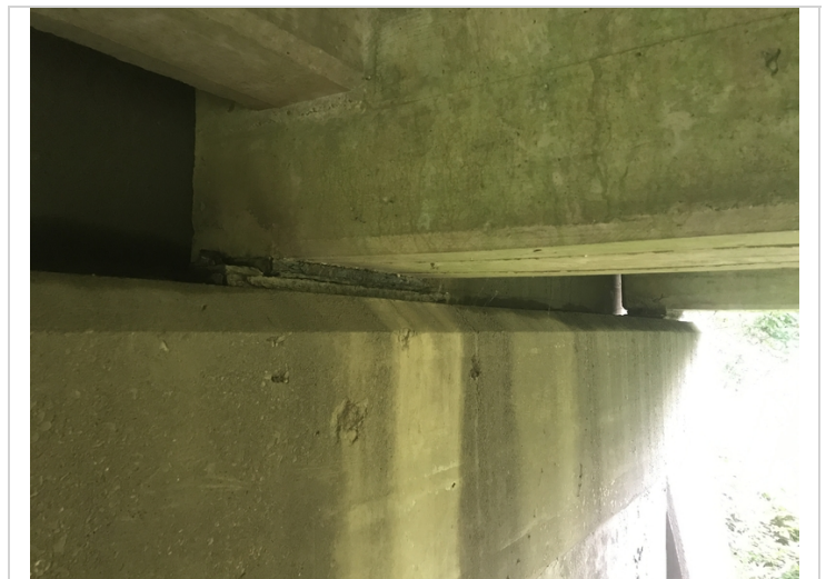
Abutment #1 bearings with active corrosion and layers of flaking rust.
