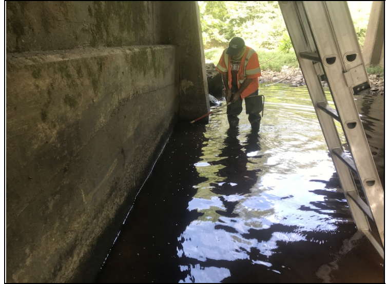
Abutment #1 Lt undermining.
