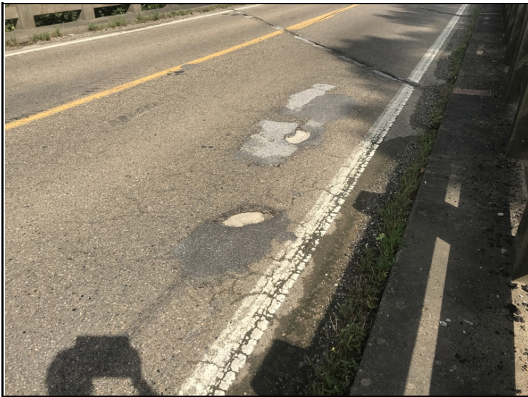
Span #1 asphalt deterioration with potholes in the northbound lane.
