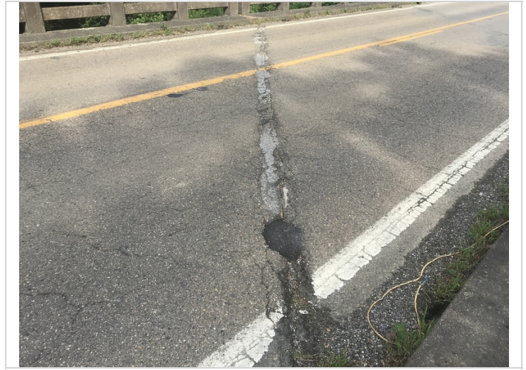
Bent #3 typical asphalt deterioration over the intermediate bents.
