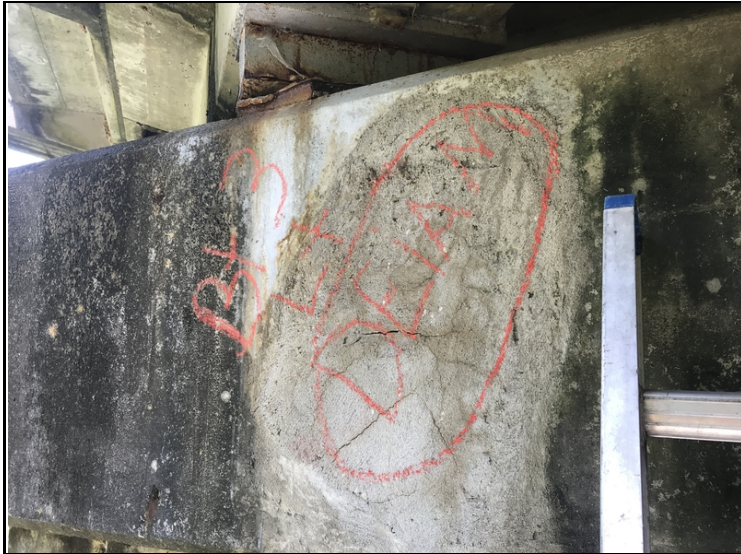
The repair to the backface of bent # 3 cap on the left side over column # 1 is cracked and delaminated.
