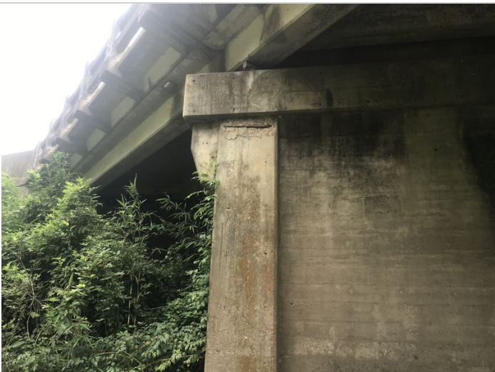
Span #2, Bent #3 Column #1 spalling with exposed reinforcing steel.
