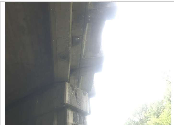
Span # 2, Lt post support over Bent # 2 has a 12" spall with exposed reinforcing steel under the deck overhang.
