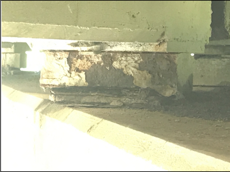
Bent # 3, bearing # 2-Corrosion with thick flaking rust.
