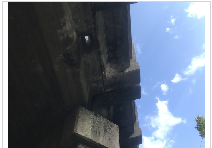
Span #1 Rt over Bent #2 spalling with exposed reinforcing steel.
