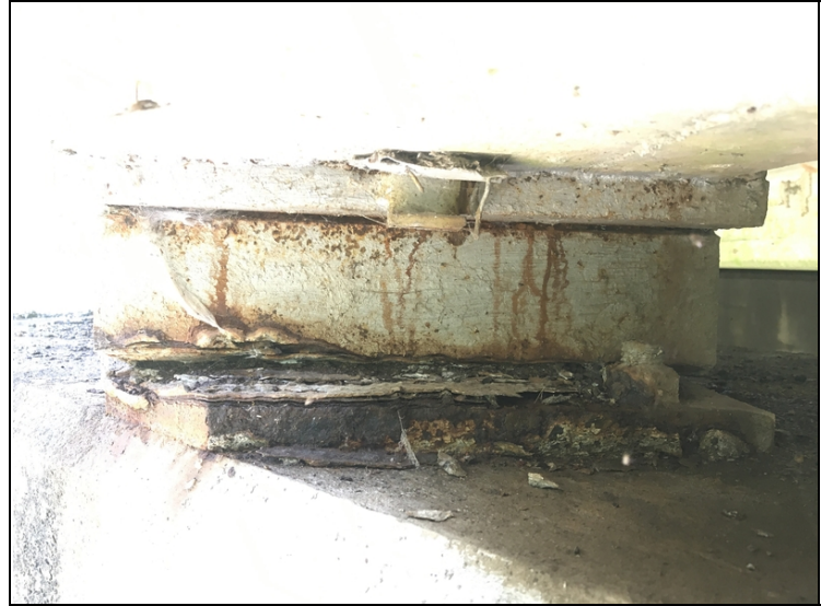
Span # 2, bearing # 1 over bent # 3-Corrosion with section loss to masonry plate.
