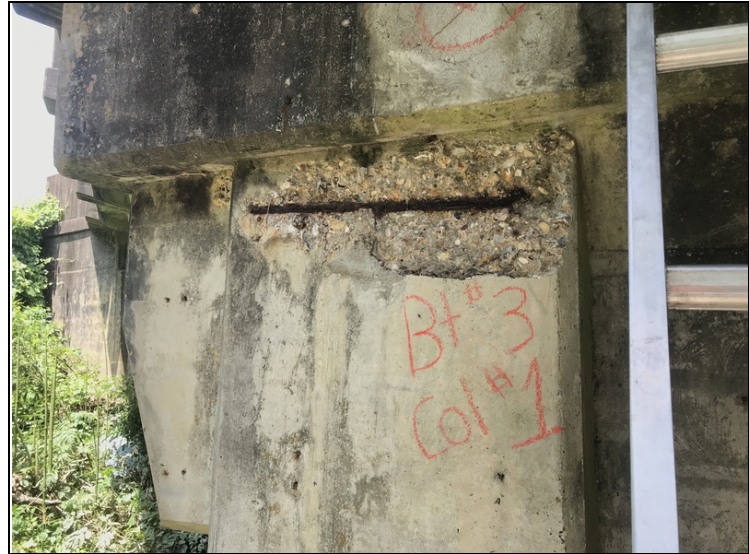
Bent # 3, column # 1-Spalling with exposed reinforcing steel.
