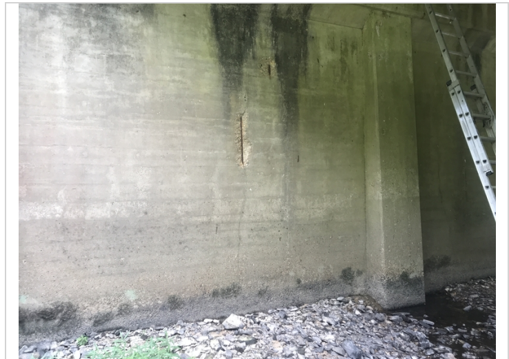
Span # 2, Bent # 3 Bay # 1 spalling with exposed reinforcing steel.
