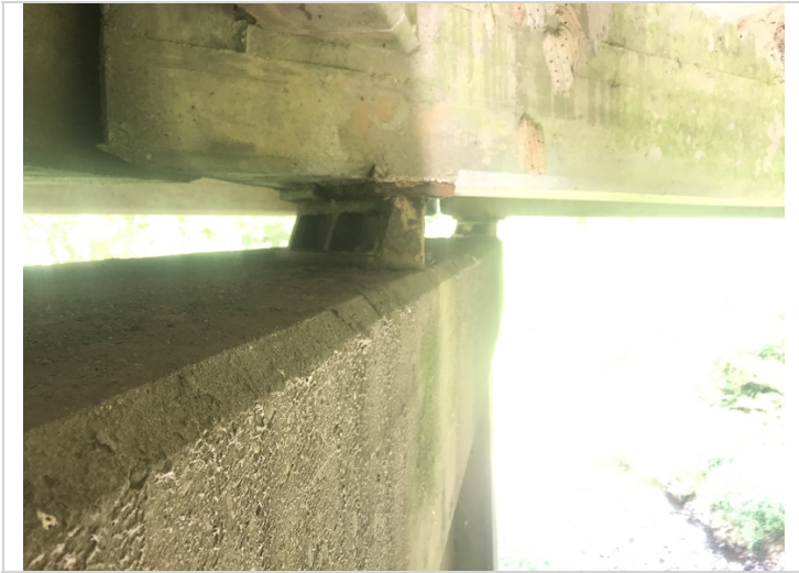
Span #2, Bent #2 bearings with active corrosion and layers of flaking rust.
