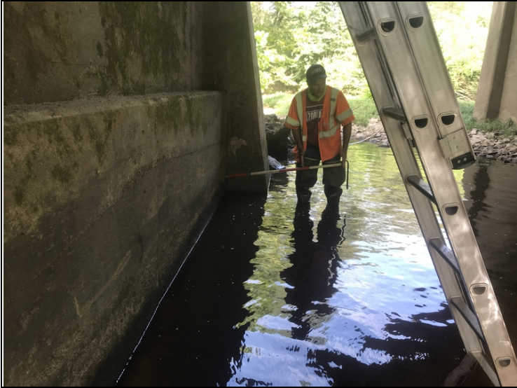
Abutment #1 Lt undermining scale.
