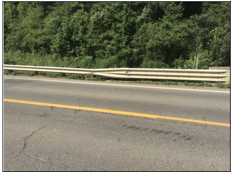
Southwest approach guardrail with minor collision damage.
