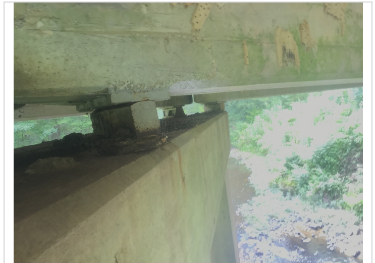
Span # 1 Bent # 2 active corrosion with layers of flaking rust between the masonry and bearings.
