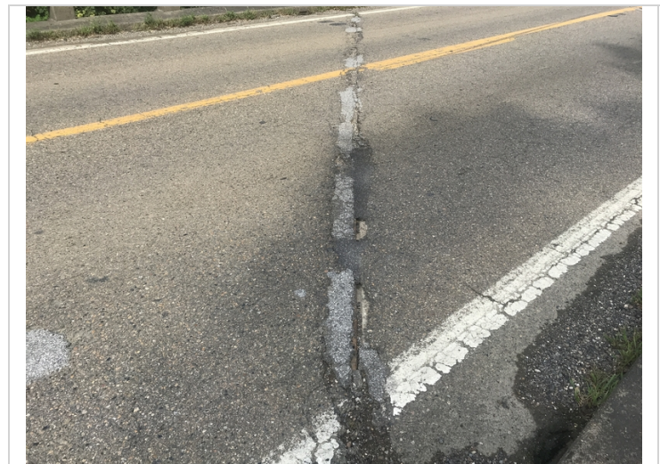
Bent #2 wearing surface over the intermediate bent.
