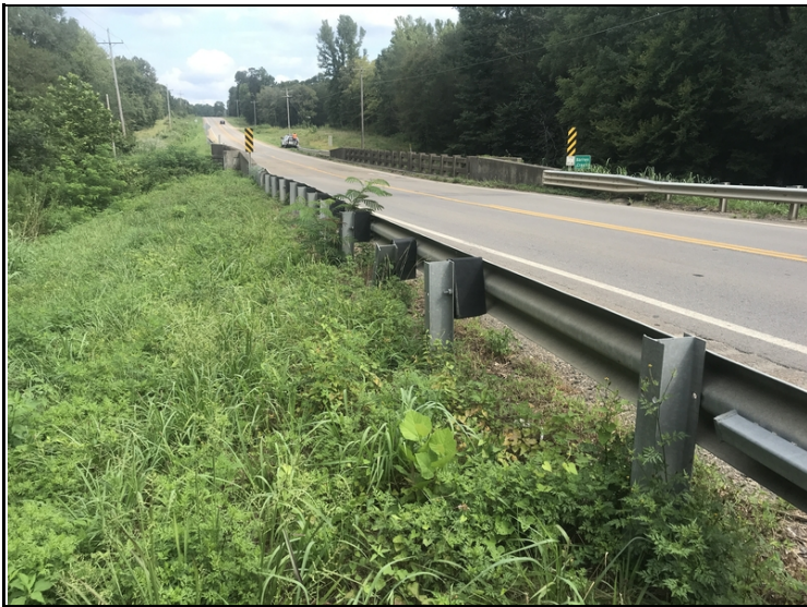
Southwest approach guardrail with minor collision damage that has damaged several rail posts.
