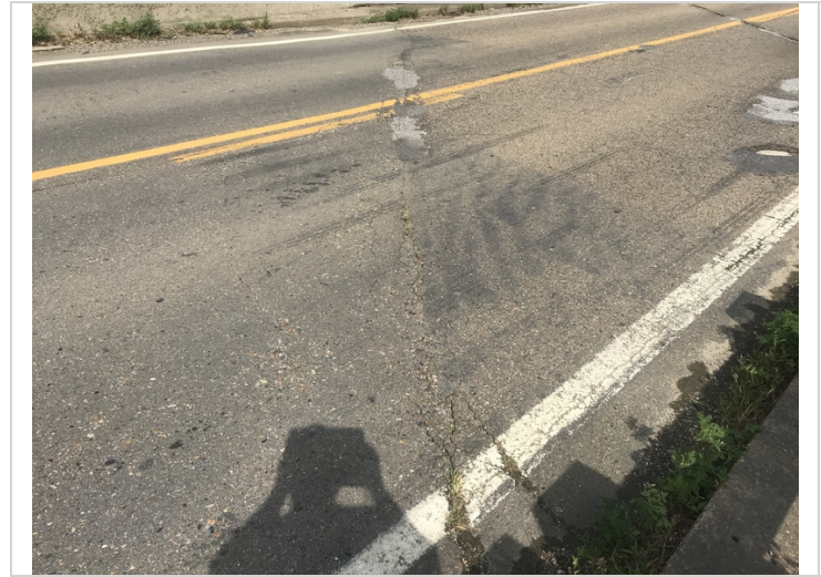
Abutment #1 wearing surface over the expansion joint.
