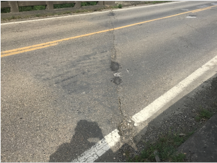
Abutment #2 wearing surface over the expansion joint.
