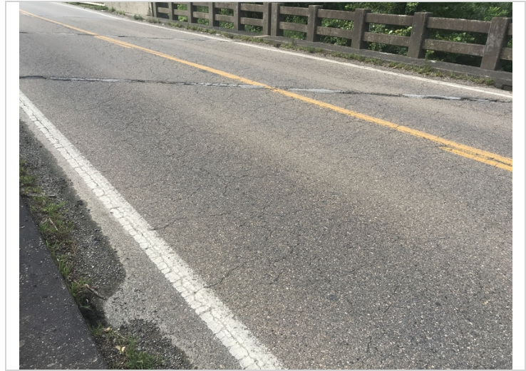
Typical driving surface cracking.
