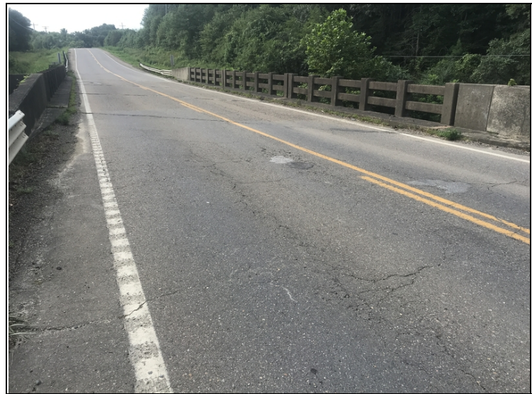
Potholes have been filled with asphalt.
