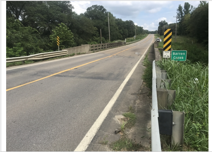
Abutment #1 with no apparent significant settlement of the approach roadway.
