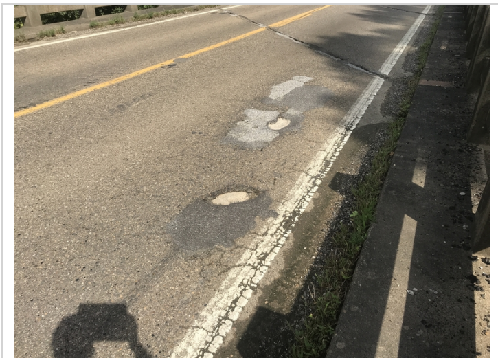
Span #1 asphalt deterioration with potholes in the northbound lane.
