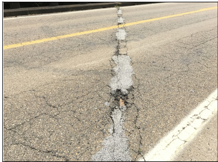
Potholes forming in driving surface over bent # 3 expansion joint.
