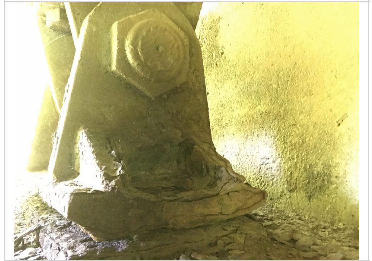
Abutment # 2, bearing # 1-Missing anchor bolt.
