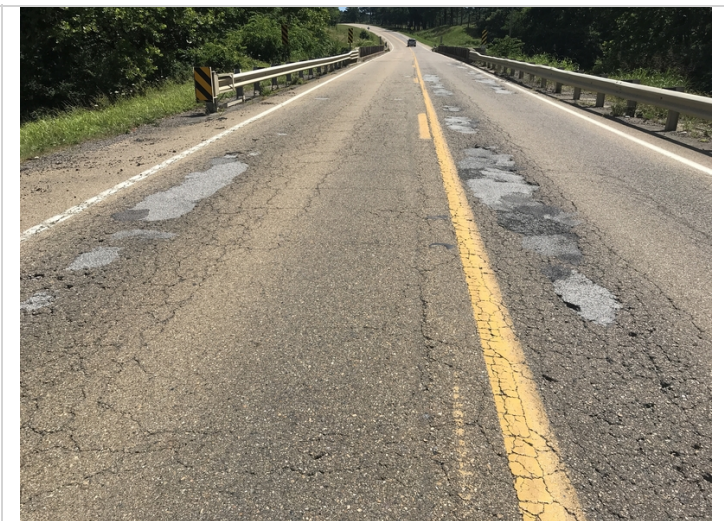
South approach roadway-Settlement in the wheel paths with potholes forming in the driving surface.
