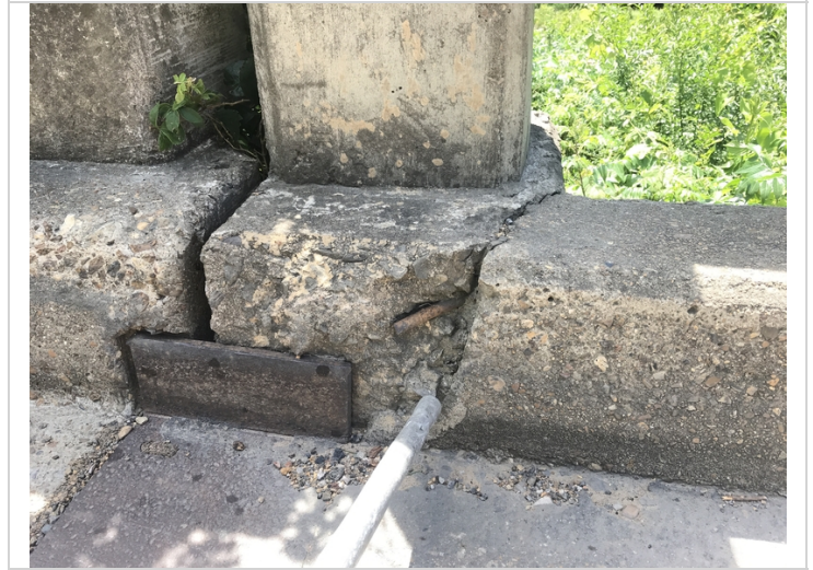
Span # 3, right side at abutment #2-Spalling with exposed reinforcing steel in curb.
