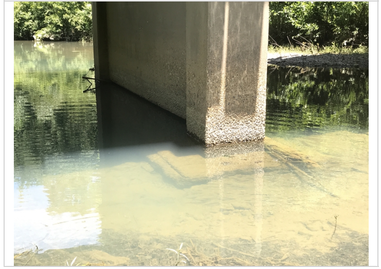
Bent # 2, column # 2 footing exposed.
