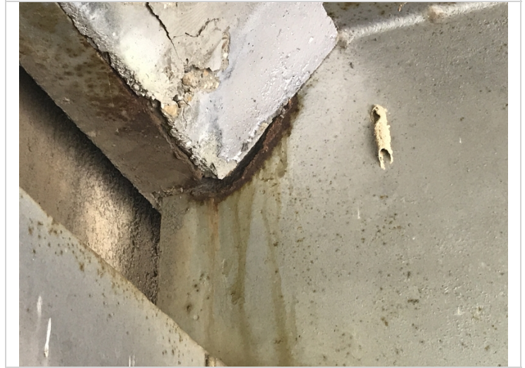
Span # 1, beam # 2 over abutment # 1 has corrosion with section loss adjacent to the expansion dam.
