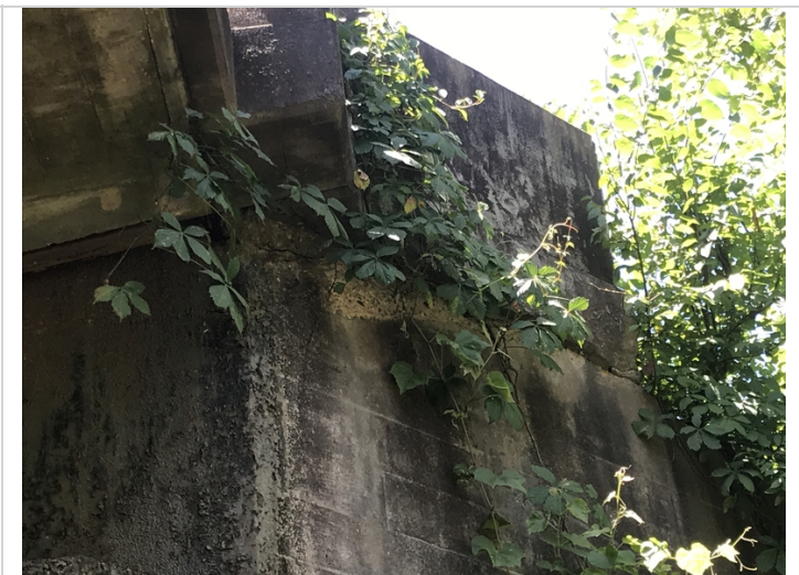
Abutment # 1-Spalling Under left end post.
