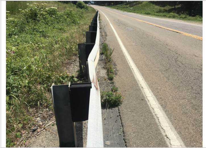
The Northwest approach railing has minor collision damage that has caused out of plane bending to the railing creating a "pocket" in the railing.
