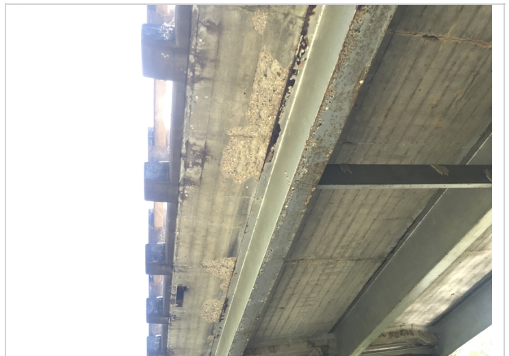
Span # 1, left side-Spalling in deck overhang adjacent to top flange.
