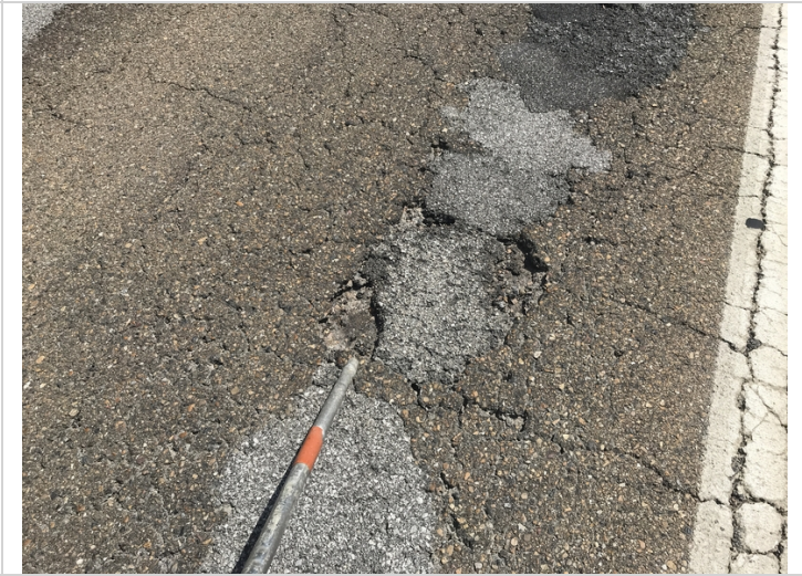
South approach roadway has settlement in the wheel paths with failing asphalt repairs and potholes in the driving surface.
