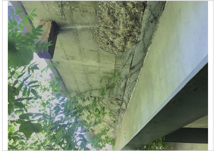
The right side of span # 3 deck overhang has large shallow spalls and delaminated areas.
