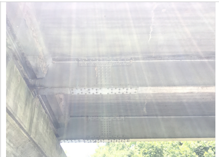
Span # 2-General view of splice plate connection # 1.
