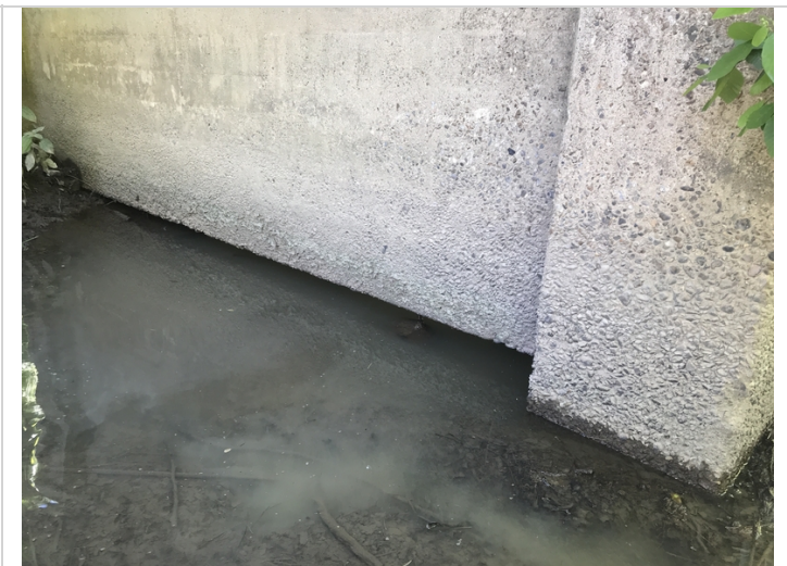
Bent # 3-Light abrasion to columns and web wall.
