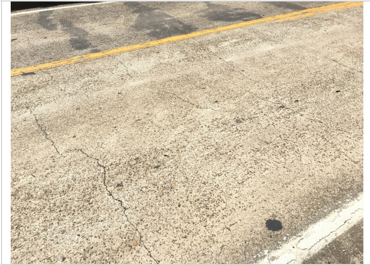
Span # 3, left lane-wide transverse cracking.
