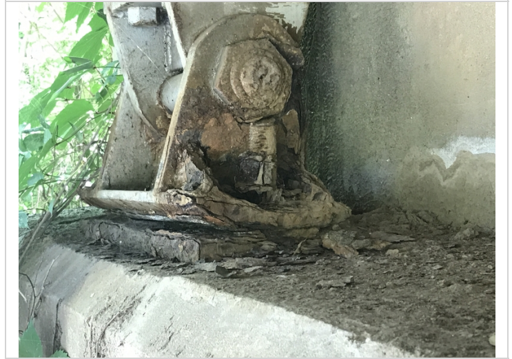
Span # 1, bearing # 3 over Abutment # 1-Corrosion with pack rust.
