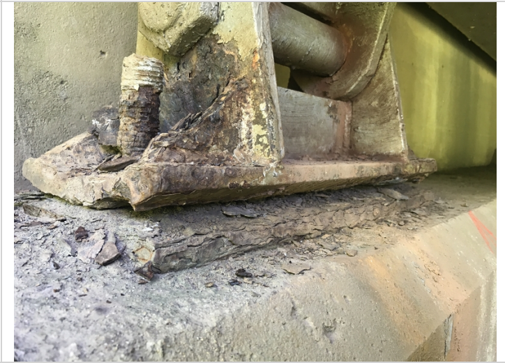
Abutment # 2, bearing # 1-Corrosion with heavy section loss.
