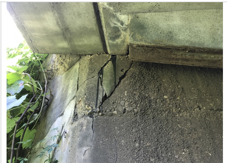
The upper portion of abutment # 2 backwall is fractured on the left and right sides at the wing wall junctures.
