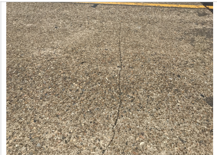
Span # 1, left lane-Moderate width transverse cracking.
