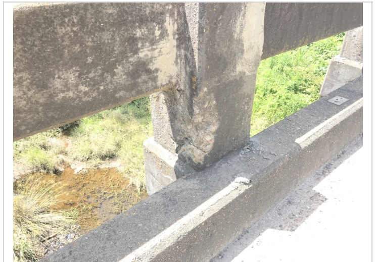
Span # 1, right bridge railing-Collision damage to post.
