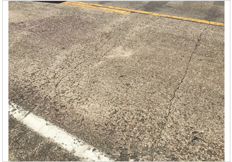
Span # 1, left lane-Transverse and mapcracking.
