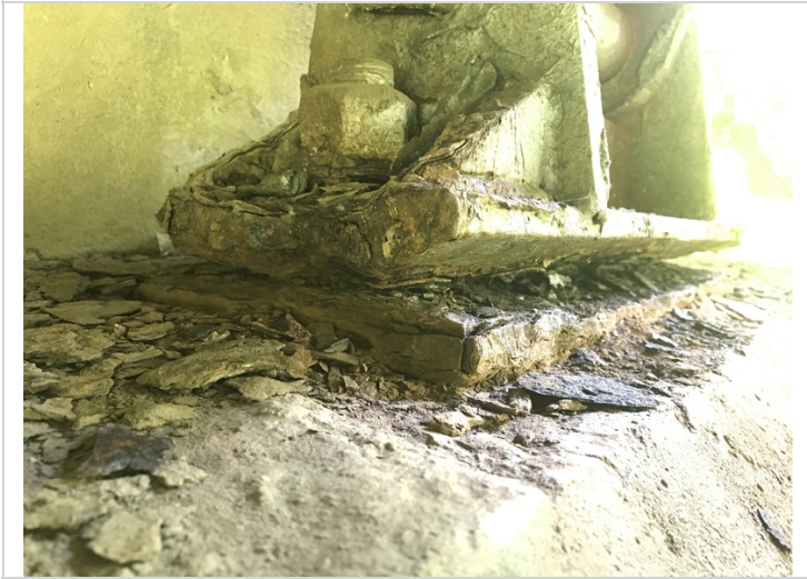
Span # 3, bearing # 3 over abutment # 2-Corrosion with heavy section loss.
