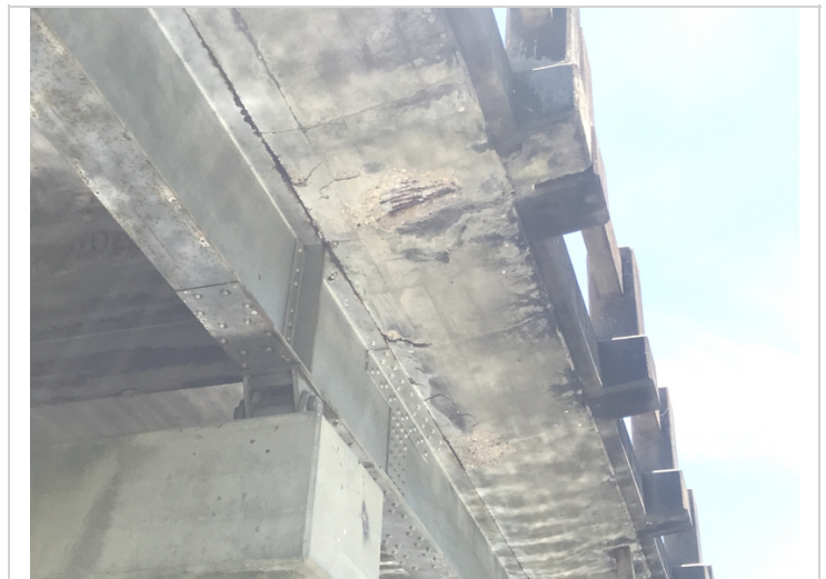
Spalling with exposed reinforcing steel in right undersurface at bent # 2.
