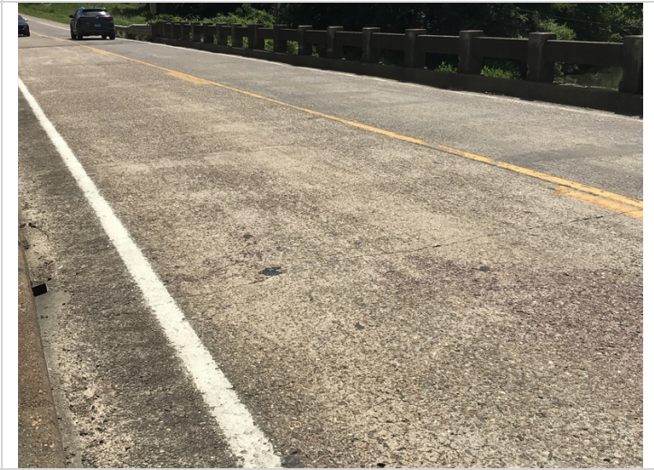
Wear to driving surface.
