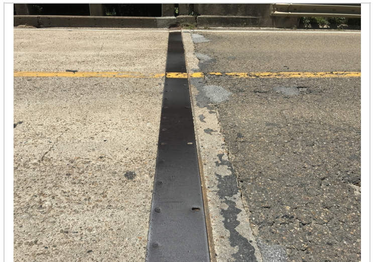
General view of abutment # 2 sliding plate assembly.
