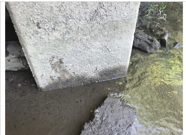
Abutment # 1, column # 1 footing-Light abrasion.
