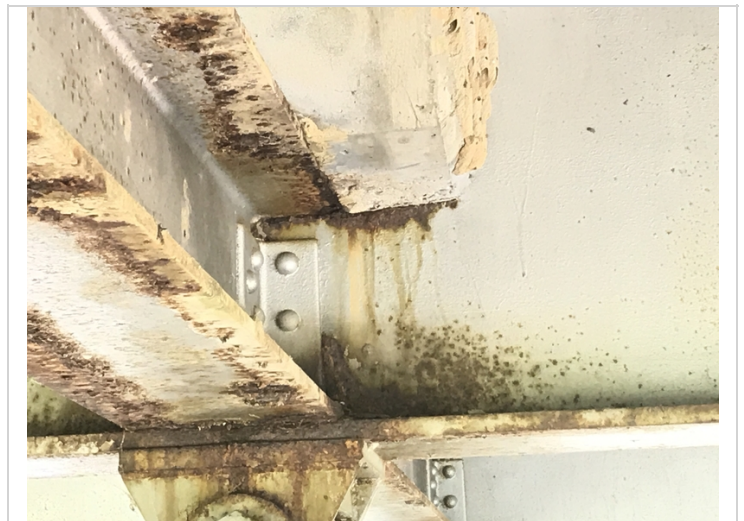
Span # 2, beam # 2 over bent # 2-Corrosion with flaking rust to web.
