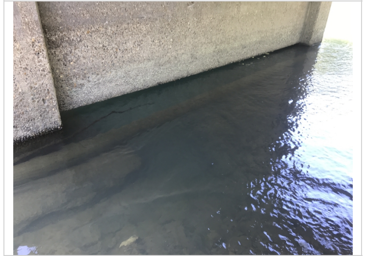
The channel has submerged drift at bent # 2 that is causing localized scour at base of columns.
