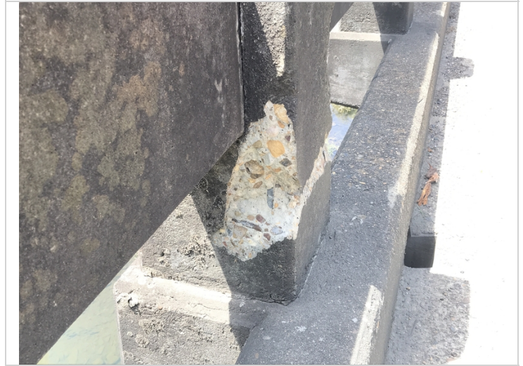
Span # 2, right bridge railing-Collision damage to post.
