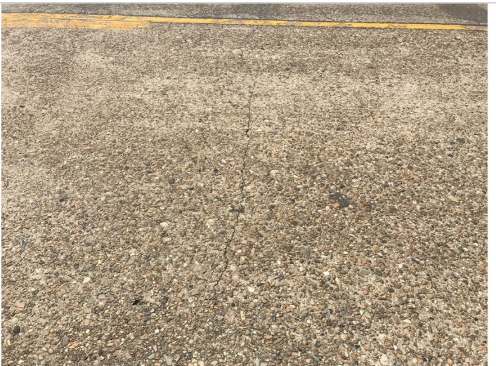
Span # 2, left lane-Transverse cracking.
