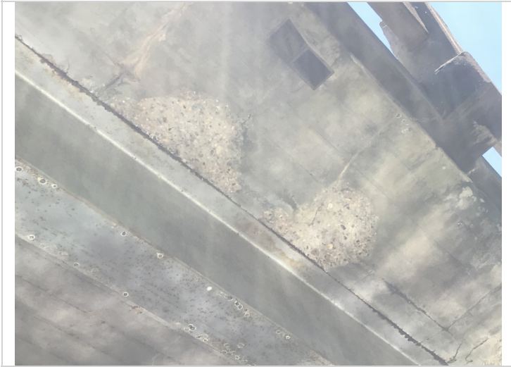
Span # 1, right side-Spalling adjacent to top flange.
