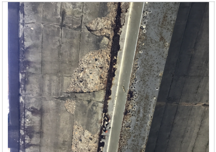
Span # 1, beam # 1-Corrosion with section loss to top flange.
