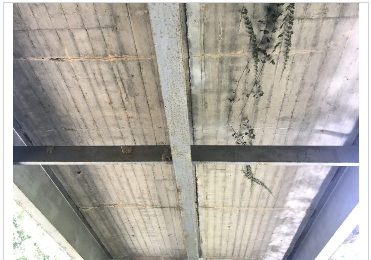
Span # 1 undersurface-Transverse cracking with leakage / staining.
