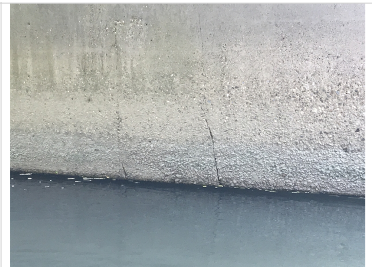
Bent # 2 web wall-Wide vertical cracking.
