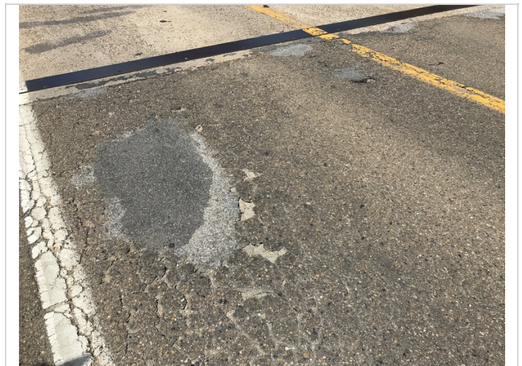
The right lane of the North approach roadway has failing asphalt repairs with potholes forming in the driving surface at the bridge end.
