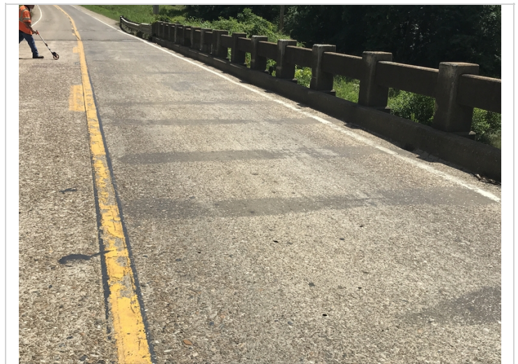
Cracks in right lane sealed.
