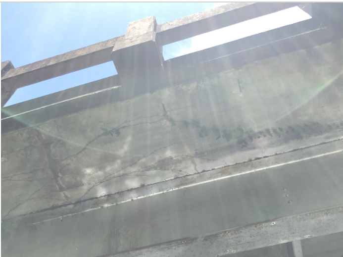
Span # 1, right side-Shallow spalling with exposed reinforcing steel.
