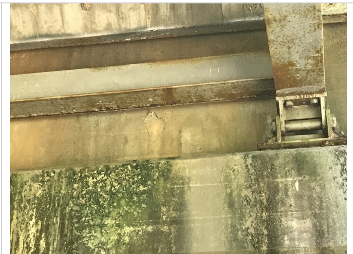
Abutment # 1 backwall-Delaminated area in bay # 1.
