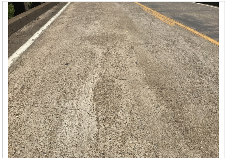
Span # 3, left lane-Moderate width transverse and random cracking.
