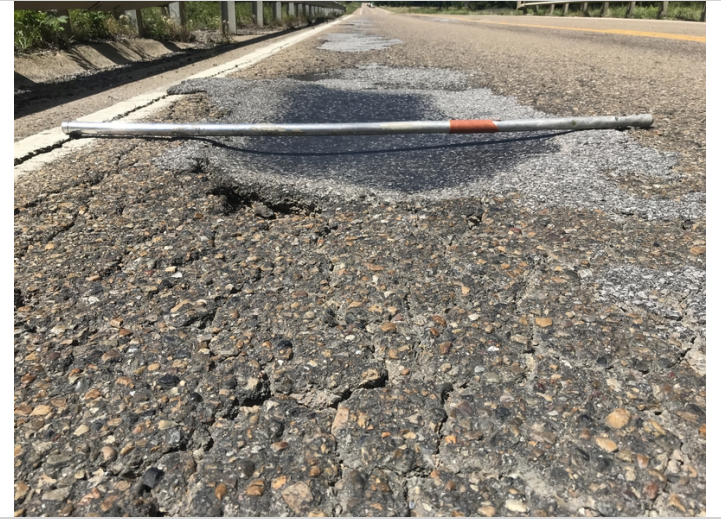
South approach roadway, right lane-Settlement with pothole in wheel path.
