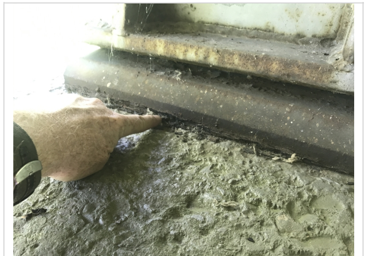
Bent # 3, bearing # 1 has corrosion with flaking rust and initial section loss to masonry plate.
