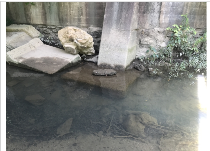
Abutment # 1, column # 1-Exposed footing.
