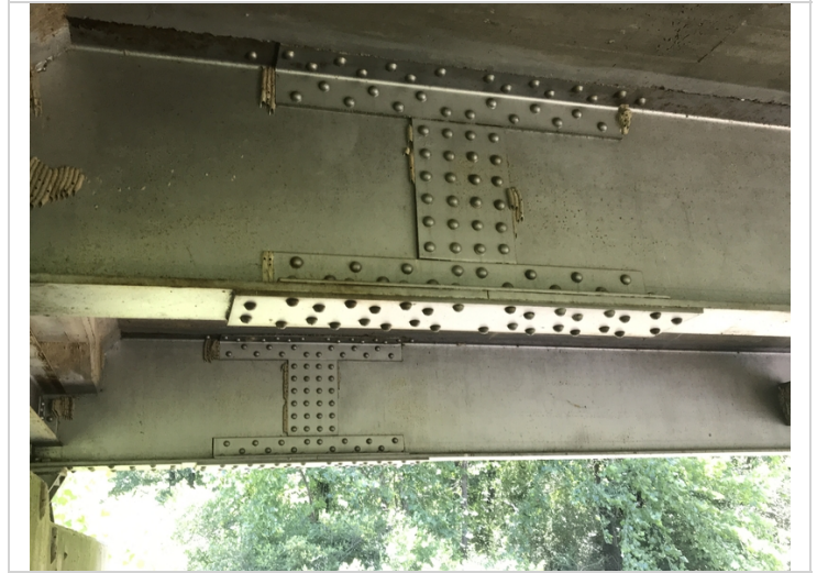
Span #2-General view of splice plate connection span 2.
