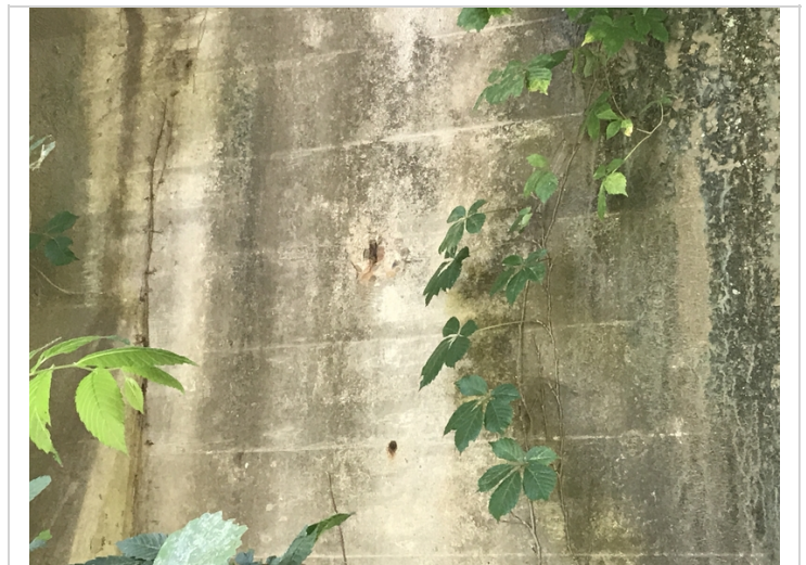
Abutment # 1 stem wall on right side-Baseball sized spall with exposed reinforcing steel.
