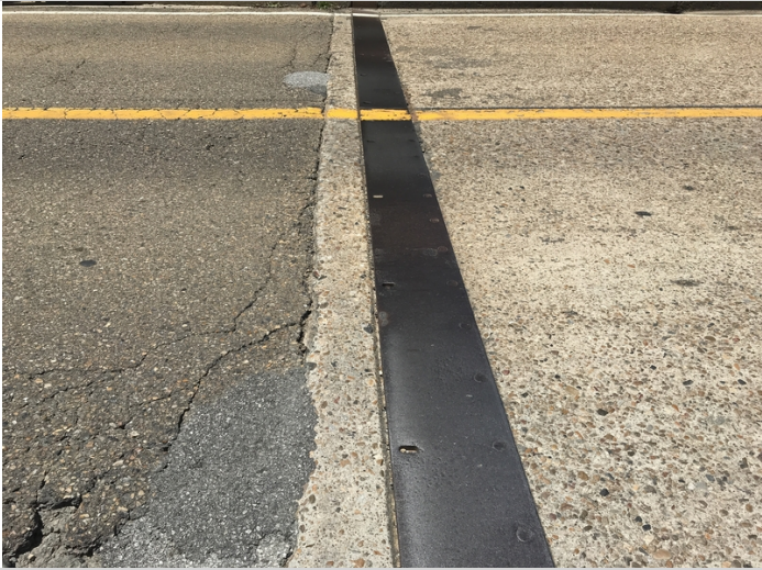
General view of abutment # 1 sliding plate assembly.
