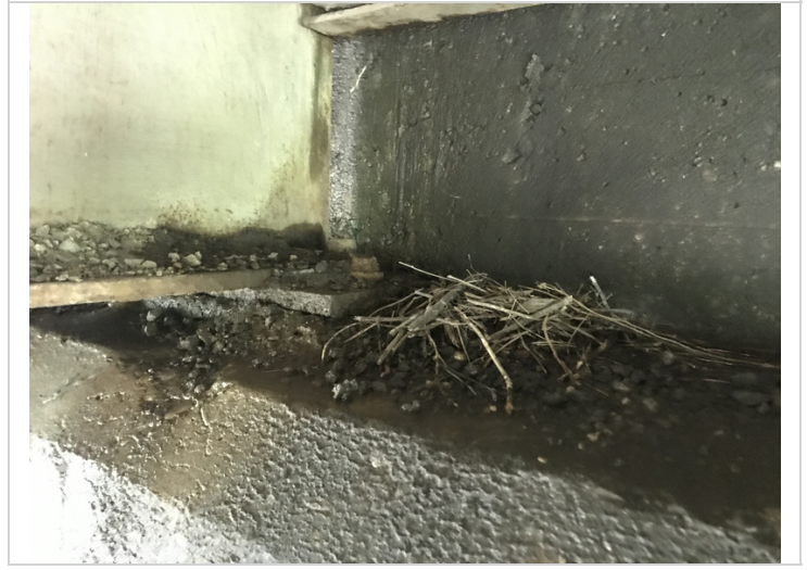
Abutment # 2-Dirt and debris accumulation.
