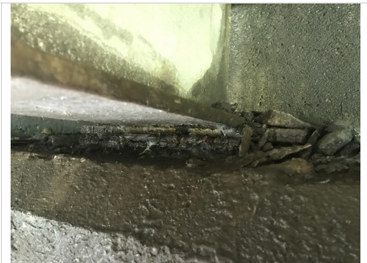
Span # 3, bearing # 4 at abutment # 2-Heavy corrosion.
