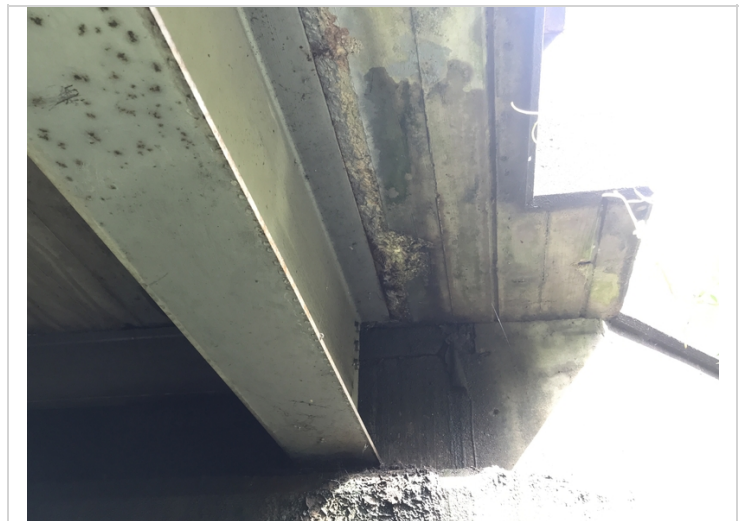
Span # 3, right side-Shallow spalling along top flange.
