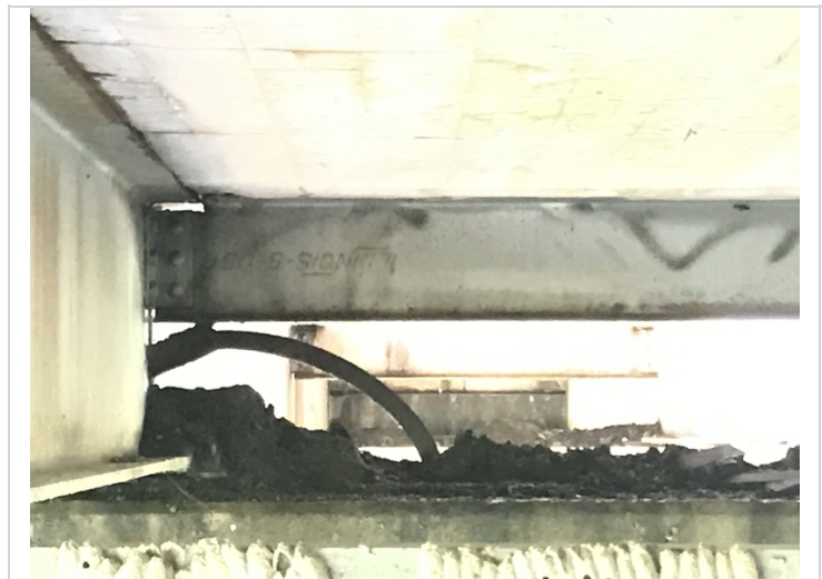
Bent # 3-Asphalt and dirt accumulation on cap.
