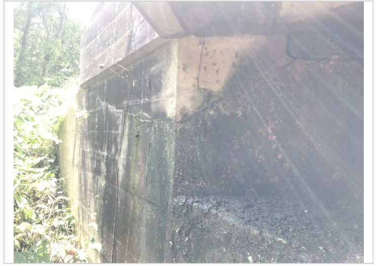
Abutment # 1, right side-Horizontal cracking.
