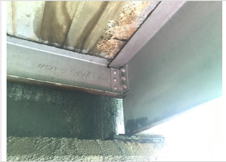
Span # 3, bay # 4 at abutment # 2-Spalling with exposed reinforcing steel in deck underside.
