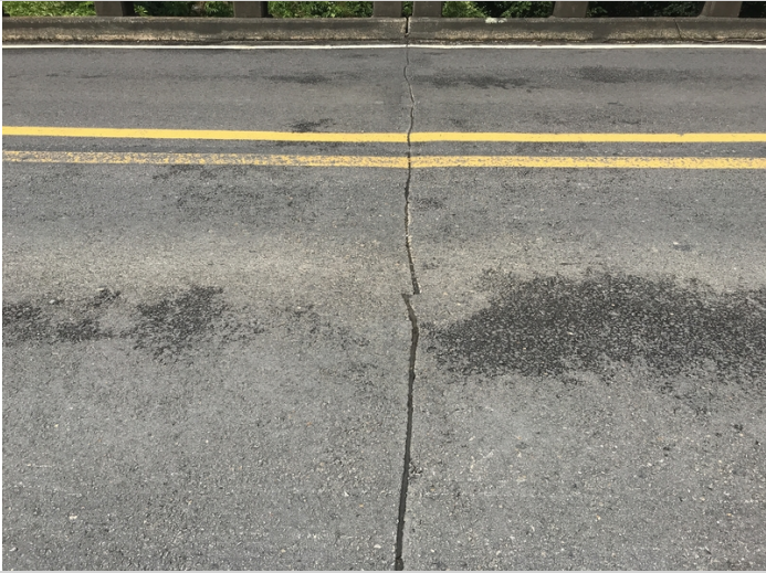
Bent # 2 expansion joint.
