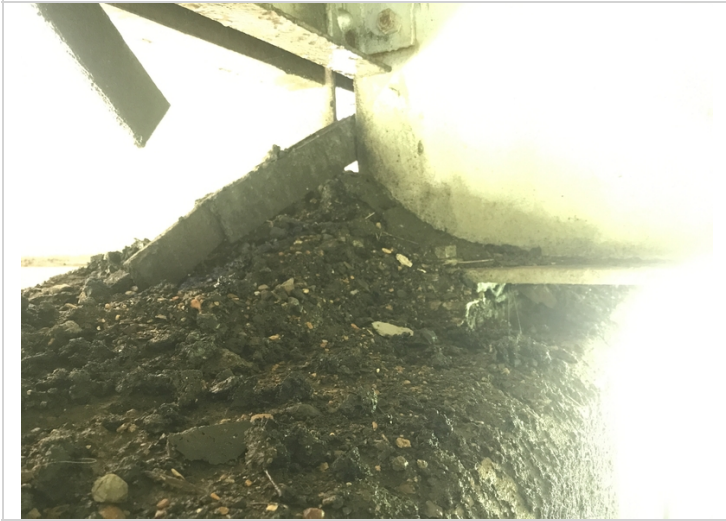
Bent # 3-Dirt and accumulation.
