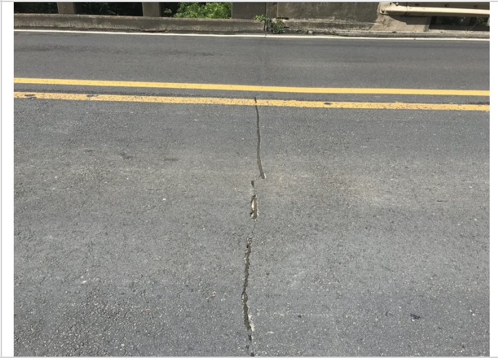
Expansion joint at abutment # 2.
