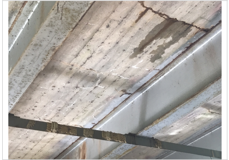
Span # 2, bay # 3-Mapcracking with efflorescence in deck underside.
