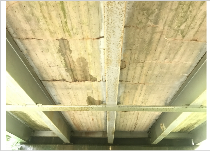
General view of span # 3 undersurface with transverse cracking and staining.
