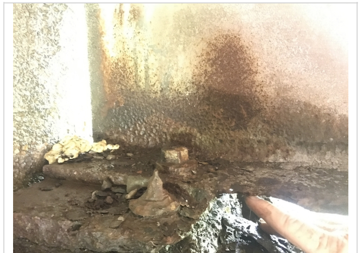
Span # 1, beam # 1 has a 3" area of knife edged section loss to bottom flange over abutment # 1.
