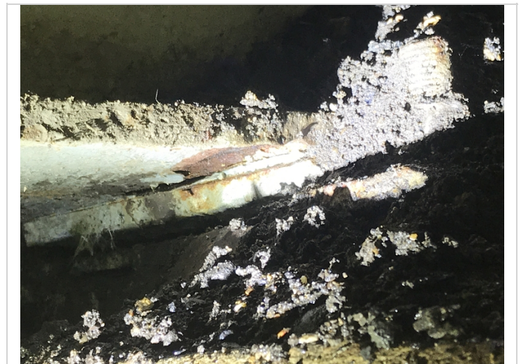
Span # 3, beam # 4 over bent # 3 has approximately 50% section loss to bottom flange.
