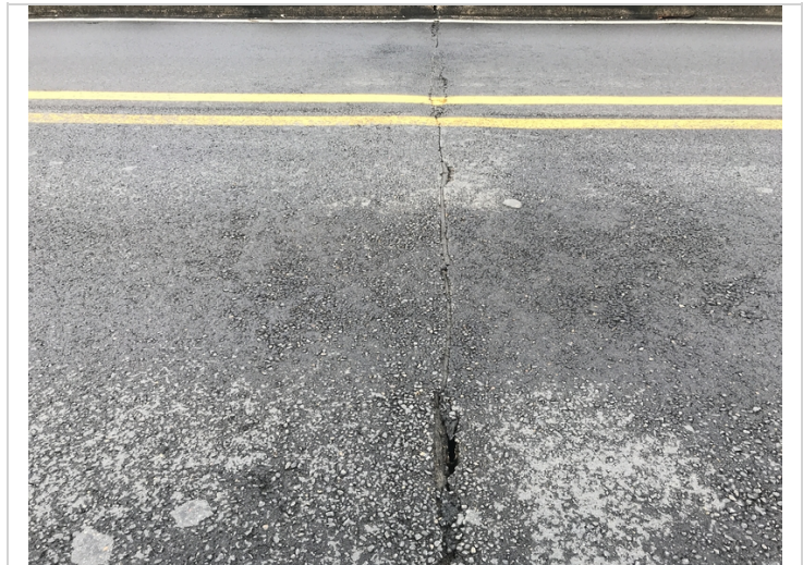
Asphalt in expansion joints.
