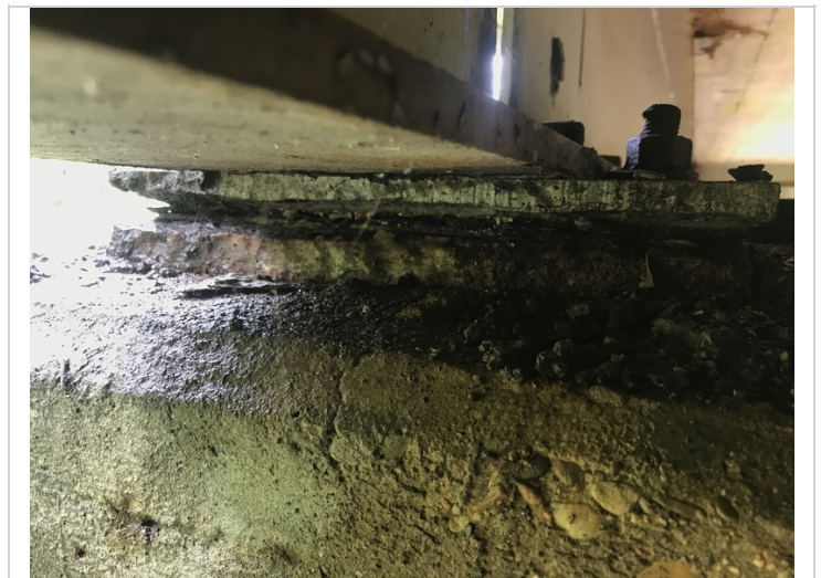
Span # 3, bearing # 5 over bent # 3-Corrosion.
