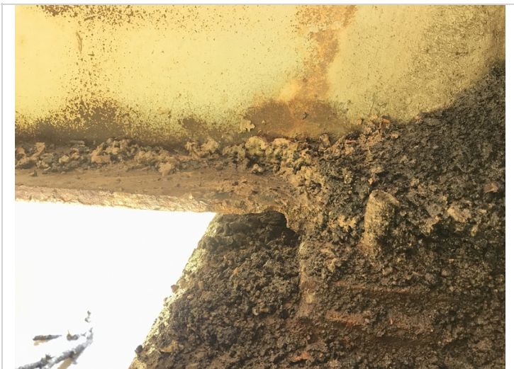
Span # 2, beam # 3 over bent # 3 has section loss to bottom flange in an area approximately 1' long with 3/16" remaining section in the affected area.
