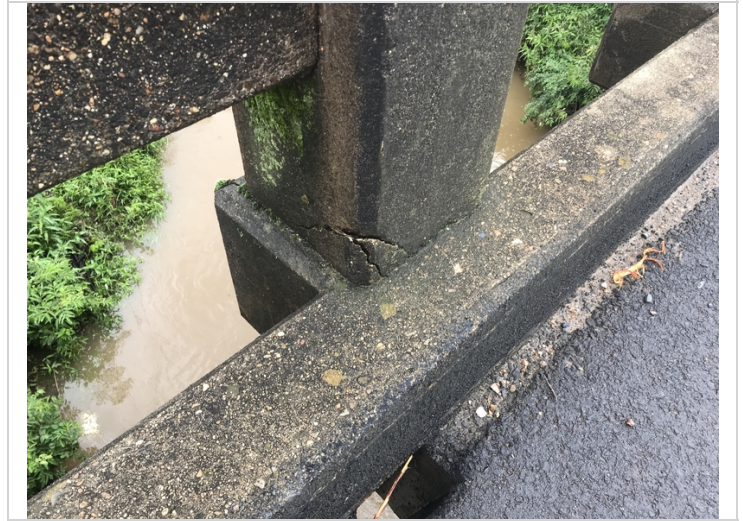
Span # 2, post #1 on right side has a softball sized spalled area at base of post.
