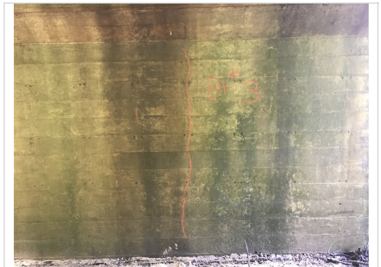
Bent # 3 web wall has a narrow vertical crack near centerline.
