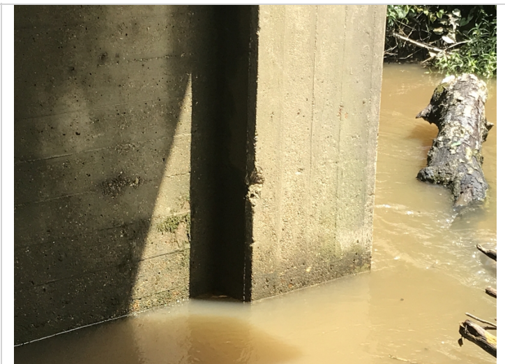
The backside of column # 2 of bent # 2 has a shallow softball sized spall with no exposed reinforcing steel near water elevation.
