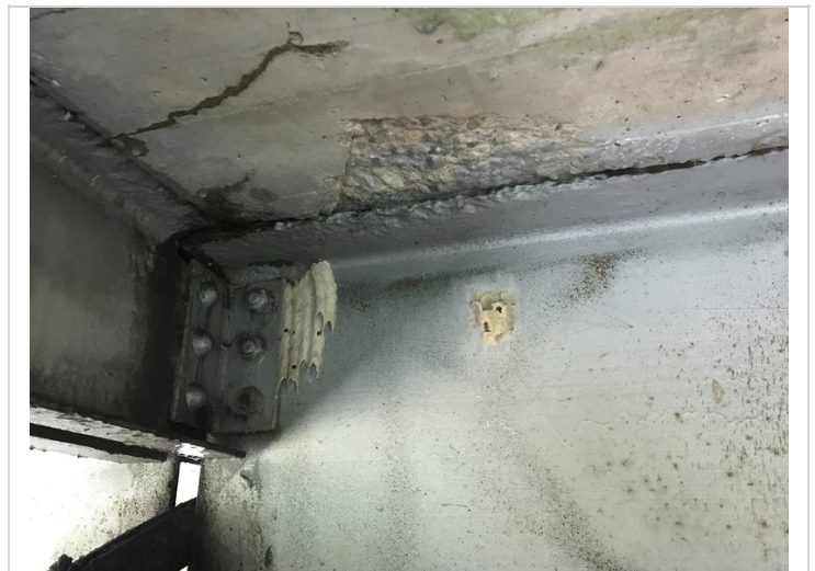
Span # 3, beam # 4-Old section loss to top flange over bent # 3.
