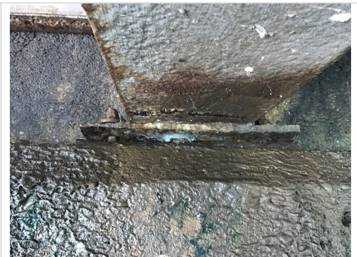
Span # 1, beam # 2 at abutment # 1-Corrosion with flaking rust.
