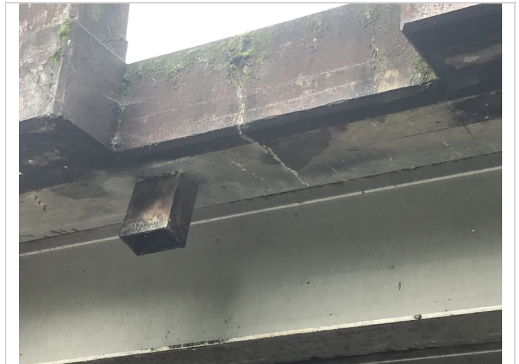
Transverse cracking with efflorescence in deck overhangs.
