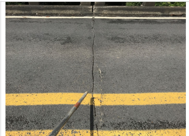
Bent # 3 expansion joint.
