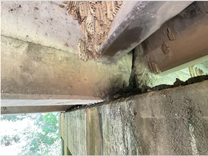
Span #1 Girder #3 Bent #2 spalling with exposed reinforcing steel.
