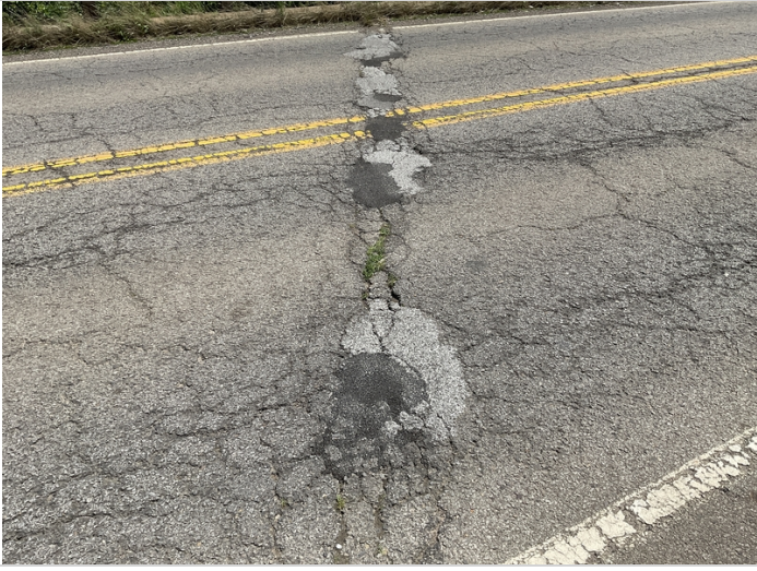
Bent #3 asphalt deterioration over the deck joint.
