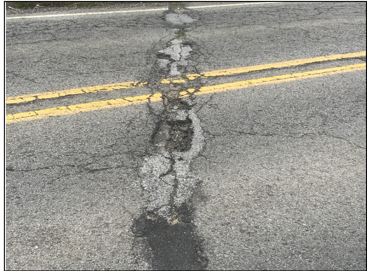
Potholes in asphalt over intermediate bents.
