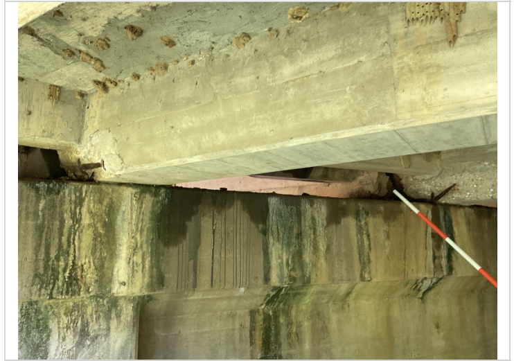
Bent # 2 Span # 2 Girder # 3 & 4 spalling with exposed reinforcing steel.
