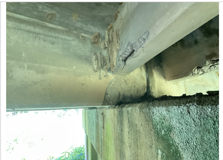
Bent #3 Girder #3 spalling with exposed reinforcing steel.
