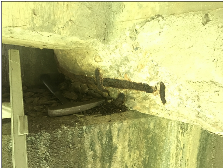
Span 2, girder 4 at bent 2-Spall with exposed reinforcing steel.
