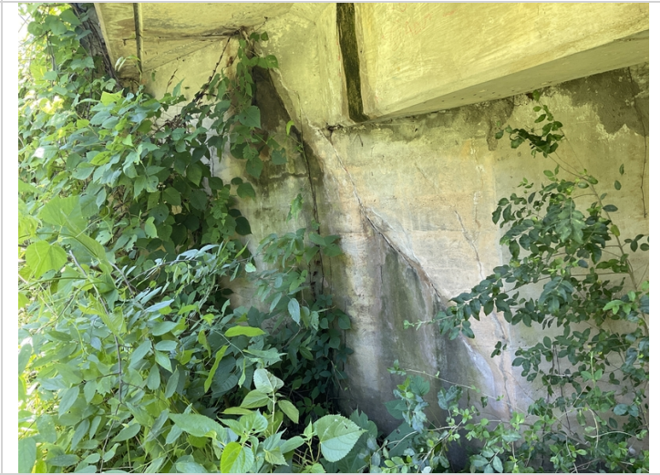
Abutment #2 Lt diagonal cracking in the wing wall.
