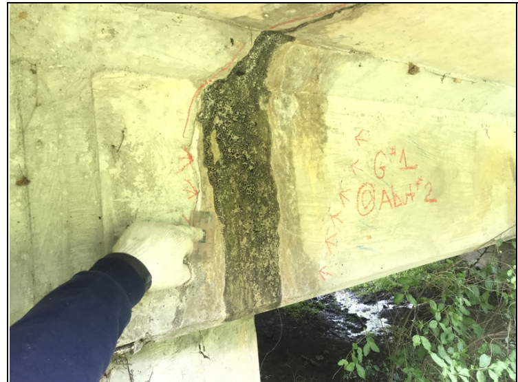
Span 3, girder 1 at abutment 2-Hairline shear type crack.
