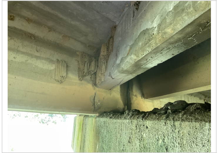
Bent # 3 Girder #2 spalling with exposed reinforcing steel.
