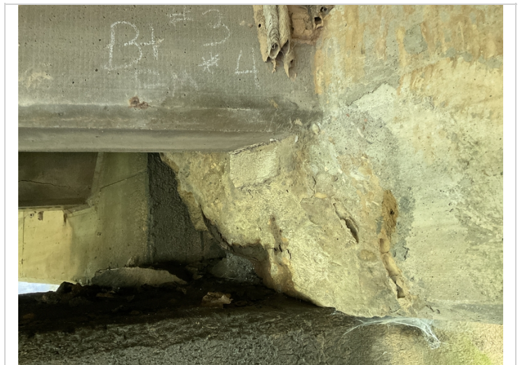
Bent #3 girder #4 spalling with exposed reinforcing steel.
