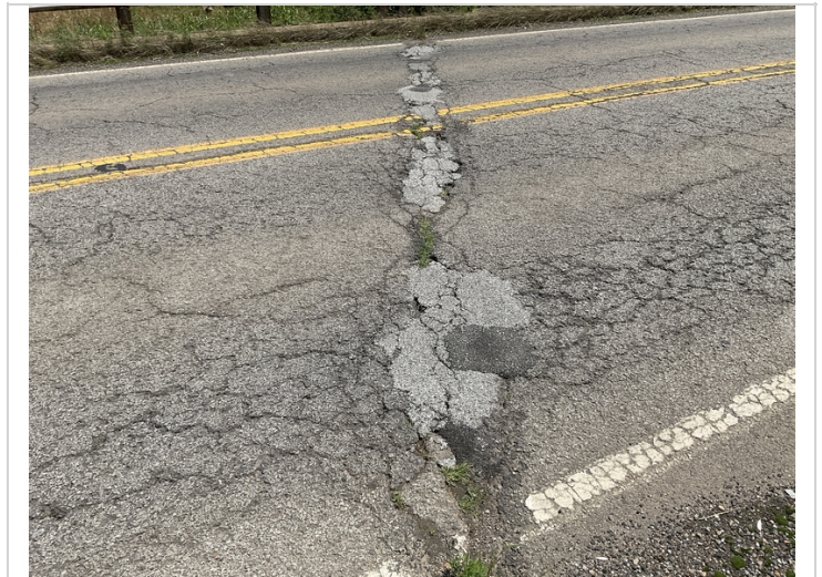
Bent #2 asphalt deterioration over the deck joint.
