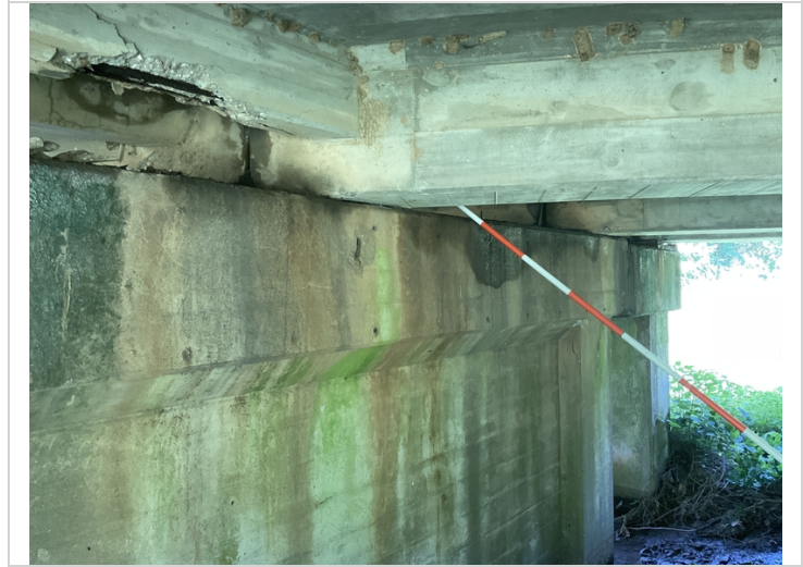
Bent #3 aheadface spalling with exposed reinforcing steel.
