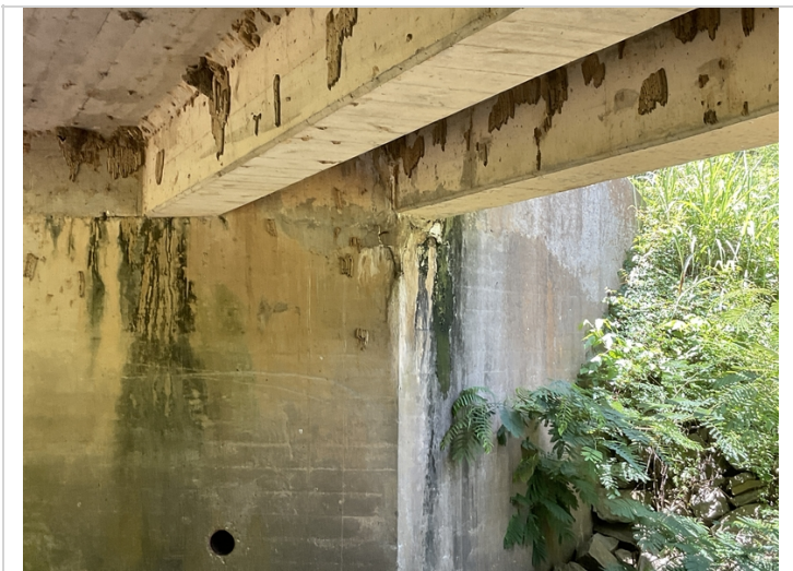
Abutment #1 Lt failing patch under girder #1.
