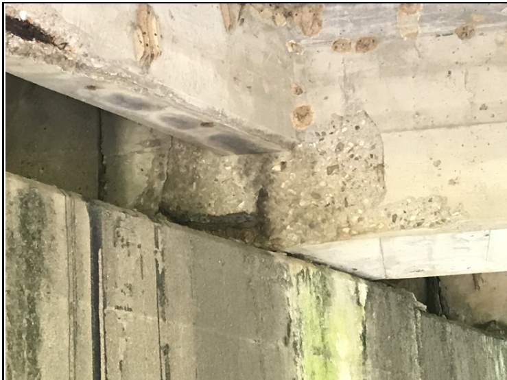
Span 1, girder 4-Spalling with exposed primary reinforcing steel over bent 2.
