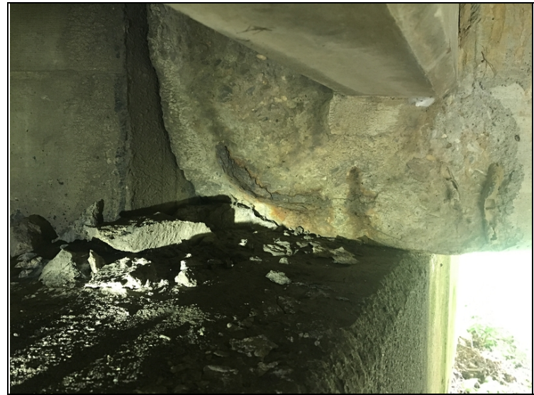
Span 2, girder 4 at bent 3-Spall with exposed reinforcing steel.
