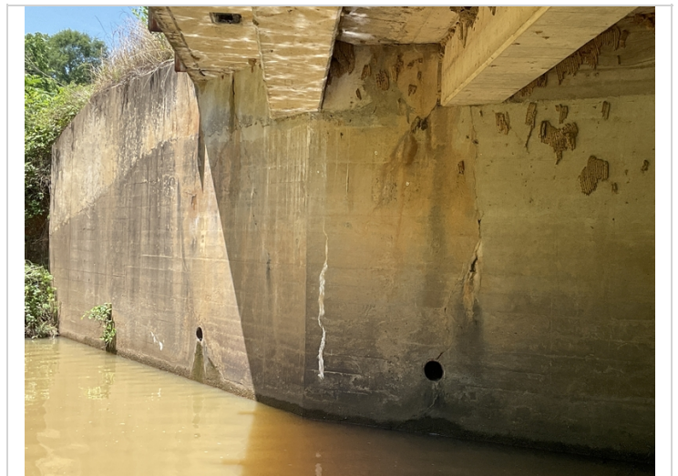
Abutment #1 Rt vertical and diagonal cracks with efflorescence buildup.
