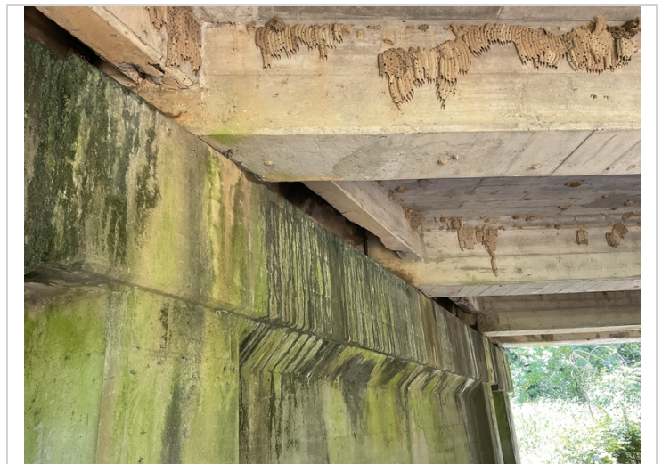
Span #1 Bent #2 spalling with exposed reinforcing steel.
