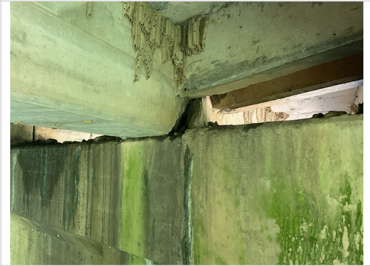
Bent #2 Span #2 Girder #2 spalling with exposed reinforcing steel.
