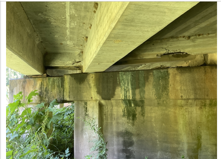
Span #3 bay # 3 & 4 spalling with exposed reinforcing steel in the expansion dam.
