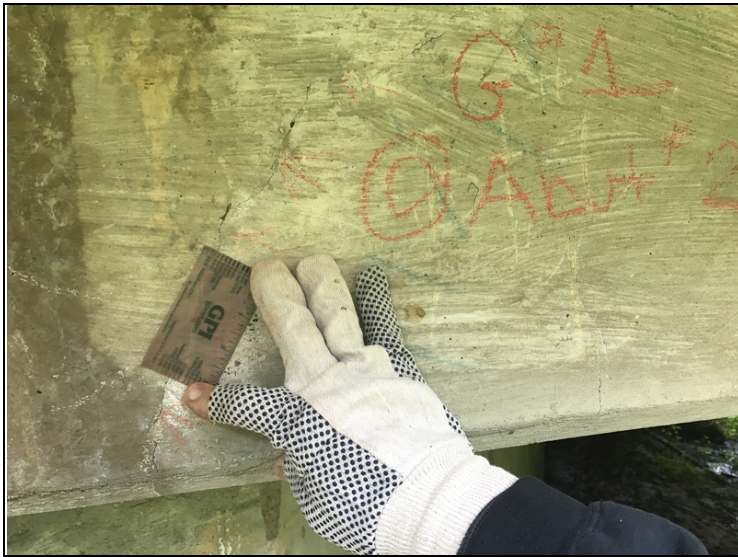
Girder 1 at abutment 2-Shear type crack.
