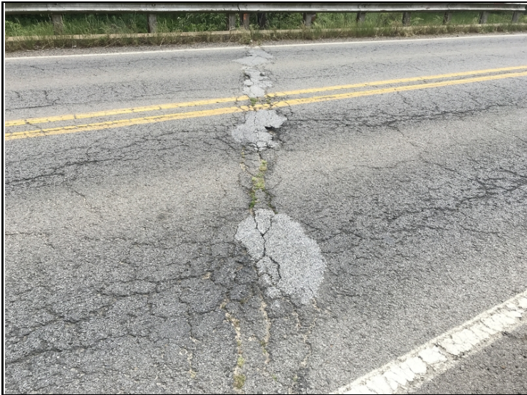
Bent 3-Asphalt breaking apart.
