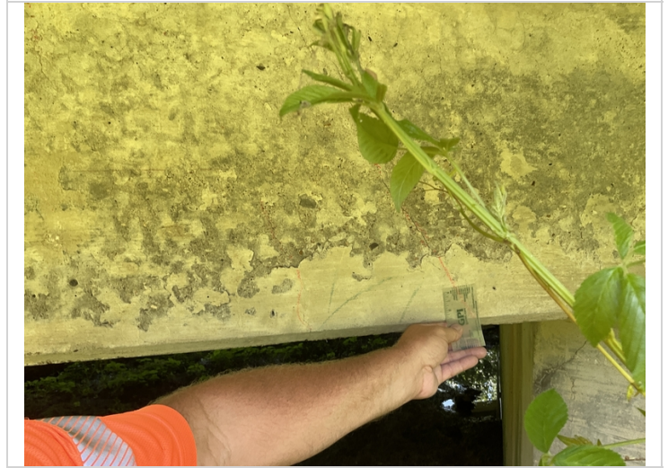
Span #3 Girder #5 exterior shear type crack.
