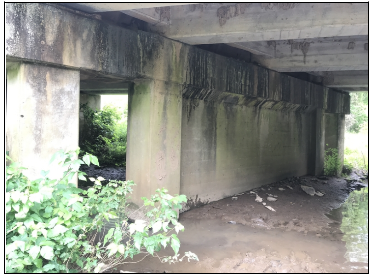
Expansion joints leak water on the substructure and on the ends of the concrete deck girders.
