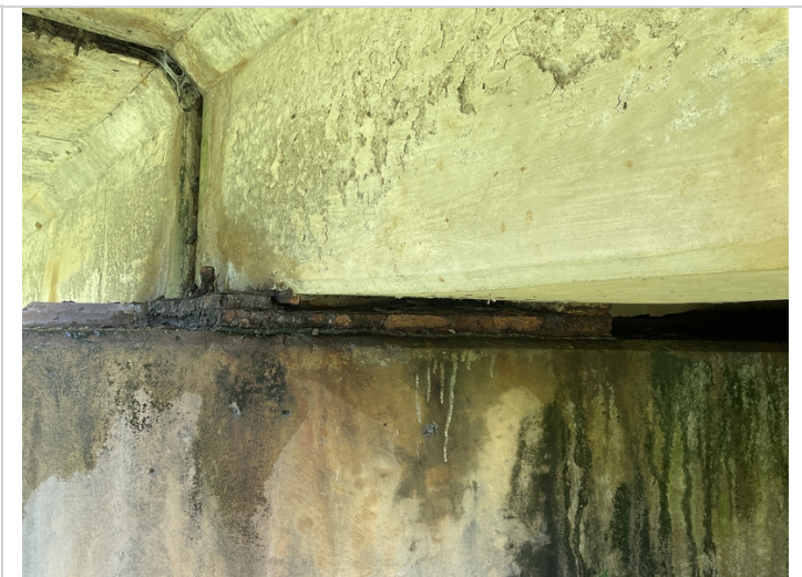
Bent #3 Span #3 Girder #5 bearing with active corrosion and pack rust.
