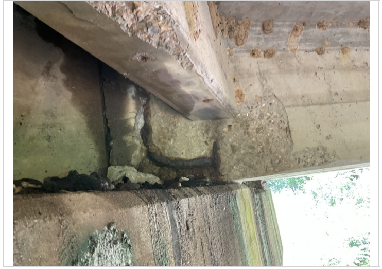
Span #1 Girder #4 Bent #2 spalling with exposed reinforcing steel.
