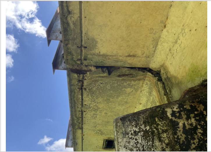
Span #2 Lt spalling with exposed reinforcing steel
