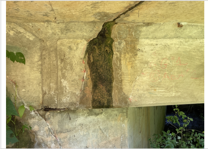
Span #3 Girder #1 Abutment #2 shear type cracks in the girder.
