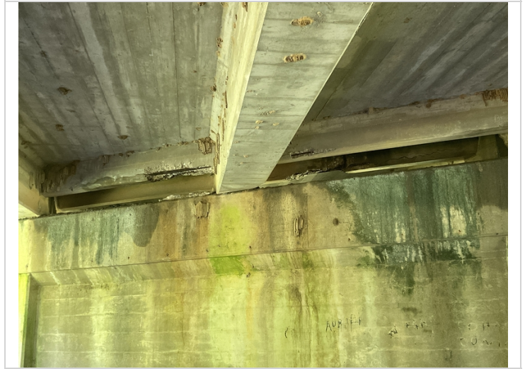
Span #2 bay # 2 & 3 spalling with exposed reinforcing steel in the expansion dam.
