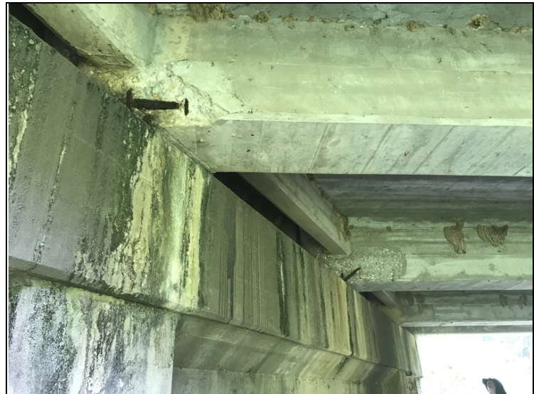
Span 2, girders 3 and 4-Spalling with exposed reinforcing steel.
