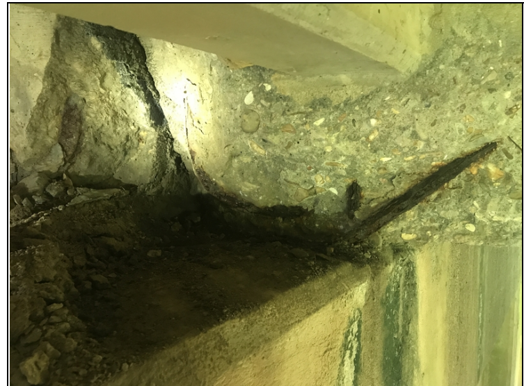
Spalling with exposed reinforcing steel to end of girder # 3 of spans 1 and 2 over bent 2.
