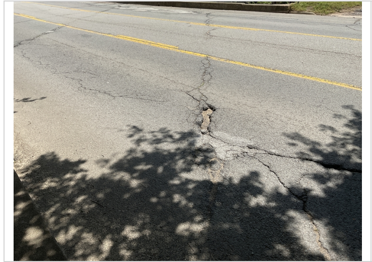
Wearing surface with potholes forming over the abutments.
