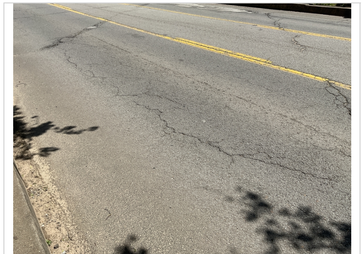
Typical cracking on the wearing surface.
