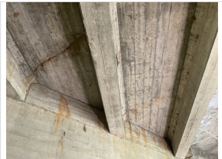
Transverse cracking with rust stains.
