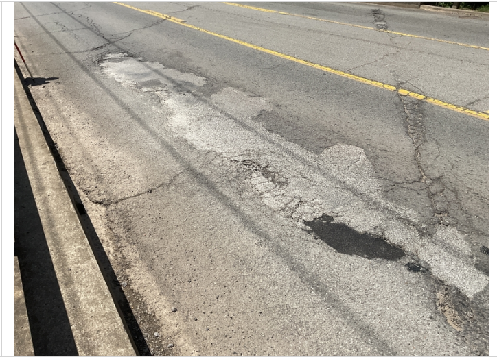
Asphalt wearing surface patched areas.
