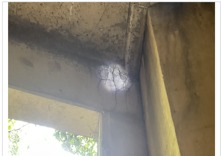
Abutment #1 Girder #7 with exposed reinforcing steel in the side of the girder.
