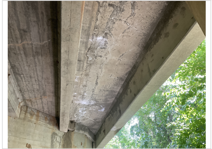
Bay #6 map cracking with efflorescence buildup.
