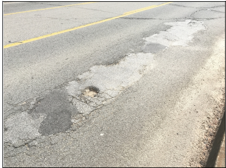
The asphalt patches in the right lane are failing in locations with potholes forming.
