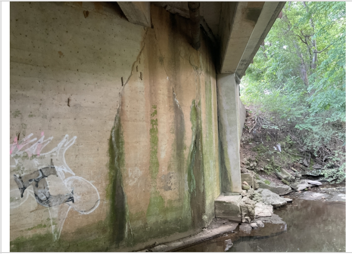
Abutment #1 Lt cracking at the wing wall juncture.
