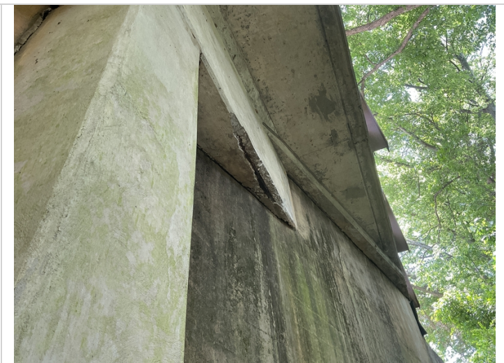
Abutment #1 girder #1 spalling with exposed reinforcing steel.
