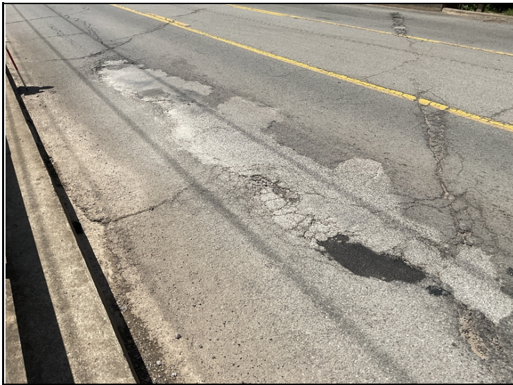
Asphalt wearing surface patched areas.
