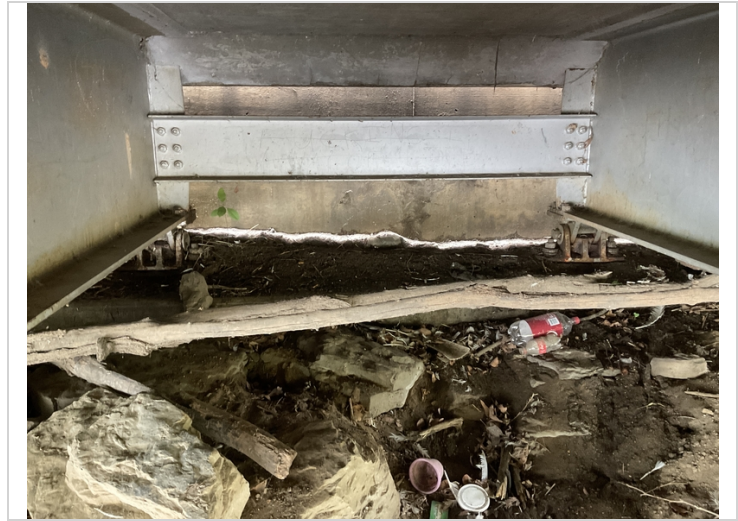
Abutment #1 debris accumulation.
