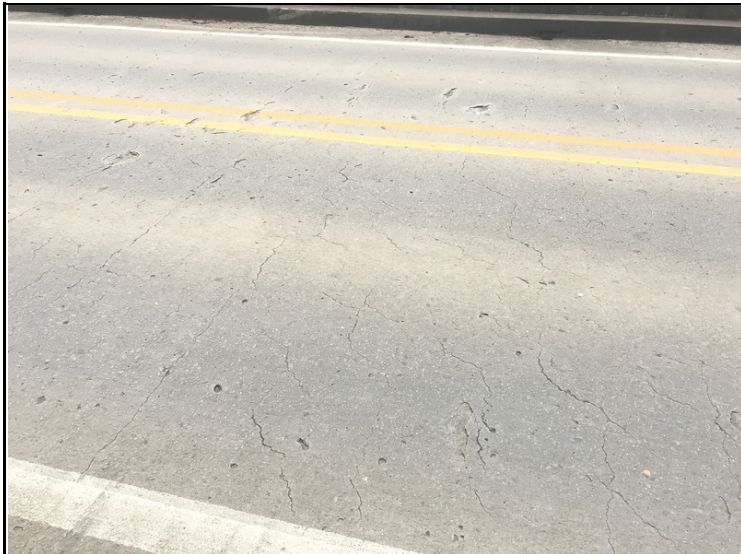
Span 2-Wide cracking with areas of spalling.
