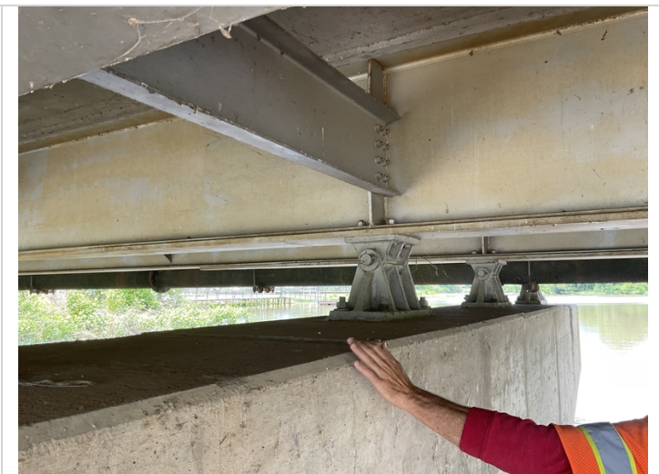
Bent #2 typical bearings
