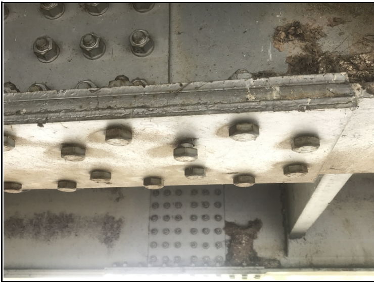
Span 2, beam 4 at splice connection 2-Loose bolts in bottom flange splice.
