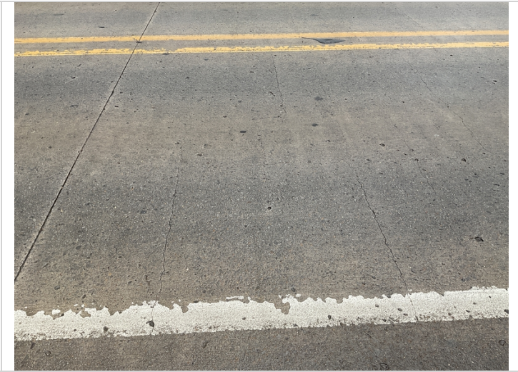
Sealable deck cracking.
