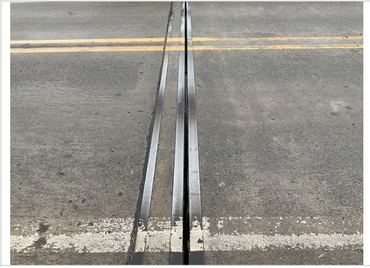
Abutment #2 missing joint seal.
