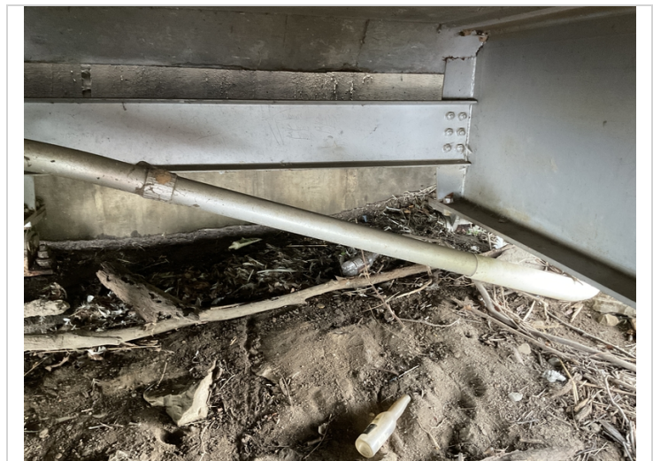
Abutment #1 Bearing #1 debris accumulation.
