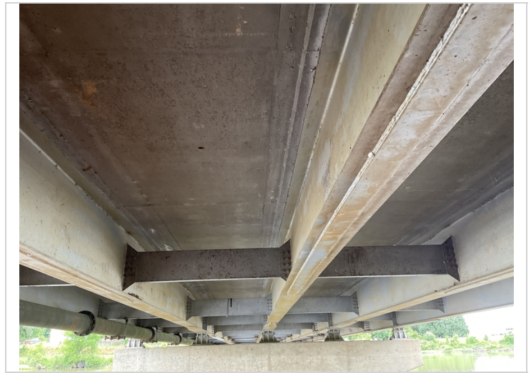
Span #1 typical undersurface of the deck.
