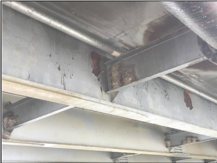
Span 2, beam 2-Flaking paint.
