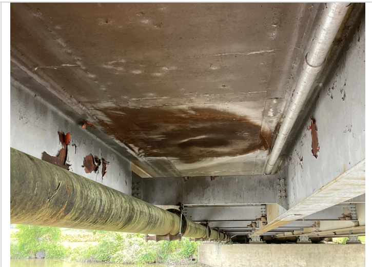
Span #2 bay #1 concrete discoloration.
