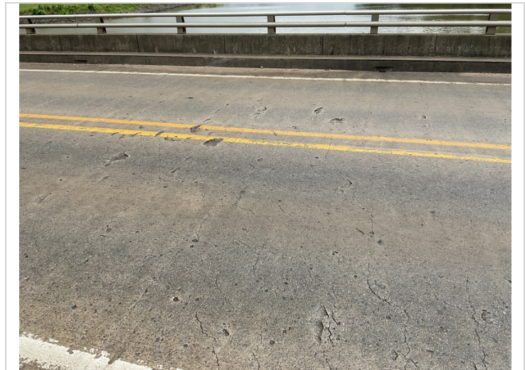
Span #2 concrete cracking and delaminating areas.
