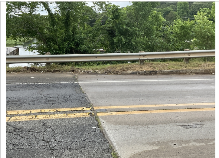
Approach drains filled with dirt.
