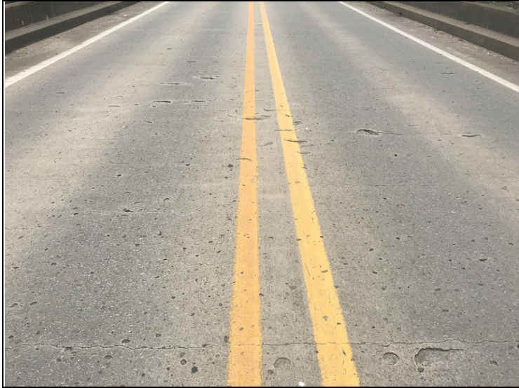
Span 2-Spalling / delaminated areas.
