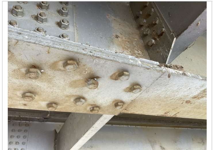
Span #2 beam #4 splice #2 loose bolt.
