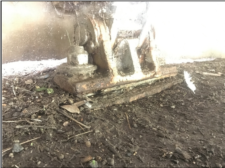
Bearing 3 over abutment 2-Corrosion with pack rust between rocker and masonry plate.
