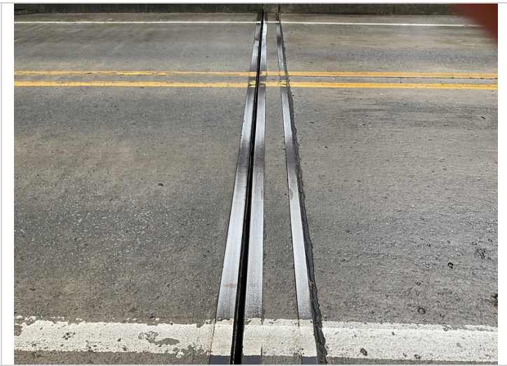
Abutment #1 joint seal missing.
