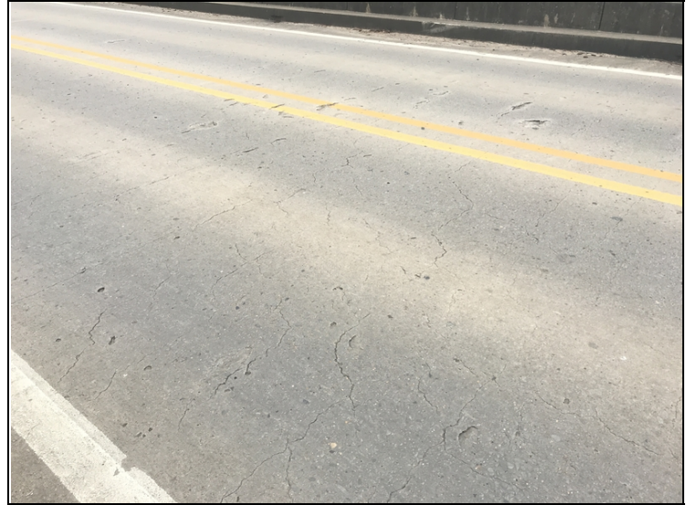
Span 2-Wide cracking.
