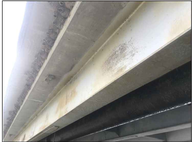
Paint system failing.
