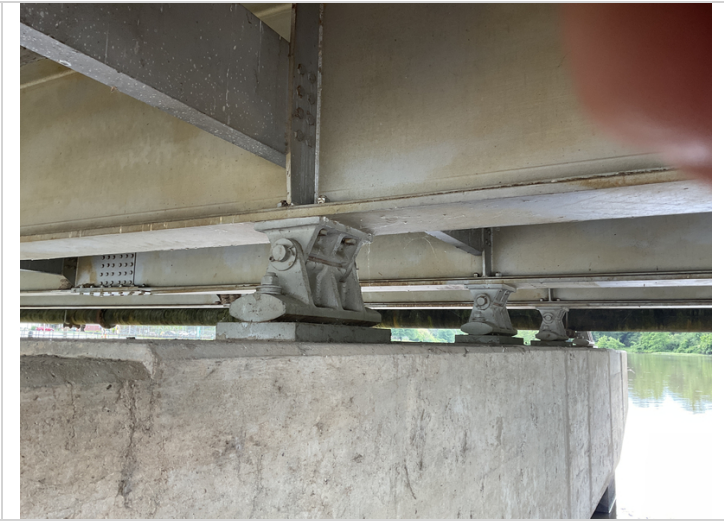
Bent #3 typical bearings.
