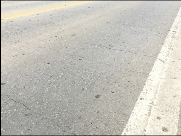
Transverse deck cracking.
