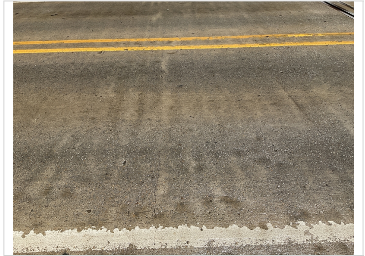
Sealable deck cracks.
