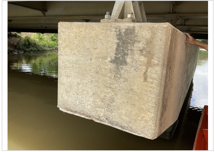
Bent #2 Rt end of the cap delamination.
