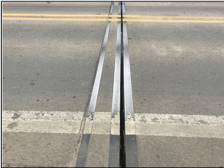
Abutment # 2 joint seal missing.
