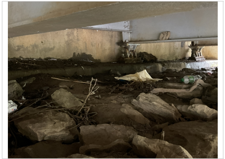
Abutment #2 bearings with active corrosion and pack rust.
