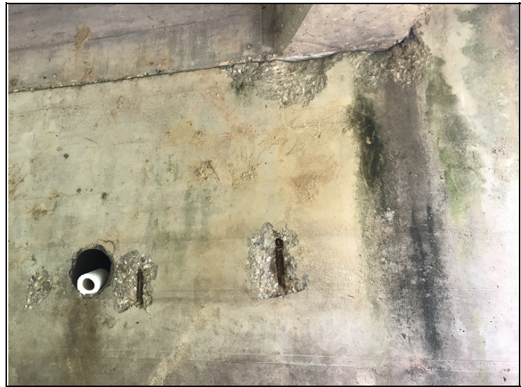
Abutment # 2 stem wall has two 10" spalls with exposed reinforcing steel on the right side.
