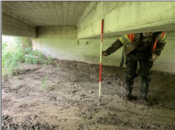
Span #2 channel restricted by stream bed material accumulation.
