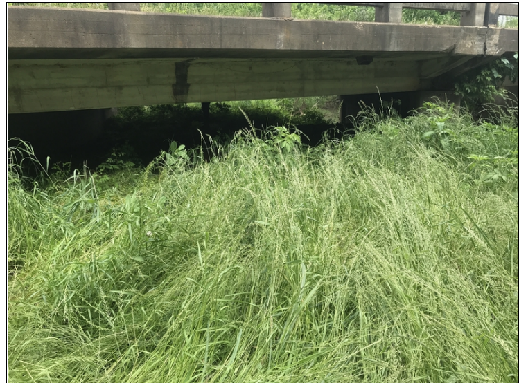
Channel has streambed accumulation under Span # 1 reducing the channel freeboard to less than 4' at this inspection.
