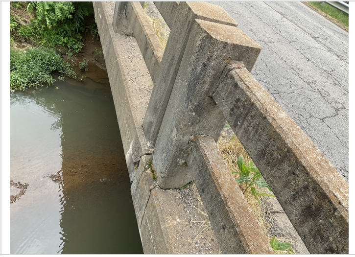
Span #1, Bent #2 Lt fractured rail and post.
