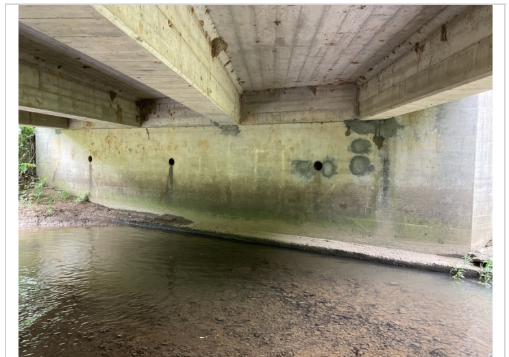
Abutment #2 grouted repairs to the spalling in the abutment stem.
