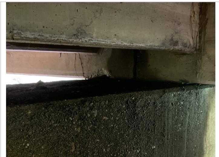
Span #2 girder #4 at Bent #2 spalling.
