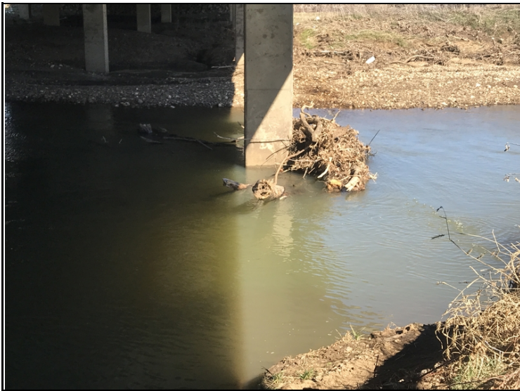
Bent #4 drift accumulation.
