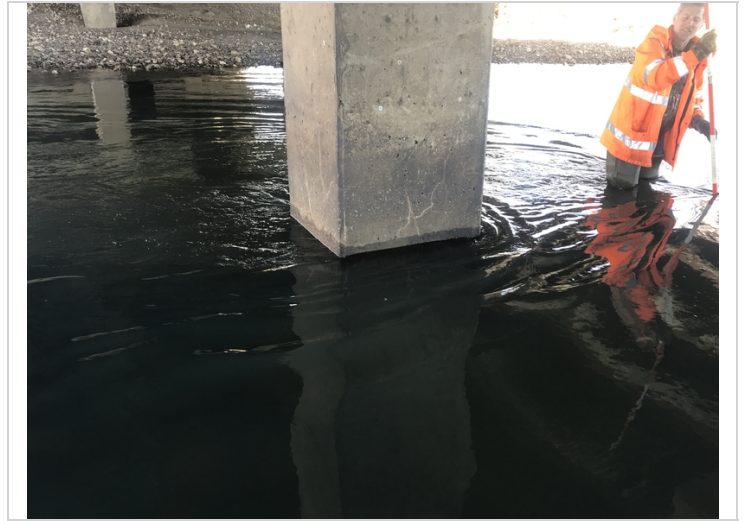
Bent #4 column #2 cracking with efflorescence buildup.
