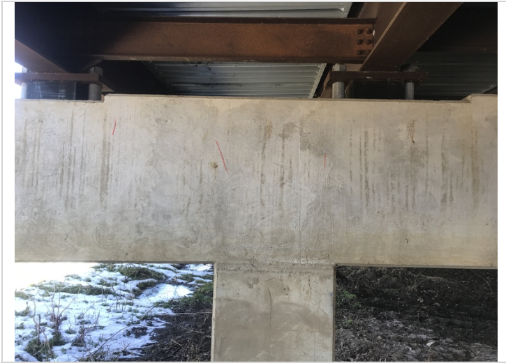
Bent #6 Lt cap cracking over column #1.
