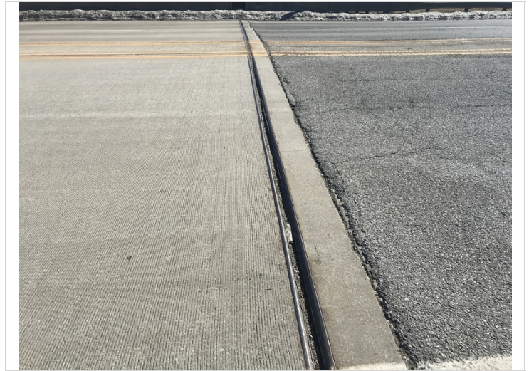
Abutment #1 debris impact in the expansion joint.
