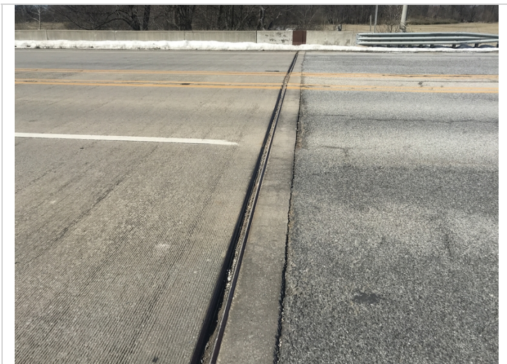
Abutment #2 joint seal debris impact.
