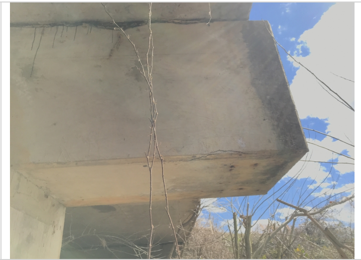
Bent # 3 Rt concrete delamination.
