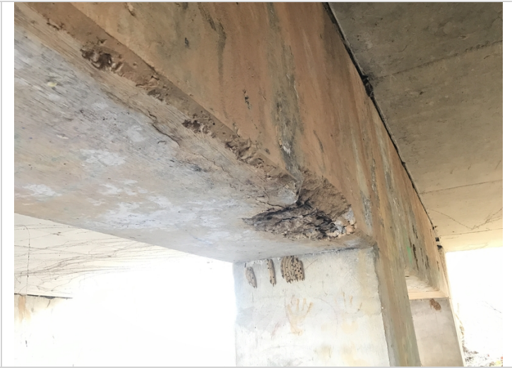
Bent # 2 cracking and spalling with exposed reinforcing steel.
