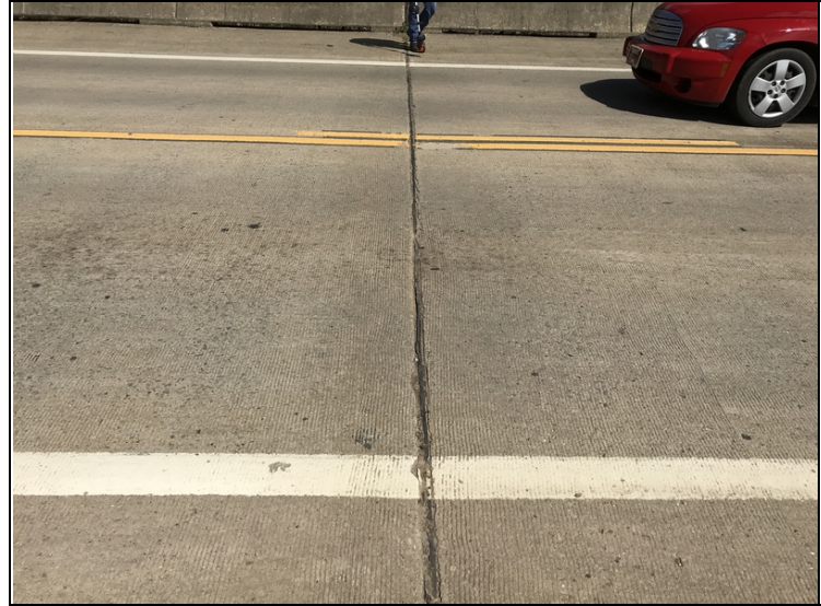
Bent # 2 joint seal deterioration with debris impaction.
