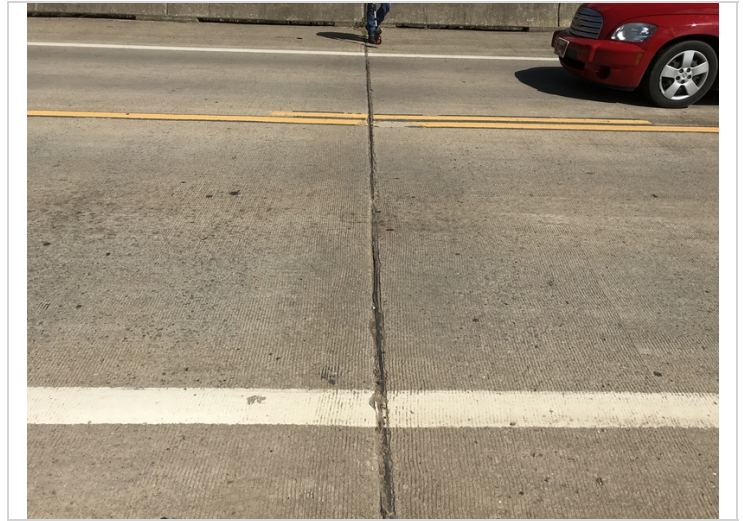
Bent # 2 joint seal deterioration with debris impactation.
