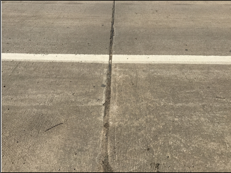
Expansion joint sealant over Bent # 2.
