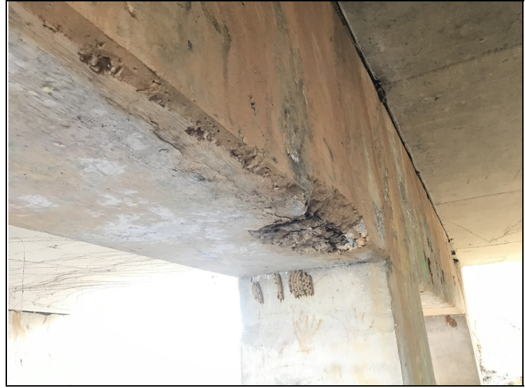
Bent # 2 cracking and spalling with exposed reinforcing steel.
