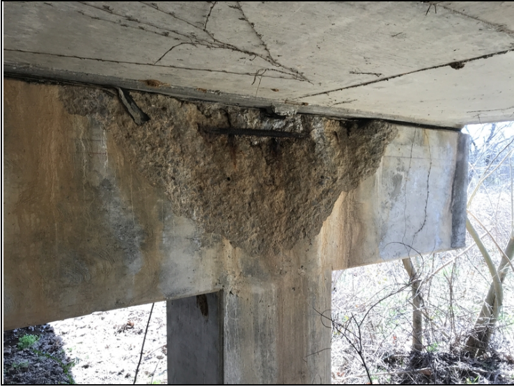
Span # 1 Bent # 2 Rt spalling with exposed reinforcing steel.
