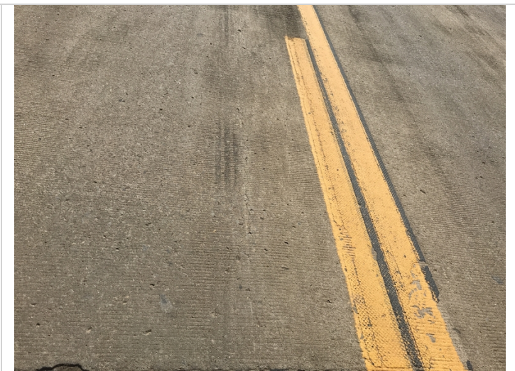
Longitudinal crack in Span # 2.
