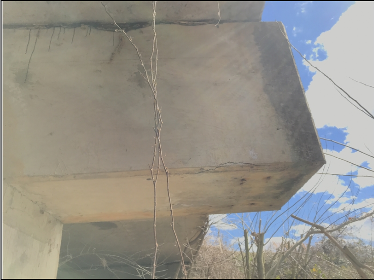
Bent # 3 Rt concrete delamination.
