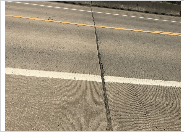
Expansion joint over Bent # 3. Typical.
