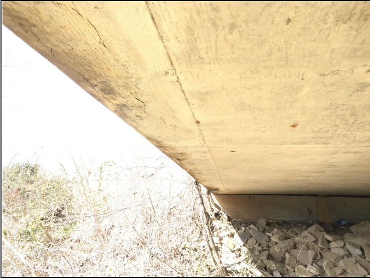
Span # 1 Rt concrete delamination along the Right edge of the slab.
