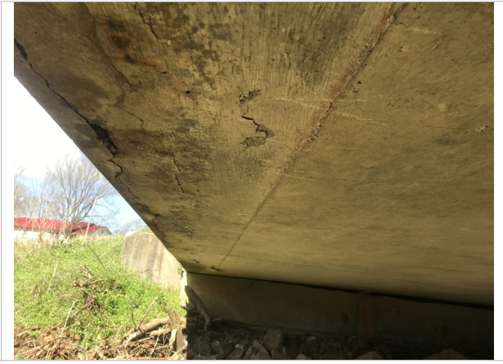
Delaminated area in the Right soffit of Span # 1.
