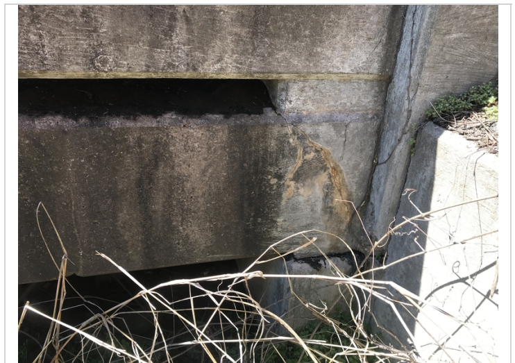
Diagonal cracking in the Left edge of Span # 1 adjacent to Bent # 1.
