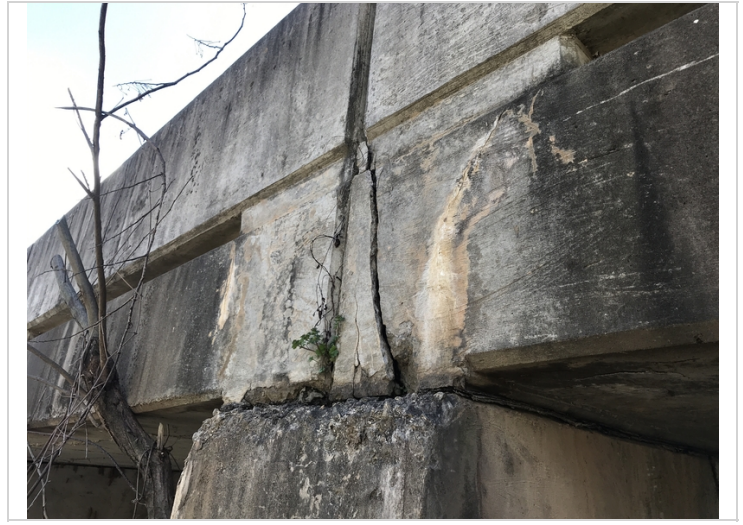
Bent # 2 Lt edge of the slab spalling with efflorescence.
