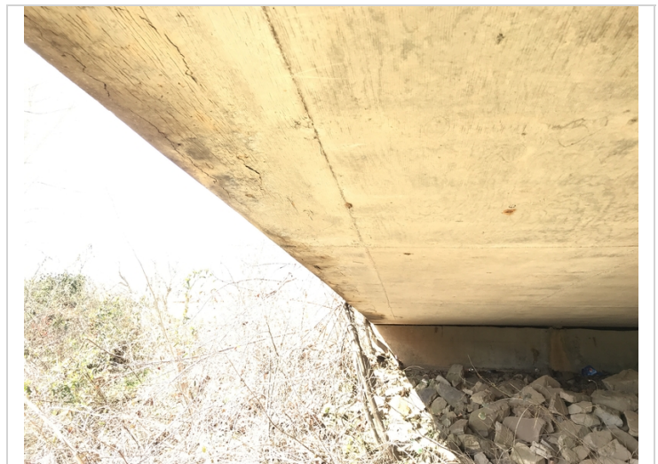
Span # 1 Rt concrete delamination along the Right edge of the slab.
