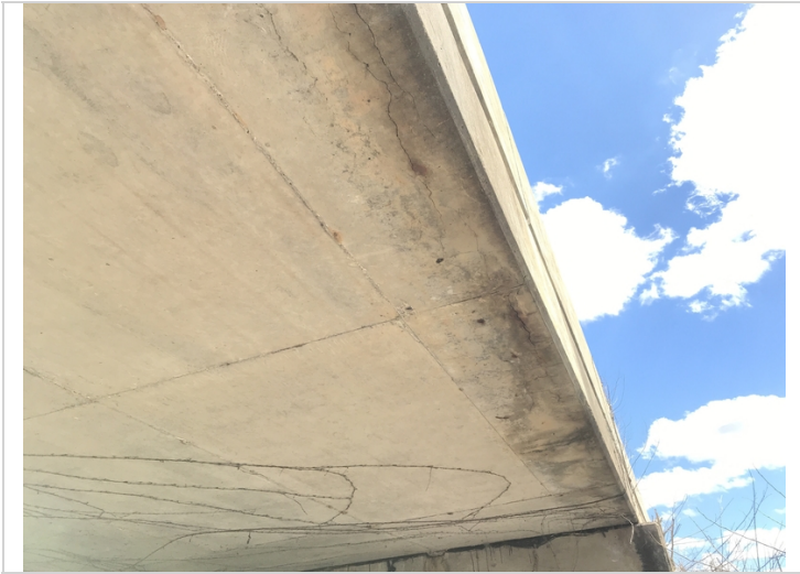
Span # 2 Rt delaminated concrete along the edge of the slab.
