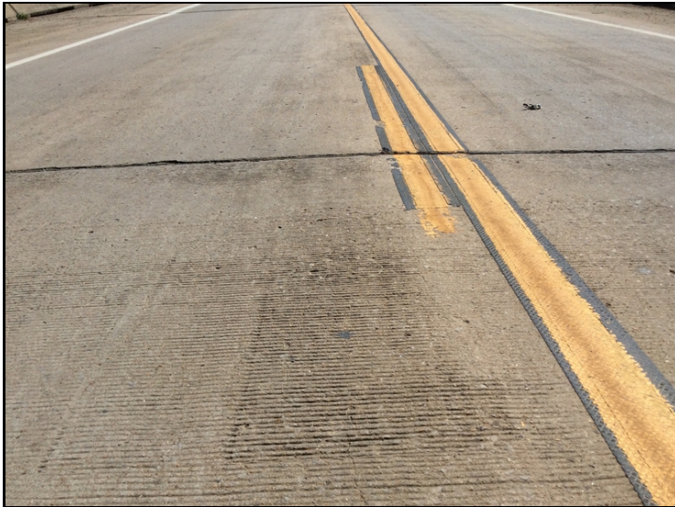
One longitudinal crack near centerline of Spans # 1, 2, and 3.
