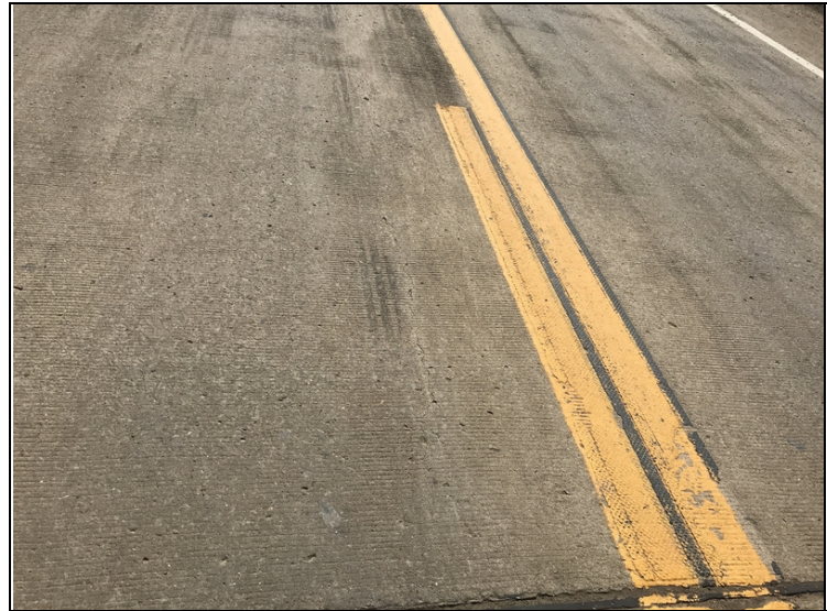
Sealable longitudinal crack in Span # 2.
