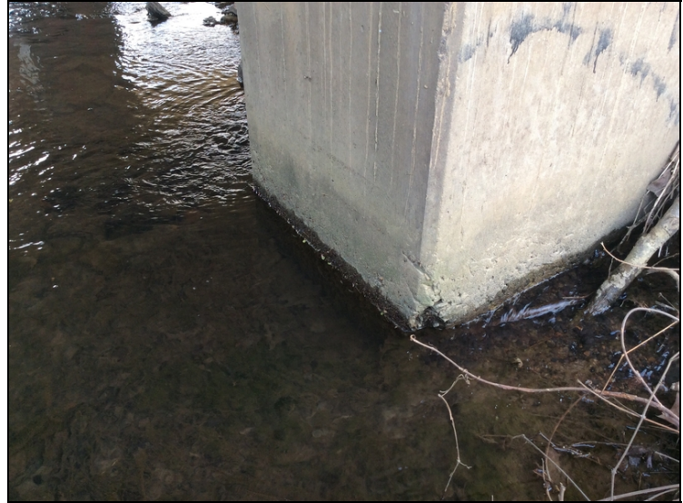
Bent # 3, Column # 1 has an area of honeycomb at the base on the Span # 3 side.
