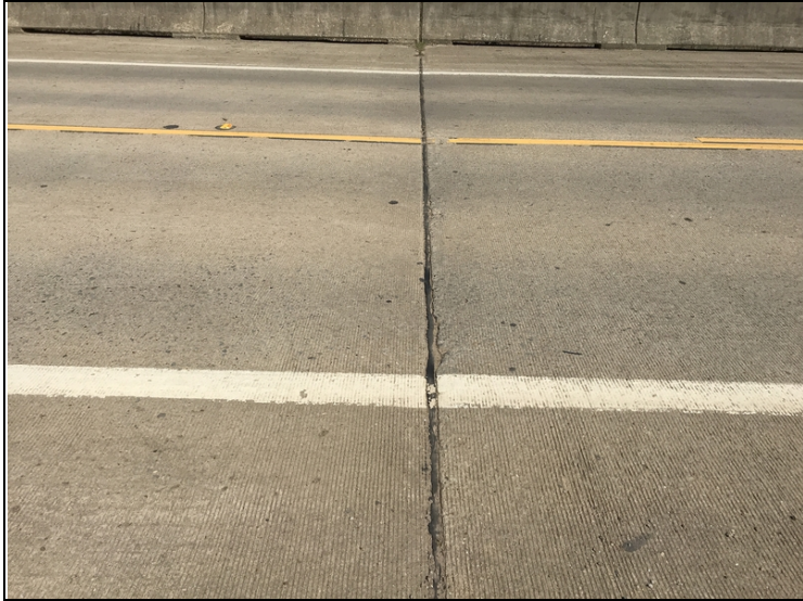
Bent # 3 joint seal debris impaction.
