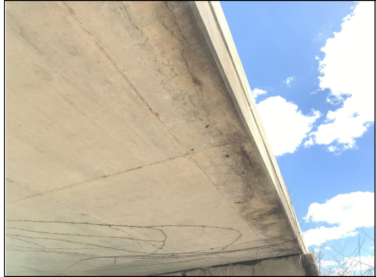
Span # 2 Rt delaminated concrete along the edge of the slab.
