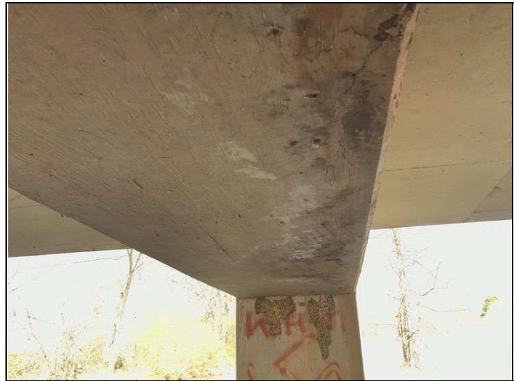
Bent # 3 cracking on the undersurface of the cap.
