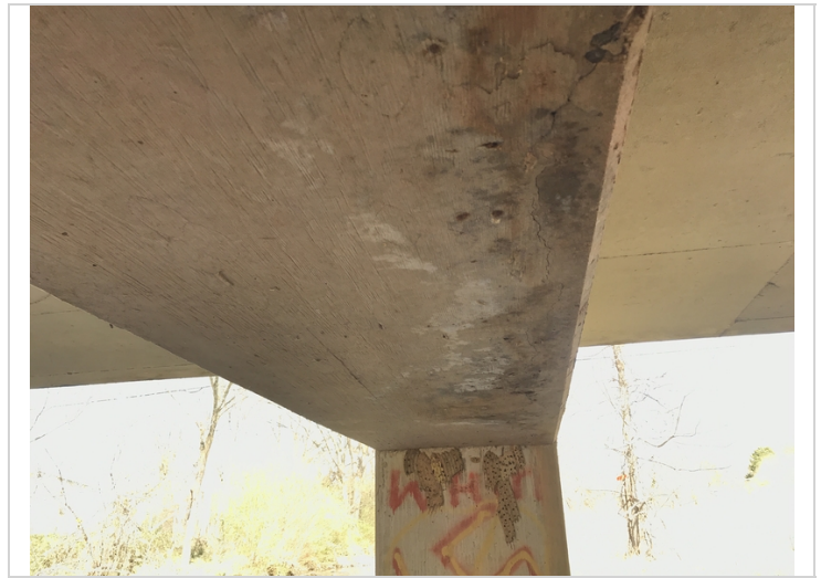
Bent # 3 cracking on the undersurface of the cap.
