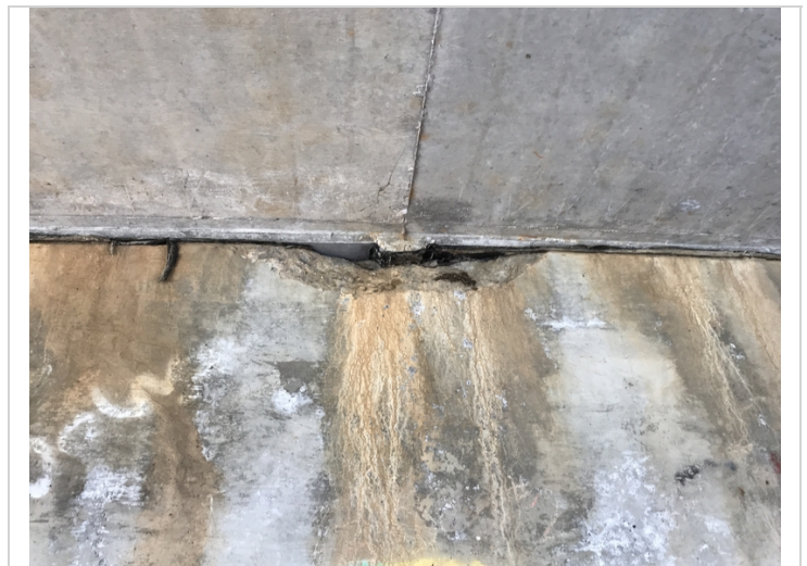
Bent # 2 Span # 2 spalling at the centerline of the Bent.
