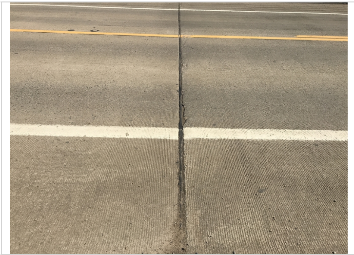
Debris accumulation in the joints. Joint over Bent # 3.
