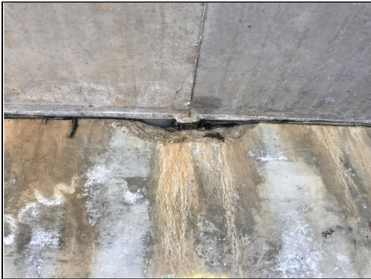
Bent # 2 Span # 2 spalling at the centerline of the Bent.
