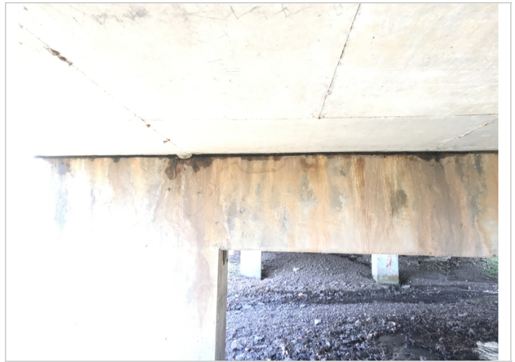
Water drains on the cap due to joint leakage.
