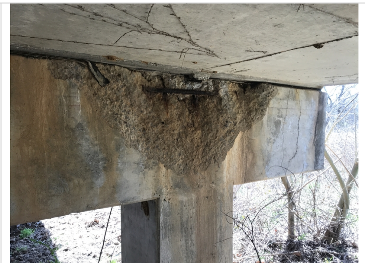
Span # 1 Bent # 2 Rt spalling with exposed reinforcing steel.
