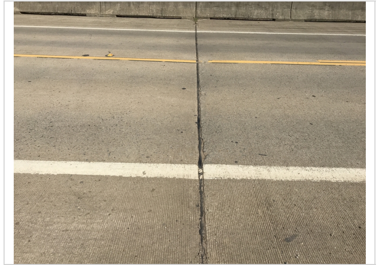
Bent # 3 joint seal debris impaction.
