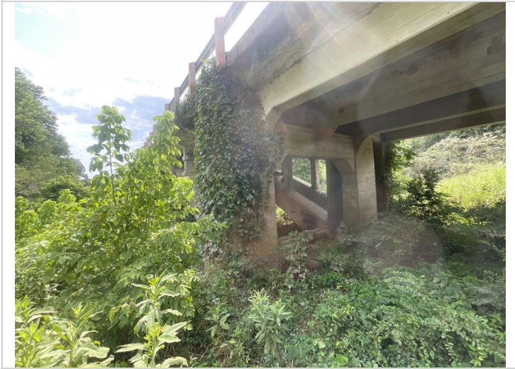
Portions of the structure are covered in vegetation during this inspection. Photo taken of the Left column of Bent # 2.
