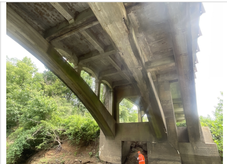
Arch Rib # 2 in proximity to Bent # 3. Spalls with exposed reinforcing steel.
