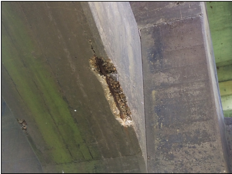
Sp #2, arch #2-Spalling with exposed reinforcing steel at bent #3.
