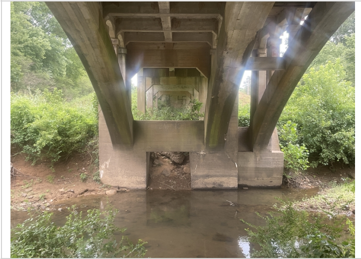
Skewback at Bent # 3. Typical.
