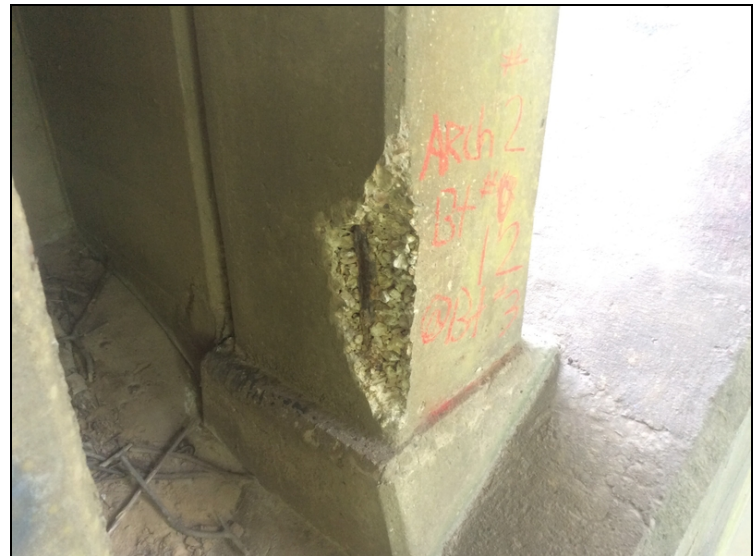
Arch #2 bent #12-Spalling with exposed reinforcing steel in column.
