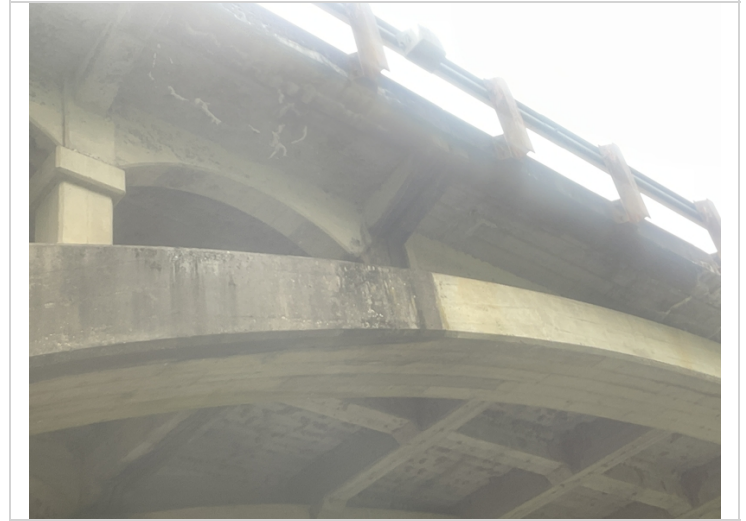
Arch Rib # 1, Column # 9 at the floor beam juncture. Diagonal crack.
