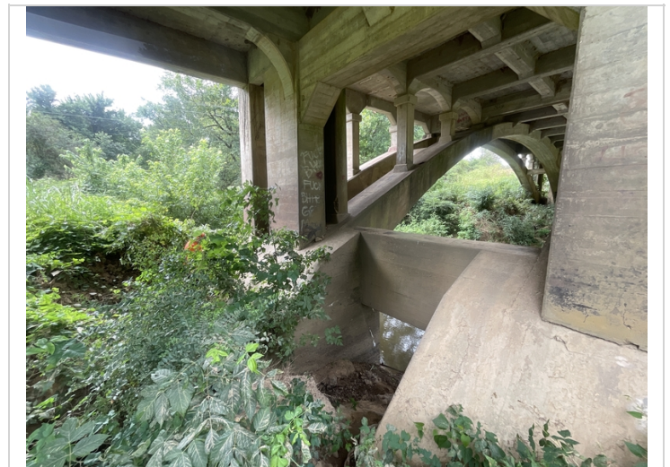
Bent # 3 Skewback arch Ribs # 2 & 3. Typical.
