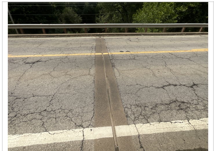
Expansion joint with previous repair on the deck over Span # 2.
