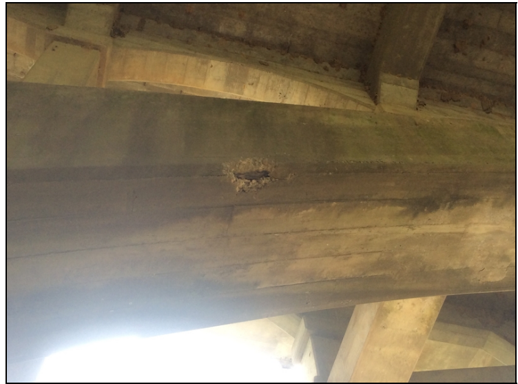
Sp #2, arch #2-Spalling in arch rib in bay #11.
