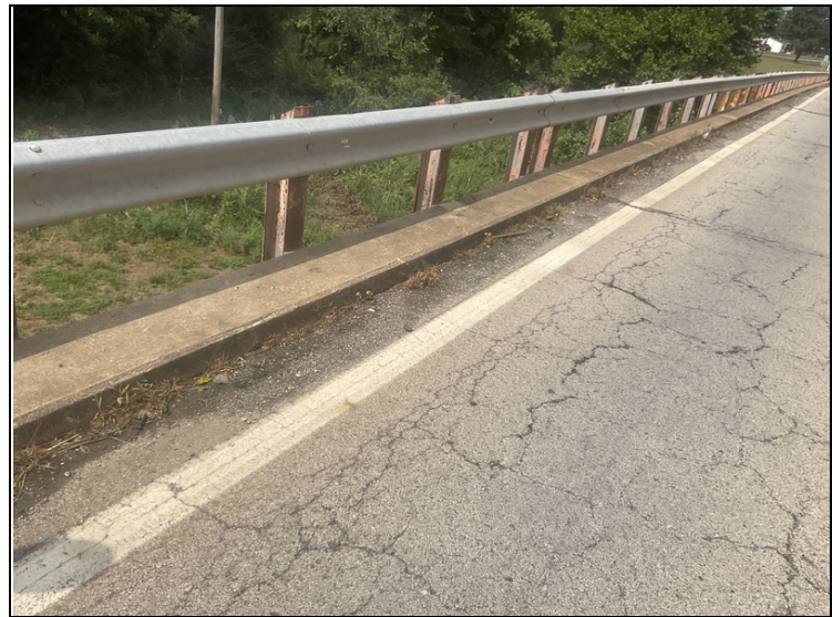
Debris accumulation in the Right gutter. Typical.
