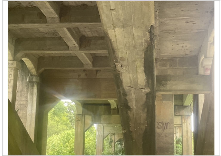
Spalls with exposed reinforcing steel in Arch Rib # 2.
