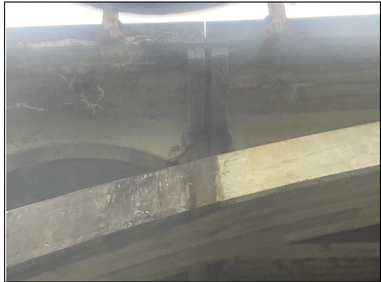
Arch Rib # 1, Column # 9 at the floor beam juncture. Diagonal crack.
