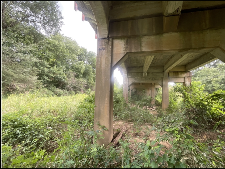
Bent # 4. Column # 1. Back face. Spall with exposed reinforcing steel.
