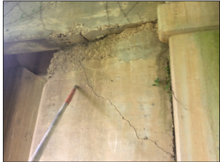
Bent # 2, column # 2-Spalling cracking on ahead face.
