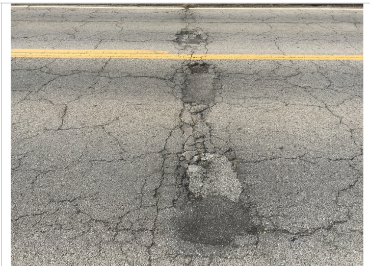
Potholes over the deck joints over the intermediate bents.
