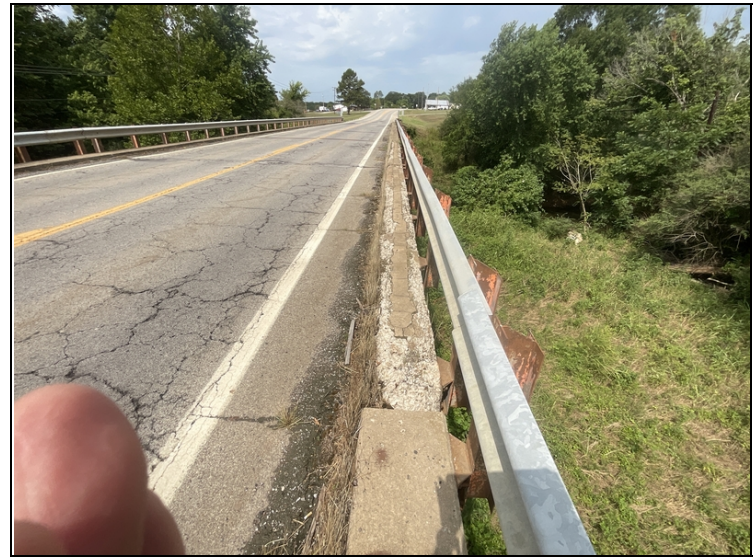
Soft deteriorated concrete in the Left curb.
