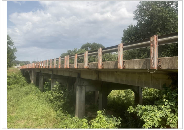
Bridge railing posts with a deteriorated paint system.
