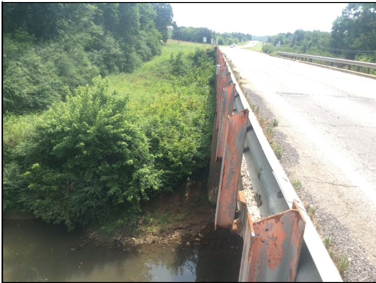
Bridge railing Post has paint failure.
