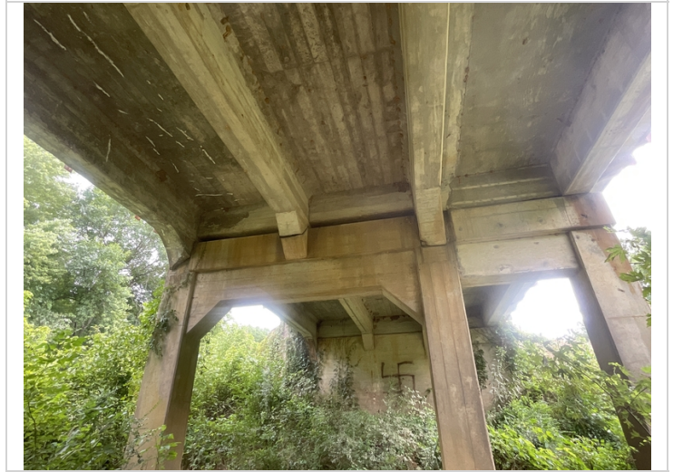
Span # 5 at Bent # 6. Spalls in the girder haunches adjacent to Bent # 6. Photo of Girder # 1 on the Left.
