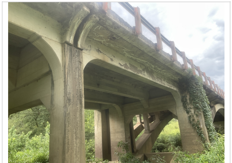
Span # 3. Girder # 1. Scale on the exterior face of the girder.
