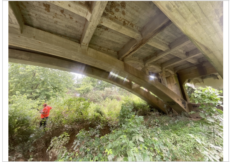
Arch Ribs # 2 & 3 adjacent to Bent # 2. Typical.
