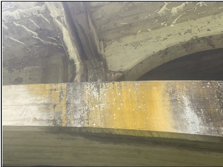
Arch Rib # 1, Column # 4 at the floor beam juncture. Diagonal crack.
