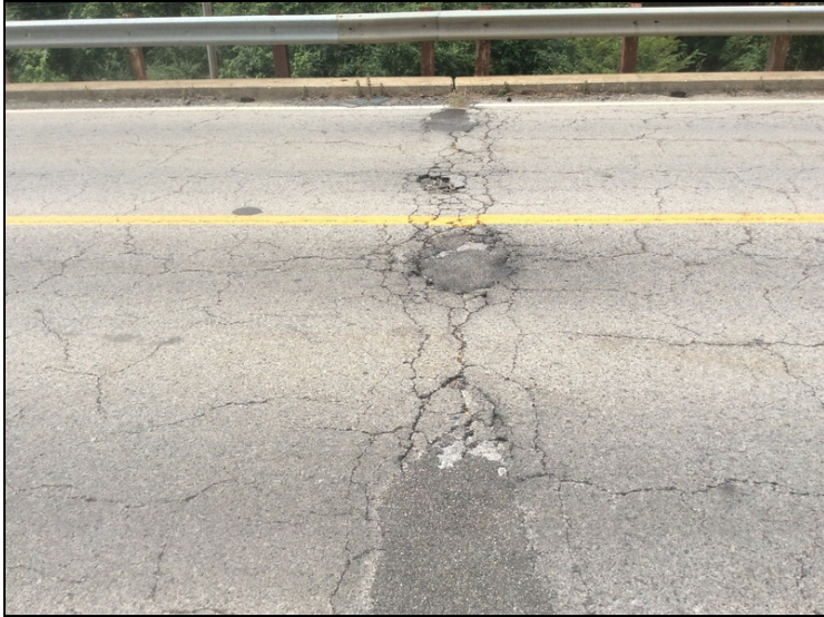
Bent #4 expansion joint-Potholes forming in driving surface.
