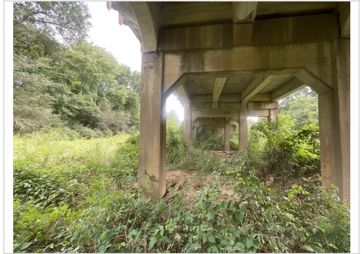
Bent # 4. Column # 1. Back face. Spall with exposed reinforcing steel.
