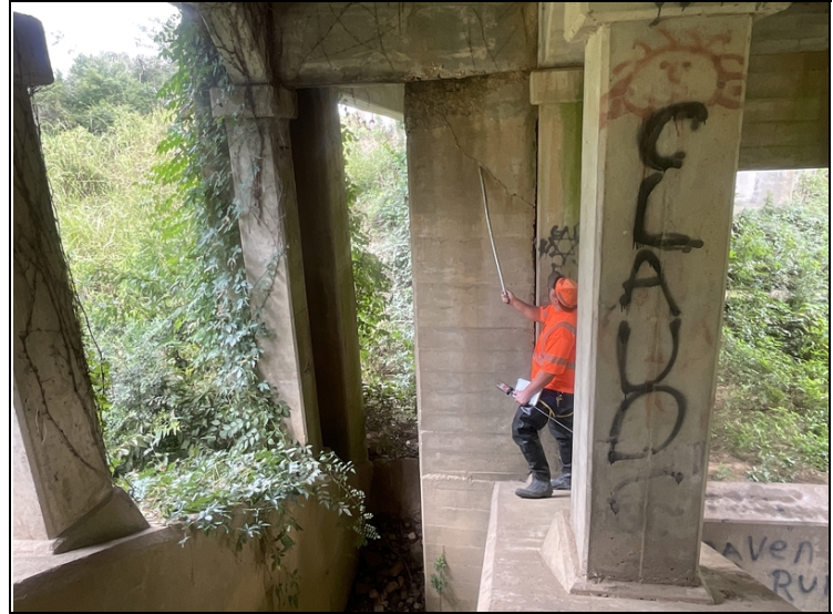
Column # 2. Bent # 2. Span # 2 ahead face. Diagonal crack with spalling at the cap juncture where the structure was widened.
