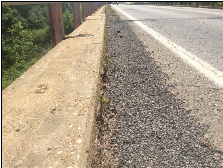
Dirt and debris in gutters.
