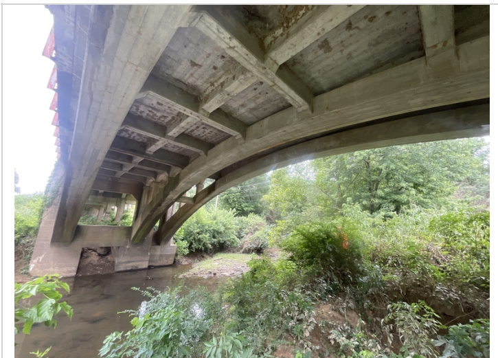
Arch Ribs # 2 & 3 adjacent to Bent # 3.
