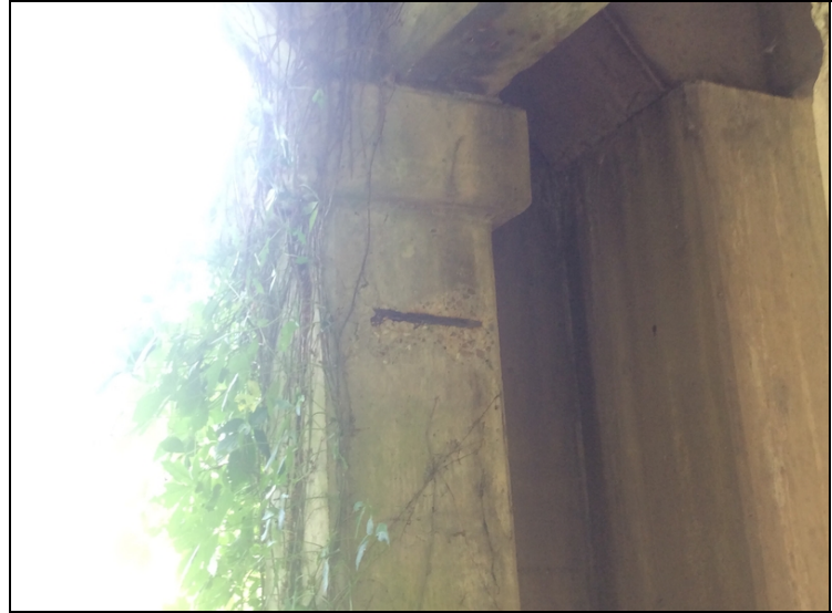
Arch #3, spandrel column #1-Spall with exposed reinforcing steel in column.
