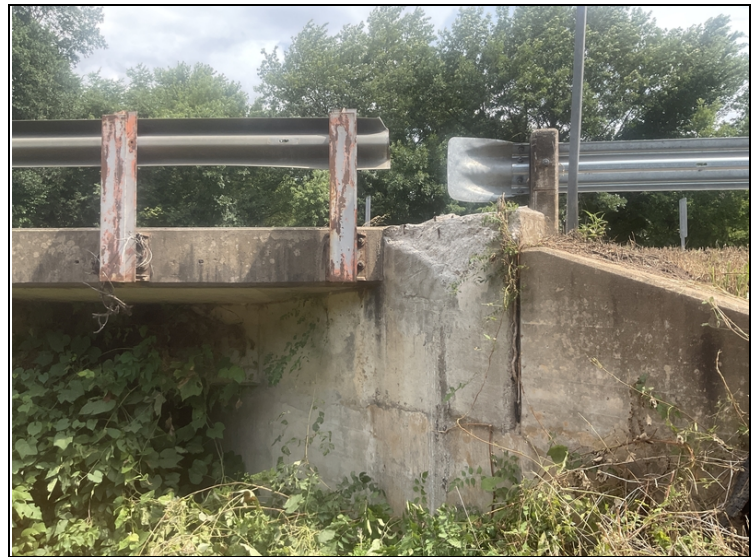
The Southeast end post has been knocked off the structure.
