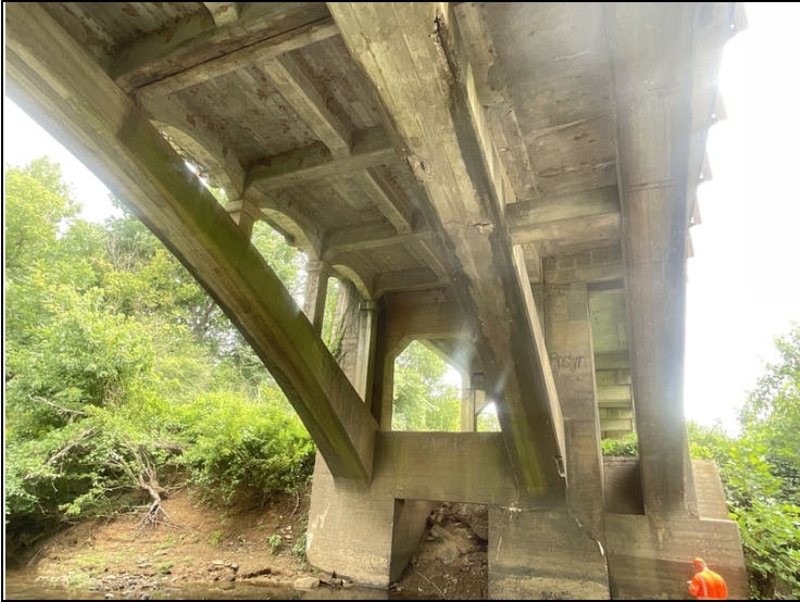
Arch Rib # 2. Spalls with exposed reinforcing steel in proximity to Bent # 3.
