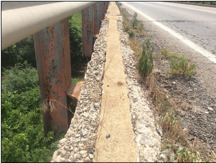
Span #2 Left-Concrete deterioration / spalling to curbs.
