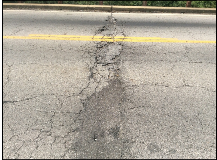
Bent #2 expansion joint-Spalling in driving surface.
