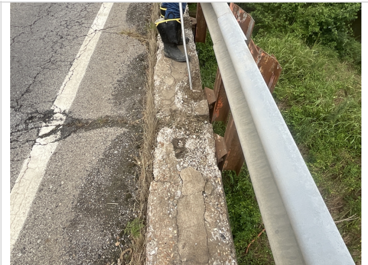
Concrete deterioration and concrete section loss in the Left curb have deterioration that exposes several of the anchors of the bridge railing posts. Photo taken from the Left side of Bent # 4.
