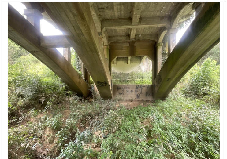
Skewback at Bent # 2. Typical.
