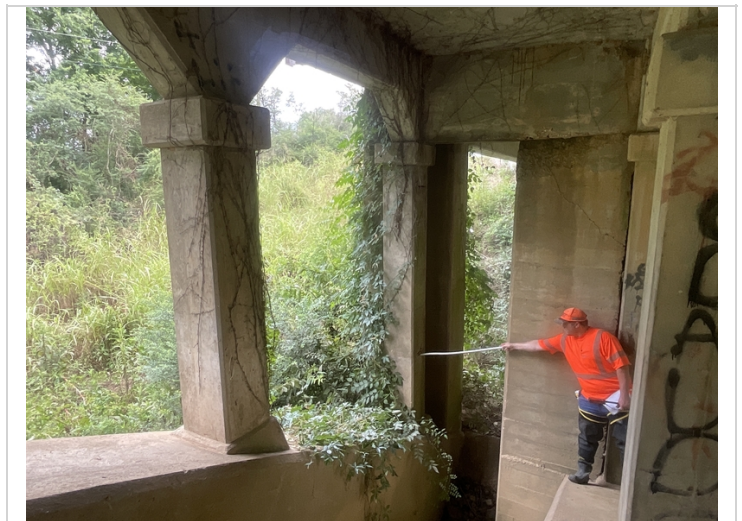
Bent # 2 ahead face of Column # 3. Spalls with exposed reinforcing steel.
