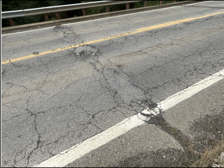
Asphalt wearing surface is breaking apart over Bent # 4.
