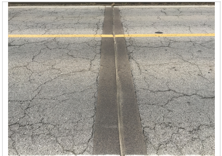
Bent # 3 joint repair.
