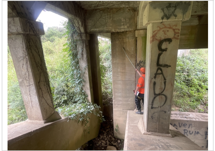
Column # 2. Bent # 2. Span # 2 ahead face. Diagonal crack with spalling at the cap juncture where the structure was widened.
