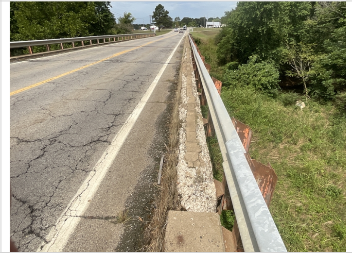
Soft and deteriorated concrete in the Left gutter.
