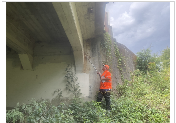
There is a diagonal crack with efflorescence on the Left side of Bent # 1 outside the bearing area.
