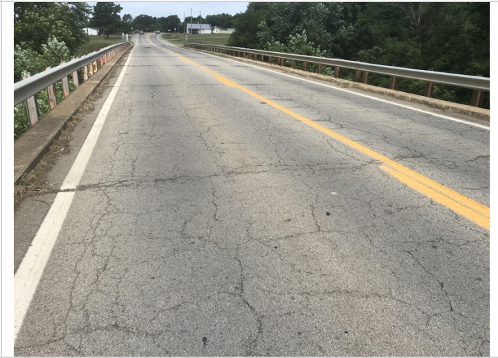
Driving surface cracking.
