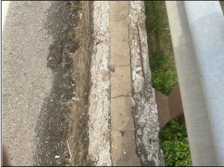
Exposed reinforcing steel in the curb - Left side of structure.
