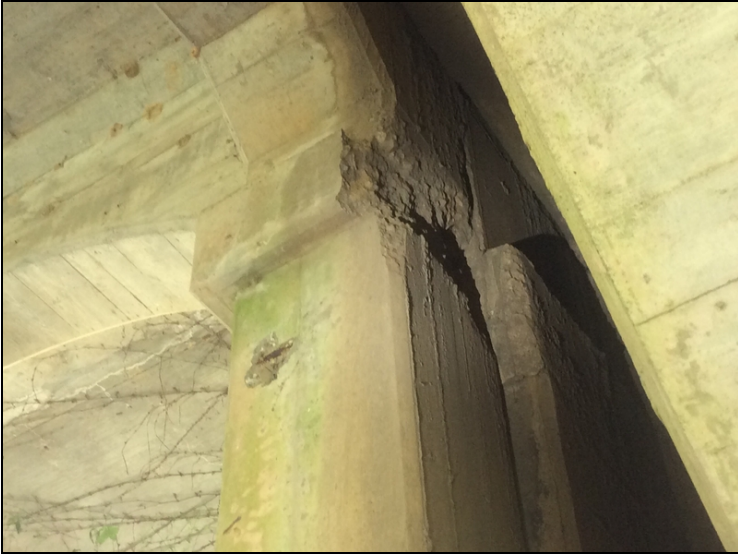
Arch rib #2, column #1-Spalling at cap juncture.
