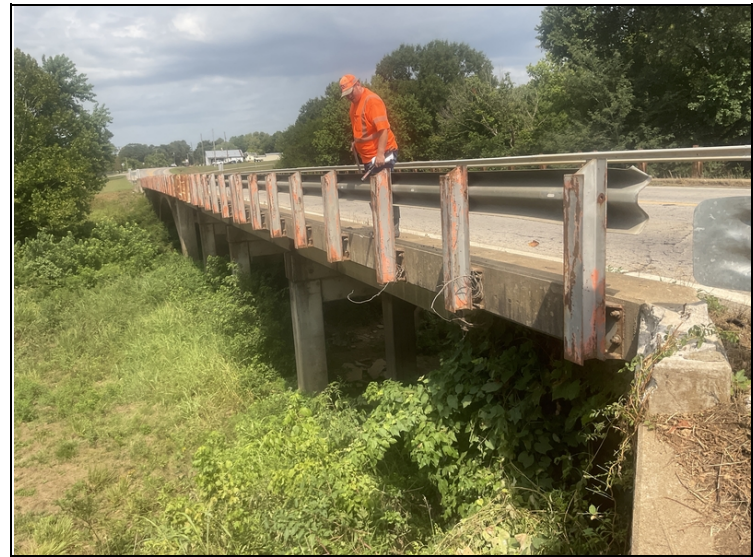
Bridge railing post on the Right side of structure. Deteriorated paint system. Typical.
