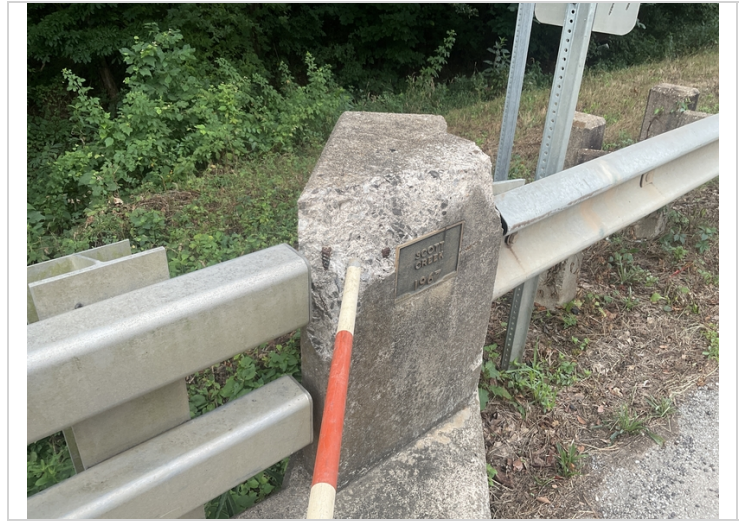
Abutment 1, right end post-Spalling with exposed reinforcing steel
