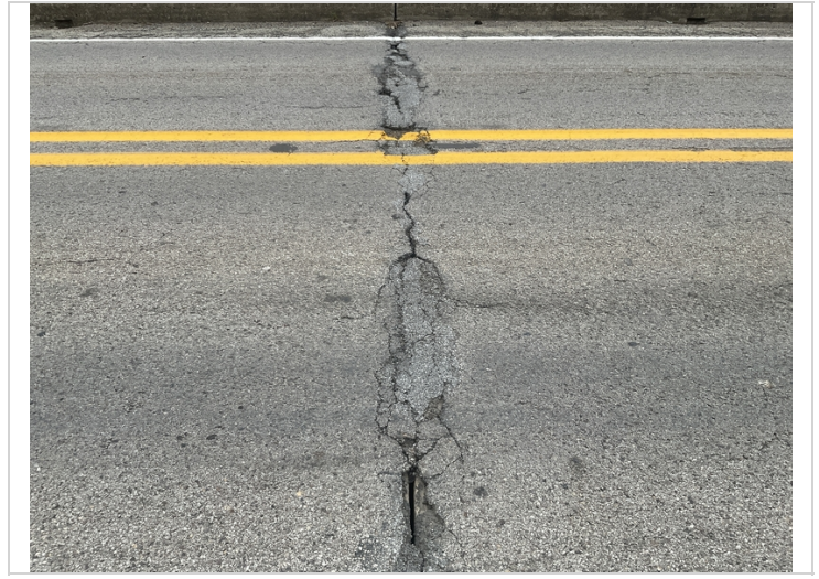
Asphalt breaking apart over bent 3
