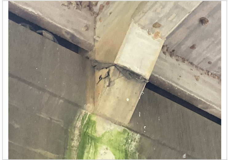
Bent 3 cap aheadface under girder 3-Spalling with exposed reinforcing steel
