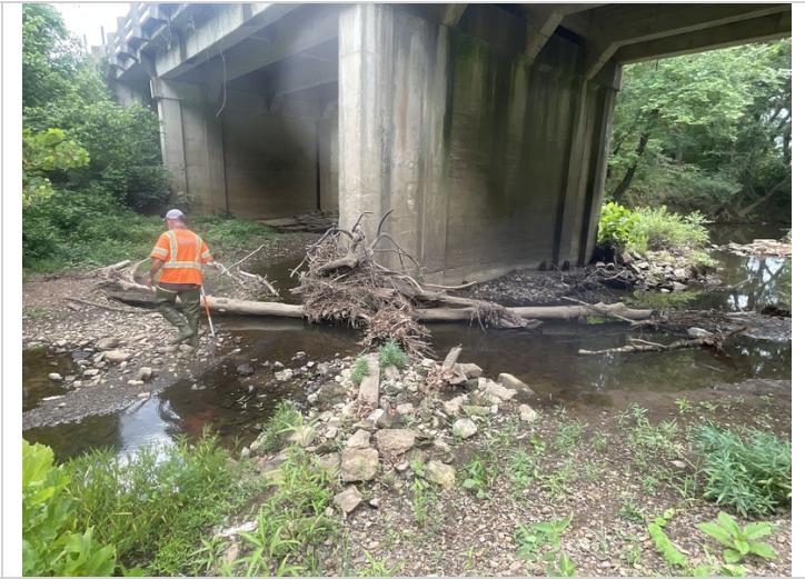
Drift accumulation at bent 3
