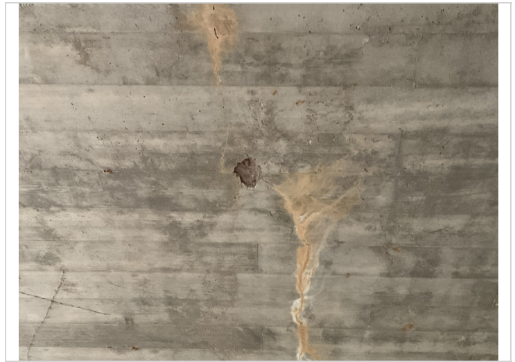
Span 3-Scaling near centerline at mid-span
