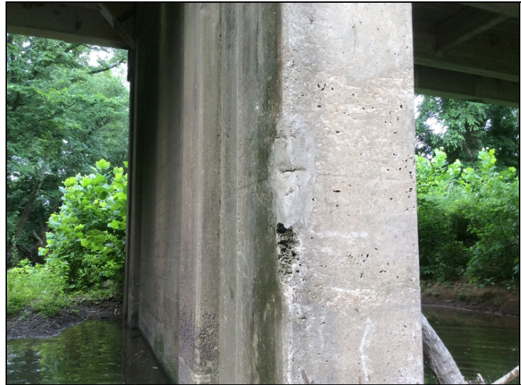
Bent # 3, column # 1 has an area of concrete section loss that is 3 inches deep and 12 inches tall near the base of column with an adjacent repair.
