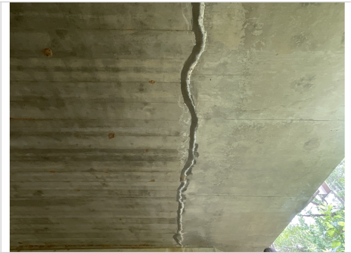
Span 4, right side-Efflorescence along construction joint
