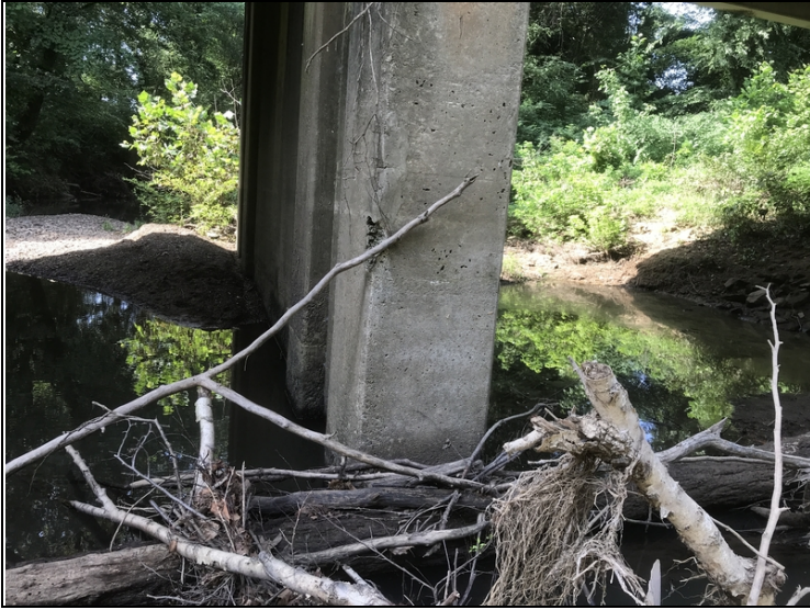
Bent # 3, Column # 1-Concrete deterioration.
