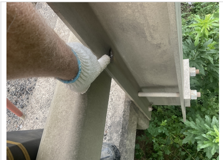
Span 1, right at bent 2-Missing bolt for bottom railing
