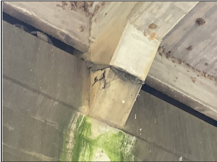
Bent # 3 cap aheadface under girder # 3-Spalling with exposed reinforcing steel.
