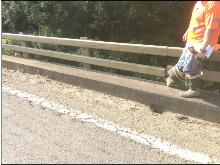
Connection is missing bolts in the right side of Span # 3.
