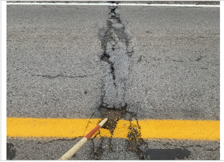
Asphalt breaking apart over bent 3
