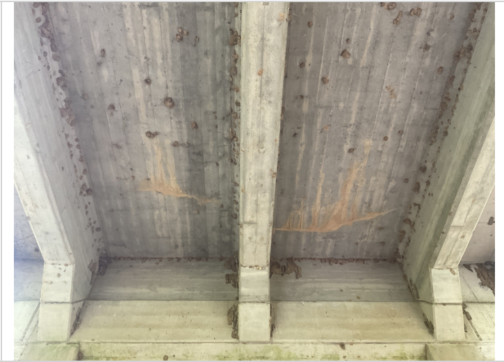
Span 3-Transverse cracking with staining
