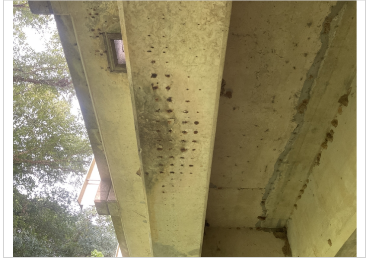
Span 1, girder 5-Exposed slab bolsters
