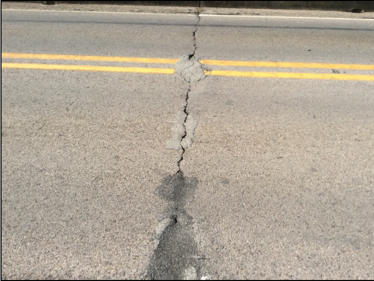
Bent # 2 asphalt deterioration over the deck joint.
