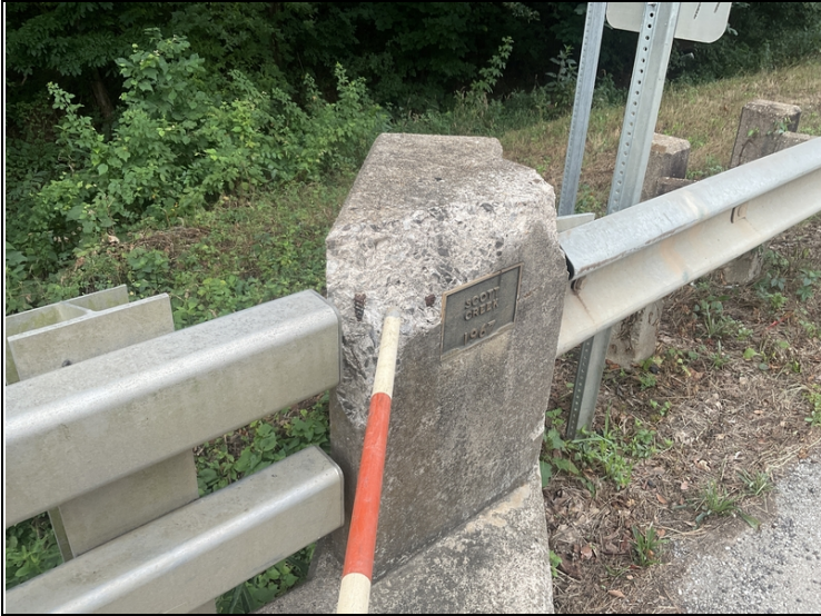
Abutment # 1, right end post-Spalling with exposed reinforcing steel.
