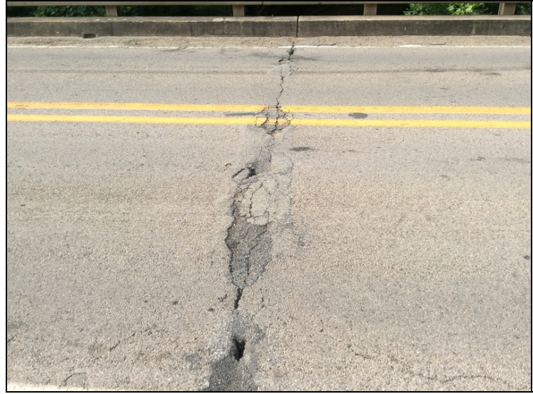
Bent # 3 asphalt deterioration over the joint.
