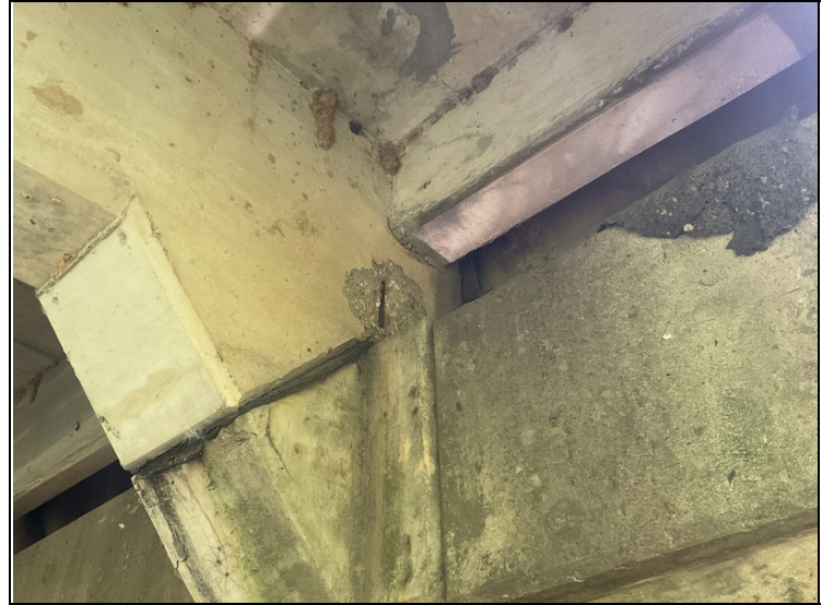
Span # 1, girder # 4 over bent # 2-Spall with exposed reinforcing steel.
