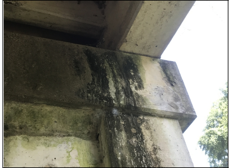
Spall with exposed reinforcing steel in the left side of bent # 2 cap.
