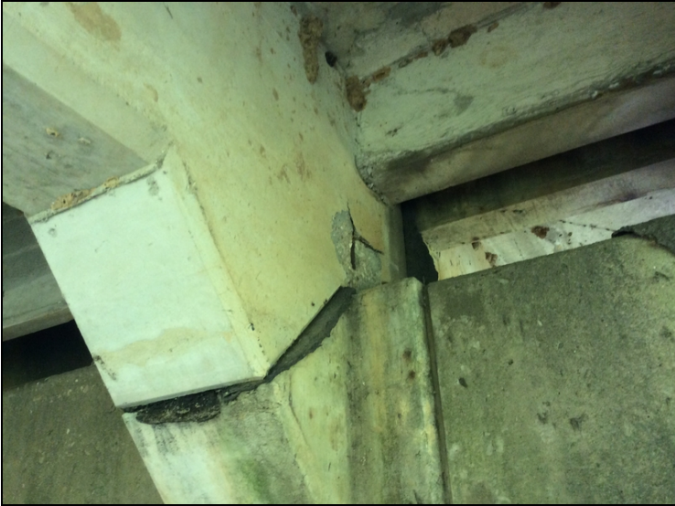
Span # 1, girder # 4 at bent # 2-Spalling with exposed reinforcing steel.
