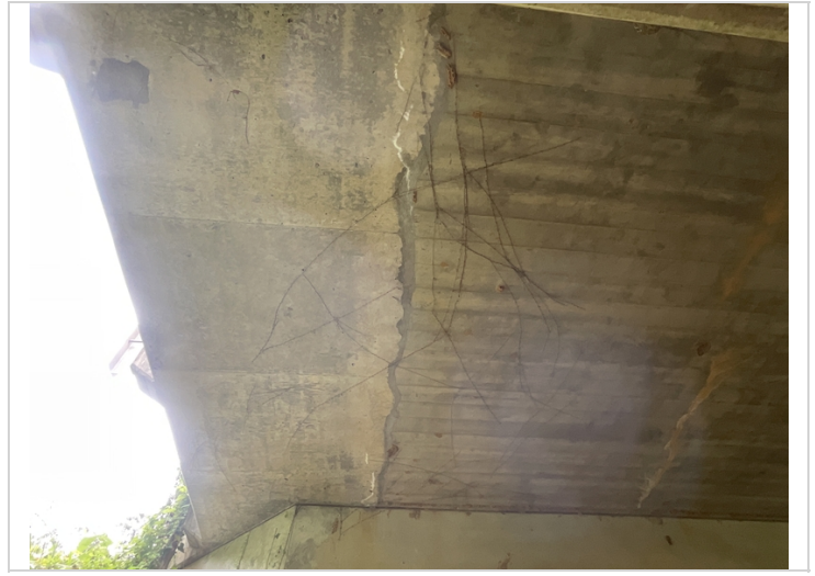
Span 4, left side-Longitudinal cracking with efflorescence along construction joint
