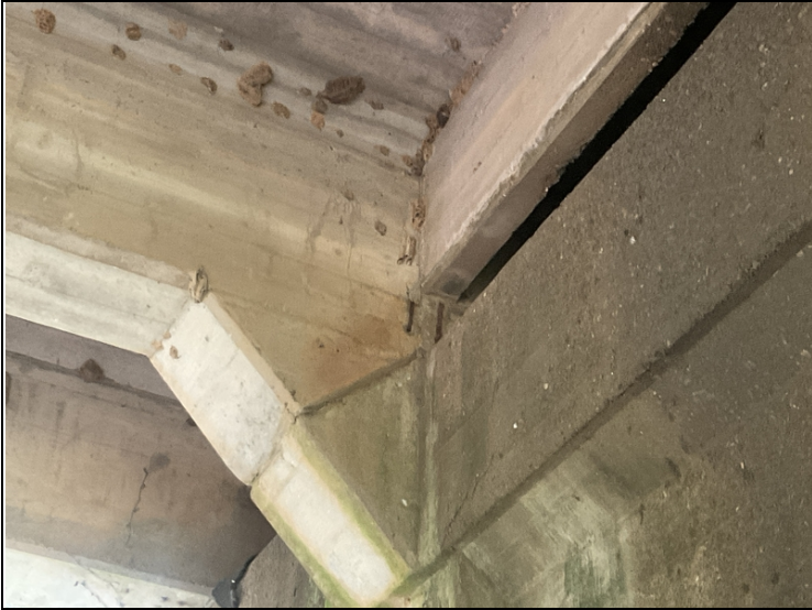
Span # 2, girder # 4 at bent # 2-Shallow spall with exposed reinforcing steel.
