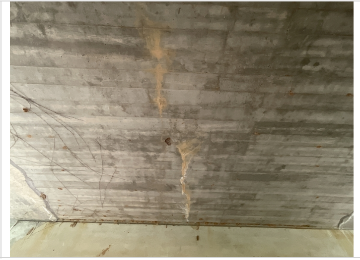
Span 4, longitudinal crack with efflorescence and staining at centerline
