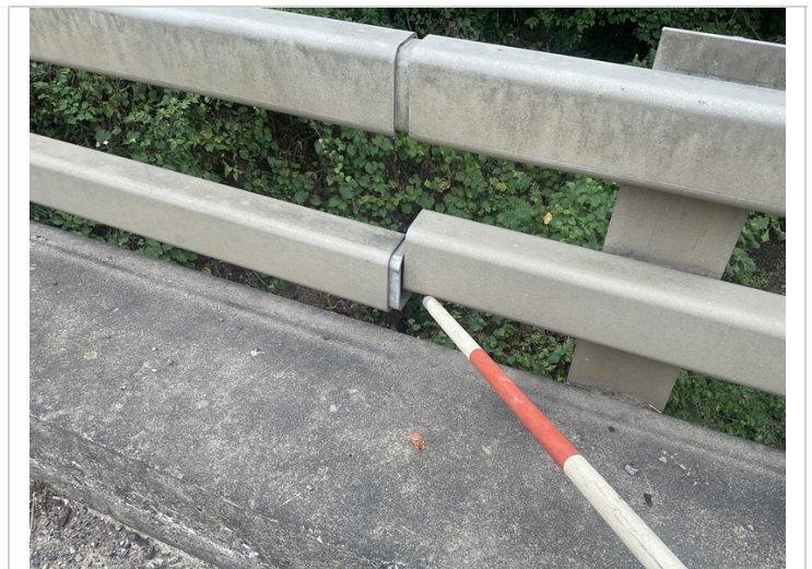
Span 3, right railing-Failed connection
