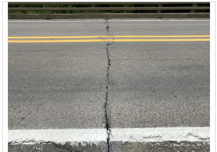
Asphalt cracked over bent 2
