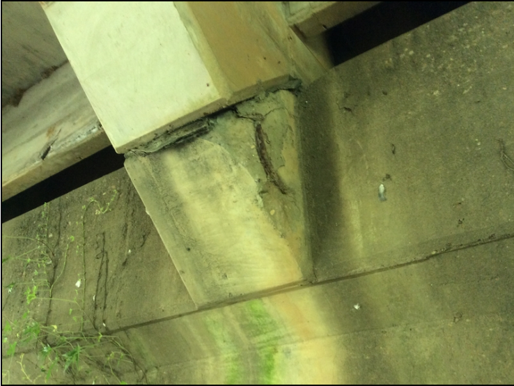
Bent # 2-Spalling with exposed reinforcing steel in cap haunch.
