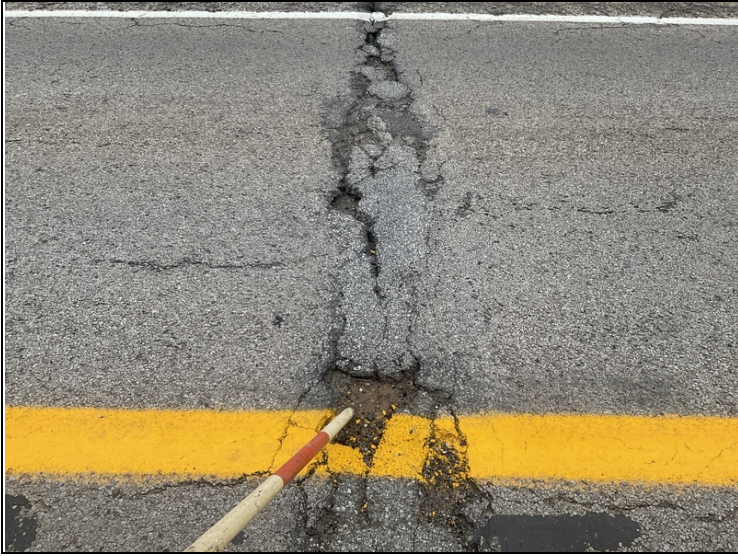
Asphalt breaking apart over bent # 3.
