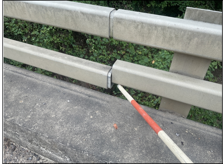
Span # 3, right railing-Failed connection.
