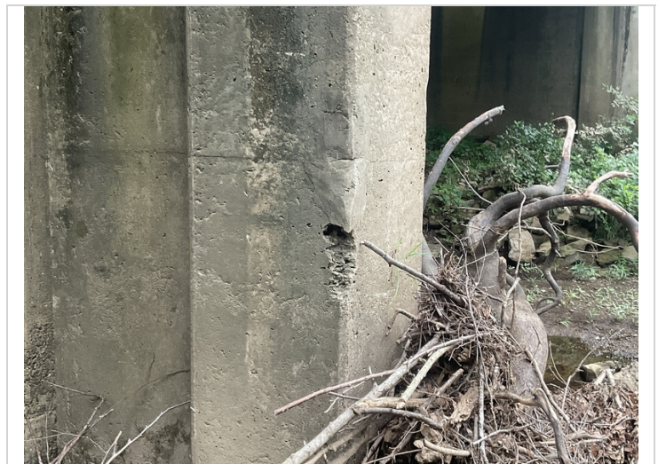
Bent 3, column 1-Concrete deterioration
