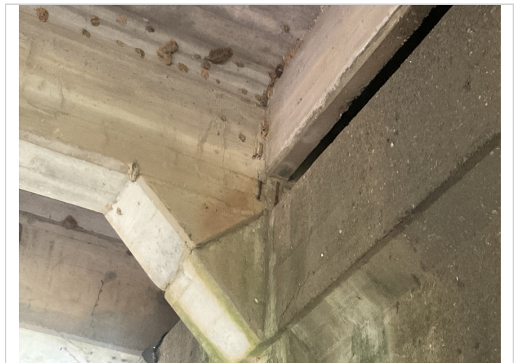
Span 2, girder 4 at bent 2-Shallow spall with exposed reinforcing steel
