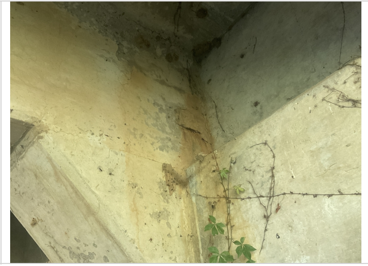
Span # 1, girder # 4 at bent # 2 has a 6" spall with exposed reinforcing steel.
