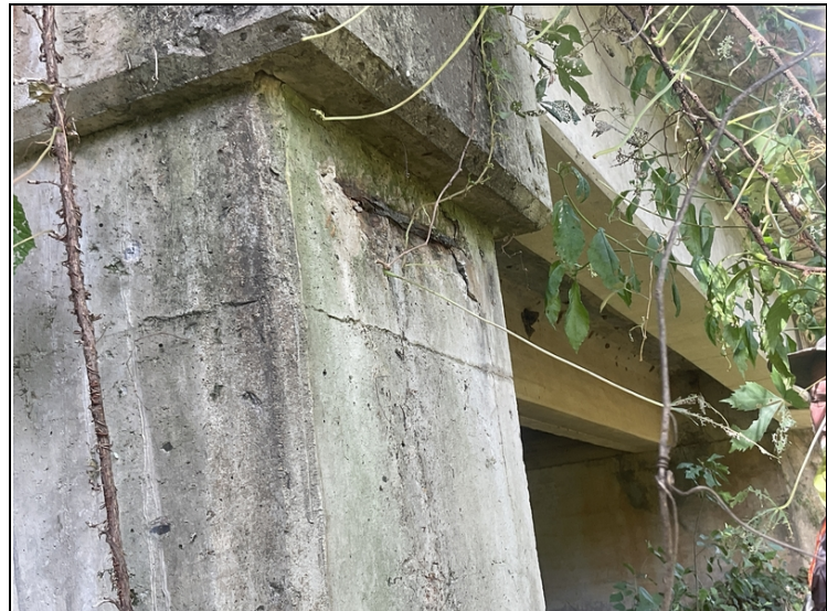
Bent # 2, column # 1-Spall with exposed reinforcing steel.
