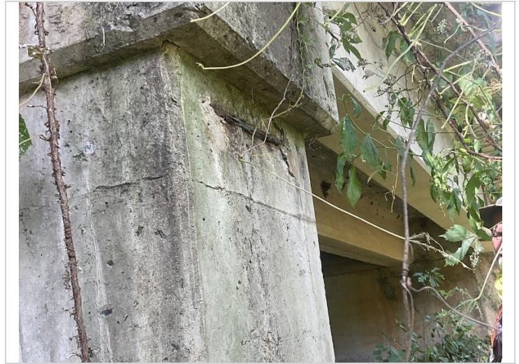
Bent 2, column 1-Spall with exposed reinforcing steel
