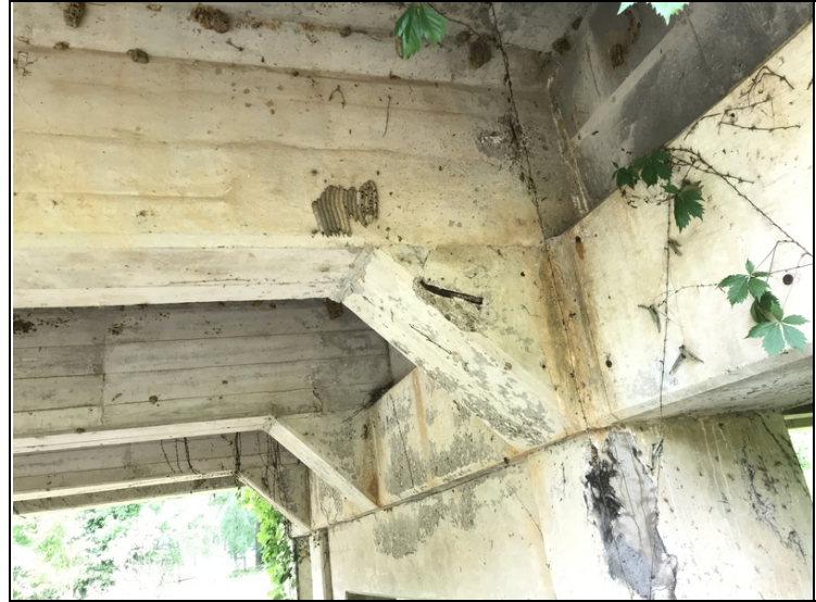
Span # 1, girders # 3 and 4 have shallow concrete spalls with exposed reinforcing steel adjacent to bent # 2.
