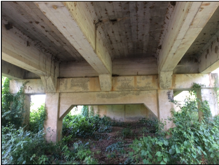
Bent # 2 staining from apparent water leakage through the deck joints.
