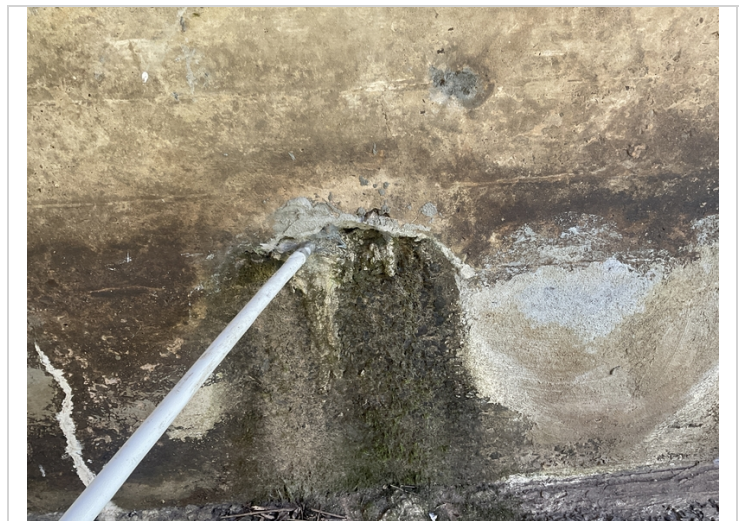
Abutment 2 stem wall-Concrete deterioration
