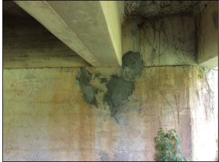
Abutment # 1 has a 30" delaminated area under girder # 2. The grouted repairs to the delaminated area have failed and sound delaminated when sounded with a geologist hammer.
