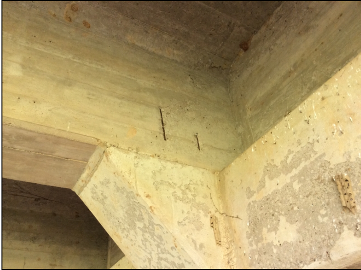
Span # 1, beam # 3-Spalling with exposed reinforcing steel over bent # 2.
