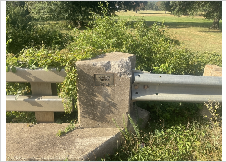
Left end post at abutment # 1 has shallow spalling to the top of post.
