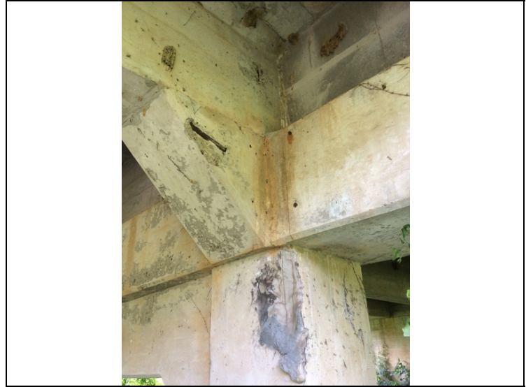
The ahead face of bent # 2 cap haunch has a spall with exposed reinforcing steel under girder # 2.
