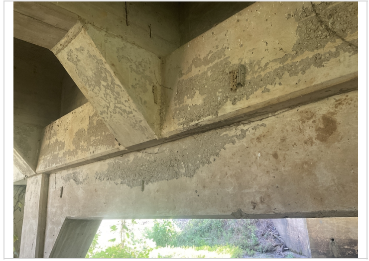
Scaling in bent 2 cap backface
