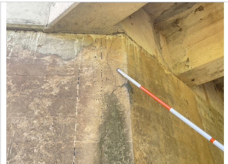
Abutment # 2 right monolithic wing wall has a moderate width vertical crack in upper portion of wall adjacent to abutment stem wall.
