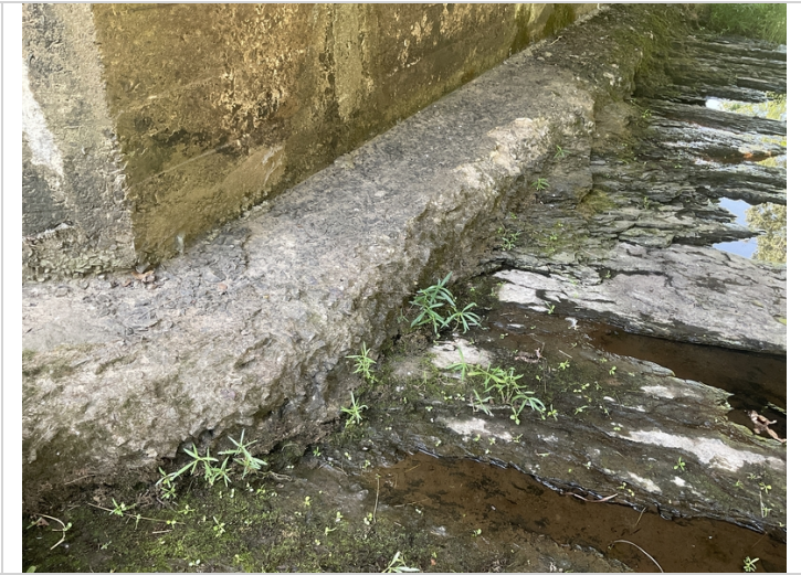
Abutment 2 footing-Concrete deterioration
