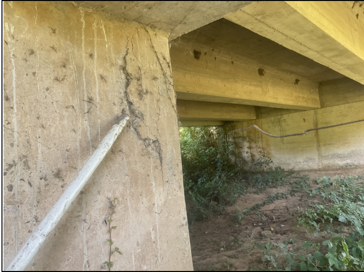
Bent # 2, column # 2 left exterior face has an 18" delaminated area at the cap juncture.
