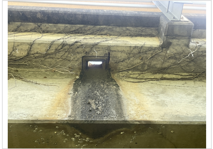
Span # 2, right deck overhang has a shallow spall with exposed reinforcing steel adjacent to the deck drain. Initial section loss to the reinforcing steel.
