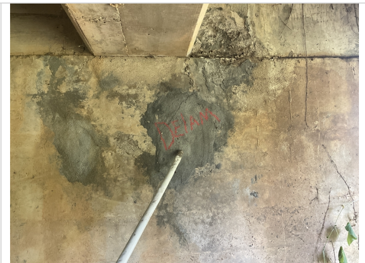
Abutment 1, left side-Delaminated repair
