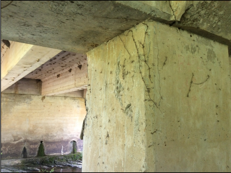
One basketball size delaminated area next to the repaired spall in Bent # 2, Column # 2.
