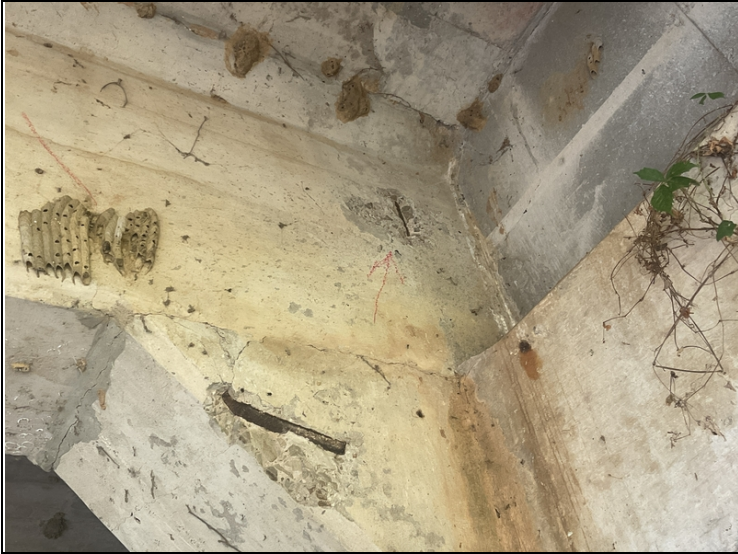
Span # 2, girder # 2 has a shallow 6" spall with exposed reinforcing steel over bent # 2.
