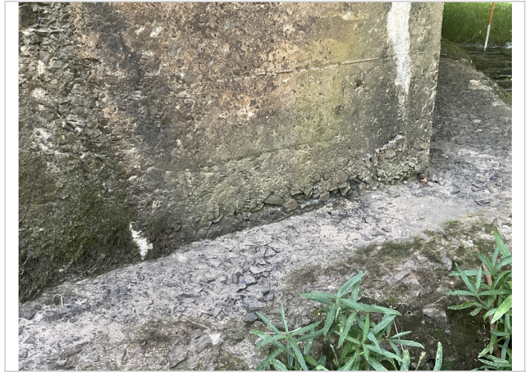
Abutment 2, right wing wall-Abrasion
