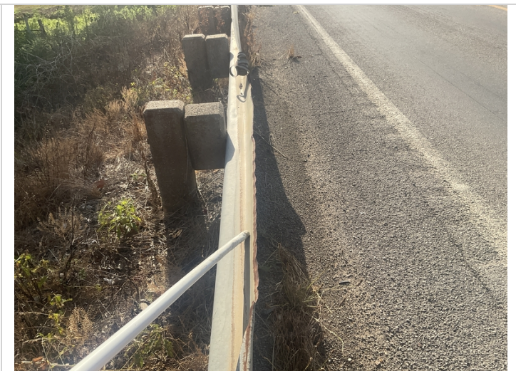
The left approach railing at abutment # 1 has collision damage that has created sharp jagged edges along the top.
