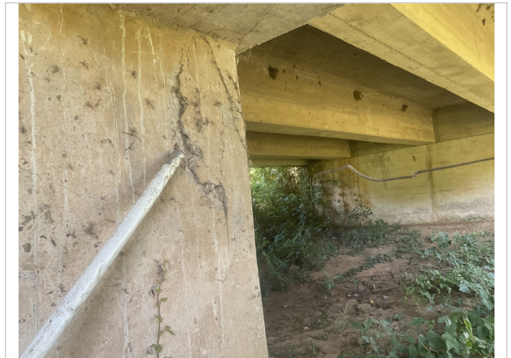
Bent # 2, column # 2 left exterior face has an 18" delaminated area at the cap juncture.
