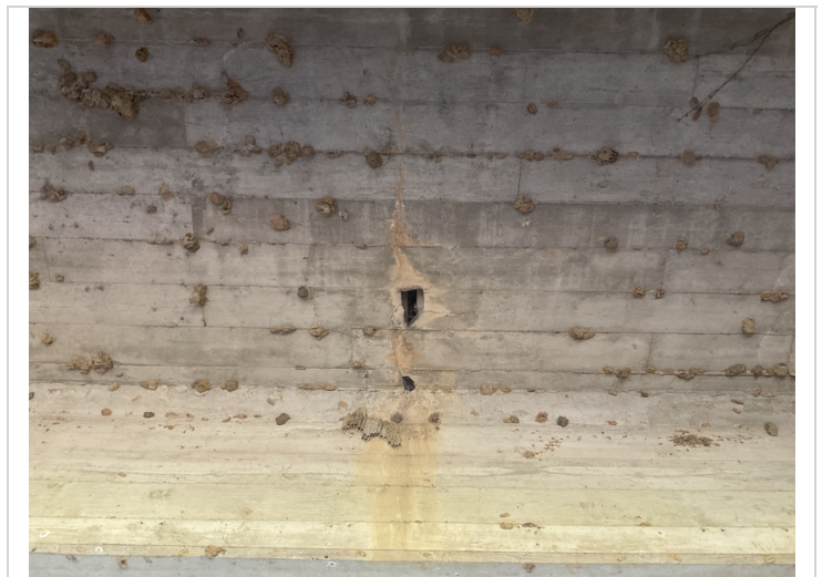
Span 2, bay 2-Void in deck undersurface
