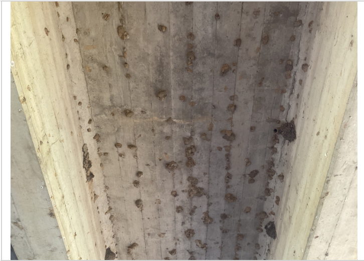
Span 2, bay 2-Transverse crack with light efflorescence
