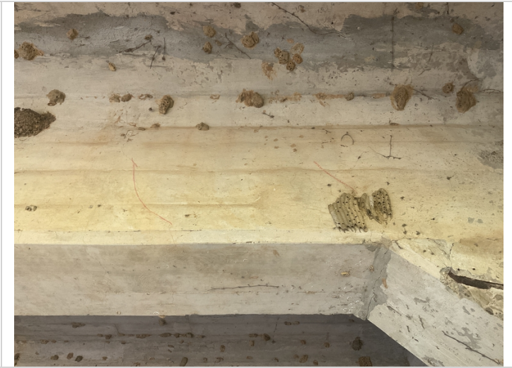
Span # 2 girder # 2 has a hairline shear type crack and spalling with exposed reinforcing steel in the beam over bent # 2.
