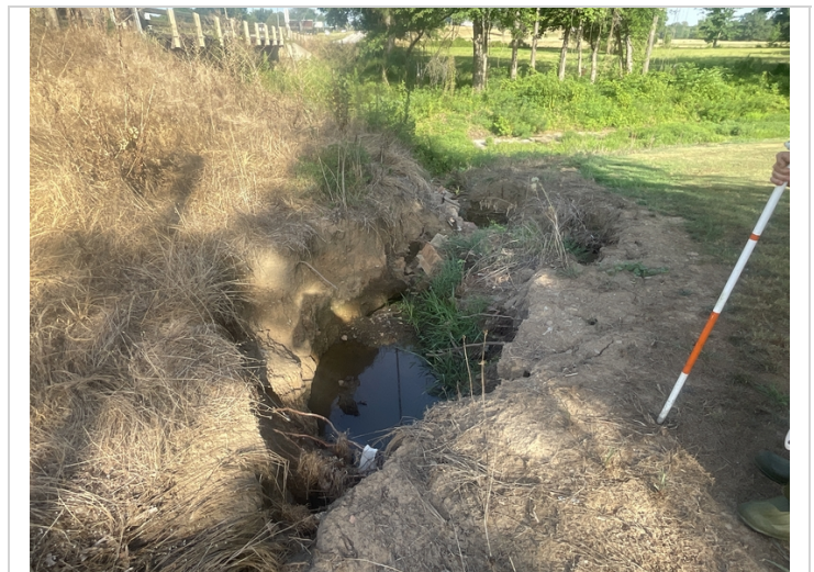
The drainage ditch on the left embankment at the East bridge end has erosion that has eroding the adjacent private property.
