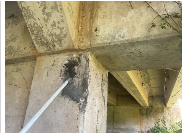
Bent 2, column 2-Repaired area
