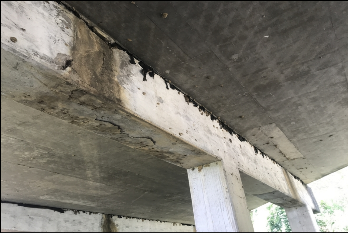
Bent #3 concrete deterioration with spalling that exposes reinforcing steel large delaminated areas on the undersurface of the cap.
