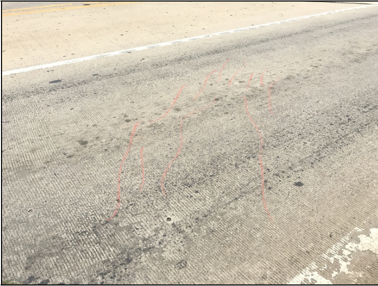
Span #3-Diagonal cracking.
