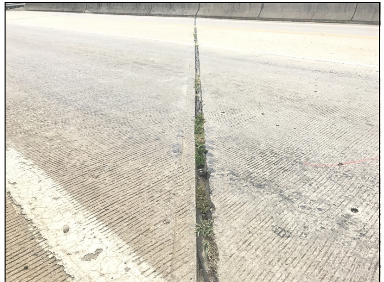
Bent #4 expansion joint seal-Adhesion failure.
