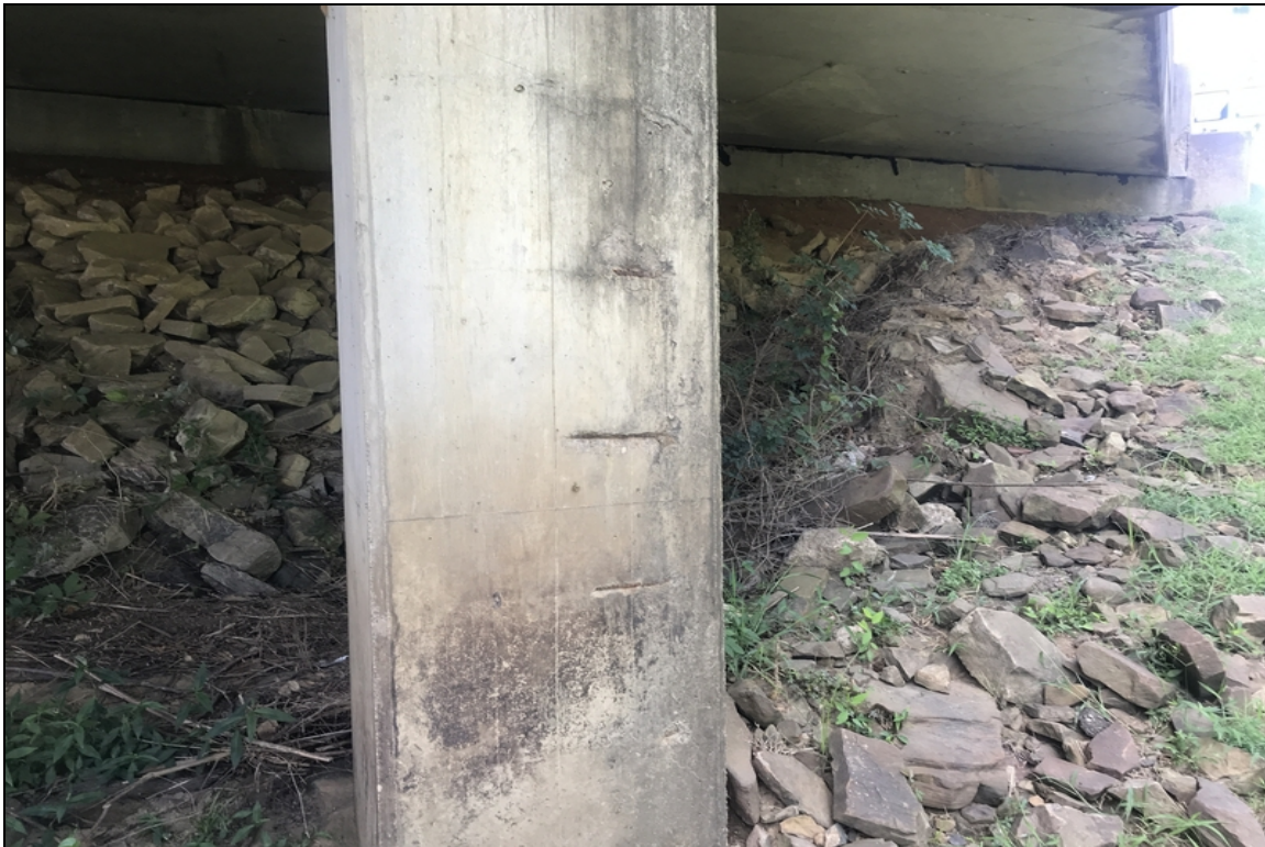
Bent #2 column #1 spalling with exposed reinforcing steel.
