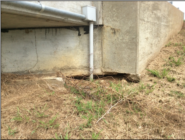
Bent # 6 Right minor settlement
