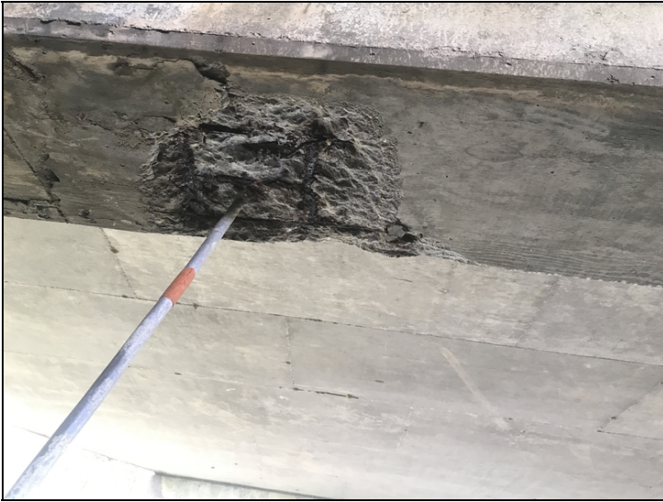
Bent #2 cap at mid-span-Spalling with exposed reinforcing steel with up to 2" of concrete section loss.
