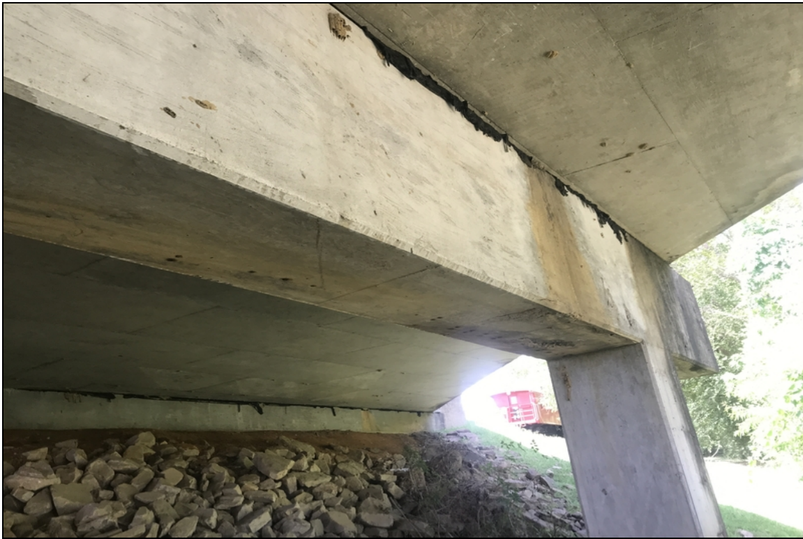
Bent #2 cap spalling and delaminated concrete.
