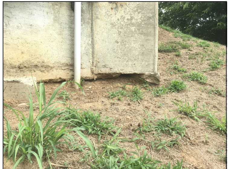
Abutment #2, right side-Minor erosion.
