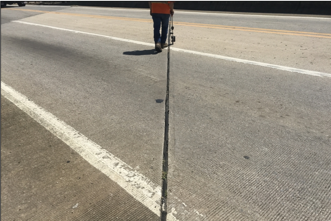
Bent #5 failing compression joint.
