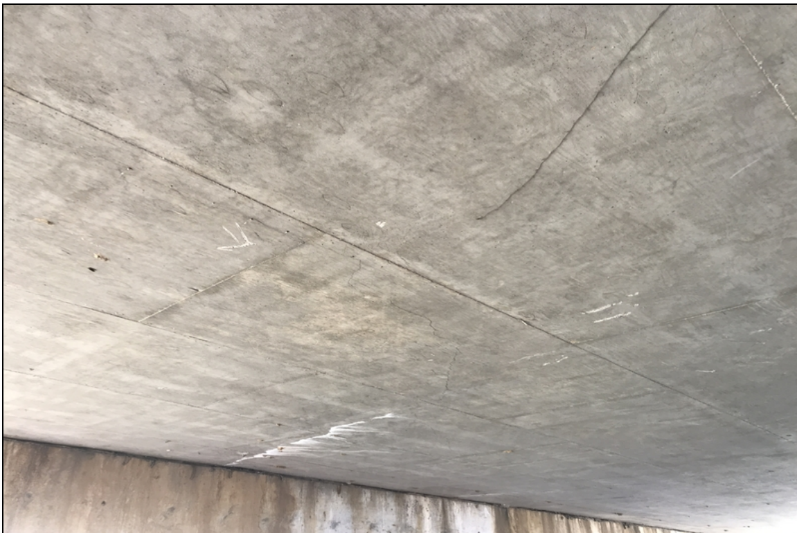
Span #4 moderate width longitudinal cracking along with cracking with efflorescence buildup.
