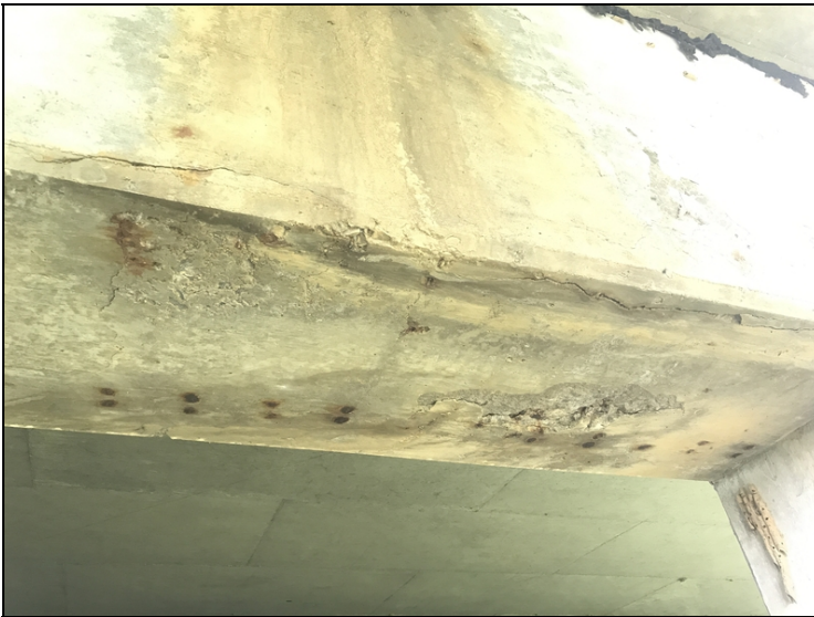
Bent #2 cap, left side-Spalling with exposed reinforcing steel with delaminated areas.
