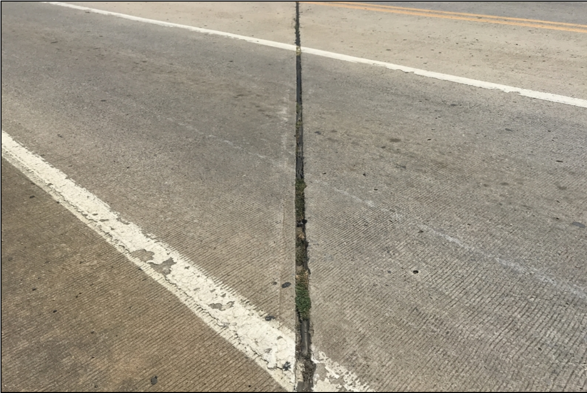
Bent #4 failing compression joint seal.
