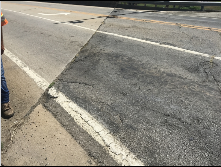
West approach asphalt breaking apart and settlement.
