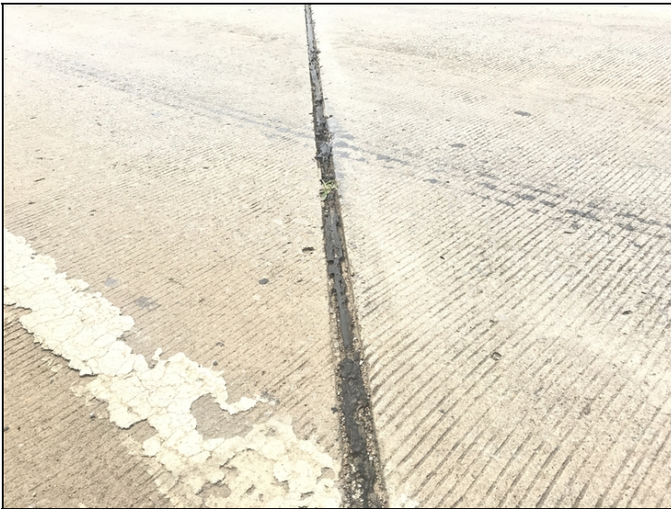
Bent #3-Adhesion failure / deteriorated joint seal.
