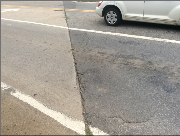
Bent # 1 Asphalt settlement at the approach
