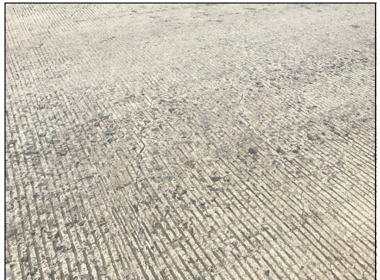
Span #4-Deck cracking perpendicular to skew angle.
