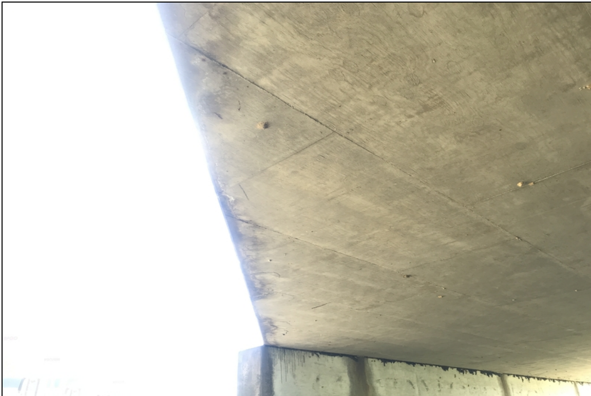
Span #4 Lt concrete delamination along the edge of the slab undersurface.
