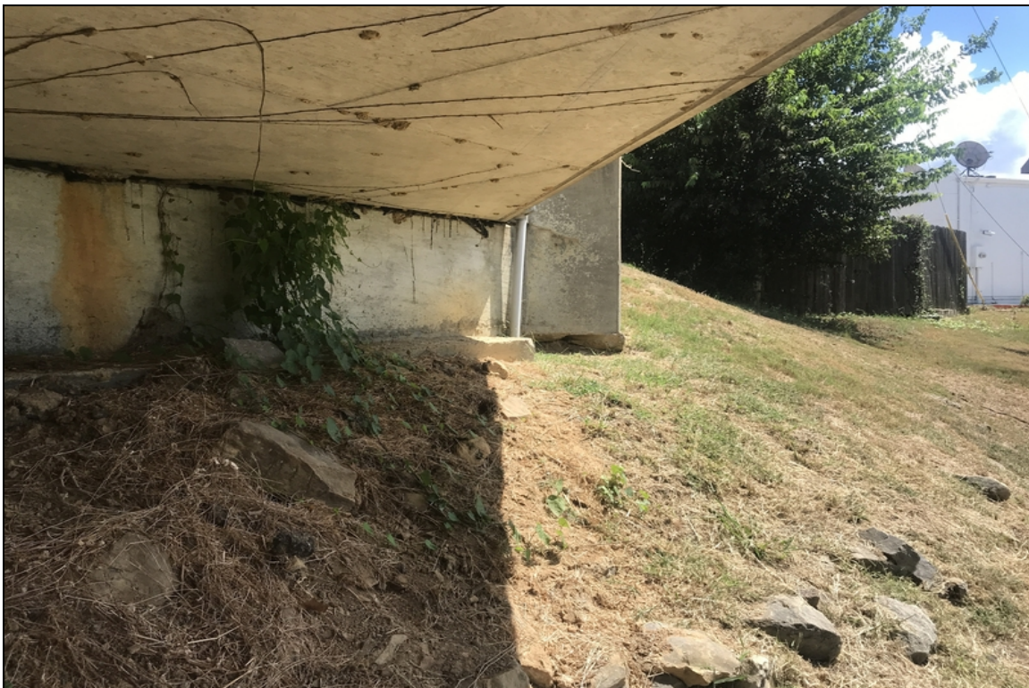
Abutment #2 Rt undermining.
