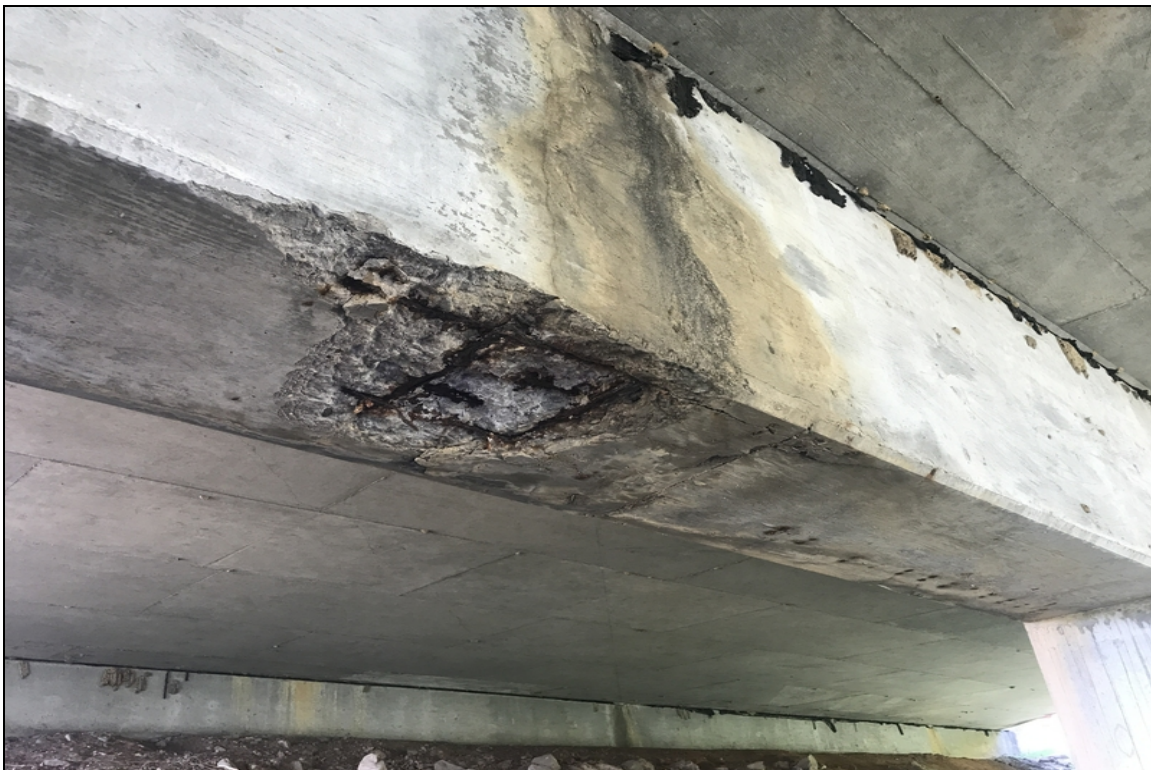
Bent #2 cap spalling with exposed reinforcing steel at centerline.
