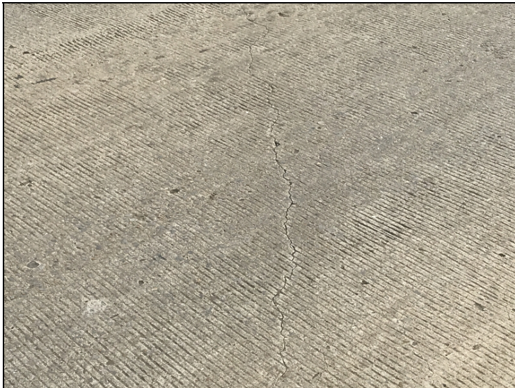
Span #3, right lane-Cracking.
