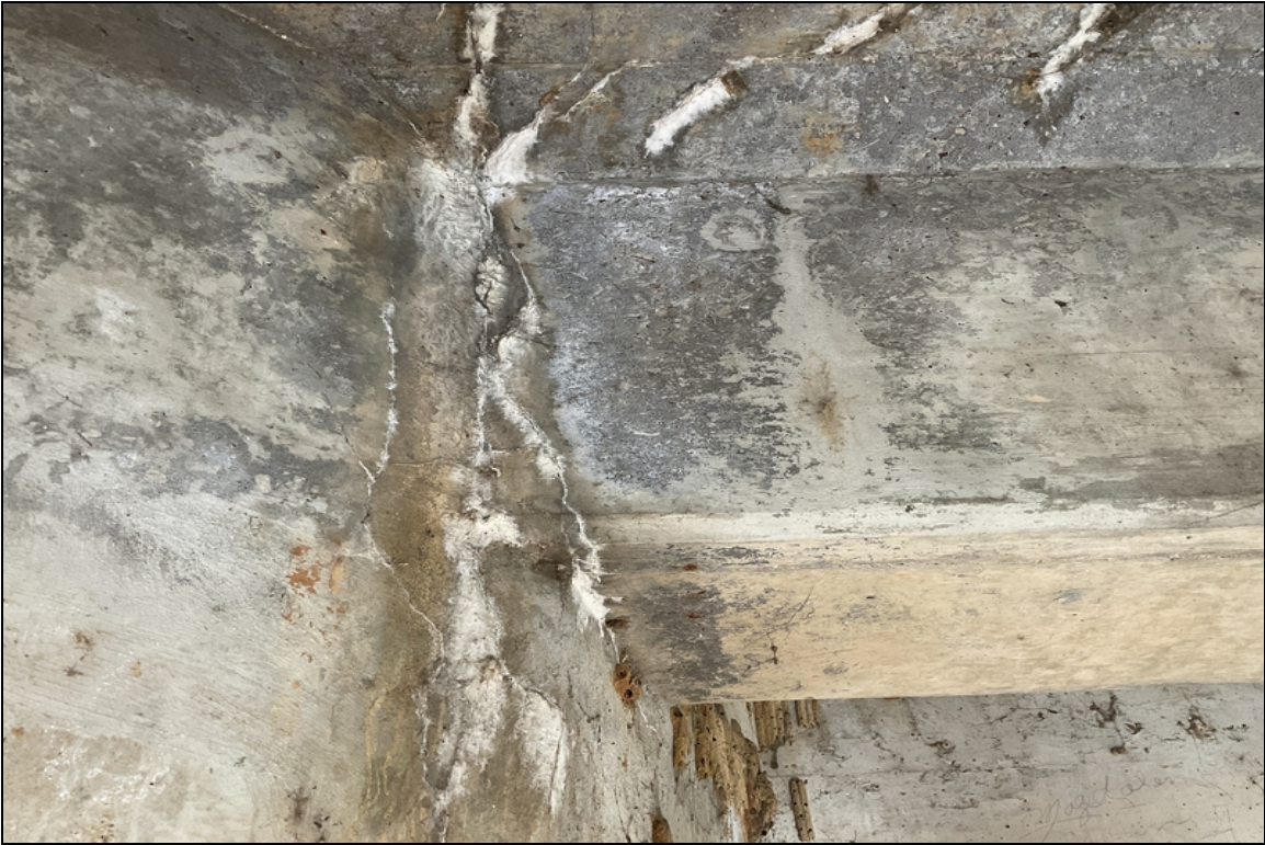
Abutment #1 beam #1 vertical crack with efflorescence buildup.
