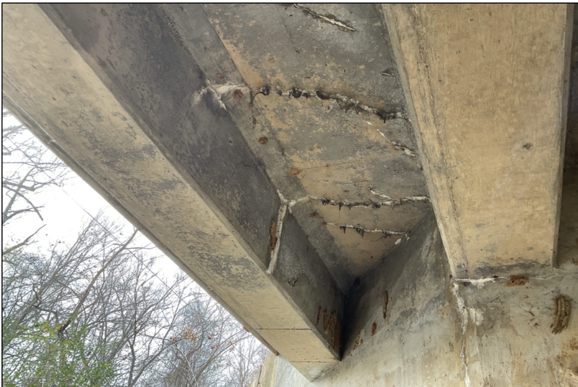
Bay #6 cracking with efflorescence buildup.
