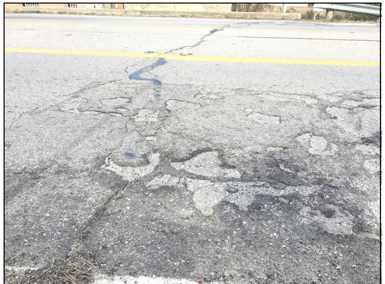
The East and West approach roadways have settlement with failing asphalt repairs at the bridge ends. East approach pictured.
