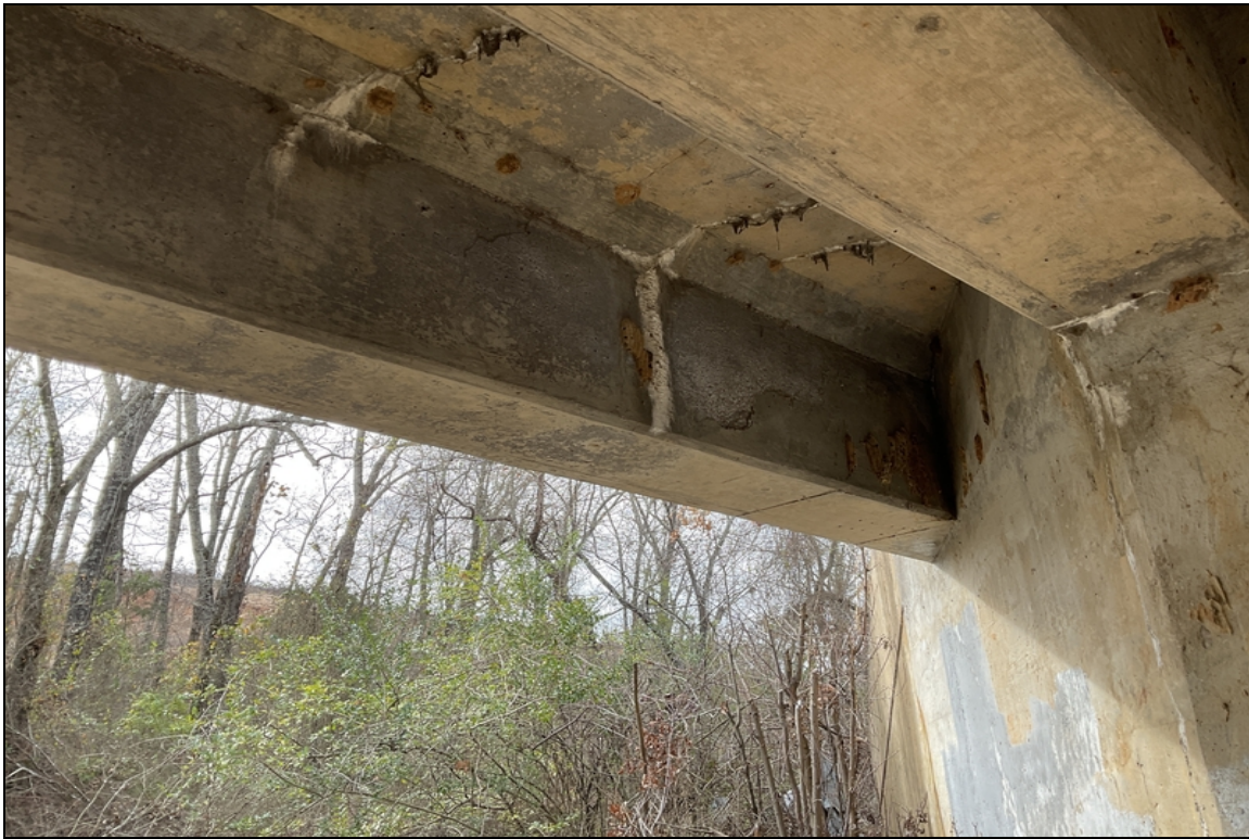
Beam #7 scaling and cracking.
