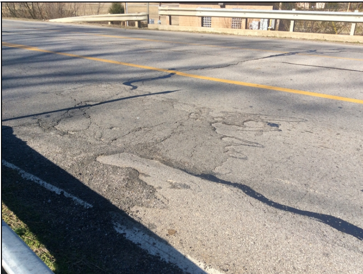
Asphalt settlement at the approaches
