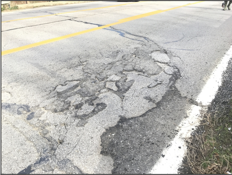
The East and West approach roadways have settlement with failing asphalt repairs at the bridge ends. West approach pictured.
