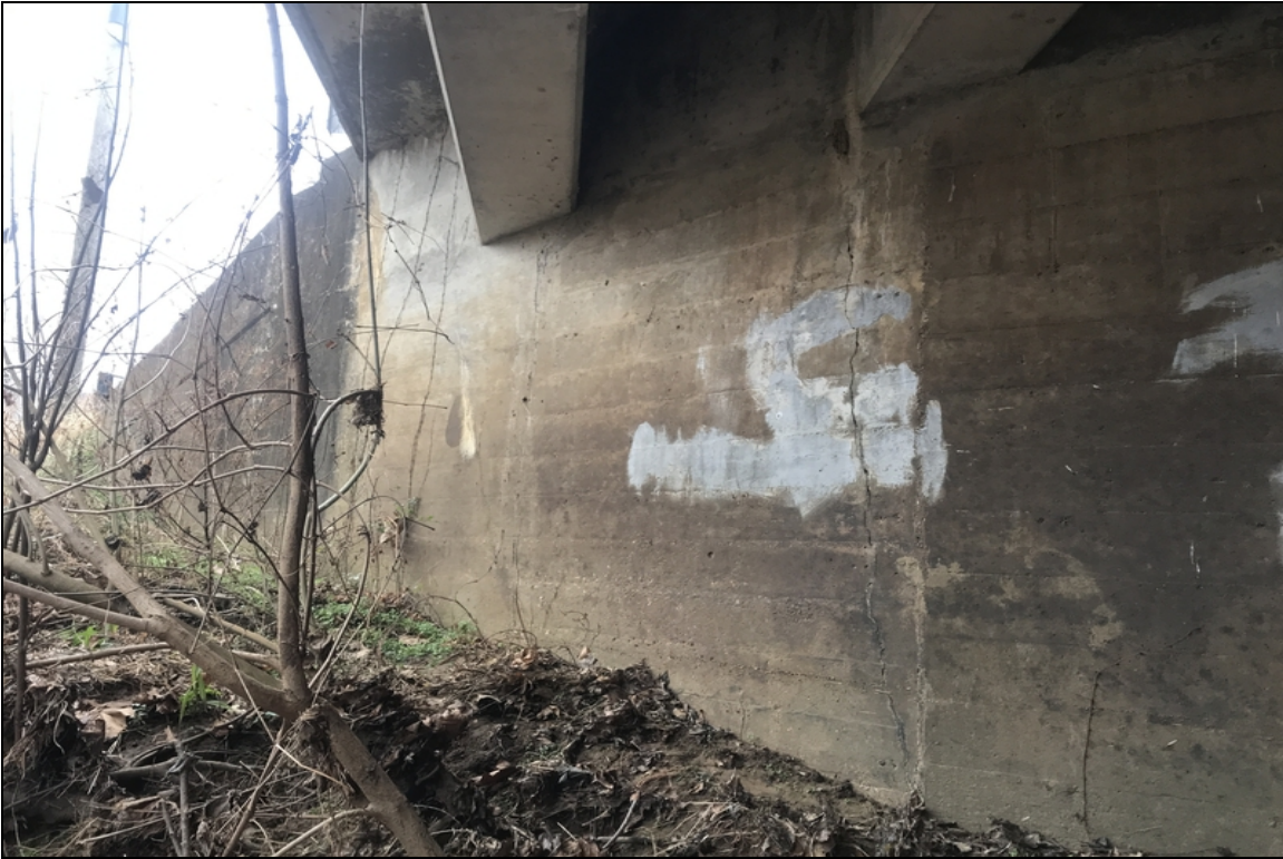
Abutment #2 Lt moderate width vertical cracking and cracking with efflorescence buildup.
