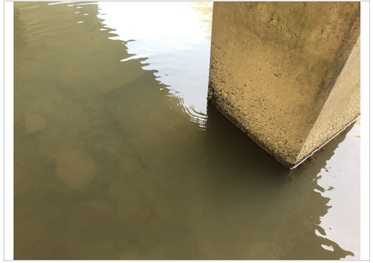
Top of footing is exposed at Bent # 3. Right column.
