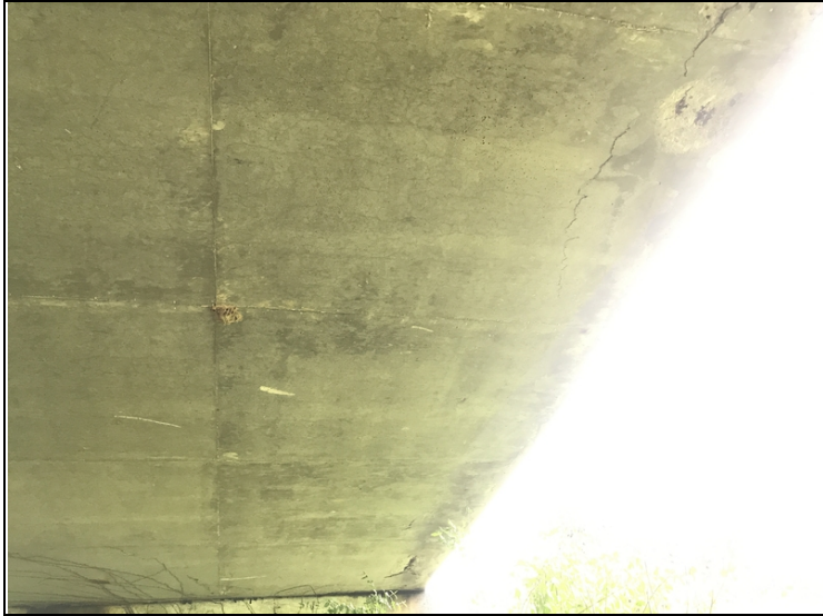
Span # 2 Left has spalling with exposed reinforcing steel.
