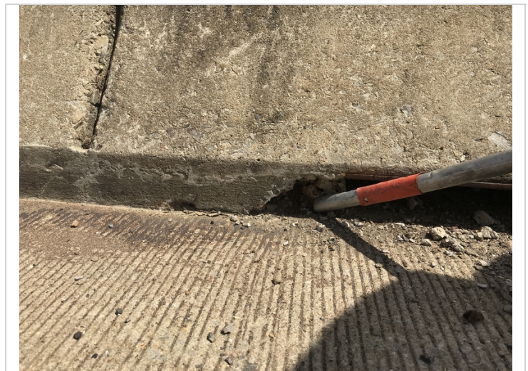
Spall with exposed reinforcing steel at the base of parapet. Span # 4. Right.
