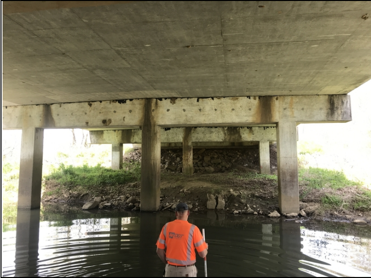
Staining on intermediate bent caps from leaking joint sealant.
