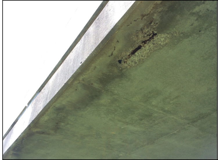
Longitudinal cracks with stains, delaminated areas, and softball sized spalls with exposed reinforcing steel visible from the undersurface of the deck, located approximately 1' from both edges of the deck. Span # 2 Left pictured.
