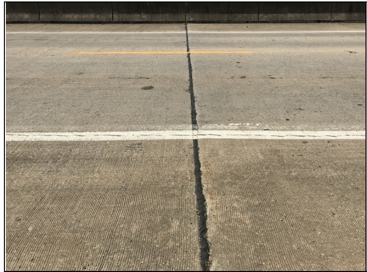
Deck joint sealant over bent # 5.
