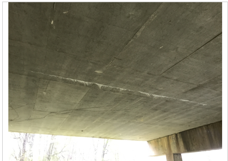
Longitudinal cracking with efflorescence in Span # 2.
