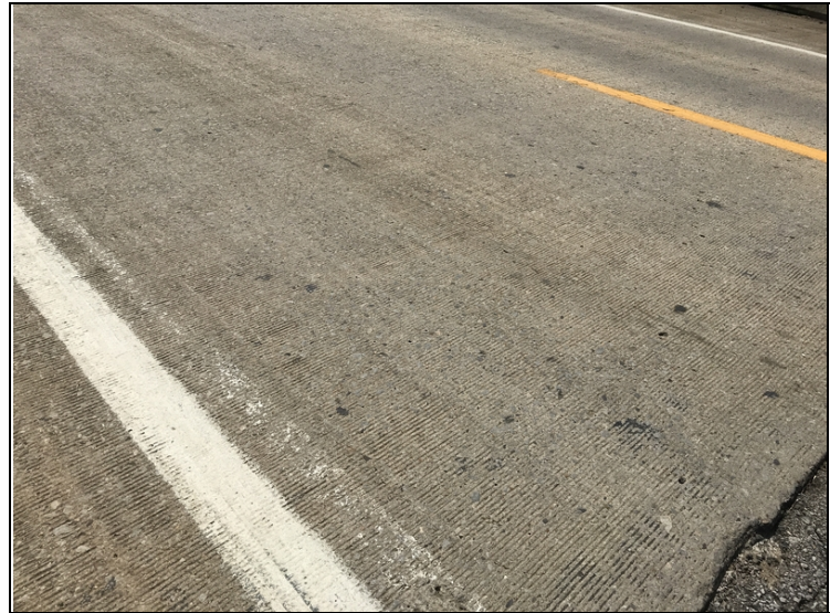
Sealable longitudinal cracking in the deck.
