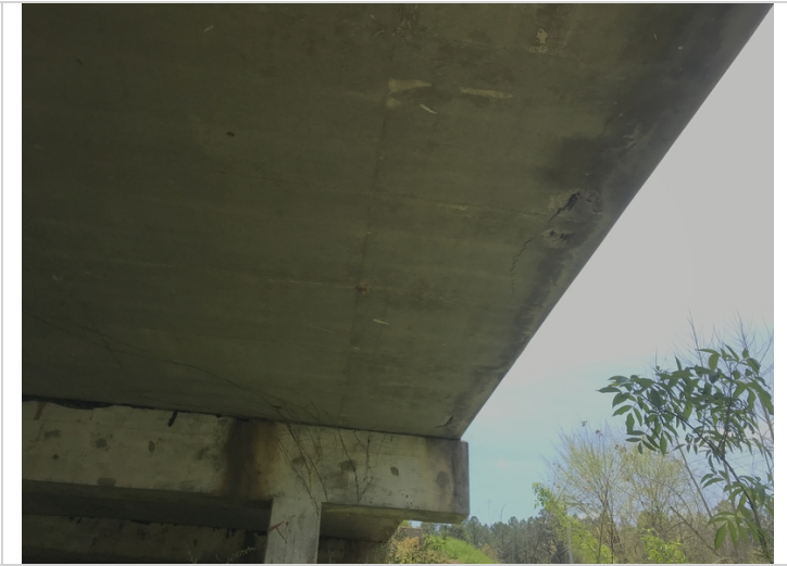
Spalls with exposed reinforcing steel in the Left edge of Span # 2.
