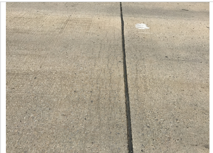
Transverse cracking in Span # 2 adjacent to Bent # 3.
