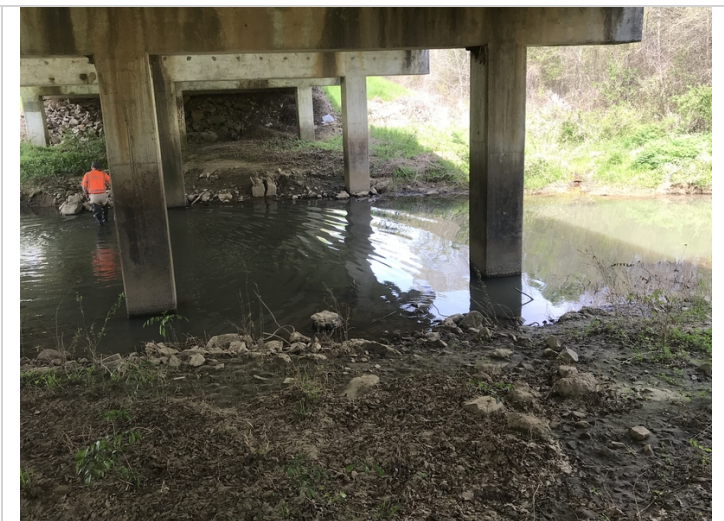
Light abrasion at the base of columns in the channel.
