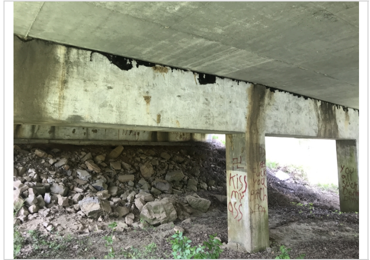
Staining in the intermediate caps from leaking joints.
