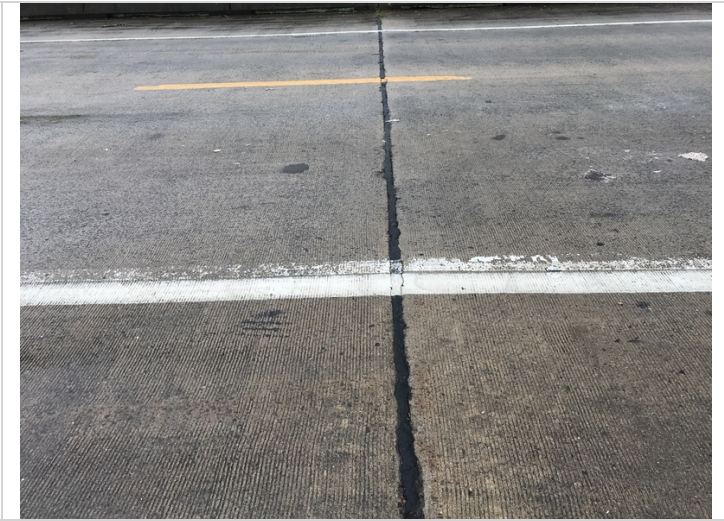
Typical joint seal.
