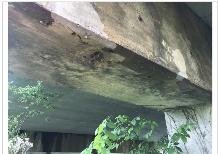
Bent # 2 Lt spalling with exposed reinforcing steel on the undersurface of the slab.
