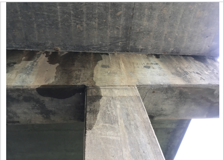
Bent # 3 Lt cap crack with efflorescence buildup.
