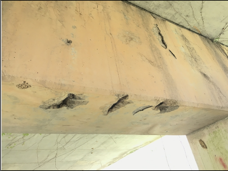
Spalls with exposed reinforcing steel in bent # 2 cap.
