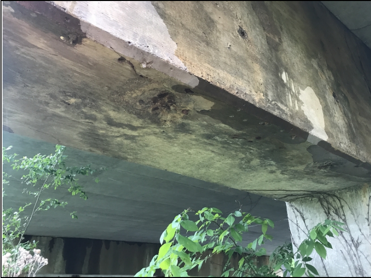
Bent # 2 Left spalling with exposed reinforcing steel on the undersurface of the slab.
