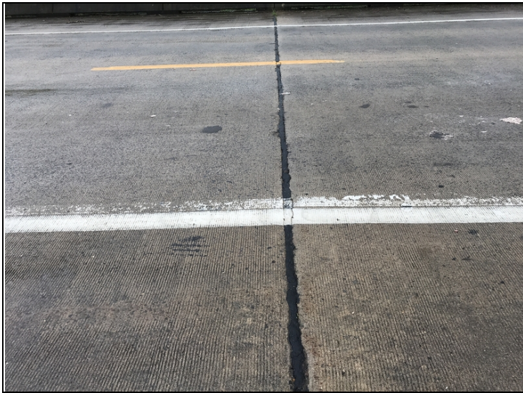
Typical joint seal.
