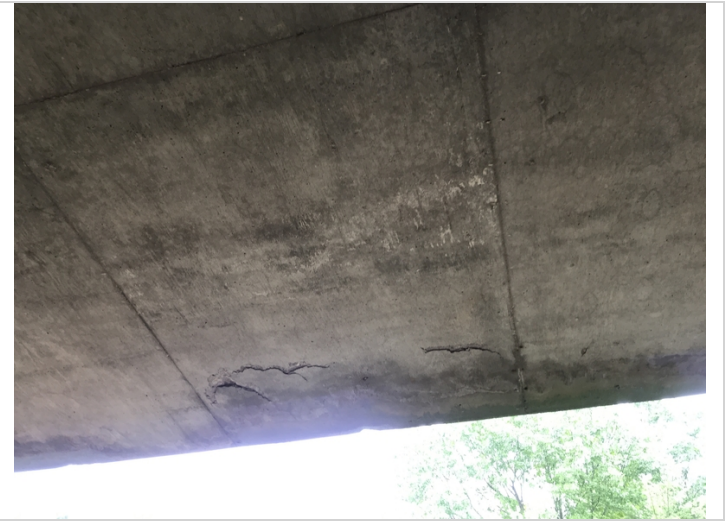
Span # 5 Rt concrete delamination along the edge of the slab.
