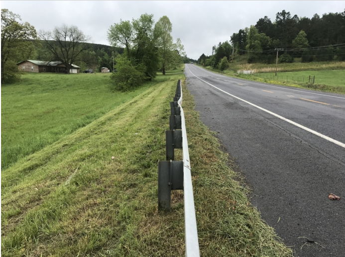
Southeast approach rail damage.
