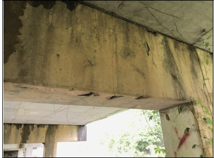
Bent # 2 spalling with exposed reinforcing steel.
