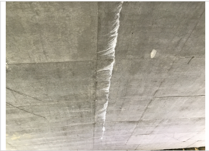
Span # 2 cracking with efflorescence on the undersurface.
