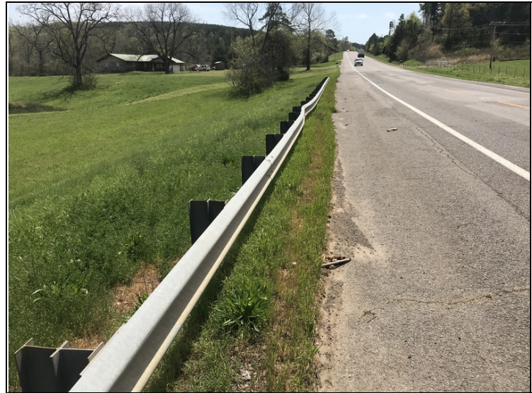
Collision damage in the southeast approach railing.
