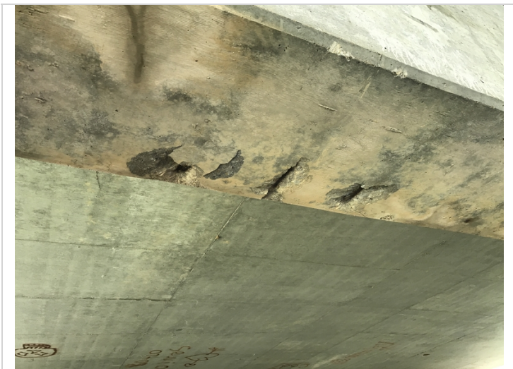
Spalls with exposed reinforcing in the undersurface of bent # 2.
