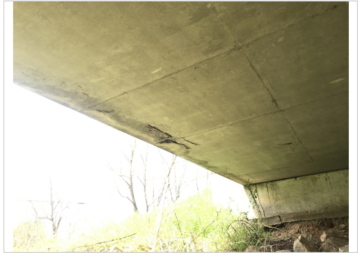
Left edge of Span # 5. Spalling with exposed reinforcing steel.
