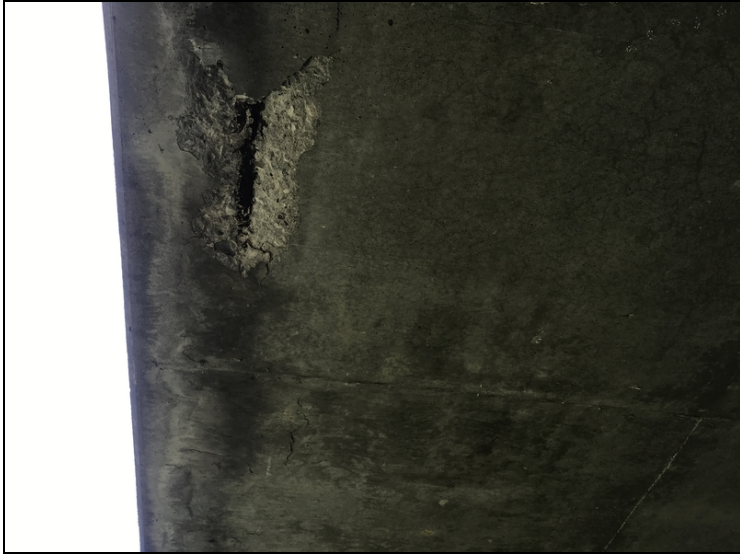
Left edge of deck soffit. Spalls with exposed reinforcing steel.
