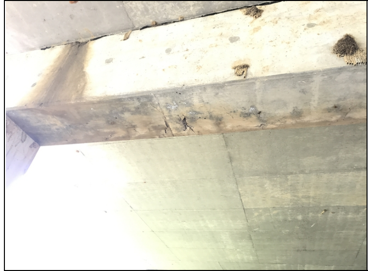
Spalls with exposed reinforcing steel in bent # 4. Left.
