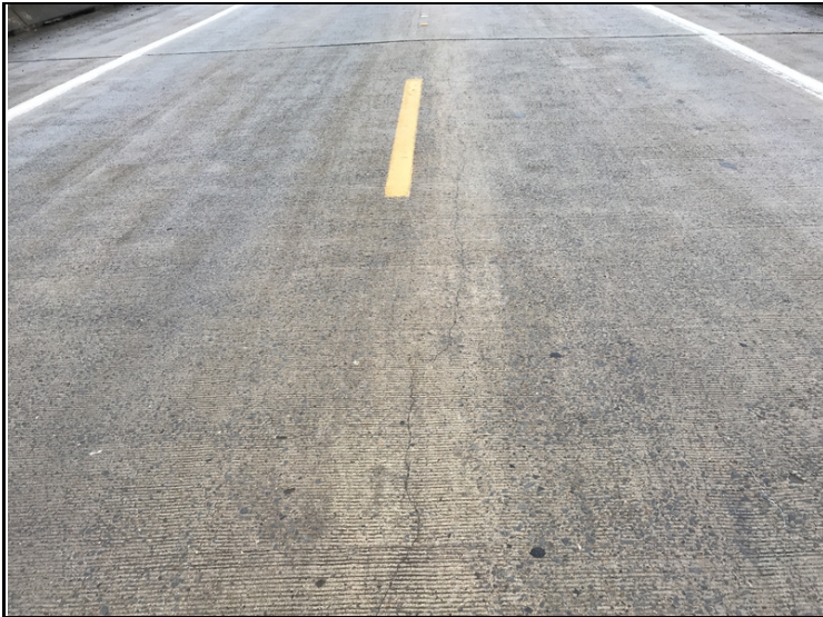
Longitudinal cracks on the driving surface of the slab.
