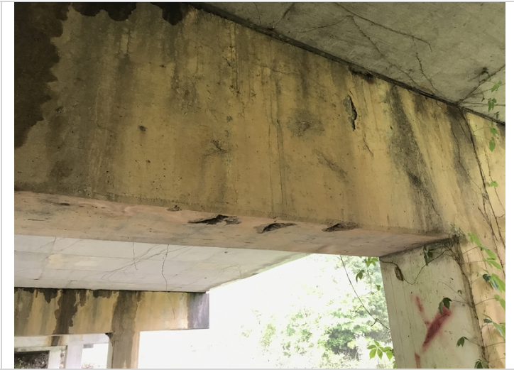
Bent # 2 spalling with exposed reinforcing steel.
