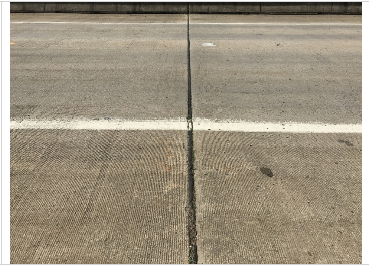
Deck joint sealant over bent # 3.
