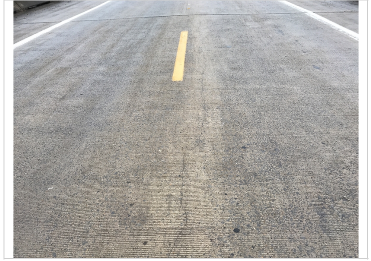
Longitudinal cracks on the driving surface of the slab.
