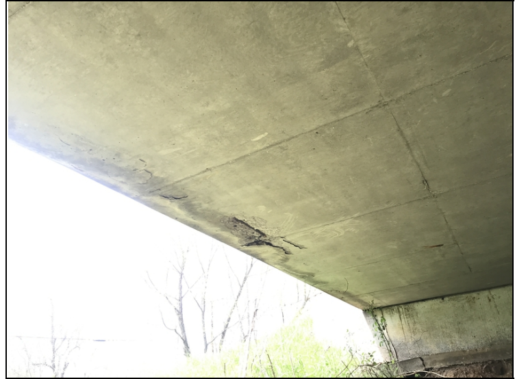
Left edge of Span # 5. Slab soffit has spalling with exposed reinforcing steel.
