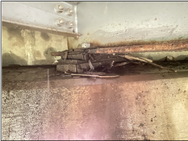
Abutment # 1, bearing # 3-Corrosion.
