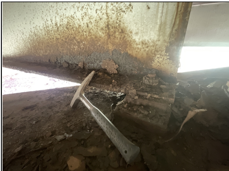
Span # 6, beam # 3 at bent # 6-Corrosion/section loss.
