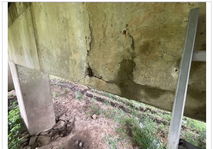
Bent 5 aheadface between columns 1 and 2-Spalling with exposed reinforcing steel
