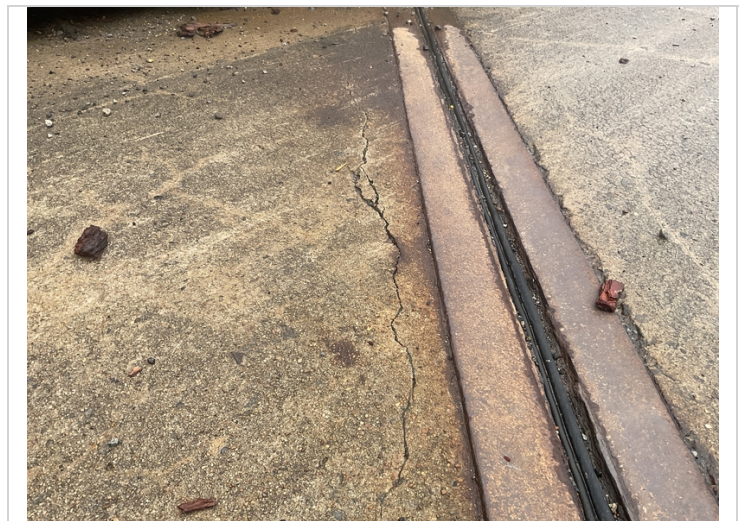
Cracking / delaminated area in left shoulder adjacent to bent expansion joint assembly
