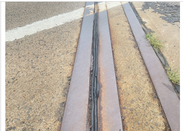
Abutment 1 expansion joint-Deterioration
