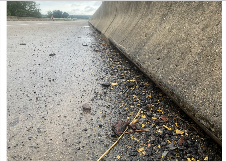
The shoulders have dirt and debris accumulation that restricts the deck drains in the parapets.
