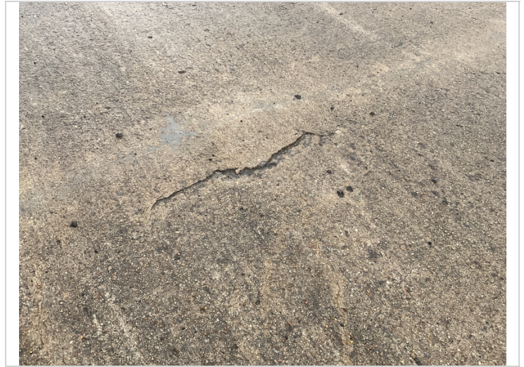
Span 1, left shoulder-Shallow delaminated area
