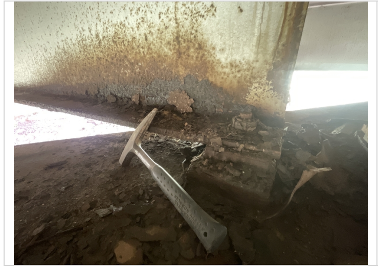
Span 6, beam 3 at bent 6-Corrosion/section loss
