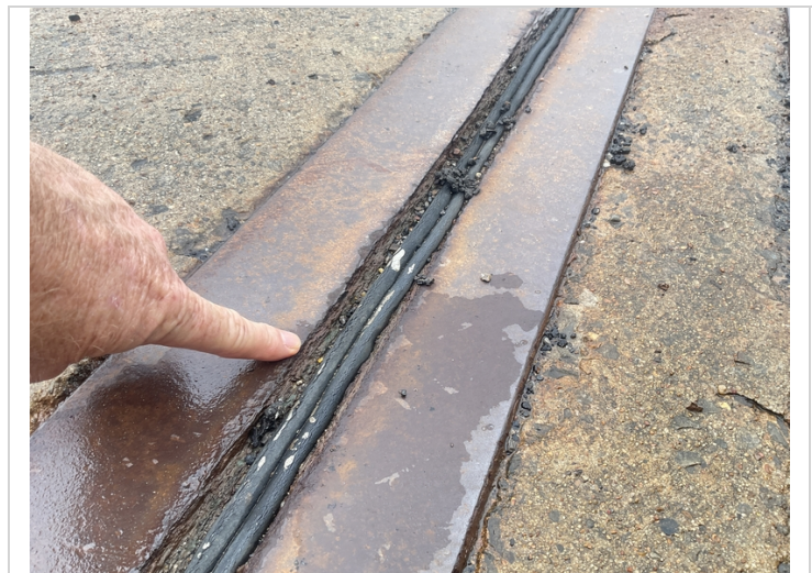
Expansion joint assemblies have corrosion with pack rust causing seal adhesion failure. Abutment 1 expansion joint pictured
