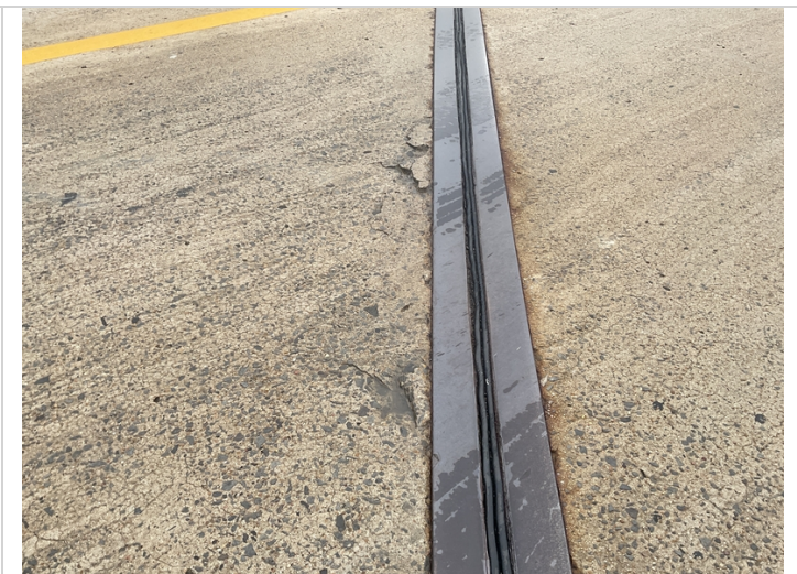
Span 2, right lane at bent 3-Delaminated/spalled area adjacent to expansion joint assembly
