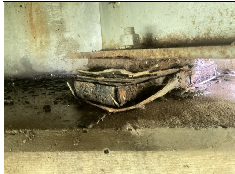
Abutment # 1, bearing # 1-Corrosion.
