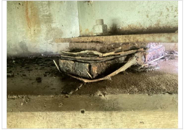
Abutment 1, bearing 1-Corrosion
