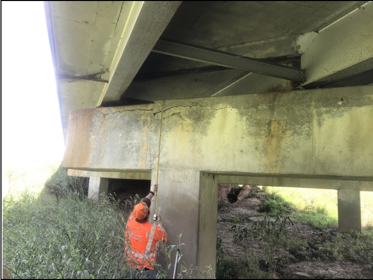
Left end of bent # 6 cap. Back face. 1/2" wide crack.
