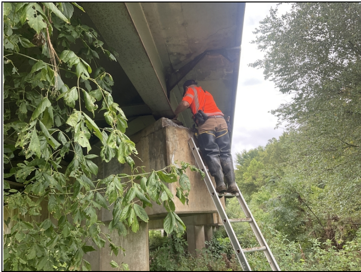
Bent # 5 cap, left end has soft and deteriorated concrete with the top of the cap spalled off outside the bearing area. The spalled area reaches the bearings but no loss of bearing area apparent at this inspection.
