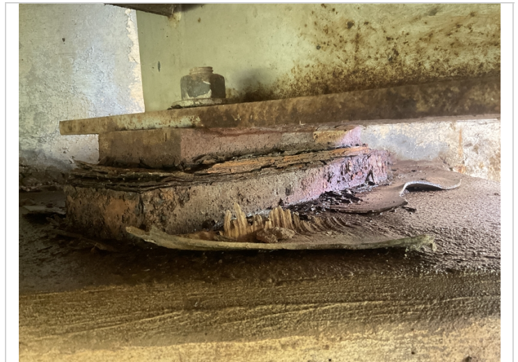
Abutment 2, bearing 6-Corrosion with pack rust between bearing plates
