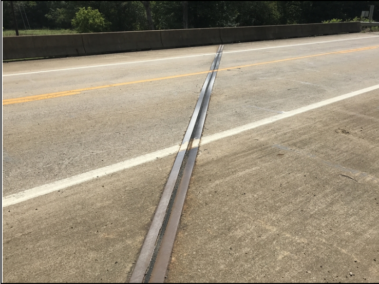
Span # 2 expansion joint seal. Typical.
