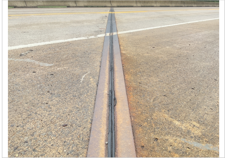
Bent 4 expansion joint-Seal deterioration
