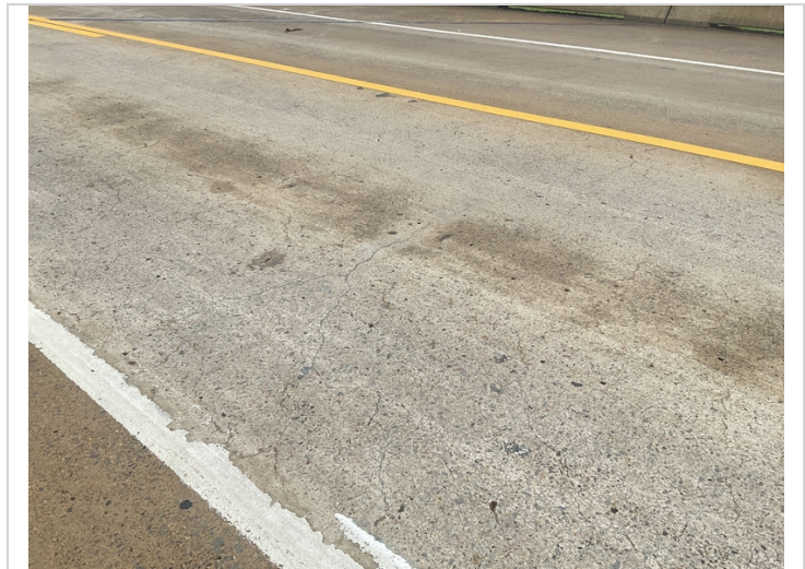
Span 3, left lane-Mapcracking
