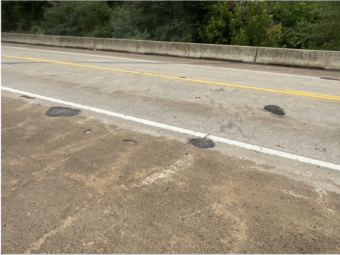
Span # 4 has several moderate sized spalls with temporary asphalt repairs.
