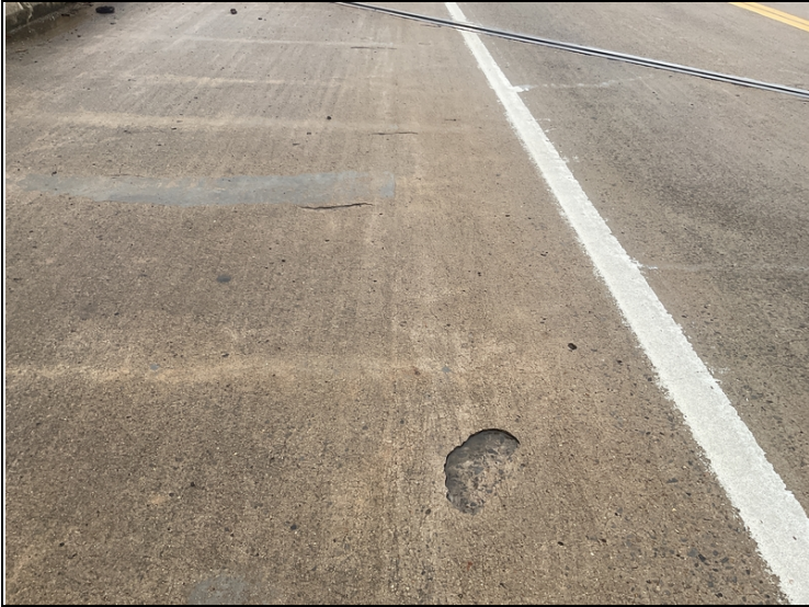
Span # 1, left shoulder-Shallow delaminated areas.
