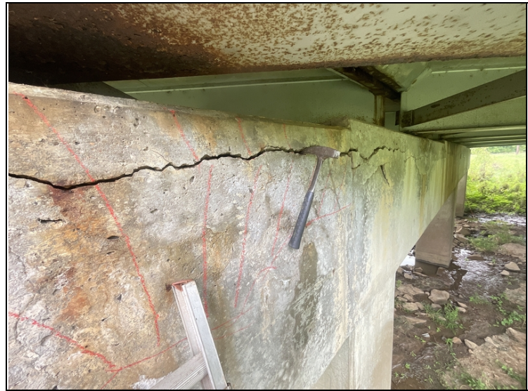
Bent # 6 cap backface, left side has 9' long delaminated area in the top and face of cap. The delaminated area appears to extend under bearing # 1 of span # 5
