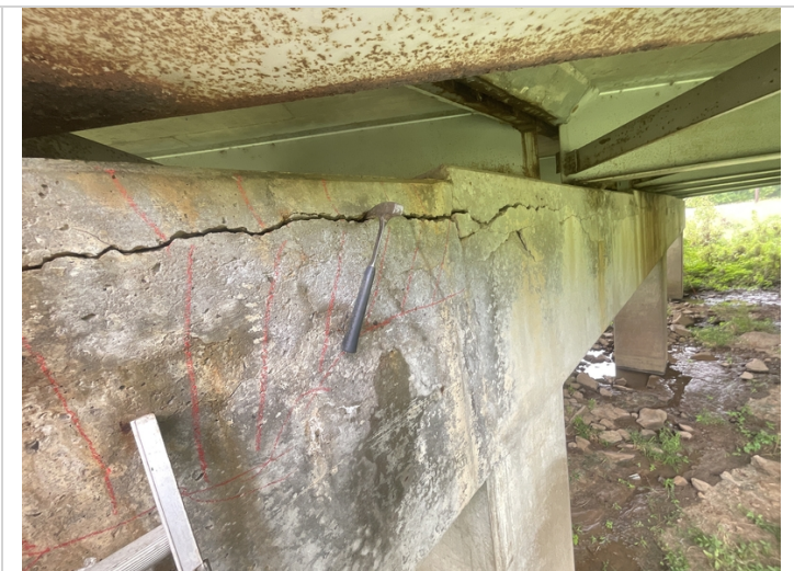
Bent # 6 cap backface, left side has 9' long delaminated area in the top and face of cap. The delaminated area appears to extend under bearing # 1 of span # 5
