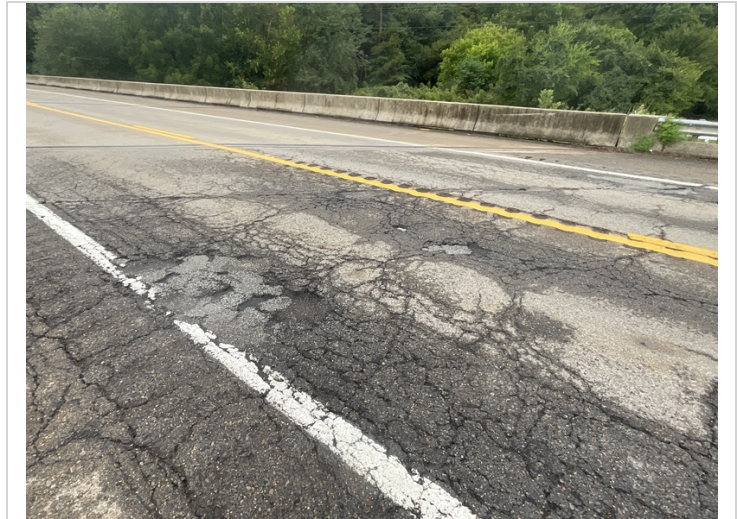
Asphalt driving surface of the North approach roadway is breaking apart with potholes forming.
