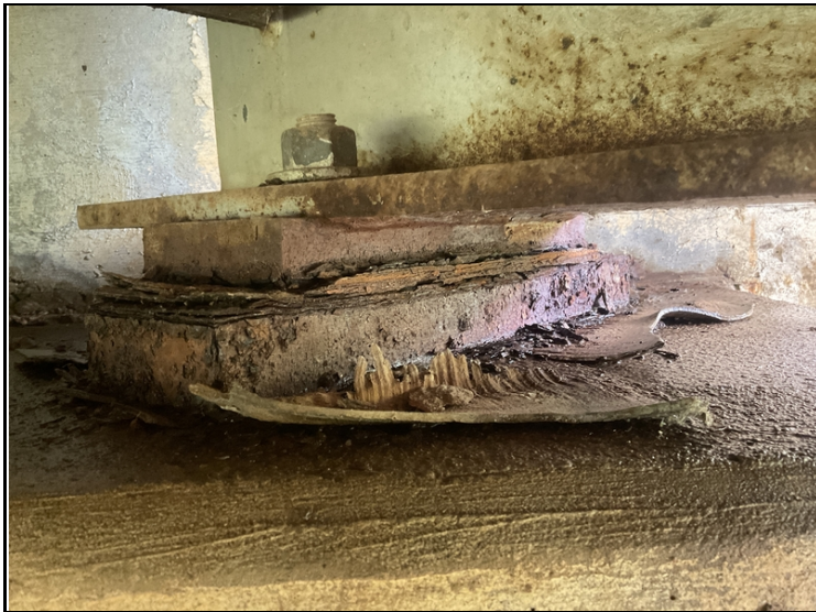
Abutment # 2, bearing # 6-Corrosion with pack rust between bearing plates.
