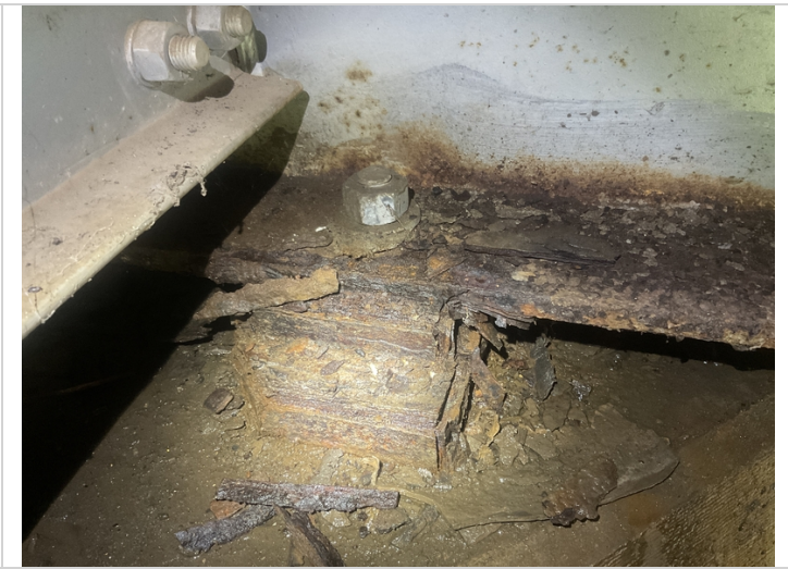
Abutment 1, beam 3-Corrosion
