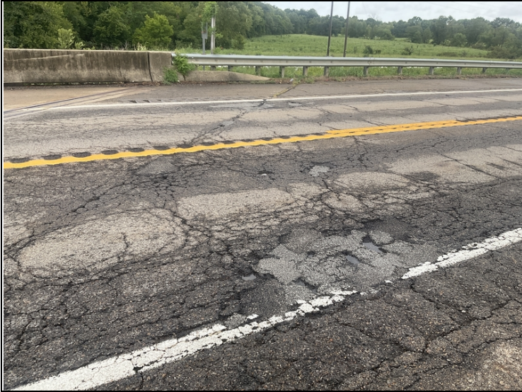
Asphalt driving surface of the North approach roadway is breaking apart with potholes forming.
