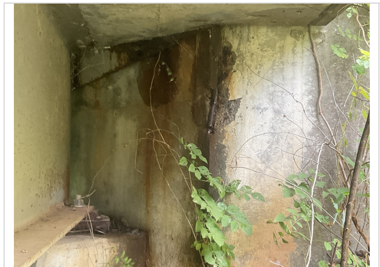
Abutment # 1 backwall left side has a 14" spall with exposed reinforcing steel at the wing wall juncture.
