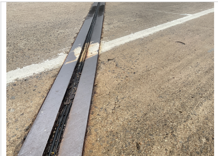
Span 2, left shoulder-Delaminated area adjacent to bent expansion joint assembly
