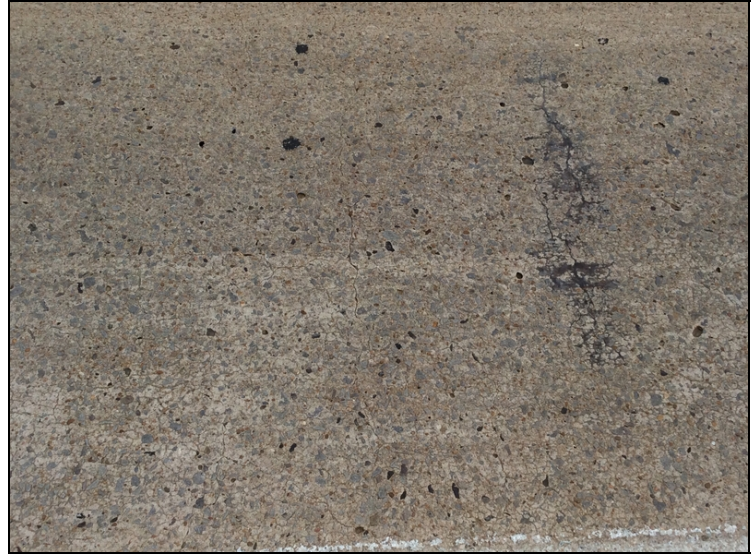
The driving surface of the deck has numerous areas of unsealed mapcracking in all spans.
