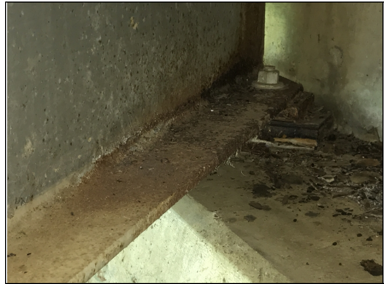
Beams have areas of active corrosion with flaking rust at the ends of beams where the expansion joint seals leak water on the superstructure. There is up to approximately 1/8" section loss to the base of webs and bottom flanges.
