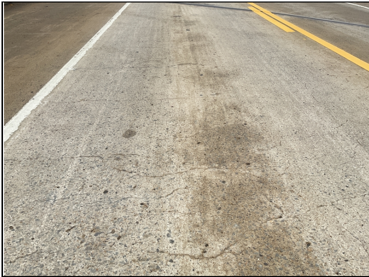
Span # 3, left lane-Mapcracking.
