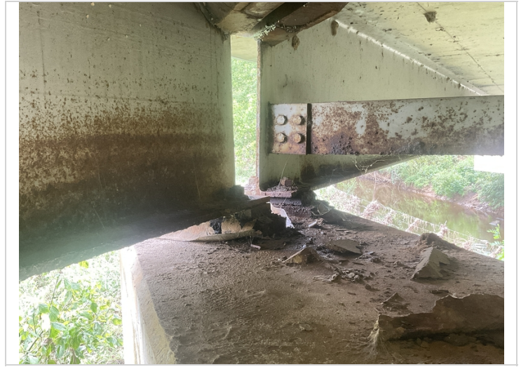
Beam 6 over bent 5-Corrosion
