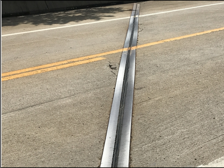
Bent # 3 expansion joint.
