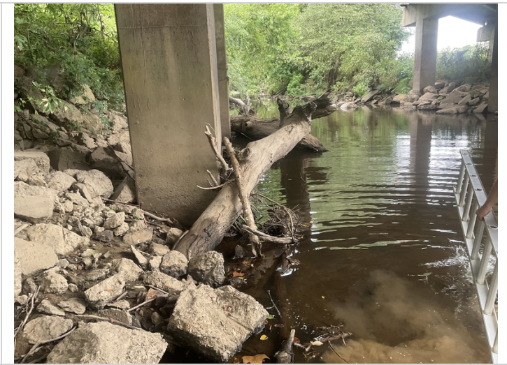
Drift at bent # 3
