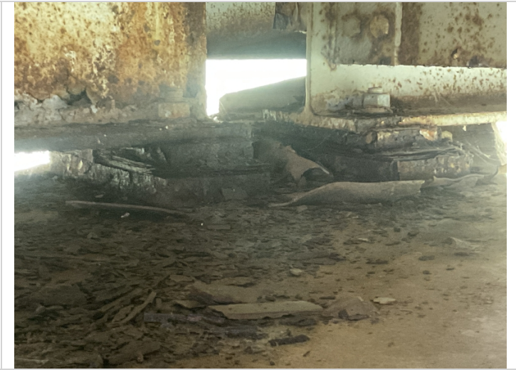
Bent 6-Heavy corrosion to bearing devices
