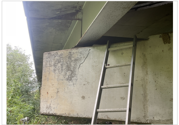
Bent 2 backface, left side-Delaminated area
