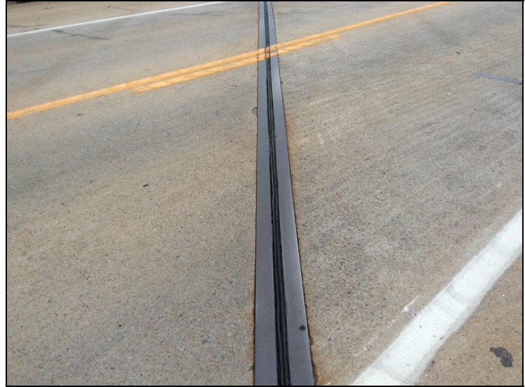
Bent # 7 joint seal condition.
