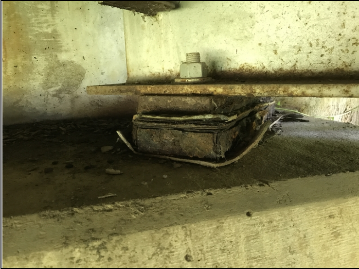
Bearings have active corrosion with flaking rust and heavy pack rust between the sole and masonry plates.
