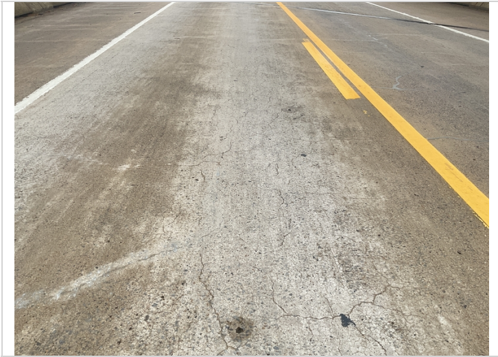
Span 1, left lane-Mapcracking
