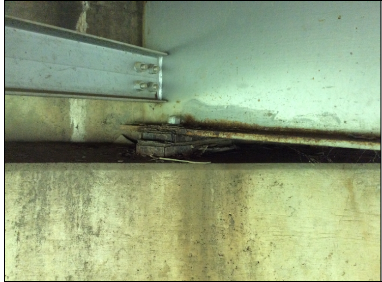
Active corrosion at the beam ends from water leakage through the expansion joints.
