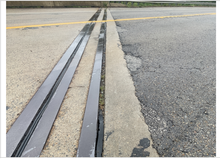
Joint sealant deteriorated and missing in locations between abutment # 1 expansion joint assembly and South approach roadway.
