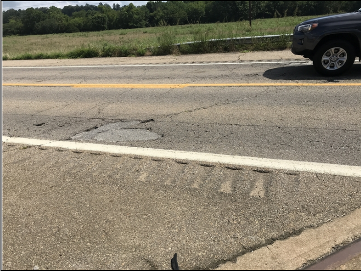
The asphalt driving surface of the North approach roadway is breaking apart with potholes forming.
