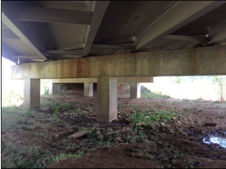
Water stains in the intermediate bents from water leakage through the deck joints.
