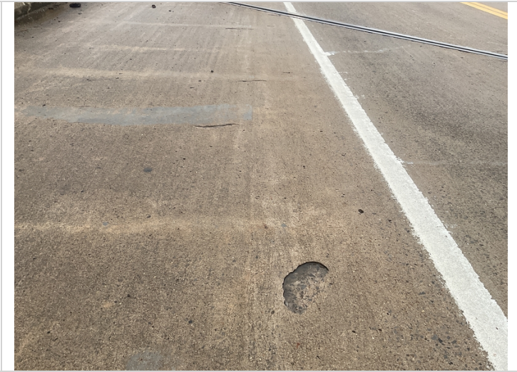
Span 1, left shoulder-Shallow delaminated areas
