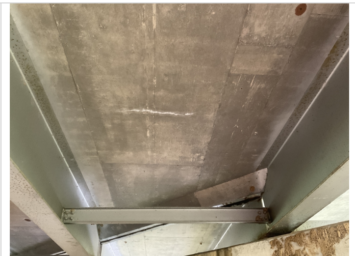
Span 1, bay 4-Transverse crack with efflorescence
