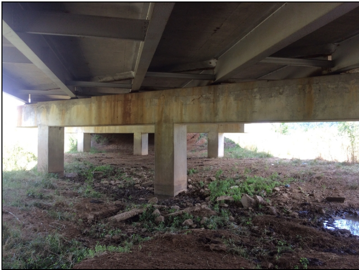
Freckled rust typical on the paint system.
