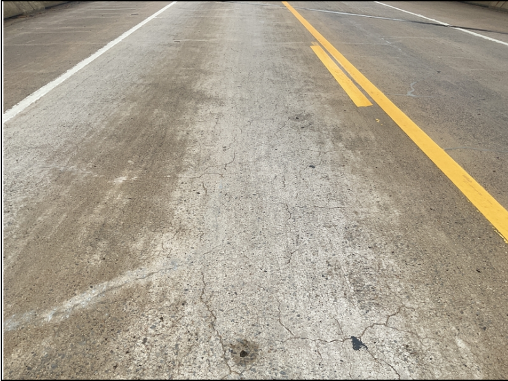
Span # 1, left lane-Mapcracking.
