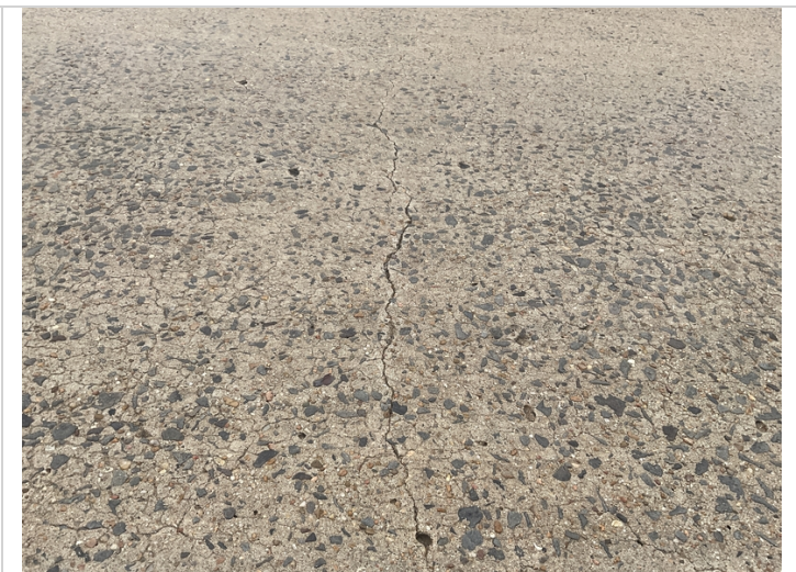
Span 1, left lane-Transverse cracking
