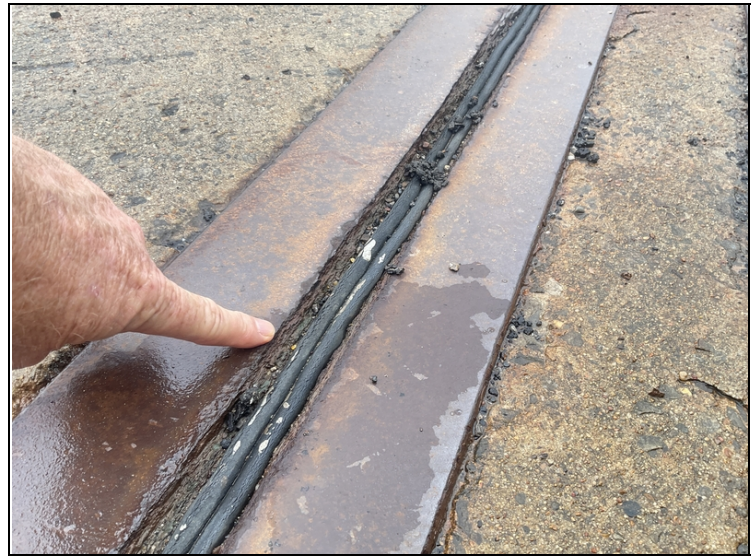
Expansion joint assemblies have corrosion with pack rust separating the seals from the assemblies. Abutment # 1 expansion joint pictured.
