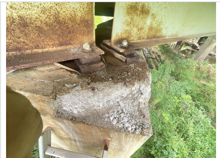
Bent # 5 cap, left end has soft and deteriorated concrete with spalling.
