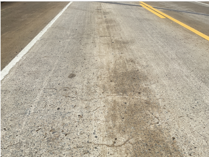
Span 3, left lane-Mapcracking
