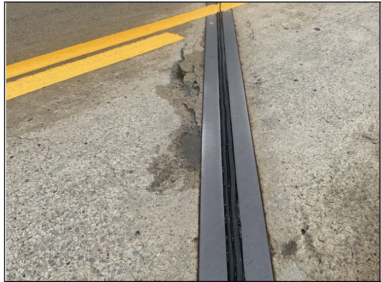
Span # 3, left lane-Spalling adjacent to expansion joint assembly.
