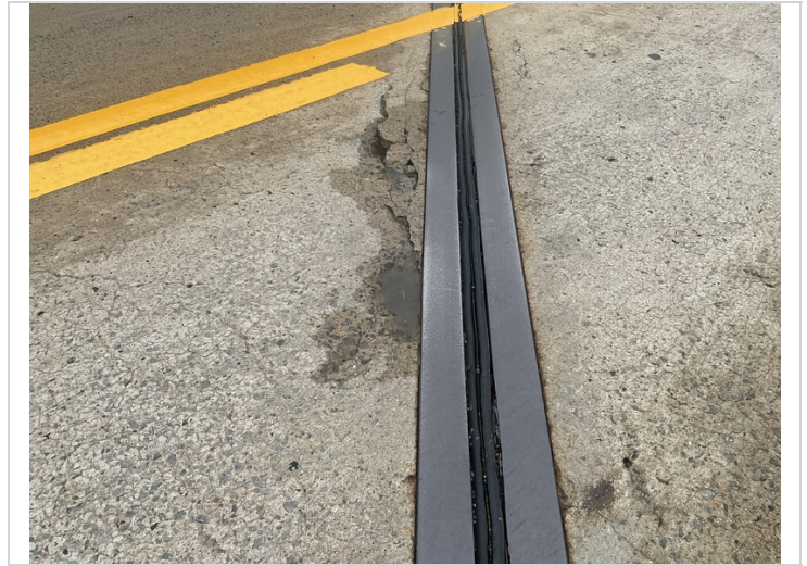
Span 3, left lane-Spalling adjacent to expansion joint assembly
