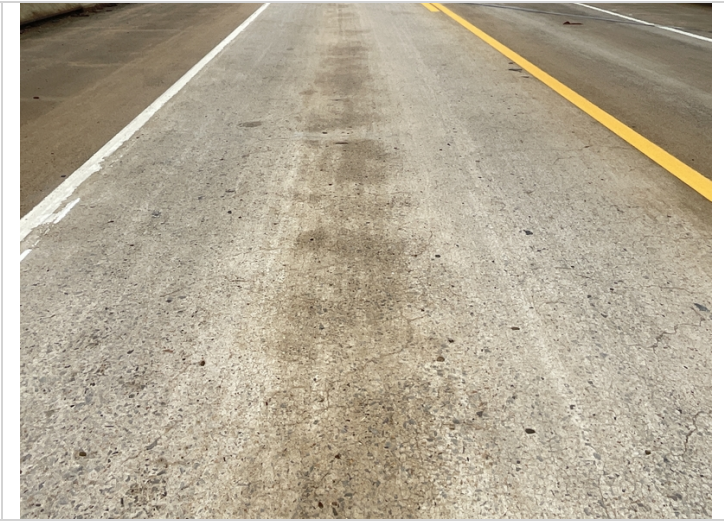
Span 3, left lane-Mapcracking
