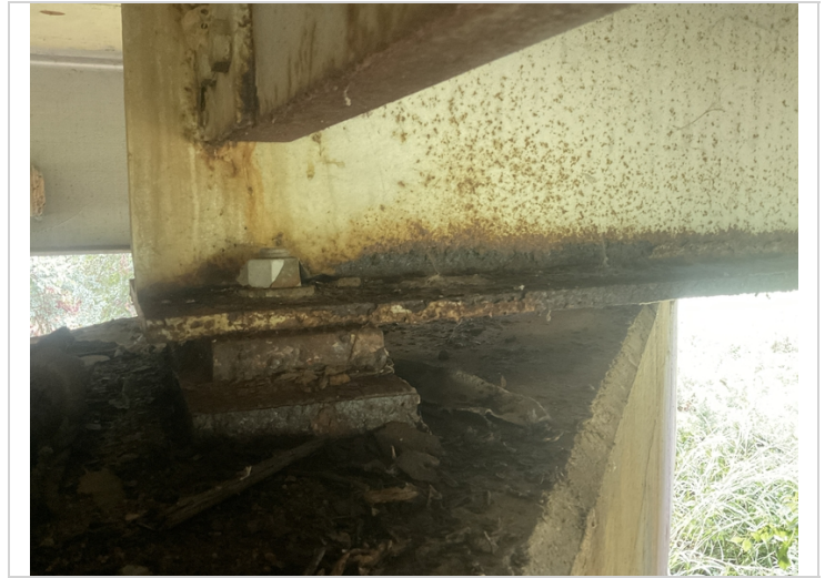
Span 5, beam 2 at bent 5-Corrosion to beam end and bearing device
