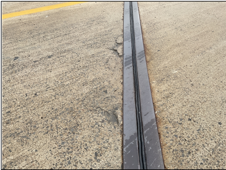
Span # 2, right lane at bent # 3- Delaminated/spalled area adjacent to expansion joint assembly.
