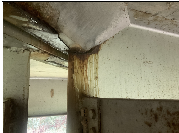
Span # 5, beam # 2 at bent # 5-Corrosion to web at expansion dam.
