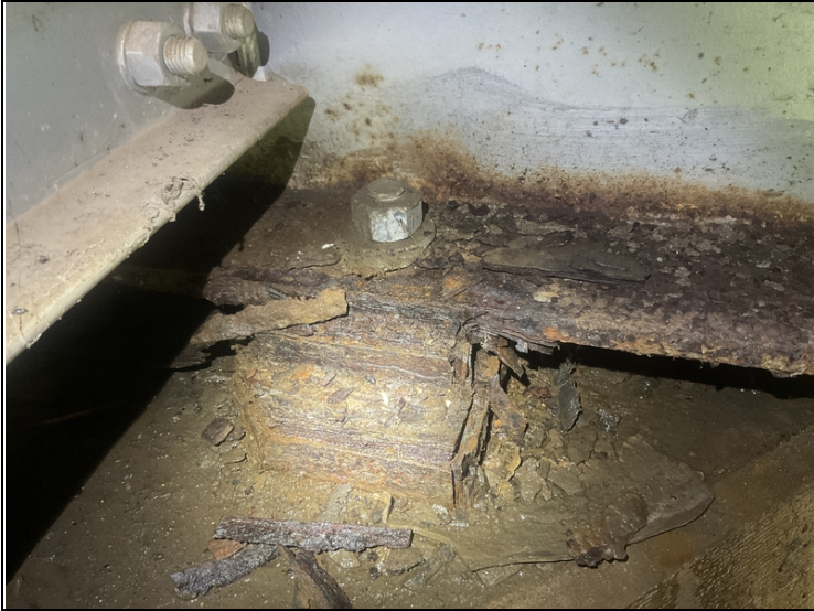
Abutment # 1, beam # 3-Corrosion.
