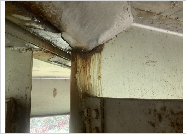
Span 5, beam 2 at bent 5-Corrosion to web at expansion dam
