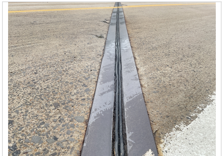
Bent 3 expansion joint-Seal deterioration
