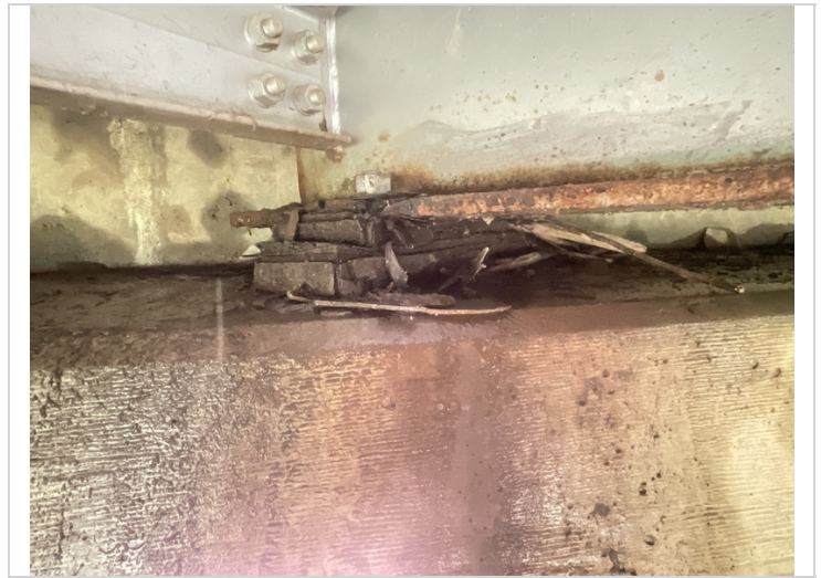
Abutment 1, bearing 3-Corrosion
