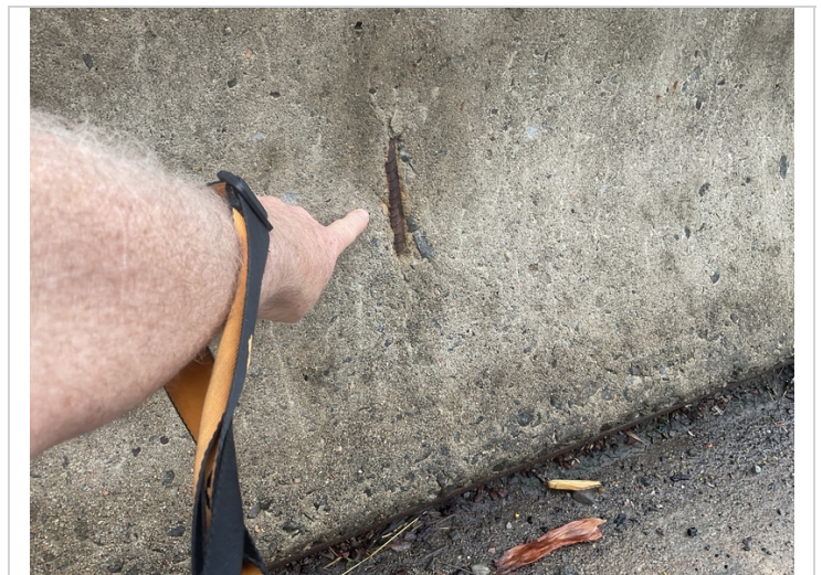
Span 1, left parapet-Shallow spall with exposed reinforcing steel
