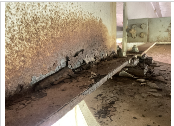
Span 6, beam 4 at bent 7-Corrosion with flaking rust
