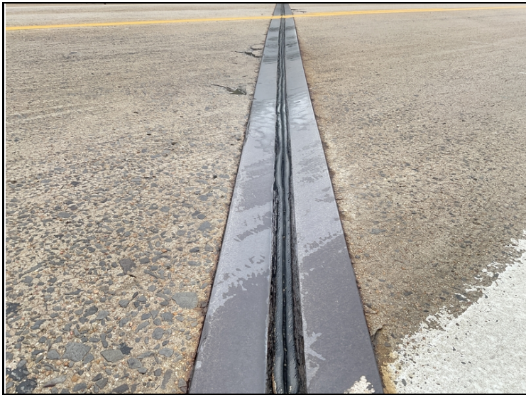
Bent # 3 expansion joint-Seal deterioration.
