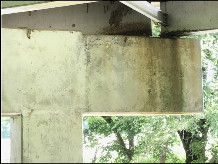
Horizontal cracking in the a right side of bent # 3. Back face.
