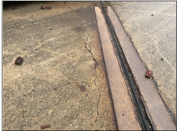
Cracking / delaminated area in left shoulder adjacent to bent # 2 expansion joint assembly.
