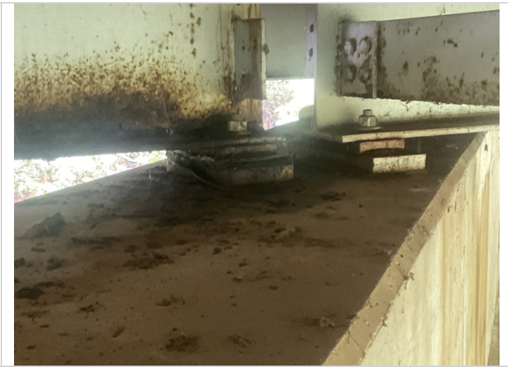
Span 2, beam 3 at bent 2-Corrosion
