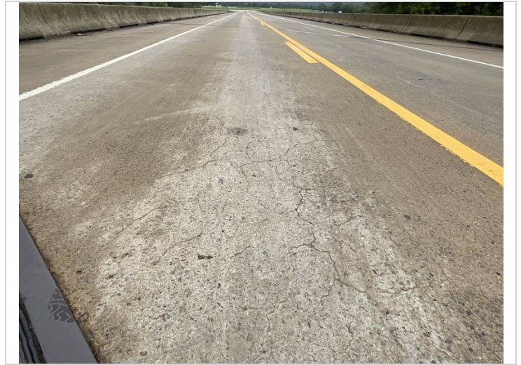
Span 1, left lane-Mapcracking
