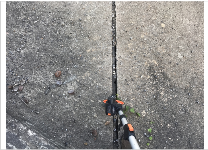
Seal adhesion failure.
