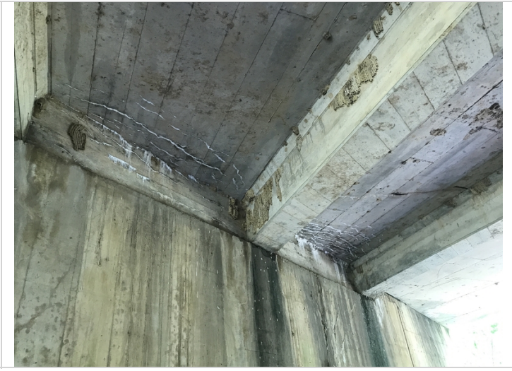
Span 2 cracking with efflorescence buildup.
