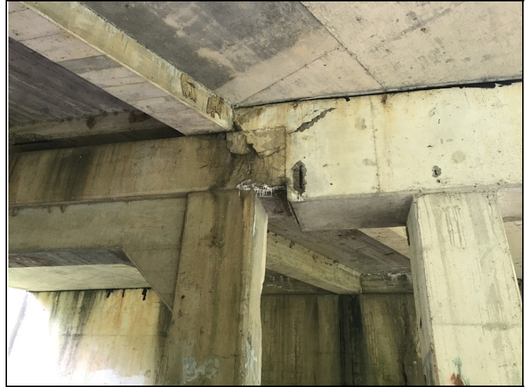
Span # 1 side of Bent # 2 cap. Spall with exposed reinforcing steel and delaminated areas.
