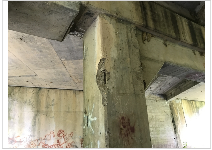
Bent 2 Column 4 spalling with exposed reinforcing steel.
