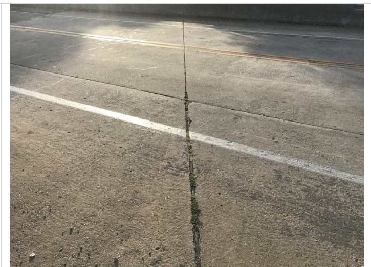
Failing joint sealant.
