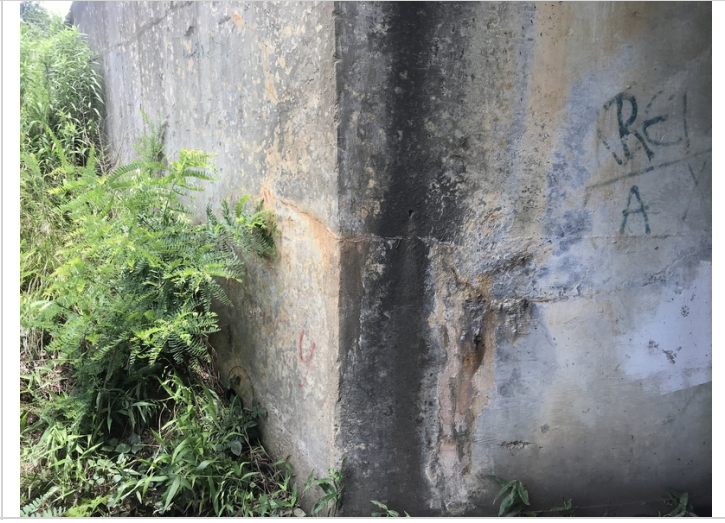
Bent # 3 Lt cracking with efflorescence.
