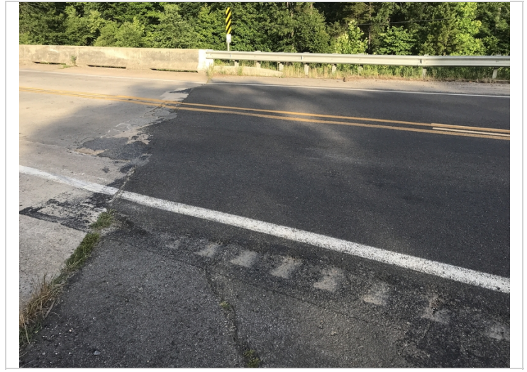
North approach asphalt repair.
