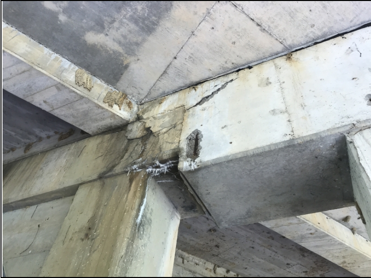
Bent # 2 over Column # 4 concrete delamination and exposed reinforcing steel.
