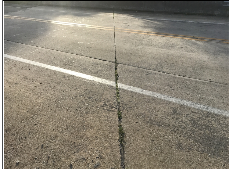
Failing joint sealant.
