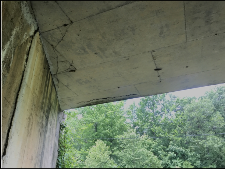
Span # 1 Left concrete delamination.
