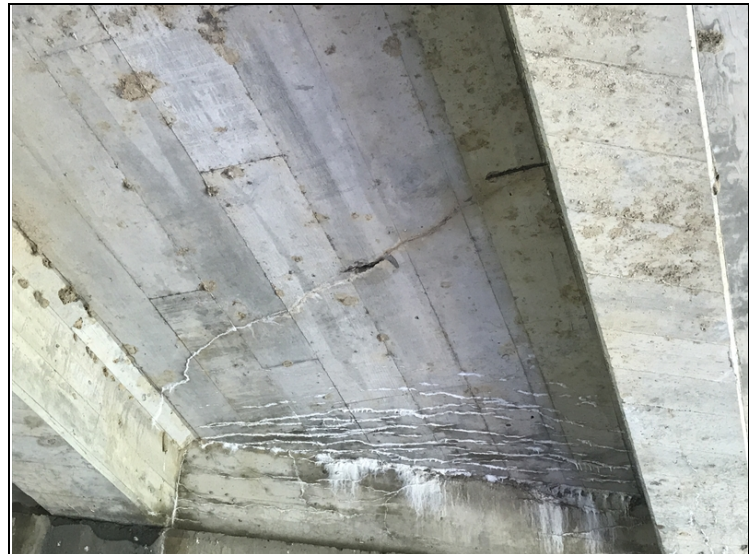
Span # 2 Bay # 2 spalling with exposed reinforcing steel.
