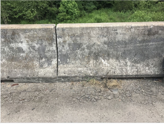
Diagonal cracking in the Left parapet of Span # 1.
