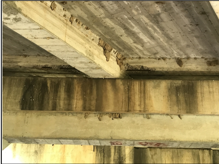
Bent # 2 deck haunch spalling with exposed reinforcing steel.
