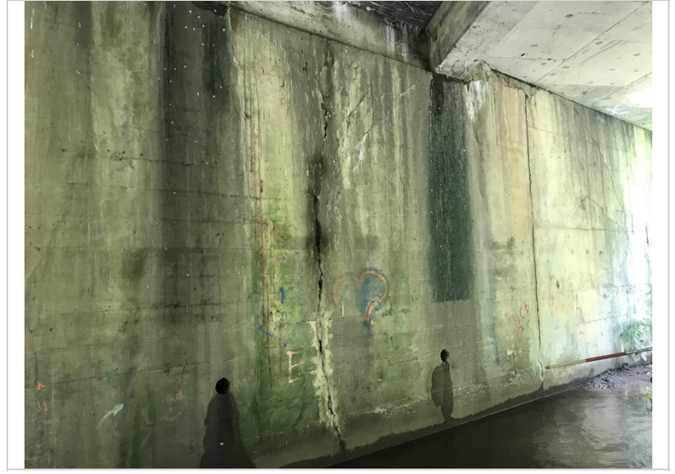
Bent 3 vertical crack.
