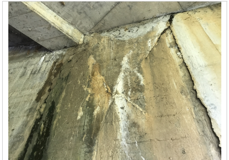
Bent 1 Lt cracking with efflorescence.
