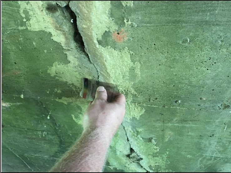
Bent # 3 abutment crack measured 0.040" during this inspection.
