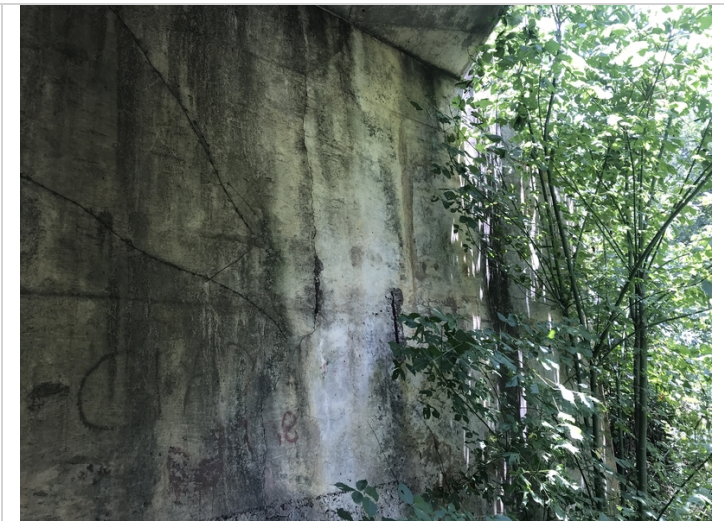
Bent 3 Rt spalling with exposed reinforcing steel.
