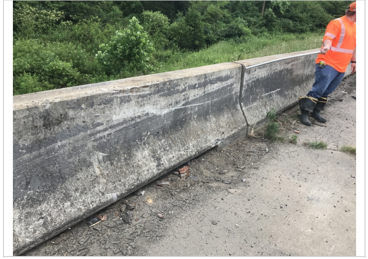
Left bridge railing in Span # 1 over Bent # 2 has collision damage. Base of wall is fractured at the deck juncture and the top is leaning out of alignment 1 1/2".
