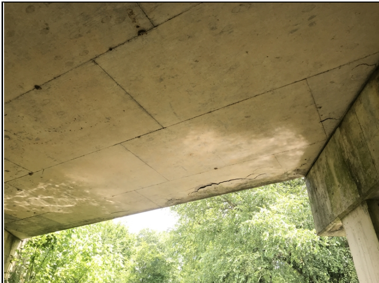
Span # 2 Right concrete delamination along the edge of the slab span.
