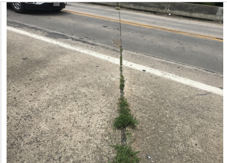
Expansion joint sealant over Bent # 2.
