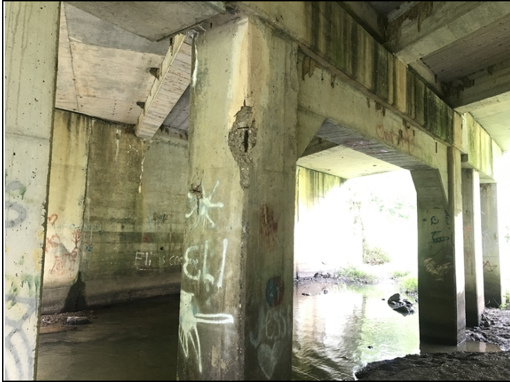
Bent # 2 column # 4. Spall with exposed reinforcing steel.
