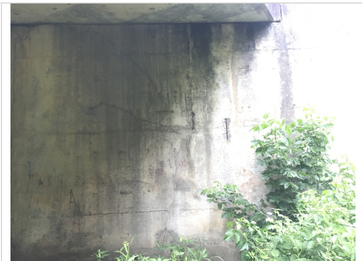
There is a vertical crack with two 2" X 10" areas of spalling with exposed reinforcing steel on the Right side of Bent # 3.
