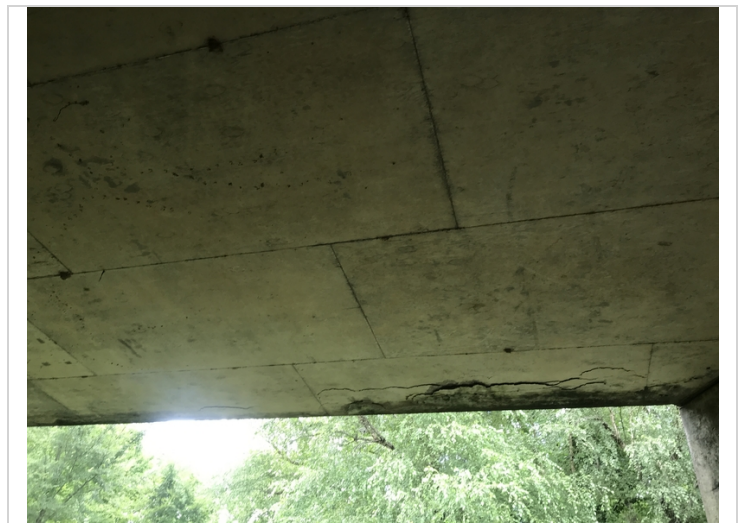
Slab soffit. Right side of Span # 2. Delaminated areas.
