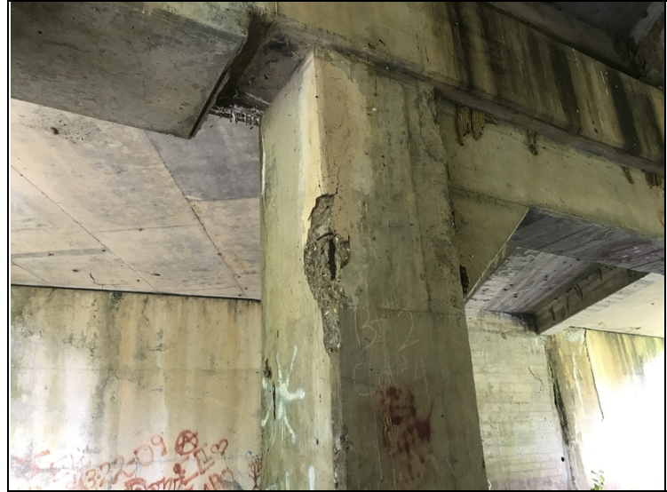
Bent # 2 Column # 4 spalling with exposed reinforcing steel.
