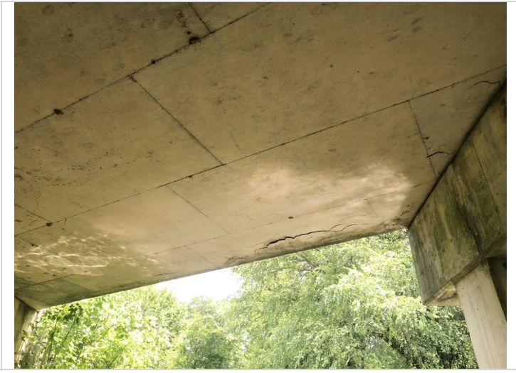
Span 2 Rt concrete delamination along the edge of the slab span.
