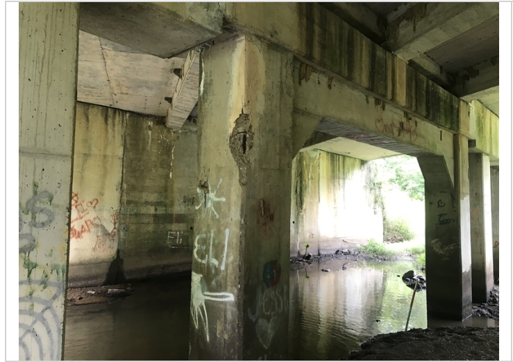
Bent # 2. Column # 4. Spall with exposed reinforcing steel.
