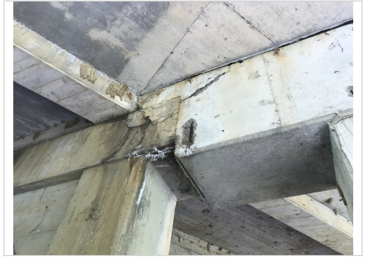
Bent 2 over Col 4 concrete delamination and exposed reinforcing steel.
