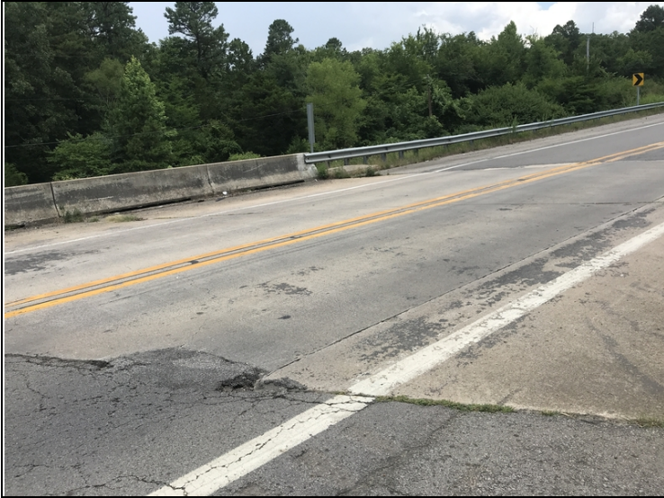
South end of bridge deck wearing surface.
