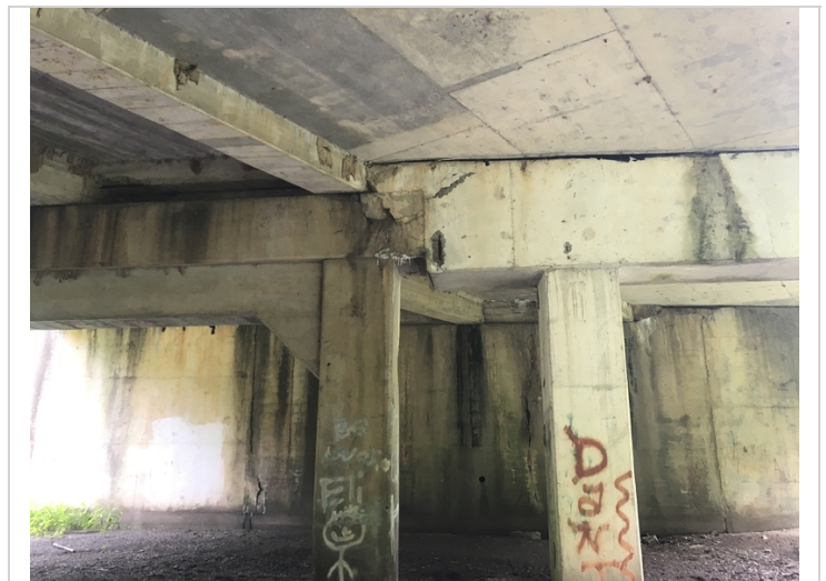
Right construction joint adjacent to Girder # 3.
