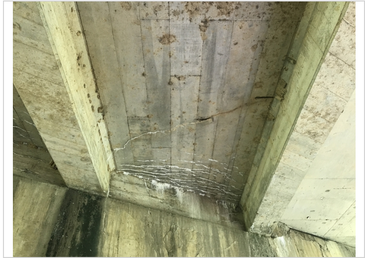
Span # 1 Deck soffit. Spall with exposed reinforcing steel in Bay # 2 adjacent to Bent # 3.
