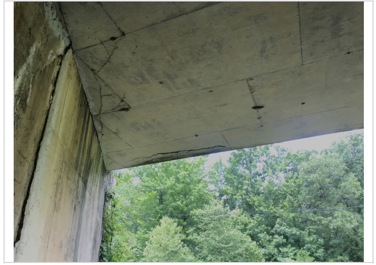
Span 1 Lt concrete delamination.
