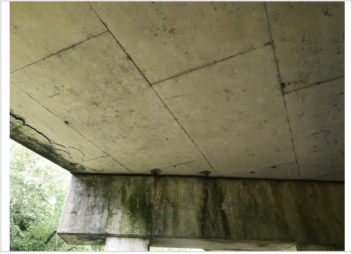
Span # 2 slab soffit adjacent to Bent # 2. Spall with exposed reinforcing steel and delaminated areas.
