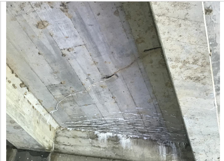
Span 2 Bay 2 spalling with exposed reinforcing steel.
