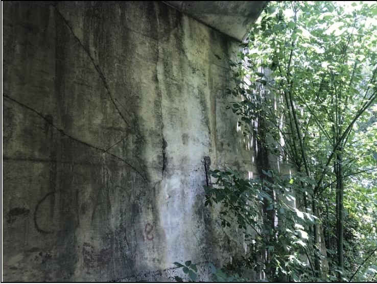
Bent # 3 Rt spalling with exposed reinforcing steel.
