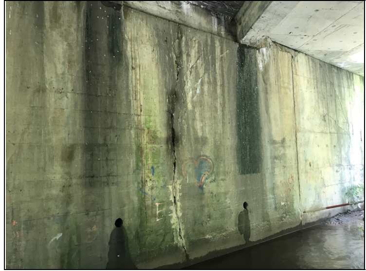
Bent # 3 vertical crack.
