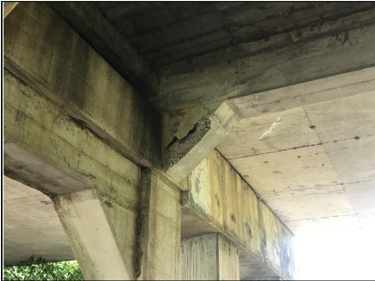
Bent # 2 Girder # 3 spalling with exposed reinforcing steel in the cap haunch.
