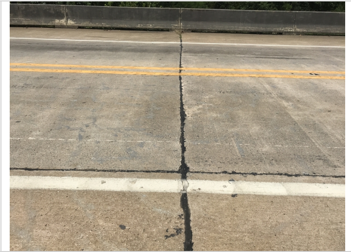
Bent # 2 joint seal.
