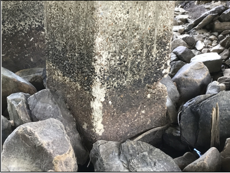
Bent # 2. Column # 4 concrete section loss.
