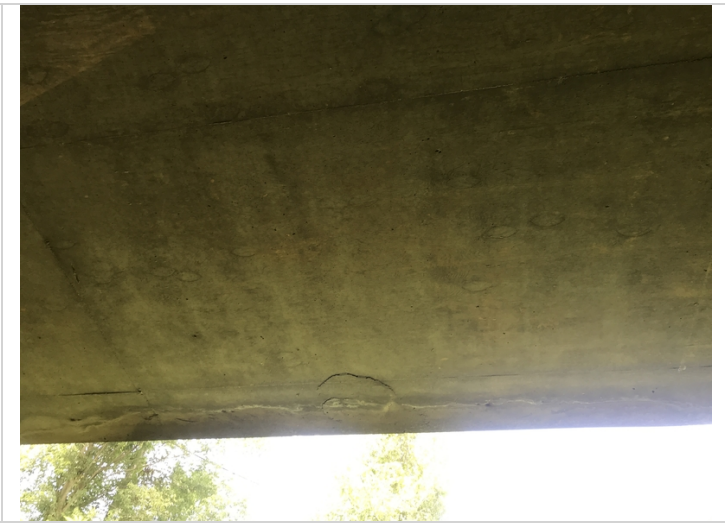
Delaminated area. Right side of Span # 3 slab soffit.
