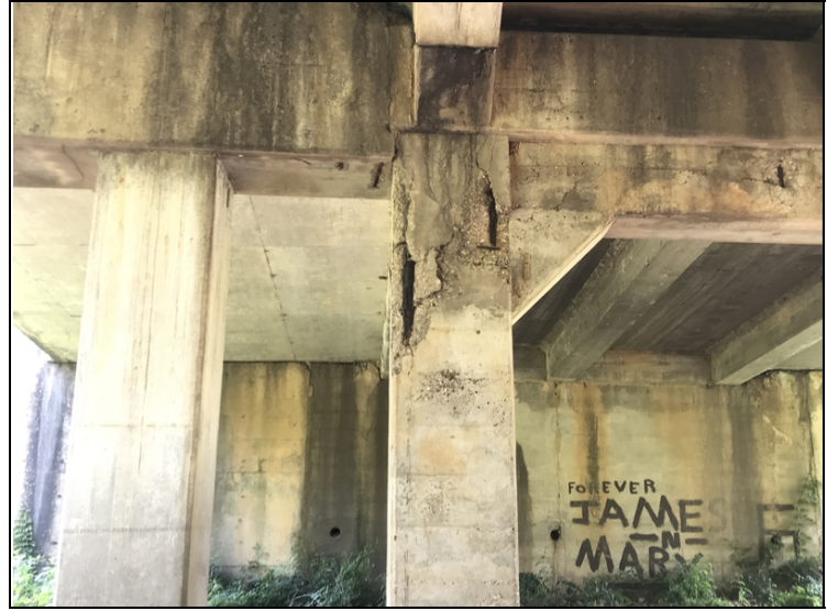
Bent # 2. Column # 4. Exposed reinforcing steel.
