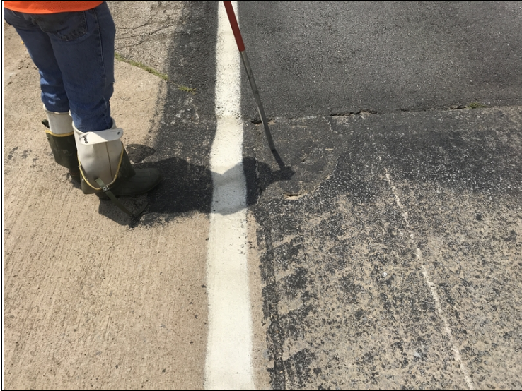
Bent # 4 Lt failing repair.
