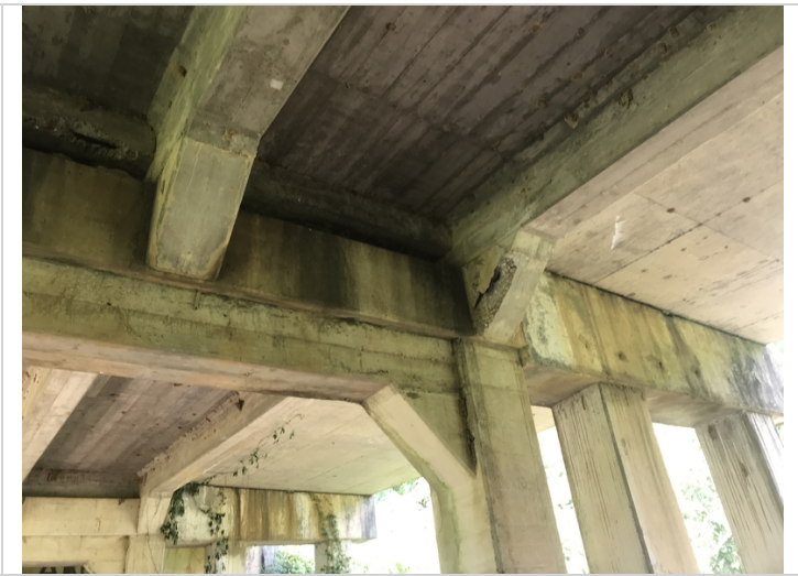
Bent # 2. Back face. Girder # 3 spall in haunch.
