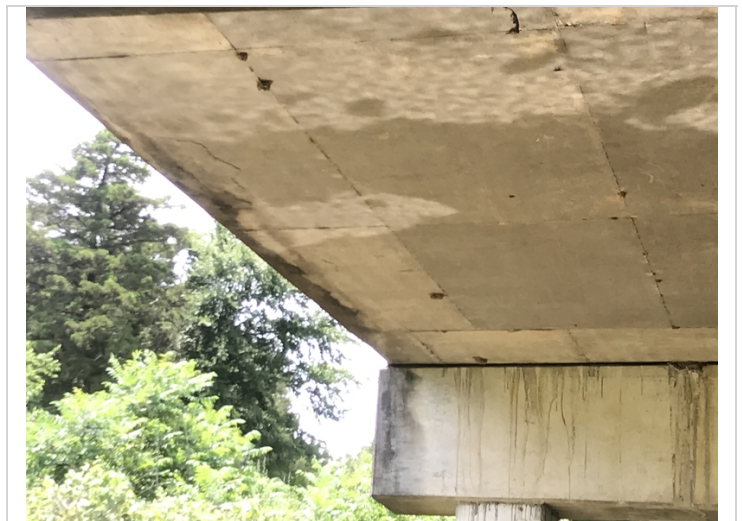
Span # 3 slab soffit. Delaminated area.
