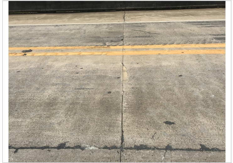
Spalling in the wearing surface over Bent # 3.
