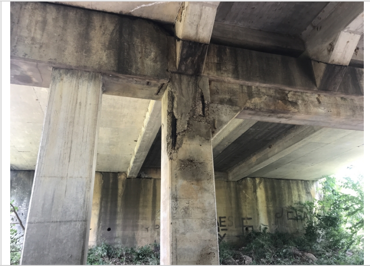
Bent # 2 Span # 2 Column # 4 spalling with exposed reinforcing steel.
