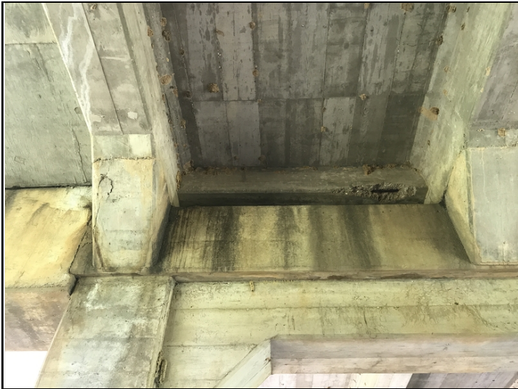
Span # 1 Girder # 1 at Bent # 2 cracking in the cap haunch and Bay # 1 spalling in the deck haunch with exposed reinforcing steel.
