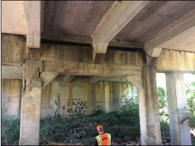
Bent # 2. Cap, span # 2 side. Spall in Column # 4.
