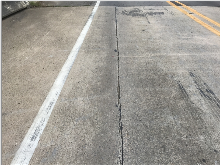
Span # 1 Rt longitudinal construction joint missing sealant.
