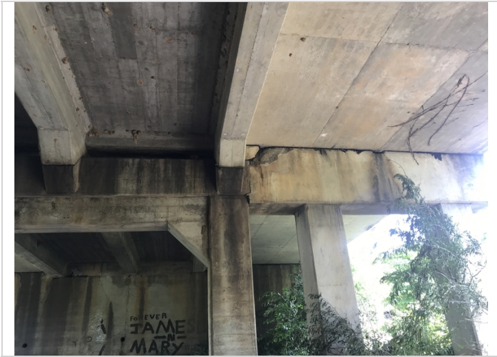
Bent # 2 Span # 2 adjacent to Girder # 1 spalling.
