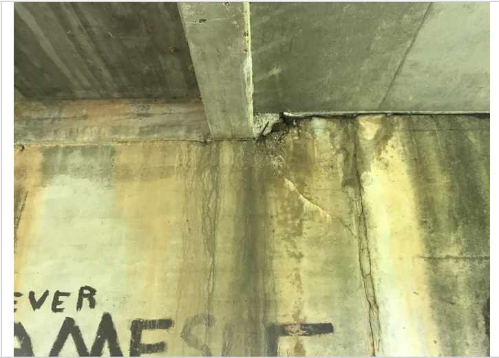
Bent # 1 at Girder # 1 spalling with exposed reinforcing steel in the bearing area.
