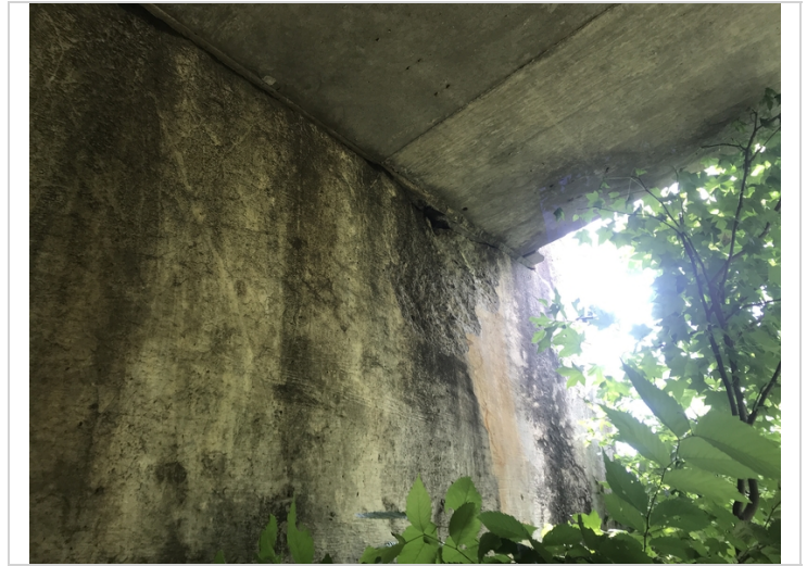
Bent # 1 Lt spalling in the bearing area.
