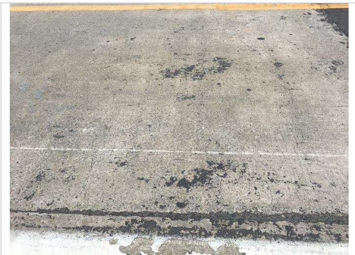
Span # 1 map cracks.
