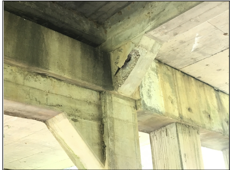
Bent # 2. Span # 1 Girder # 3 haunch. Spall with exposed reinforcing steel.
