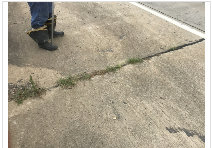
Expansion joint over Bent # 2. Vegetation growing in the joint.
