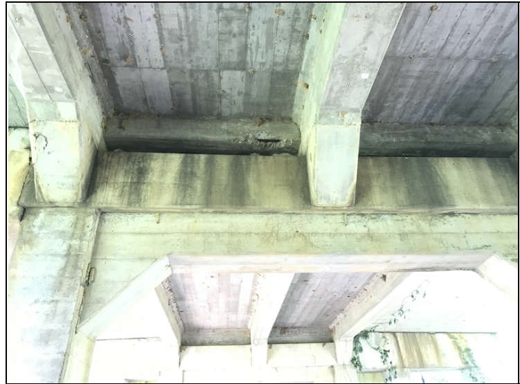
Span # 1 expansion dam over Bent # 2. Spall with exposed reinforcing steel.
