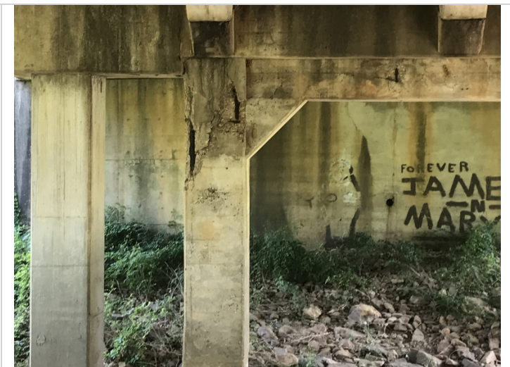
Bent # 2. Column # 4. Ahead face. Spalling with exposed reinforcing steel.
