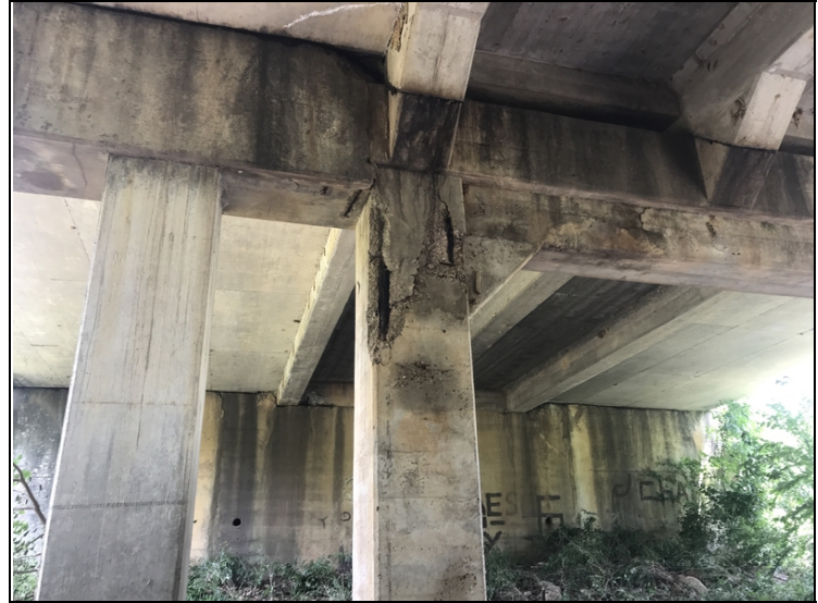
Bent # 2 Span # 2 Column # 4 spalling with exposed reinforcing steel.
