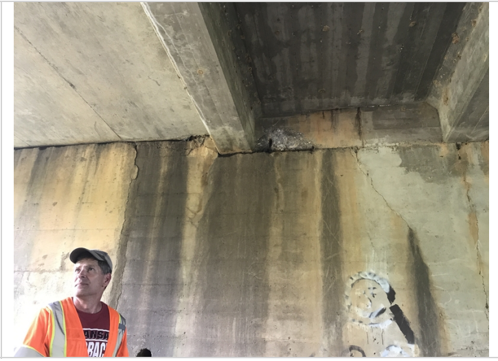
Bent # 1 adjacent to Girder # 3 spalling with exposed reinforcing steel.
