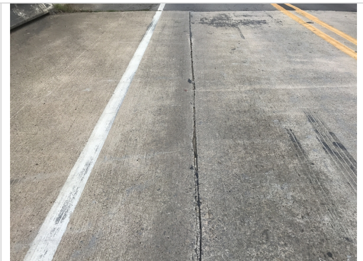
Span # 1 Rt longitudinal construction joint missing sealant.
