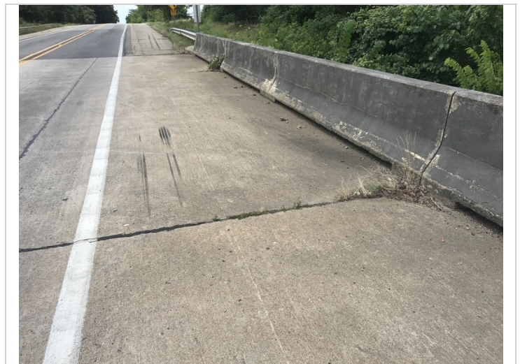
Dirt and vegetation in the deck joints along the gutters.
