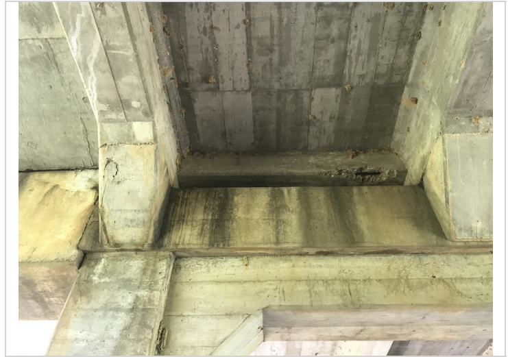
Span # 1 Girder # 1 at Bent # 2 cracking in the cap haunch and Bay # 1 spalling in the deck haunch with exposed reinforcing steel.
