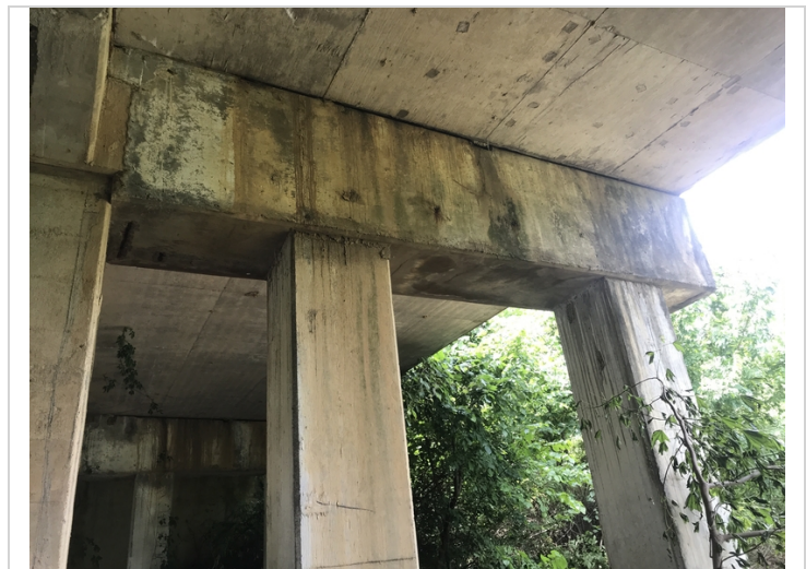
Bent # 2 Rt widened portion of cap with spalling that exposes reinforcing steel on the cap under surface at both ends.
