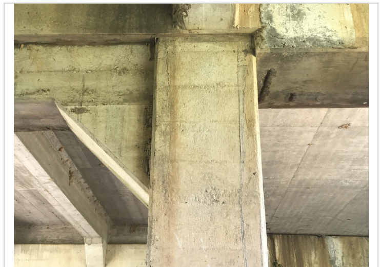
Bent # 2 Column # 4 vertical cracking at the cap juncture.
