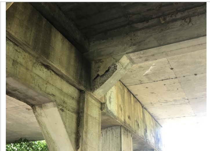
Bent # 2 Girder # 3 spalling with exposed reinforcing steel in the cap haunch.
