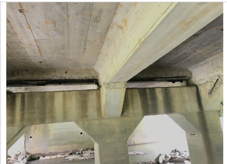
Spalling with exposed reinforcing steel in the deck haunches over Bent # 2. Span # 1.
