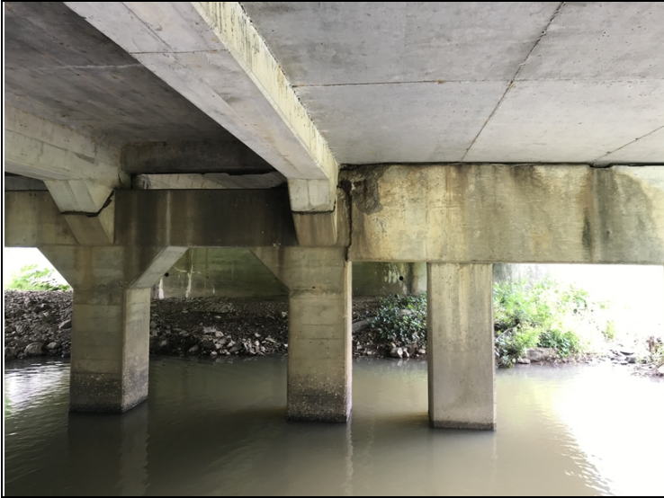
Span # 2 bent # 2. Spall with exposed reinforcing steel adjacent to girder # 1.
