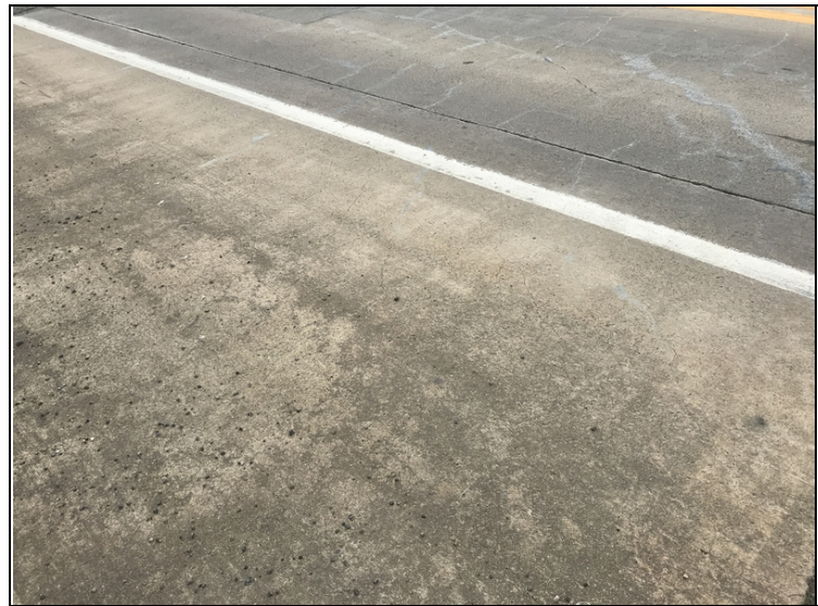
Map cracking in the driving surface of the right shoulder.
