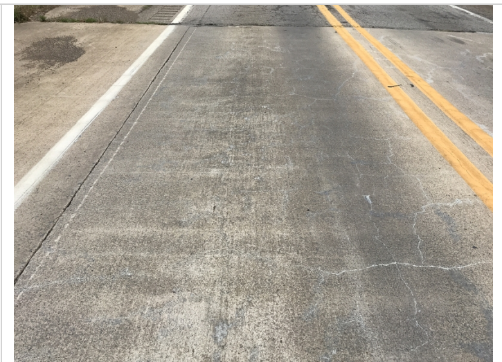
Typical cracking on the wearing surface of the deck.
