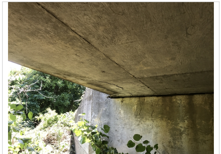
Span # 1 Bent # 1 Rt concrete delamination.
