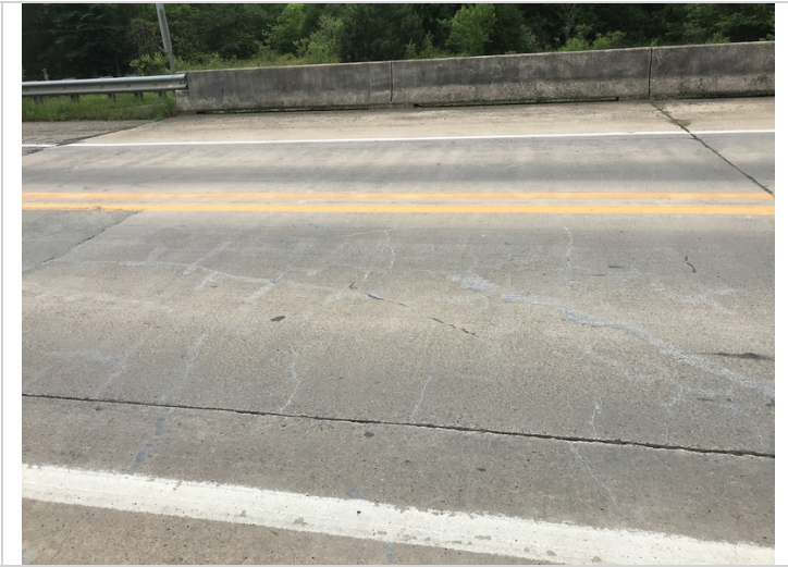
Map cracking in the wearing surface.
