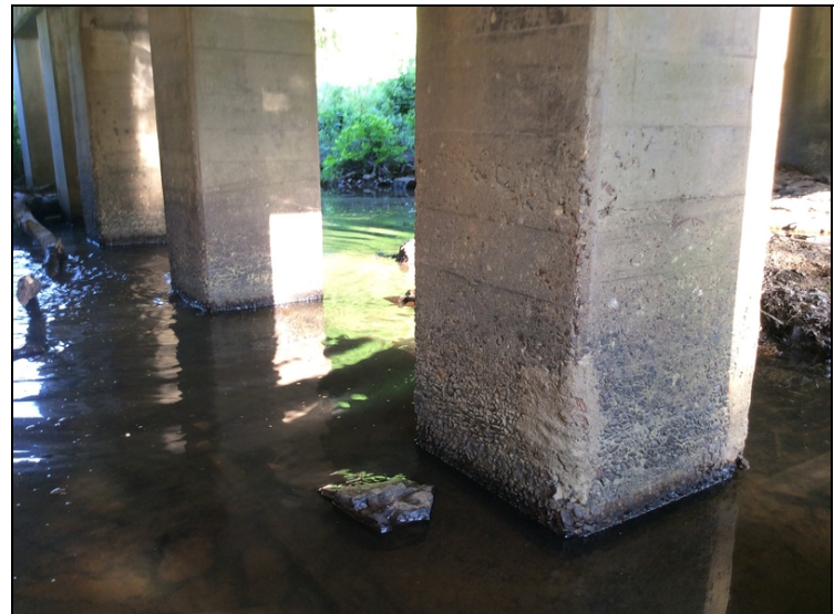
Concrete deterioration at the base of columns at Bent # 2 with up to 2" of concrete section loss at the base of columns that has been grouted since the last inspection.
