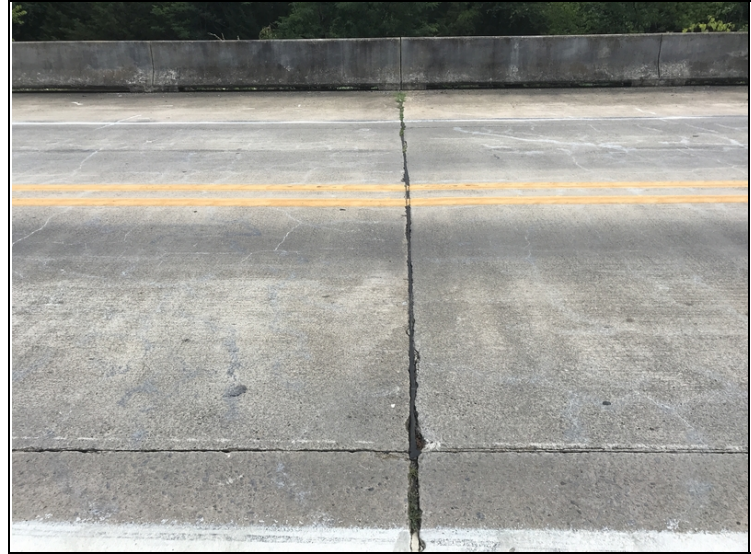
Bent # 2 joint seal adhesion failure.
