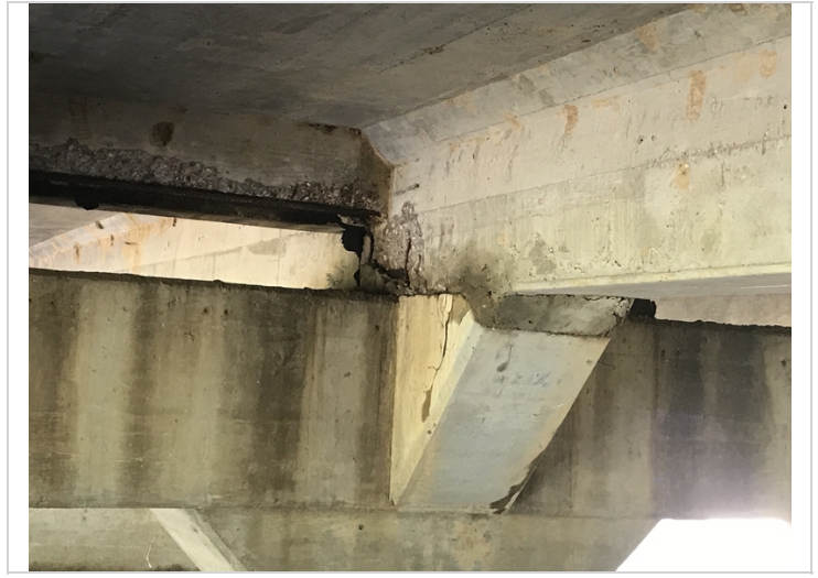
Span # 2 Bent # 2 Girder # 2 spalling with exposed reinforcing steel.
