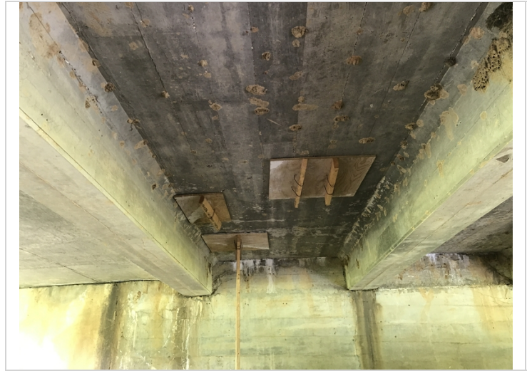
Full depth repairs in Span # 1. Bay # 2. Temporary form work left in place.
