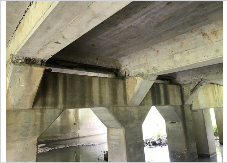
Spalling with exposed reinforcing steel in span # 1 concrete girders over bent # 2.
