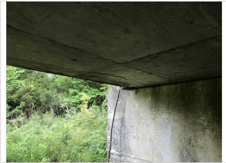
Delaminated area in undersurface of right slab. Span # 1.
