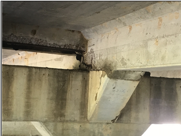
Span # 2 Bent # 2 Girder # 2 spalling with exposed reinforcing steel.
