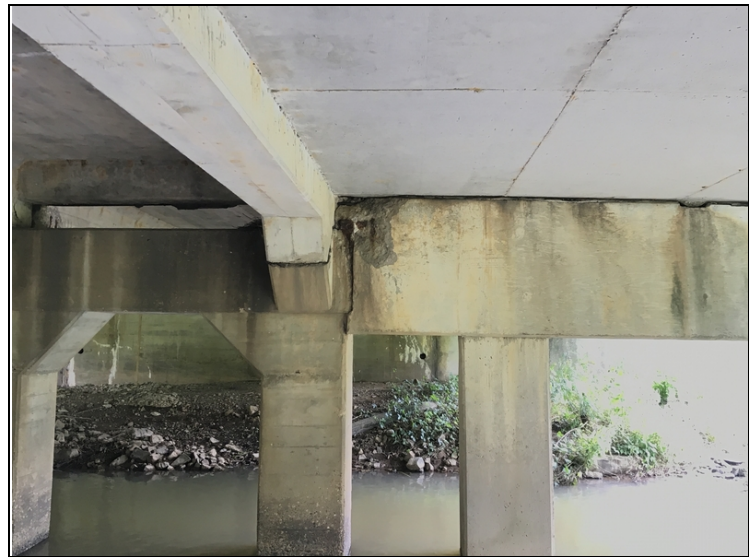
Span # 2. Spall with exposed reinforcing steel adjacent to girder # 1.
