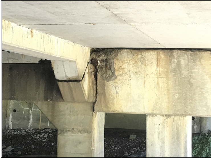
Bent # 2 Cap Span # 2 Column # 3 spalling with exposed reinforcing steel.
