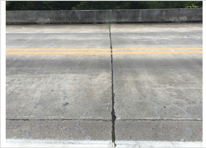
Bent # 2 joint seal adhesion failure.
