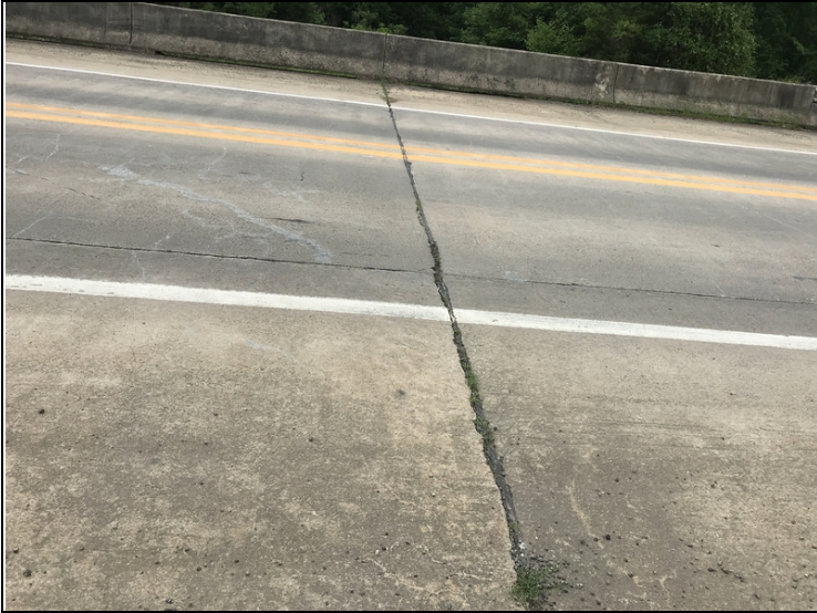
Expansion joint seal is deteriorated and missing in locations.
