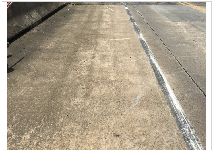
Span # 1 Rt has light map cracking.
