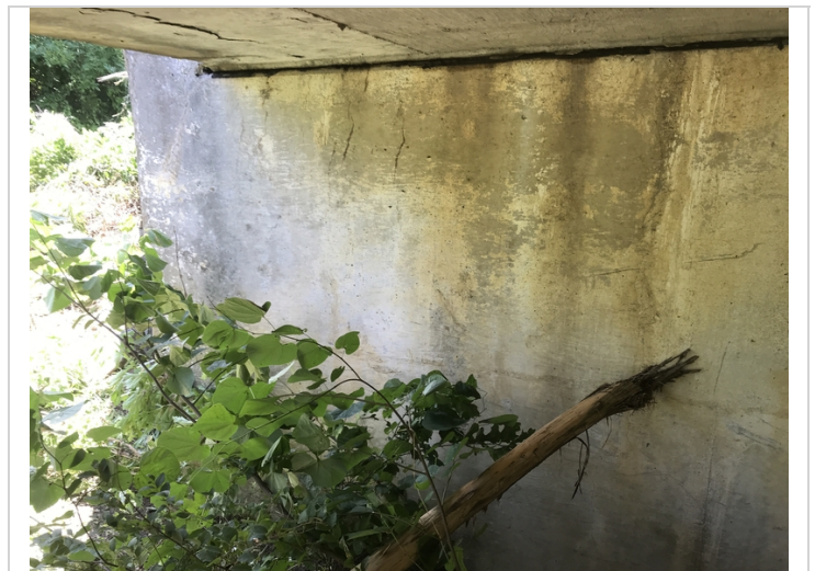
Bent # 1 Rt vertical cracks in the abutment stem.
