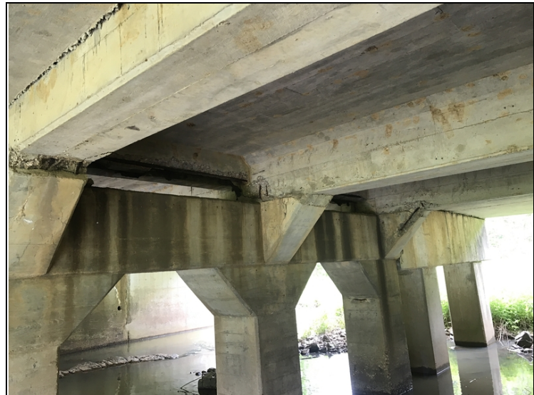
Spalling with exposed reinforcing steel in the concrete girders. Span # 1.
