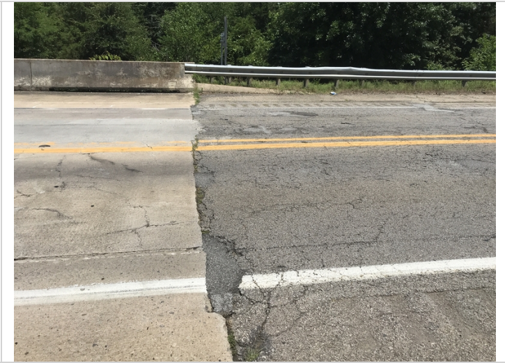
South approach rutting and achm breaking apart.
