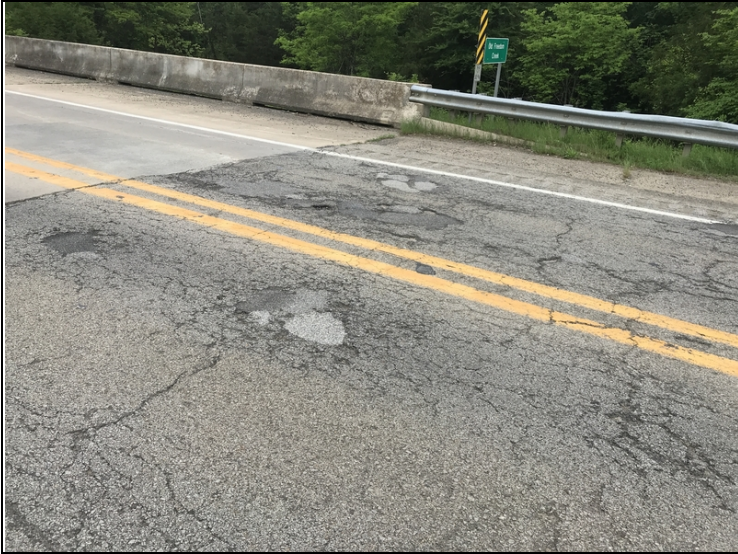
South approach roadway is breaking apart.
