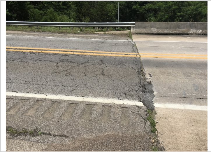
North approach roadway deterioration.
