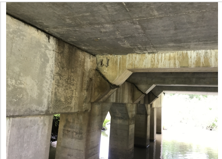
Span # 2. Girder # 3 over bent # 2. Spalls with exposed reinforcing steel.
