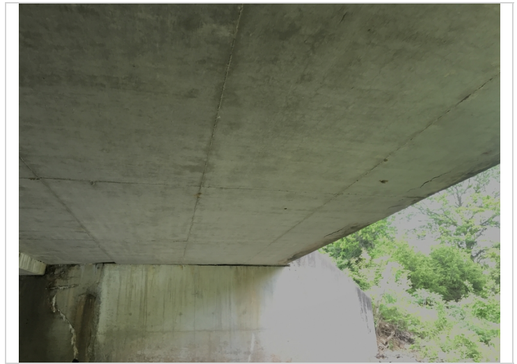
Right slab soffit. Span # 2. Delaminated areas in edge of deck.
