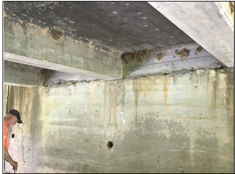
Original portion of bent # 3 has shallow spalls with exposed reinforcing steel at top of stem wall.
