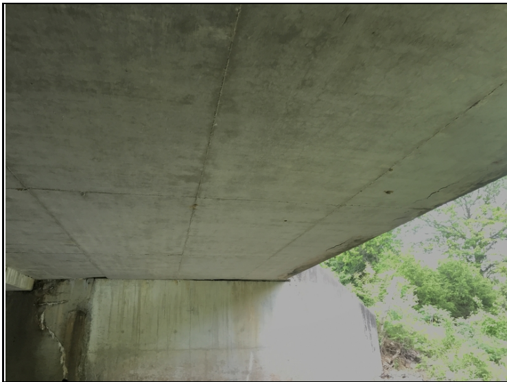
Right slab soffit. Span # 2. Delaminated areas in edge of deck.
