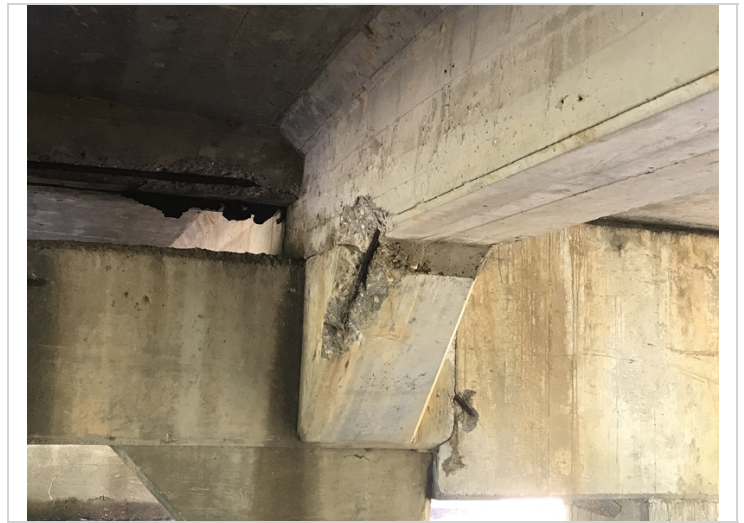
Span # 1 Girder # 3 spalling with exposed reinforcing steel.
