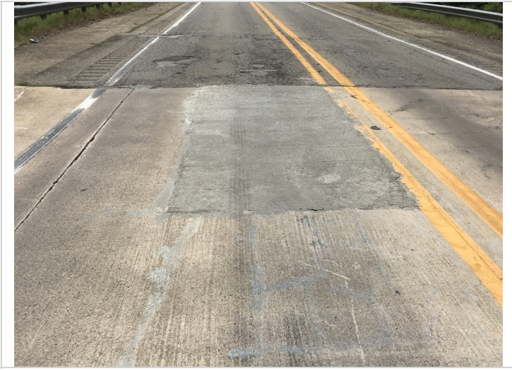
Span # 1 concrete repair.
