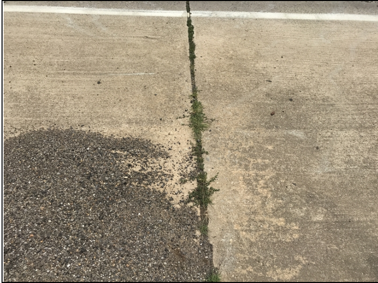
Dirt and debris accumulation in the deck joints.
