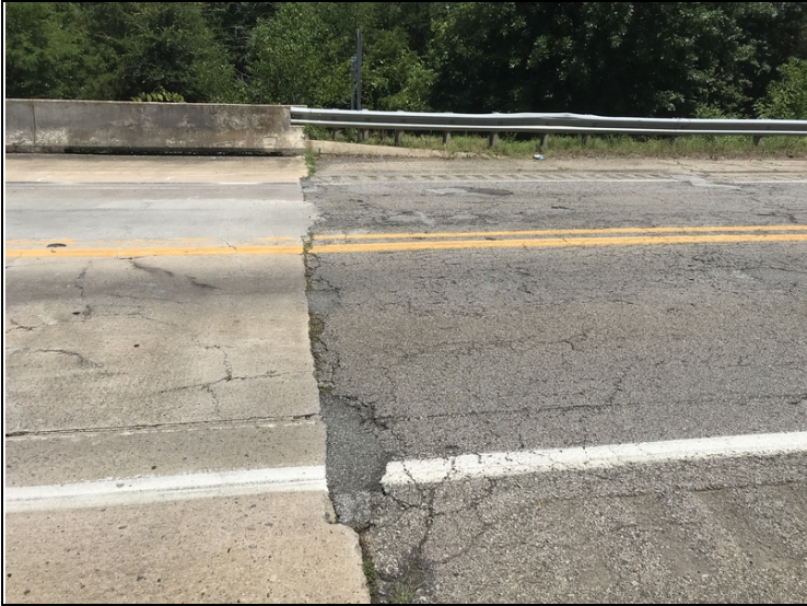
South approach rutting and achm breaking apart.
