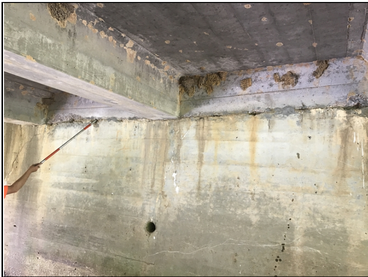
Shallow spalls with exposed reinforcing steel in the original portion of Bent # 3.
