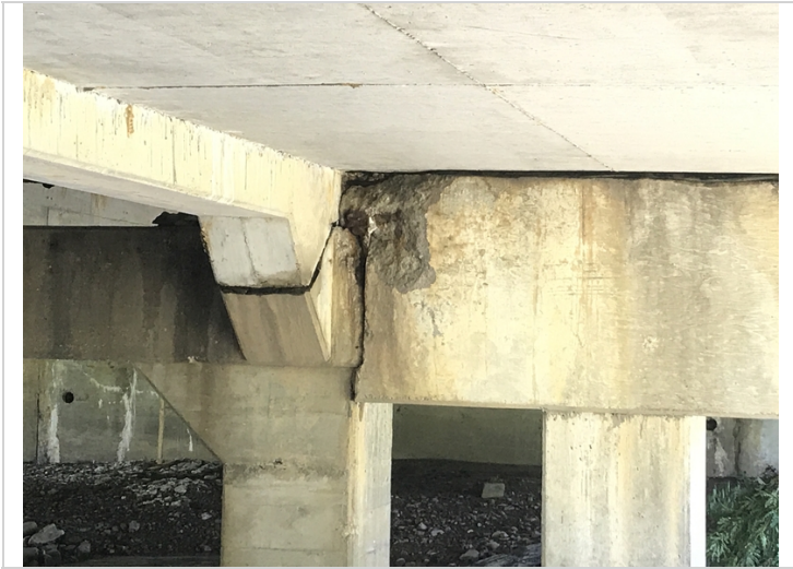
Span # 2 Column # 3 spalling with exposed reinforcing steel.
