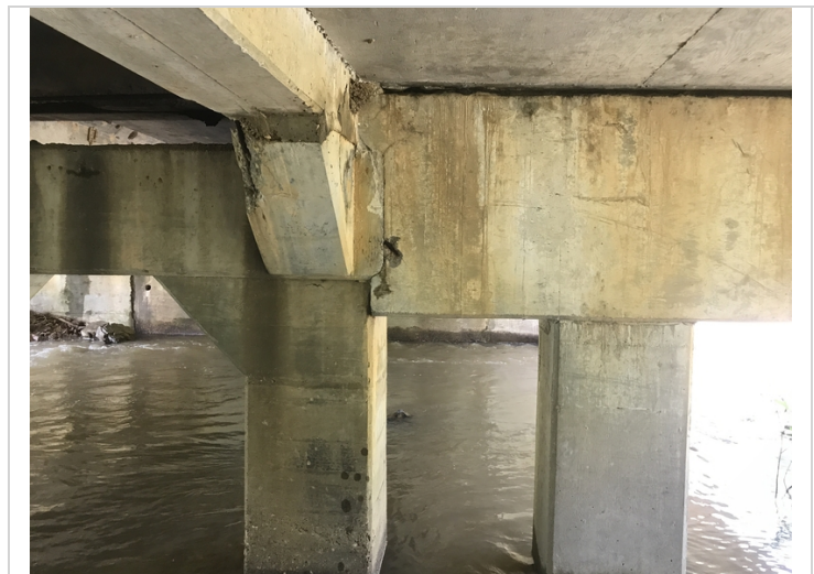
Bent # 2 Rt spalling with exposed reinforcing steel.
