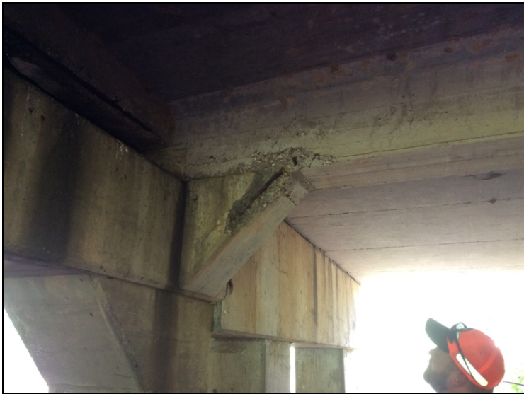
Spall Span # 1, Girder # 3, Bent # 2.
