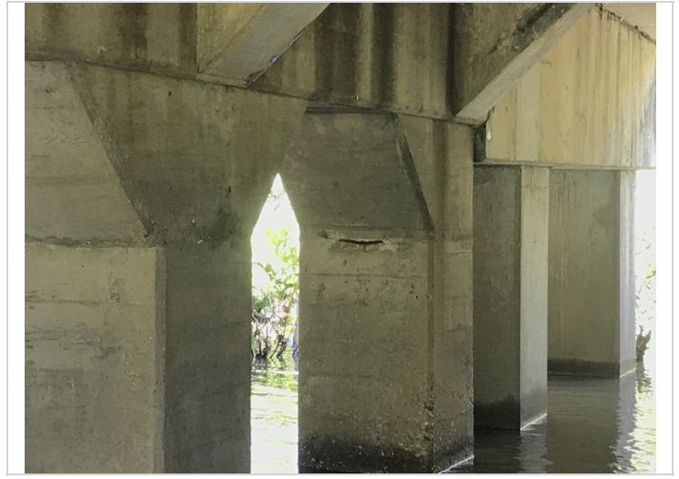
Bent # 2 Column # 5 spalling with exposed reinforcing steel.
