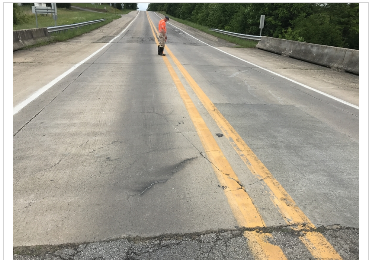
Wearing surface of the top flange. Typical.
