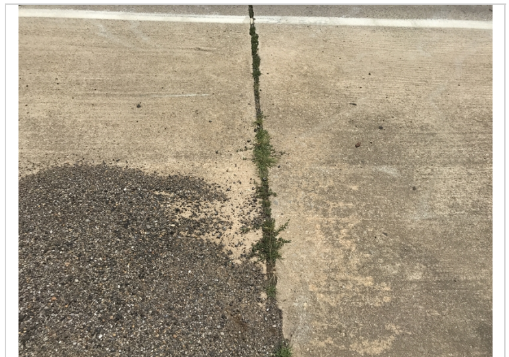
Dirt and debris accumulation in the deck joints.
