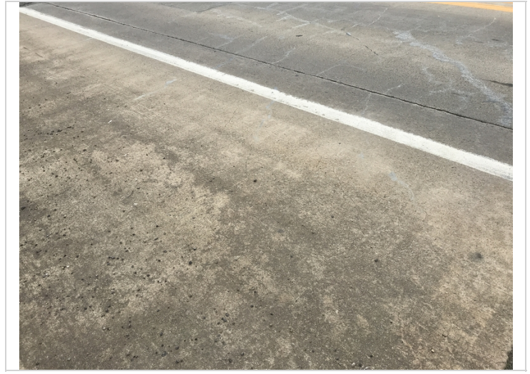
Map cracking in the driving surface of the right shoulder.
