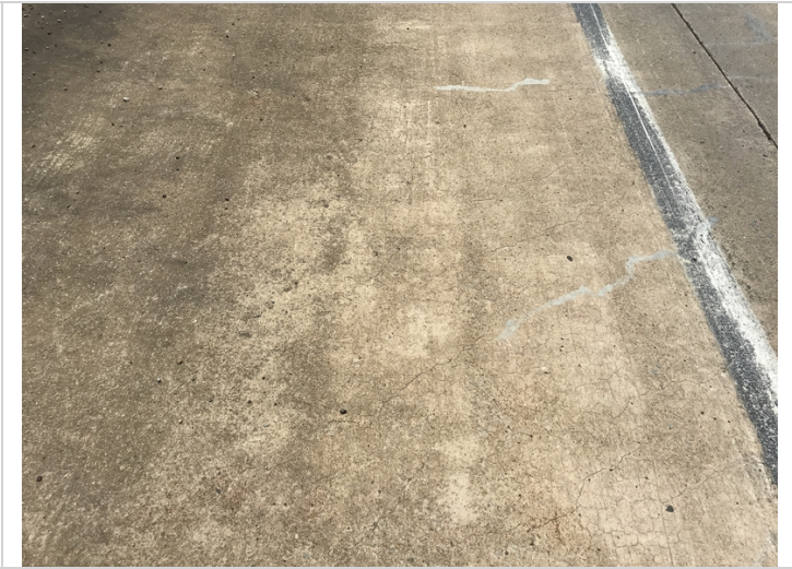
Span # 1 Rt sealable cracking on the slab span.
