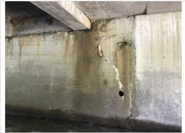
Bent # 3 at Girder # 3 cracking with efflorescence.
