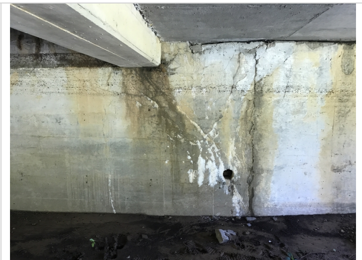
Bent # 1 Lt with cracking with efflorescence , concrete delamination's and shallow spalling.
