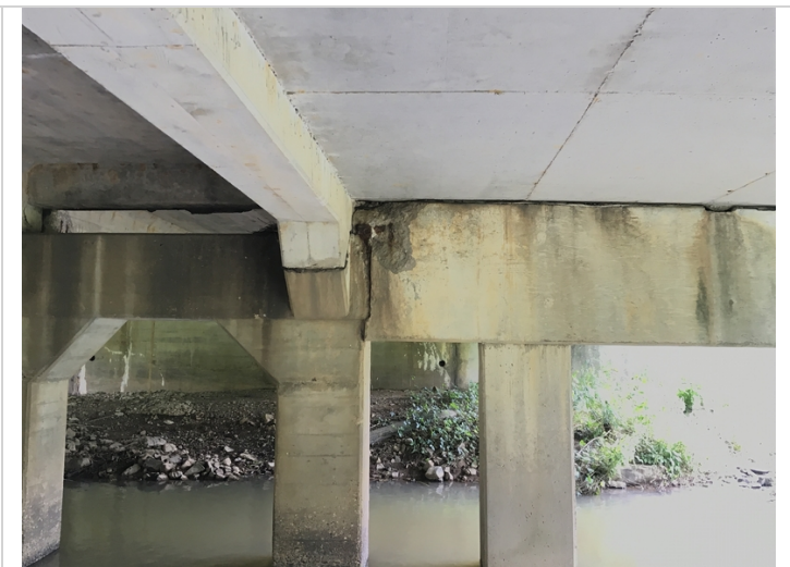
Span # 2. Spall with exposed reinforcing steel adjacent to girder # 1.
