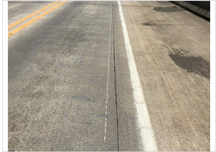
Missing sealant at the longitudinal construction joint.
