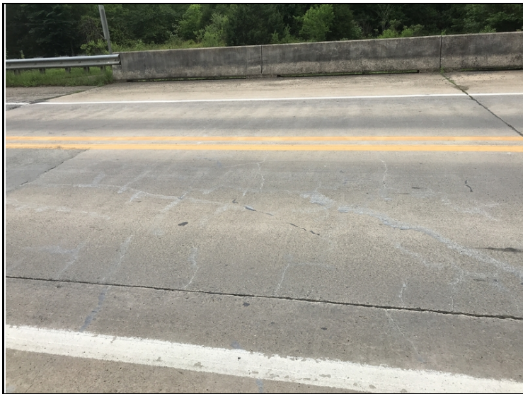
Map cracking in the wearing surface.
