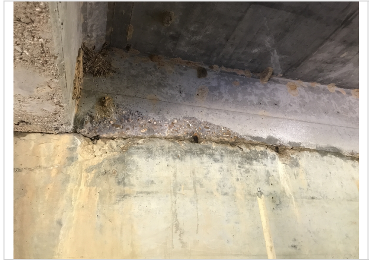
Bent # 3 Bay # 1 small spalls with exposed reinforcing steel.
