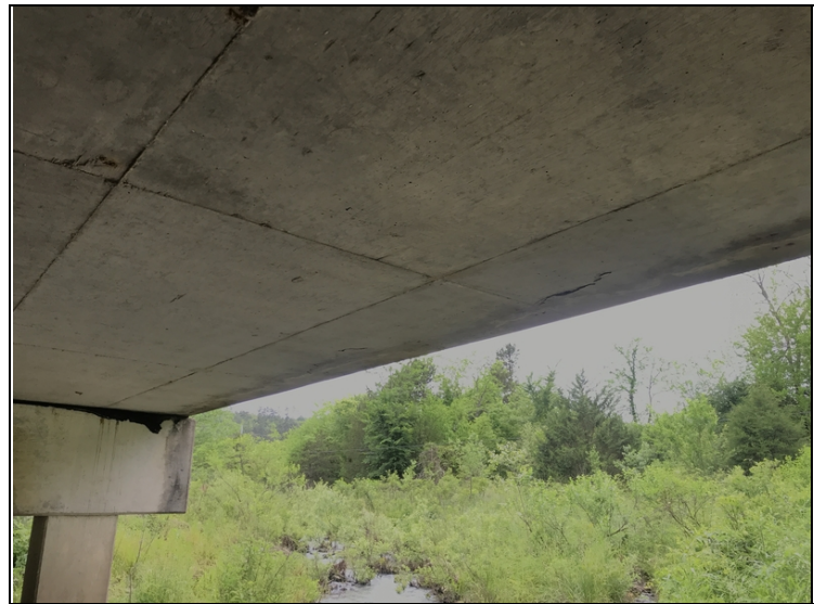
Left edge of span # 2 slab soffit. Delaminated areas.
