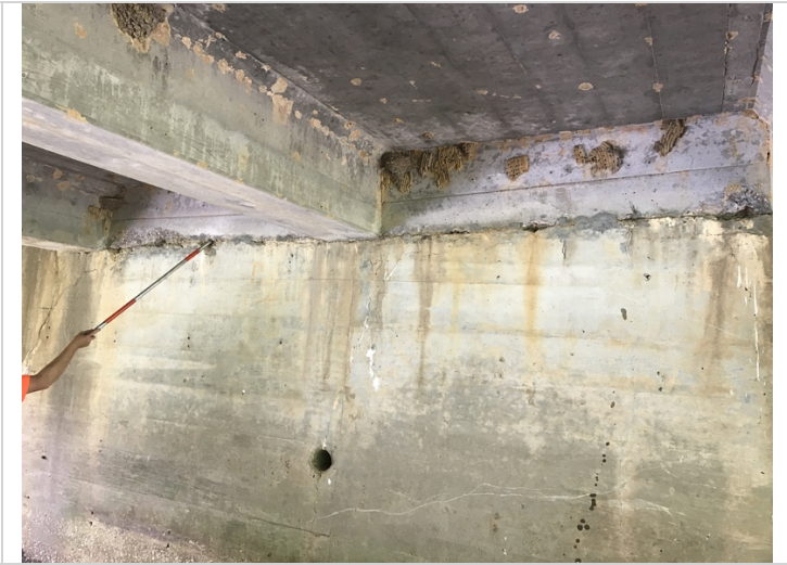
Shallow spalls with exposed reinforcing steel in the original portion of Bent # 3.
