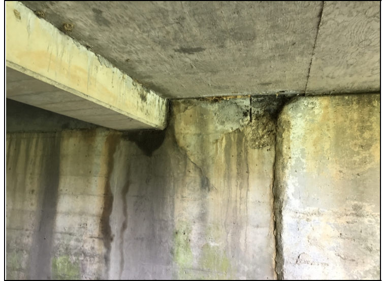
Bent # 1 Left. Spall with exposed reinforcing steel.
