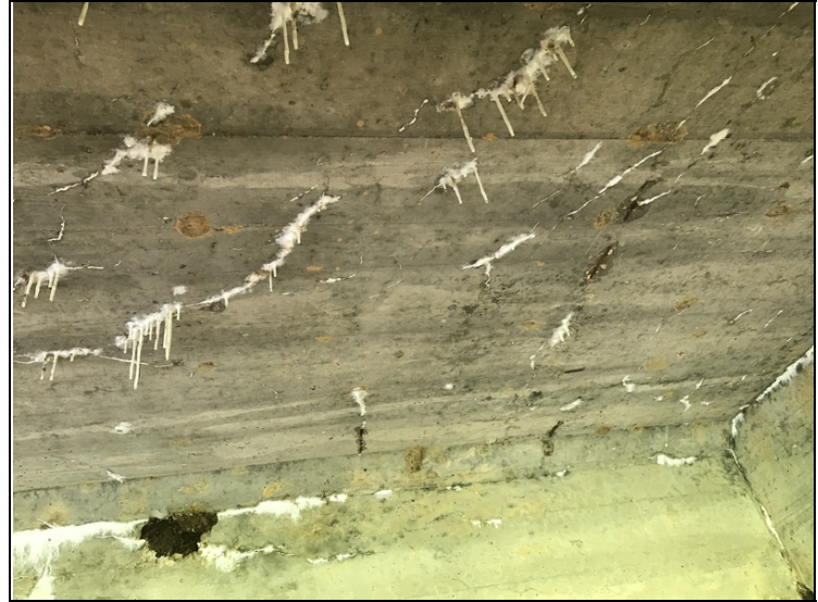
Span # 1 spalls with exposed reinforcing steel.
