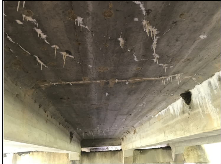
Span # 1 Bay # 1 cracking with efflorescence buildup.
