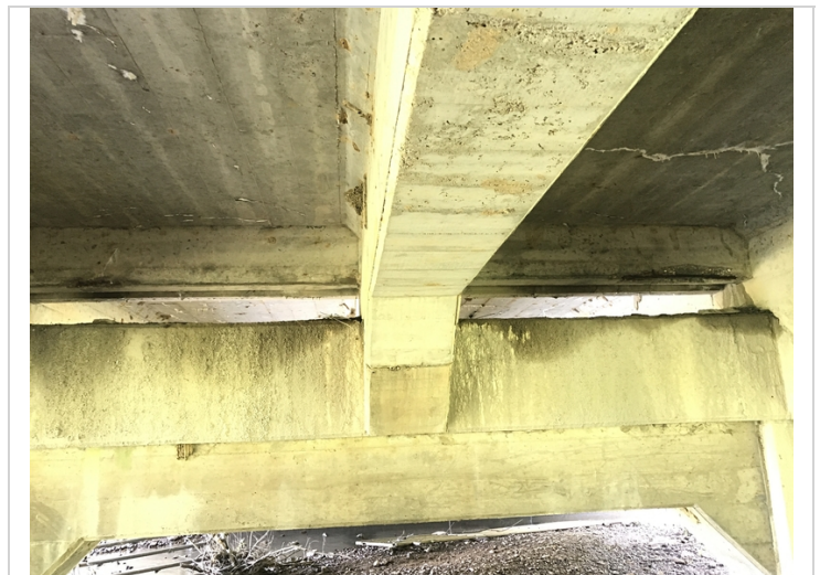
Span 1 spalling with exposed reinforcing steel in the deck expansion dam.
