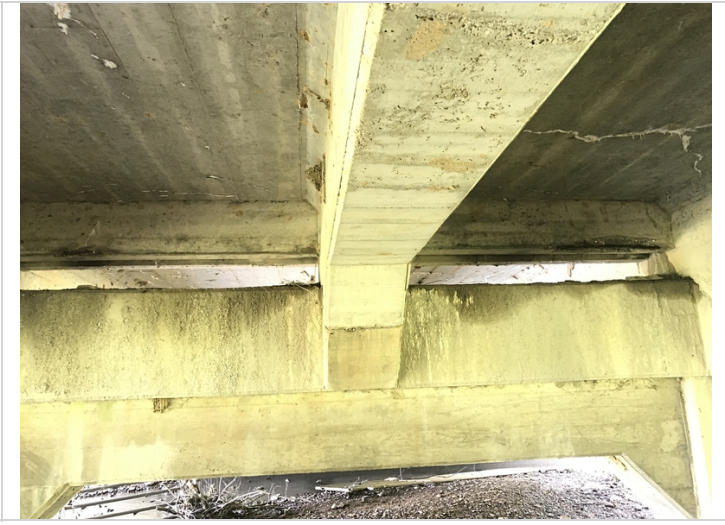
Span # 1 spalling with exposed reinforcing steel in the deck expansion dam.
