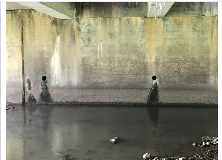
Light abrasion at the base of Bent # 3.
