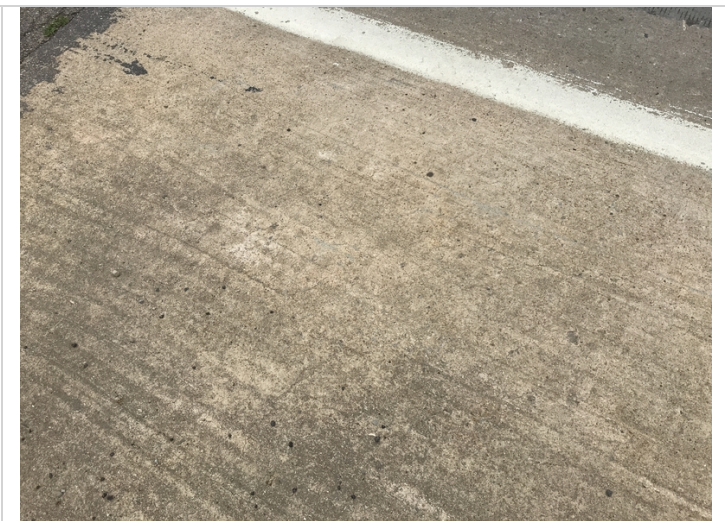
Minor map cracks. Span # 2. Left side of slab.
