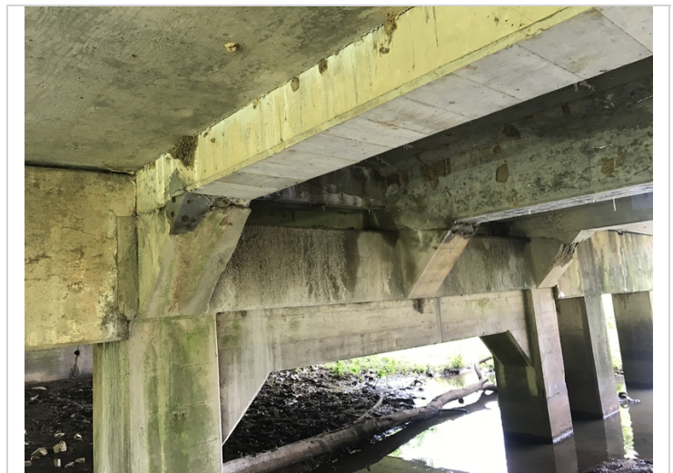
Repair still holding. Span # 2 Bent # 2 Girder # 3.
