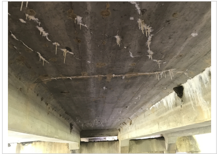
Span # 1 Bay # 1 cracking with efflorescence buildup.
