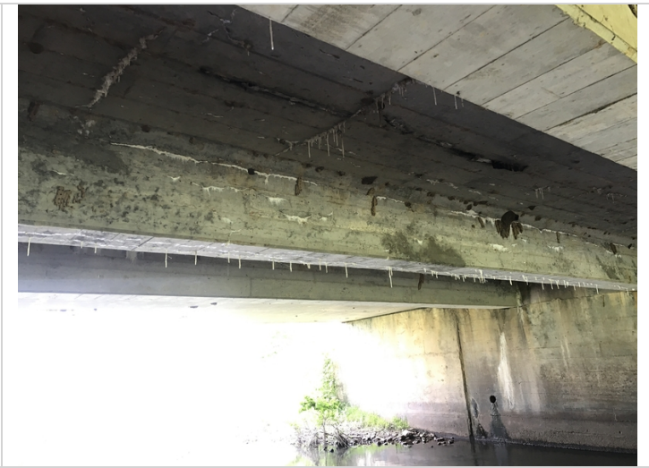
Span # 2, Girder # 2. Cracks with efflorescence.
