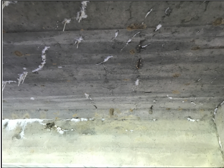
Span # 1 Bay # 1 spalling with exposed reinforcing steel adjacent to Bent # 1.
