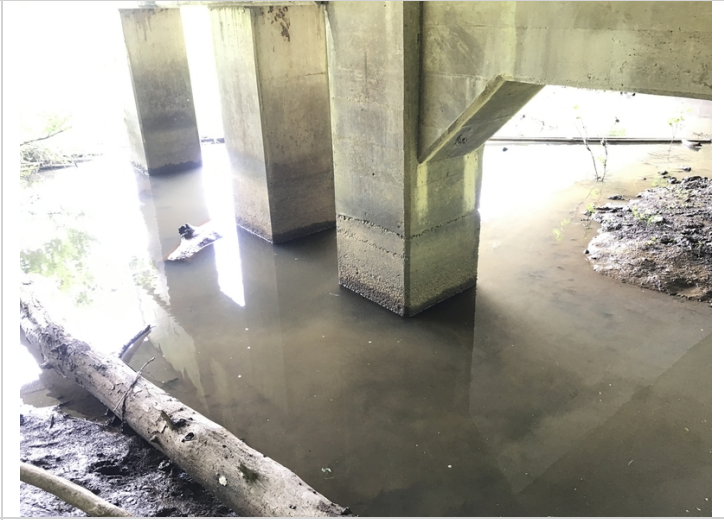
Bent # 2, Column # 3 construction joint.
