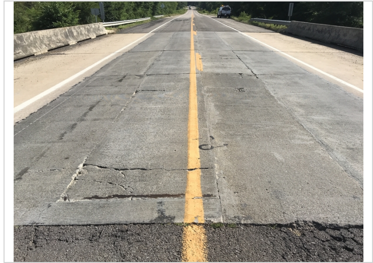
Span # 1 wearing surface breaking apart.
