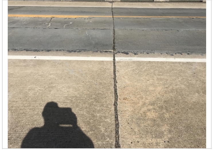
Typical joint seal deterioration.
