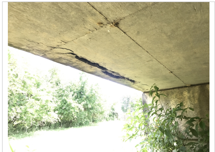
Span 2 Rt spalling with exposed reinforcing steel.
