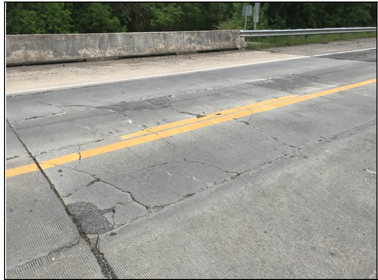
Span # 1 wearing surface is breaking apart.
