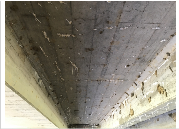
Span 2 Bay 1 cracks with efflorescence.
