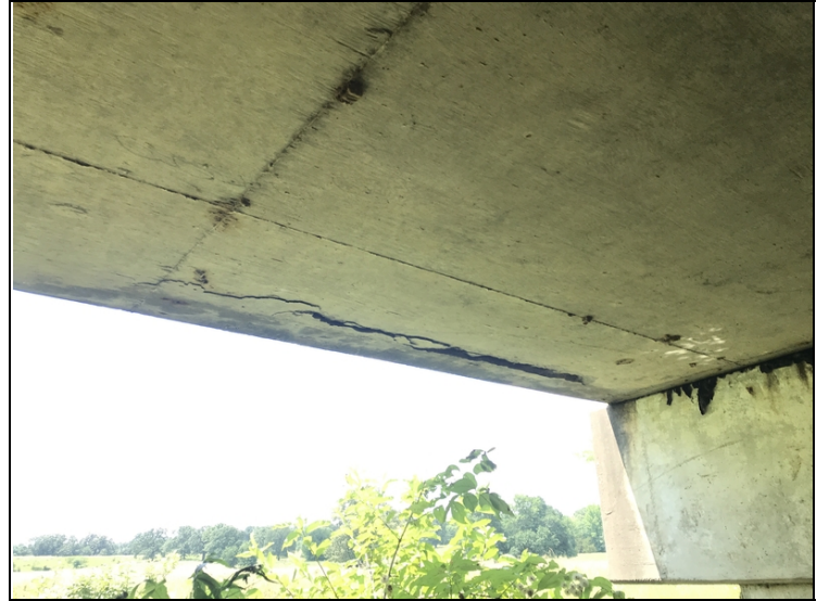
Span # 1 Bent # 2 concrete delamination and spalling with exposed reinforcing steel.
