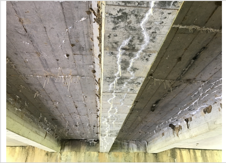
Span # 2 deck soffit. Map cracking and transverse cracking with efflorescence.
