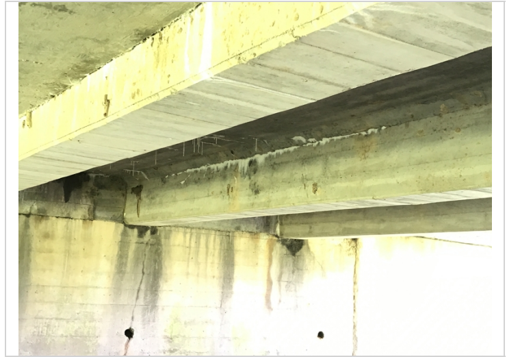
Span # 1. Girder # 2. Horizontal crack with efflorescence.
