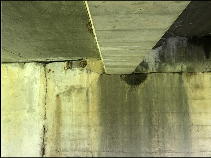
Bent # 1 Right. Spall with exposed reinforcing steel.
