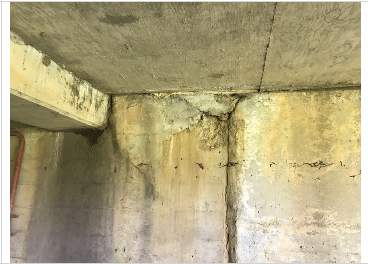
Bent 1 Lt spalling with exposed reinforcing steel adjacent to Girder 1.
