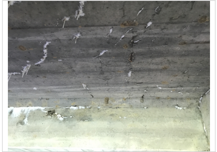
Span 1 Bay 1 spalling with exposed reinforcing steel adjacent to Bent 1.
