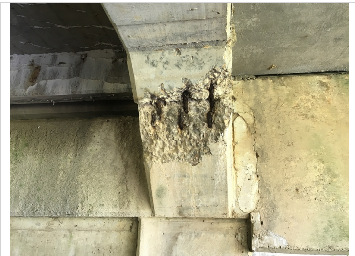
Span 2 Bent 2 Girder 1 spalling with exposed reinforcing steel.
