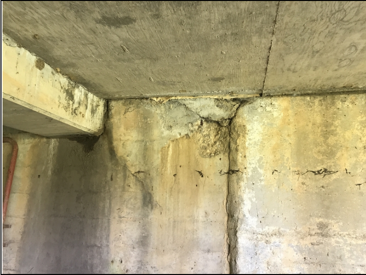
Bent # 1 Lt spalling with exposed reinforcing steel adjacent to Girder # 1.
