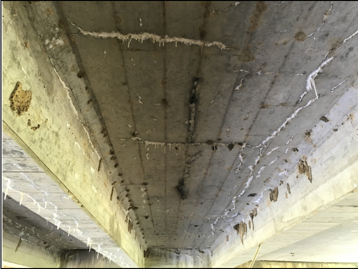
Span # 2 Bay # 2 cracking with efflorescence on the undersurface.
