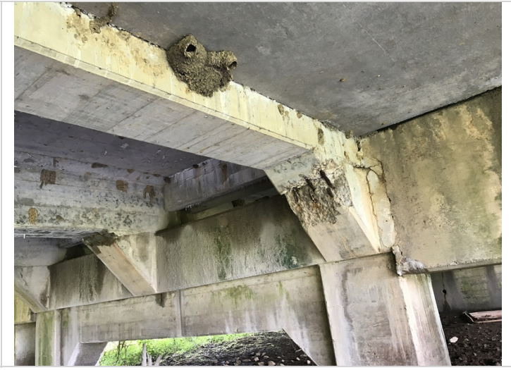
Span # 2, Girder # 1 at Bent # 2. Spalling with exposed reinforcing steel at the cap haunch.
