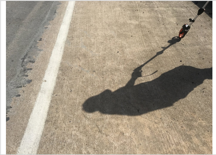
Map cracking on the slabs.
