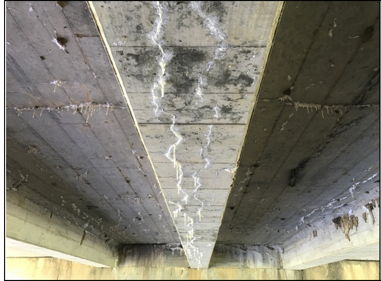
Span # 2 Girder # 2 cracking with efflorescence.
