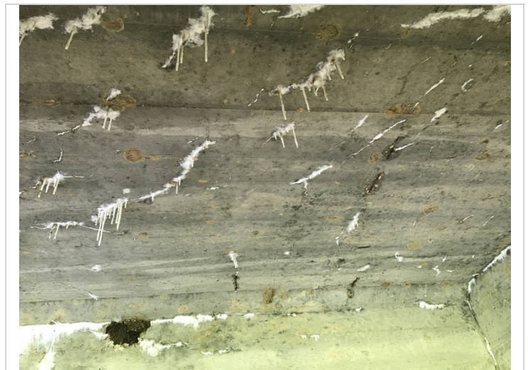
Span # 1, Bay # 1. Spalls with exposed reinforcing steel in proximity to Bent # 1.
