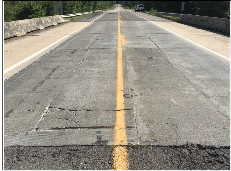
Span # 1 wearing surface breaking apart.
