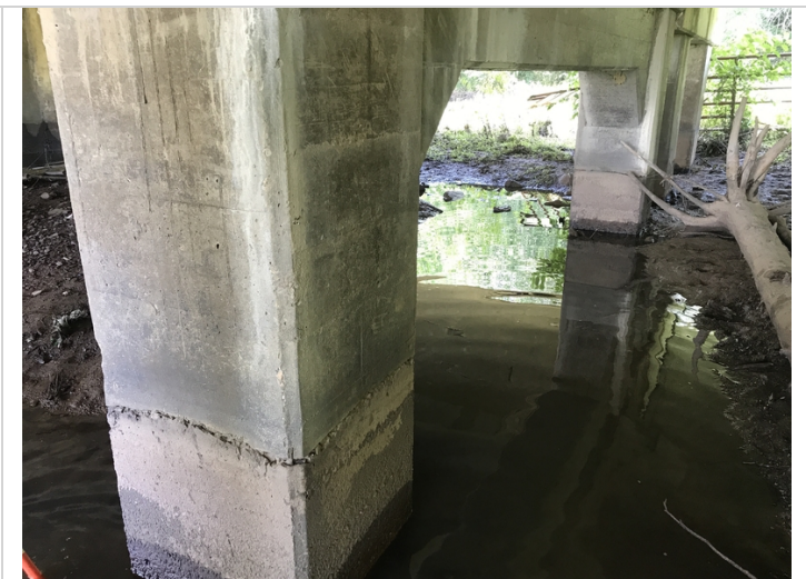
Bent 2 columns 3 & 4 abrasion and concrete deterioration.
