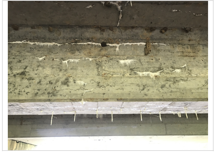
Cracking in Span # 2, Girder # 2. Typical.
