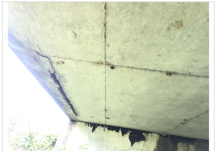
Span # 1. Left slab soffit. Spalling with exposed reinforcing steel.
