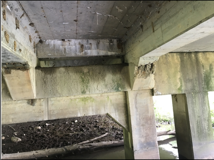
Span # 2 Bent # 2 Girder # 1 spalling with exposed reinforcing steel.
