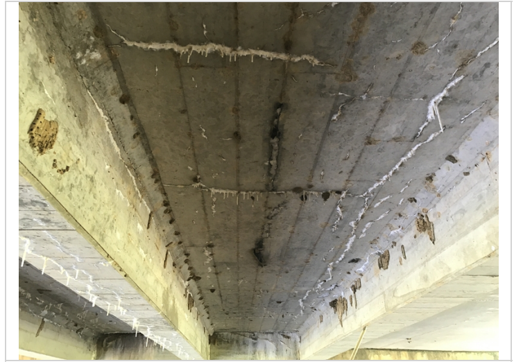
Span 2 Bay 2 cracking with efflorescence on the undersurface.
