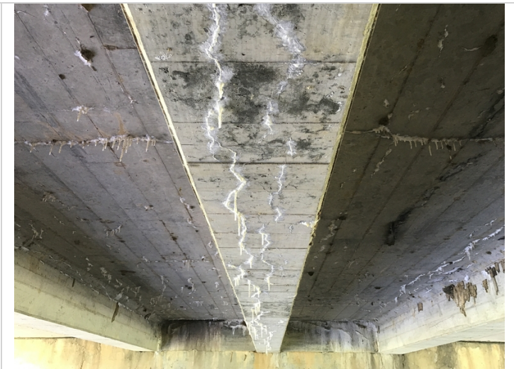
Span 2 Girder 2 cracking with efflorescence.
