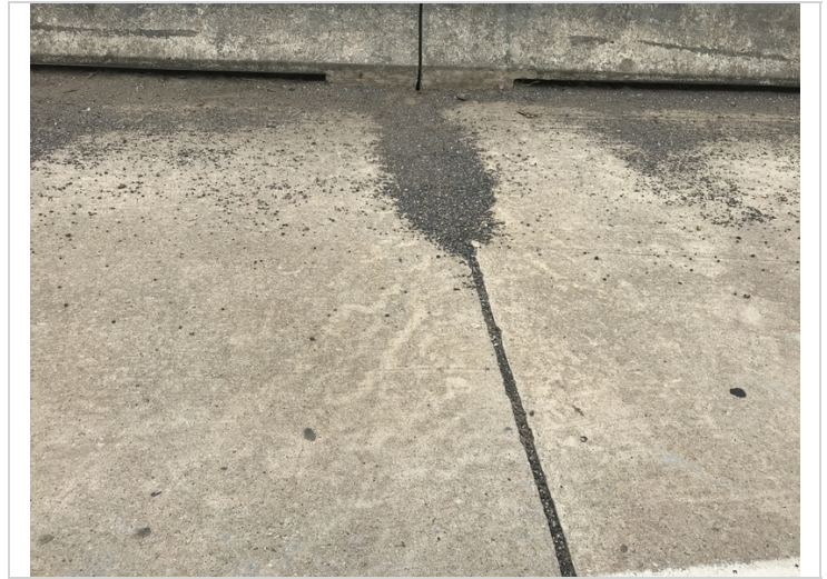
Expansion joint sealant over Bent # 2. Left side of structure.
