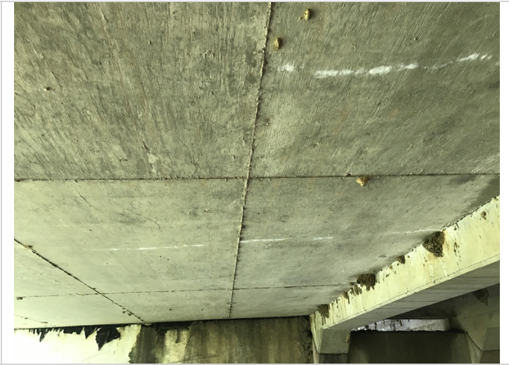
Transverse hairline cracks in the Left side of Span # 1.
