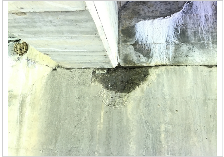
Bent # 1 has a 12" spalled area with exposed reinforcing steel under Girder # 3.
