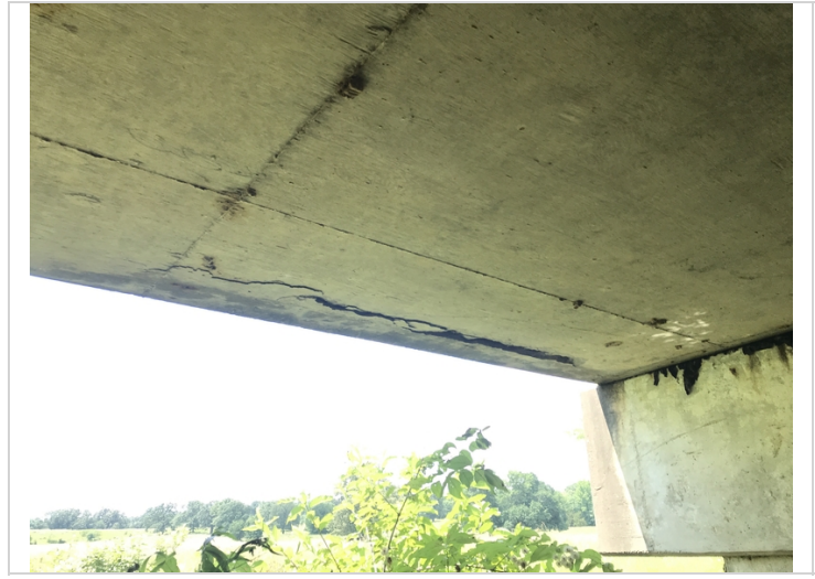
Span 1 Bent 2 concrete delamination and spalling with exposed reinforcing steel.
