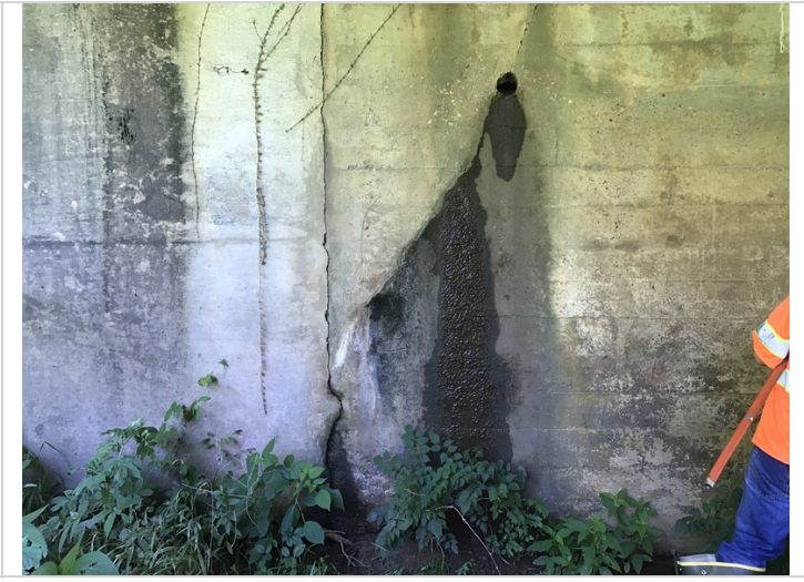
Bent # 4 Lt diagonal crack with efflorescence and rust stains.
