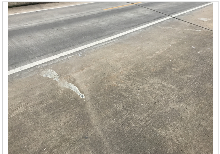
Transverse crack. Right side of Span # 2.
