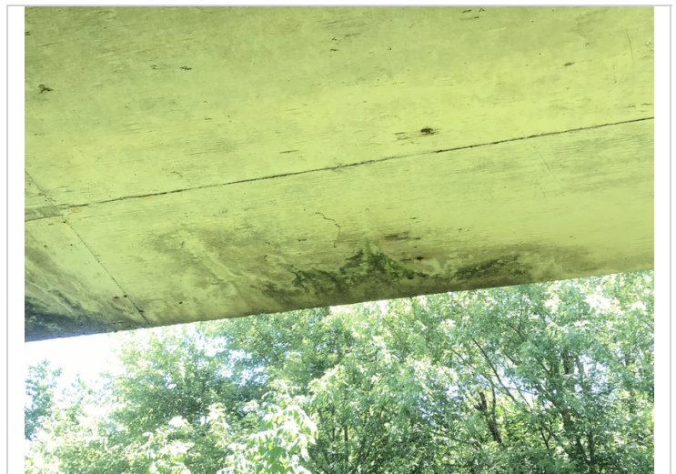
Span # 1 Rt small concrete delamination's along the edge.
