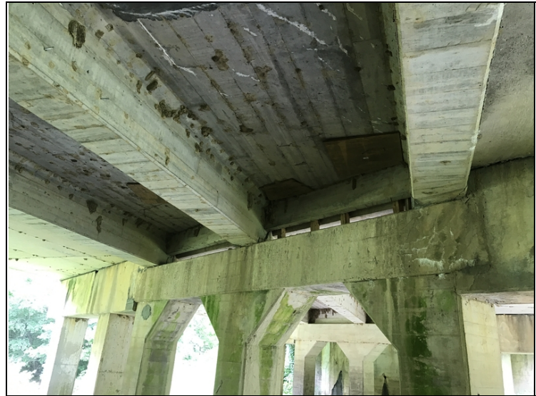
Delaminated areas in Span # 1 Girders over Bent # 2.
