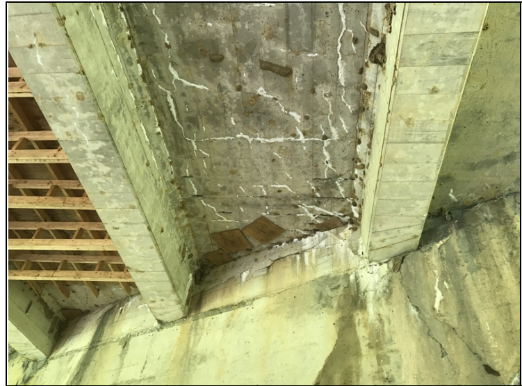
Span # 3 bay # 2. Spalls with exposed reinforcing steel adjacent to bent # 4.
