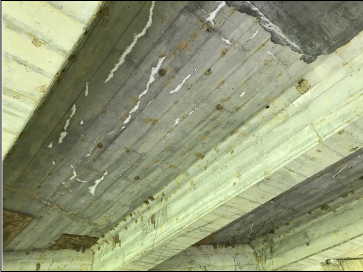
Map cracking with efflorescence in deck soffit of Span # 1.
