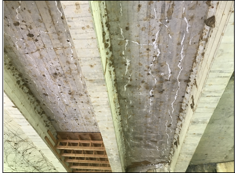
Map cracking with efflorescence in the deck soffit of Span # 3.
