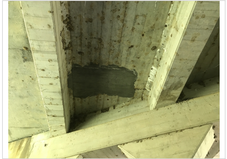
Span # 3 Bay # 2 deck repair.
