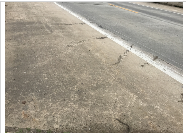
Left side of Span # 2. Transverse cracks.
