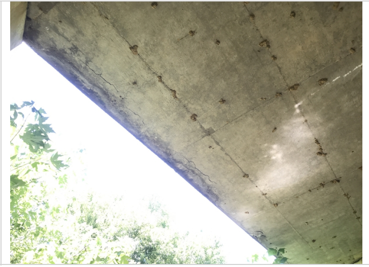
Span # 2 Rt concrete delamination's along the edge of the slab.
