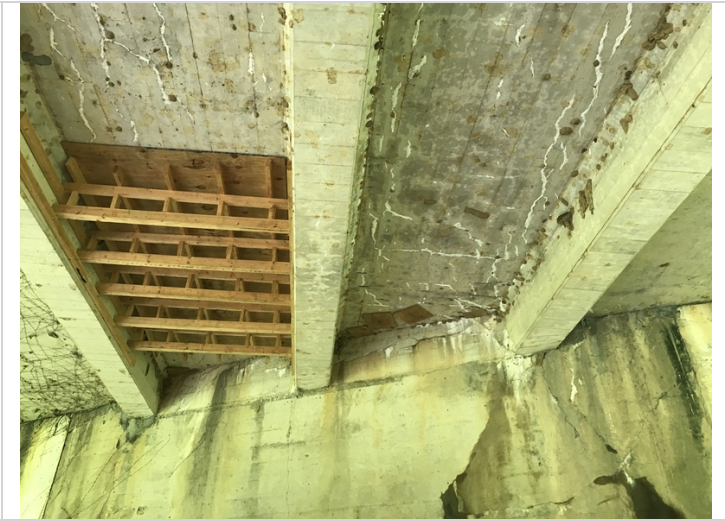
Span # 3. Adjacent to Bent # 4. Spalls with exposed reinforcing steel and full depth repairs with temporary form work left in place.
