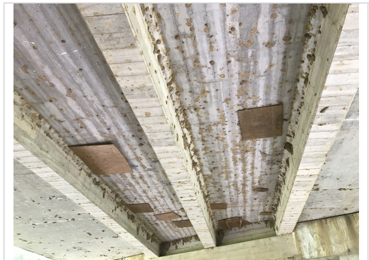
Deck soffit span # 2. Several full depth repairs with temporary form work left in place.
