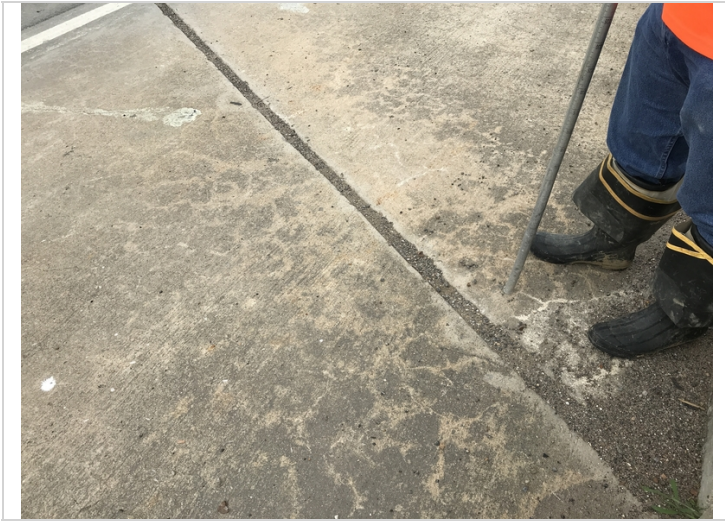
Hairline map cracking in the gutters.
