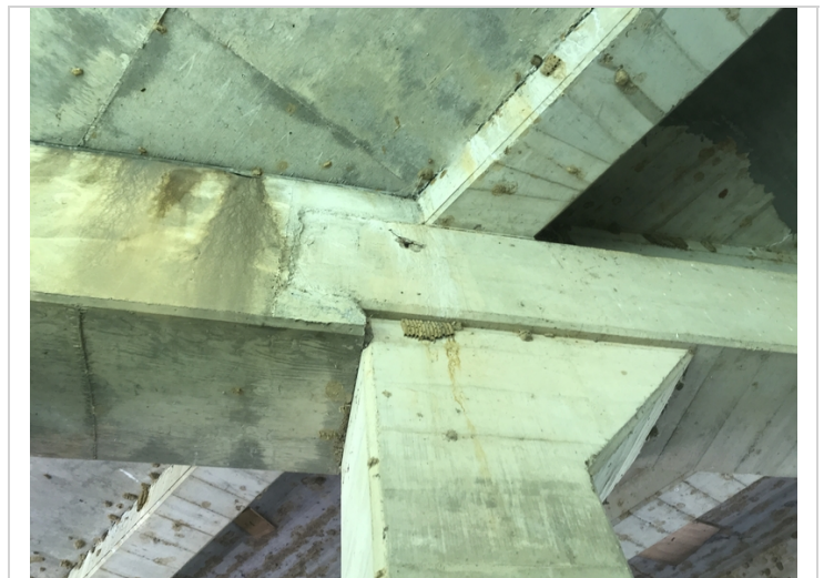
Bent # 3 over Col # 5 spalling with exposed reinforcing steel.
