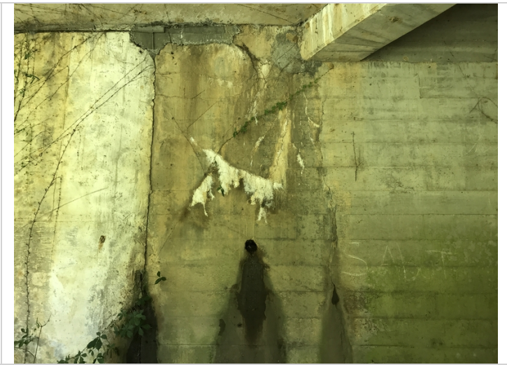
Bent # 1 Rt at Girder # 3 cracking with efflorescence and repairs.
