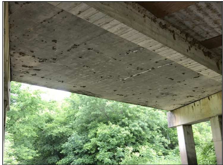
Left slab soffit of Span # 2. Delaminated areas along edge of slab.
