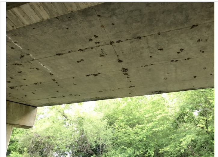
Right slab soffit. Span # 2. Delaminated areas along edge of slab.
