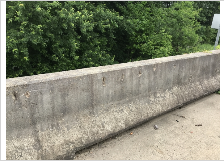
Several Spalls with exposed reinforcing steel in the Left parapet of Span # 3.
