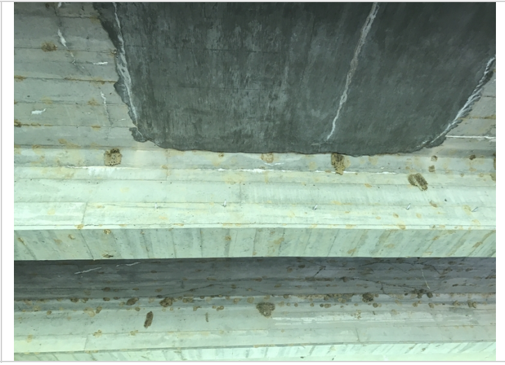
Span # 1 Girder # 2 longitudinal cracking near mid span with efflorescence.
