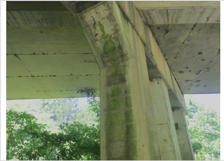
Bent # 2 column # 3 vertical cracking and concrete delamination's.
