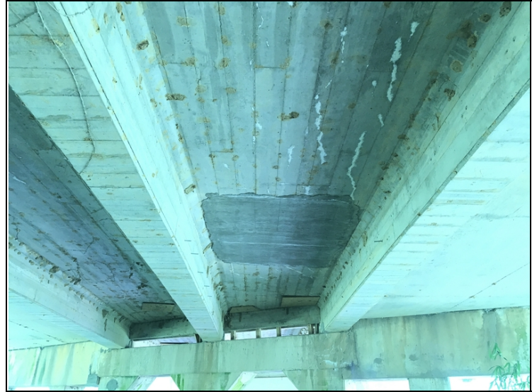
Span # 1 Bay # 3 cracking with efflorescence.
