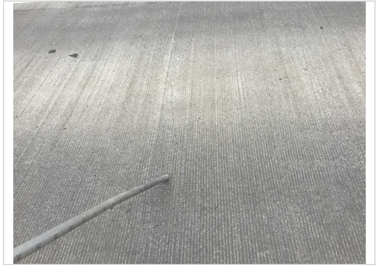
Transverse crack in the wearing surface of the deck.
