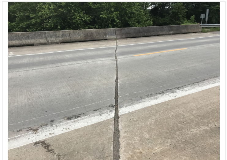
Expansion joint over Bent # 2. Typical.
