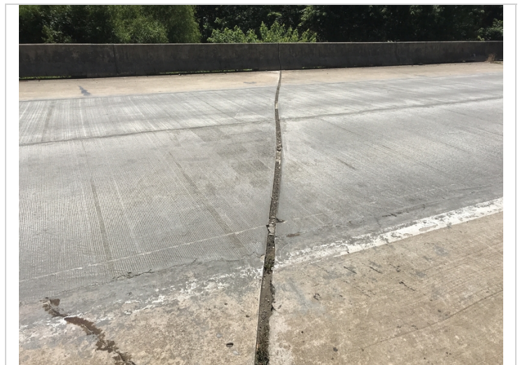
Bent # 2 & 3 poured joint seals.
