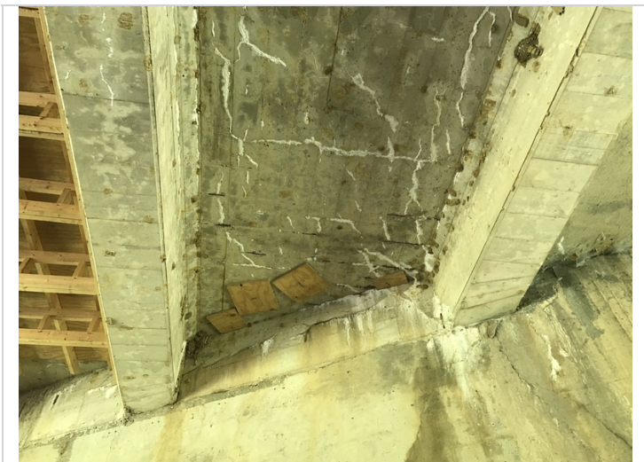
Span # 3 Bay # 2 exposed reinforcing steel.
