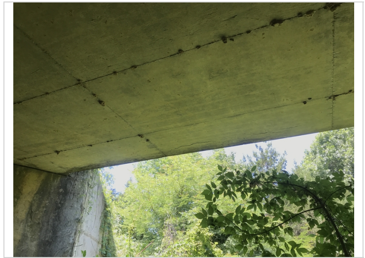
Span # 1 Lt concrete delamination along the slab edge.
