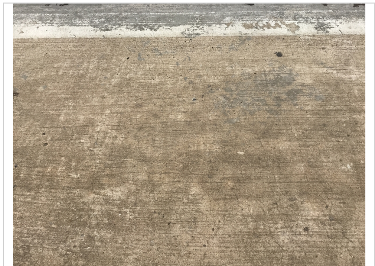
Typical map cracking on the concrete slab spans.
