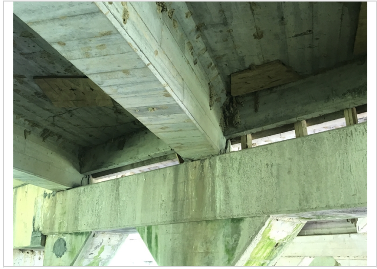
Span # 1 Bent # 2 spalling at the ends of the girders.
