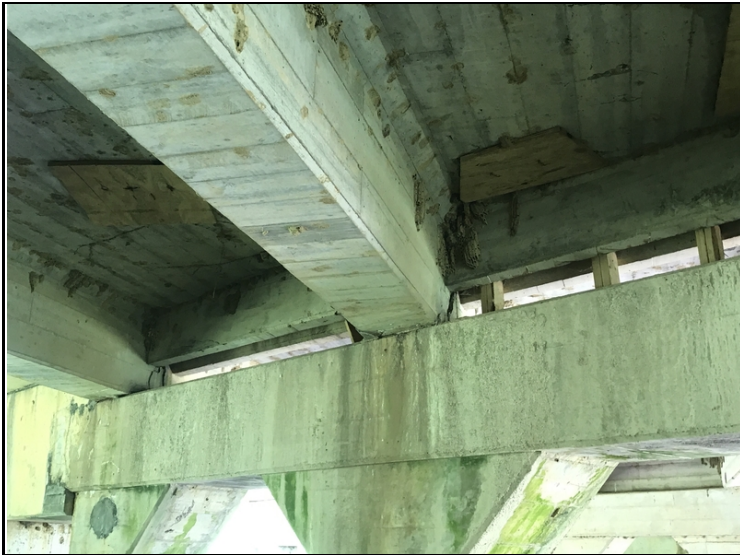
Span # 1 Bent # 2 spalling at the ends of the girders.
