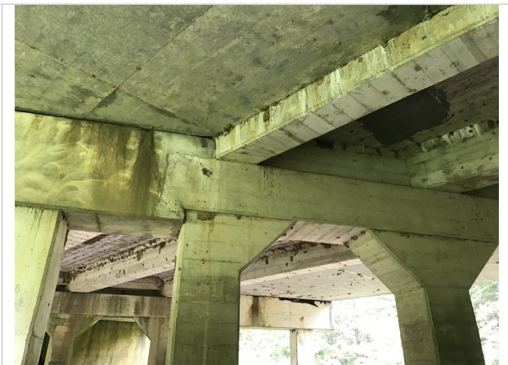
Spall with exposed reinforcing steel in span # 3 side of Bent # 3 under Girder # 3.
