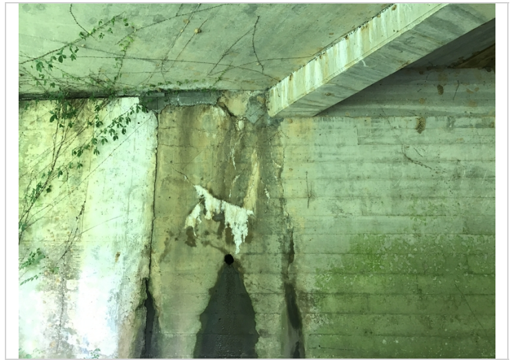
Diagonal and map cracking with efflorescence and grouted repairs adjacent to girder # 3 in Bent # 1.
