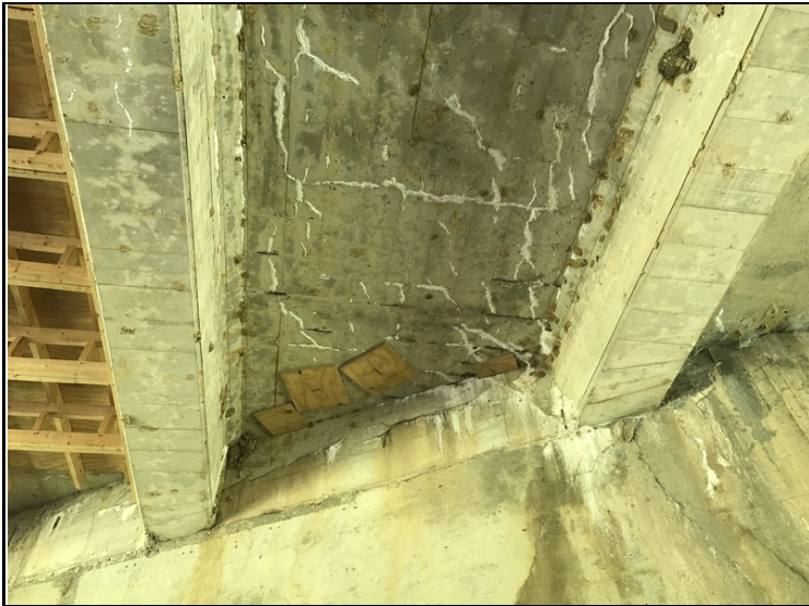
Span # 3 Bay # 2 exposed reinforcing steel.
