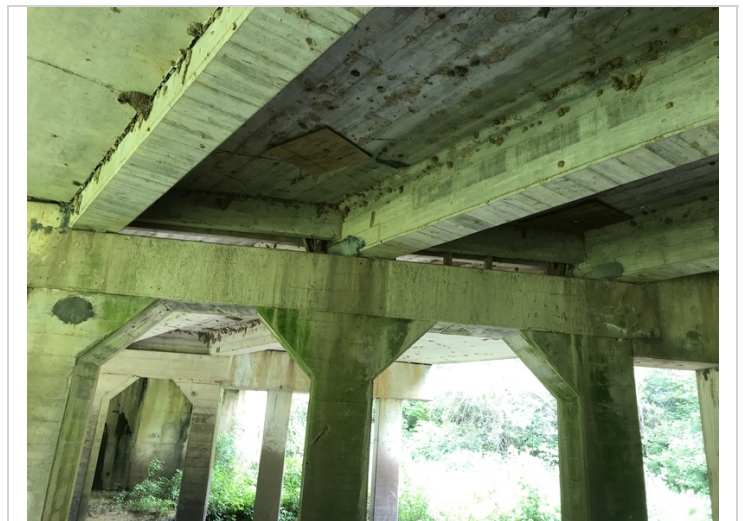
Grouted repairs in Span # 1 girders over Bent # 2.
