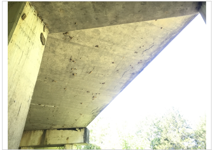
Span # 2 concrete delamination along the Left edge.
