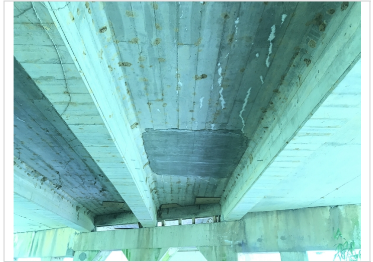
Span # 1 Bay # 3 deck repair.
