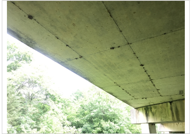
Left slab soffit. Span # 1. Delaminated areas.
