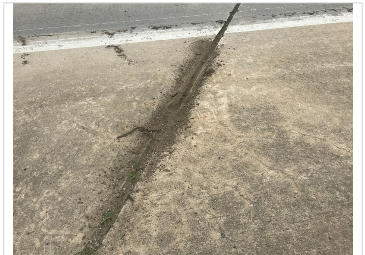
There is dirt accumulation in the slab span portions of the joints.
