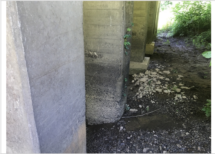
Bent # 3 column with medium abrasion.
