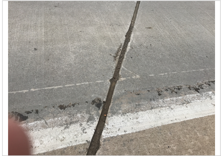
There are scrape marks in the edge of the Left Lane with shallow spalls at the expansion joints.
