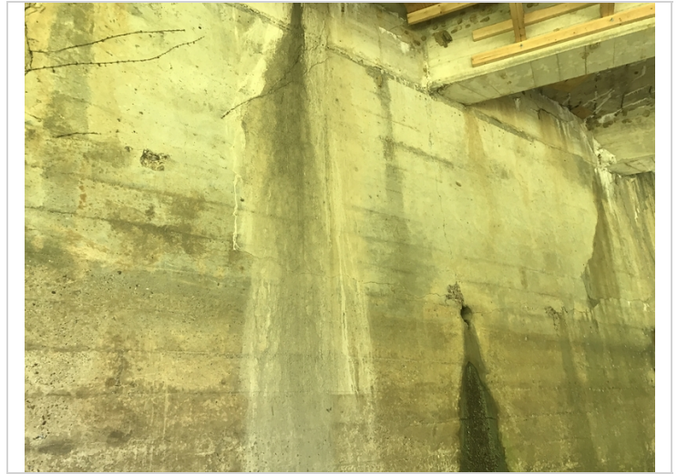
Bent # 4 Vertical and horizontal cracking.
