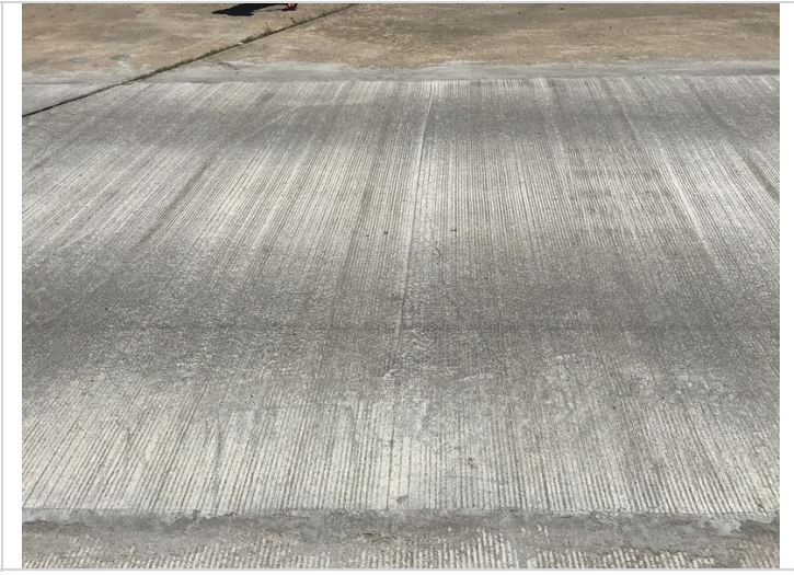
Sealable cracking on the new driving surface of the deck.
