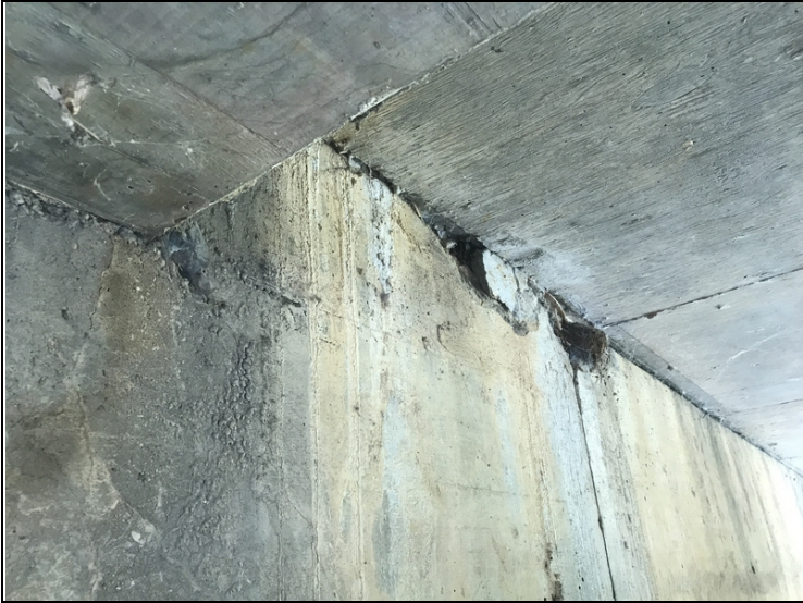
Bent # 1 spalling with exposed reinforcing steel.
