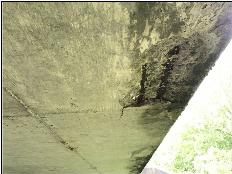
Left deck soffit. Spall with exposed reinforcing steel.
