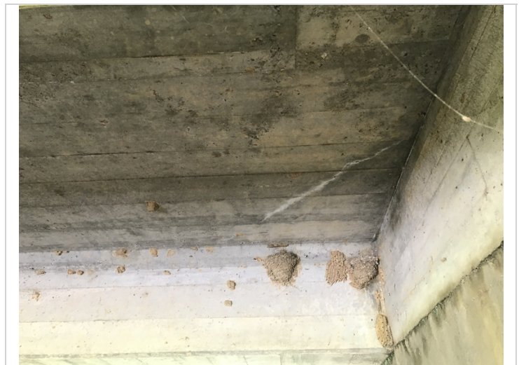
Diagonal hairline crack with light efflorescence in the deck soffit adjacent to Girder # 1 at Bent # 2.
