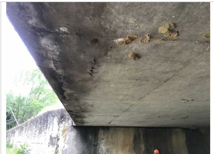
Delaminated area in the Right slab soffit.
