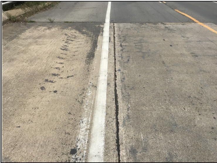
Missing joint sealant.
