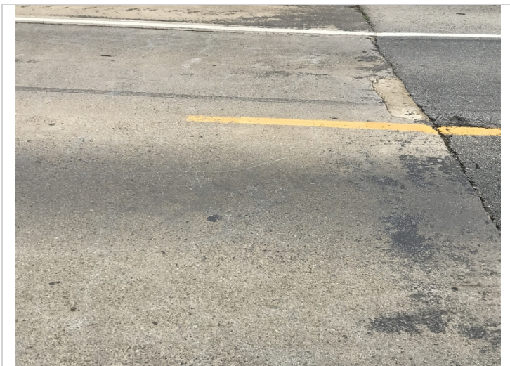
Patched area in the wearing surface of the deck located in the Right lane over Bent # 1.
