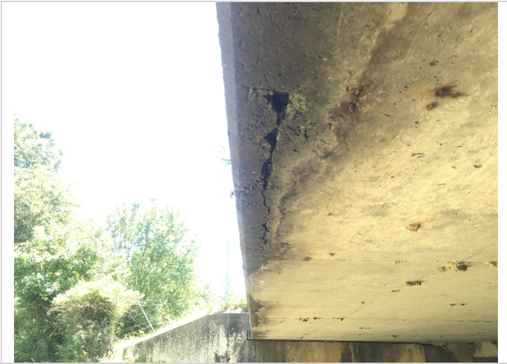
Spalling with exposed reinforcing steel and delaminated concrete along the right side.
