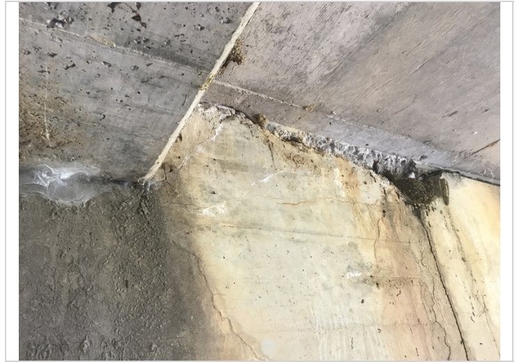
Bent # 2 Lt cracking with efflorescence.
