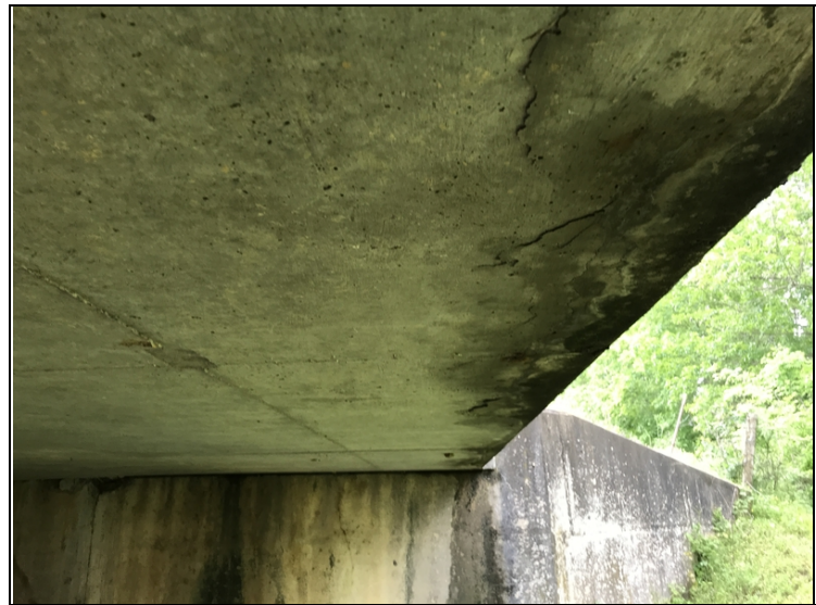
Left edge of deck soffit. Delaminated areas. Typical along both edges of the structure.
