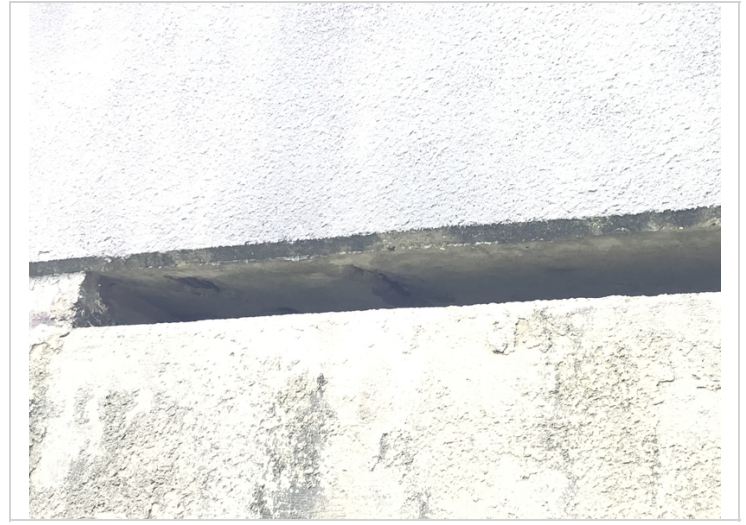
Spalls with exposed reinforcing steel inside the drain openings of the parapet walls.
