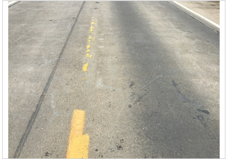
Rigid concrete wearing surface over the original T Beam portion of the deck.
