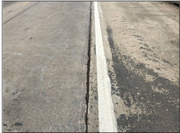
Missing sealant in the longitudinal construction joint.
