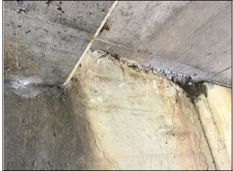
Bent # 2 Lt cracking with efflorescence.
