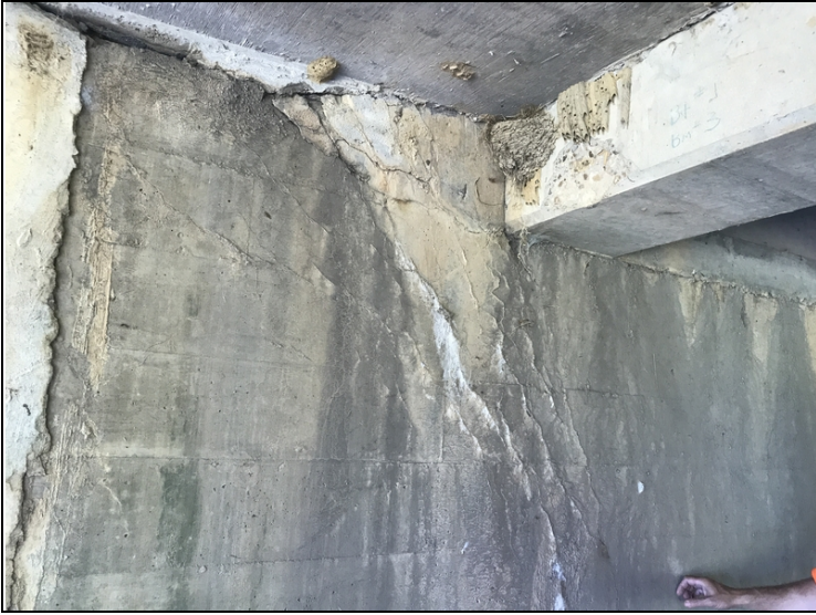
Bent # 1 Rt cracking with efflorescence buildup.
