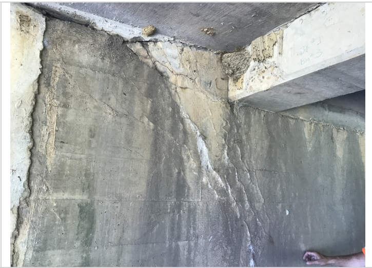
Bent # 1 Rt cracking with efflorescence buildup.
