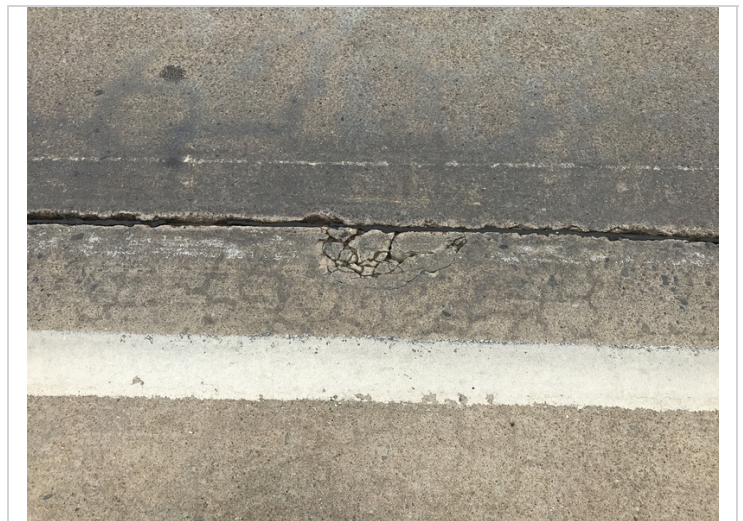
There is a 12" area that is breaking apart along the Left longitudinal construction joint.
