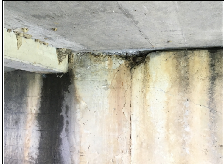
Bent # 2 adjacent to Girder # 3. Spall with exposed reinforcing steel.
