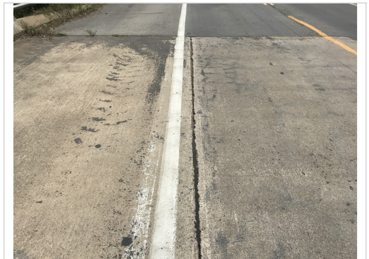
Missing joint sealant.
