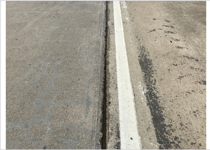
Longitudinal construction joint with missing sealant.
