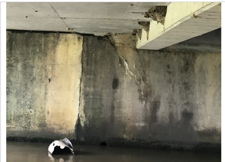
Spalling with diagonal cracking with efflorescence in the Right side of Bent # 1 adjacent to Girder # 3.
