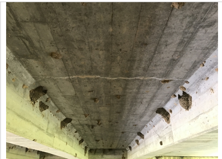
Transverse hairline crack in the deck soffit.
