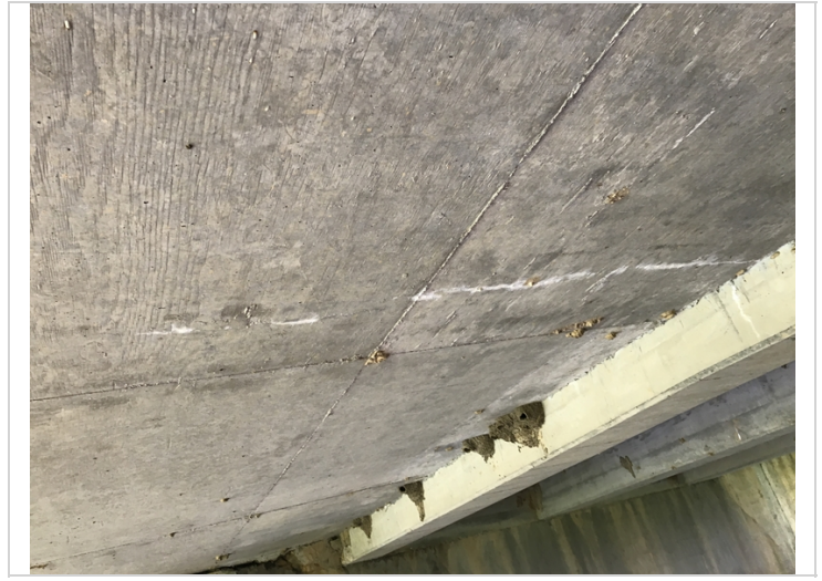
Transverse hairline crack with light efflorescence in the Right slab soffit.
