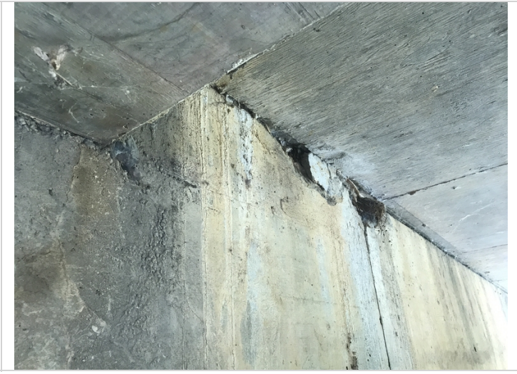
Bent # 1 spalling with exposed reinforcing steel.
