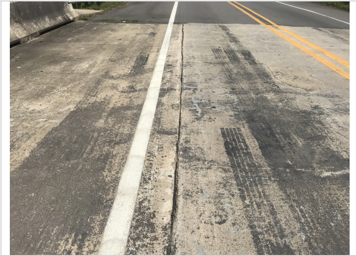
Failing joint sealant between the slab and wearing surface.
