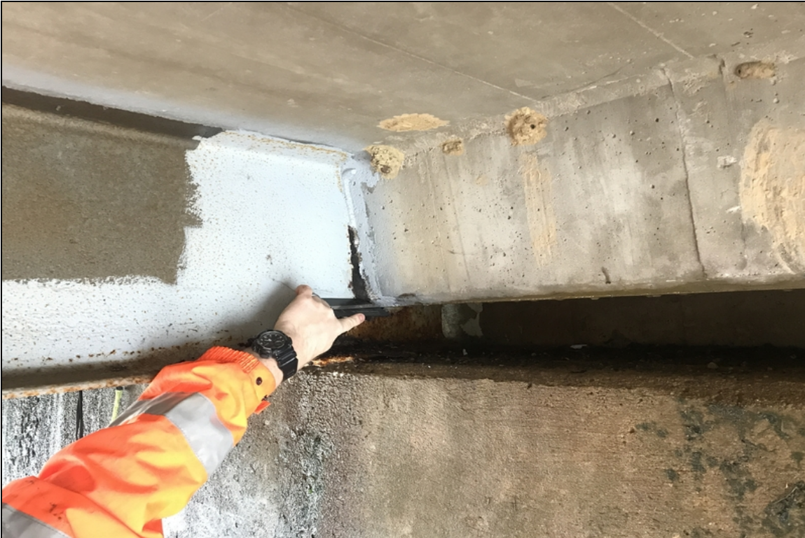
Bent # 1. Beam # 3. There is 1/4" section loss in the vertical face of the web adjacent to the expansion dam.
