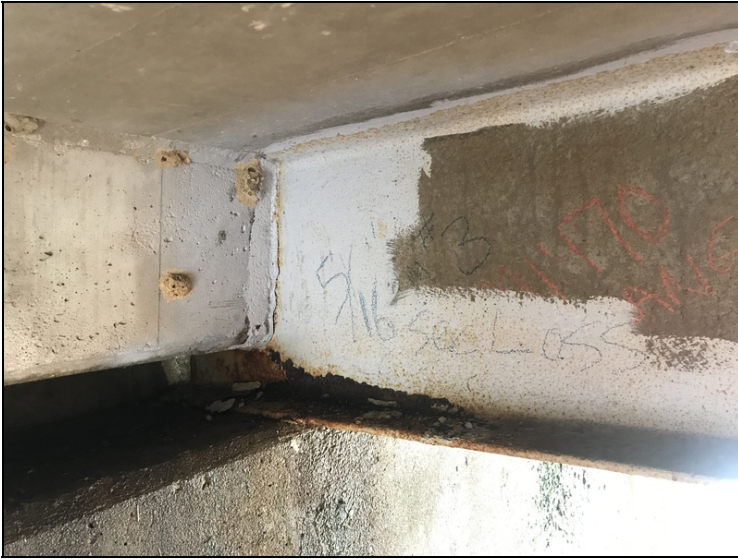
Bent # 1, Beam # 3 has 5/16" section loss to the base of the web.
