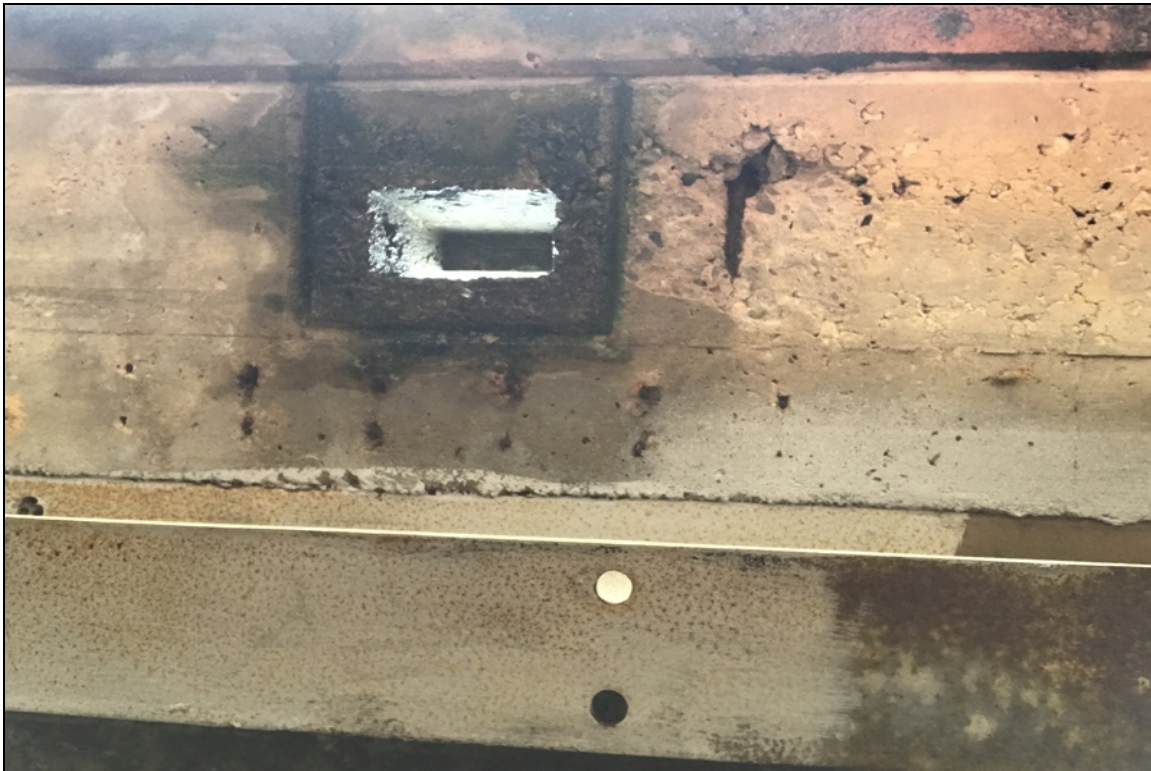
Spall with exposed reinforcing steel adjacent to the deck drains in Span # 2.
