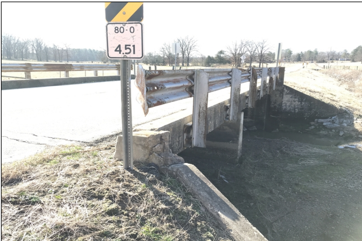
Bent # 3 Lt missing end post.
