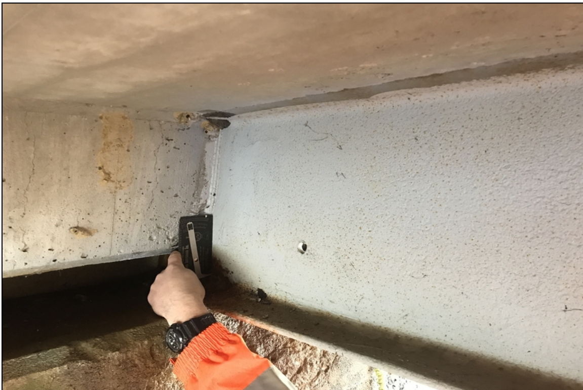
Bent # 3. Beam # 5. Base of web has 7/16" section loss.
