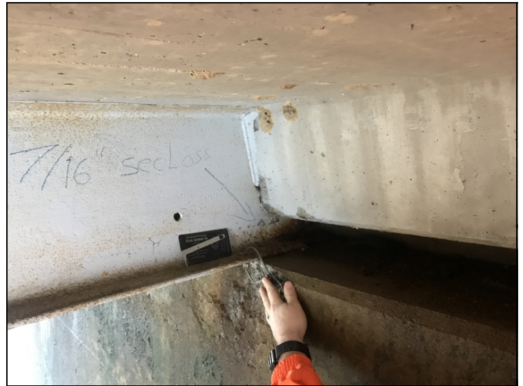
Active corrosion under the paint system has 7/16" section loss to the base of web. The bottom flange is reduced to 3/16".
