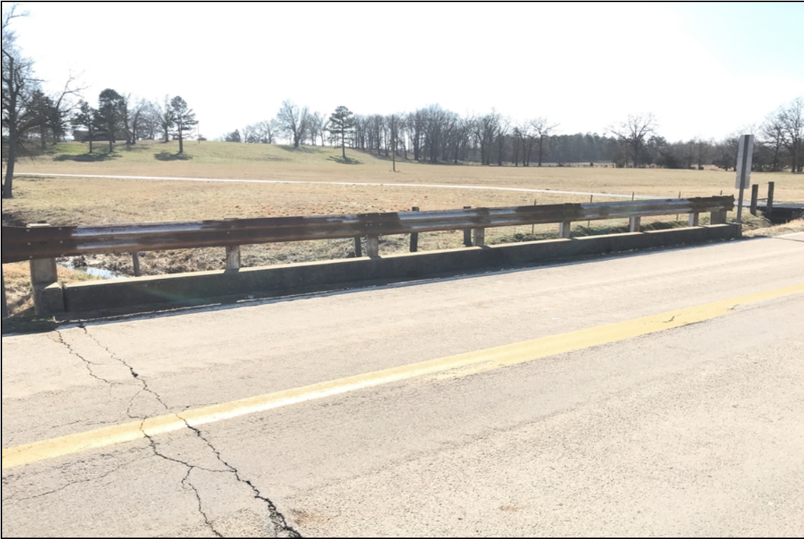
Failing paint system on the bridge rails.
