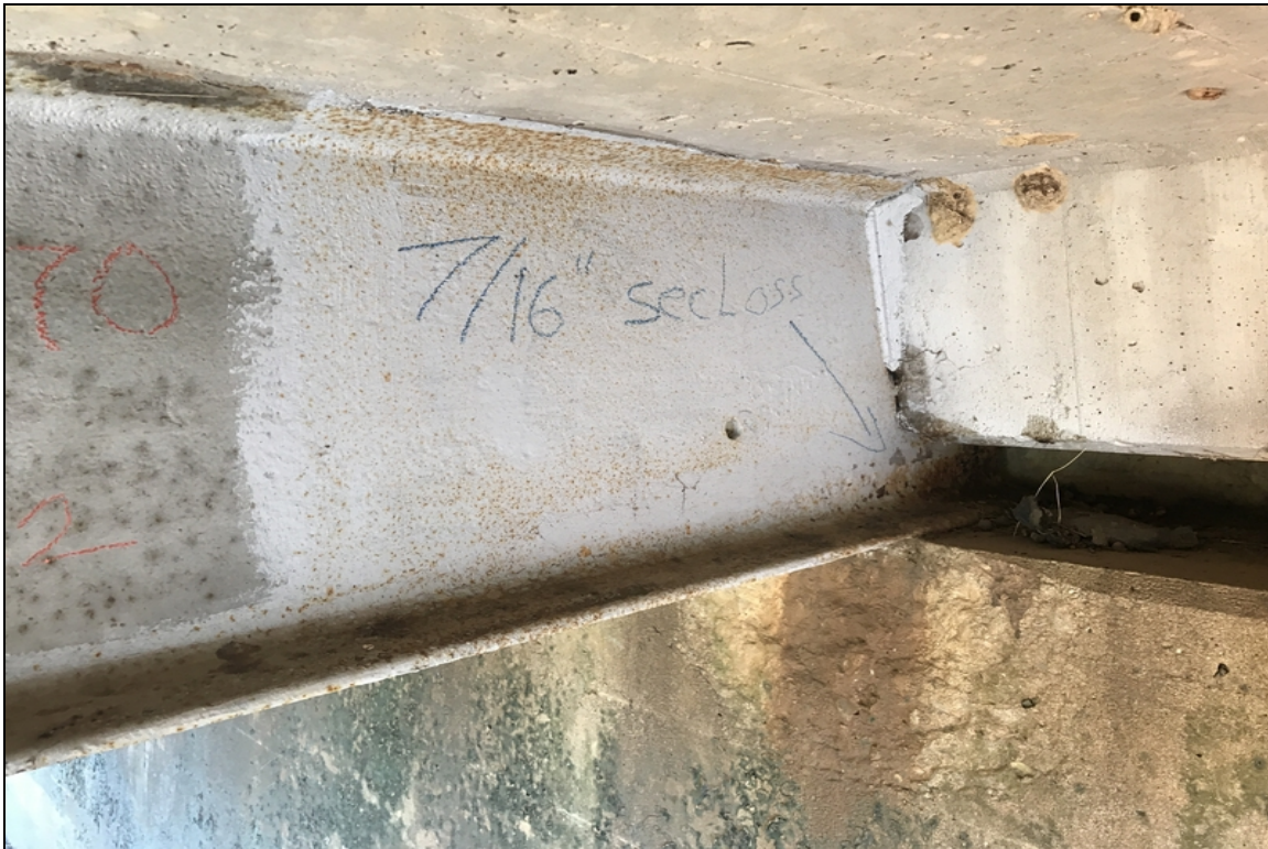
Beam # 5 at Bent # 3. Section loss.
