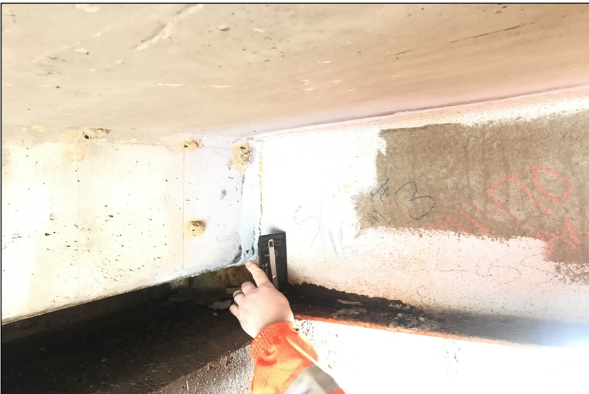
Beam # 3 at Bent # 1 has 5/16" section loss to the base of the web.
