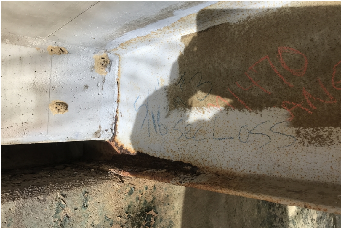
Bent # 1. Beam # 3. Corrosion with section loss.
