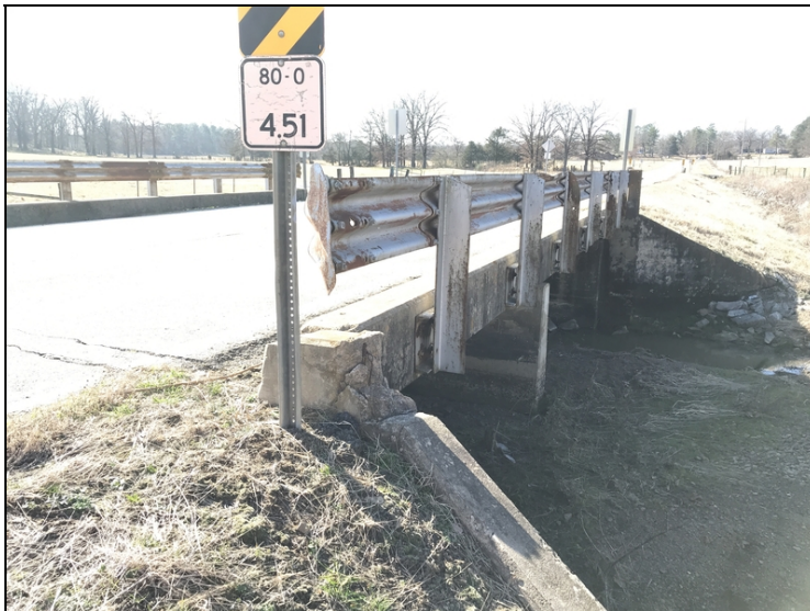
Bent # 3 Lt missing end post.
