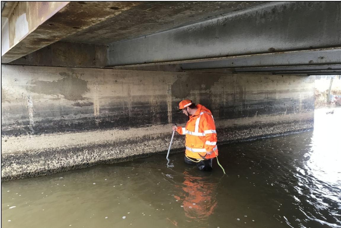
Bent # 2. Back face. Typical. Wading and probing substructure.
