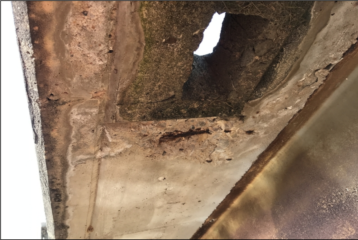
Spall with exposed reinforcing steel adjacent to the Right deck drain in Span # 2.
