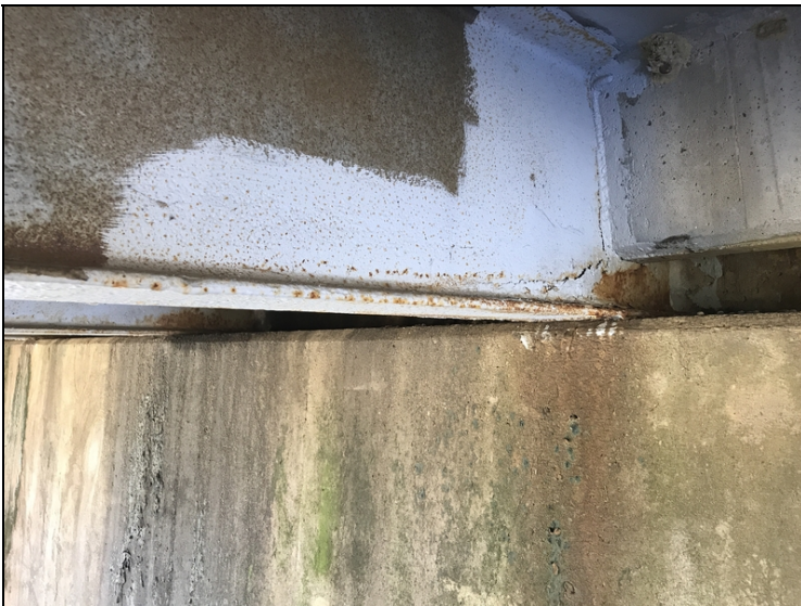
Bent # 1 Beam # 3 active corrosion with layers of flaking rust at the ends of the beams.
