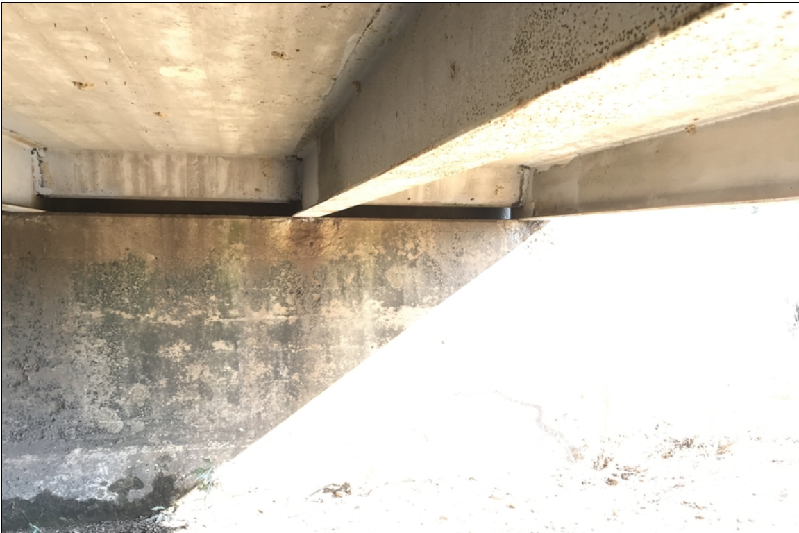
Bent # 3 spalling in the bearing area of beams # 1, 5, & 6.
