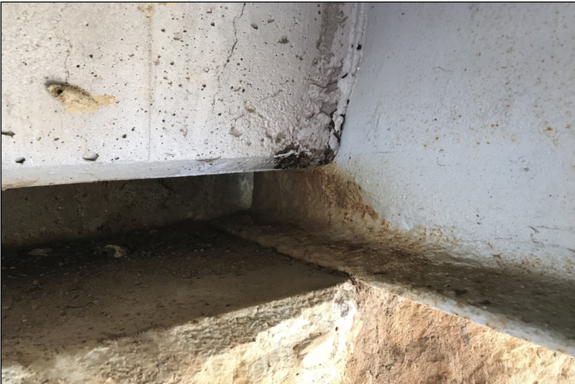
Old section loss scars.
