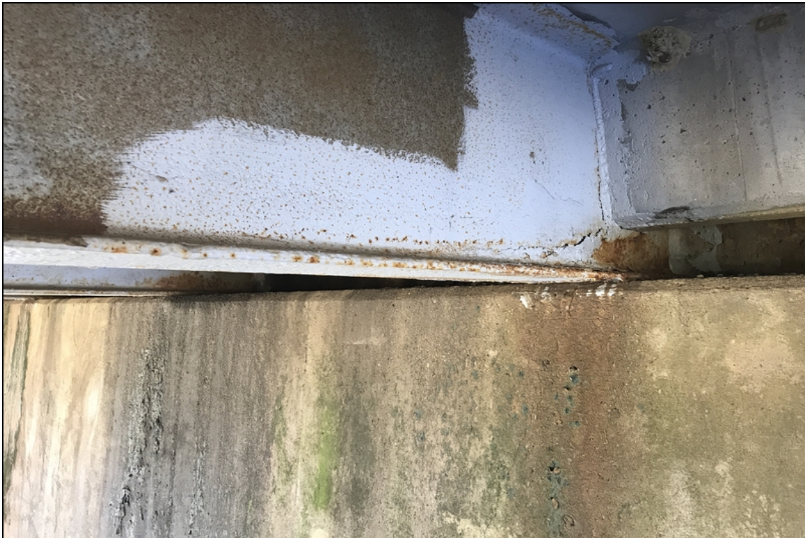
Bent # 1 Beam # 3 active corrosion with layers of flaking rust at the ends of the beams.
