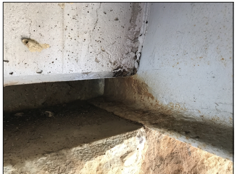
Old section loss scars.
