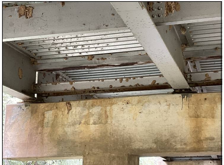
Bent # 3 bearing corrosion.
