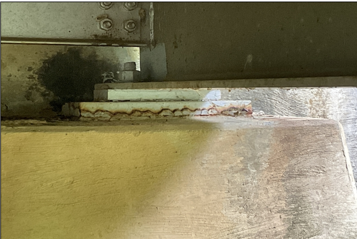
Bent # 4. Beam # 4 bearing corrosion showing through the paint system.
