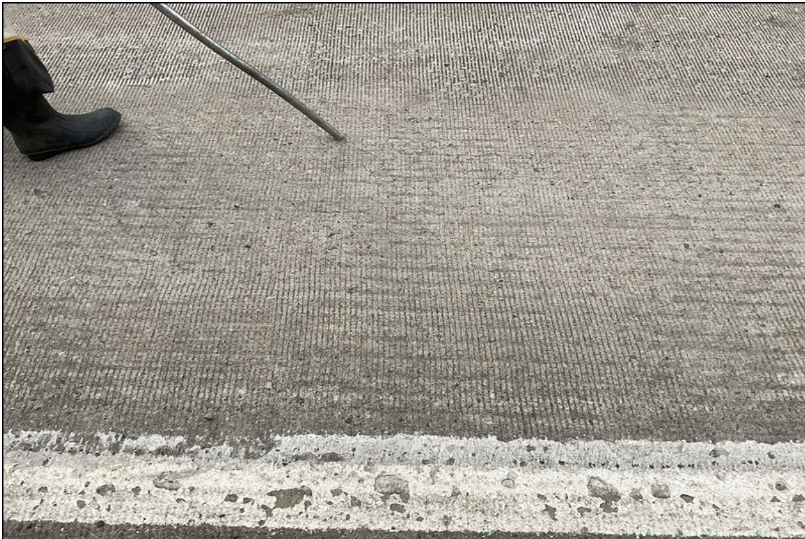
Transverse crack in Span # 1.
