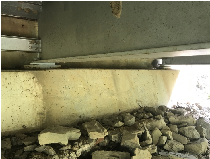
Bent # 4 Beams # 3 & 4 active corrosion with layers of flaking rust on the masonry plates.
