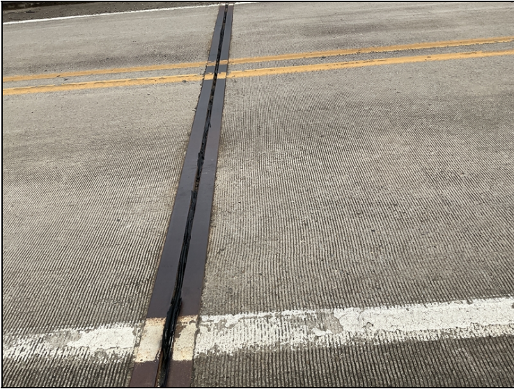
Bent # 3 expansion joint seal.
