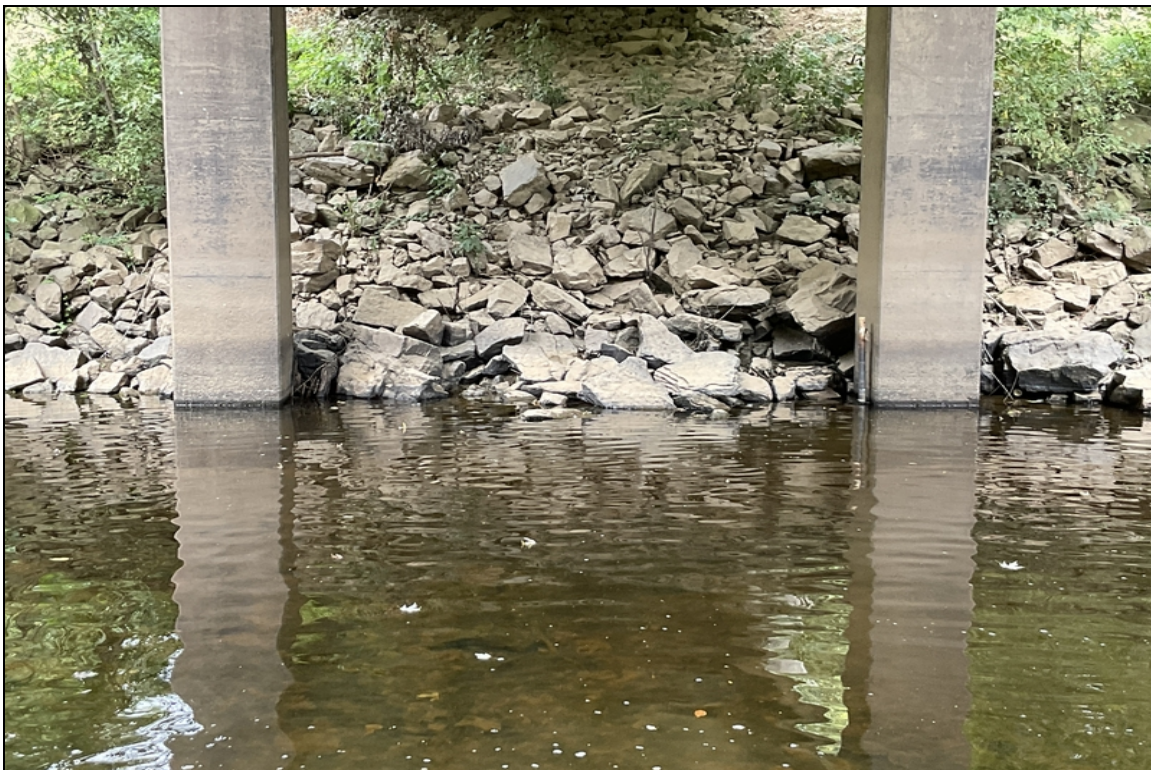
Light abrasion at the base of Bent # 2 columns.
