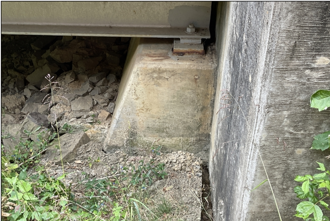
Hairline map cracking in the right end of Bent # 4.
