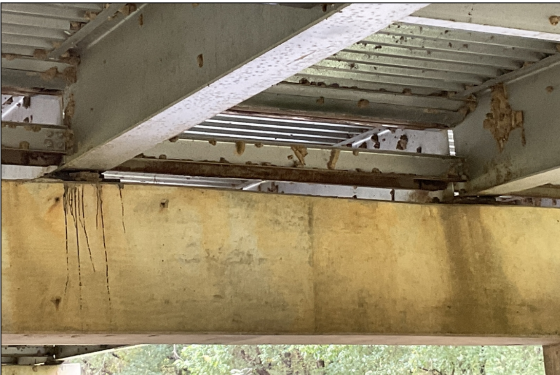
Span # 1 side of Bent # 2 - Expansion bearings. Typical.
