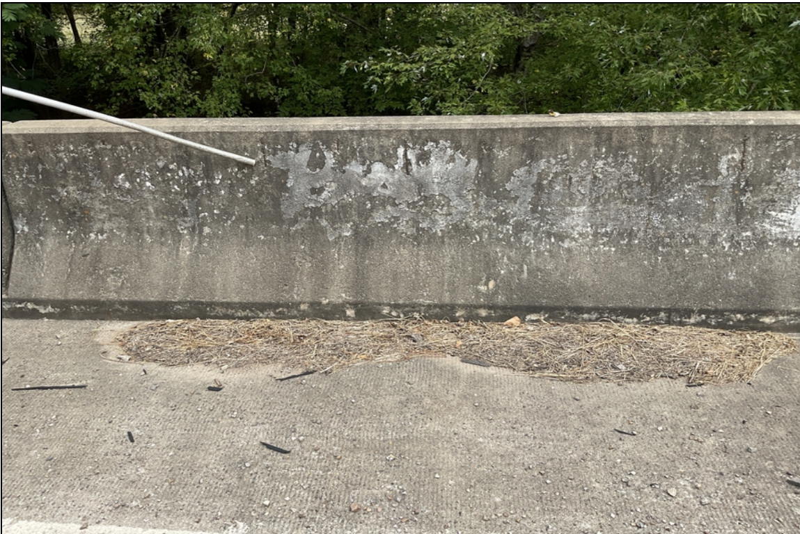
Spalls with exposed reinforcing steel in the Left parapet of Span # 1.
