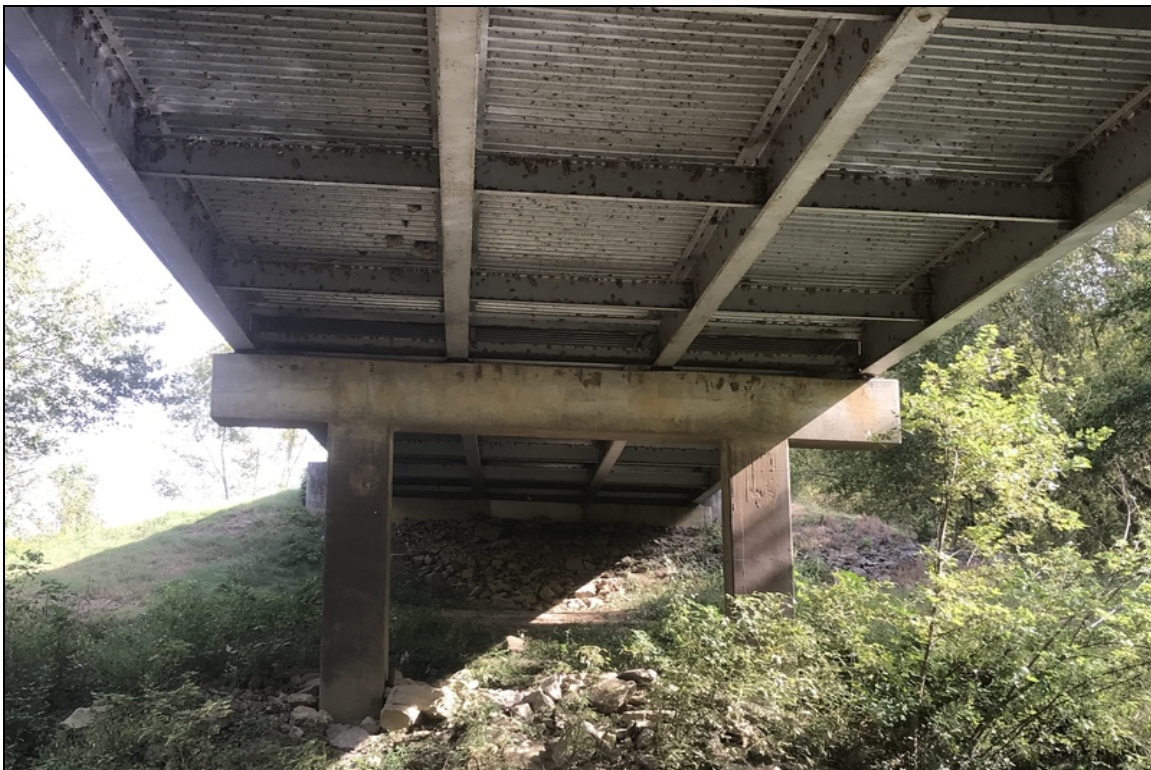
Typical cap staining from water leakage through the deck joints.
