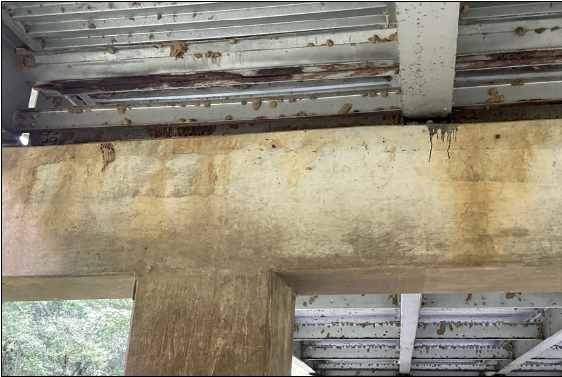
Horizontal crack in the Ahead face of Bent # 3 cap.
