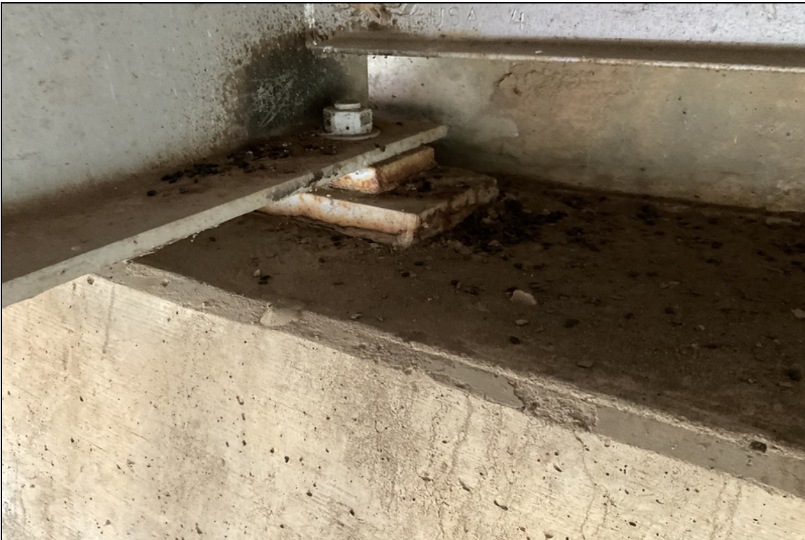
Bent # 1. Beam # 2 bearing. Typical.
