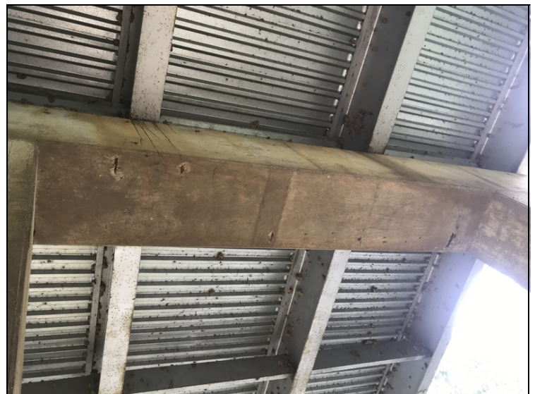
Bent # 2 shallow spalling with exposed reinforcing steel on the cap undersurface.
