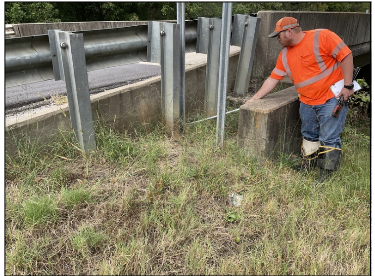
Void under the Northeast approach gutter.
