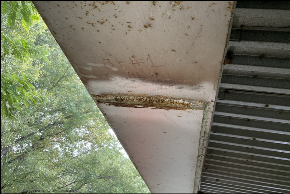
Welded repair to the end of the cover plate at Span # 1, Beam # 1 is still holding during this inspection.
