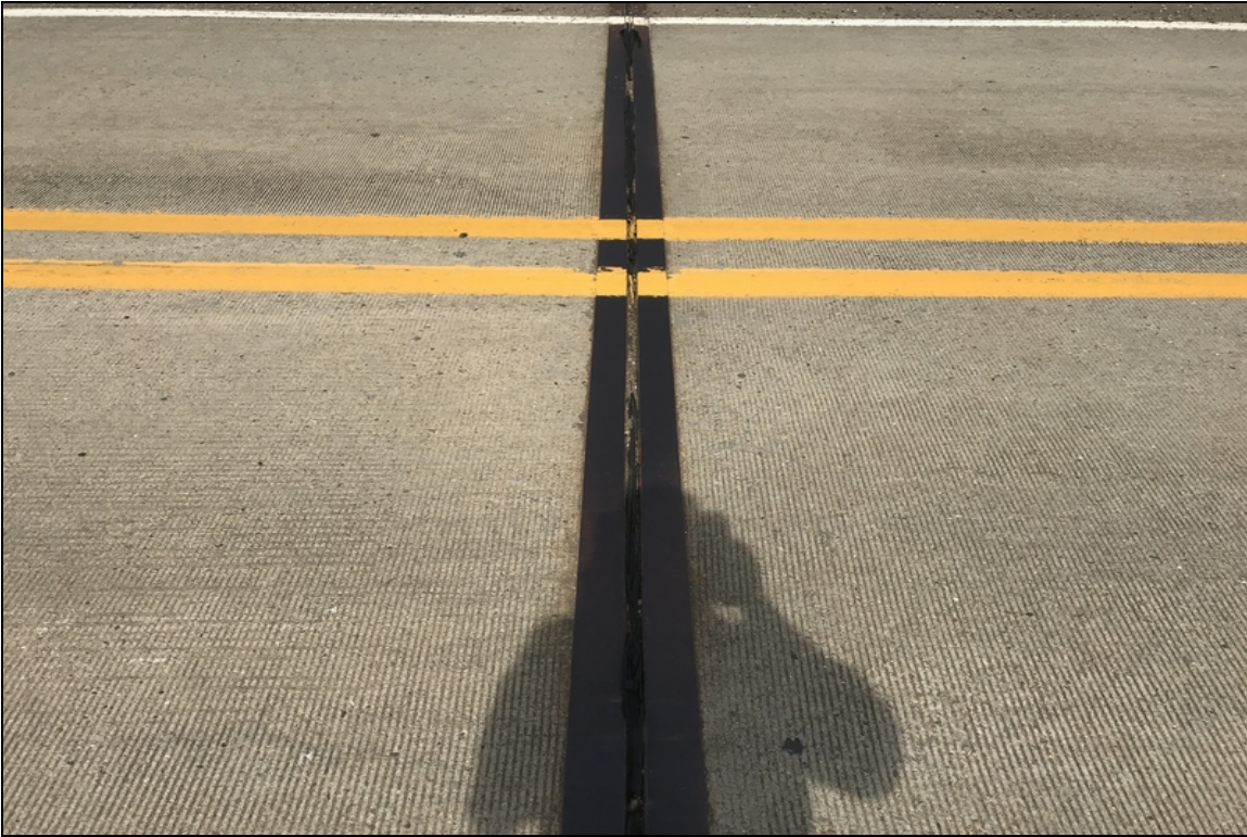
Bent 3 compression joint seal tears and partially missing.
