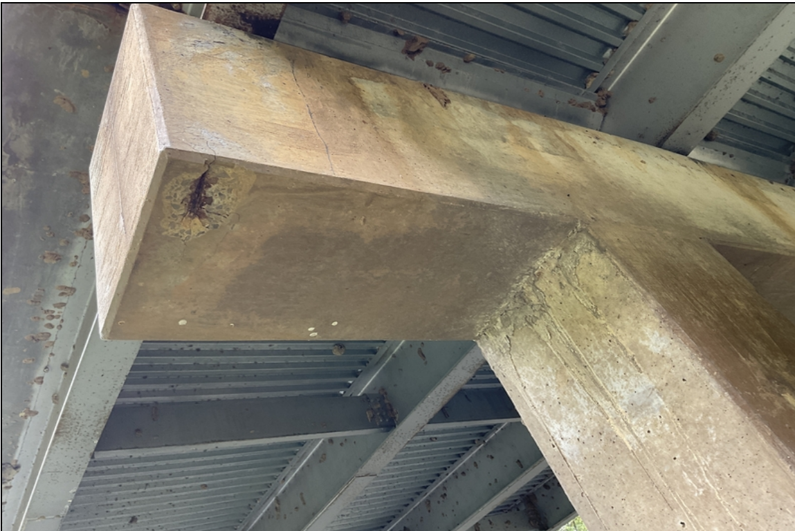
Right end of Bent # 3 cap. Undersurface. Spall with exposed reinforcing steel.
