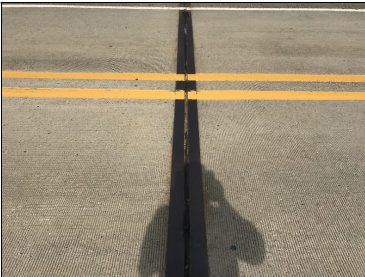
Bent # 3 compression joint seal tears and partially missing.
