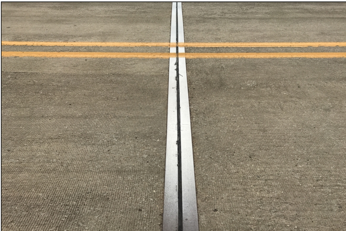
Bent 2 compression joint seal cracking.
