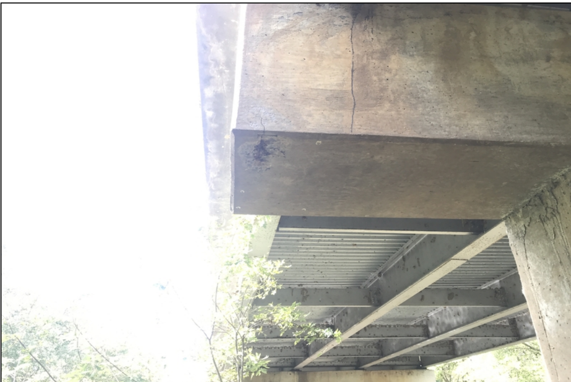
Bent 3 Rt cap undersurface spalling with exposed reinforcing steel.
