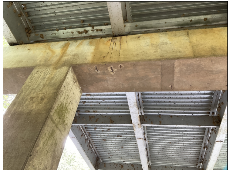
Undersurface of Bent # 2 cap. Spalls with exposed reinforcing steel.
