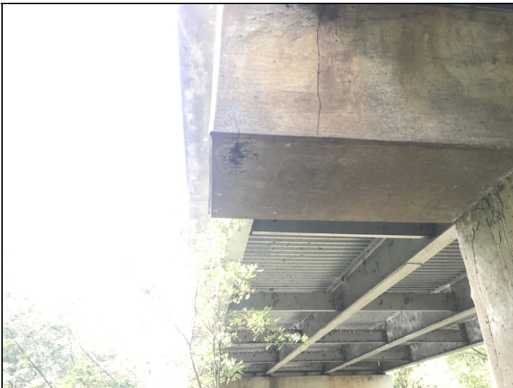
Bent # 3 Rt cap undersurface spalling with exposed reinforcing steel.
