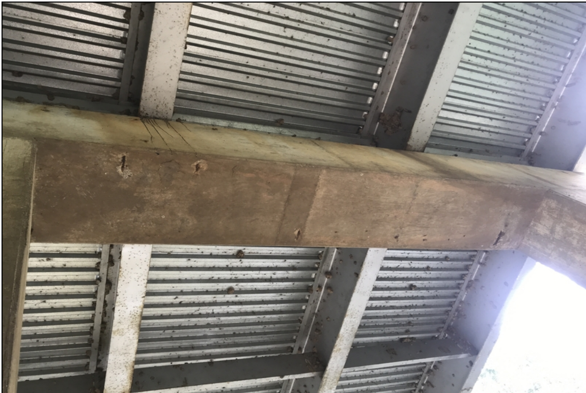
Bent 2 shallow spalling with exposed reinforcing steel on the cap undersurface.
