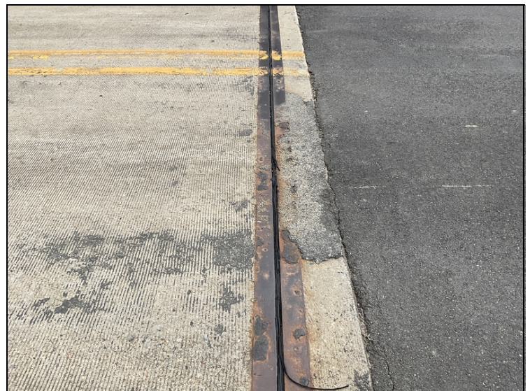
Bent # 4 compression joint seal tears.
