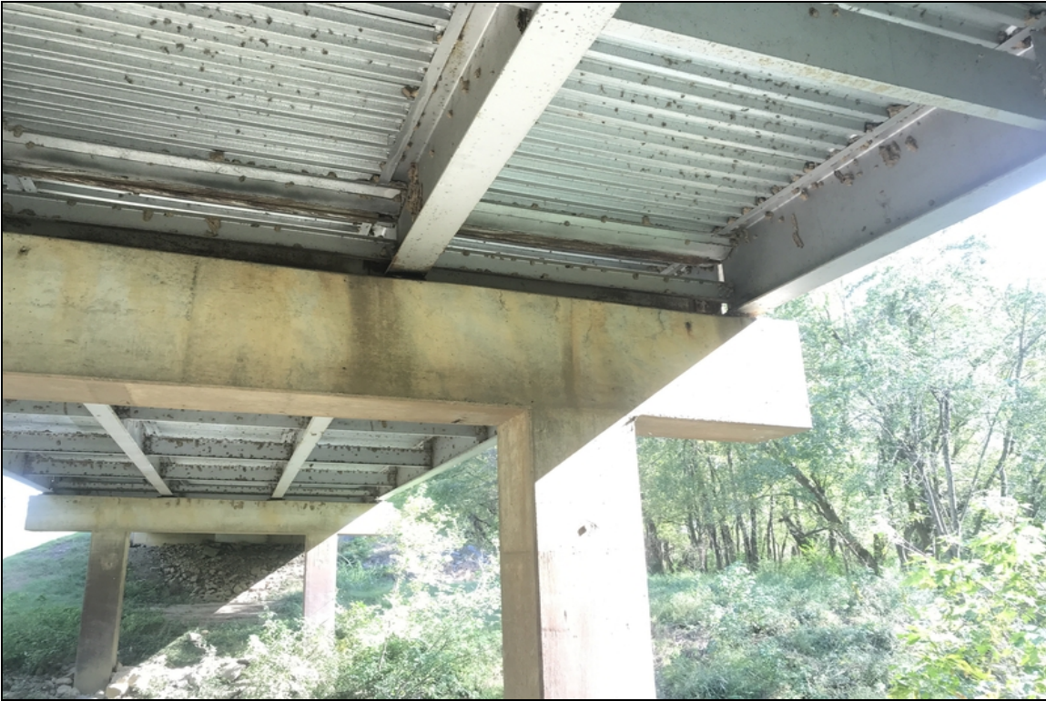
Typical vertical cracking in the caps.
