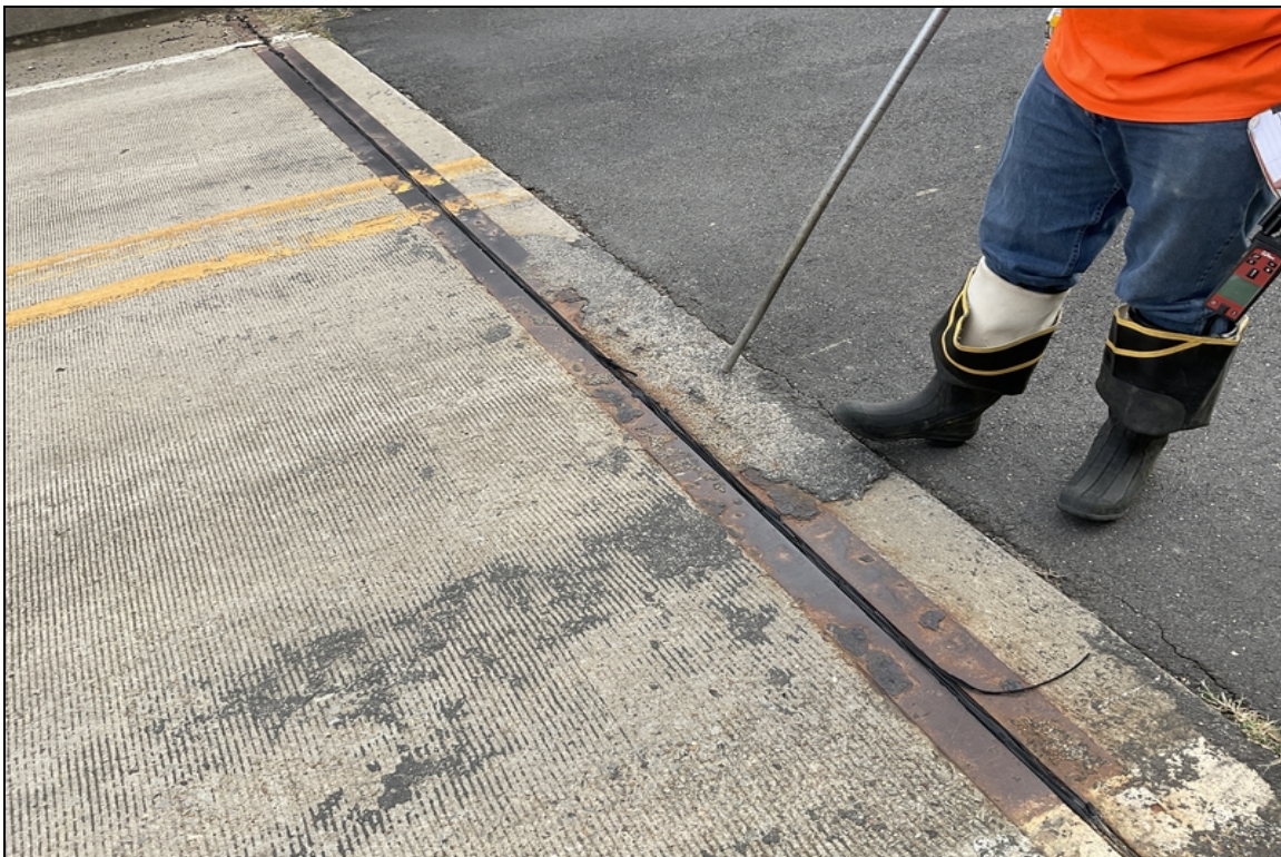
Torn expansion joint seal over Bent # 4.
