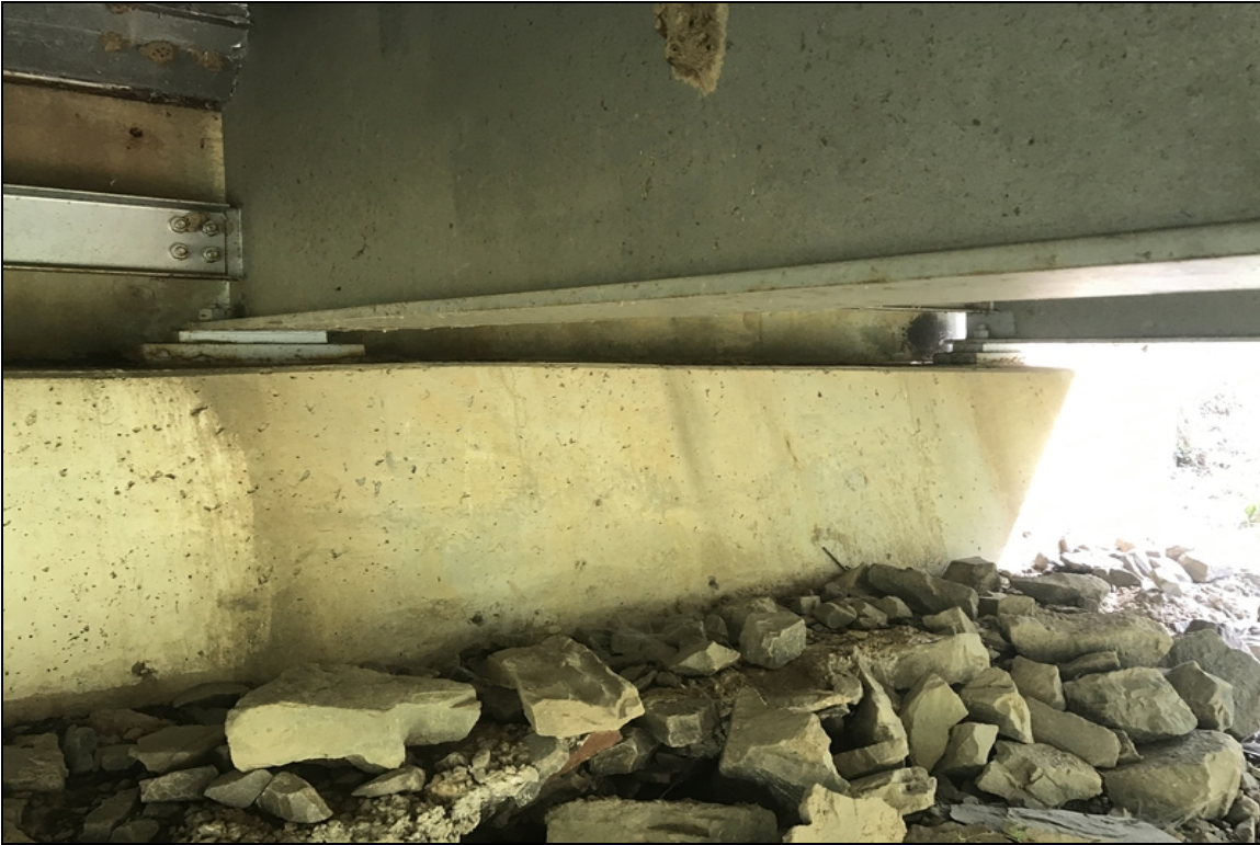
Bent 4 Beams 3 & 4 active corrosion with layers of flaking rust on the masonry plates.
