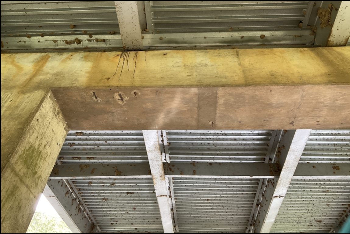
Undersurface of Bent # 2 cap. Spalls with exposed reinforcing steel.
