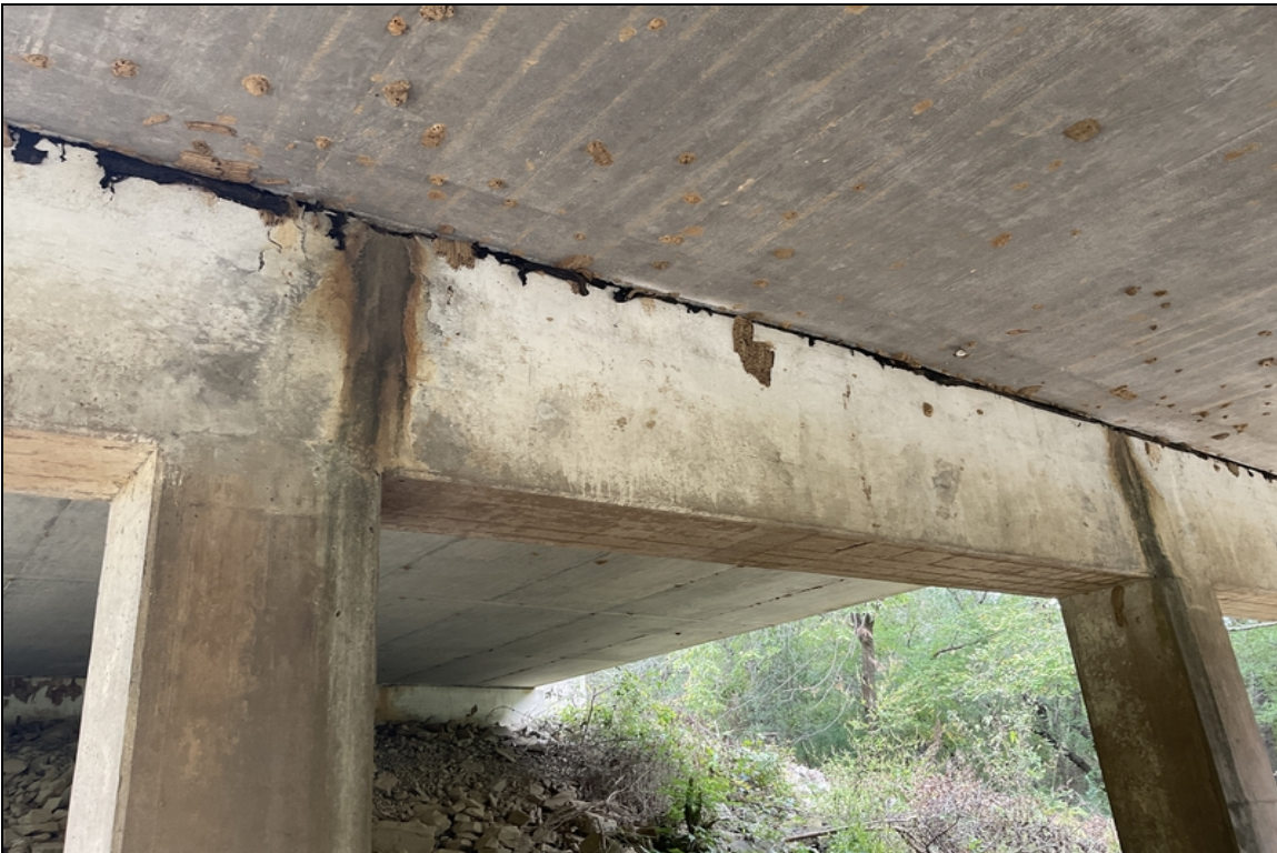
Staining and delaminated areas in the substructure caps from leaking deck joints.
