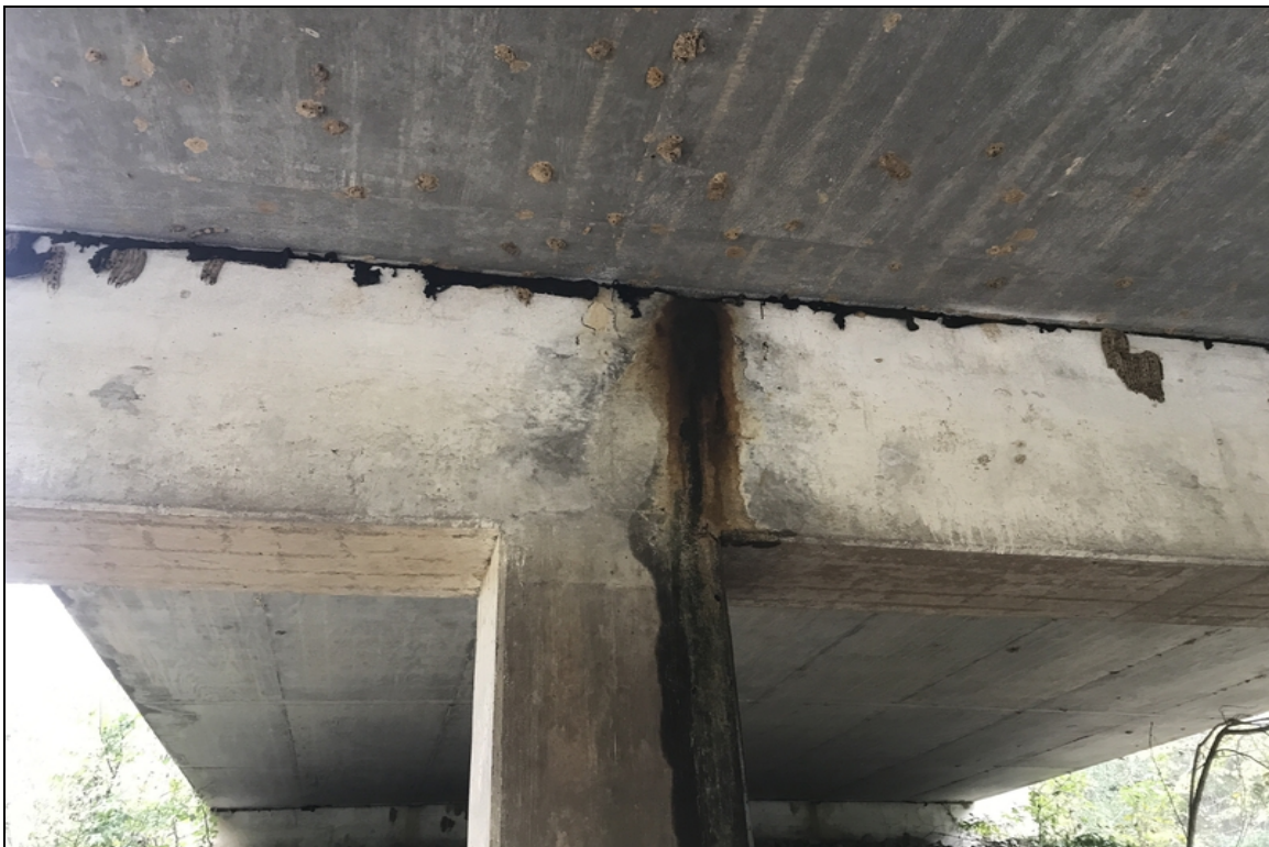
Span 2 Bent 2 Rt delaminated concrete.
