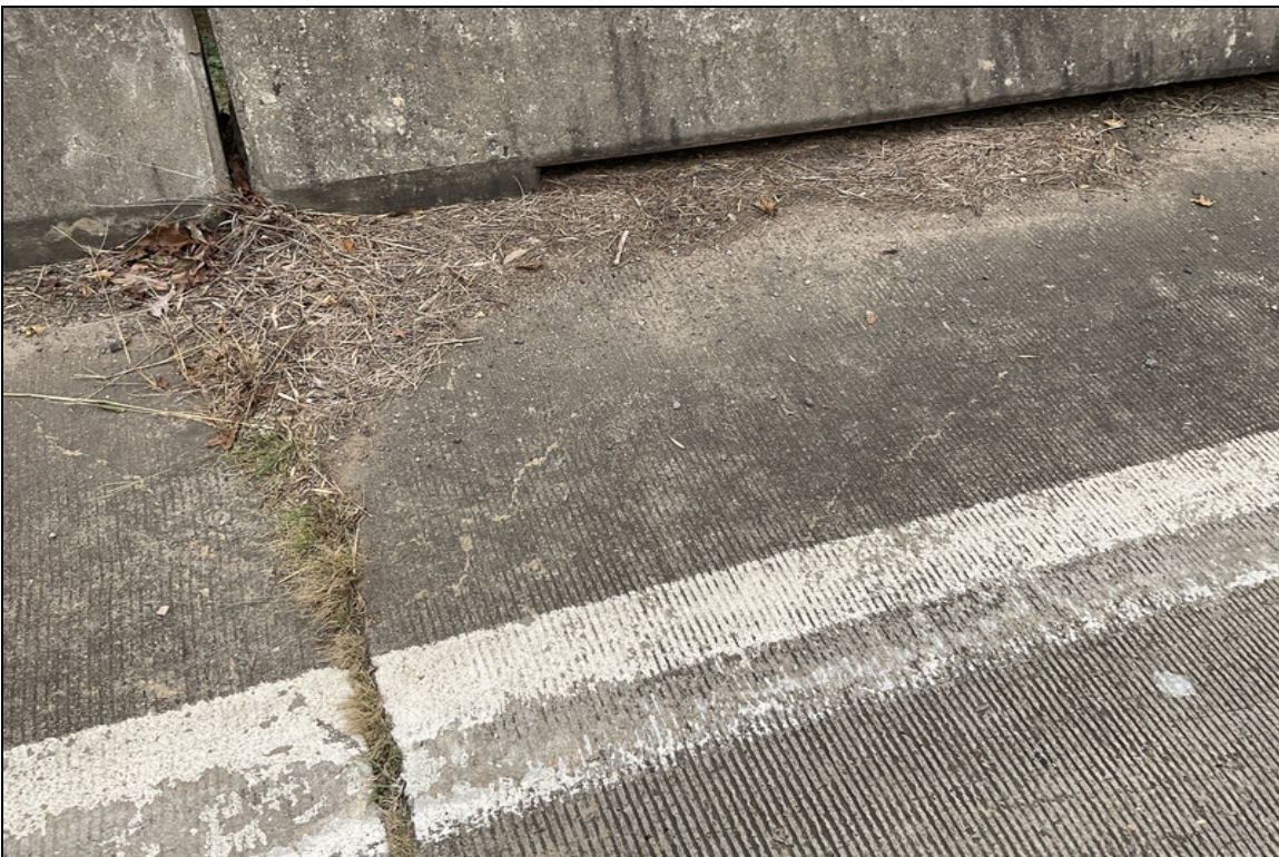
Hairline diagonal cracking in the corners of the slab spans.
