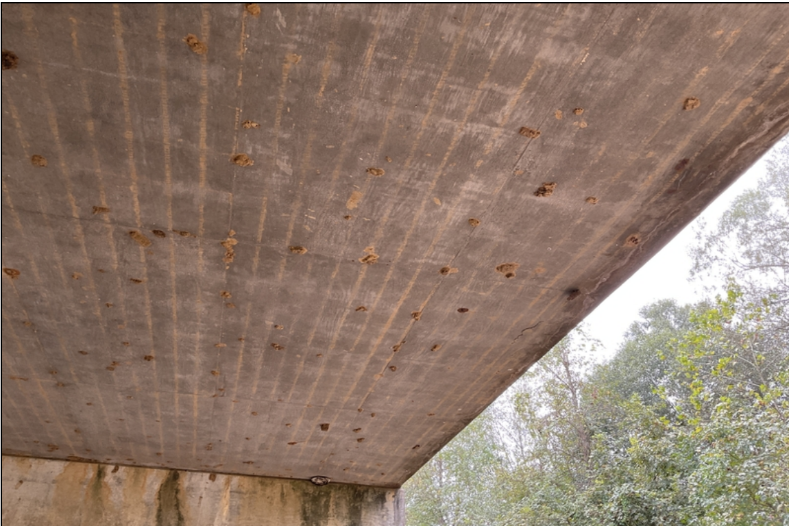
Span # 2. Right. Delaminated area on the undersurface of the slab.
