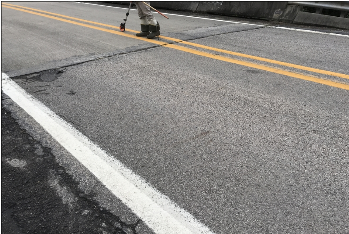
North approach asphalt settlement.
