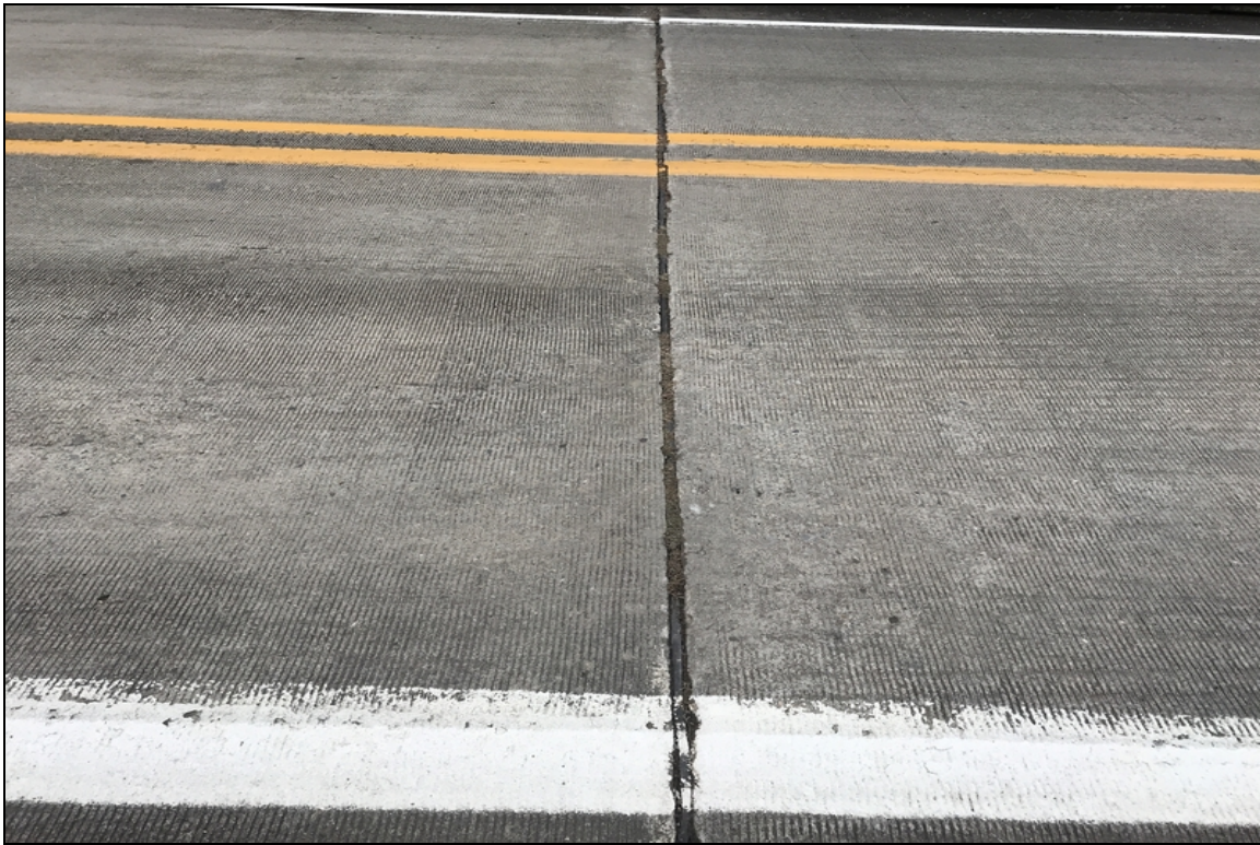
Bent 2 joint seal deterioration.
