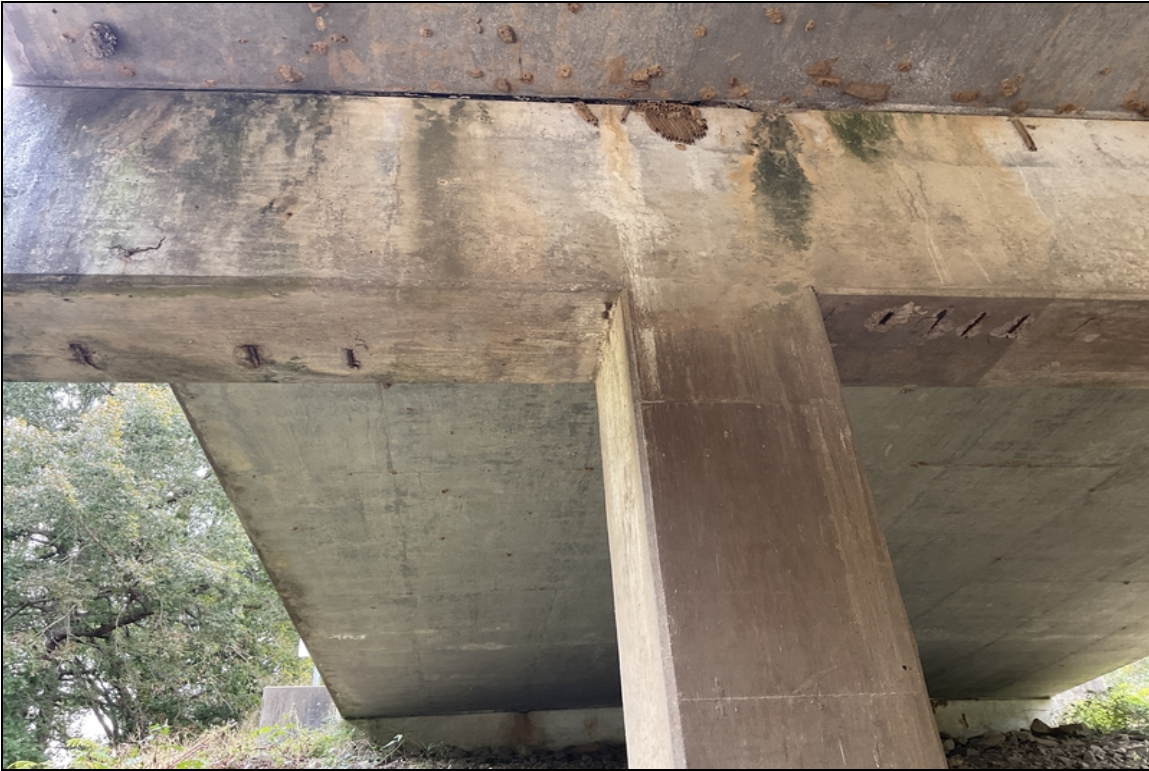
Spalls with exposed reinforcing steel on the undersurface of bent # 3 cap. Exposed reinforcing steel has up to initial section loss during this inspection.
