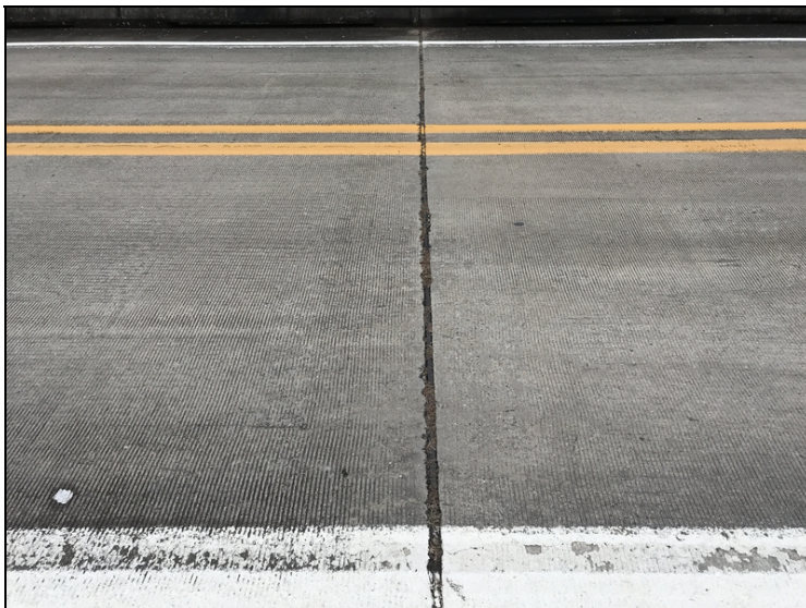
Bent # 3 failed joint seal.
