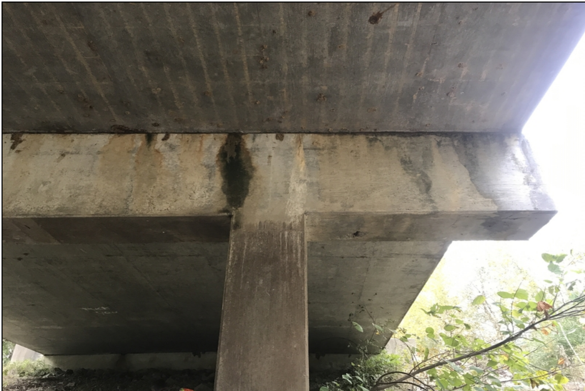
Typical vertical cracking with light efflorescence buildup over the exterior edge of the columns.
