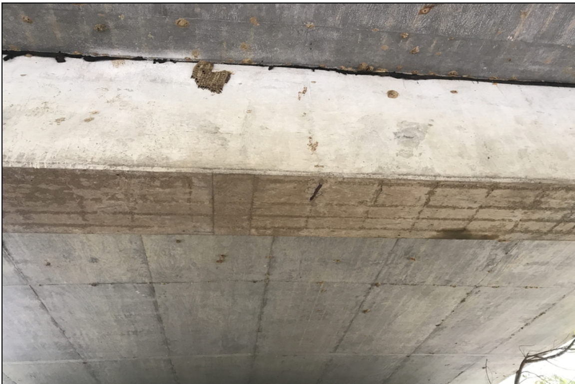
Bent 2 cap undersurface spalling with exposed reinforcing steel.
