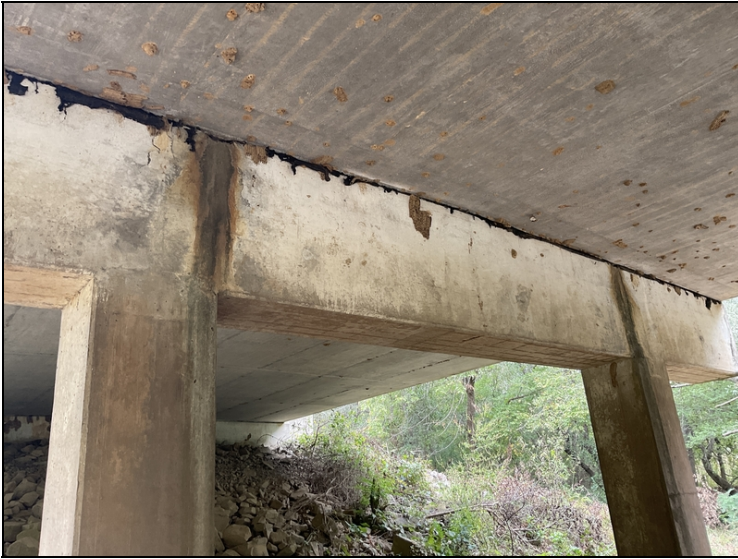
Stains and delaminated areas in Bent # 2 cap from leaking deck joints.
