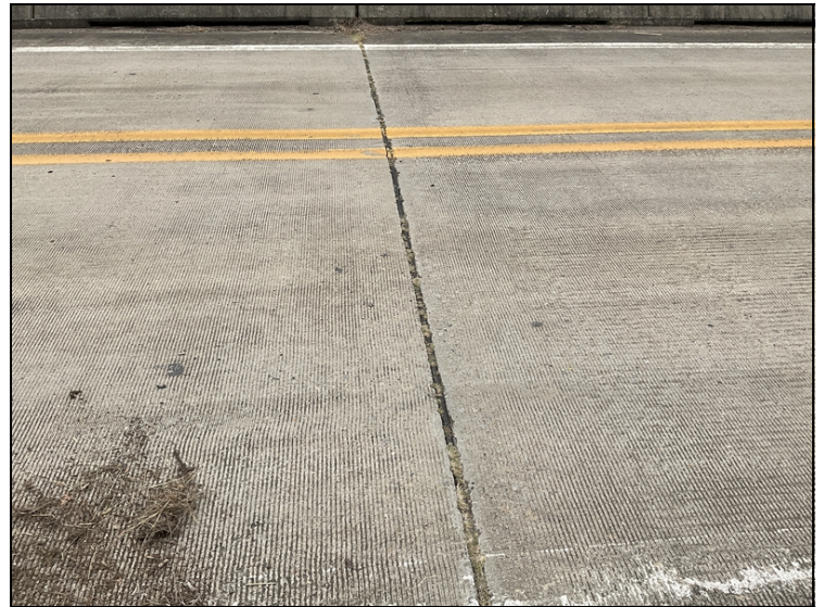
Leaking expansion joint sealant over Bent # 3.
