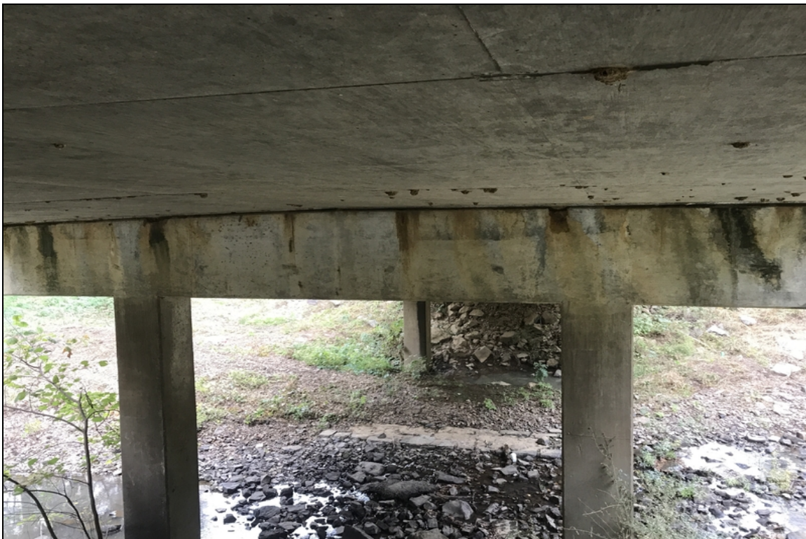
Typical staining from water leakage through the deck joints.
