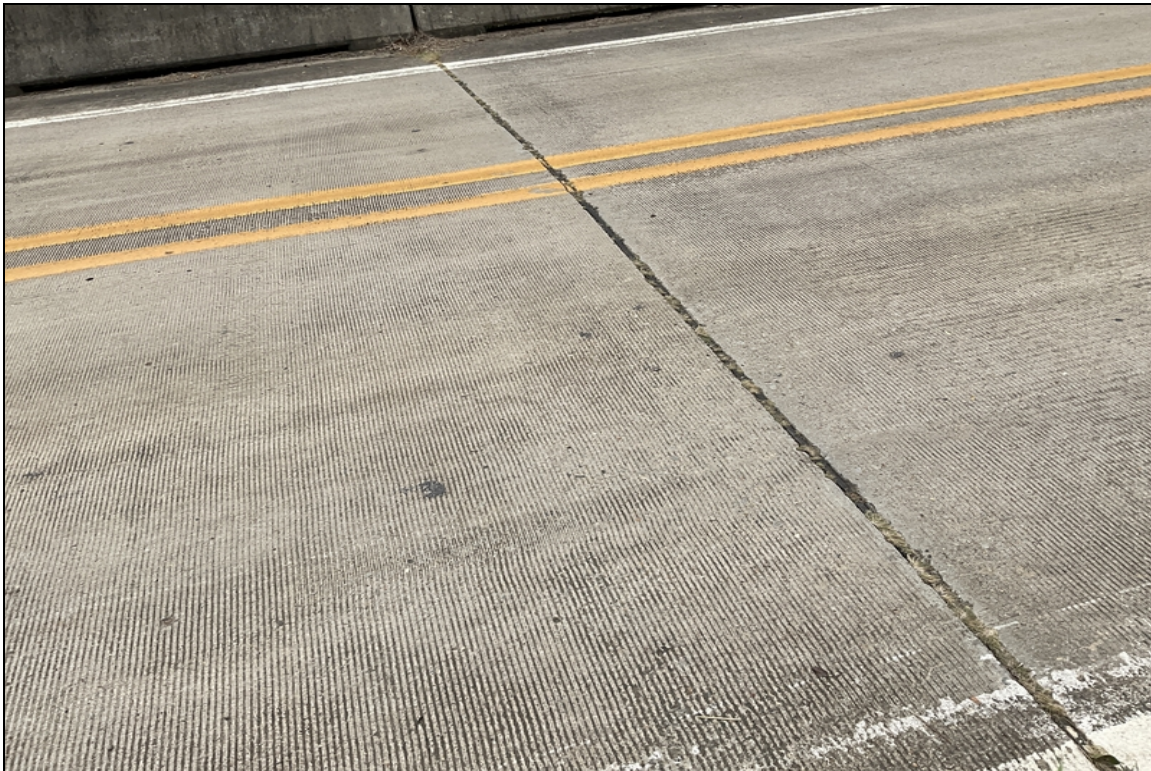
Leaking expansion joint sealant over bent # 3.
