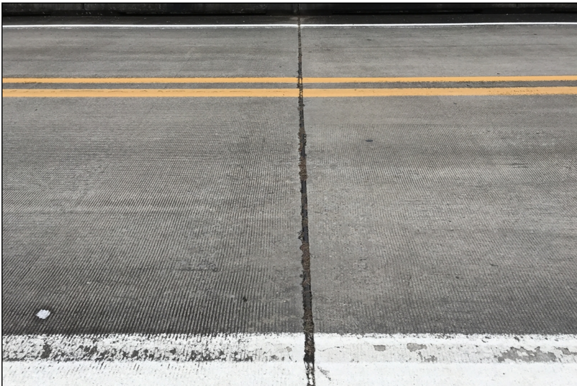
Bent 3 failed joint seal.
