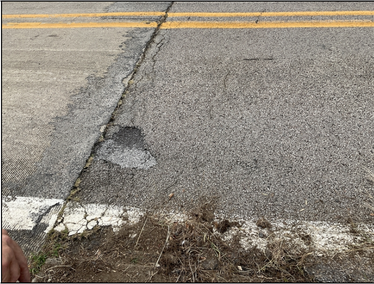
Asphalt settlement at the North approach roadway.
