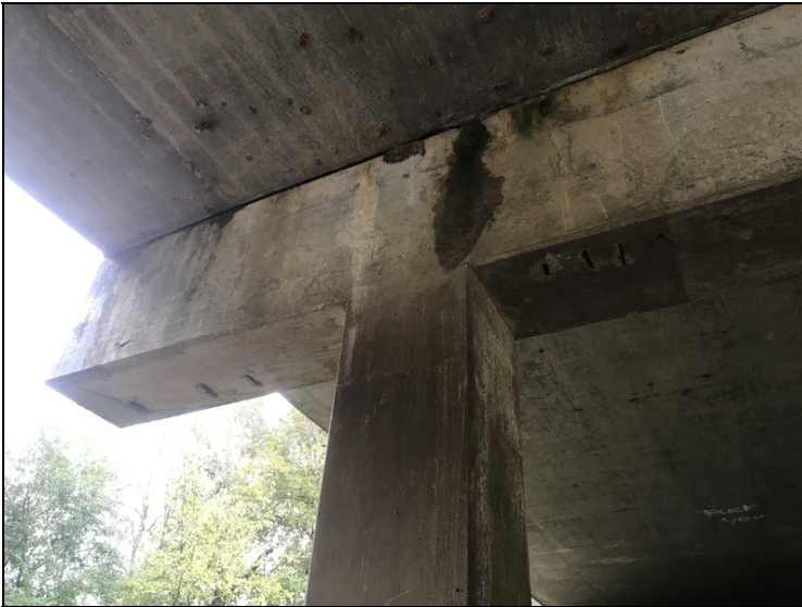
Bent # 3 Lt spalling with exposed reinforcing steel.
