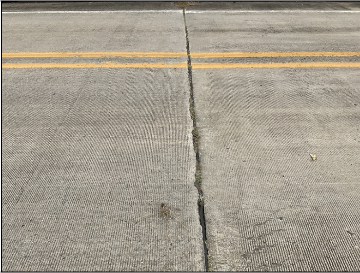
Leaking expansion joint sealant over Bent # 2.
