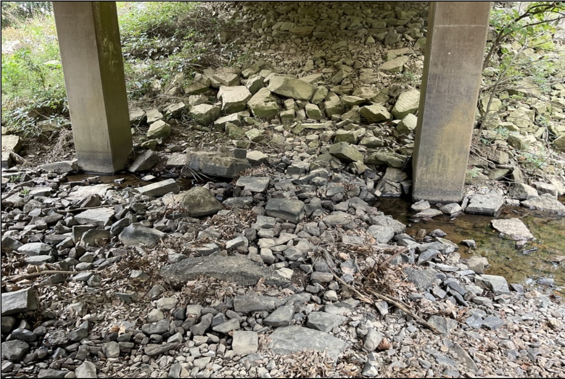
Bent # 3 columns. Light abrasion.
