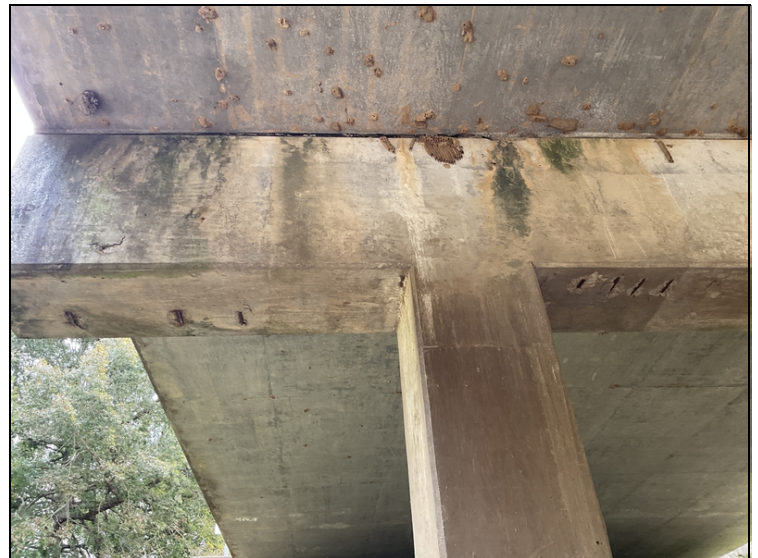
Left end of bent # 3. Spalls with exposed reinforcing steel.
