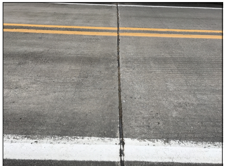
Bent # 2 joint seal deterioration.
