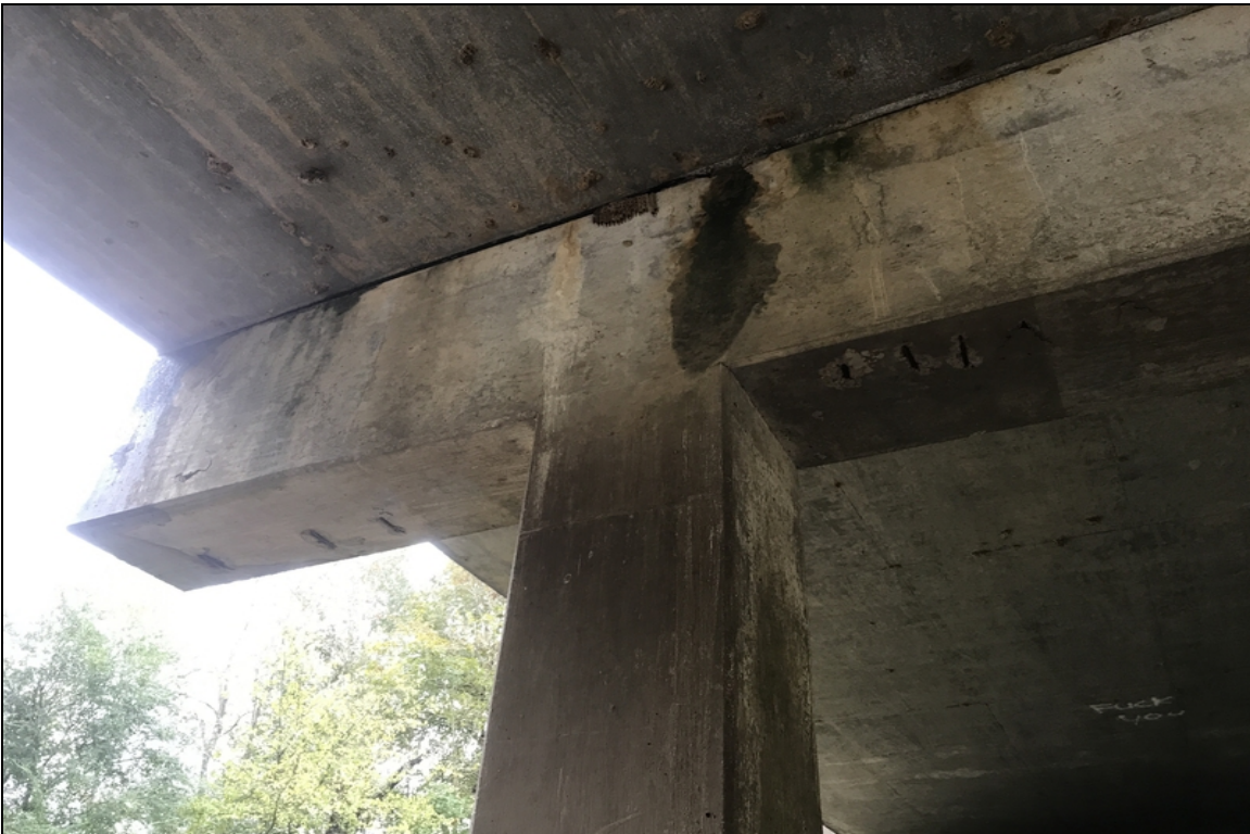
Bent 3 Lt spalling with exposed reinforcing steel.
