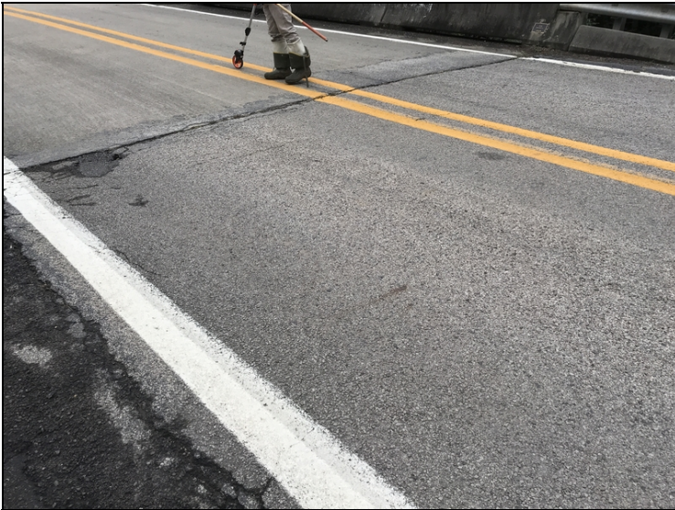
North approach asphalt settlement.
