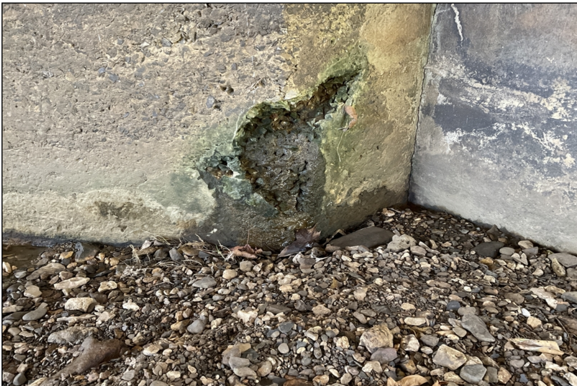
Abutment # 2-Concrete deterioration at base of stem wall near centerline.
