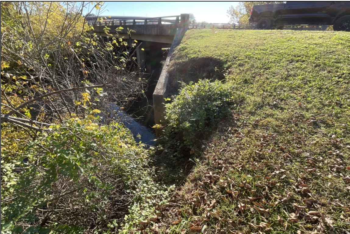
Embankment erosion behind abutment # 2 right wing wall due to lateral stream migration.
