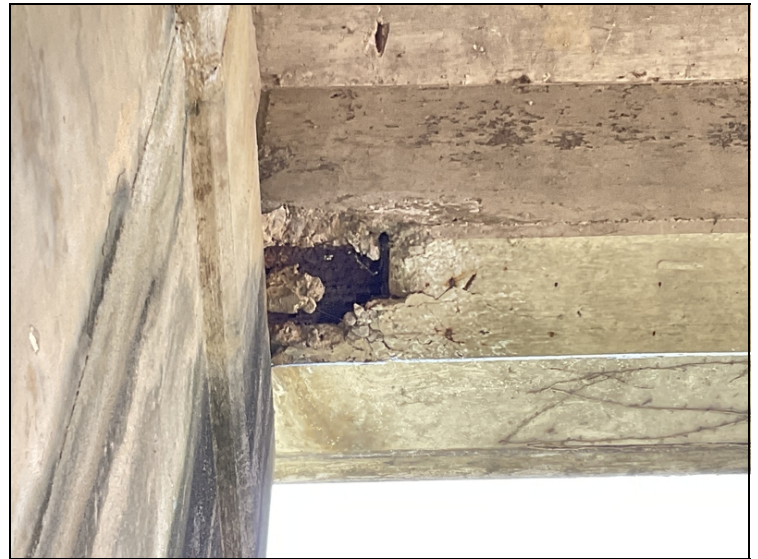
Span 2, girder # 1-Spalling in undersurface that exposes steel loading plate.
