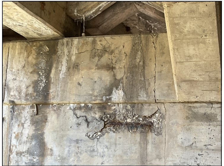
Bent 2, left side-Horizontal cracking in cap with spalling in pier wall.
