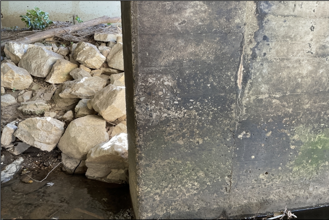
Bent 2, column 1-Shallow spall in ahead face.
