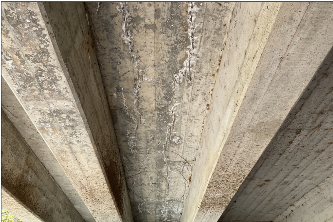
Span 1, bay 2-Efflorescence.
