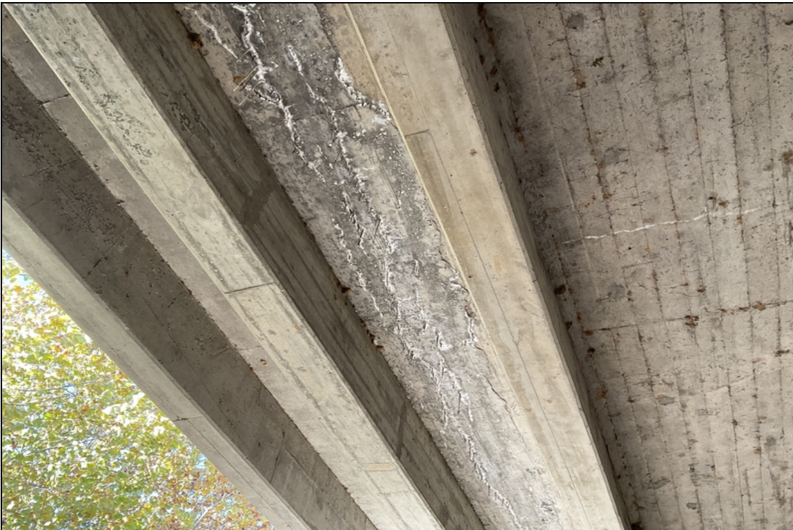
Span 2, bay 2-Cracking with efflorescence.
