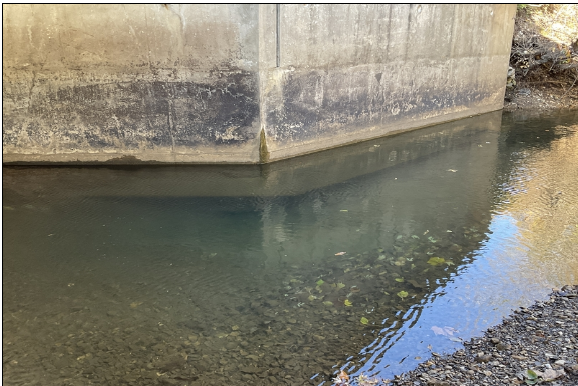
Abutment 2, right side-Footing exposed.
