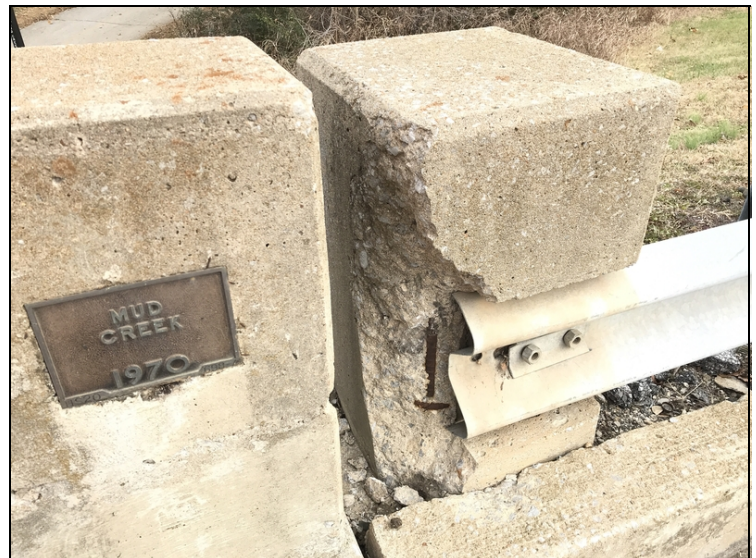
Collision damage to the Southeast end post.
