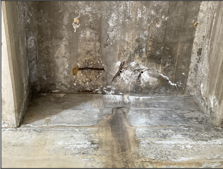
Span # 3, bay # 4 adjacent to abutment # 2- Spalling with exposed reinforcing steel.
