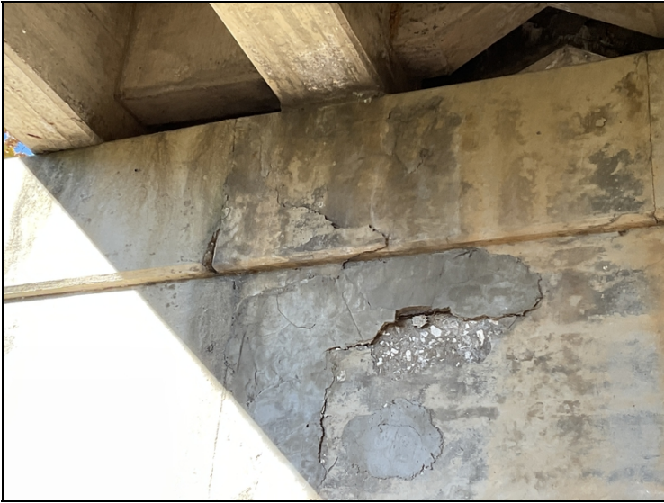
Bent 3, left side-Delaminated area in cap and spalling with failing repairs to pier wall backface.
