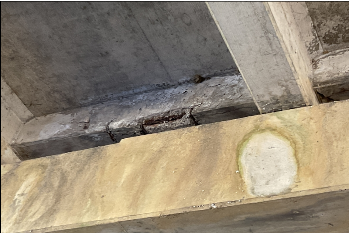
Span 2, bay 8 over bent 2-Spalling with exposed reinforcing steel in expansion dam.
