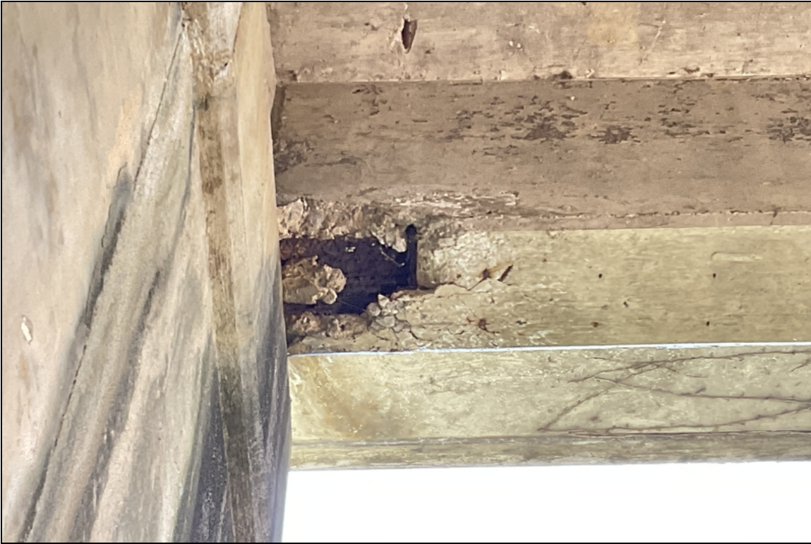
Span 2, girder # 1-Spalling in undersurface that exposes steel loading plate.
