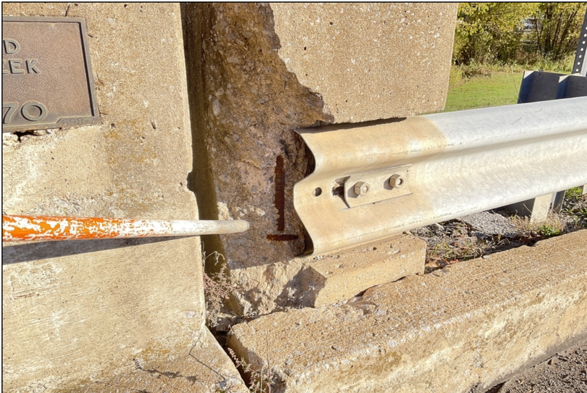
The Southeast approach railing end post on the right side of abutment # 2 has apparent collision damage that has a large spalled area with exposed reinforcing steel.
