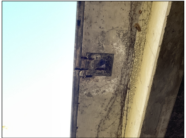
Span # 2, right side-Spalling with exposed reinforcing steel adjacent to deck drain.
