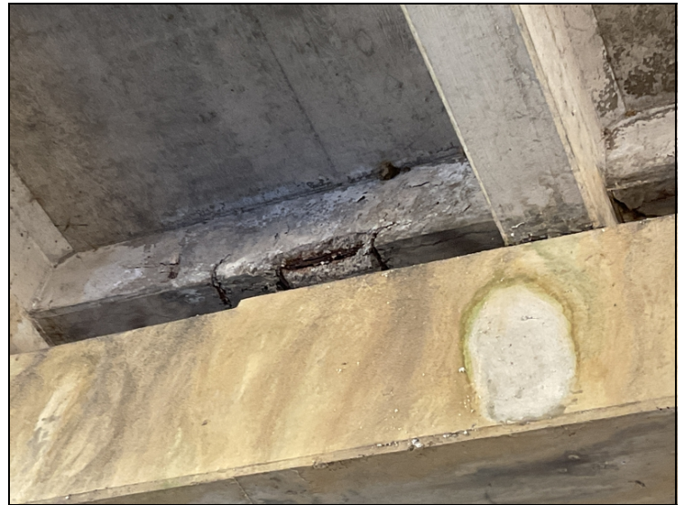
Span # 2, bay # 8 over bent # 2-Spalling with exposed reinforcing steel in expansion dam.
