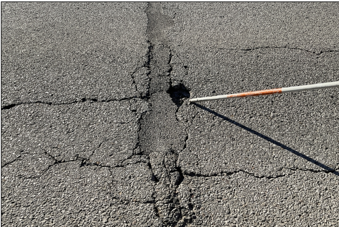
Pothole forming in asphalt driving surface in left lane at abutment # 1.
