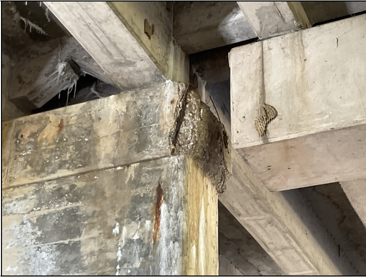
Bent # 3 cap-Spalling with exposed reinforcing steel at centerline.
