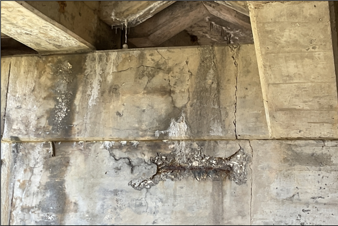
Bent 2, left side-Horizontal cracking in cap with spalling in pier wall.
