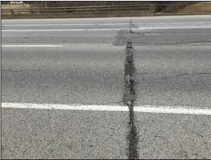
Expansion joint over Bent # 4.
