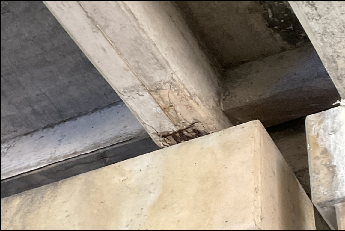
Span # 2, Beam # 7 has an 8" spall with exposed reinforcing steel adjacent to Bent # 2. There is a 10" Delaminated area adjacent to the spall.
