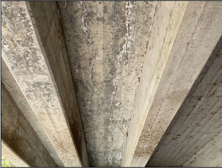
Span # 1, bay # 2-Efflorescence.
