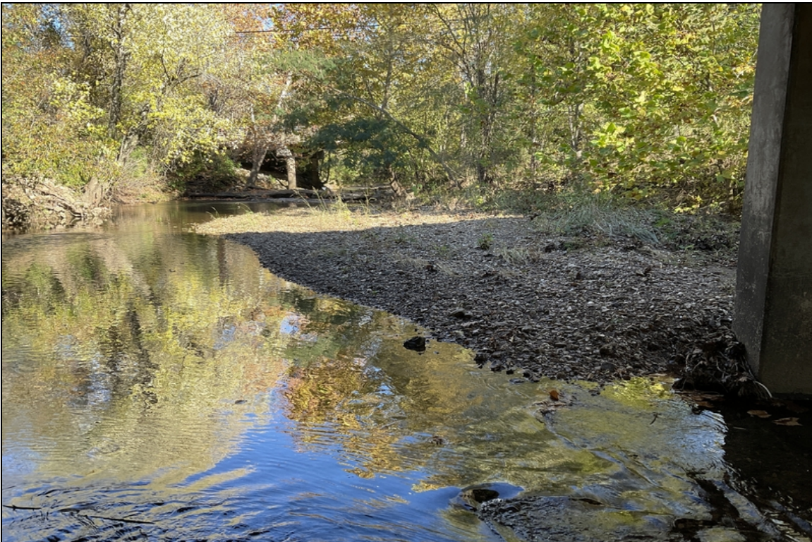
Streambed material accumulation in upstream channel is causing lateral stream migration and directing channel flow into abutment # 2 causing scour along the abutment exposing the top and approximately 16" of the vertical face of footing at the inlet end.
