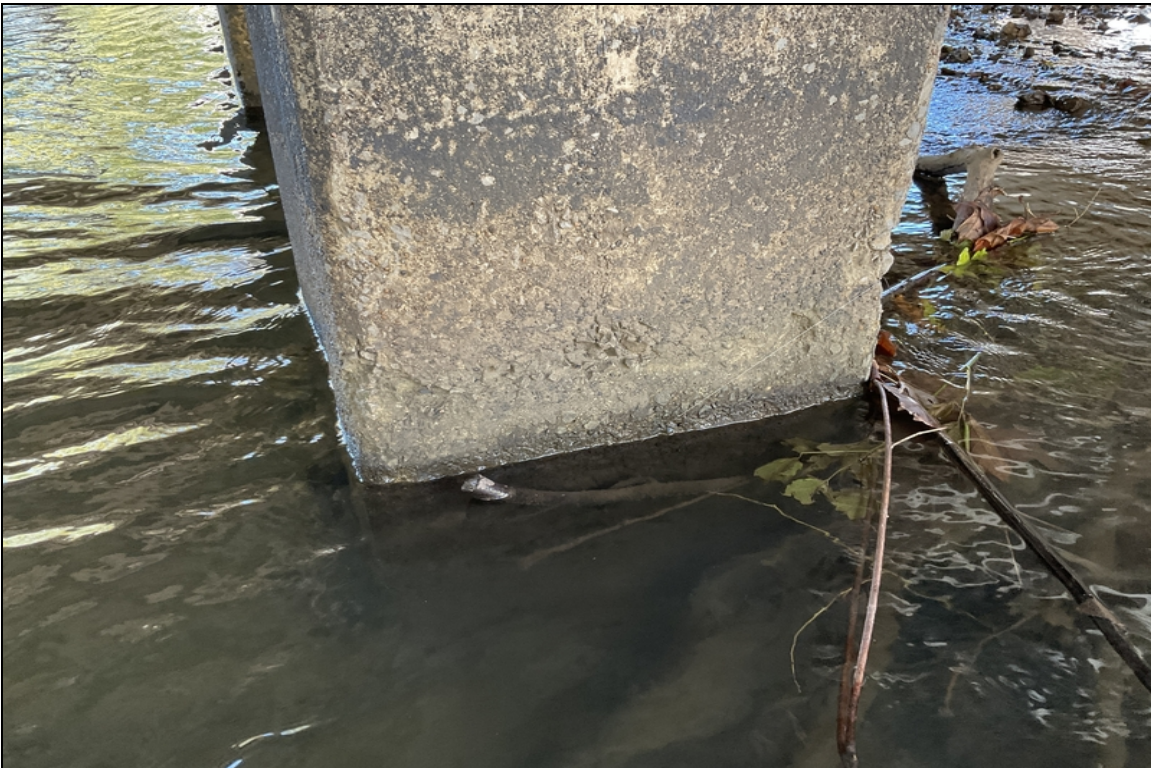
Bent 3, column 3-Abrasion / concrete deterioration.
