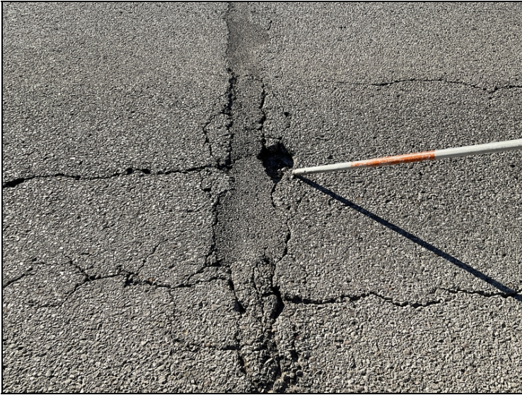
Pothole forming in asphalt driving surface in left lane at abutment # 1.
