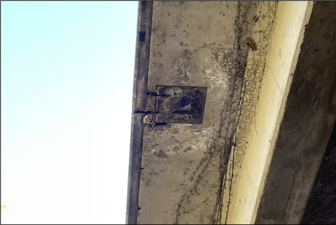
Span 2, right side-Spalling with exposed reinforcing steel adjacent to deck drain.
