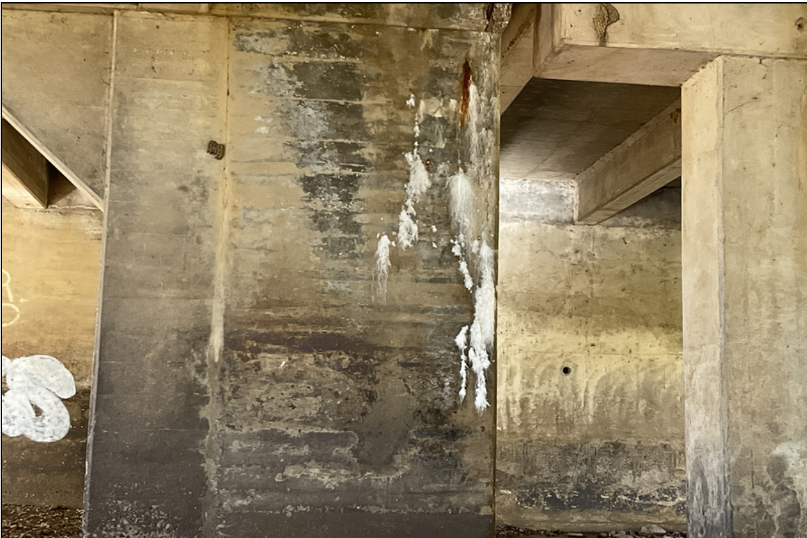
Bent 3 pier wall at centerline-Cracking with efflorescence.
