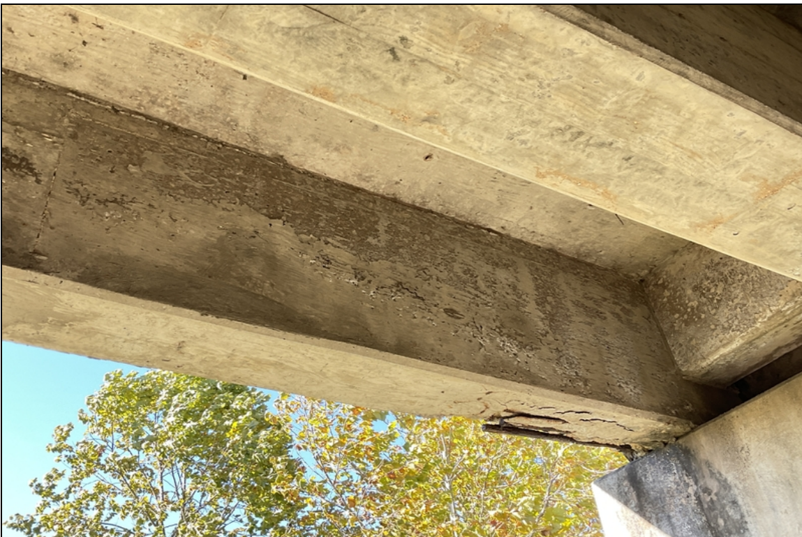
Span # 1, girder # 1 at bent # 2 has light scaling.
