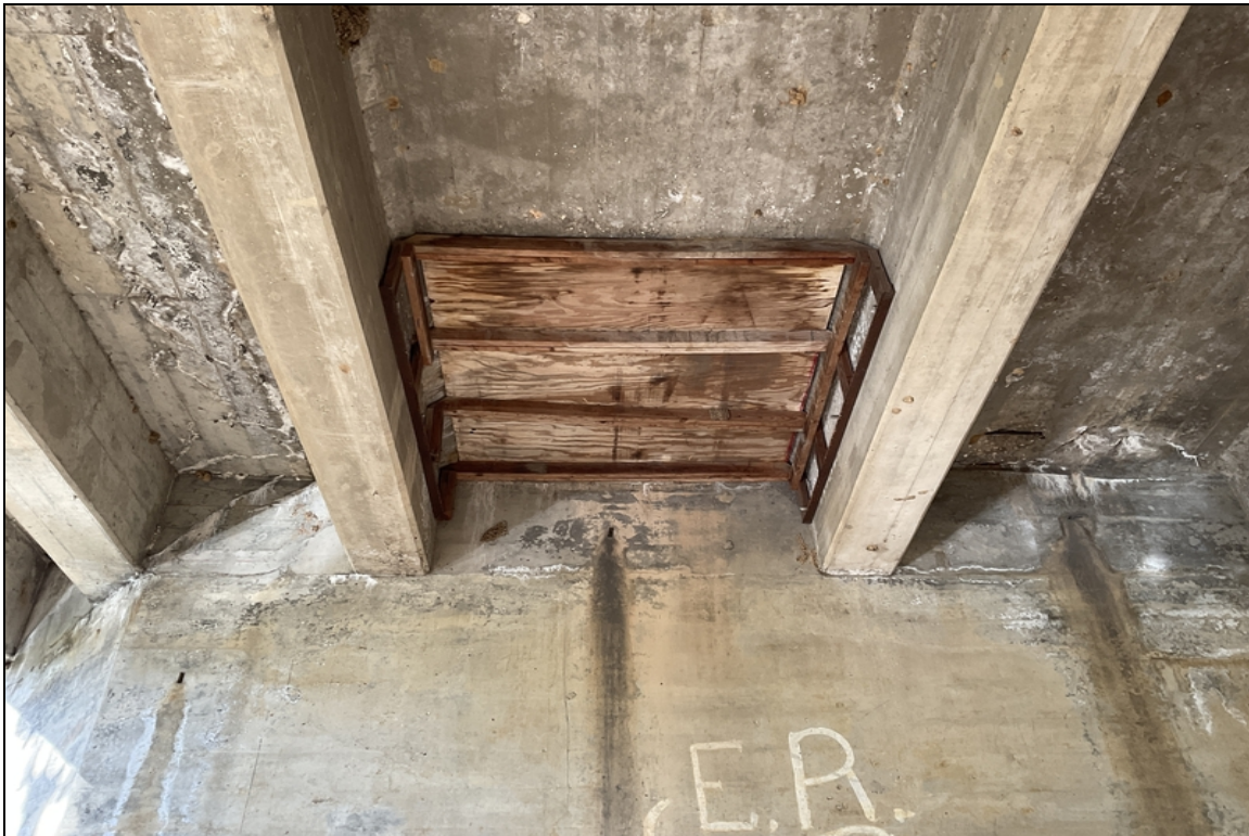
Span 3, bay 3 adjacent to abutment 2-Form work left in place.
