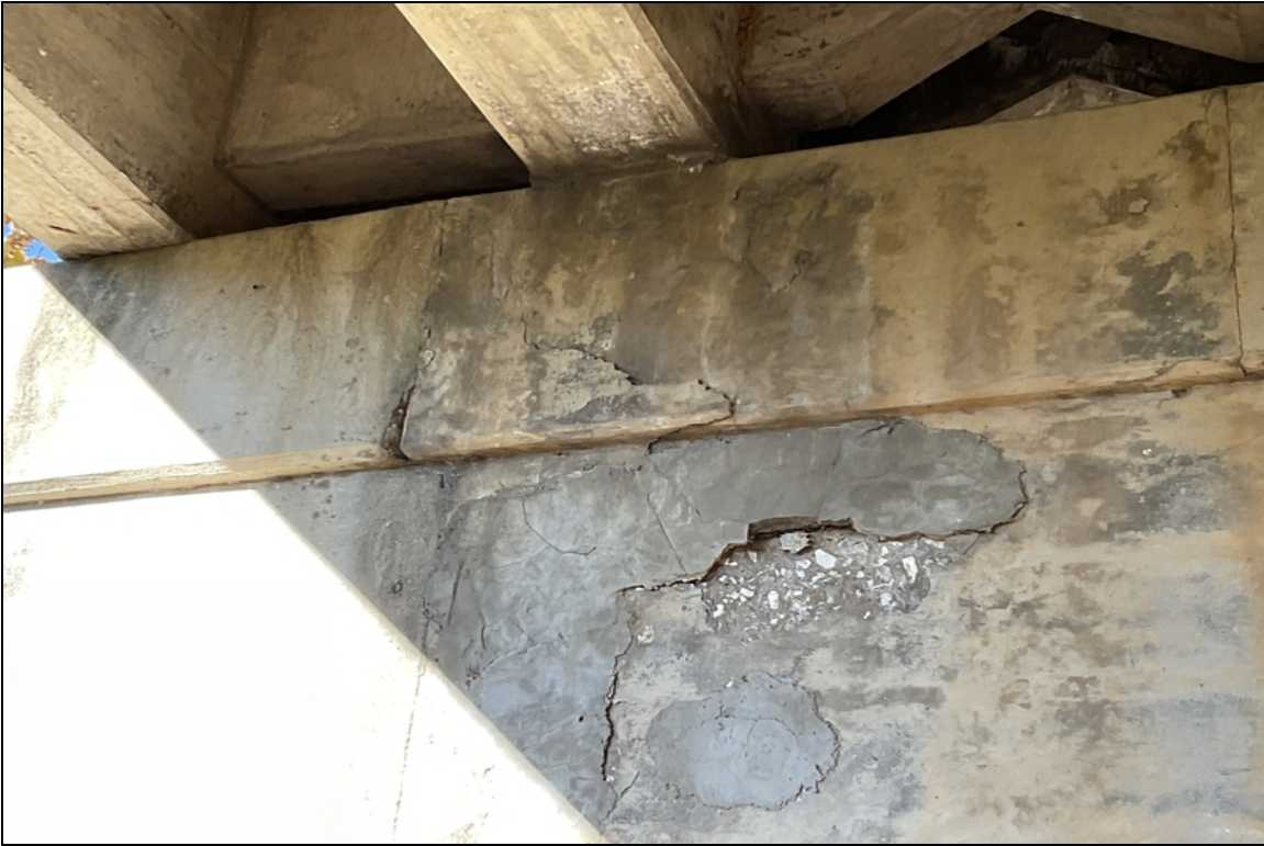
Bent 3, left side-Delaminated area in cap and spalling with failing repairs to pier wall backface.
