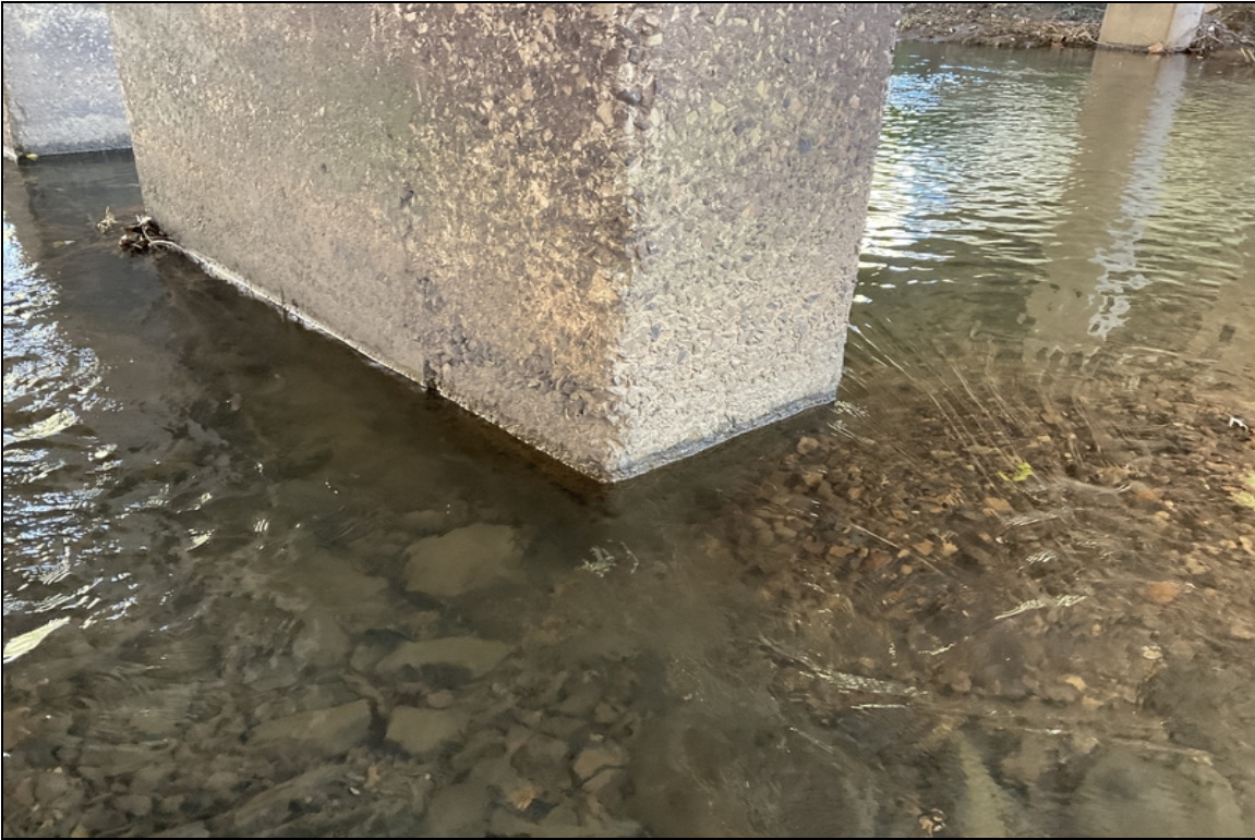
Bent 3, column 2-Abrasion.
