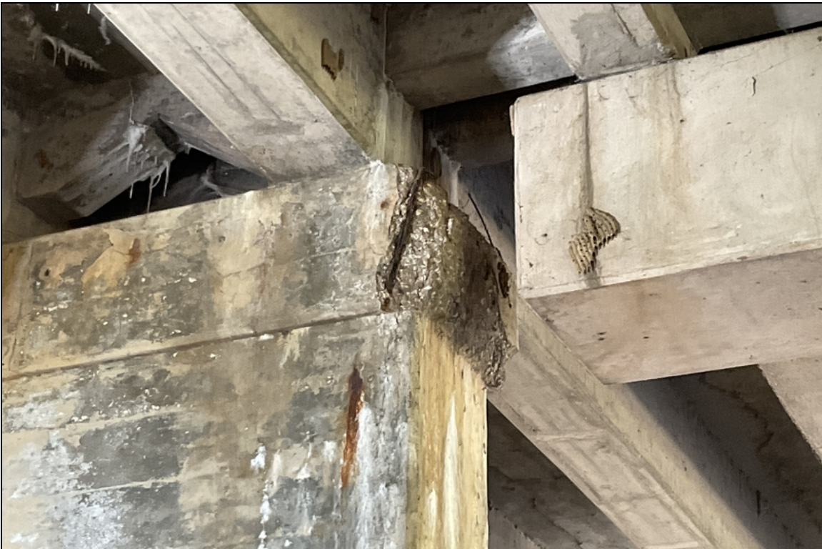
Bent # 3 cap-Spalling with exposed reinforcing steel at centerline.
