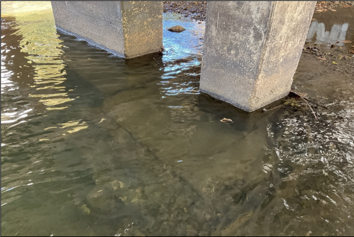
The footings for the portion of bent # 3 pier wall at centerline and column # 3 are exposed with approximately 12" of the vertical face of footings exposed at this inspection.
