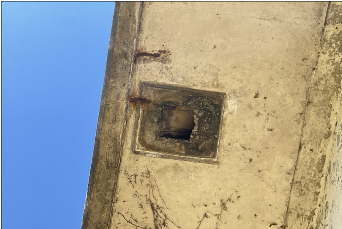
Span 1, left side-Spalling in deck overhang adjacent deck drain.
