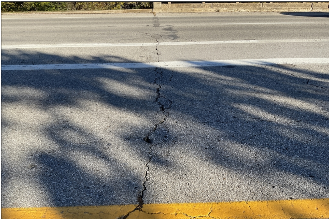
Asphalt cracking over abutment 2.
