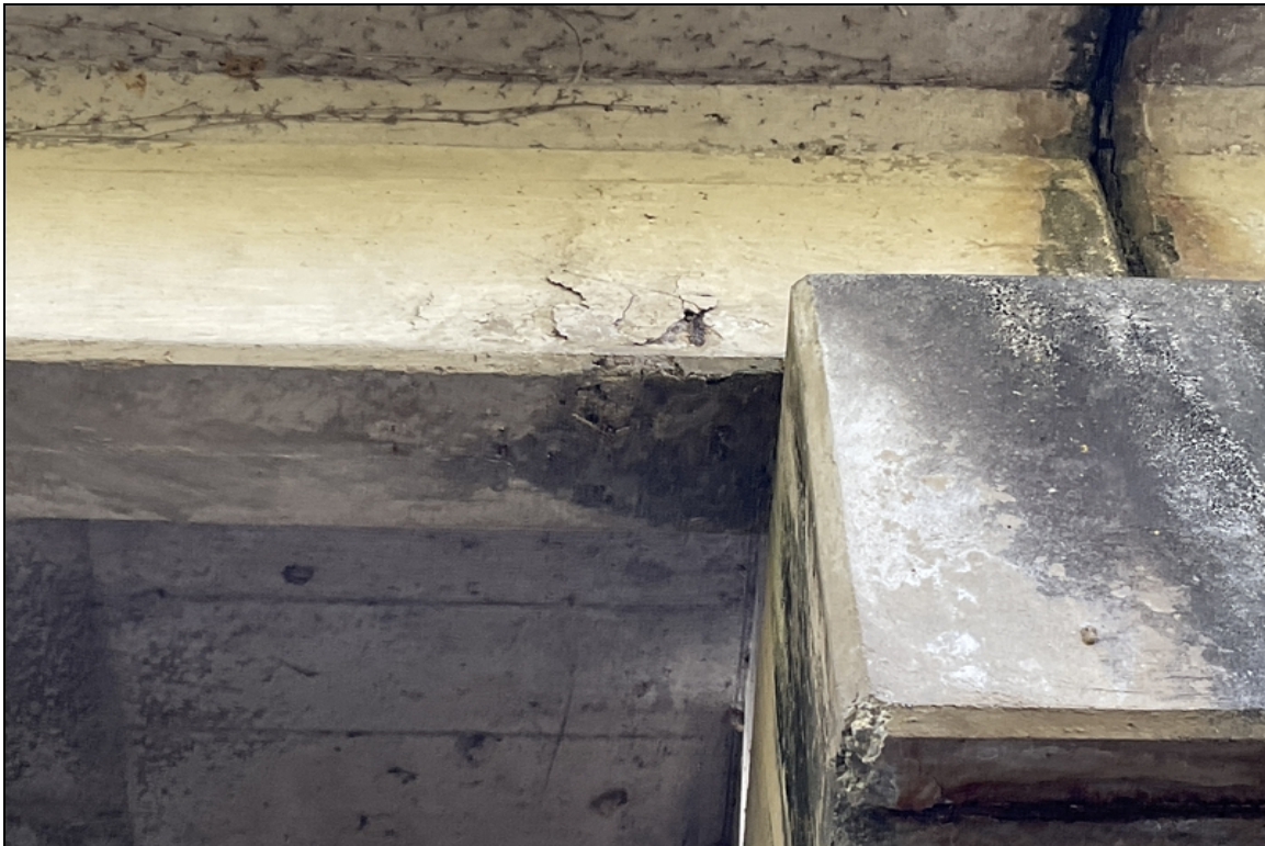
Span 2, girder 10-Spall / Delaminated areas
