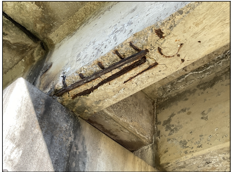
Span # 1, girder # 1 at bent # 2 has an area of spalling in the undersurface of girder that exposes 3 of the primary longitudinal reinforcing bars. The exposed bars appear to be short pieces of reinforcing steel that terminate approximately 30" from the bent. The interior of girder at bent # 2 has light scaling.
