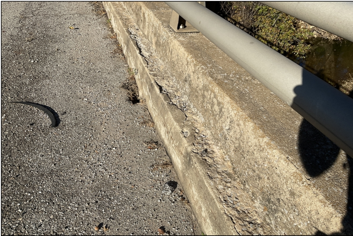
Span 3, left railing-Concrete deterioration.
