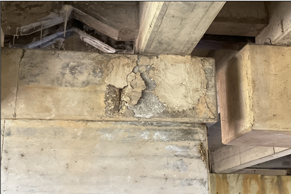
Bent # 2 cap has a 12" x 6" spall with exposed reinforcing steel in the backface under girder # 6 where a previous repair has failed.
