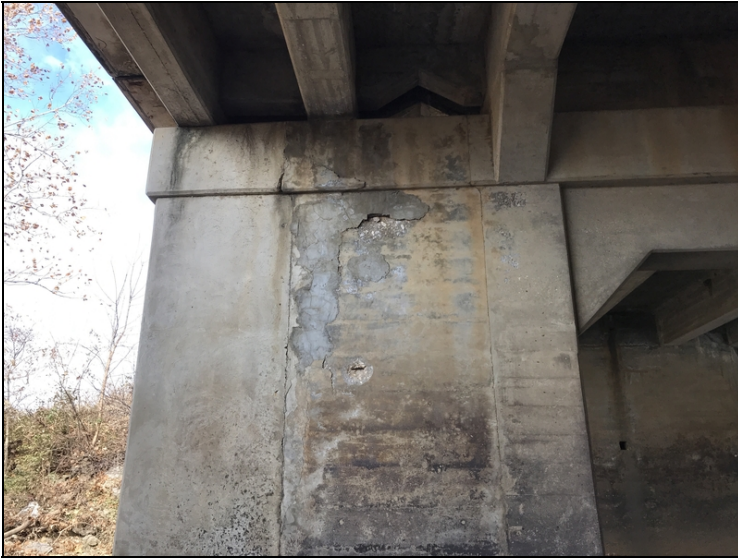
Left end of Bent # 3. Delaminated repairs.
