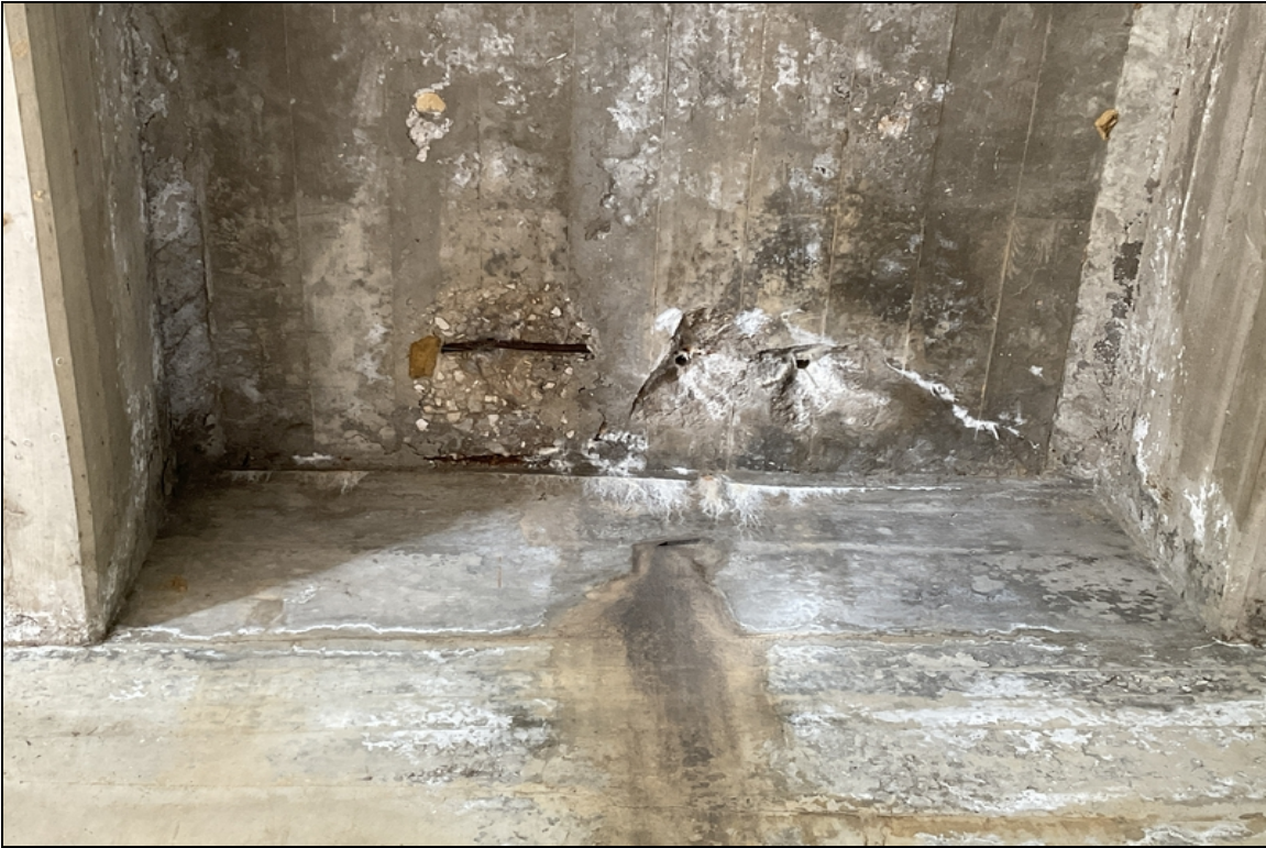
Span # 3, bay # 4 adjacent to abutment # 2-Spalling with exposed reinforcing steel.
