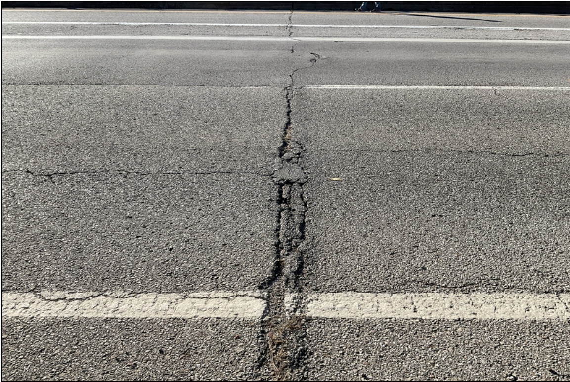
Asphalt cracking over bent 2.
