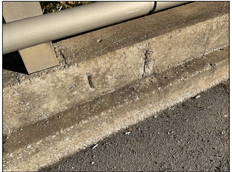
Span # 2, left railing-Shallow spalls with exposed reinforcing steel.
