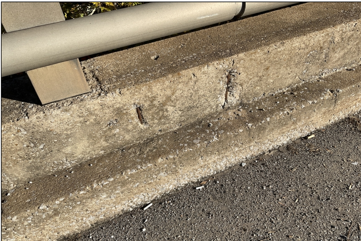
Span 2, left railing-Shallow spalls with exposed reinforcing steel.
