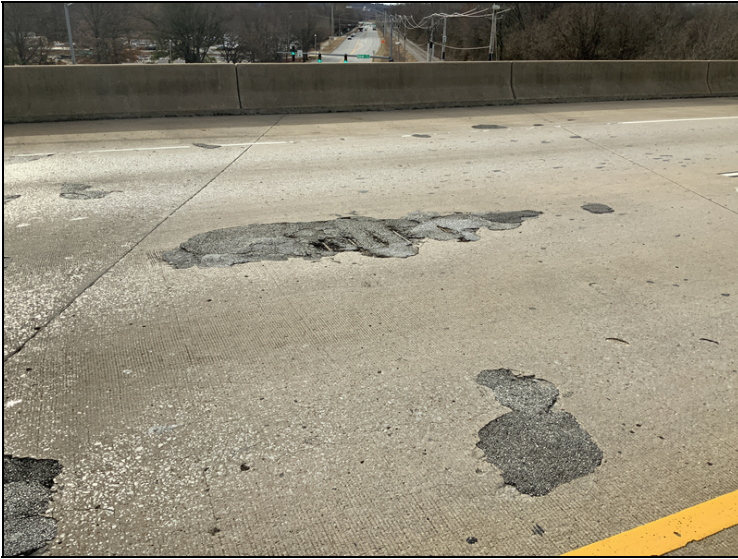
Span 3 spalling with exposed reinforcing steel.
