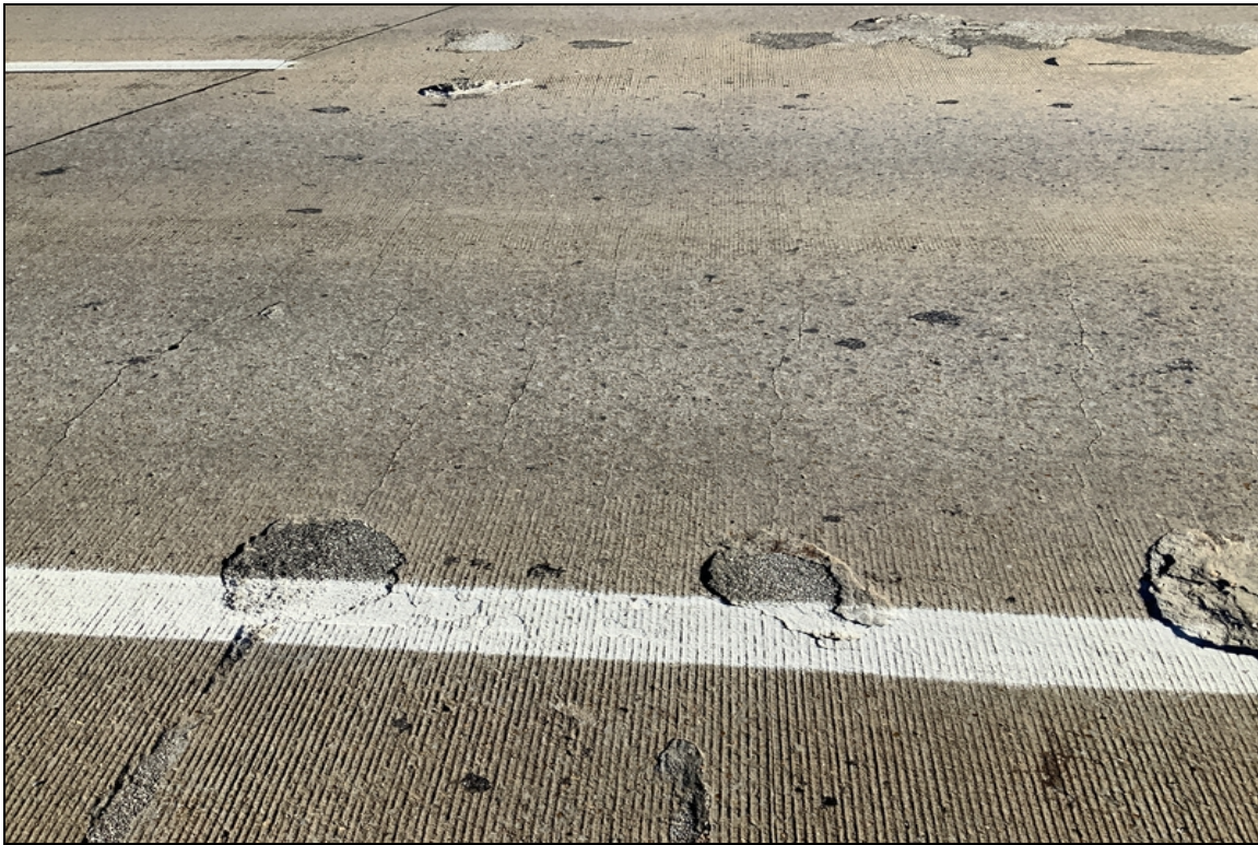
Span 4, transverse cracks and spalls/patches.
