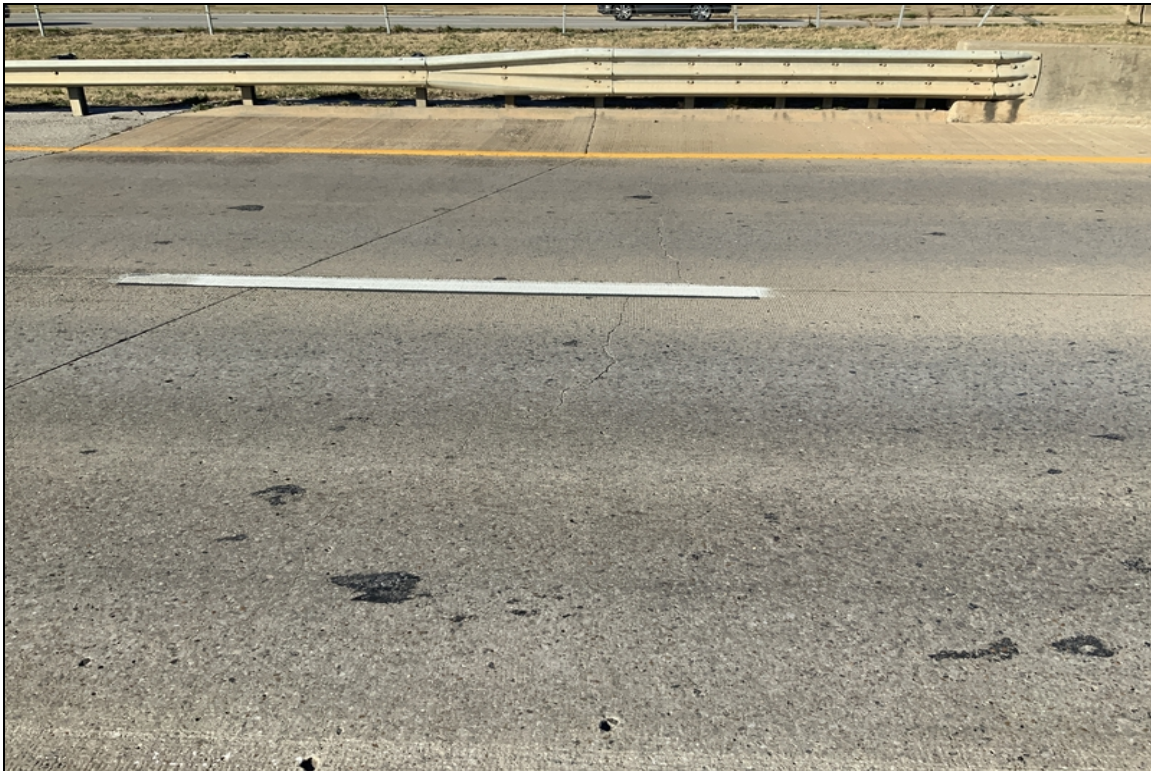
West approach slab, large transverse cracks.
