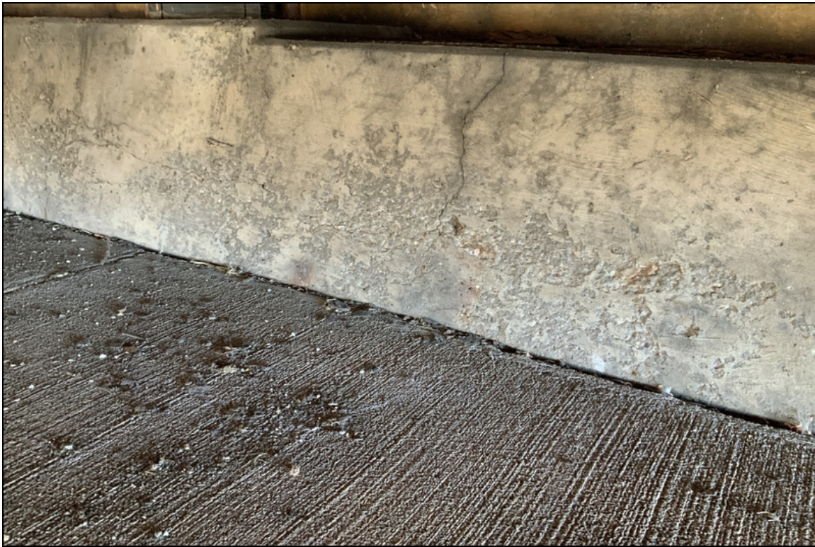
Abrasion and cracks in bent 5.
