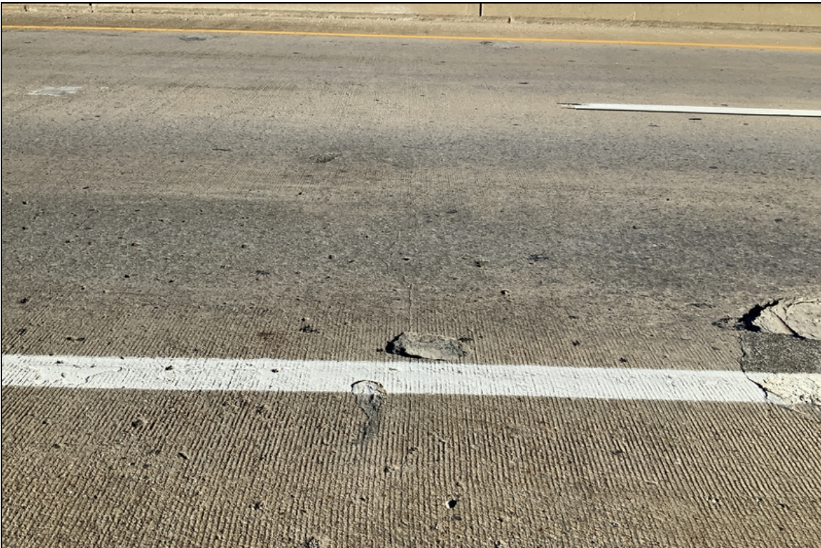
Span 3, spall and abrasion.
