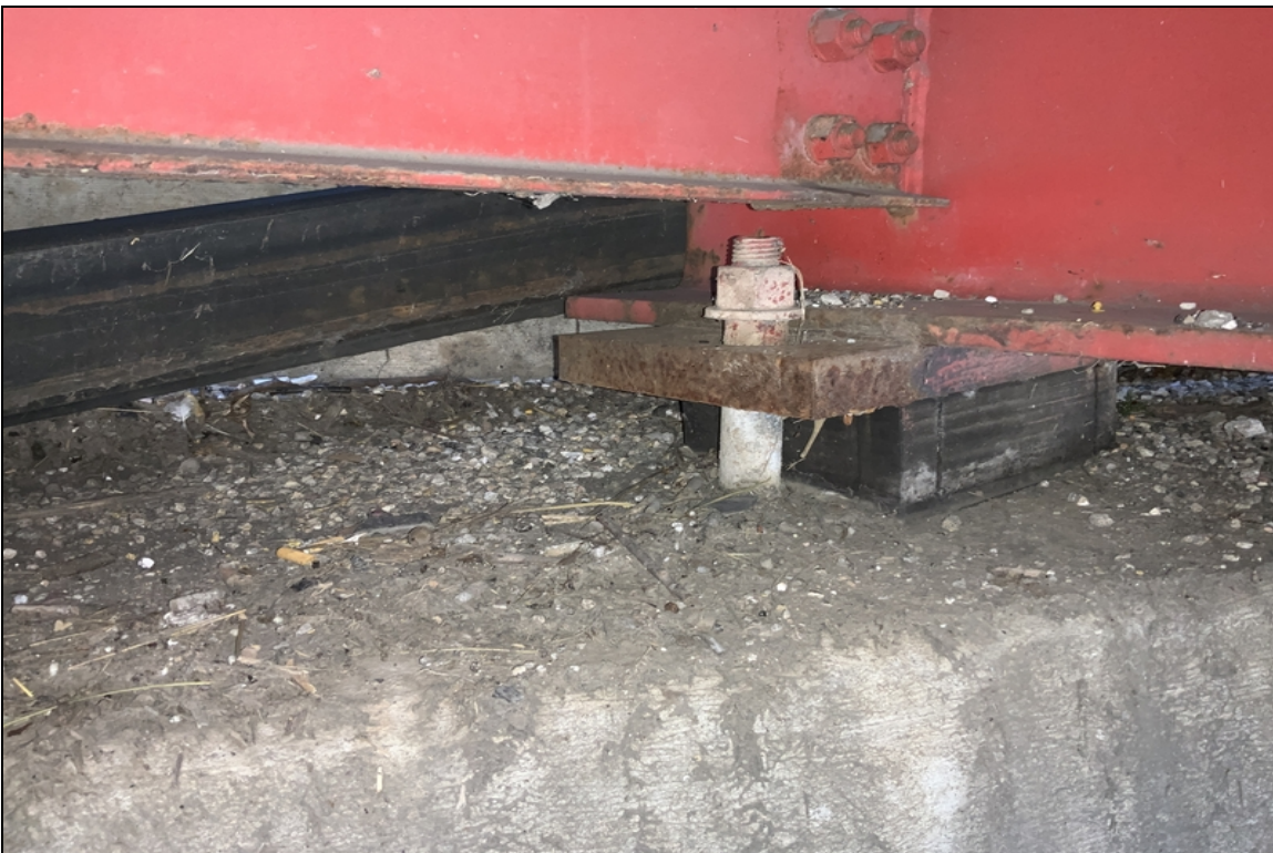
Bent 5 bearing 2, flaking rust,
