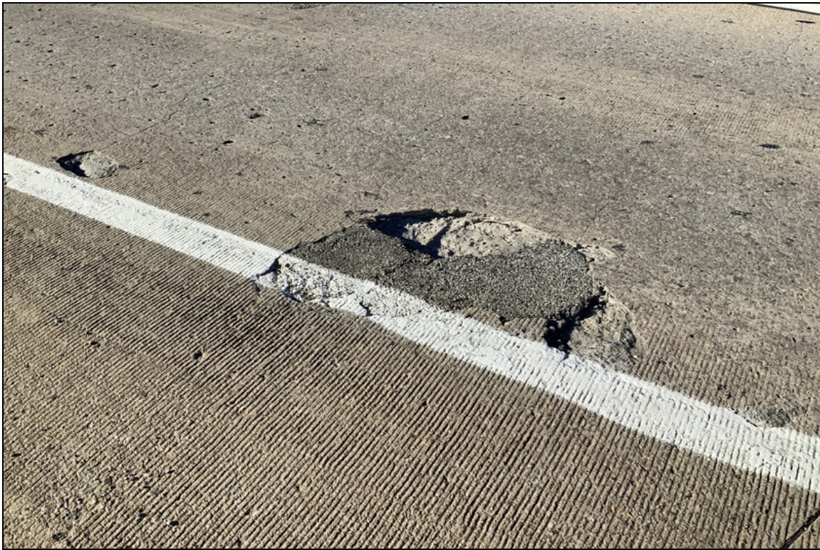
Span 3, spall with exposed rebar
