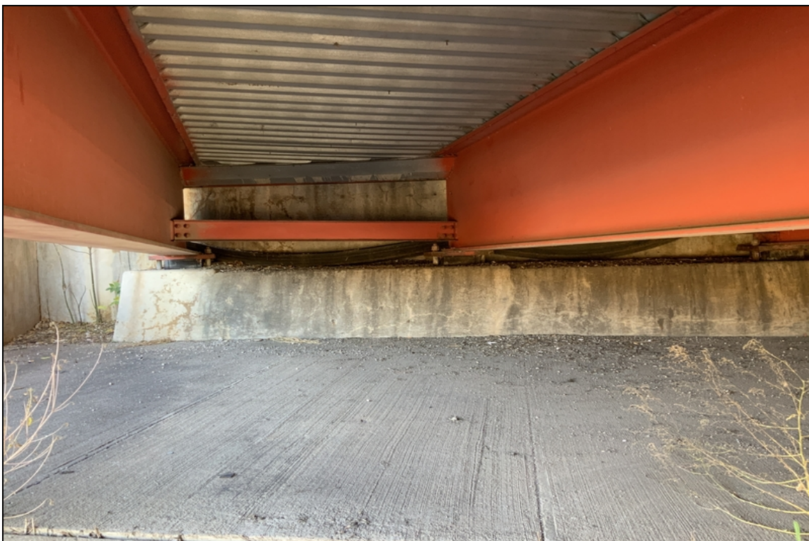
Bent 5, joint laying on cap.
