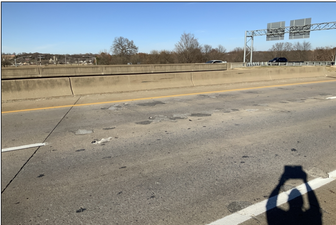
Span 4, large areas of failing patches and spall.
