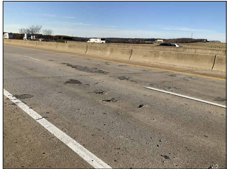
Span 3, spalls and failing patches.
