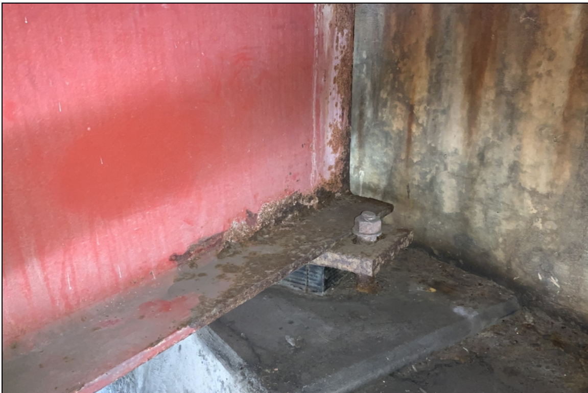
Bent 5 girder 4, corrosion
