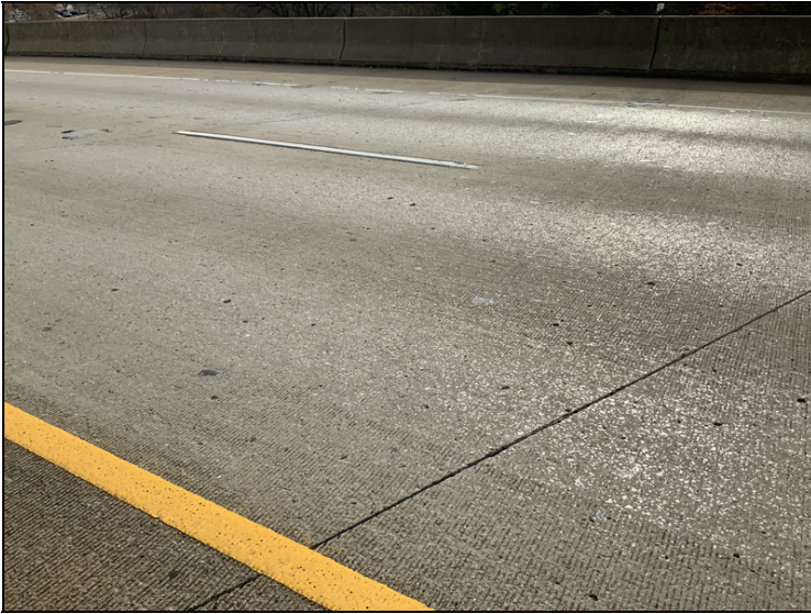
Typical seal-able deck cracking throughout the structure.
