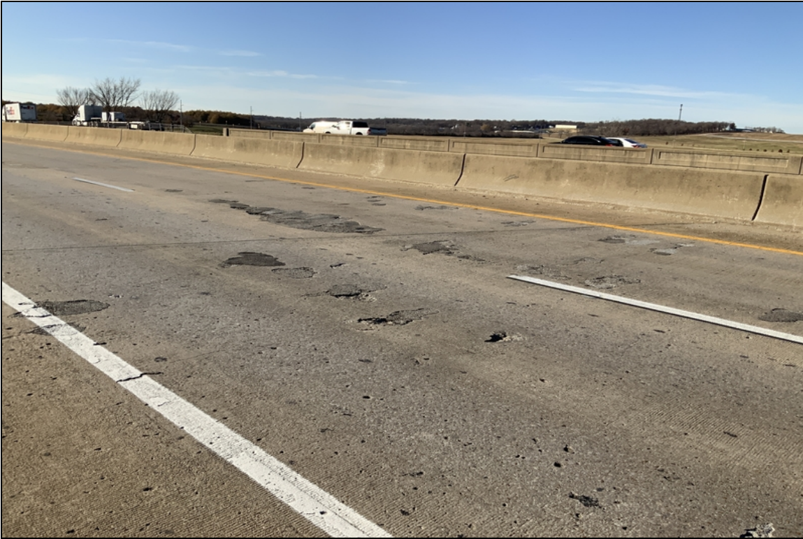
Span 3, spalls and failing patches.
