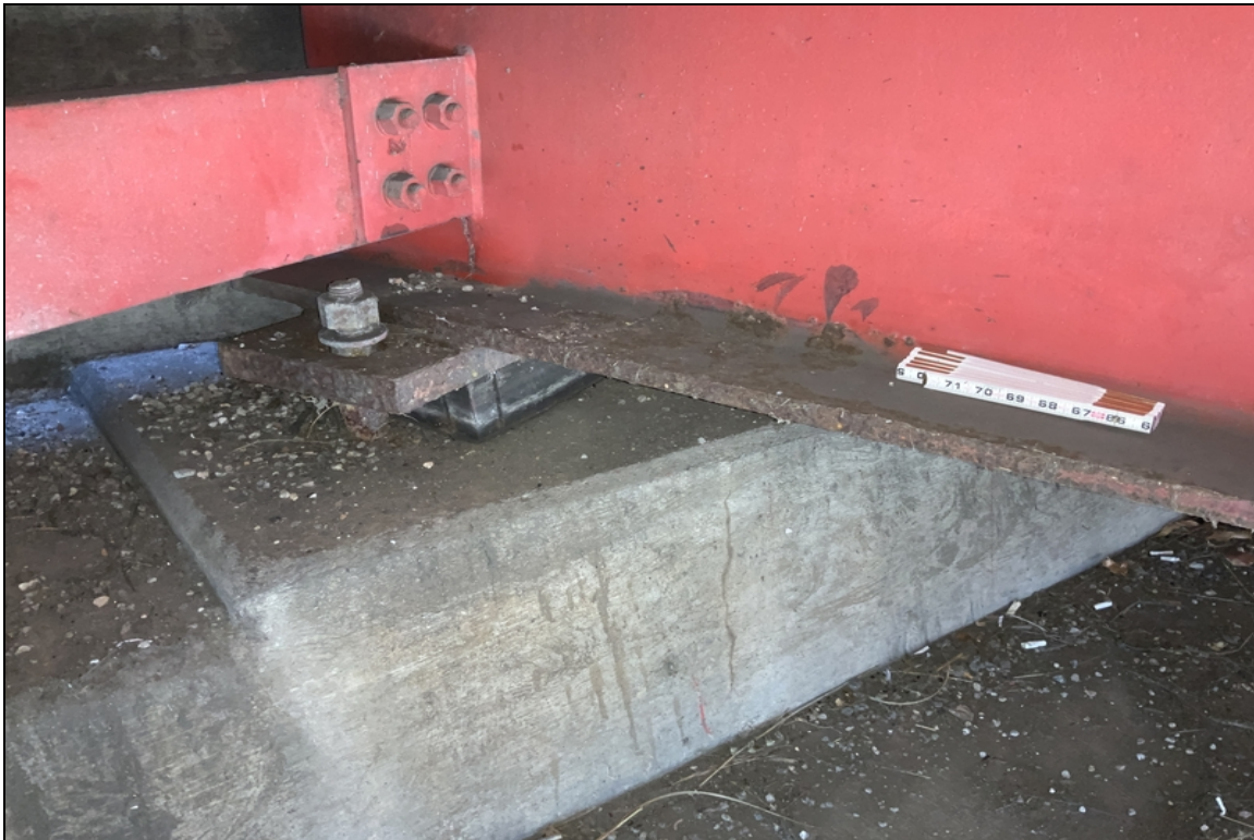
Bent 1 girder 4, corrosion bottom flange.
