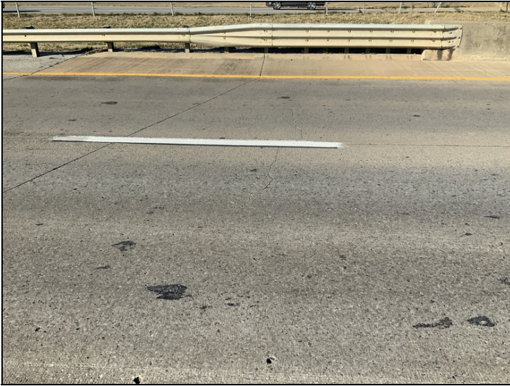
West approach slab, large transverse cracks.
