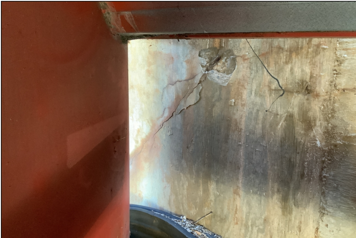
Bent 5 behind girder 1, rebar and crack in back wall.
