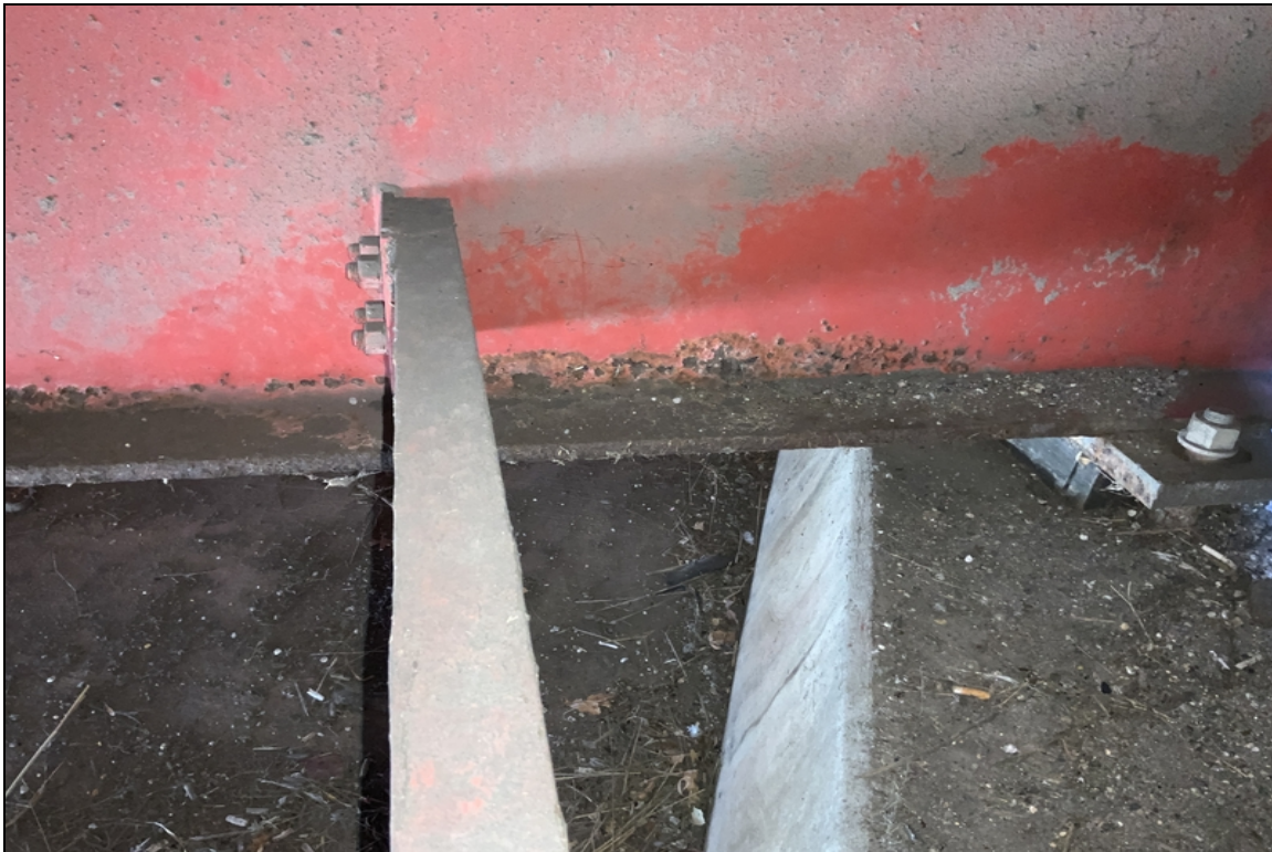
Bent 1 girder 3, corrosion on the bottom flange.
