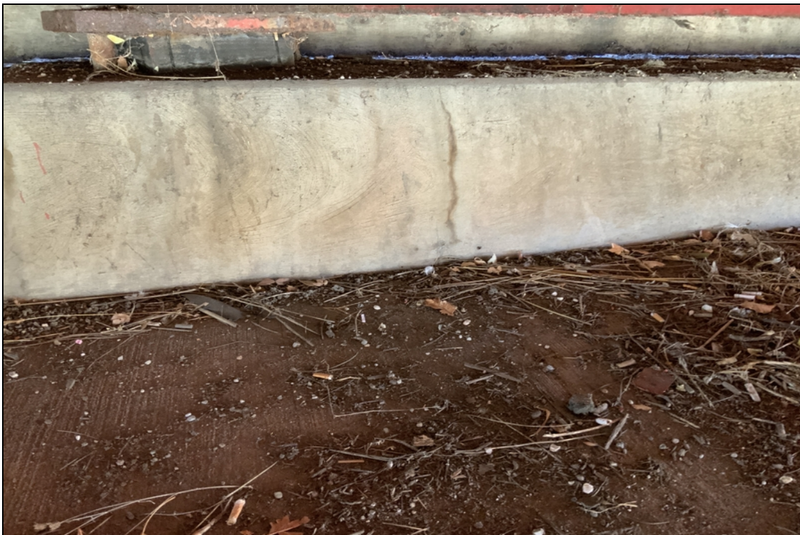
Bent 1, crack in the beam seat.
