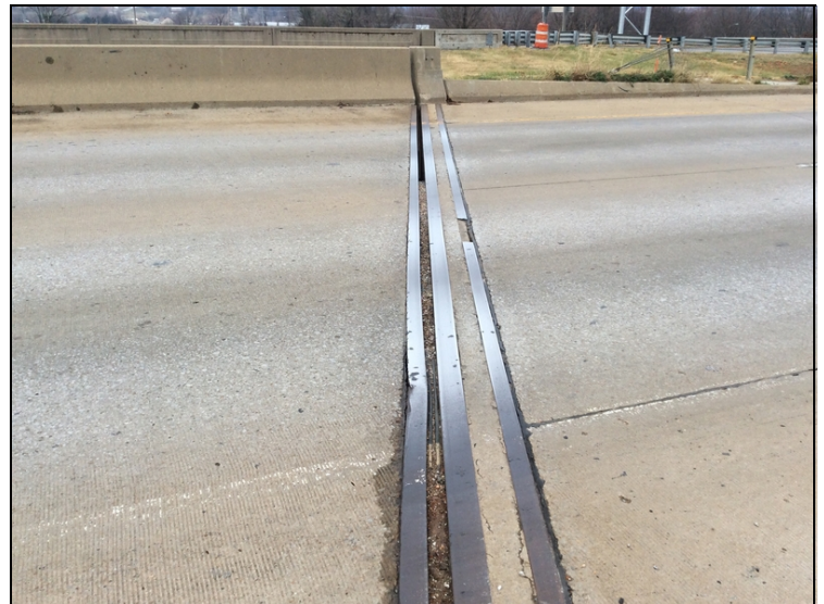
Bent # 5 joint seal.
