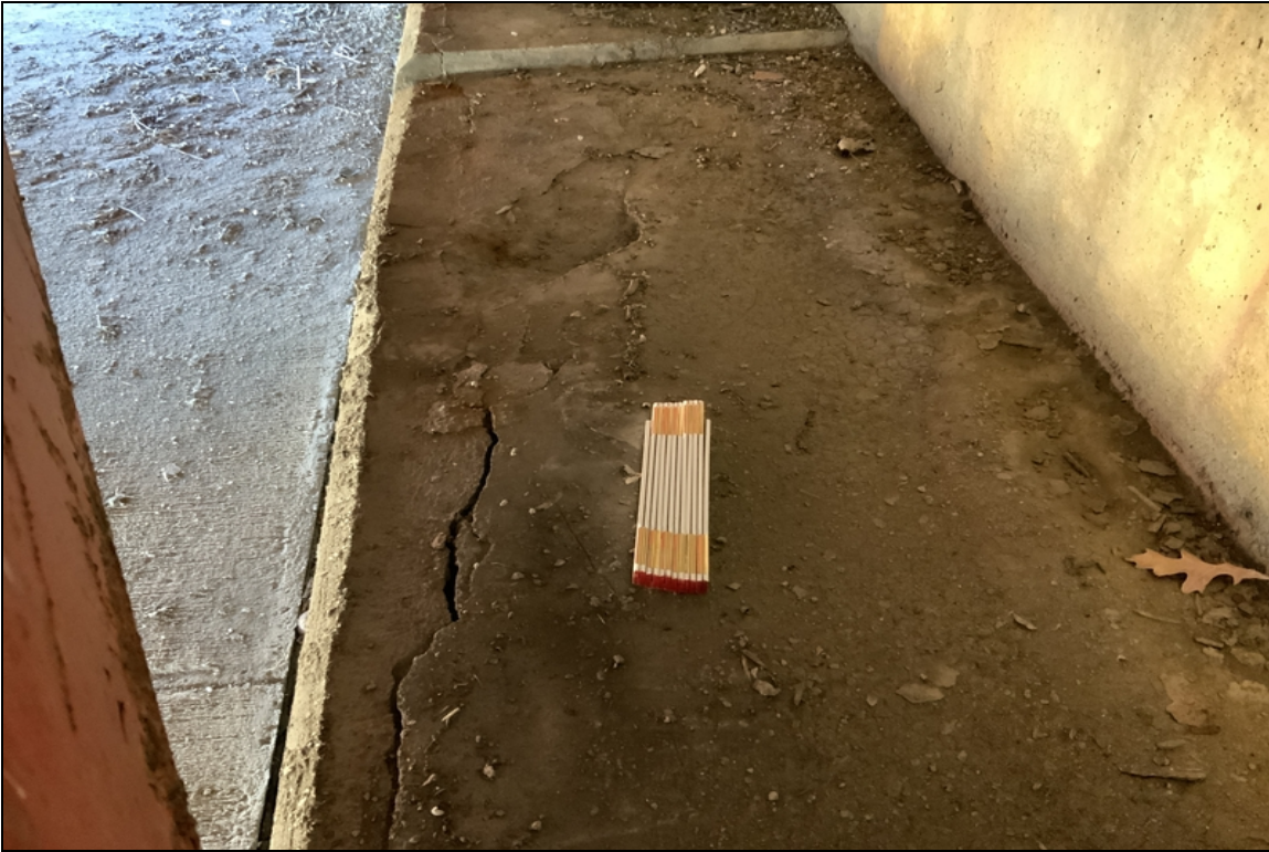
Large crack and delaminating concrete in the beam seat between girders 3 and 4.
