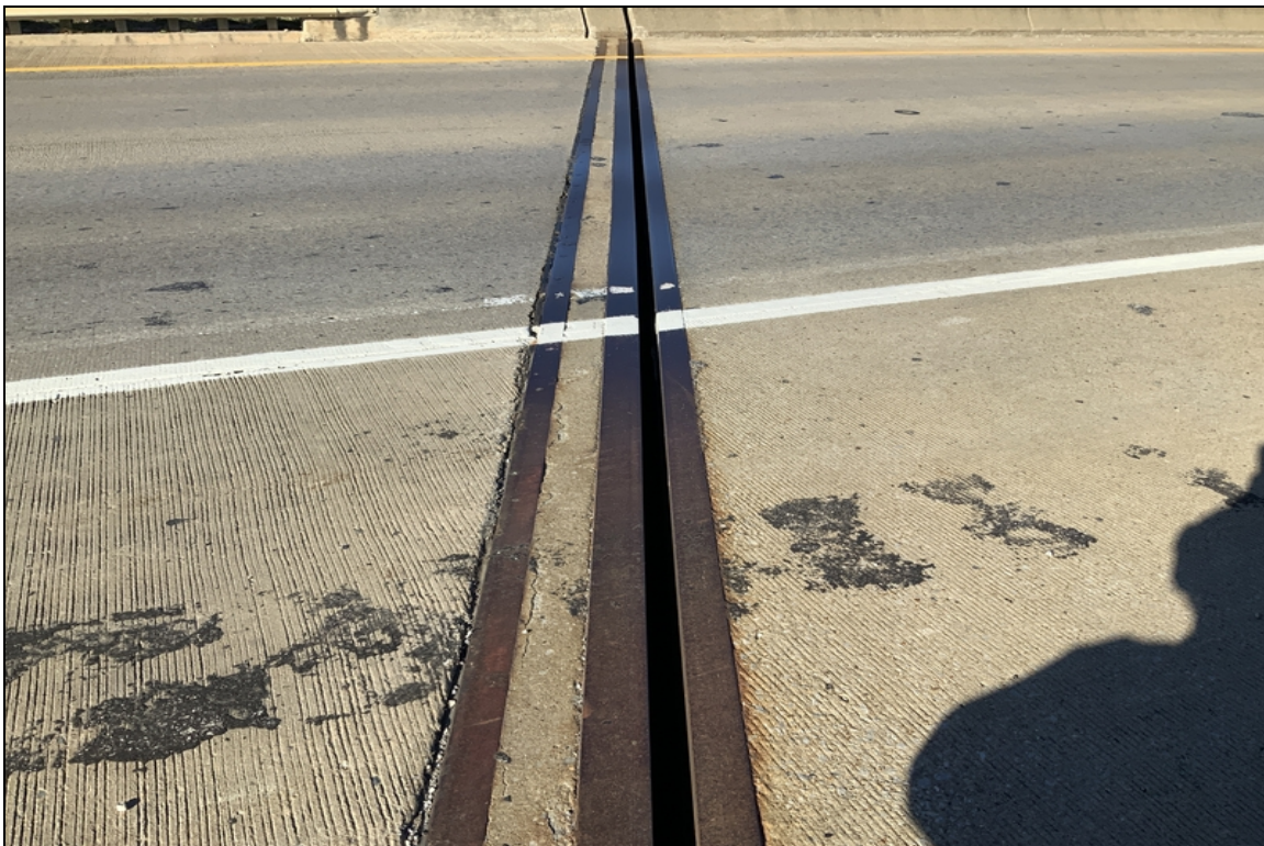
Bent 1 joint has fallen out.
