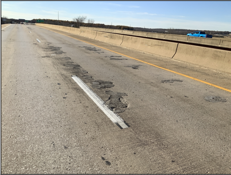
Span 4, several spalls and failing patches.
