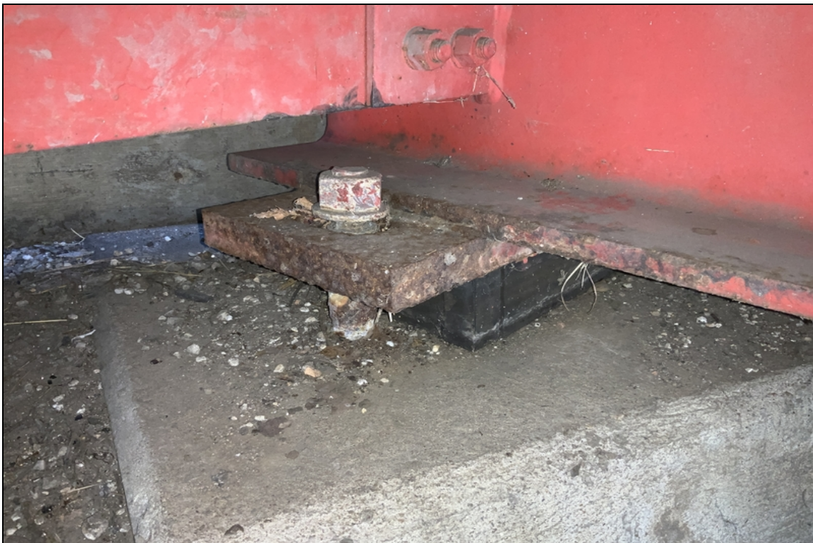
Bent 1 girder 5 and bearing 5.
