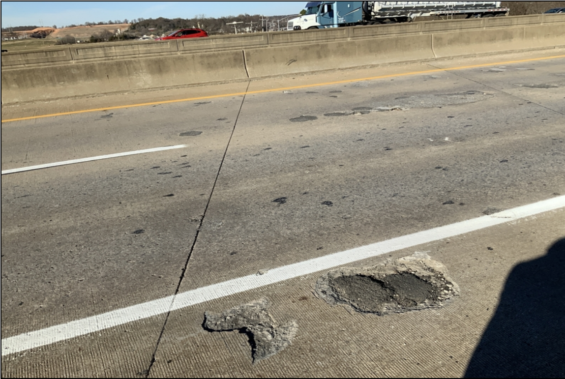
Span 2, spalls and failing patches.
