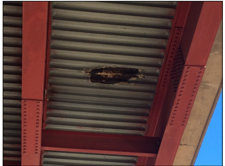
The metal SIP forms have areas with active corrosion at Span 2, Bay 5.
