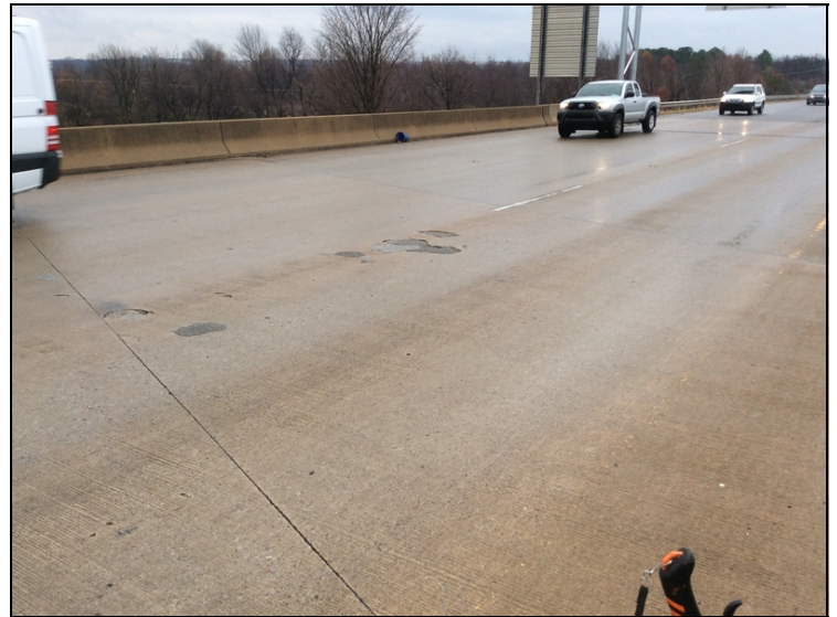
Span # 4 near centerline concrete delamination's and spalls with exposed reinforcing steel.
