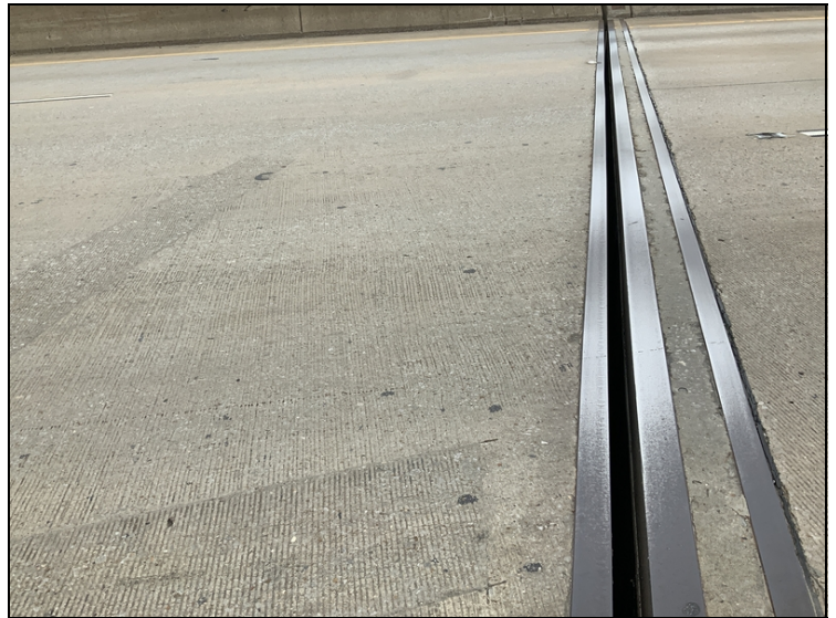
Bent 1 (West Abutment) and Bent 5 (East Abutment) compression joints are both missing and are leaking water along with dumping road debris on top of the bridge set and causing the active corrosion to the girder ends and bearings.
