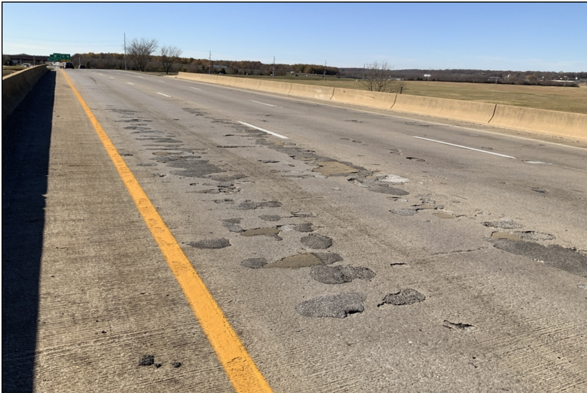
Span 3, several spalls and failing patches.
