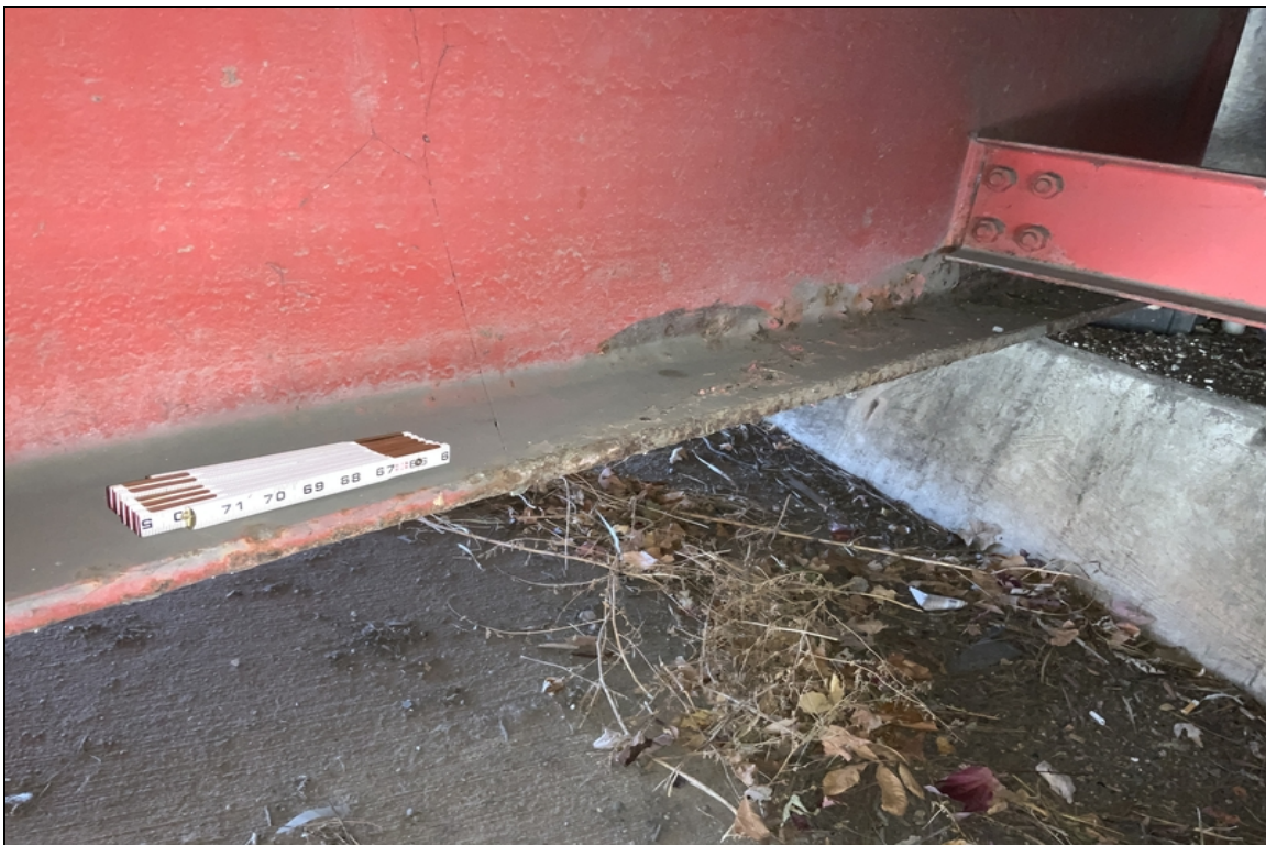
Bent 1 girder 5, corrosion
