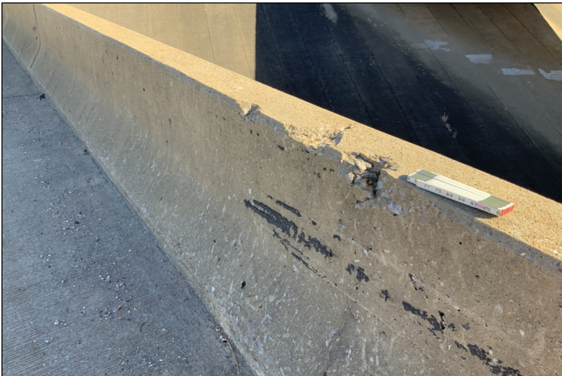
Right bridge rail, small spalls in the top of the rail.
