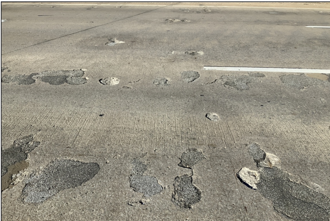
Span 3, spalls and failing patches.
