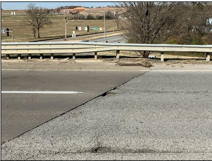
Pothole in approach roadway, East side of bridge.
