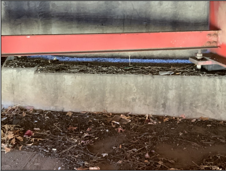
Bent 1 debris on cap
