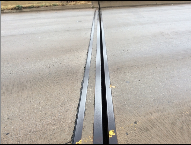
Bent # 1 open expansion joint.
