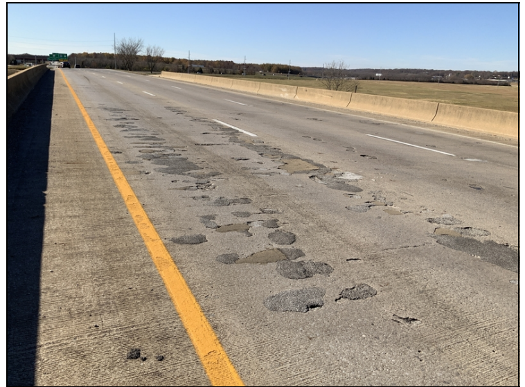
Span 3, several spalls and failing patches.
