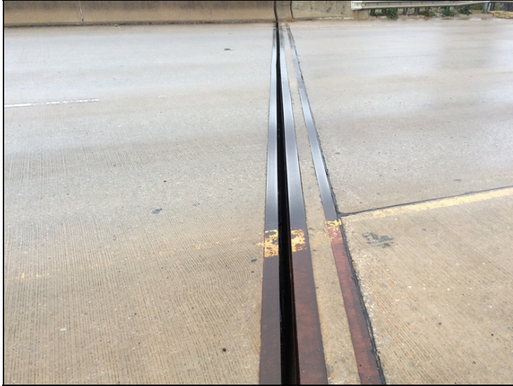
Bent # 5 open expansion joint.
