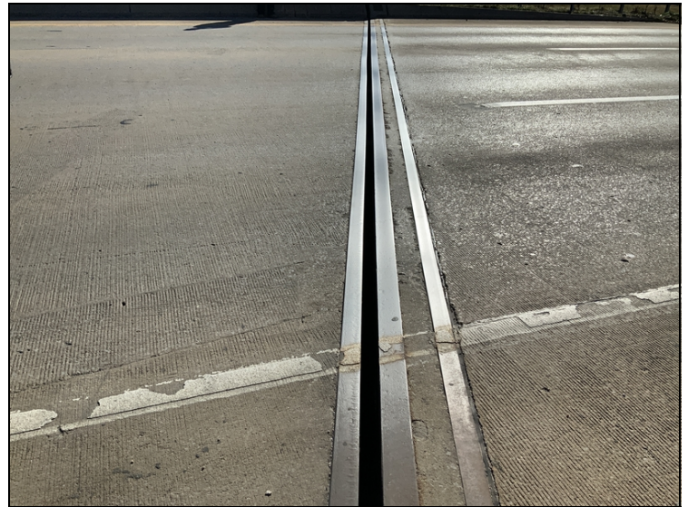
Bent 1, joint seal has fallen out.
