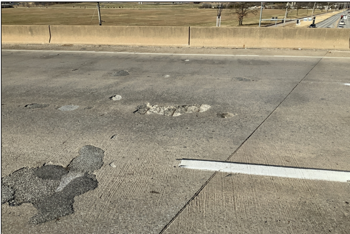
Span 3, large spall with exposed rebar.
