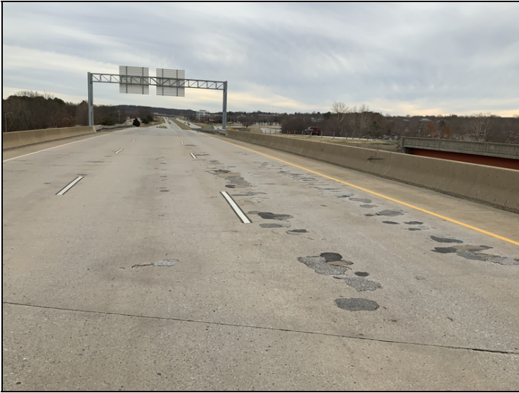
Span 3 has numerous failed asphalt patched areas along with exposed reinforcing steel that has initial section loss.
