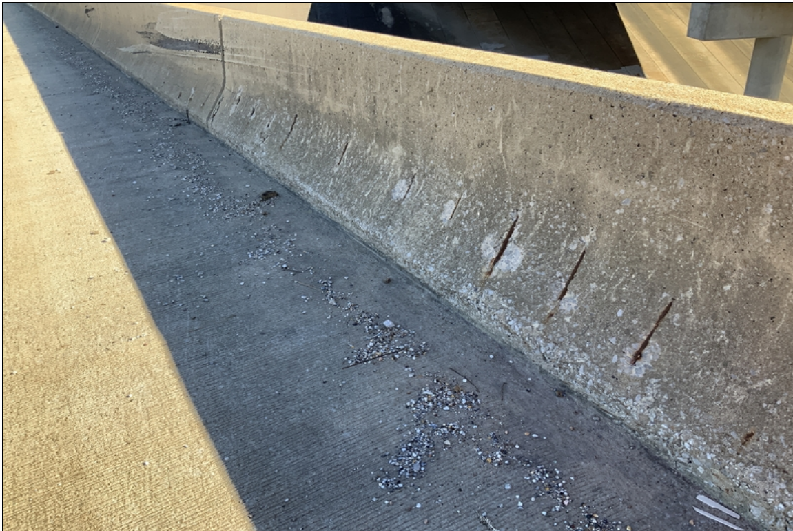
Right bridge rail has exposed rebar.
