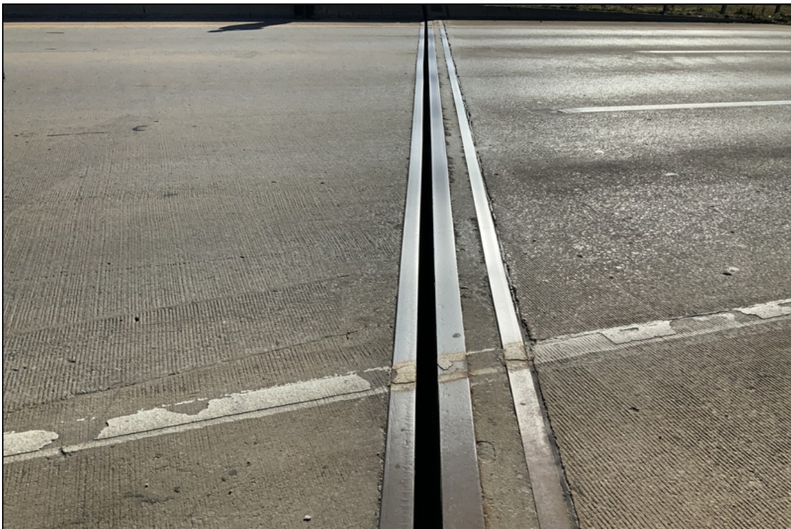
Bent 1, joint seal has fallen out.
