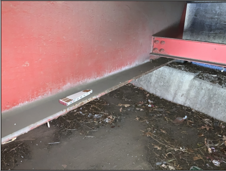
Bent 1 girder 4, corrosion to the bottom flange.
