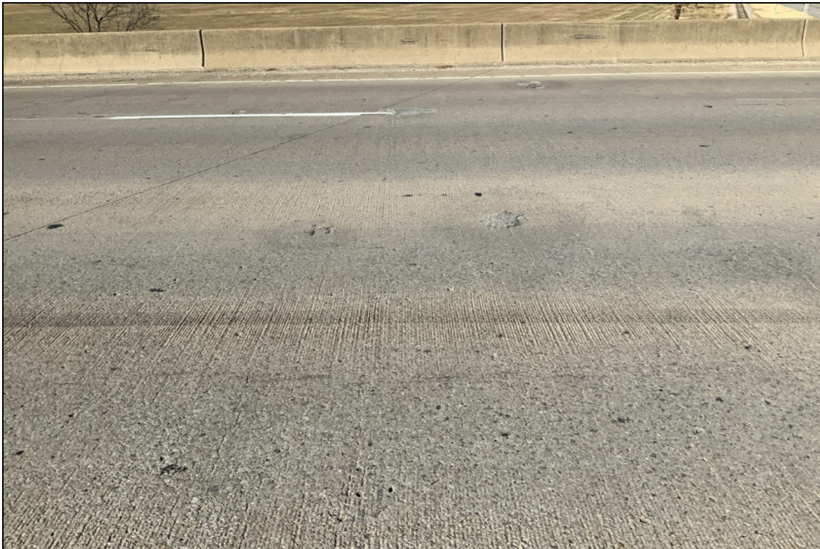
Span 2, transverse cracks and patches.
