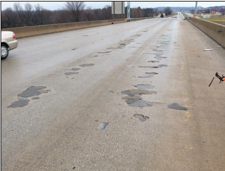
Span # 3 Right lane delamination's and spalling with exposed reinforcing steel.
