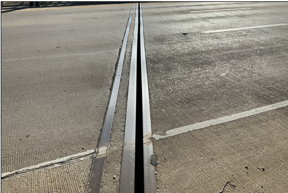
The joint seal at bent 5 has fallen out.
