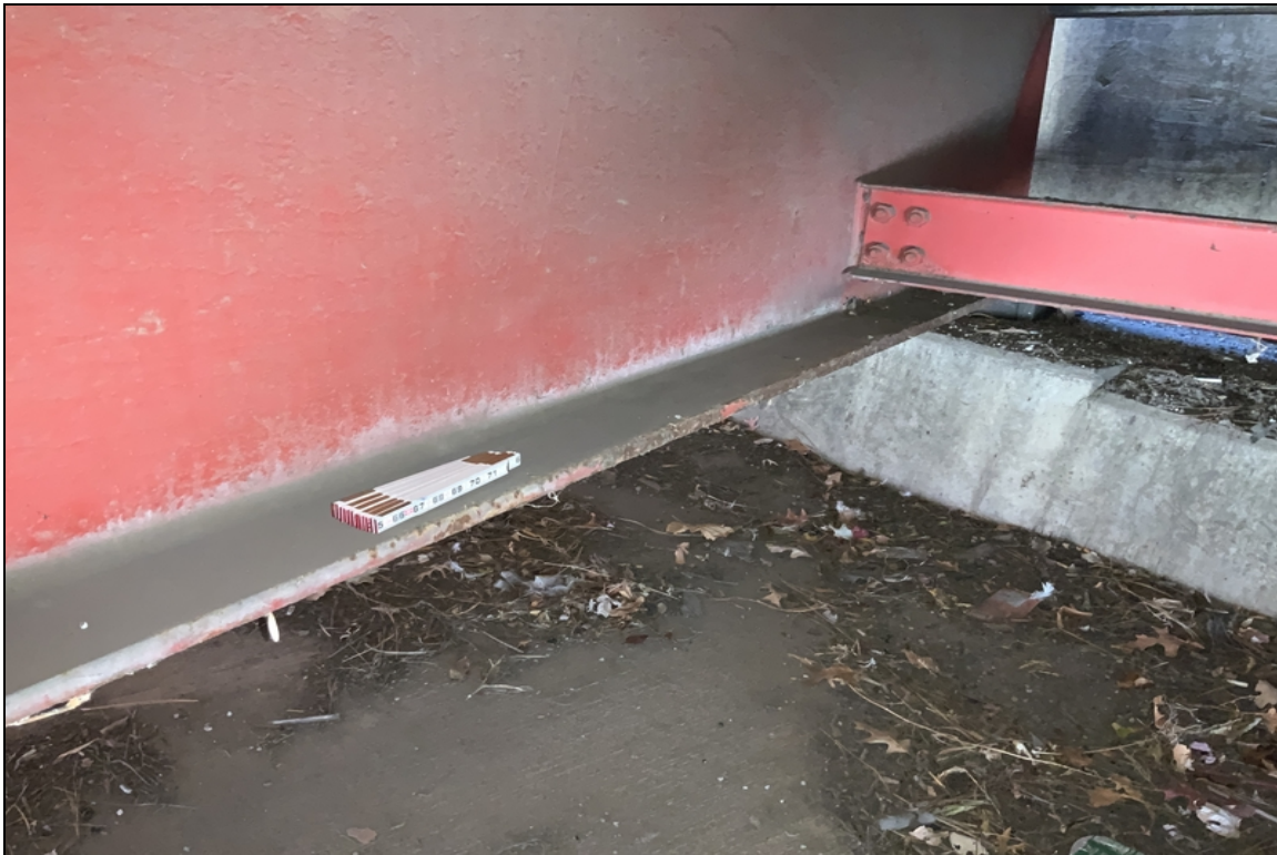
Bent 1 girder 4, corrosion to the bottom flange.
