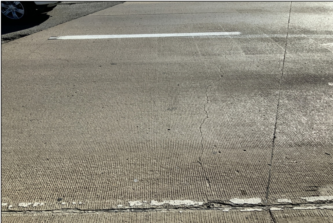
East approach slab, large transverse cracks.
