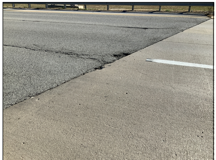
Pothole in approach roadway
