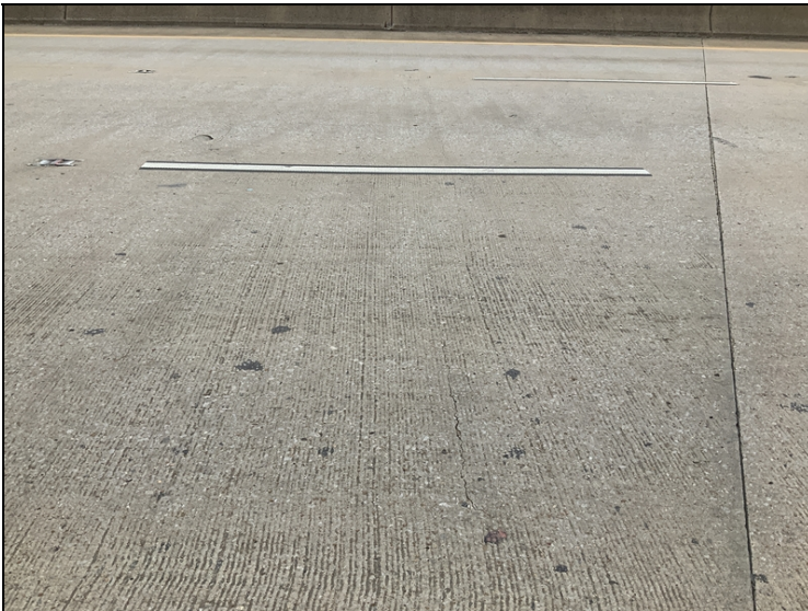
Typical seal-able cracking throughout the driving surface.
