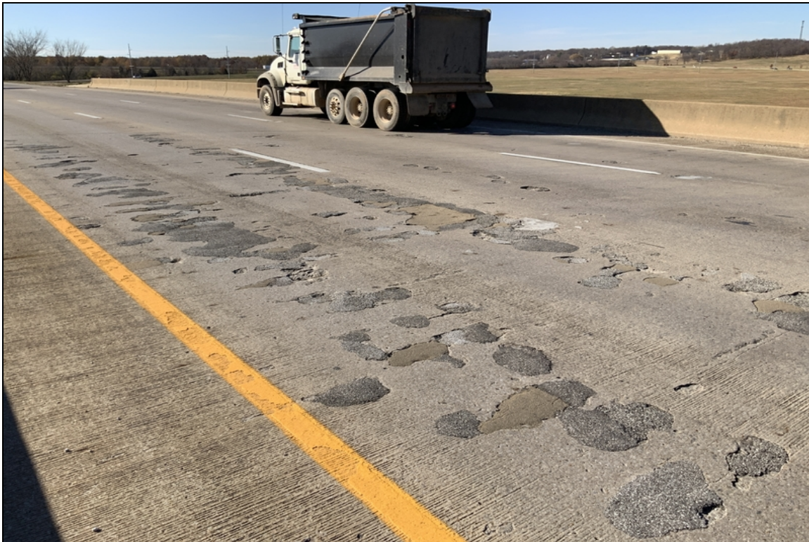
Span 3, several spalls and failing patches.
