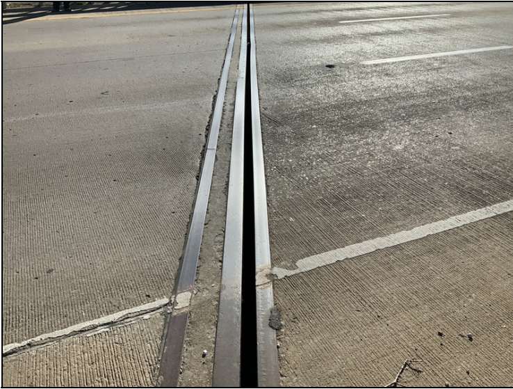
The joint seal at bent 5 has fallen out.
