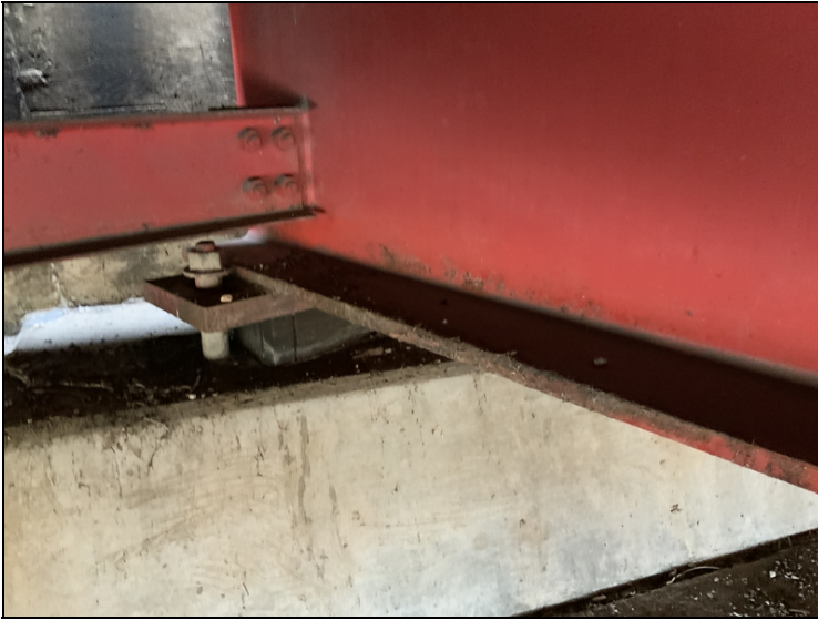
Bent 1 (West Abutment) and Bent 5 (East Abutment) girders 1 - 7 have active corrosion with flaking rust and pitting.
