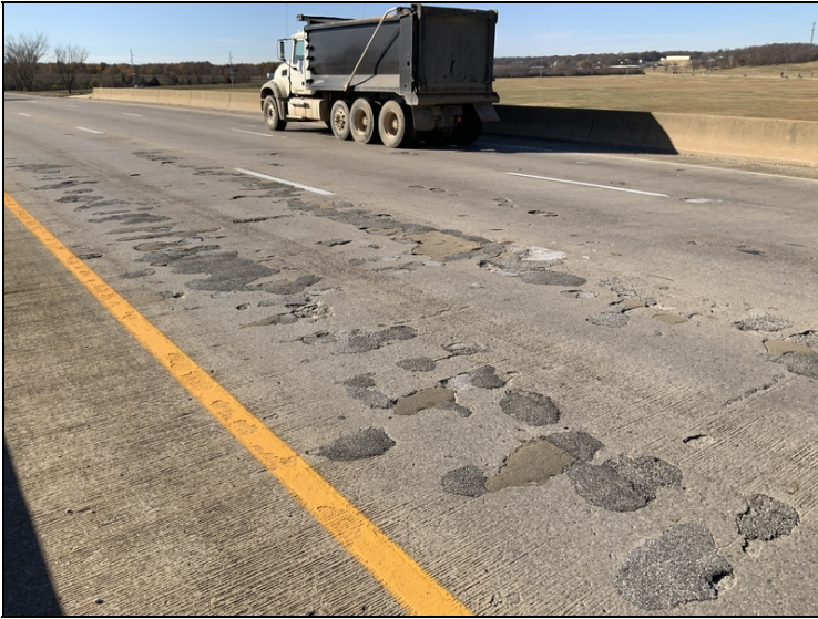
Span 3, several spalls and failing patches.
