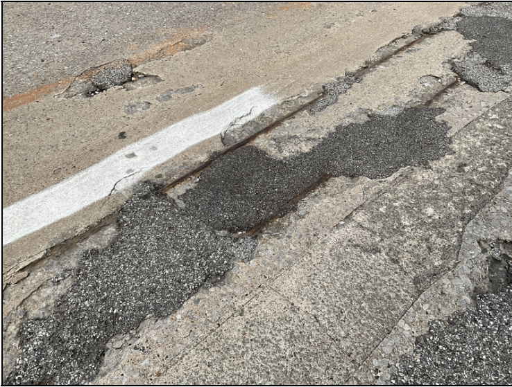
Span 1, right lane-Large area of spalling with exposed reinforcing steel.
