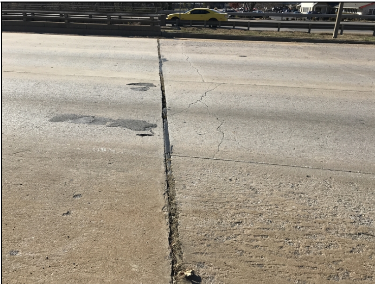
Expansion joint at Bent # 4.
