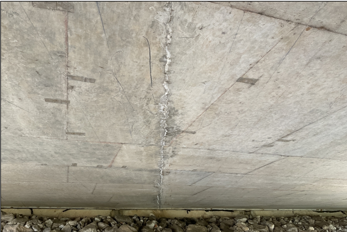
Span 1 undersurface-Efflorescence at construction joint.
