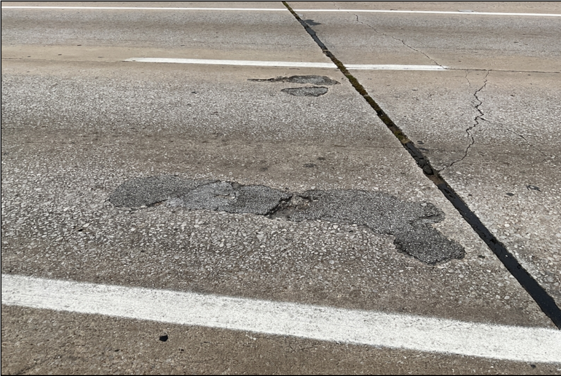
Span 3, right lane-Spalls in driving surface.
