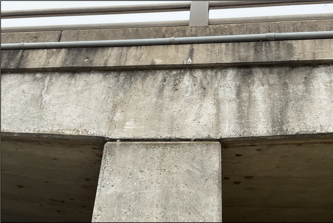
Vertical cracking in slab exterior edge on right side over bent 3.
