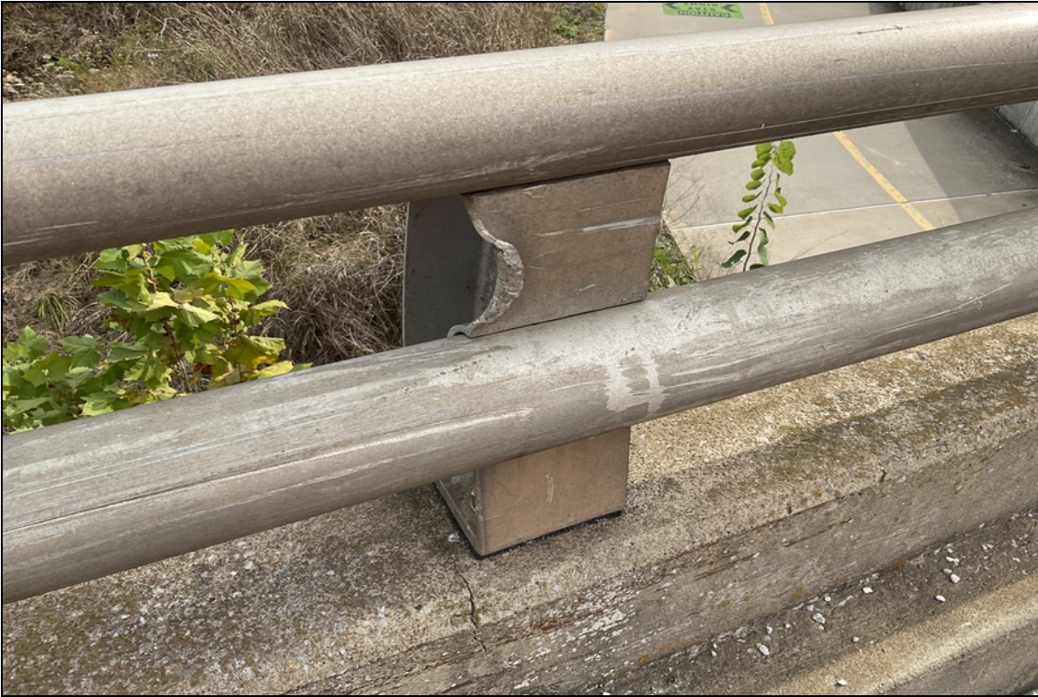
Post # 7 of the right bridge railing has minor collision damage.
