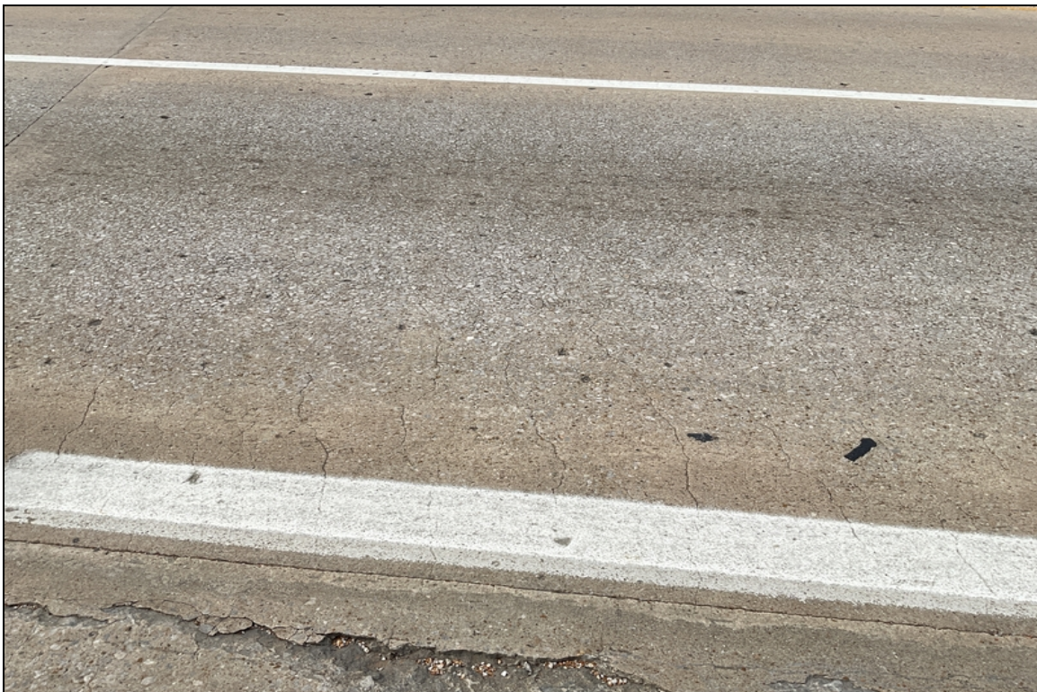
Span 2, center lane-Mapcracking.
