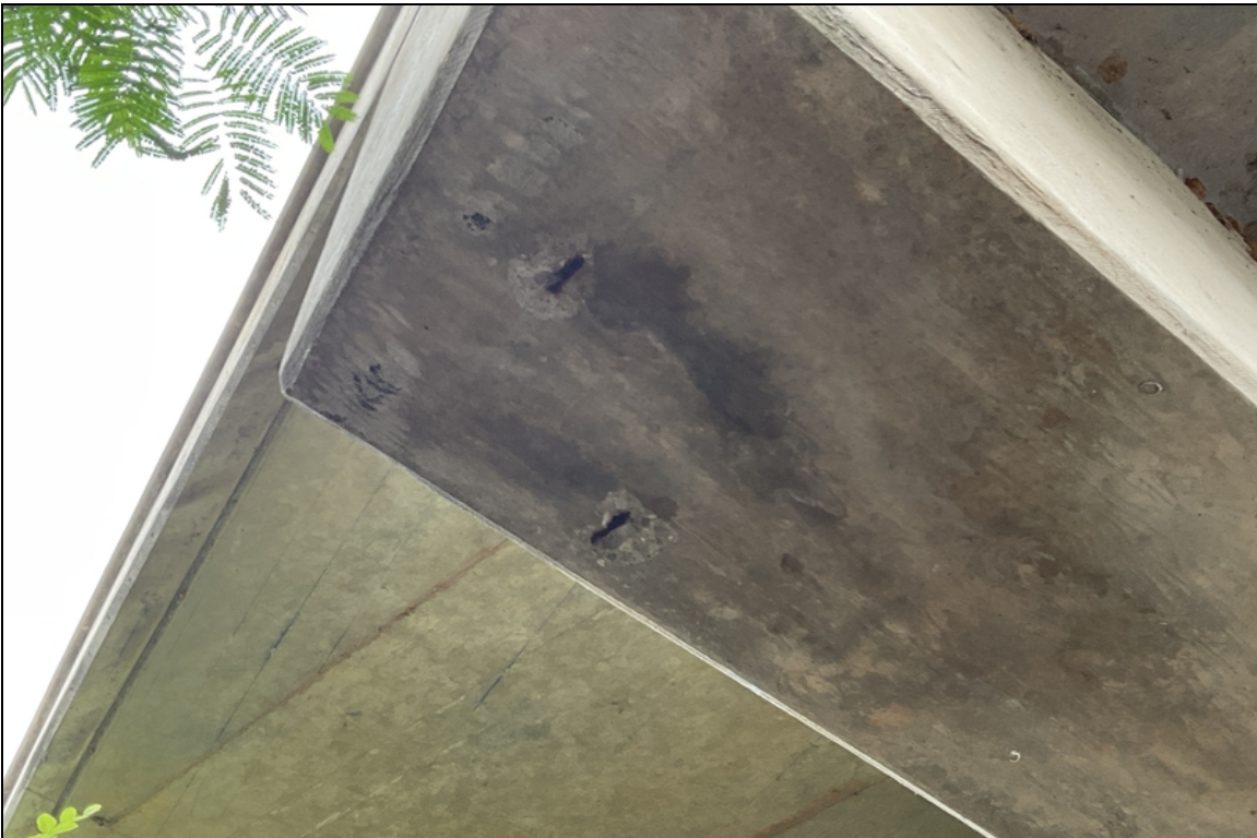
Bent 3 cap, left side-Shallow spalls with exposed reinforcing steel in undersurface.
