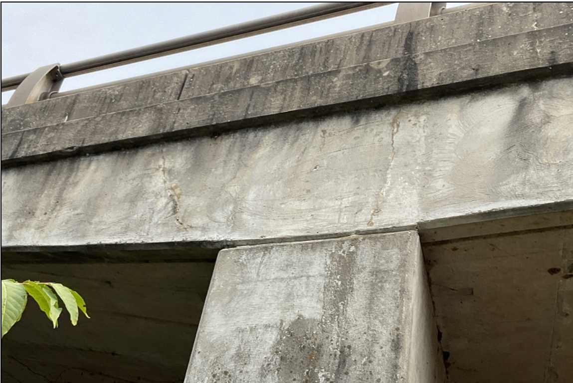
Vertical and diagonal cracking in left exterior side of slab over bent # 2.
