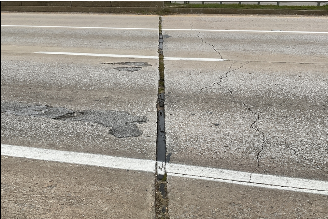
Abutment # 2 expansion joint sealant has failed with incompressible material in the joint.
