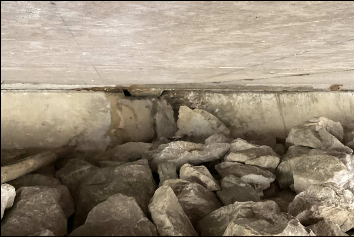
Abutment 2-Spall at key way near centerline.
