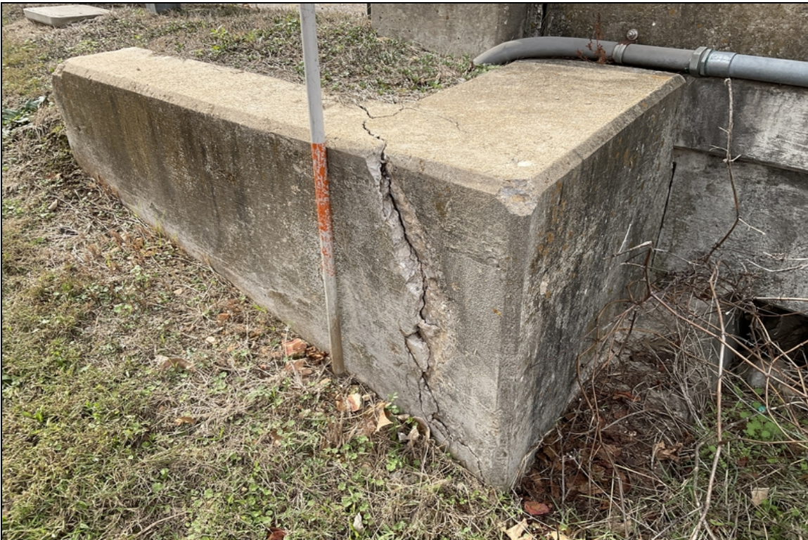
The right turn back portion of abutment # 1 is fractured outside the bearing area.
