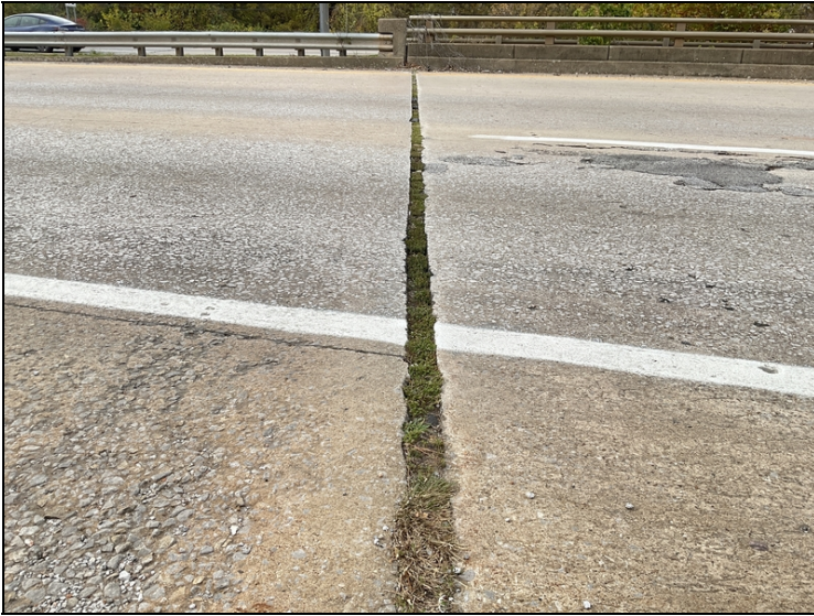
Abutment # 1 expansion joint-Debris impaction.
