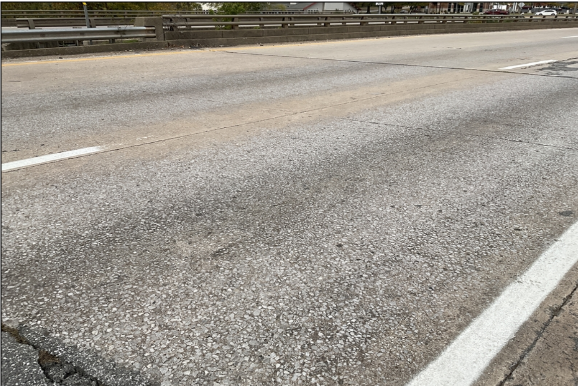
South approach slab-Wear / abrasion.
