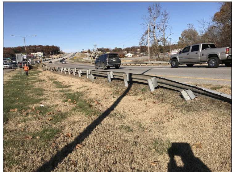
Southwest approach guardrail. Collision damage.
