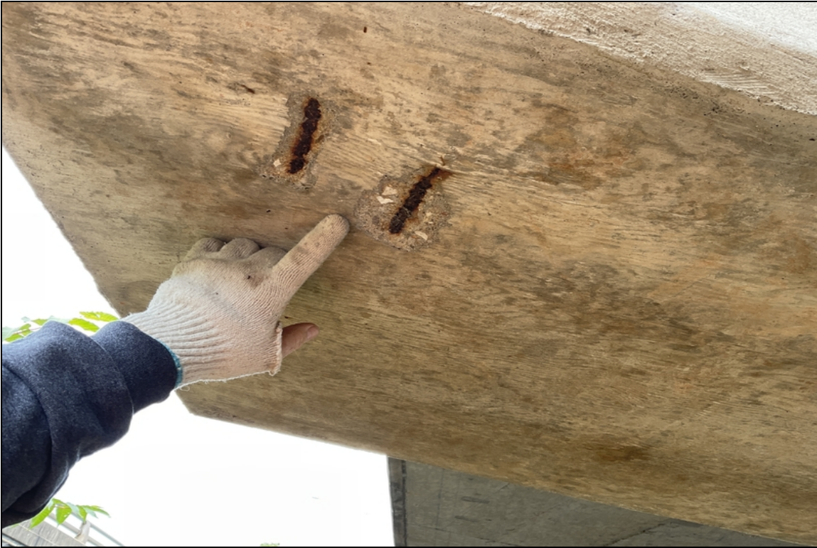
Bent 2 cap, left end-Shallow spalls with exposed reinforcing steel in undersurface.
