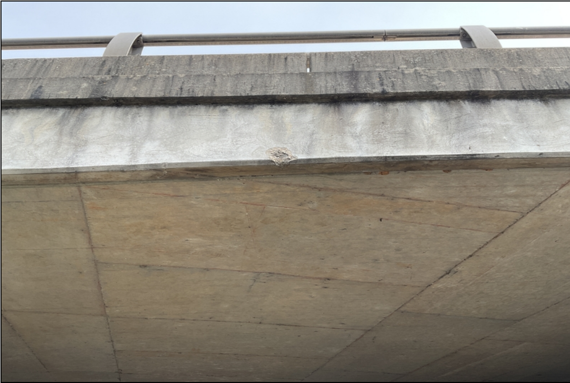
Span 1, left side-Shallow spall over pedestrian trail.
