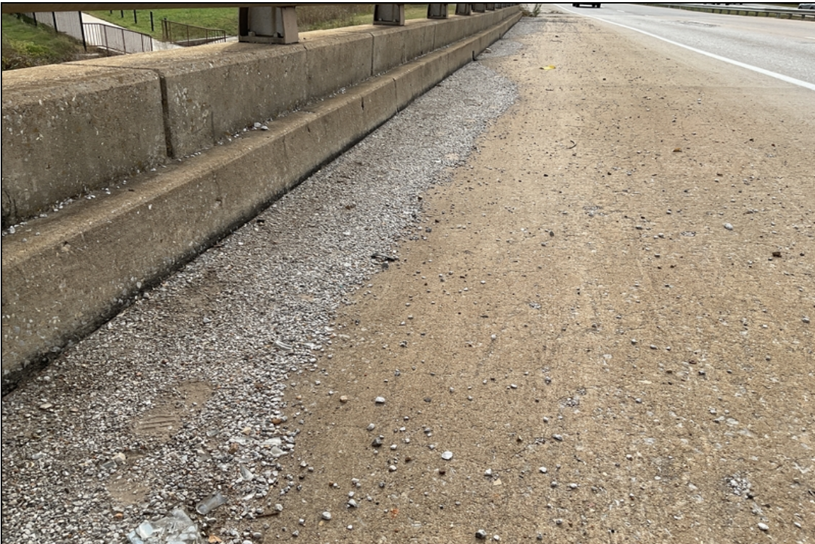
Dirt and debris in gutters.
