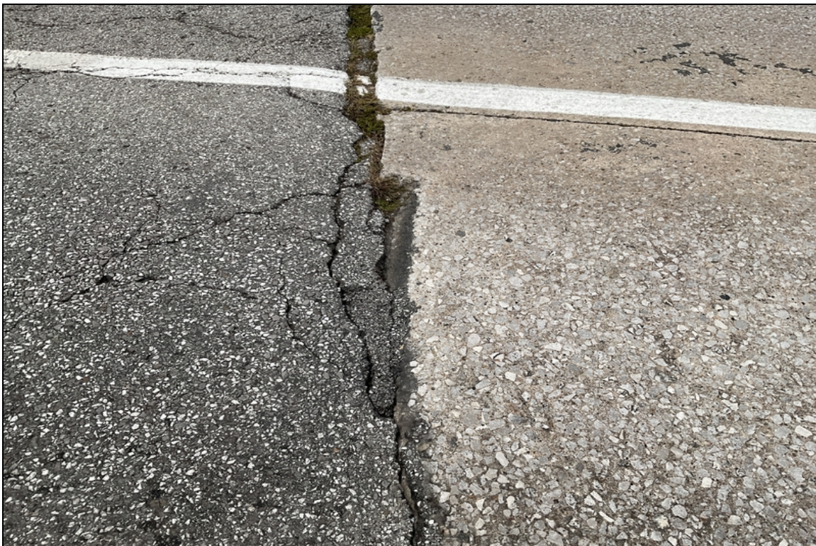
South approach slab-Spall at roadway juncture.
