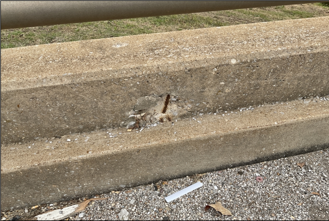
Span 3, right concrete railing at abutment # 2-Spall with exposed reinforcing steel.
