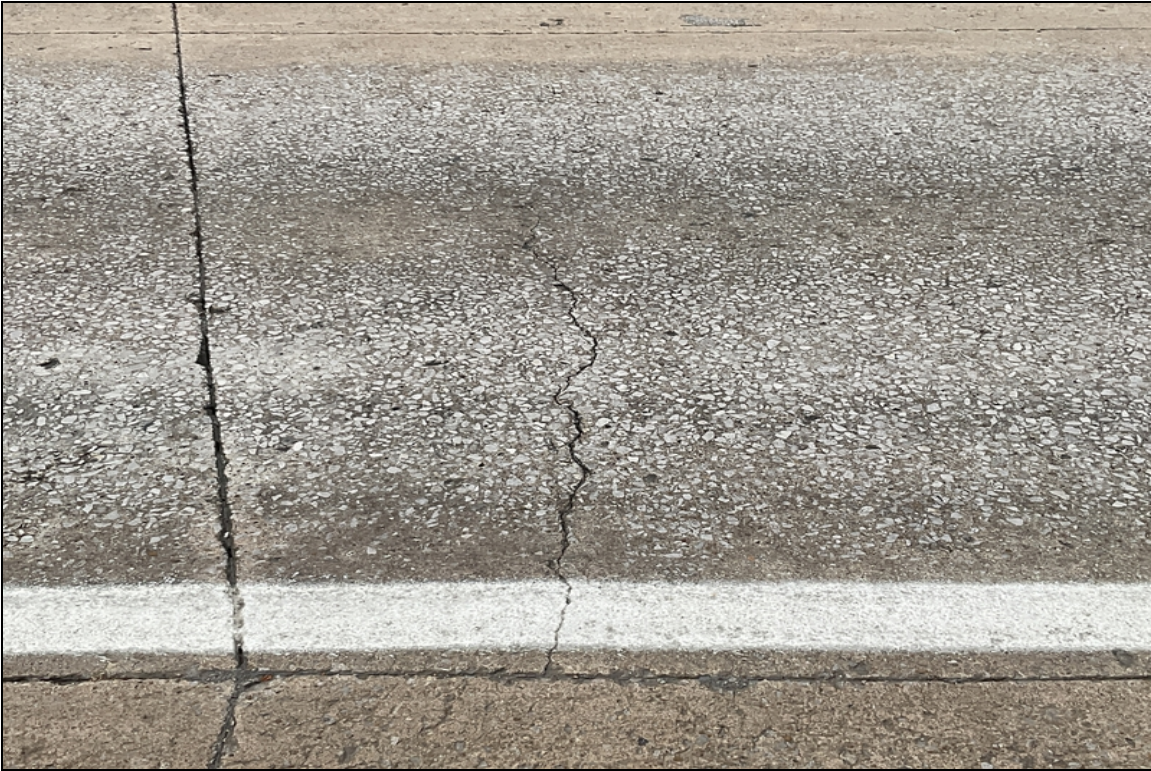
South approach slab, right lane-Moderate width transverse crack.
