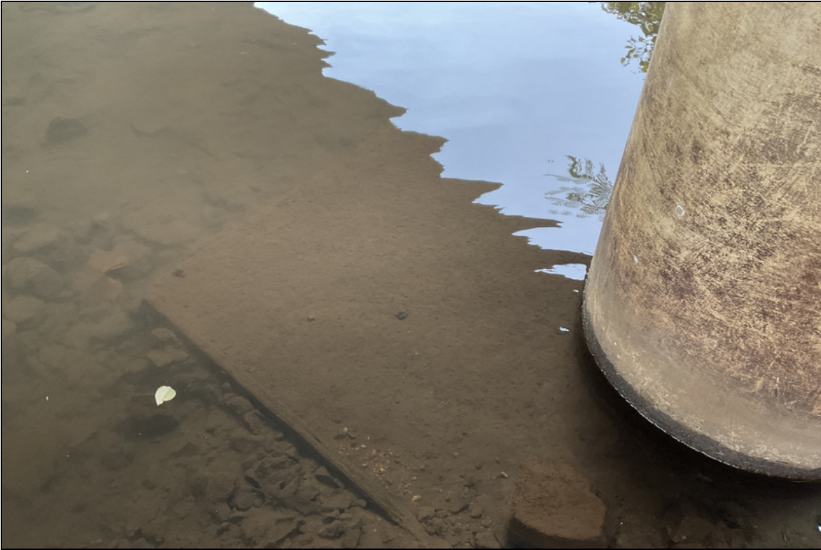
Bent 3, column 1 footing exposed.
