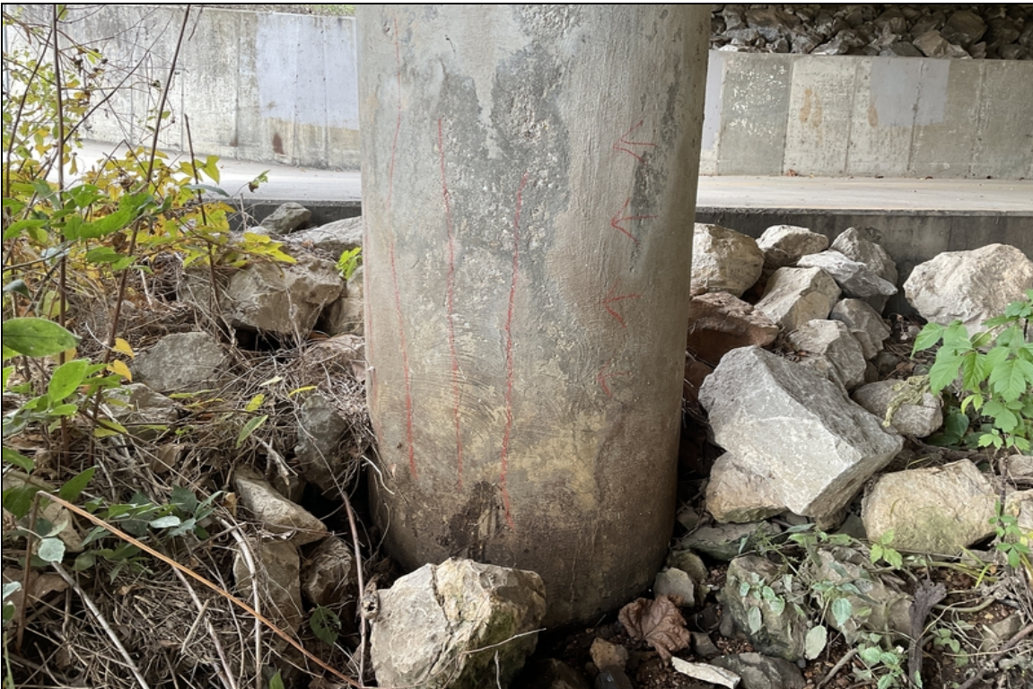
Bent # 2, column # 3-Numerous vertical cracks on approximately 6" spacing.
