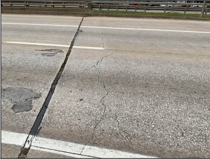
North approach slab-Wide transverse cracking.
