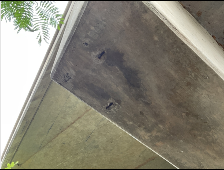
Bent 3 cap, left side-Shallow spalls with exposed reinforcing steel in undersurface.
