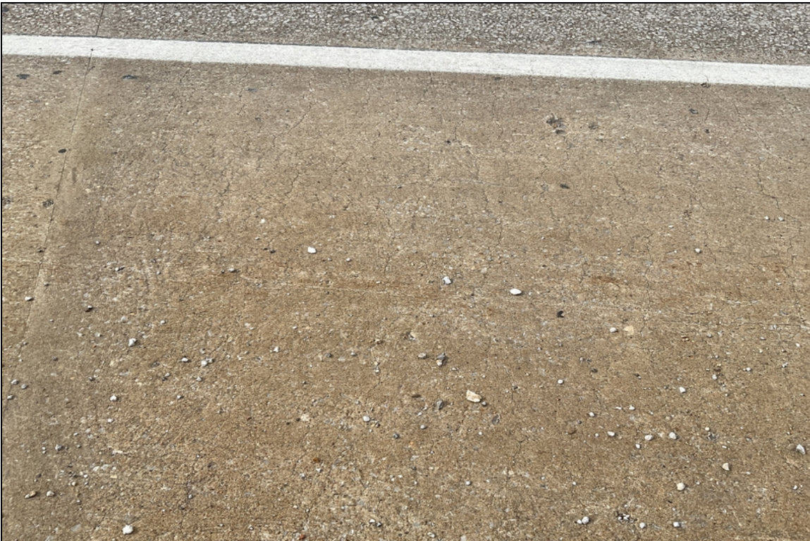
Span # 2, right shoulder-Mapcracking.
