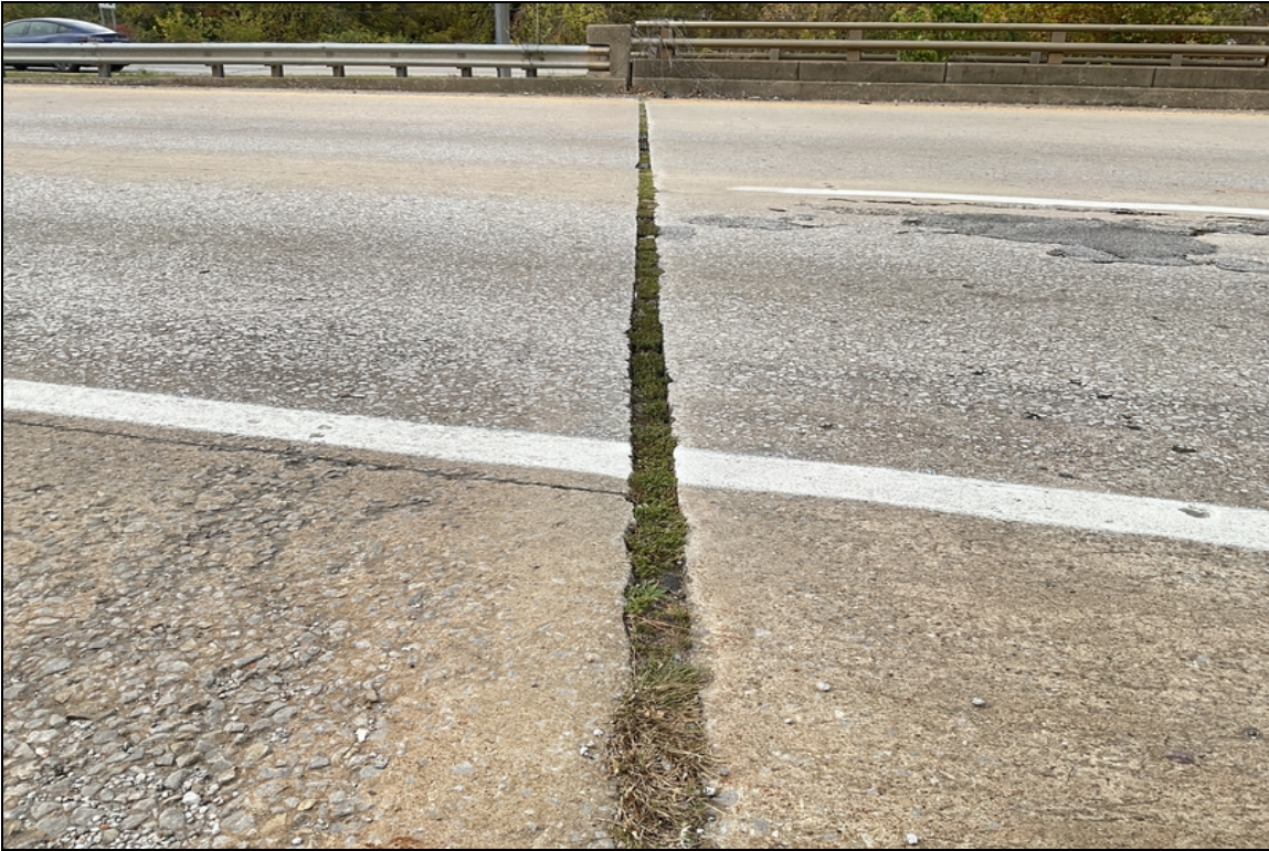
Abutment # 1 expansion joint-Debris impaction.
