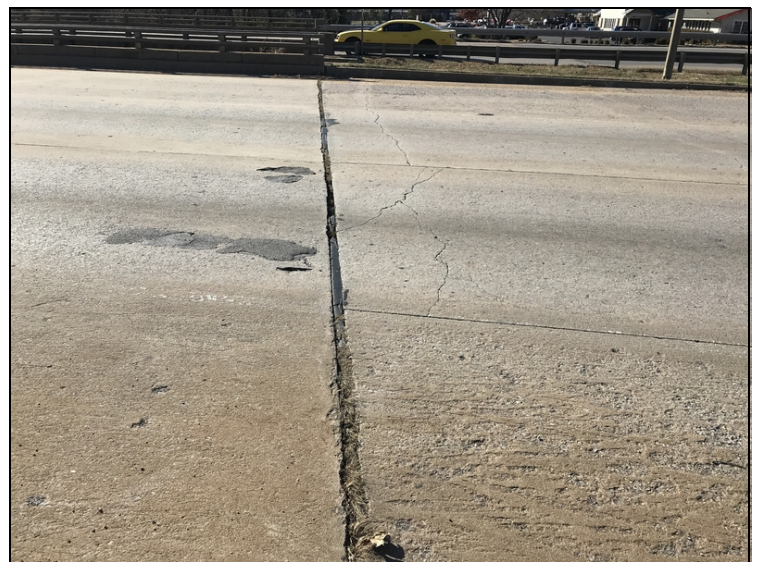
Expansion joint at Bent # 4.
