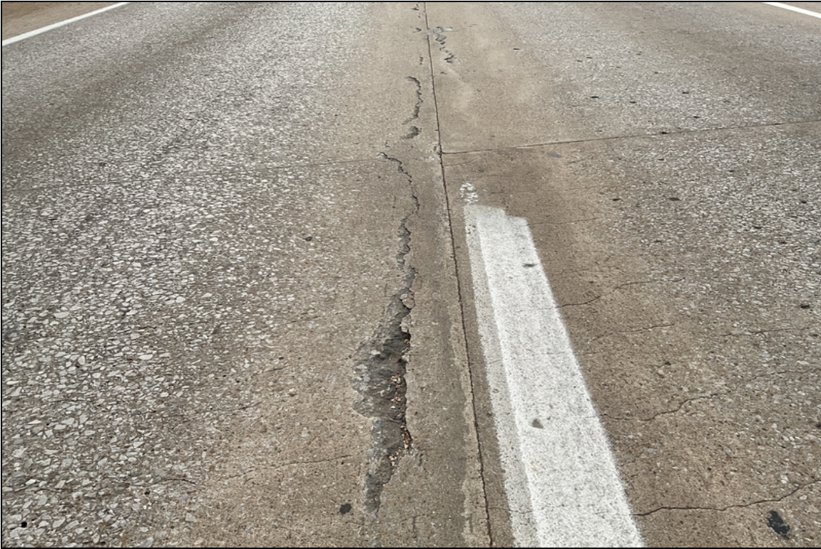
Delaminated areas along centerline.
