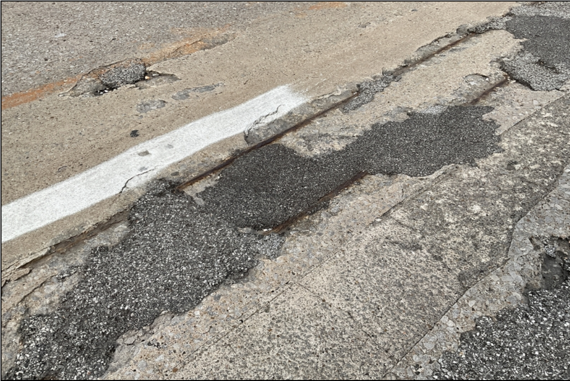
Span 1, right lane-Large area of spalling with exposed reinforcing steel.
