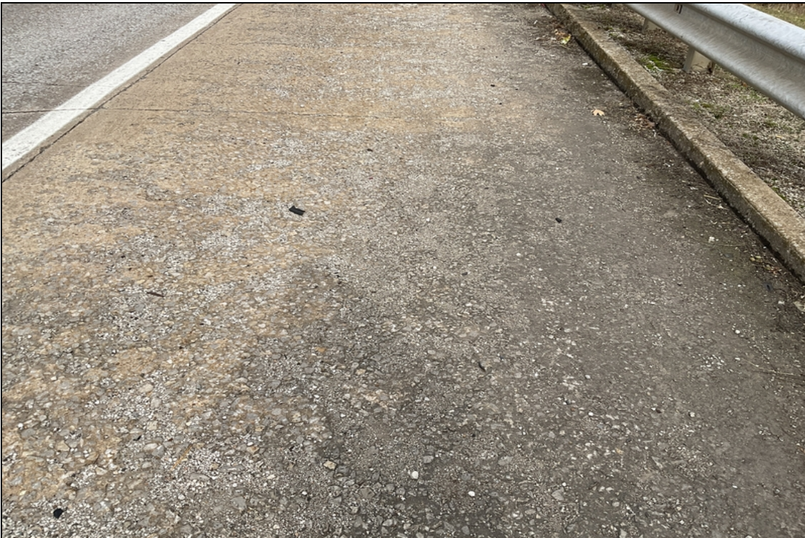
The gutters of the South approach roadway has medium scaling.
