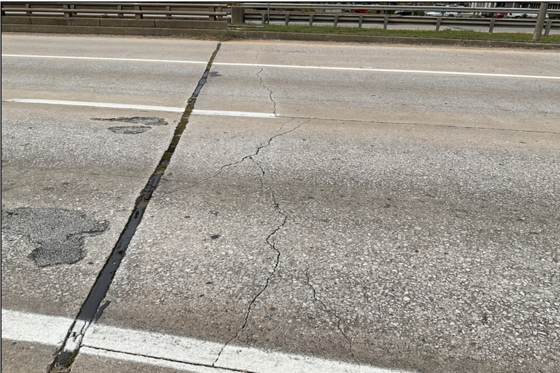
North approach slab-Wide transverse cracking.
