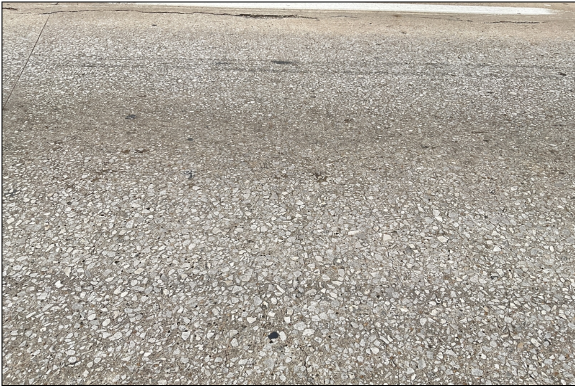
Span # 2, right lane-Mapcracking.
