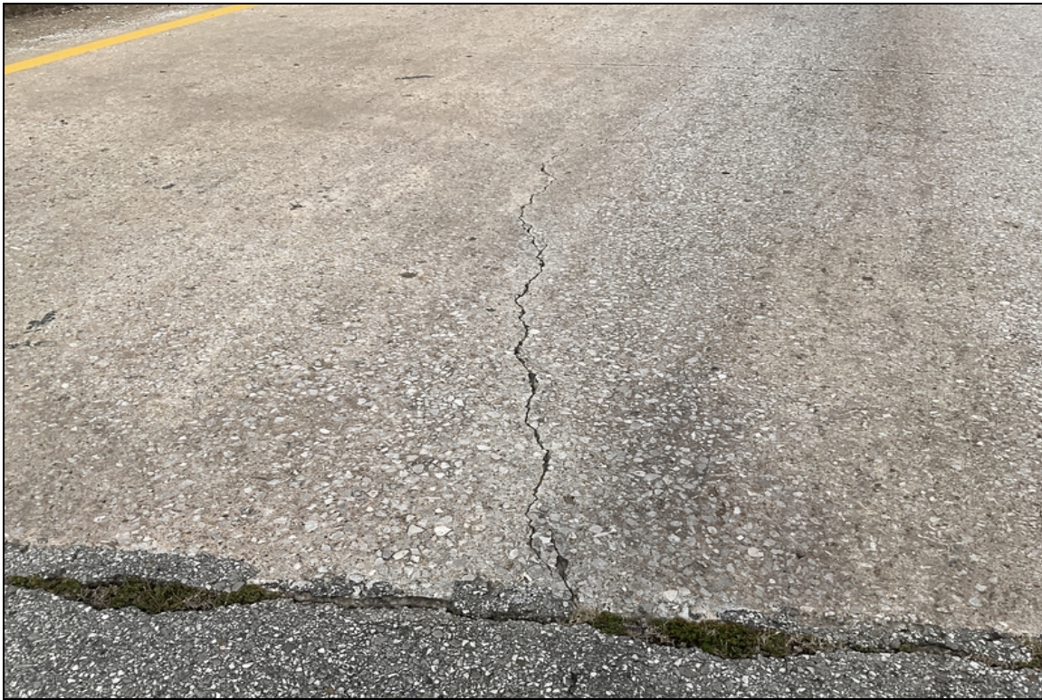
South approach slab, left lane-Wide longitudinal crack.
