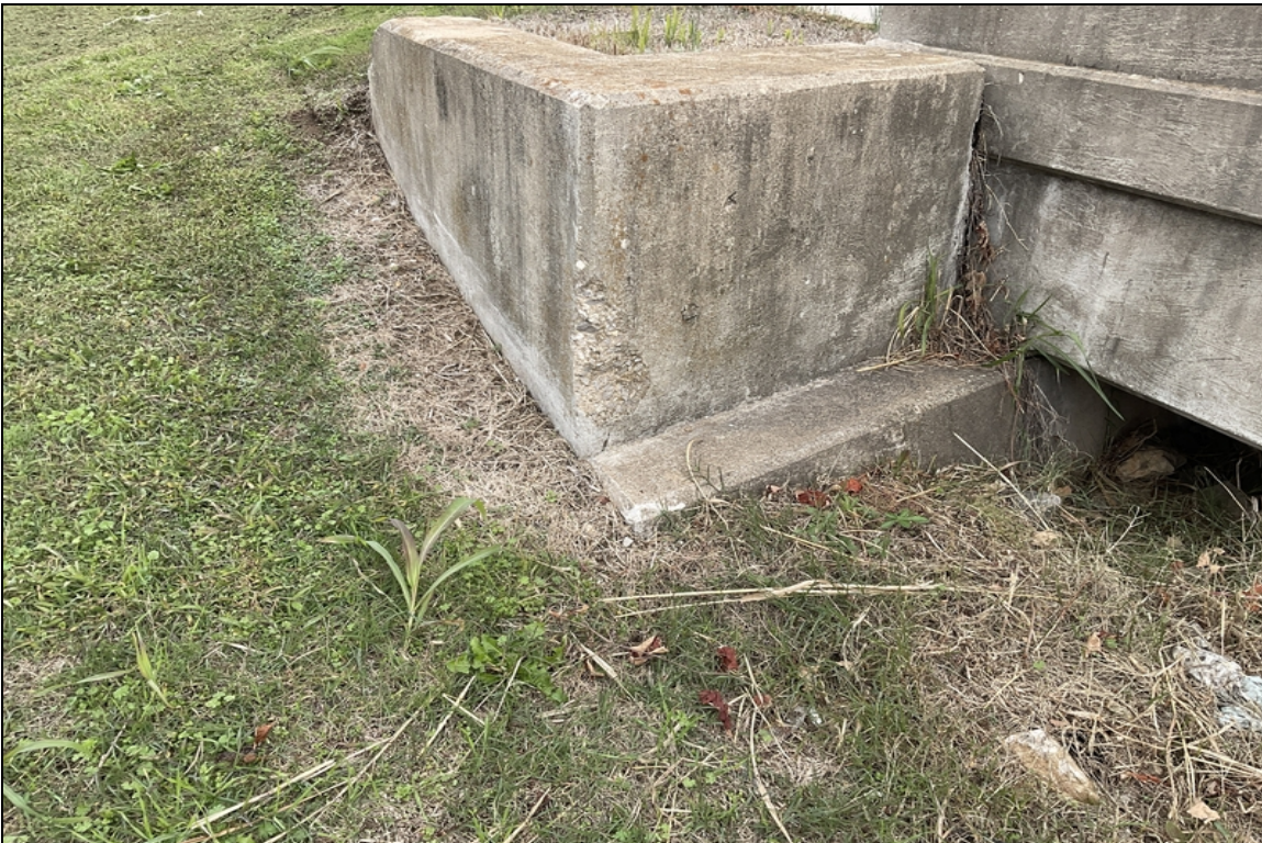
Abutment 2, left side-Shallow spall that appears to be from mowing operations.
