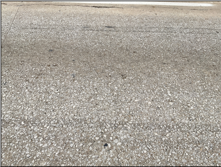
Span # 2, right lane-Mapcracking.
