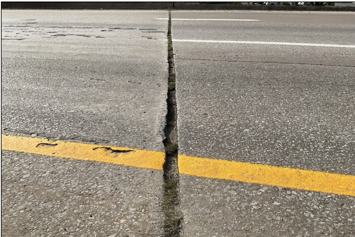
Abutment 2 expansion joint-Failing sealant with debris impactation.
