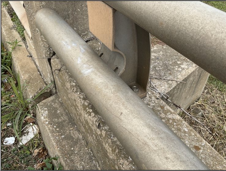
Span 3, right side at abutment 2-Missing bolt at post connection.
