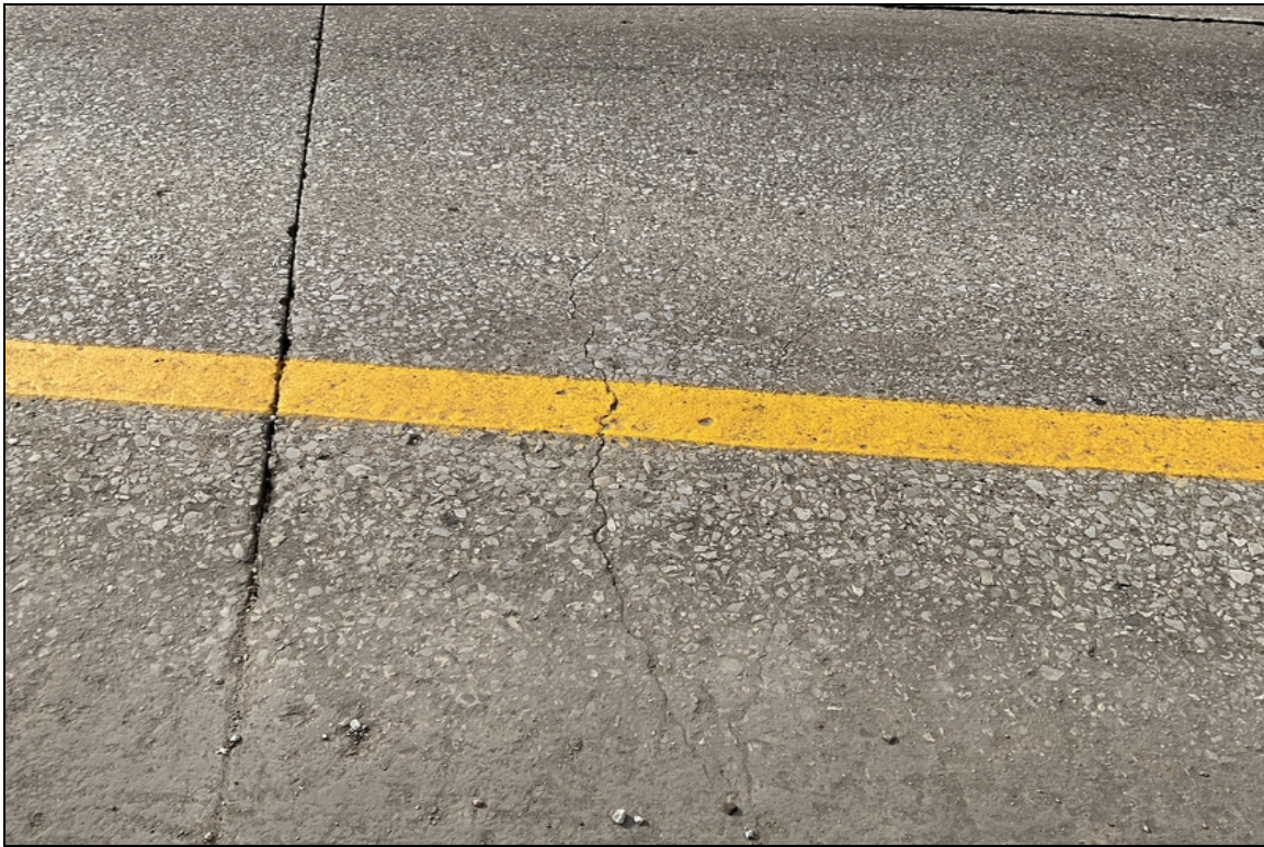
South approach slab-Transverse crack.
