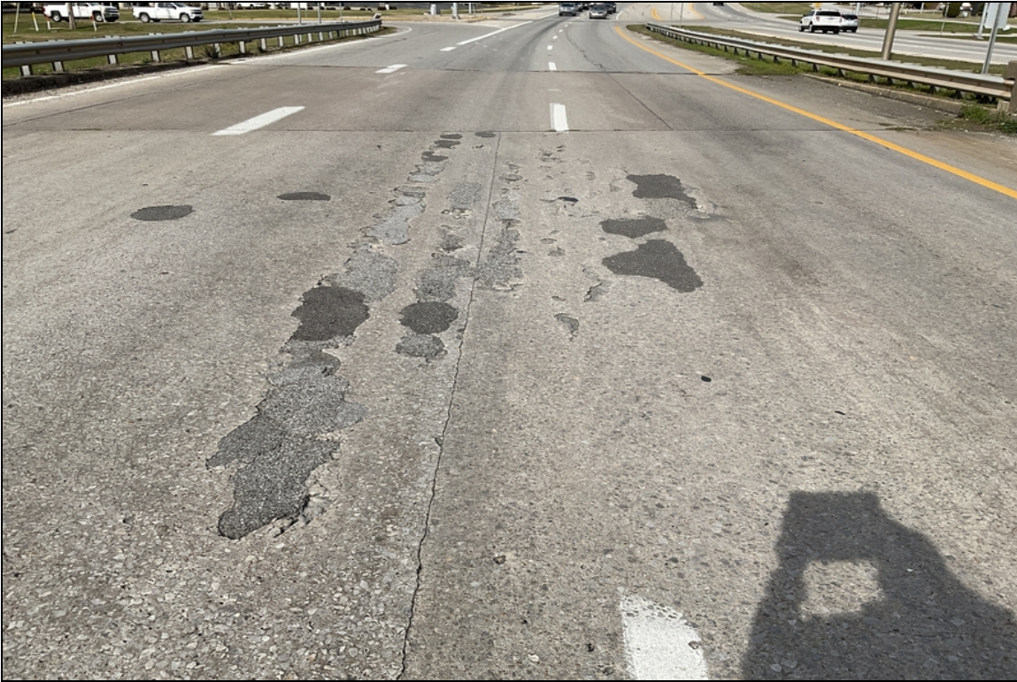
Driving surface of span # 3 has an area of spalling with failing asphalt repairs approximately 30' long x 5' wide located near centerline.
