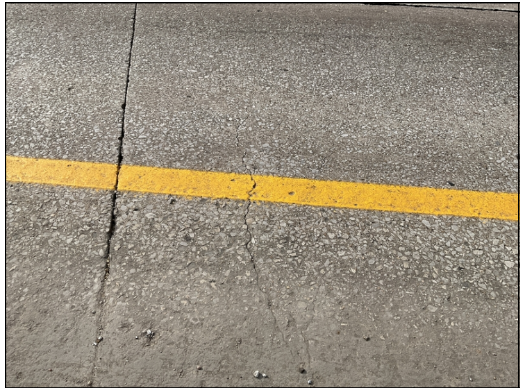
South approach slab-Transverse crack.
