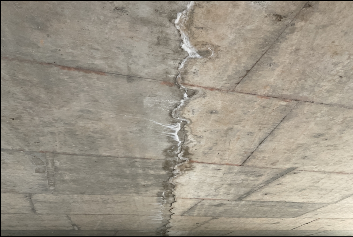
Span 1-Efflorescence at centerline construction joint.
