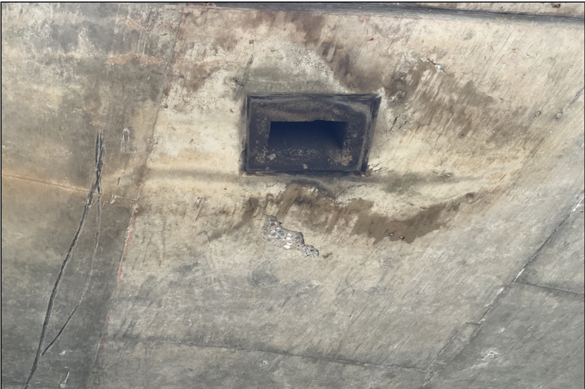
The undersurface of Span # 1 has a shallow spall and delaminated areas adjacent to the deck drain at mid-span.
