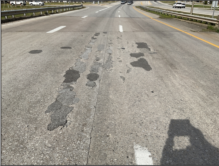
Driving surface of span # 3 has an area of spalling with failing asphalt repairs approximately 30' long x 5' wide located near centerline.
