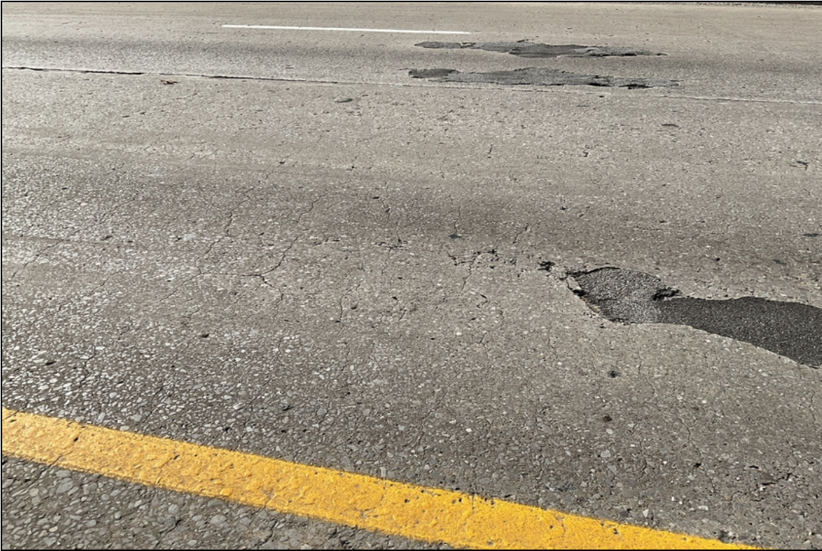
Span -Mapcracking.
