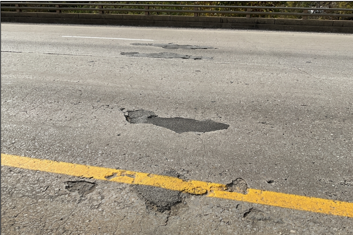
Spalls with asphalt repairs over bent 2.
