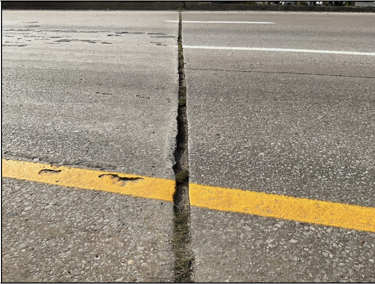
Abutment # 2 expansion joint-Failing sealant with debris impaction.
