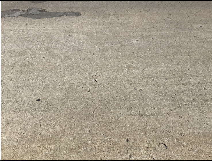
Transverse and map cracking over Bent # 2.
