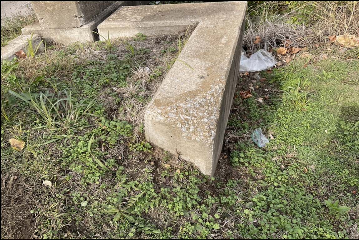
Abutment 1, right side-Spall in turn back portion of abutment.
