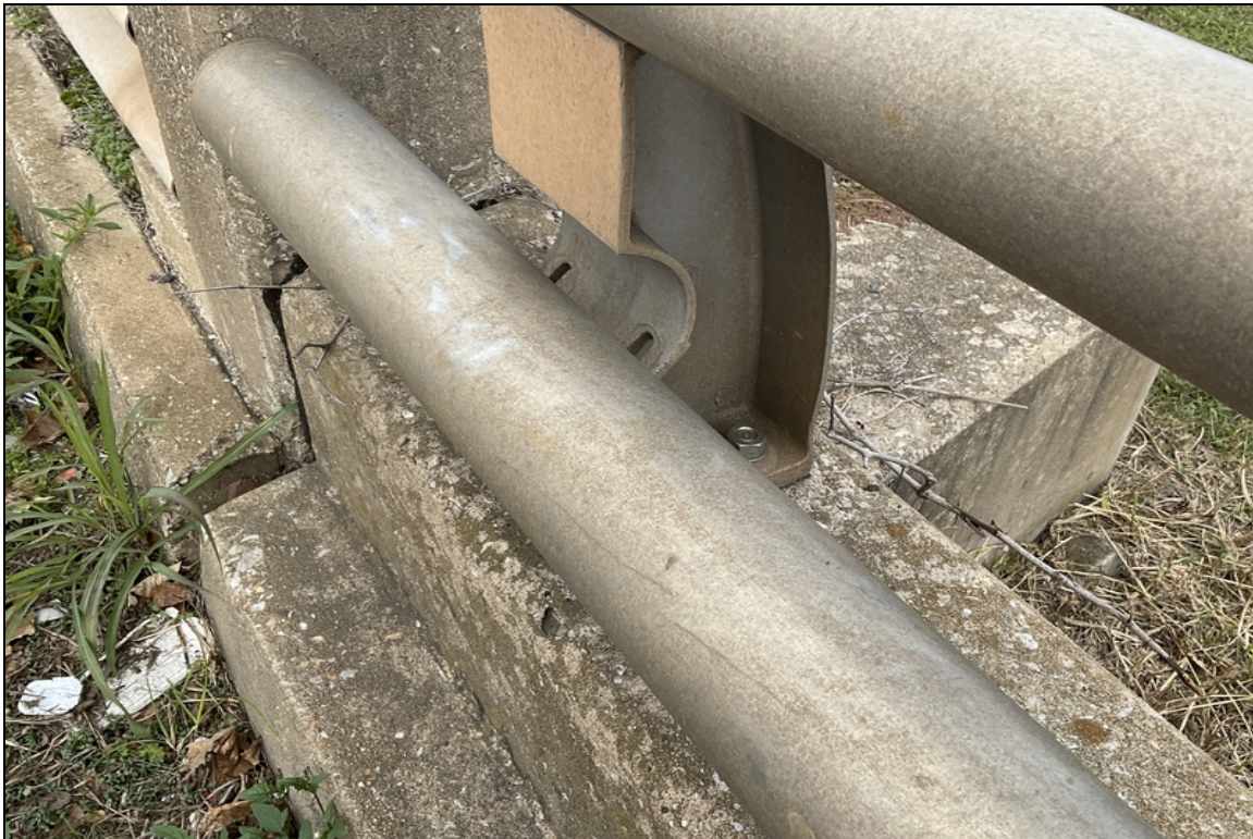
Span 3, right side at abutment 2-Missing bolt at post connection.
