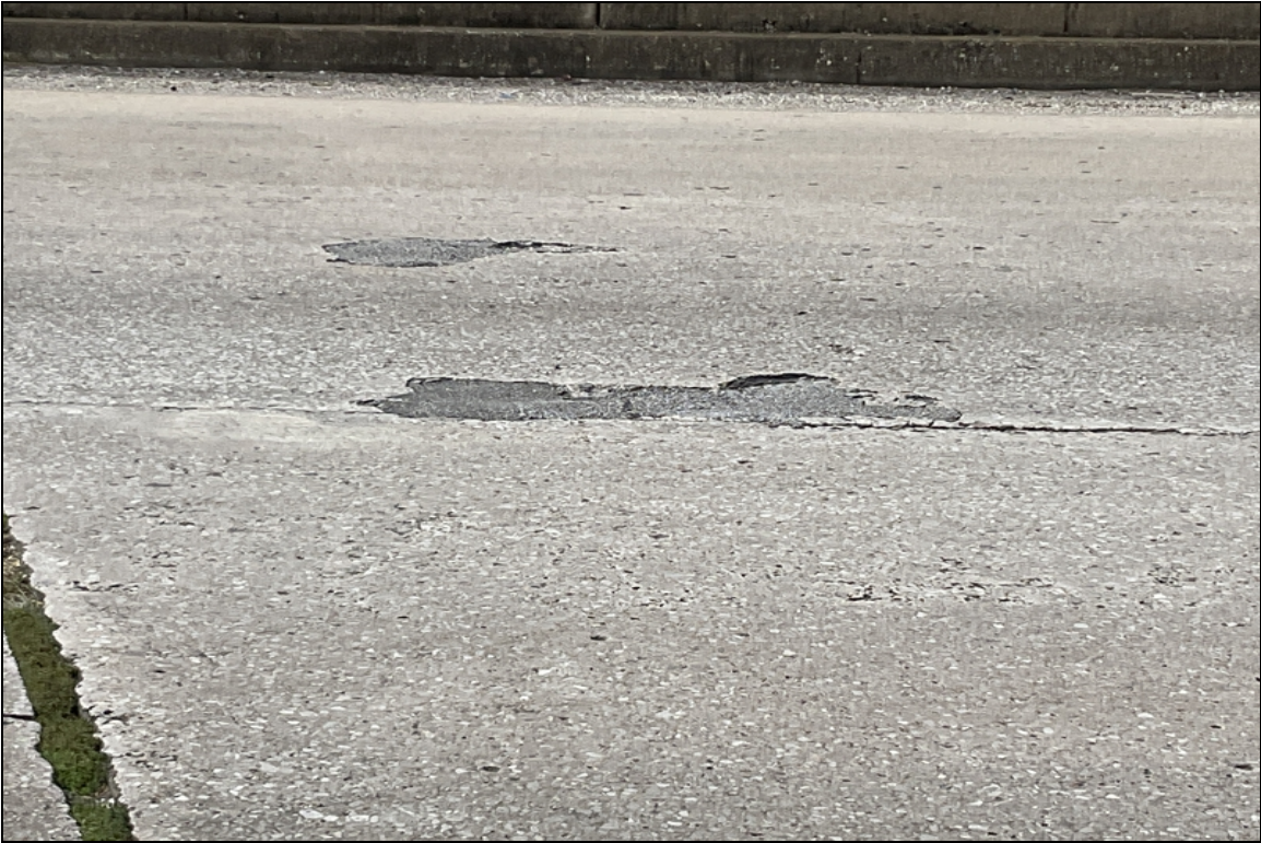
Span 1, center lane-Spalls with asphalt repairs.
