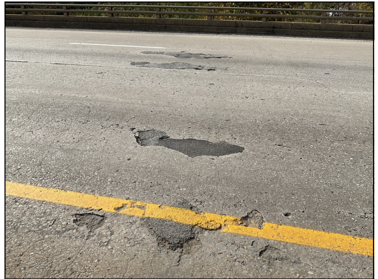
Spalls with asphalt repairs over bent 2.
