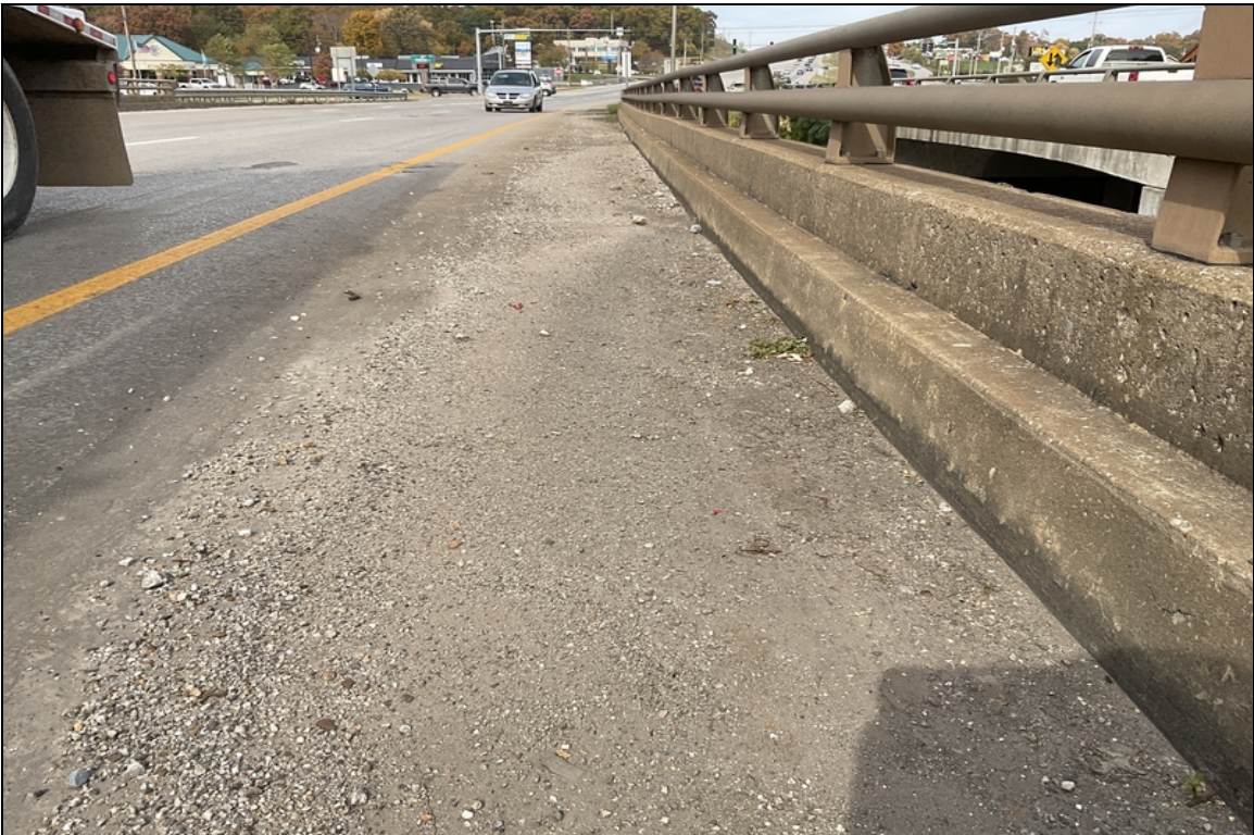
Dirt and debris accumulation in gutters.
