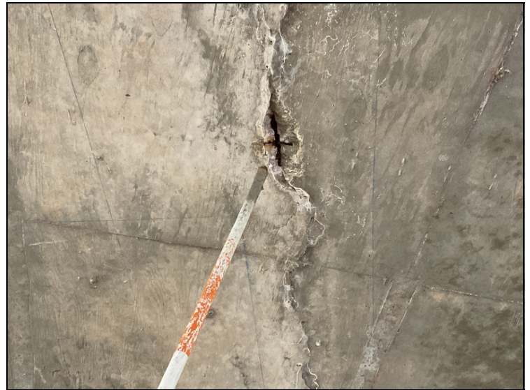
Span # 3-Spall with exposed reinforcing steel in slab undersurface in centerline construction joint.
