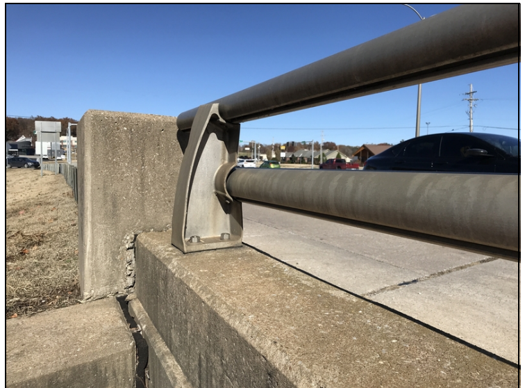
Span # 3 loose bridge railing.
