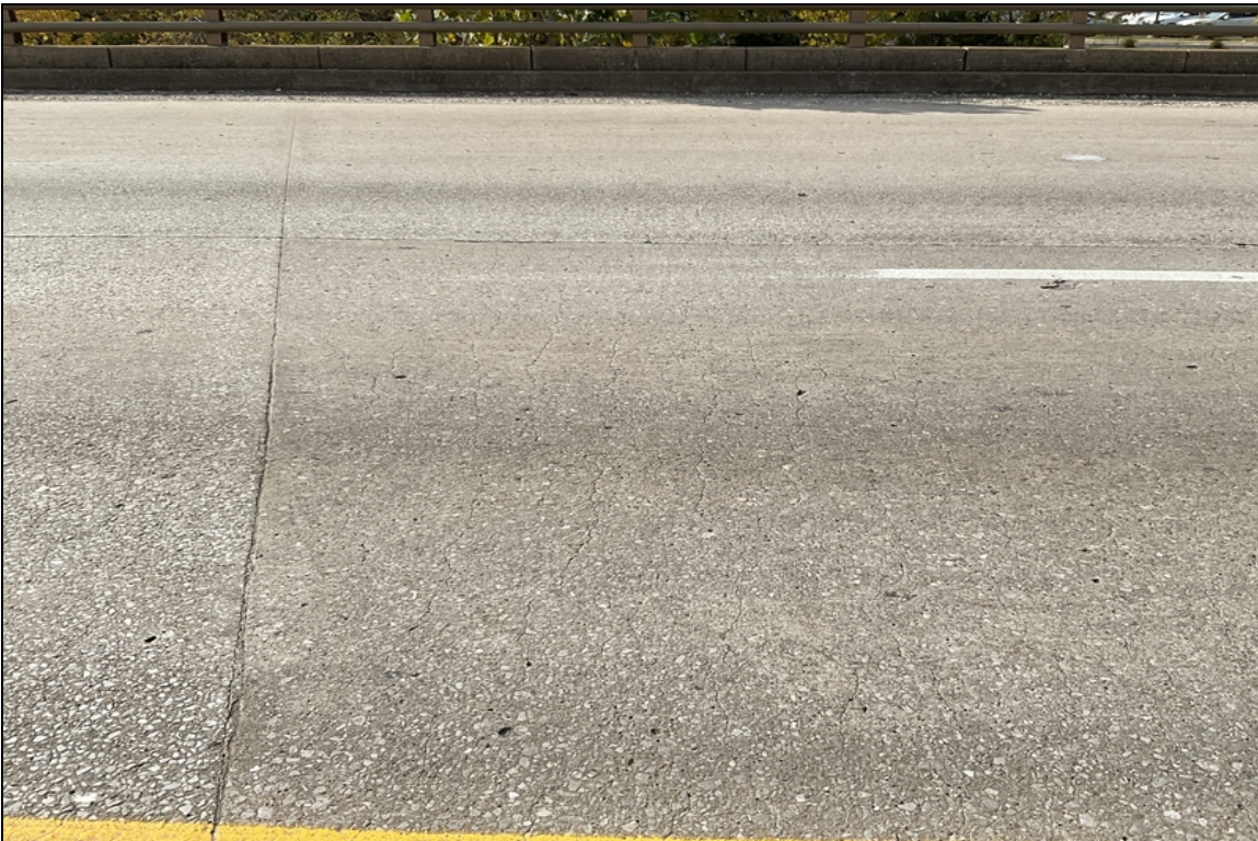
Span 2-Mapcracking.
