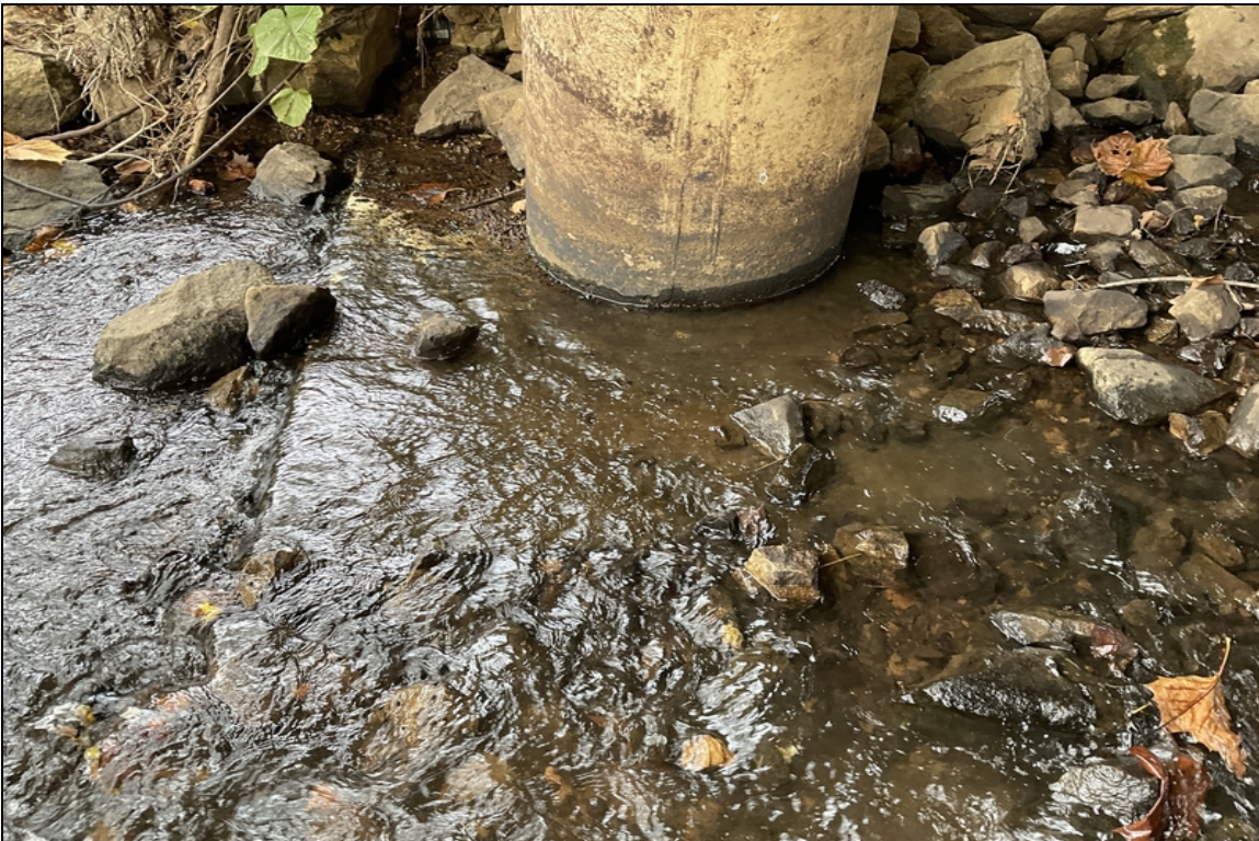
Bent 3, column 1 footing exposed.
