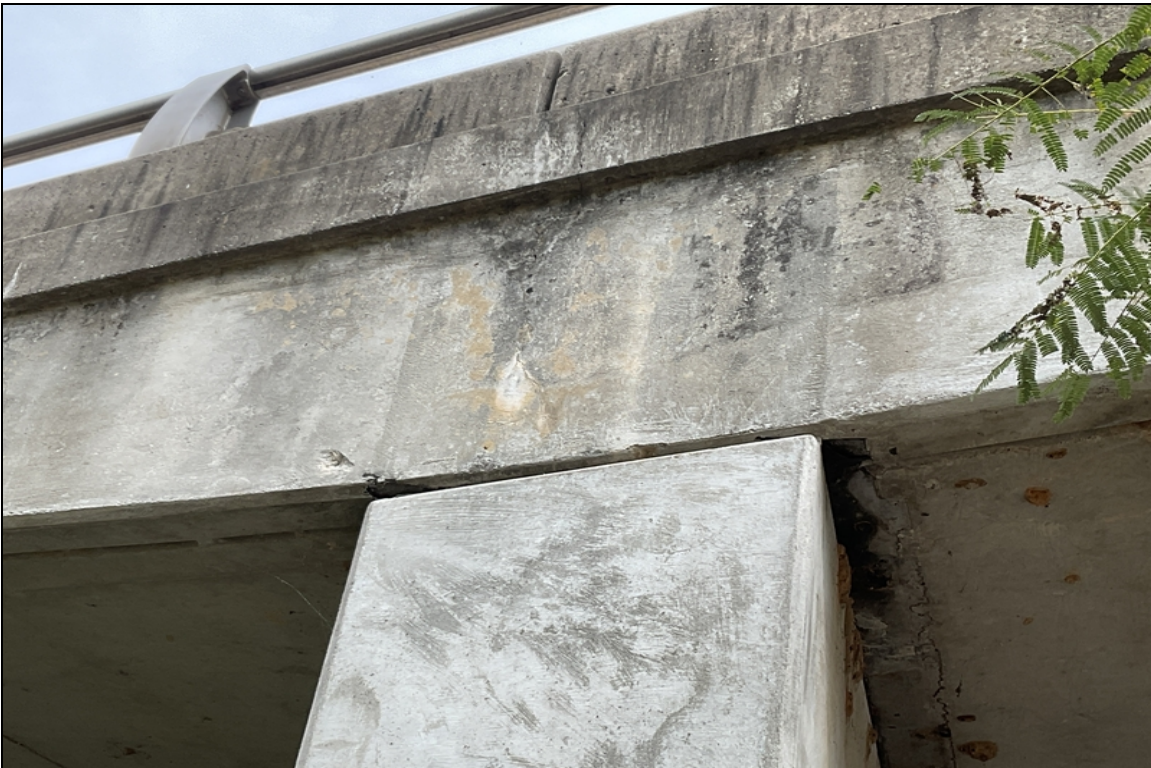
Vertical crack with light efflorescence on exterior side of slab over bent # 2.
