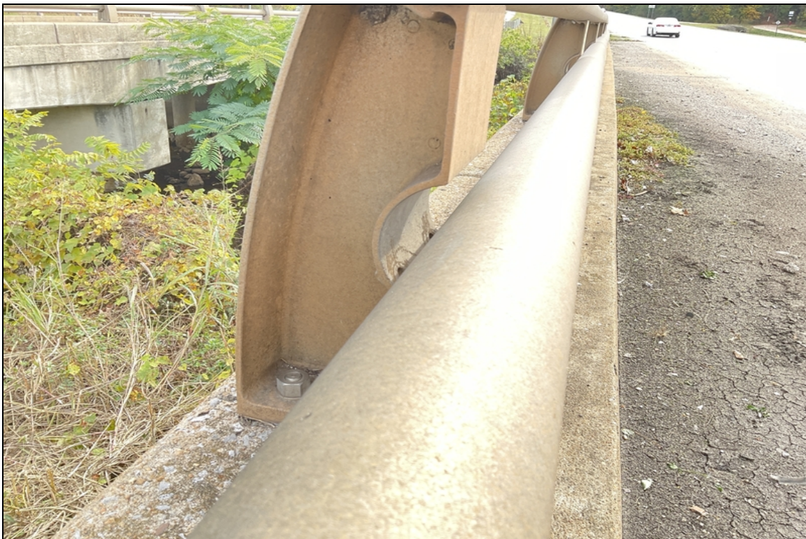
Span 3, right side-Missing bolt at post connection.
