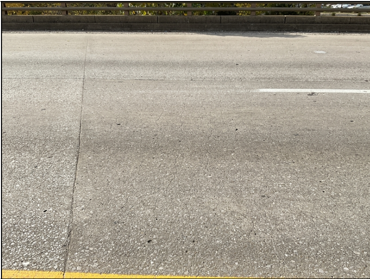
Span 2-Mapcracking.
