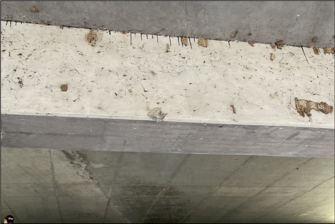
Bent 2 cap-Shallow spall in backface right of centerline.
