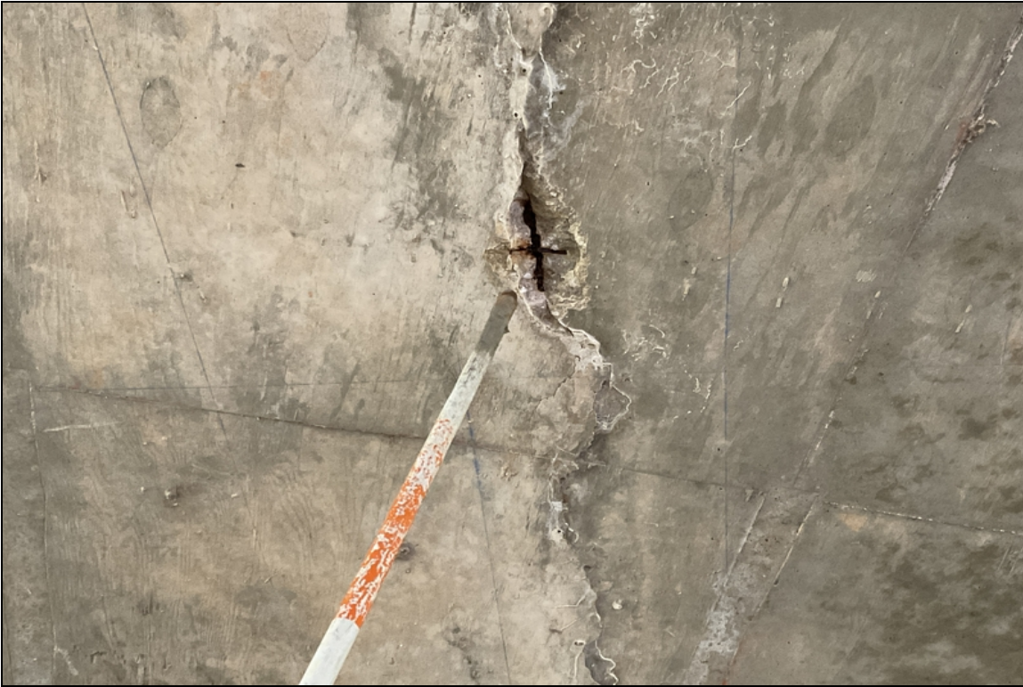
Span # 3-Spall with exposed reinforcing steel in slab undersurface in centerline construction joint.
