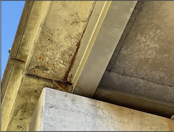
Span # 3, beam # 7 over bent # 4-Corrosion to top flange.
