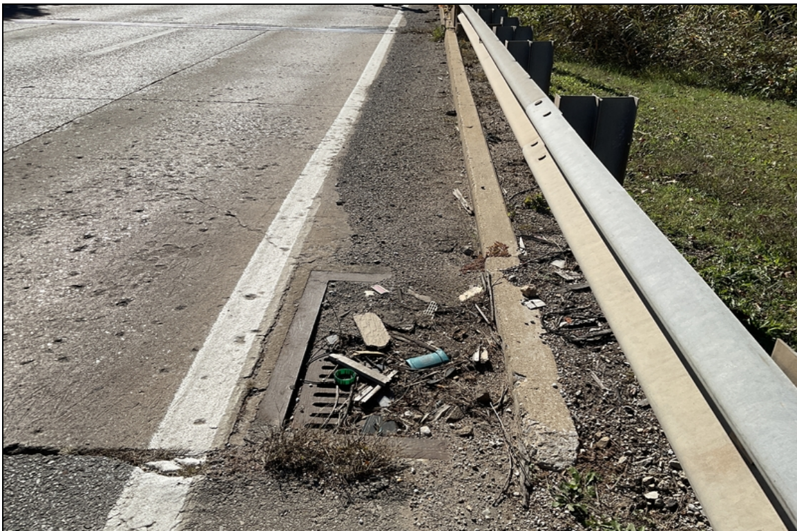
The North approach gutter has heavy dirt and debris accumulation that restricts drop inlet.
