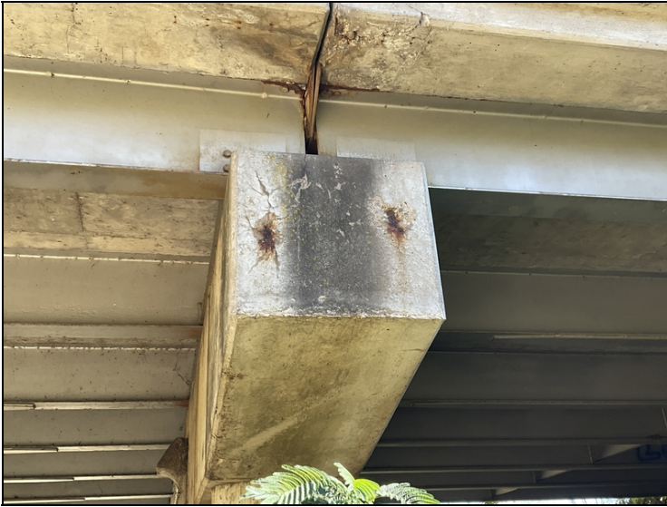
Bent 2 cap, left end-Spalls with exposed reinforcing steel.
