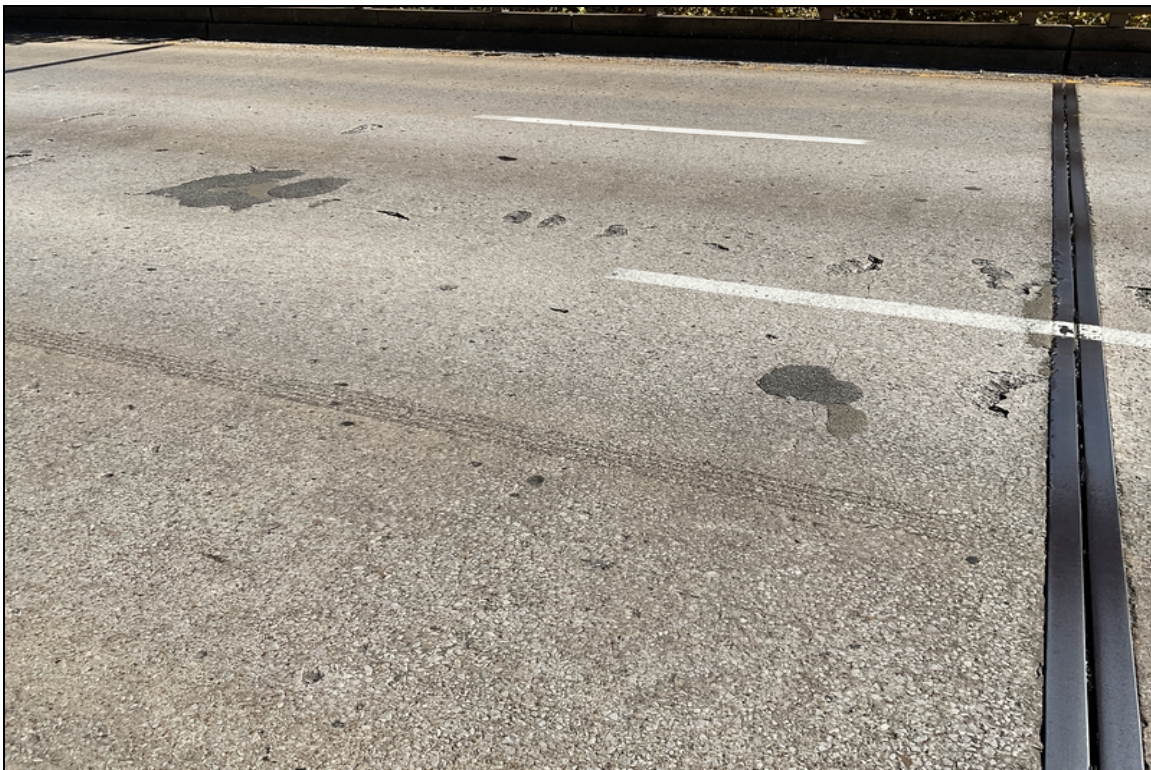
Span 3-Spalls in driving surface.
