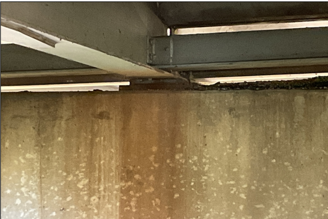
Span 1, bearing 2 over bent 2-Fretting with noise under live load.
