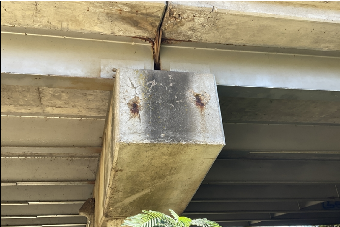
Bent 2 cap, left end-Spalls with exposed reinforcing steel.
