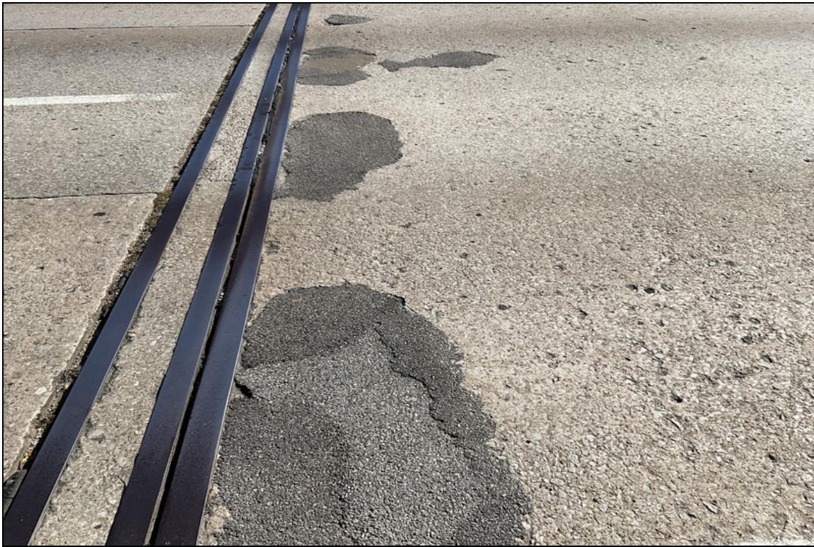
Span 4-Spalls at abutment 2.
