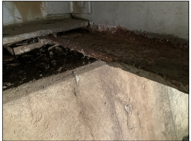
Beam # 3 at abutment # 2-Corrosion to beam end.
