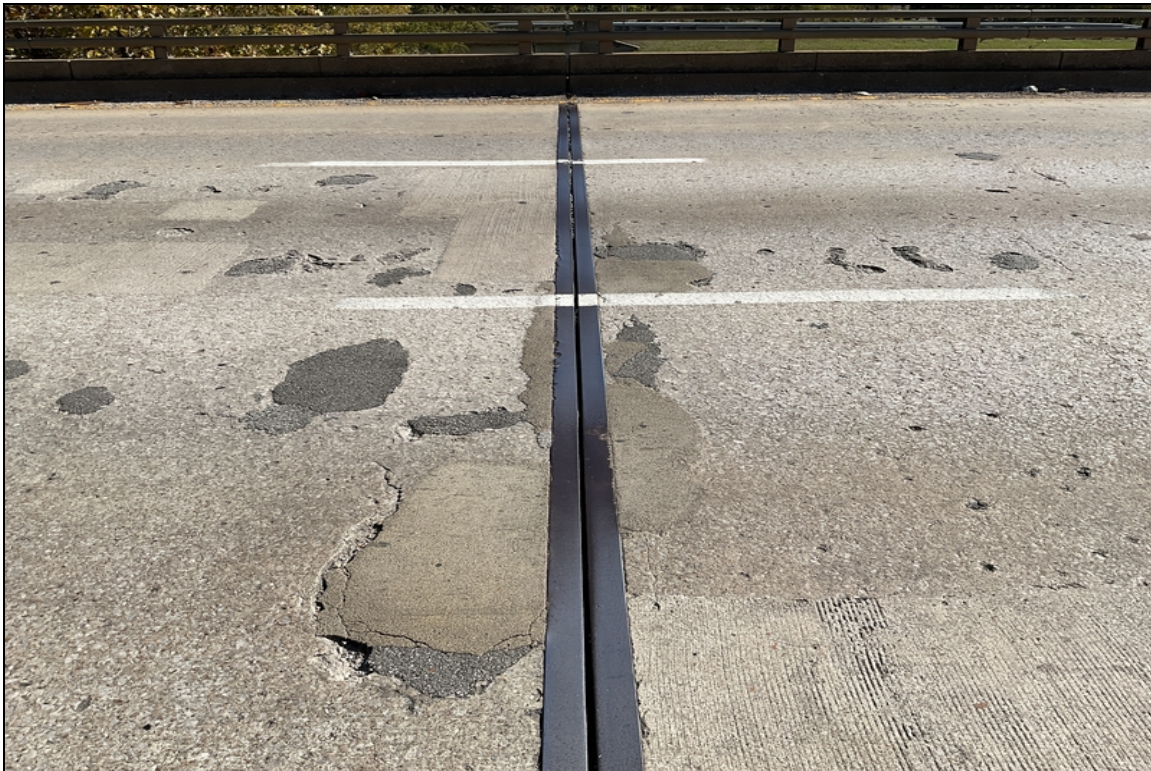
Spans 1 and 2 at bent 2-Spalls and delaminated areas.
