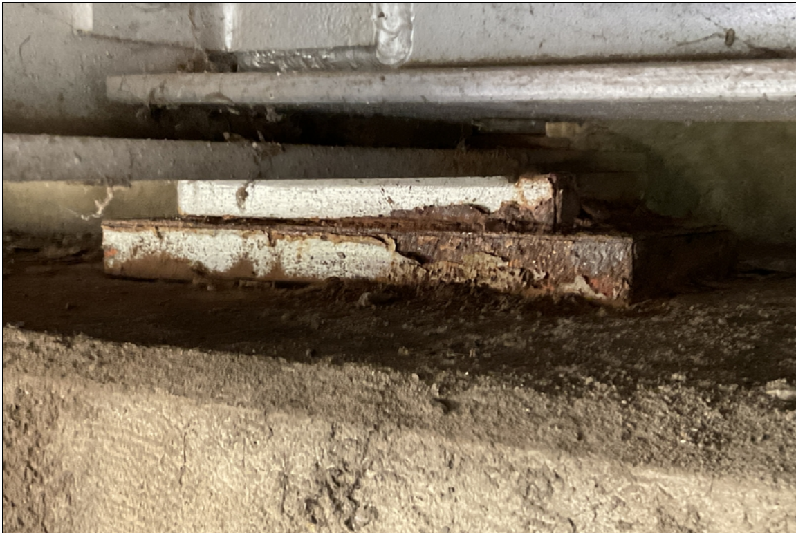
Span 1, bearing 4 at abutment 1-Corrosion.
