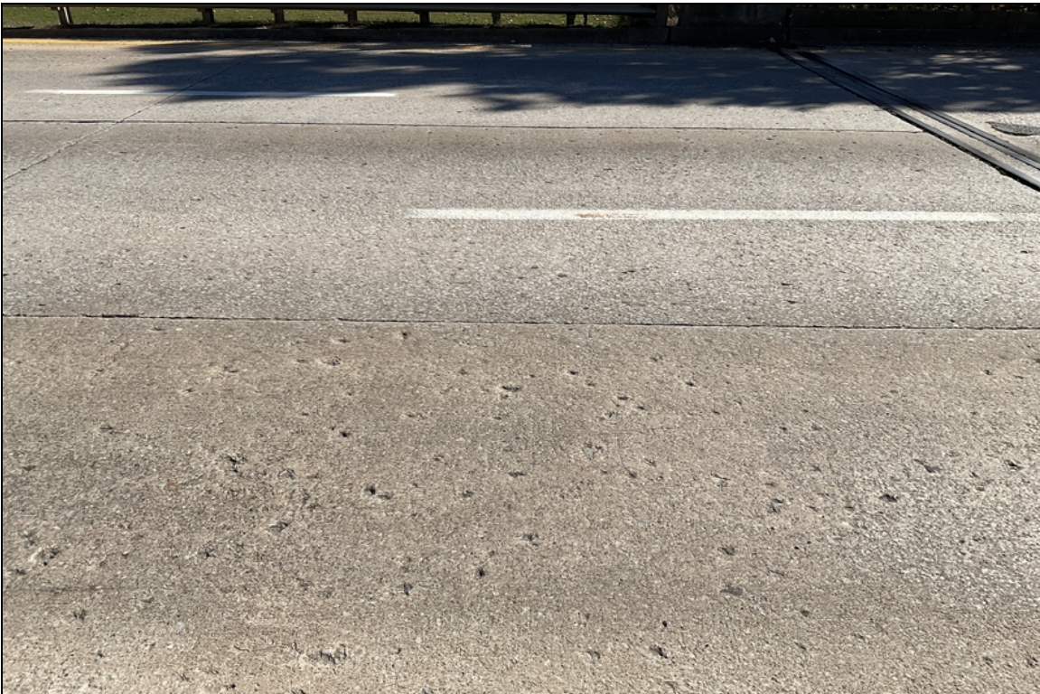
North approach slab-Light abrasion with numerous pop outs.
