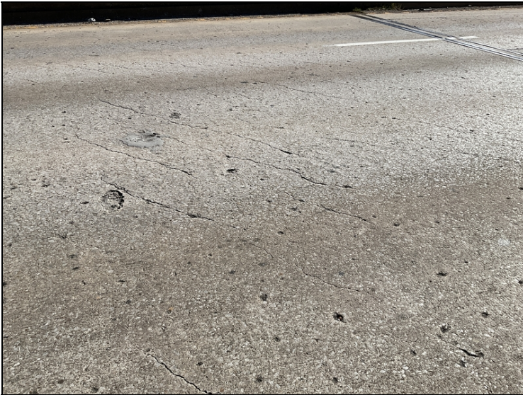
Span # 1 numerous moderate width diagonal cracks.
