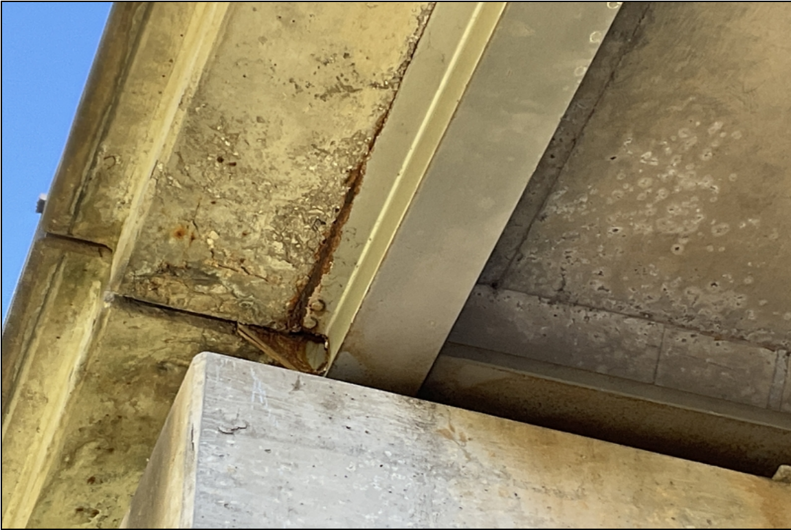
Span 3, beam 7 over bent 4-Corrosion to top flange.
