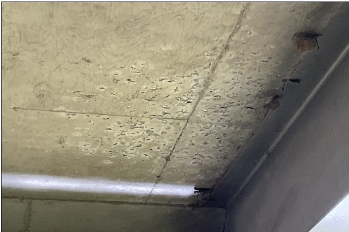
Span #4 bay #1 scaling to the undersurface
