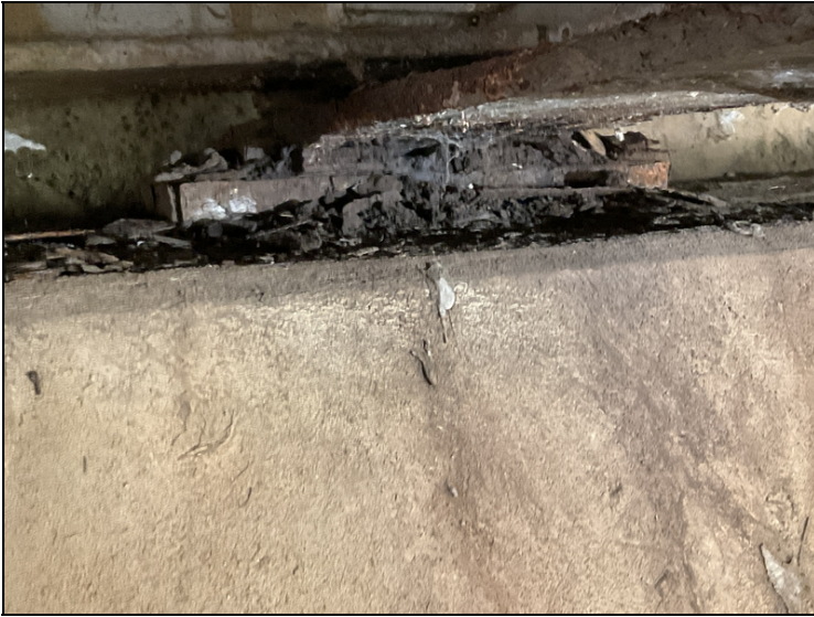
Abutment # 2 bearing # 3-Corrosion.
