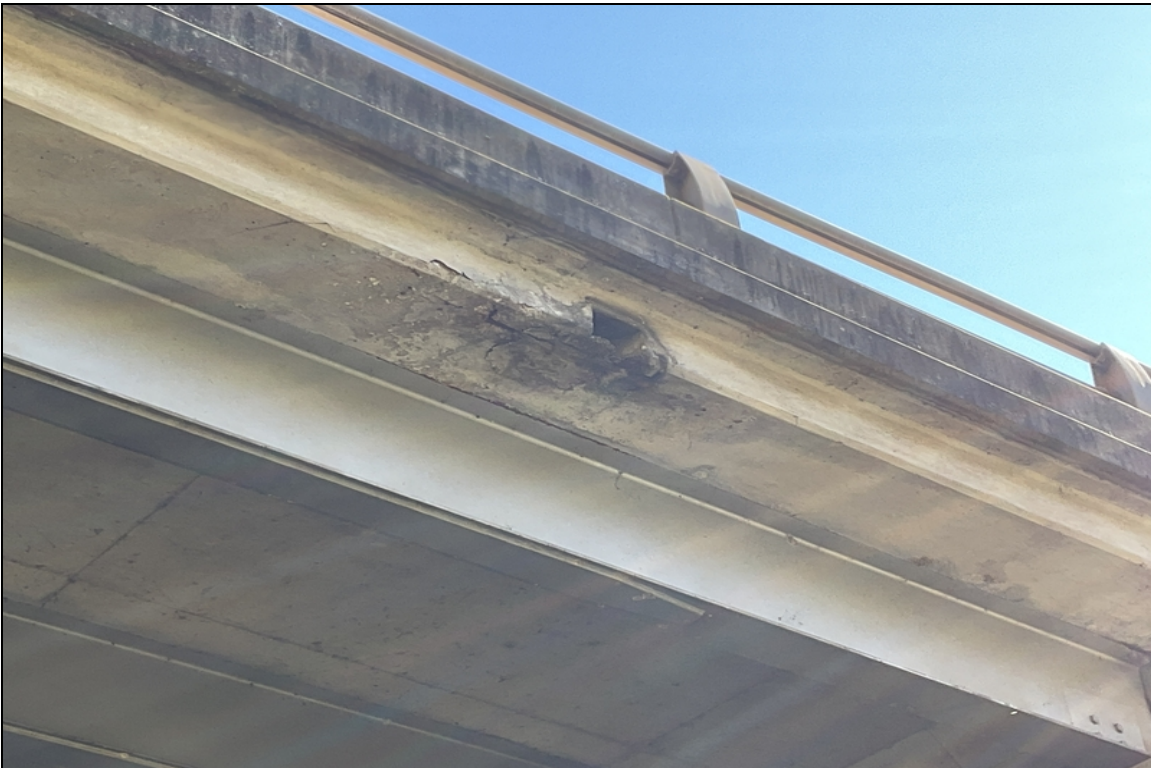
Span 3, left side-Spall / delaminated area adjacent to deck drain.
