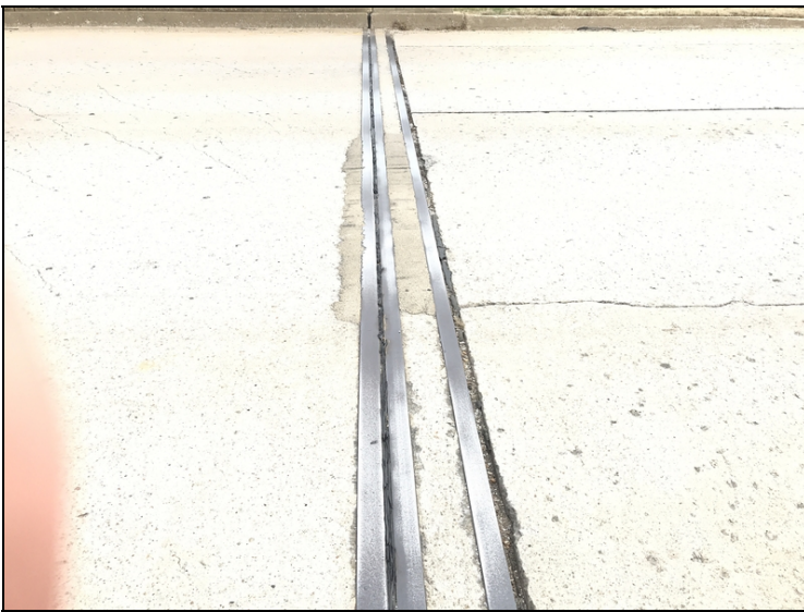
Abutment # 1 expansion joint.
