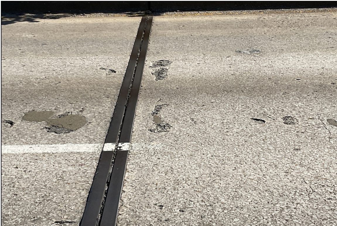
Span # 3 has spalls and delaminated areas adjacent to bent # 4 expansion joint assembly.
