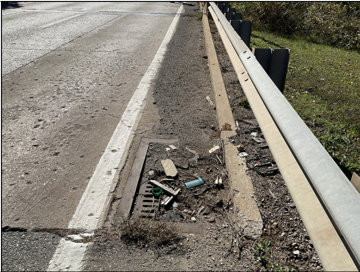
The North approach gutter has heavy dirt and debris accumulation that restricts drop inlet.
