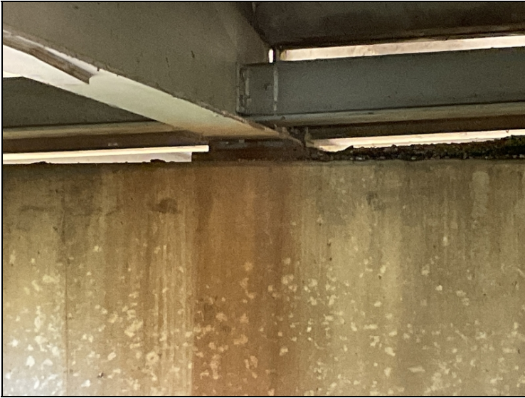
Span # 1, bearing 2 over bent # 2-Fretting with noise under live load.
