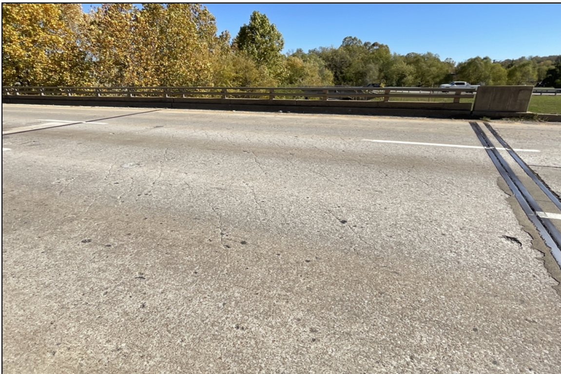
Span # 1 driving surface has numerous moderate width diagonal cracks.
