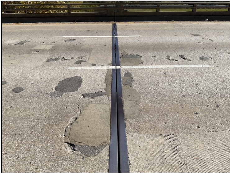
Spans 1 and 2 at bent 2-Spalls and delaminated areas.
