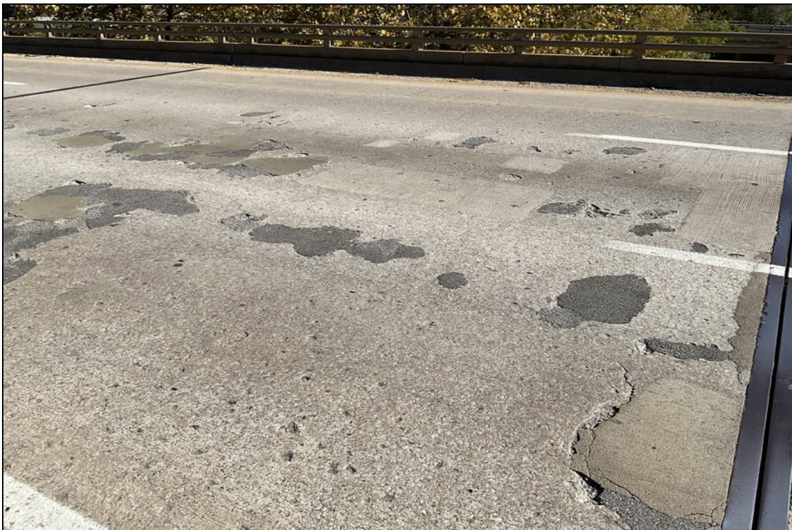
Span 2-Spalls with failing repairs.
