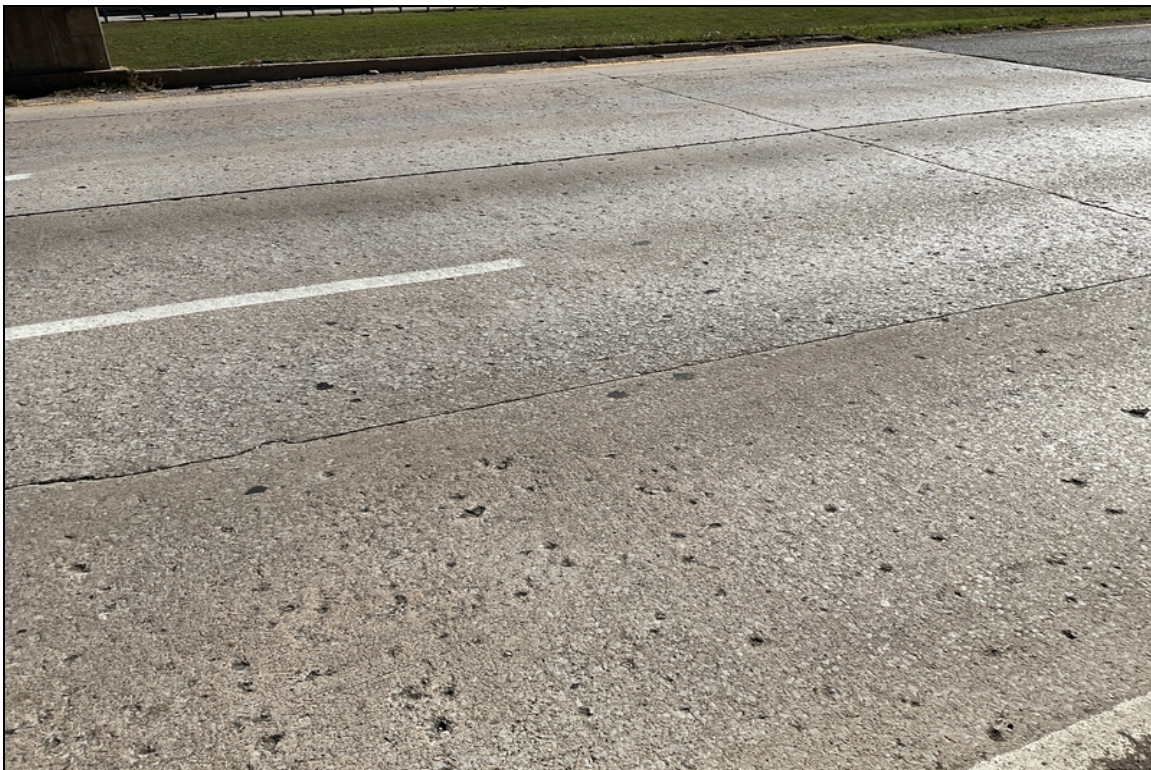
South approach slab-Abrasion with numerous pop outs.
