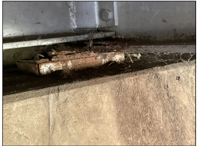
Abutment # 2 bearing #5-Corrosion.
