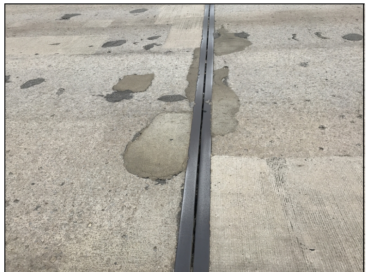
Compression joint seals are torn, deteriorated, and leak water on the substructure caps, bearings, and ends of the beams.
