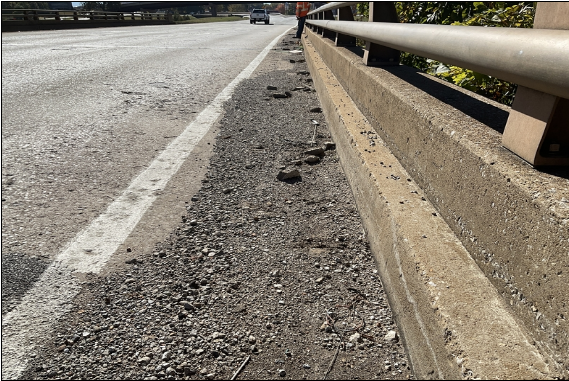
Heavy dirt and debris in gutters.
