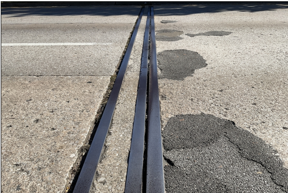
Abutment 1 expansion joint-Seal deteriorated.
