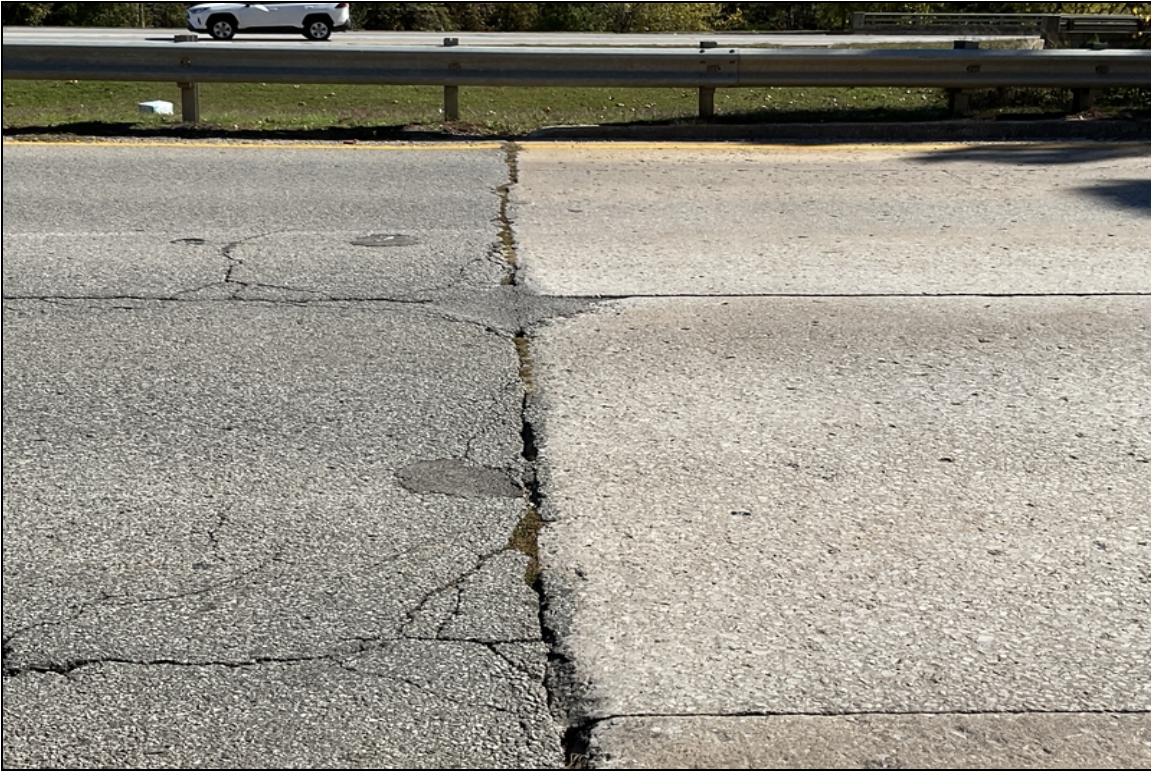
North approach slab-Spall at roadway juncture.
