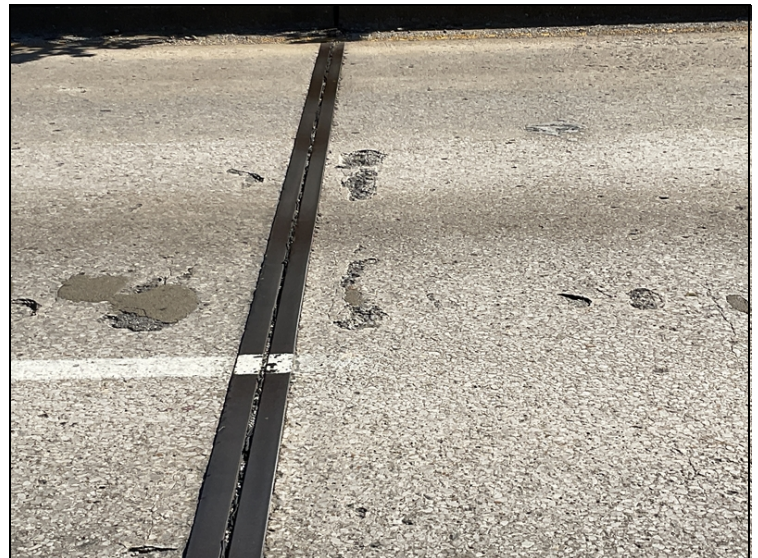
Span # 3 has spalls and delaminated areas adjacent to bent # 4 expansion joint assembly.
