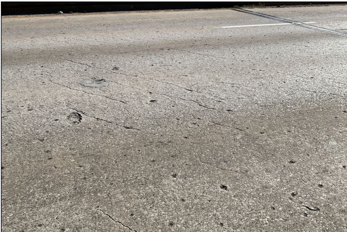
Span 1 diagonal cracks.
