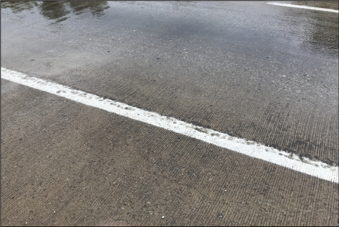
Typical map cracking
