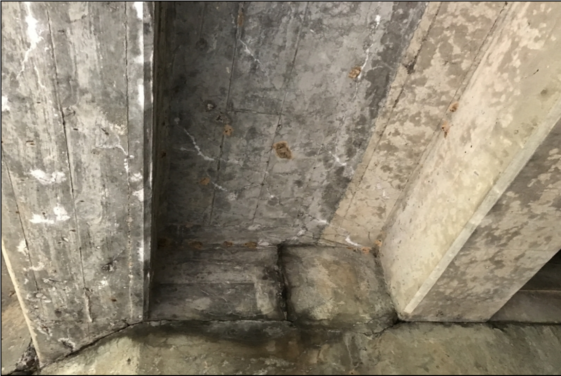
Bay 5 cracking with efflorescence
