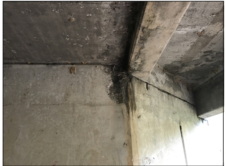
Bent 1 spalling with exposed reinforcing steel adjacent to girder 2 and slab unit
