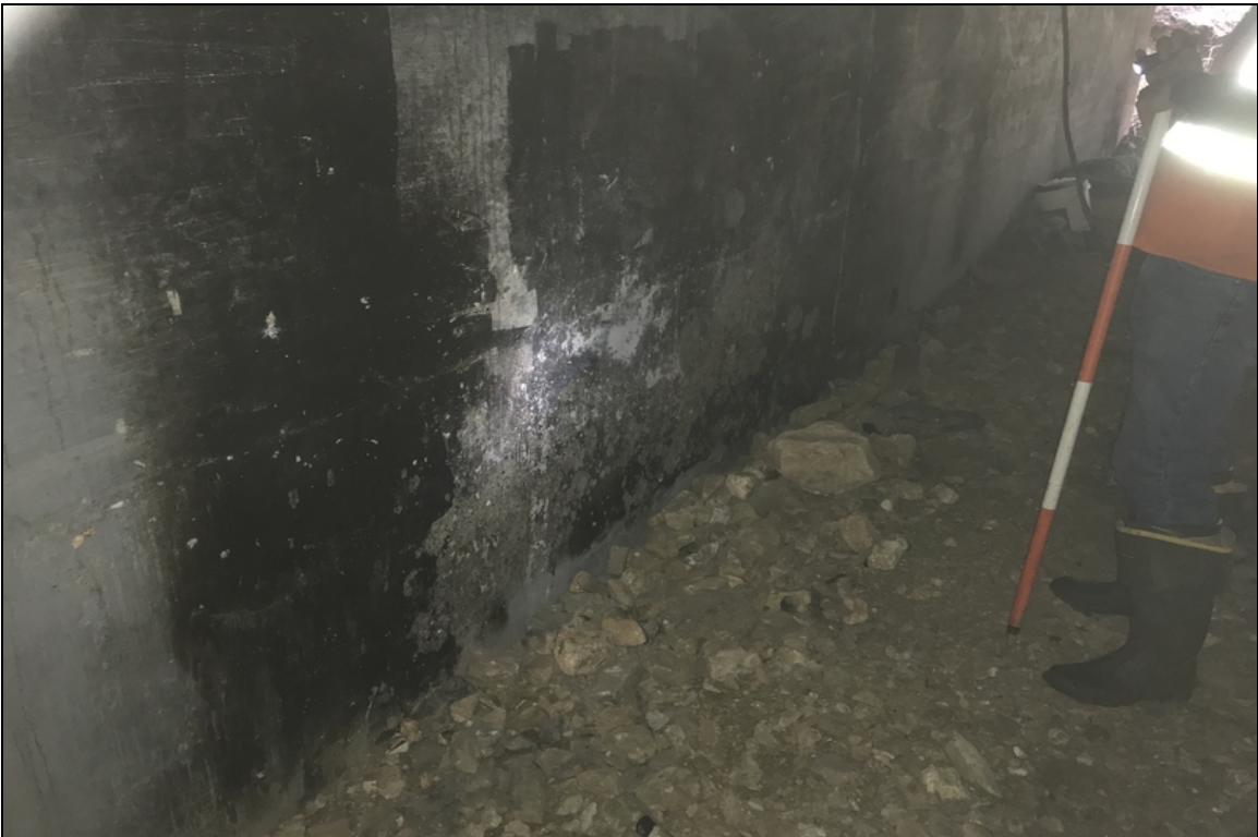
Bent 2 shallow spalling
