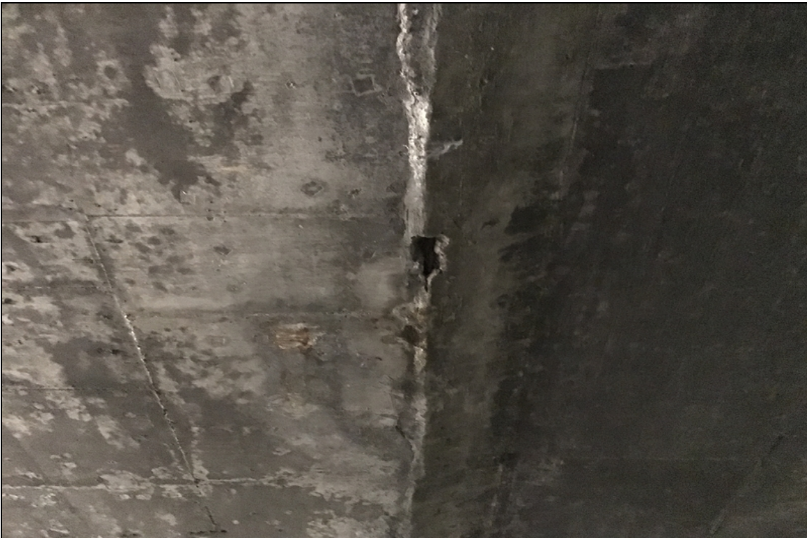
Slab span construction joint cracking with efflorescence and spalling with exposed reinforcing steel
