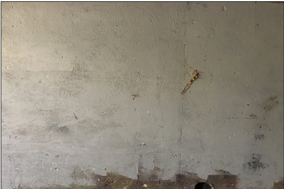
Bent 1 vertical cracking
