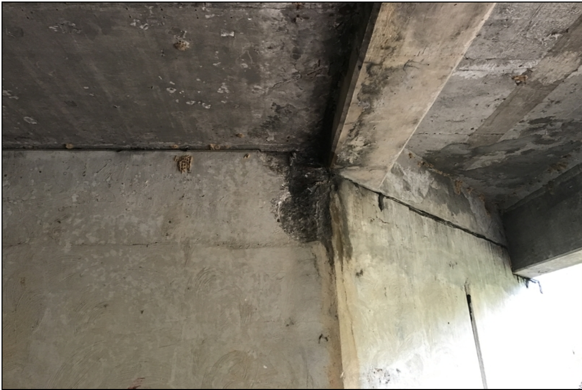
Bent 1 spalling with exposed reinforcing steel adjacent to girder 2 and slab unit
