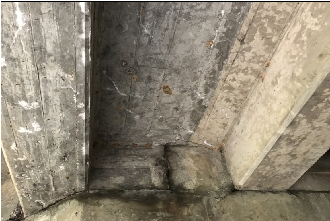
Bay 5 cracking with efflorescence
