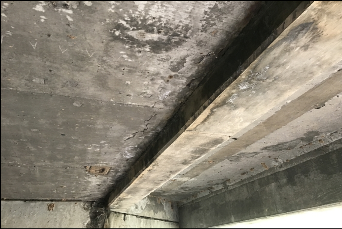
Slab unit adjacent to girder 2 delam
