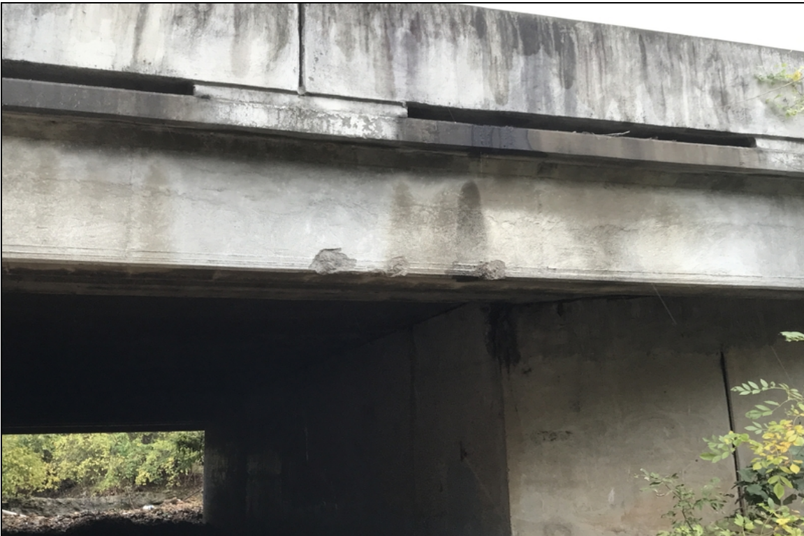
Outside girder 1 spalling
