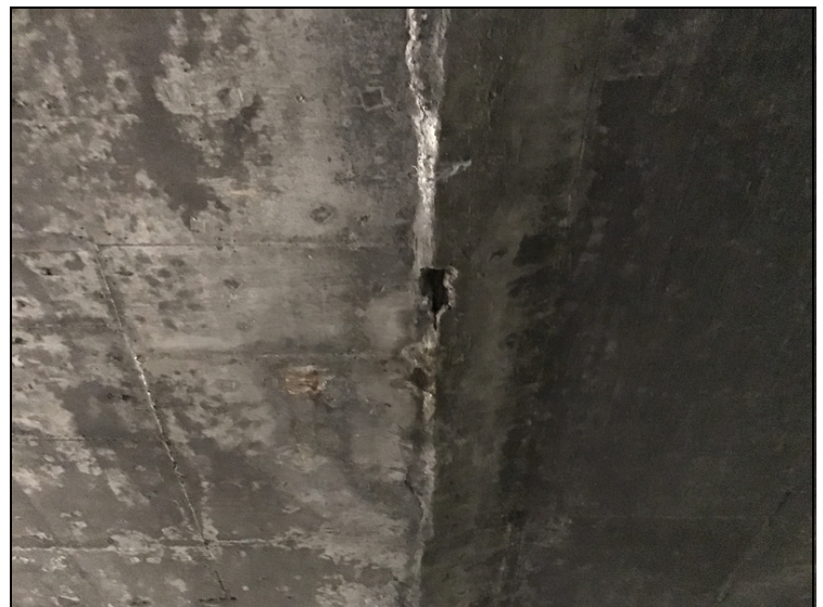
Slab span construction joint cracking with efflorescence and spalling with exposed reinforcing steel
