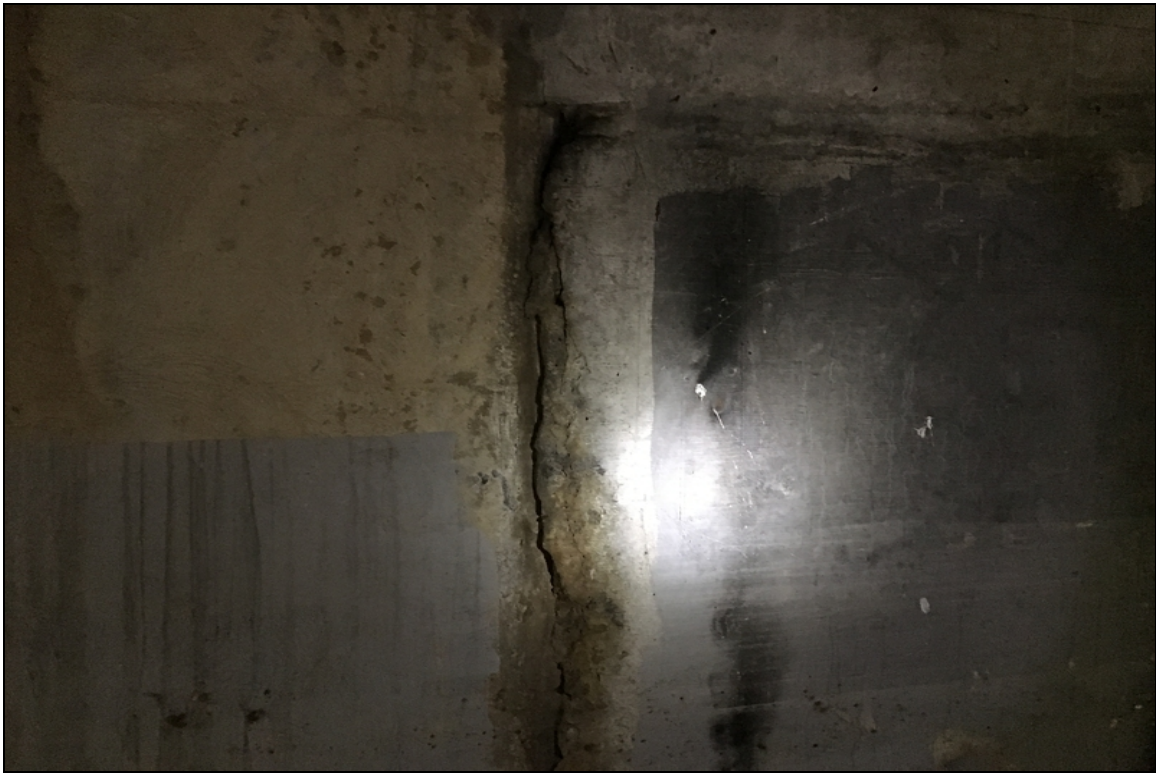
Bent 2 vertical cracking at construction joint
