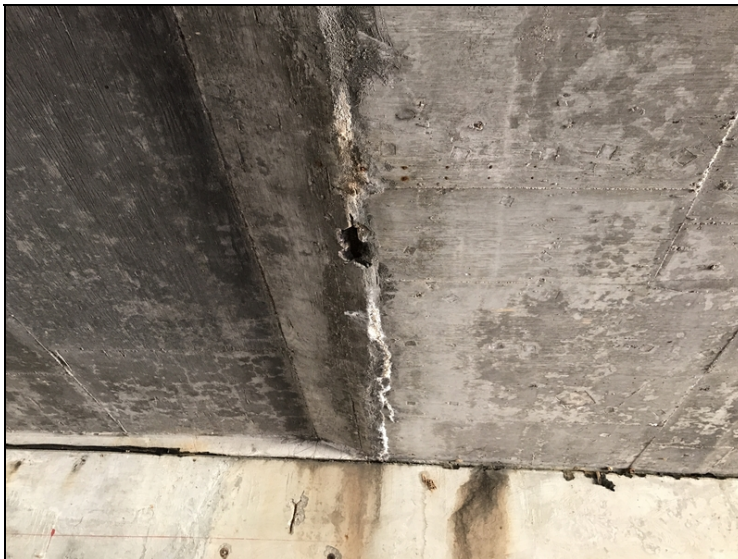
Slab soffit construction joint with exposed reinforcing steel.
