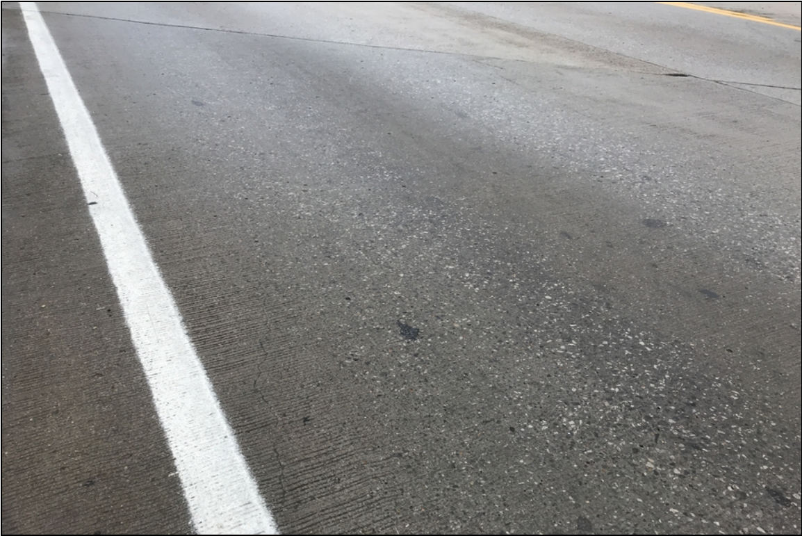
Abrasion in wheel paths typical
