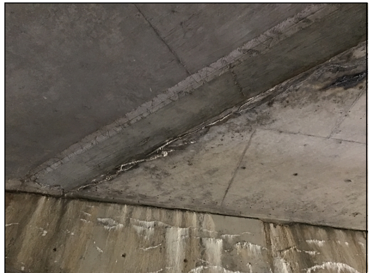
Span 2 slab construction joint cracking with efflorescence
