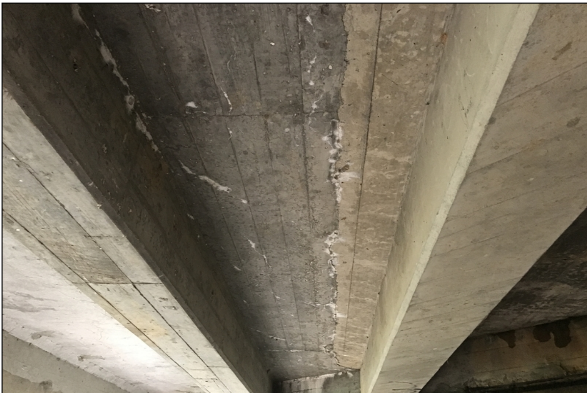
Span 3 under surface cracking with efflorescence
