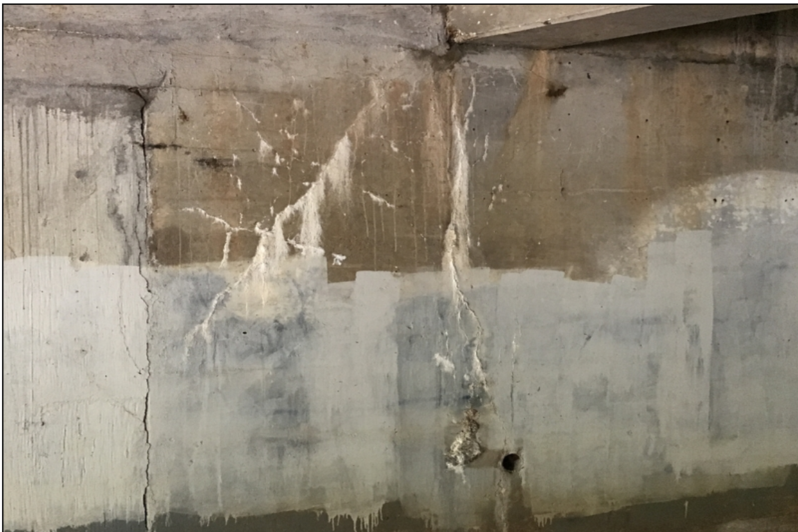
Bent 4 cracking with efflorescence
