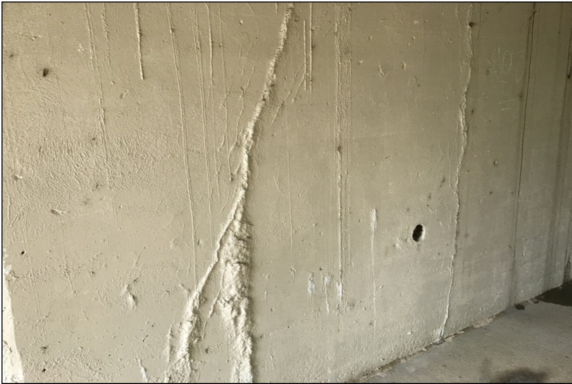
Bent 1 cracking with efflorescence
