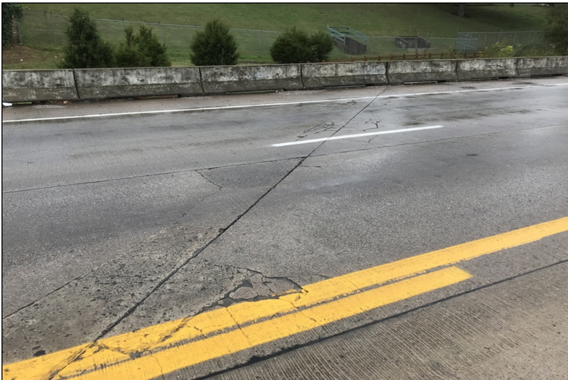
Span 2 spalling in wheel path
