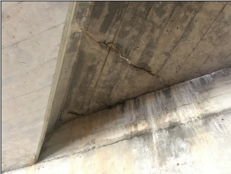
Deck Soffit - Span # 3. Bay # 2. Spalls with exposed reinforcing steel adjacent to Bent # 4.
