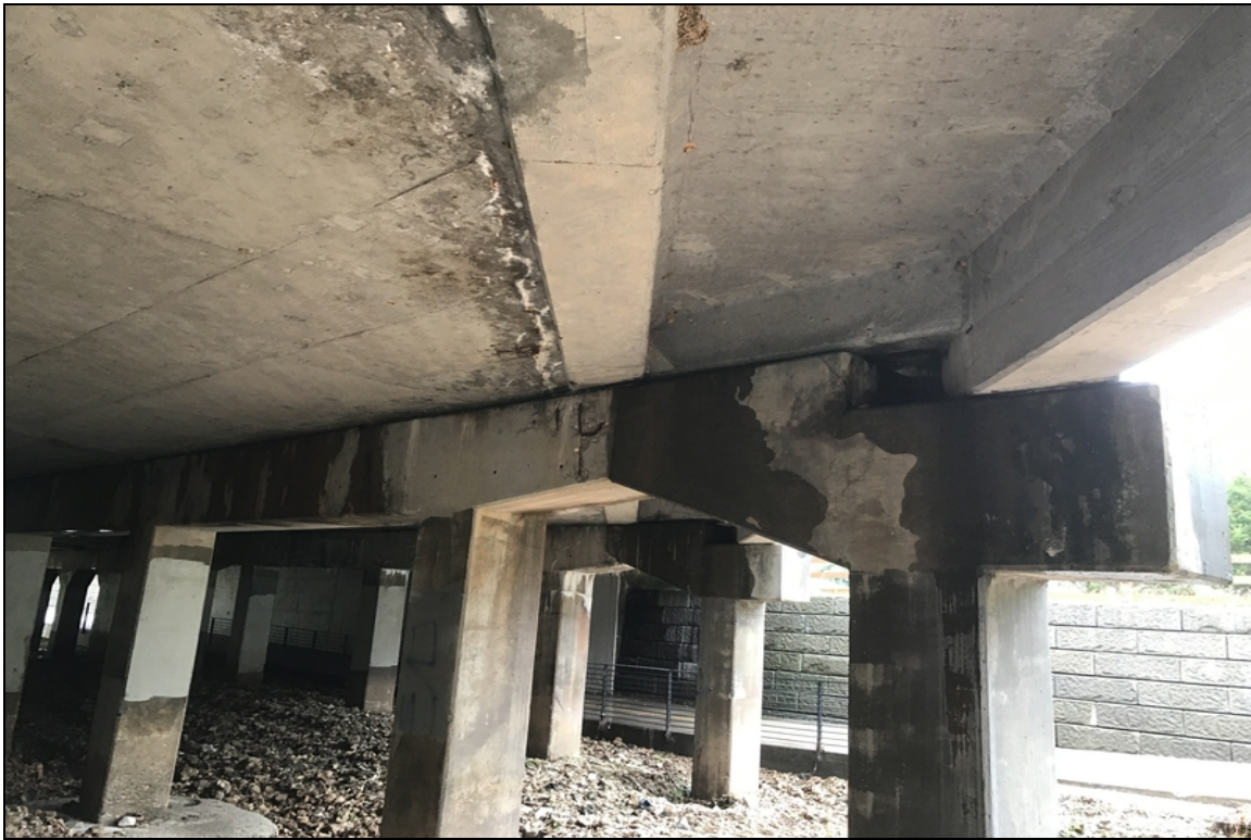
Bent 3 spalling with exposed reinforcing steel (both sides)
