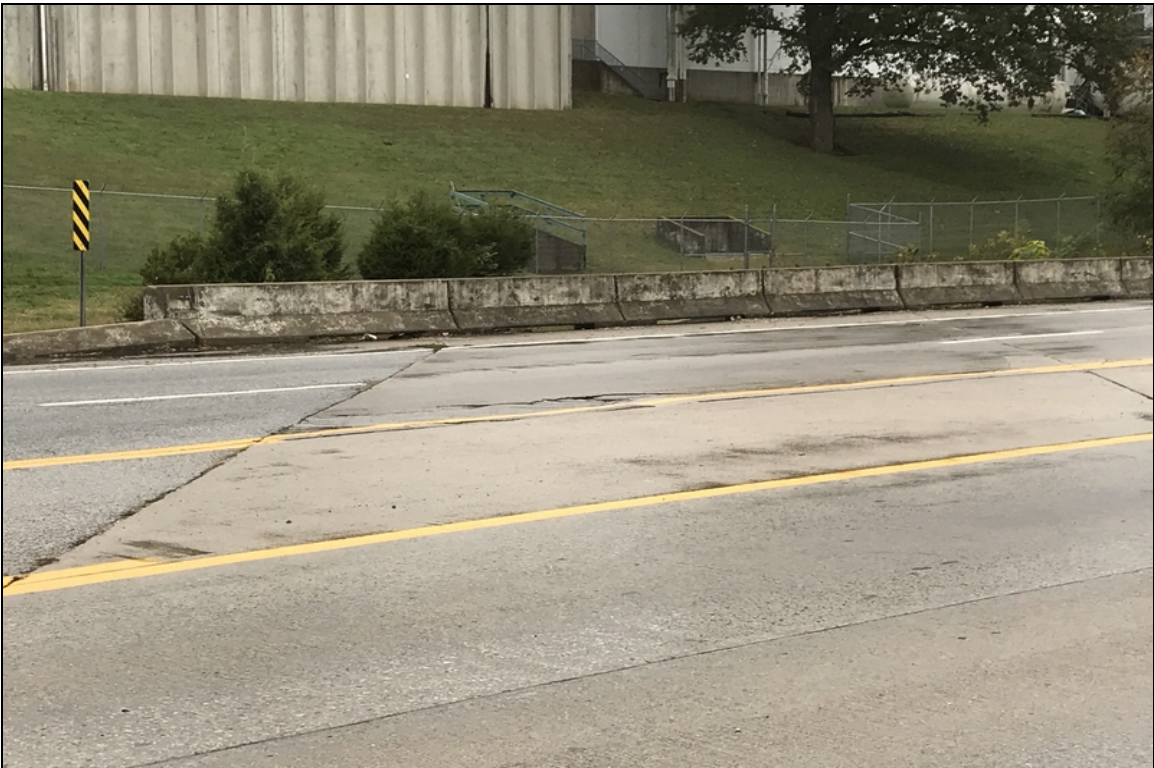
Span 1 spalling on inside southbound lane in wheel path
