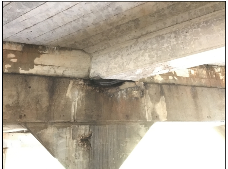
Bent 2 spalling at bearing area adj to girder 4 (Bk)
