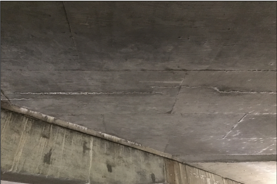
Span 2 slab cracking with efflorescence
