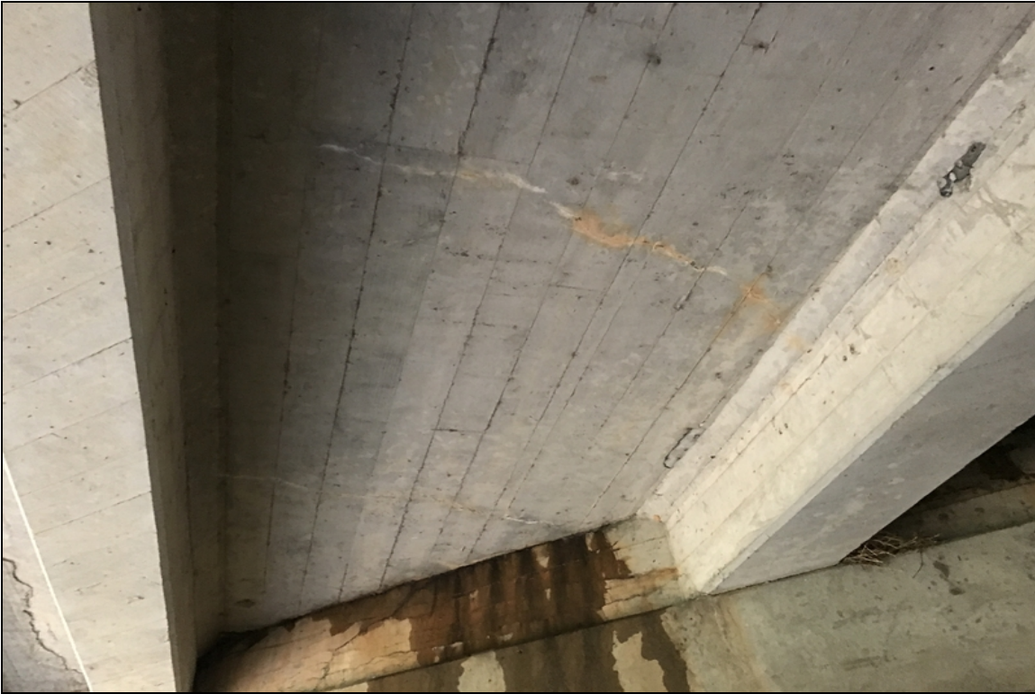
Span 2 under surface cracking with efflorescence
