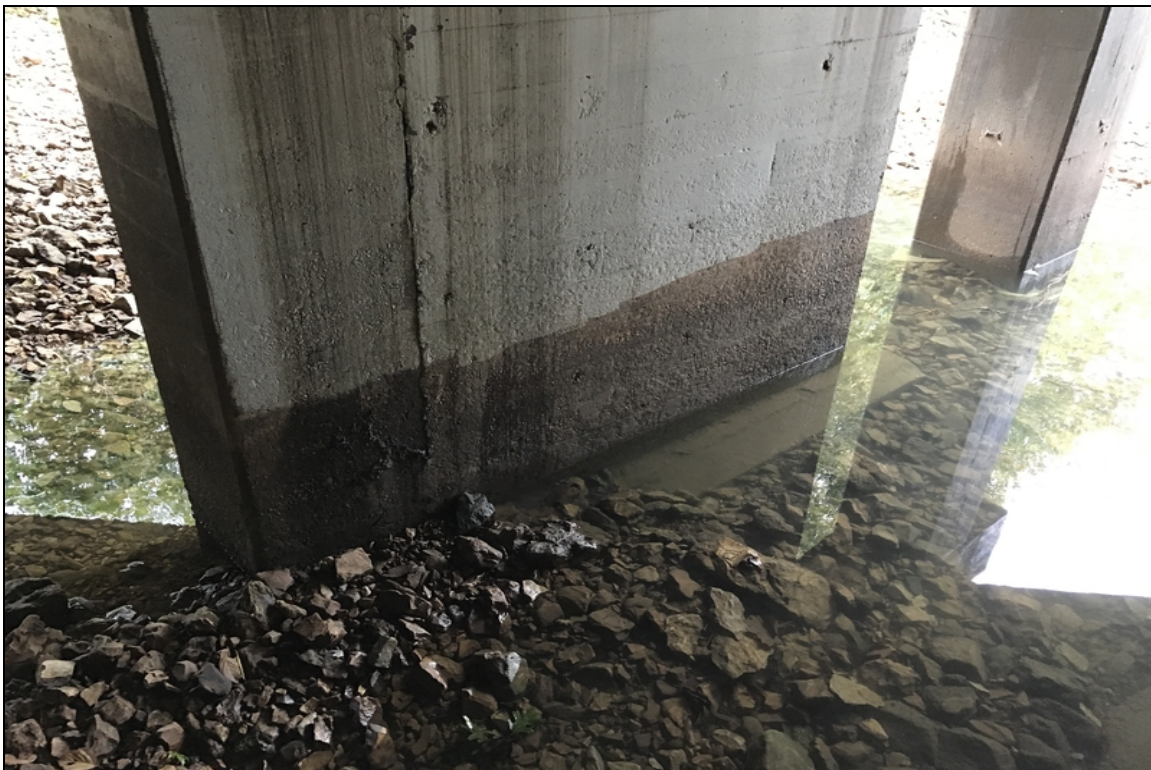
Bent 2 pier wall abrasion
