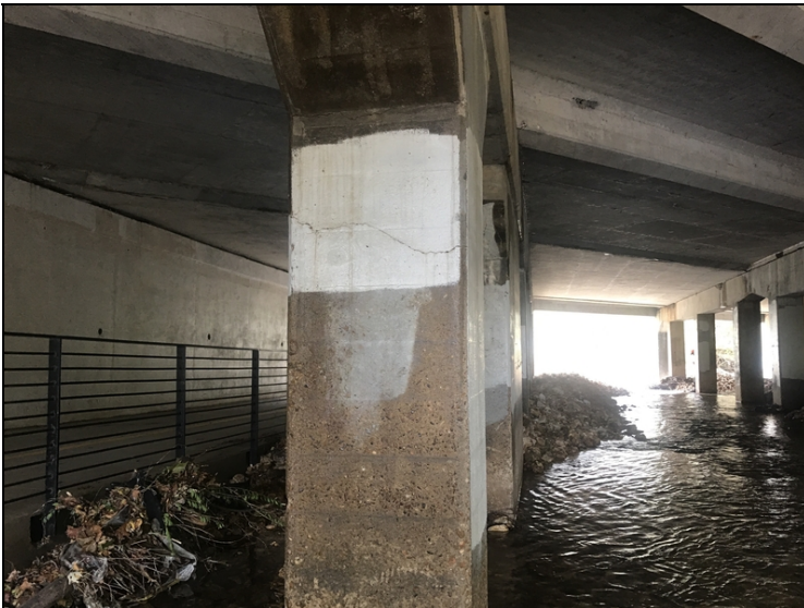
Crack column # 7. Bent # 2.
