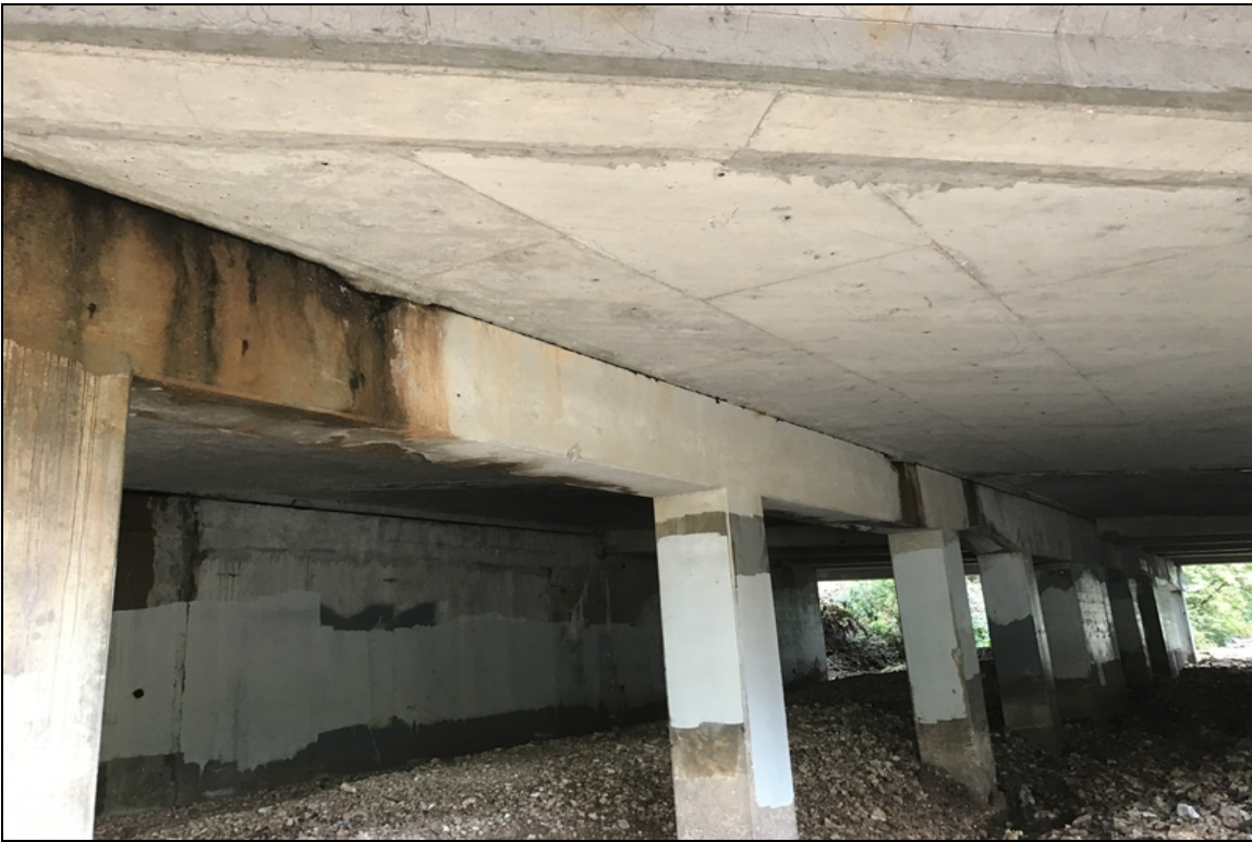
Bent 3 has 2 spalls (bk)
