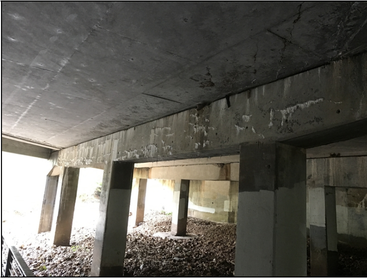
Bent 2 cap cracking with efflorescence (Both sides)
