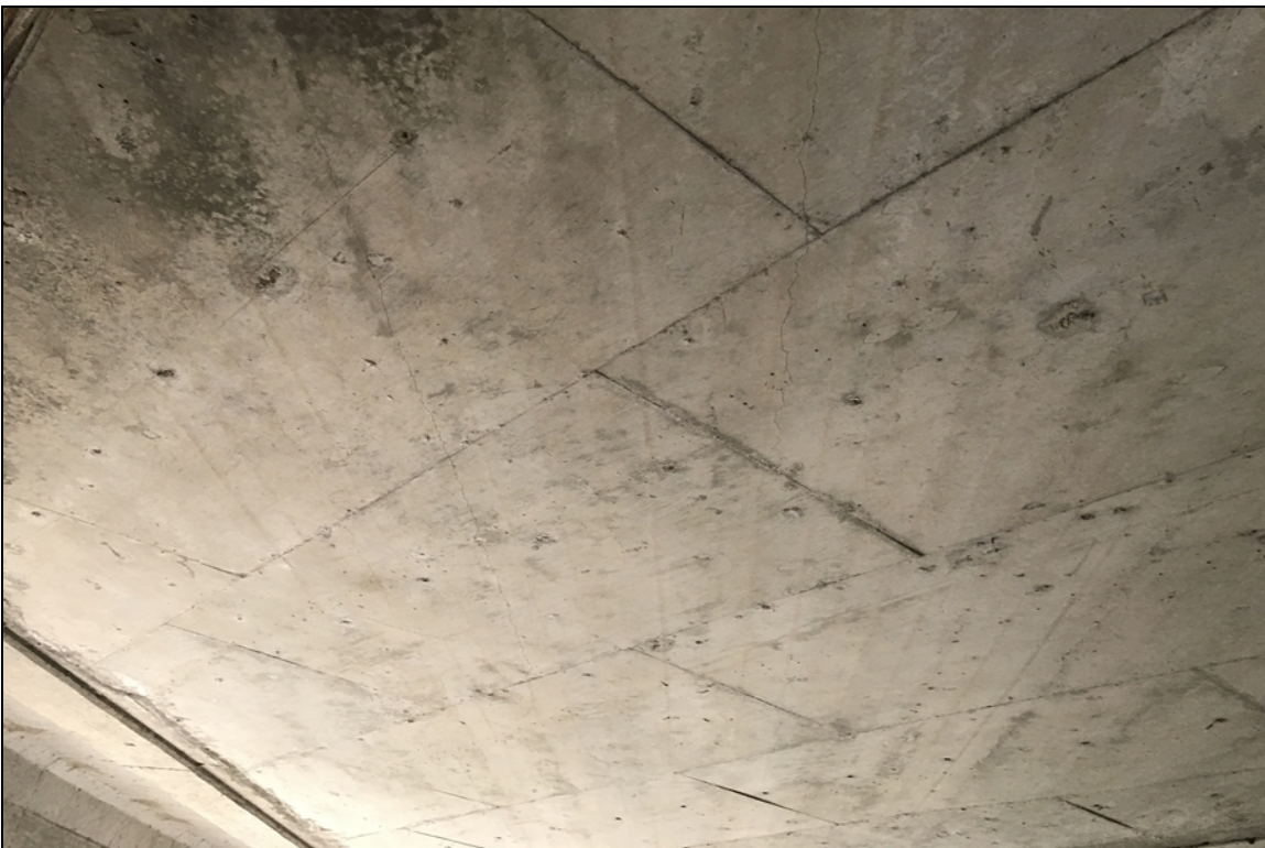
Span 2 longitudinal cracking
