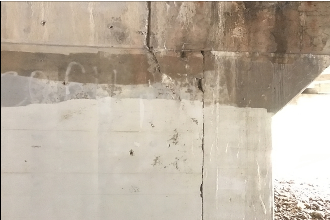
Bent 2 pier wall cracking with efflorescence
