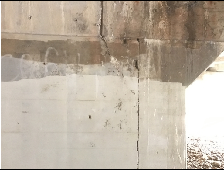
Bent 2 pier wall cracking with efflorescence
