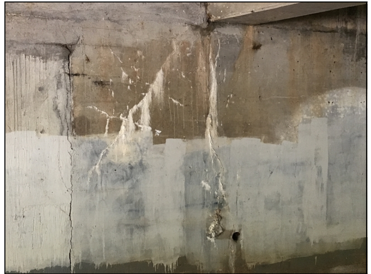
Bent 4 cracking with efflorescence
