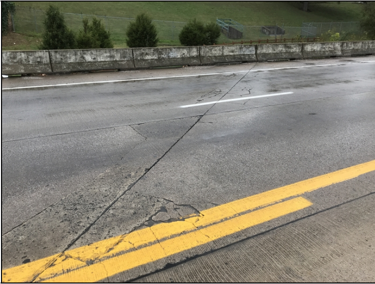
Span 2 spalling in wheel path
