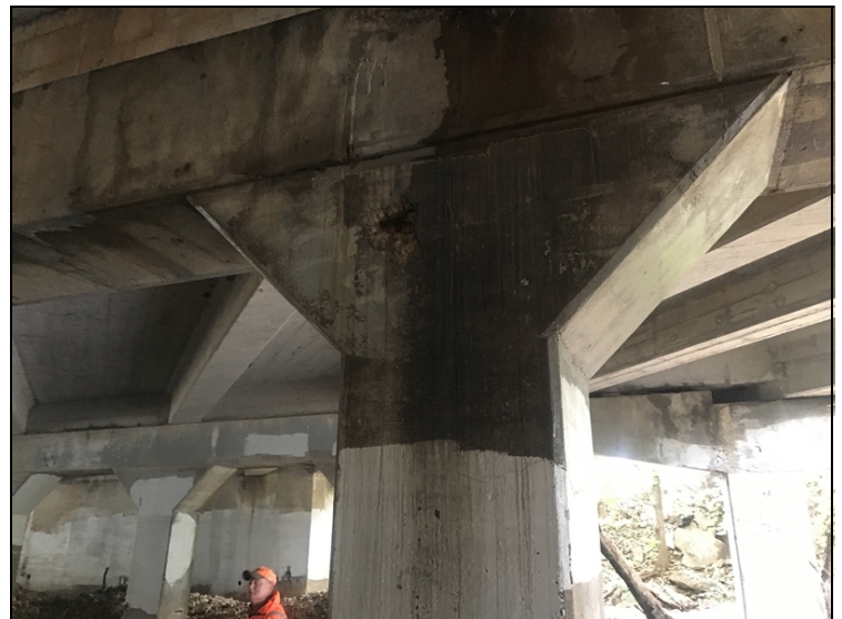
Spall with exposed reinforcing steel. Bent # 2. Column # 7.
