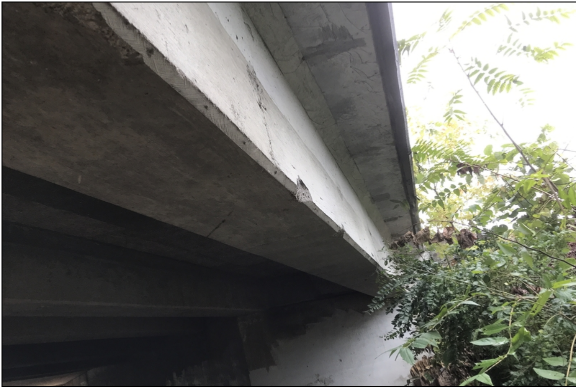
Span 3 girder 7 spall
