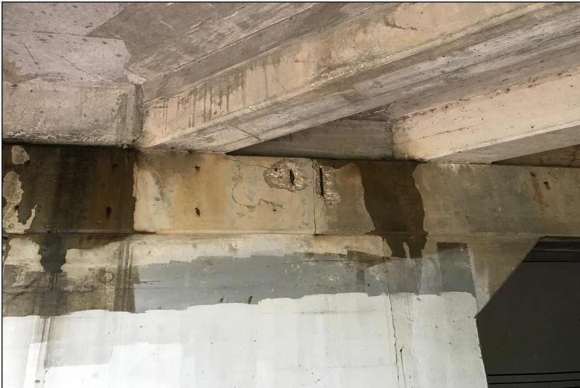
Bent 2 cap (ahd) spalling with exposed reinforcing steel
