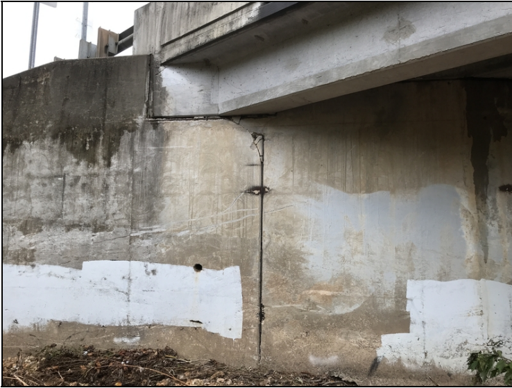
Bent 4 spalling with exposed reinforcing steel at construction joint
