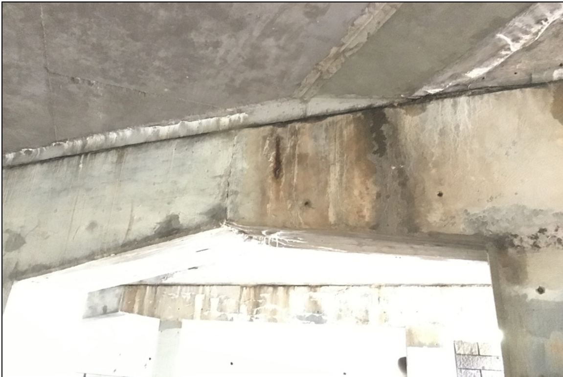
Bent 3 spalling with exposed reinforcing steel
