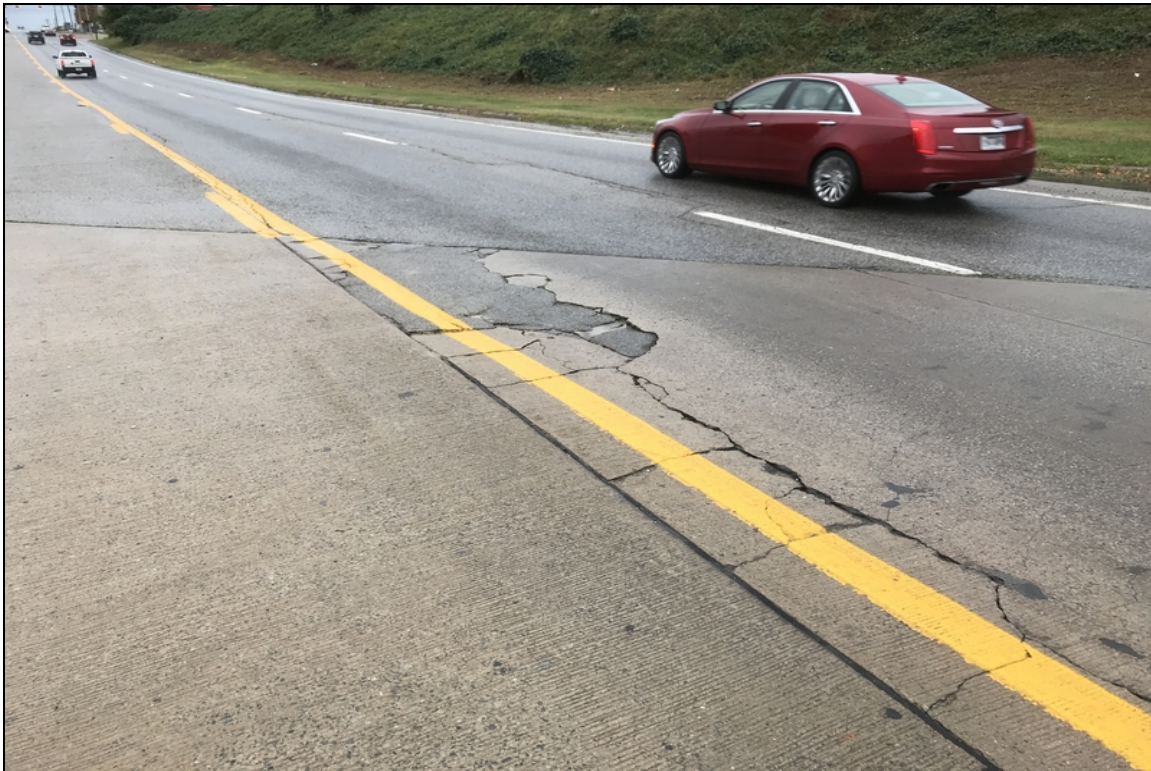
Span 1 spalling in wheel path
