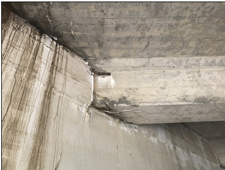
Girder # 3 adjacent to Bent # 1. Map cracking with efflorescence. Spall with exposed reinforcing steel.
