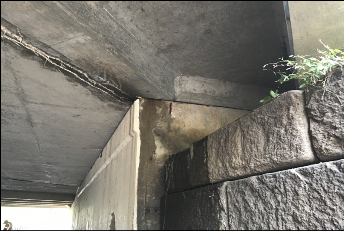
Bent 1 adjacent to girder 2 spalling with exposed reinforcing steel
