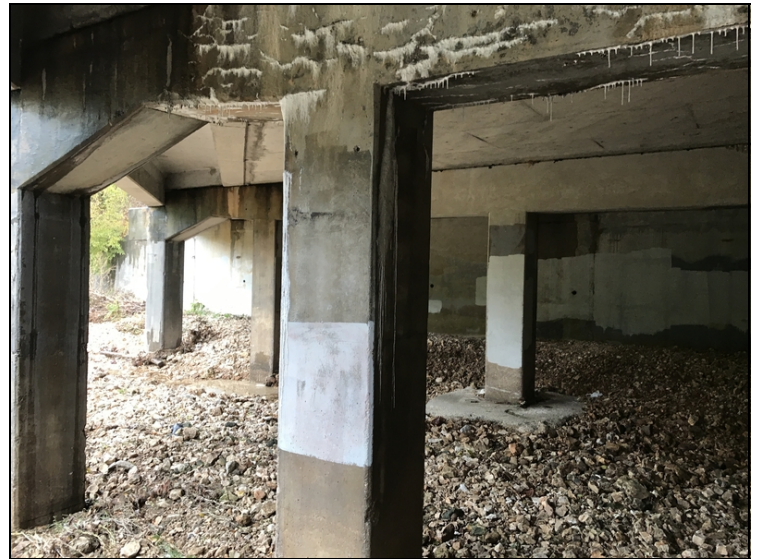
Bent 2 columns 2 & 3 cracking with efflorescence
