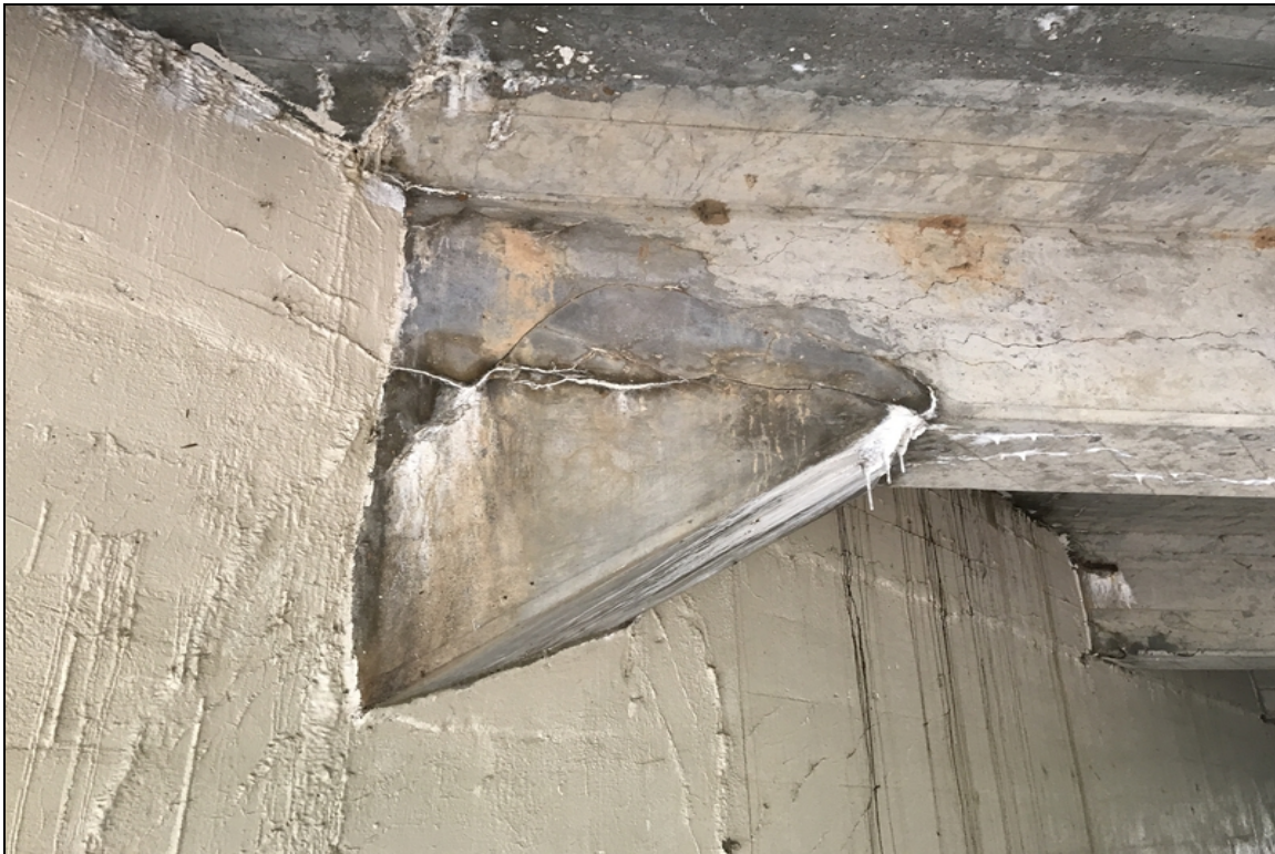
Span 1 bent 1 girder 5 shear type crack
