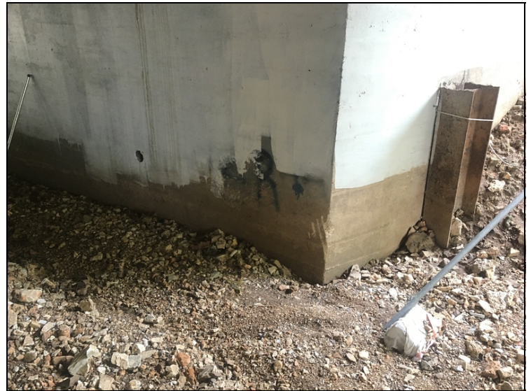
Concrete deterioration. Right end of Bent # 4.
