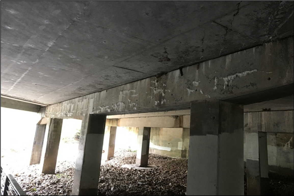
Bent 2 cap cracking with efflorescence (Both sides)
