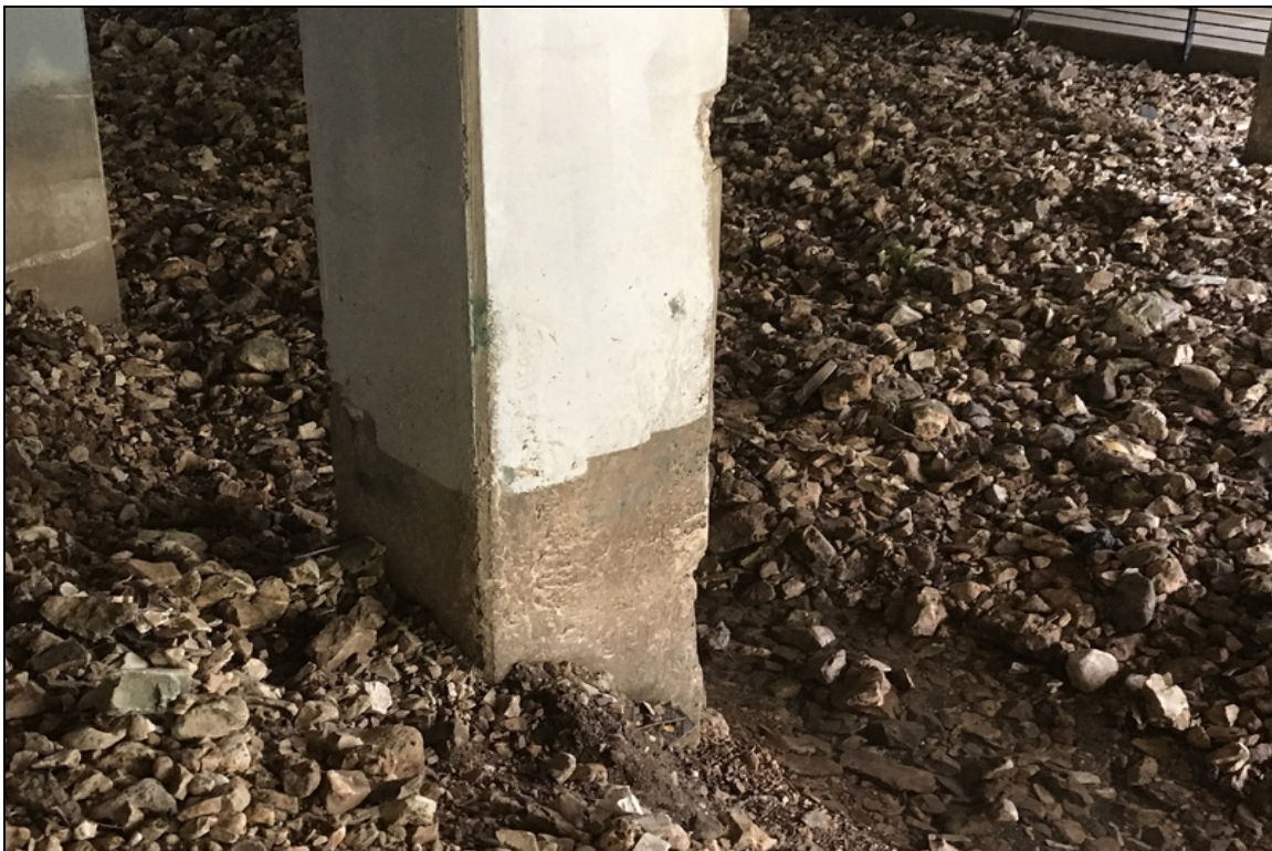
Bent 3 column 4 spalling
