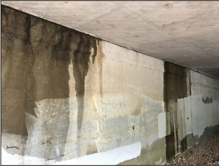
Joints leaking onto substructure
