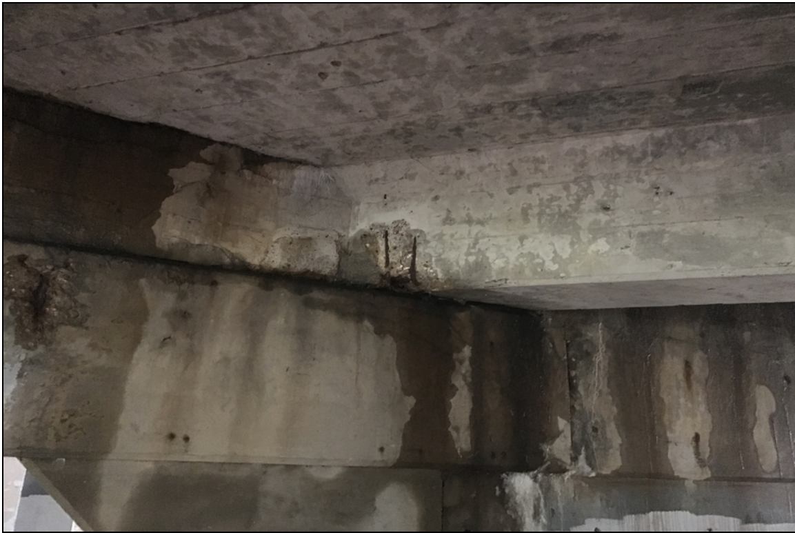
Span 3 girder 3 bent 3 spalling with exposed reinforcing steel
