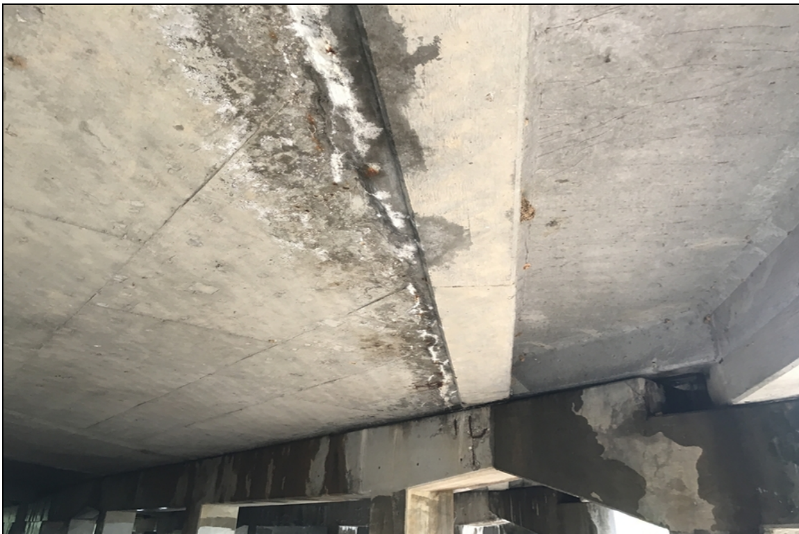
Span 3 construction joint cracking with efflorescence
