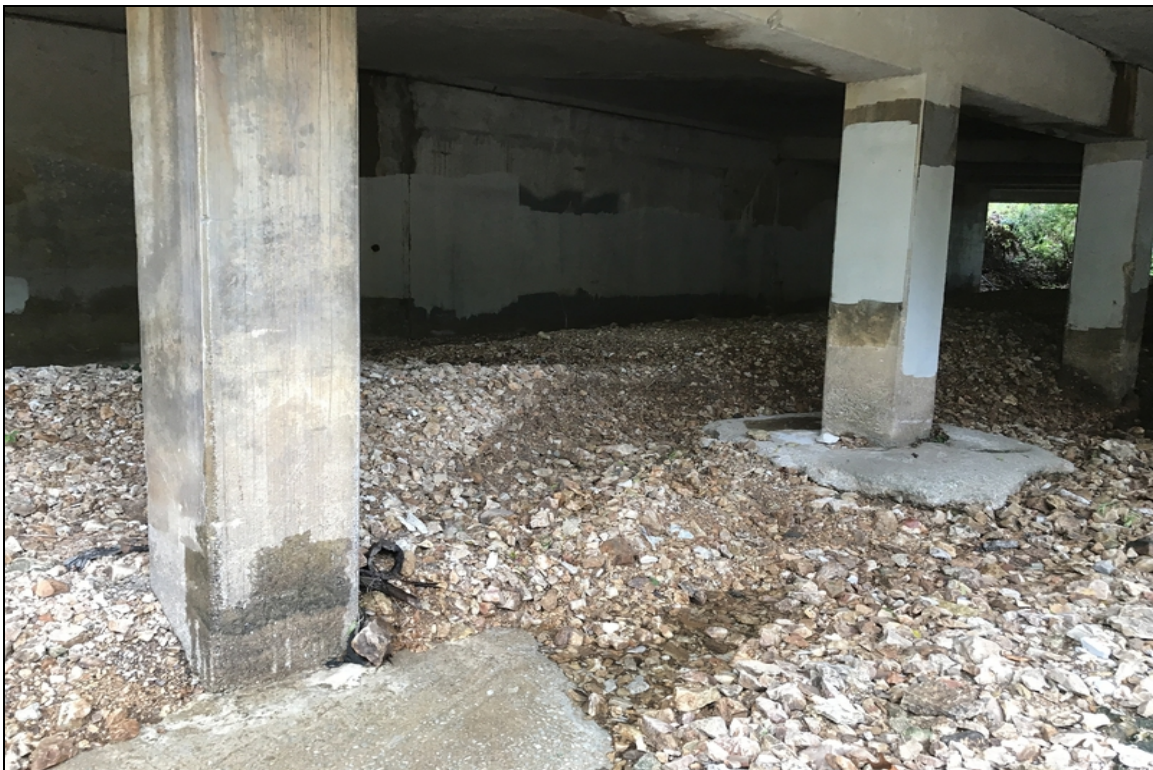
Bents 2 & 3 columns have abrasion
