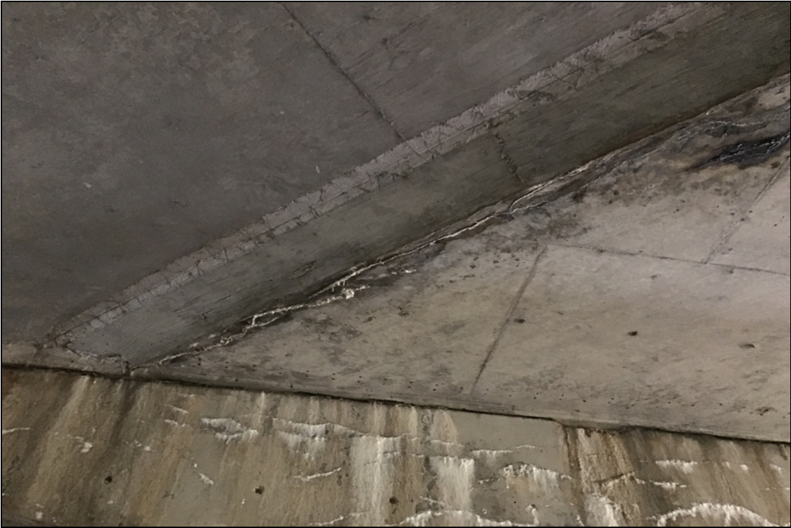
Span 2 slab construction joint cracking with efflorescence
