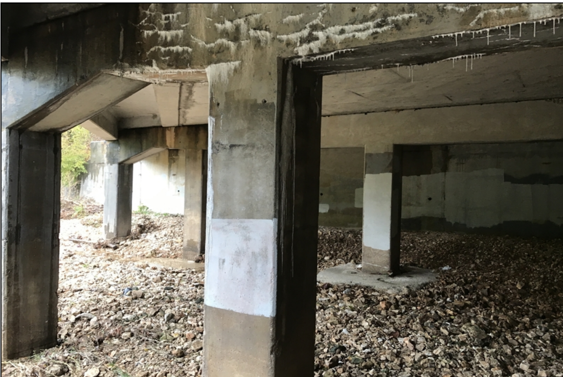
Bent 2 columns 2 & 3 cracking with efflorescence
