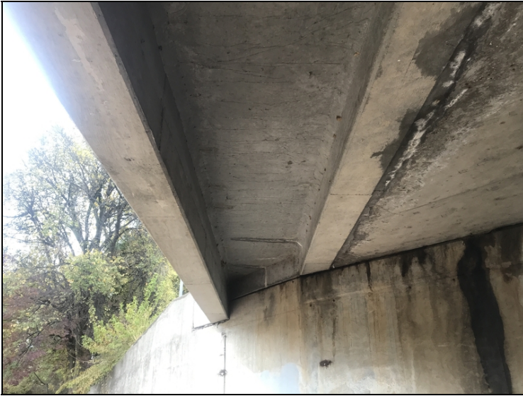
Span # 3. Left. Transverse cracks with efflorescence.
