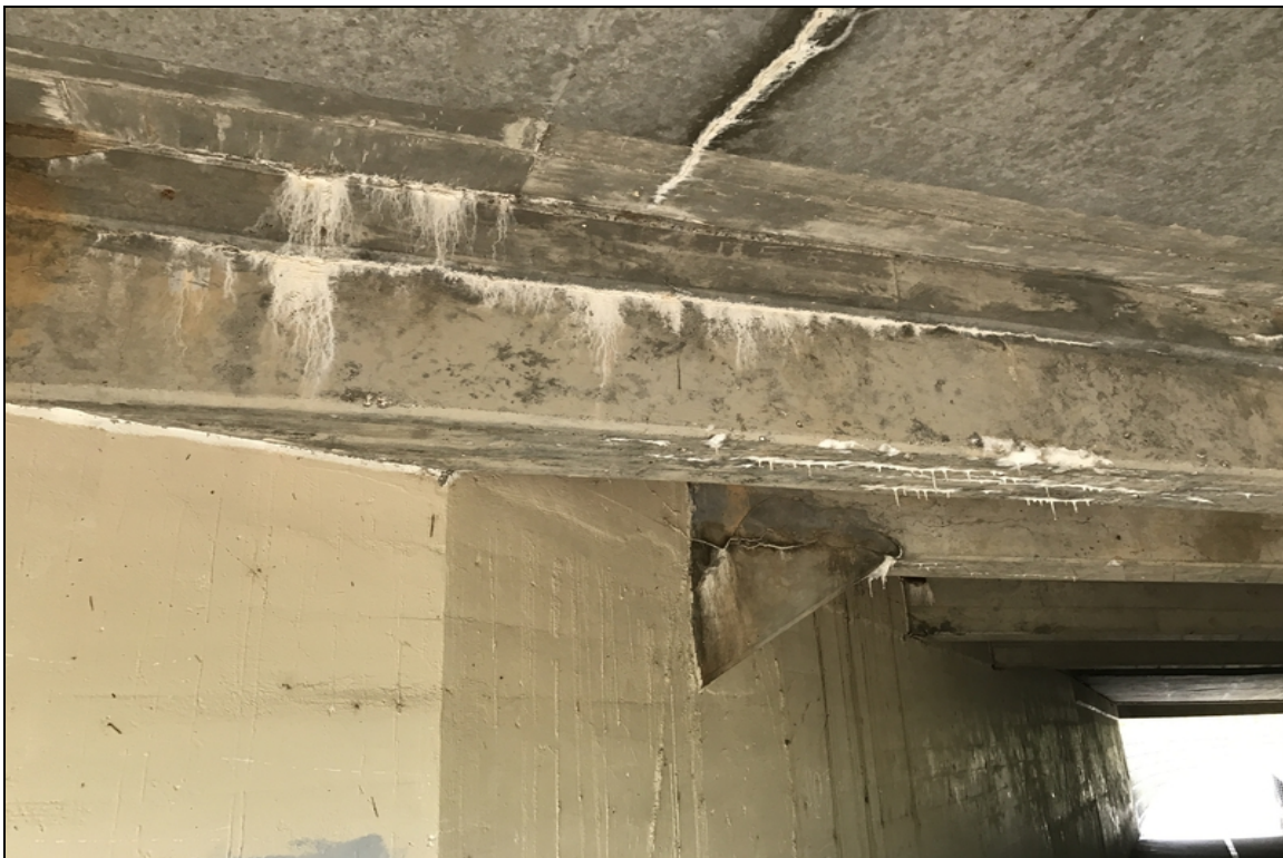
Span 1 girders 5 & 6 cracking with efflorescence
