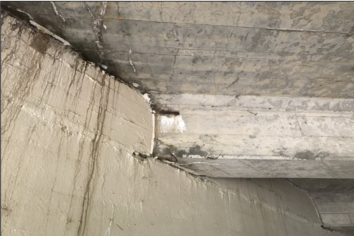
Span 1 bent 1 girder 4 spalling with exposed reinforcing steel
