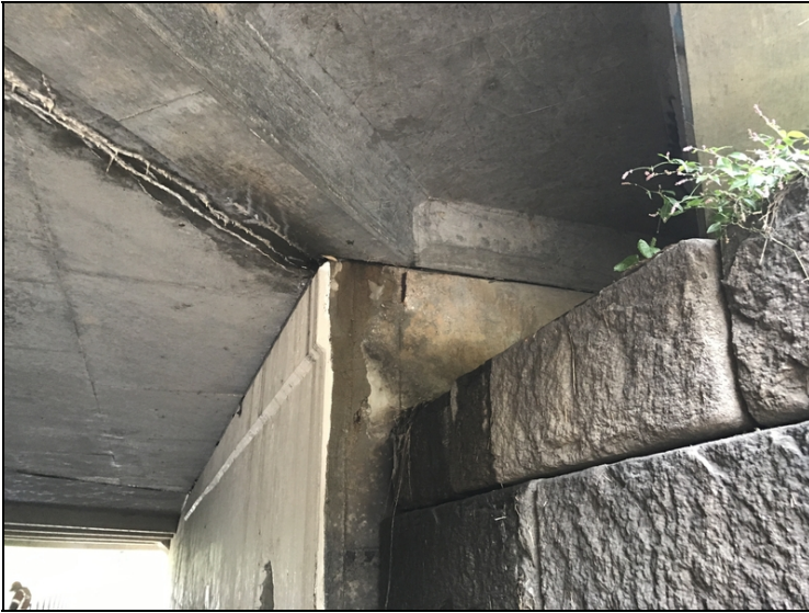
Bent 1 adjacent to girder 2 spalling with exposed reinforcing steel
