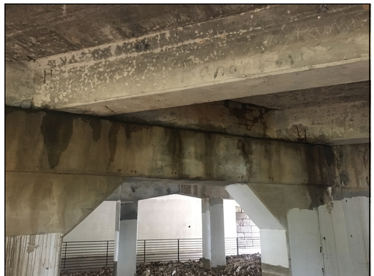
Span # 3. Girders # 3 & 4 over Bent # 3. Spalls with exposed reinforcing steel.
