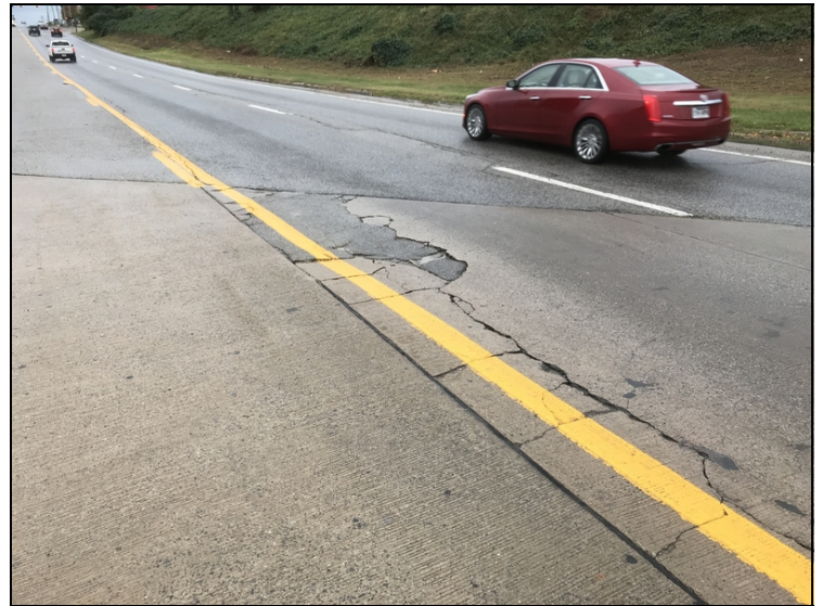
Span 1 spalling in wheel path
