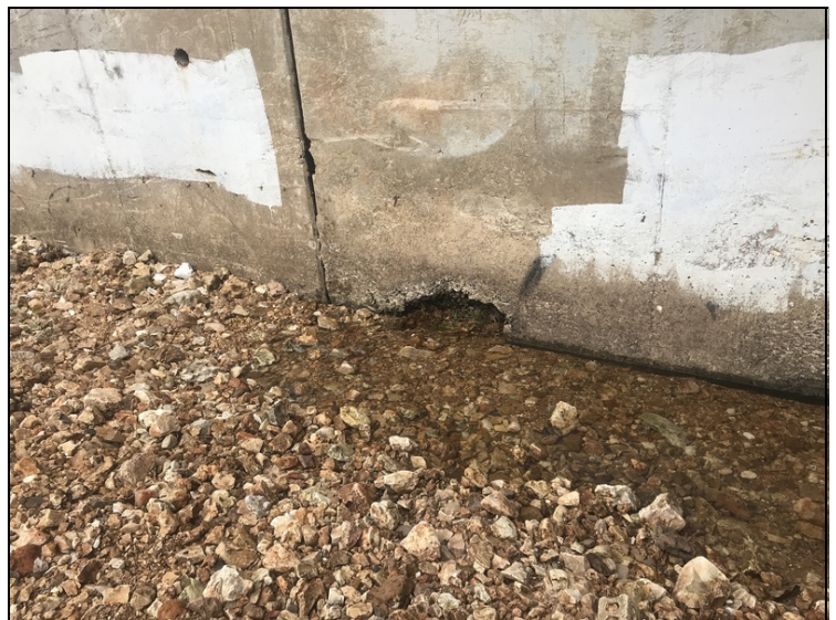
Concrete deterioration. Left end of Bent # 4.
