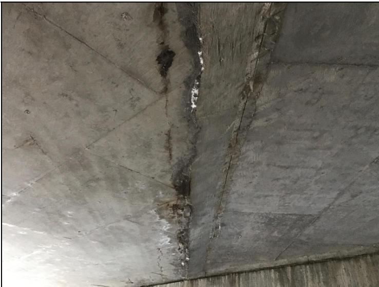
Span 1 slab cracking with efflorescence at construction joint
