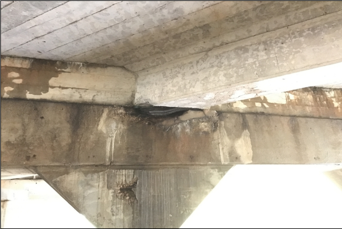
Bent 2 spalling at bearing area adj to girder 4 (Bk)
