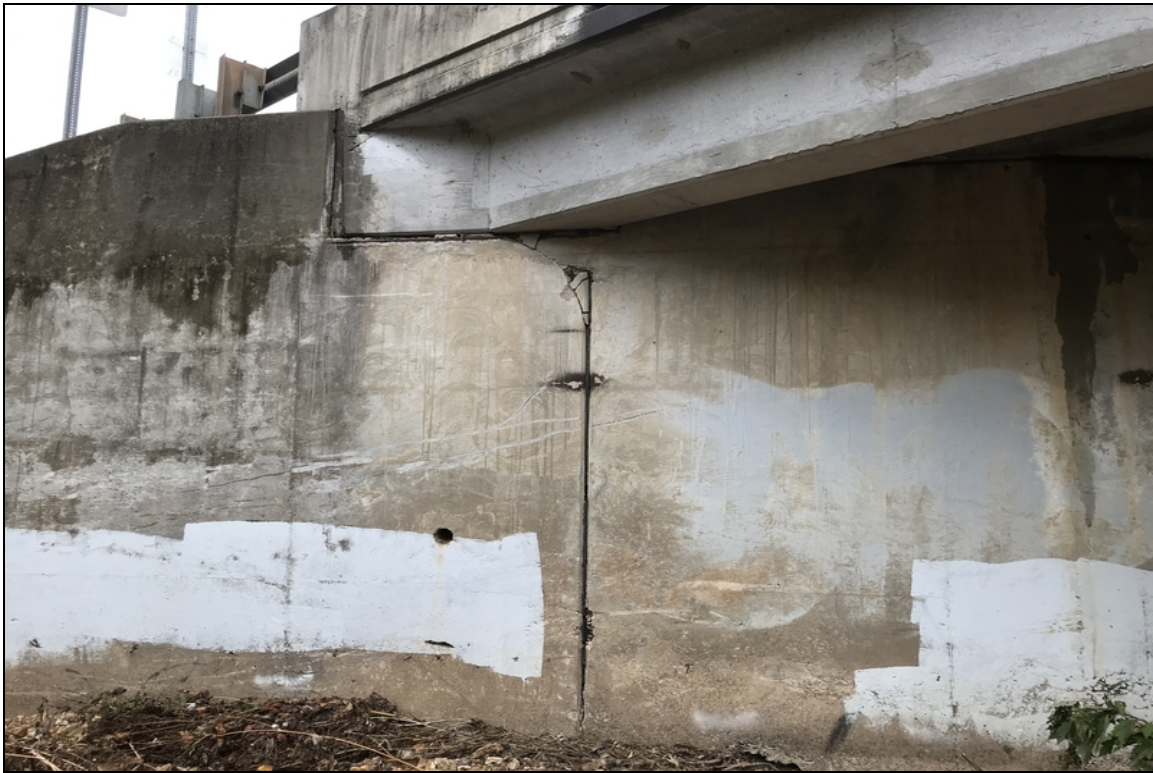
Bent 4 spalling with exposed reinforcing steel at construction joint
