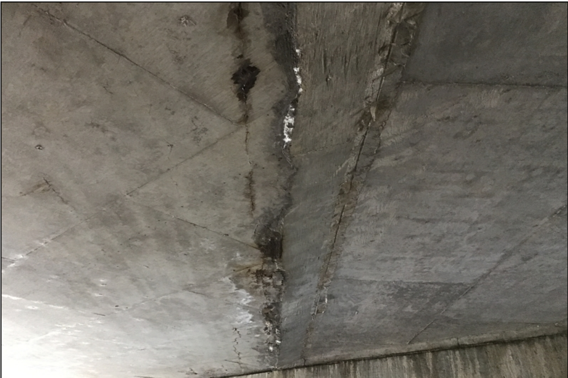
Span 1 slab cracking with efflorescence at construction joint
