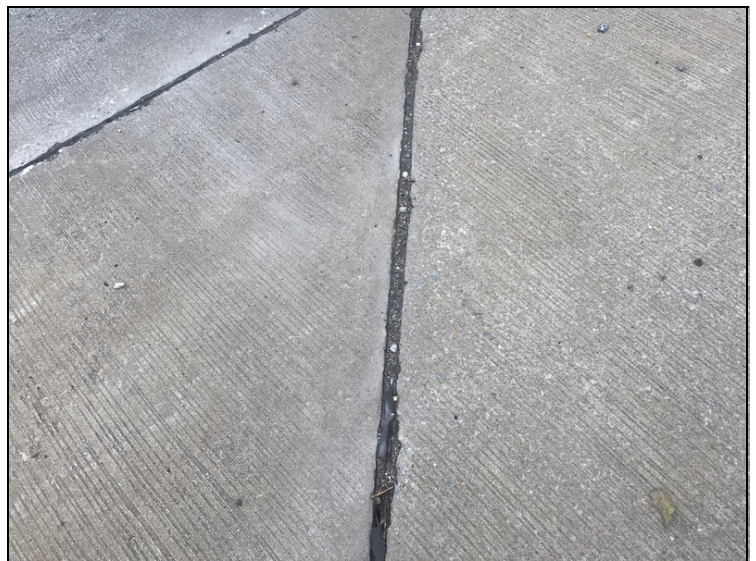
Joint Sealant. Deteriorated and missing.
