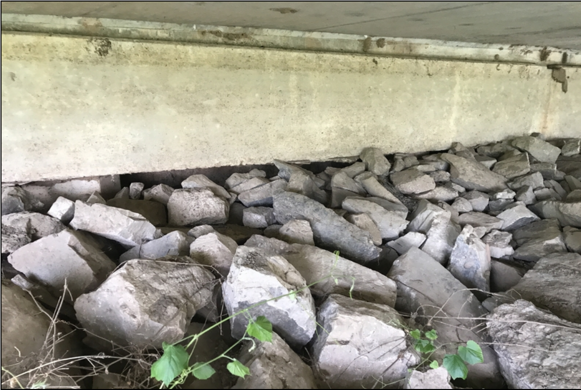
Bent # 4 earth settlement under the abutment cap.
