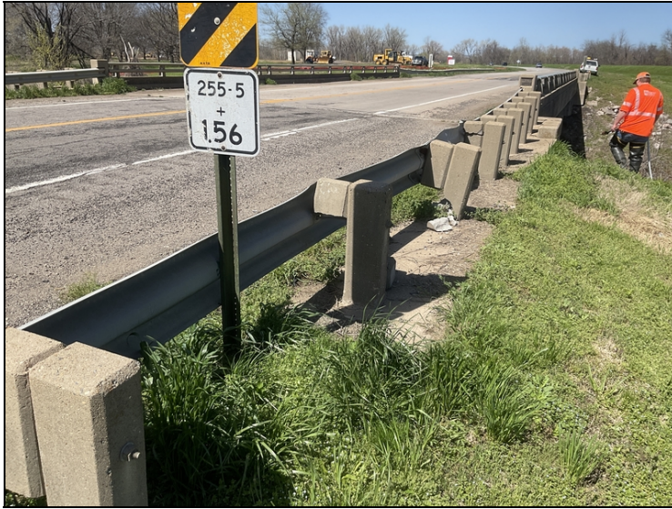
The Southeast approach guardrail has collision damage with several fractured concrete posts and spacer blocks.
