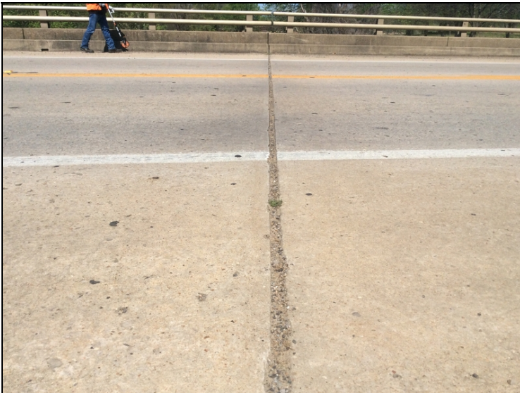
Bent # 3 expansion joint-Debris impaction.
