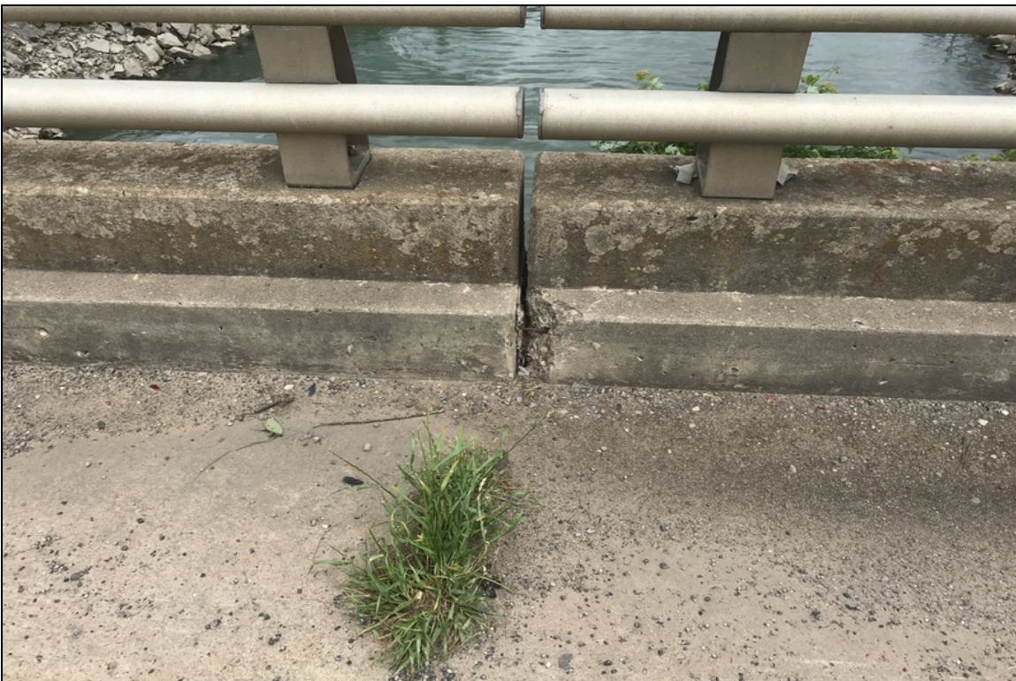
Span # 1, Bent # 2 Rt spalling with exposed reinforcing steel in the base of the bridge rail.
