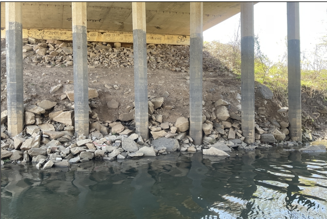
Bent # 2 concrete piling. Typical.
