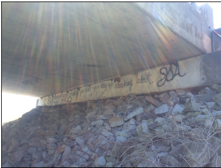
Abutment # 1 -Minor settlement of embankment.
