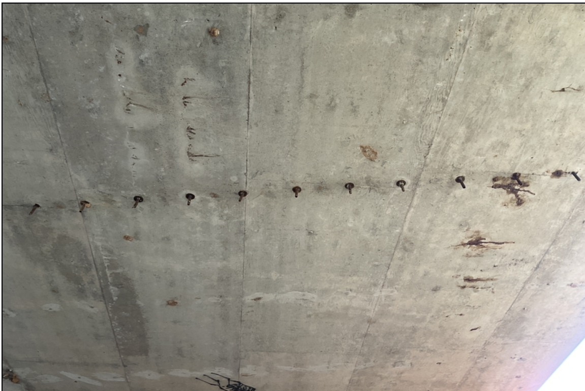
Span # 1 slab soffit has cracking with rust stains.
