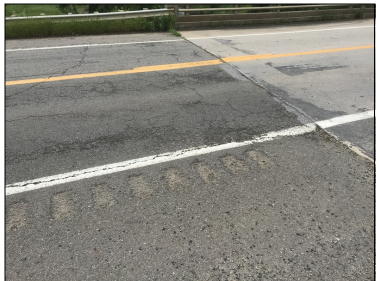
Bent # 1 asphalt settlement.
