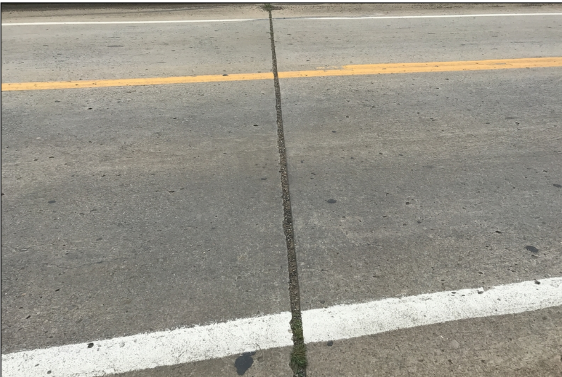
Bent # 2 debris impact in the joint seal.
