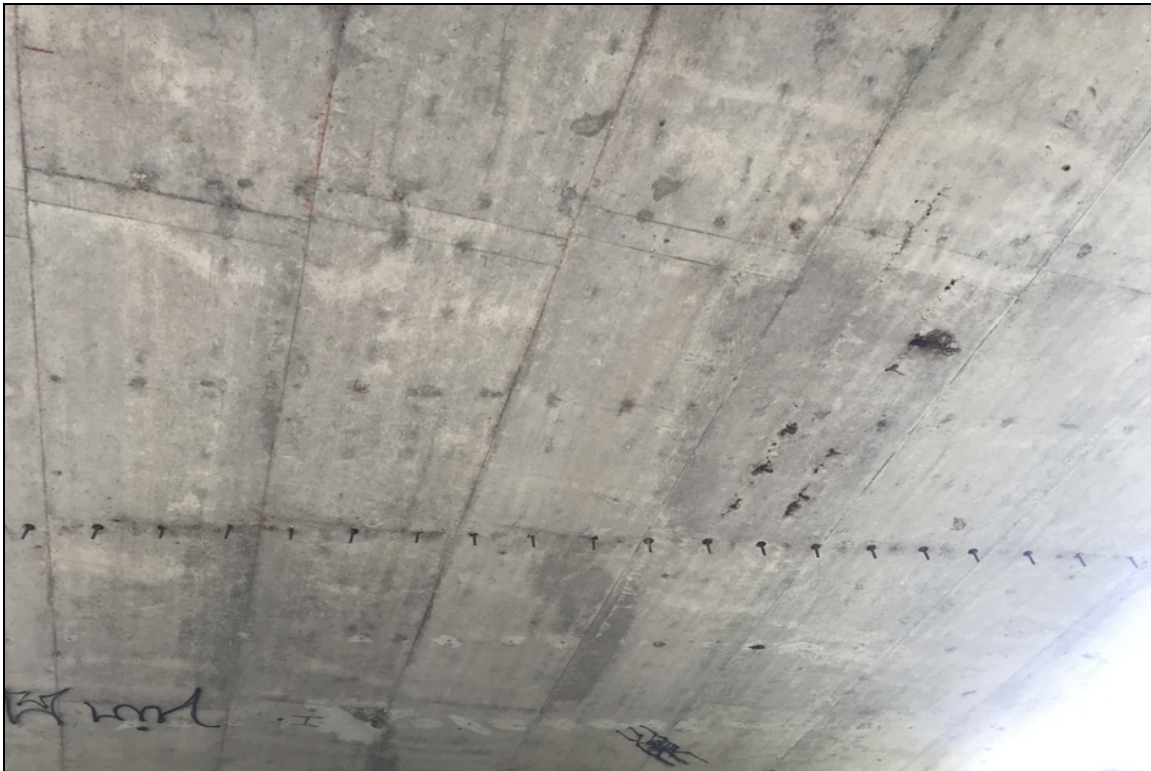
Span # 1 longitudinal cracking with leakage visible from the undersurface of the slab.
