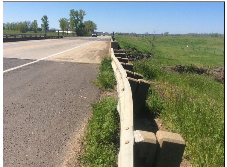
Northwest approach railing-Collision damage.
