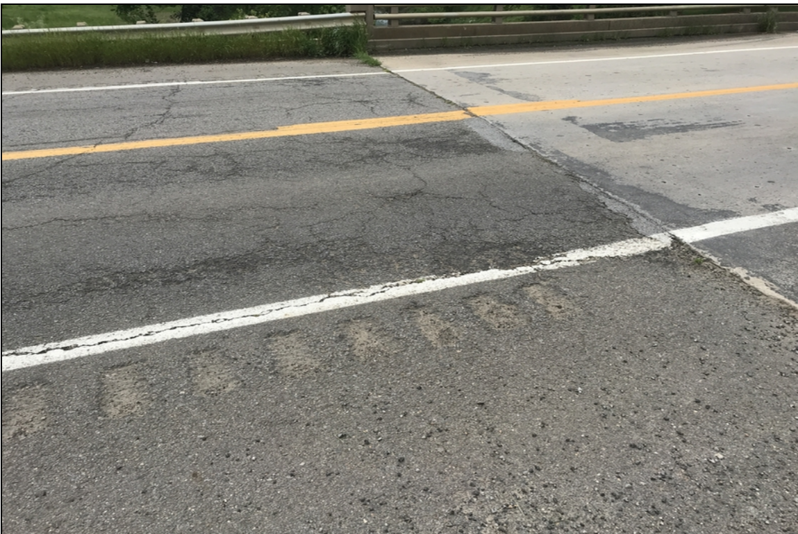
Bent # 1 asphalt settlement.
