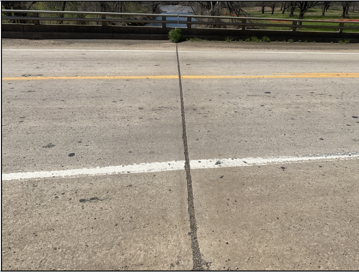
Expansion joint over Bent # 3. Debris impaction.
