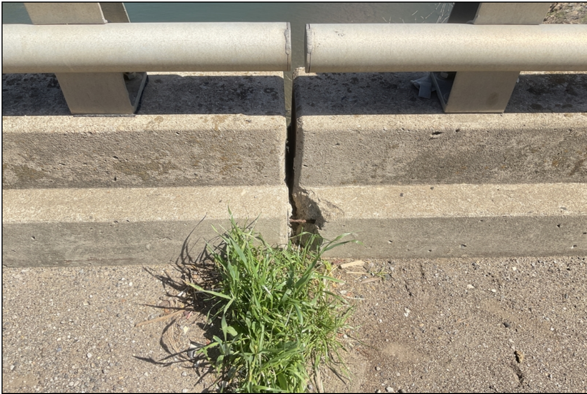
Spall with exposed reinforcing steel in the Right curb over Bent # 2.
