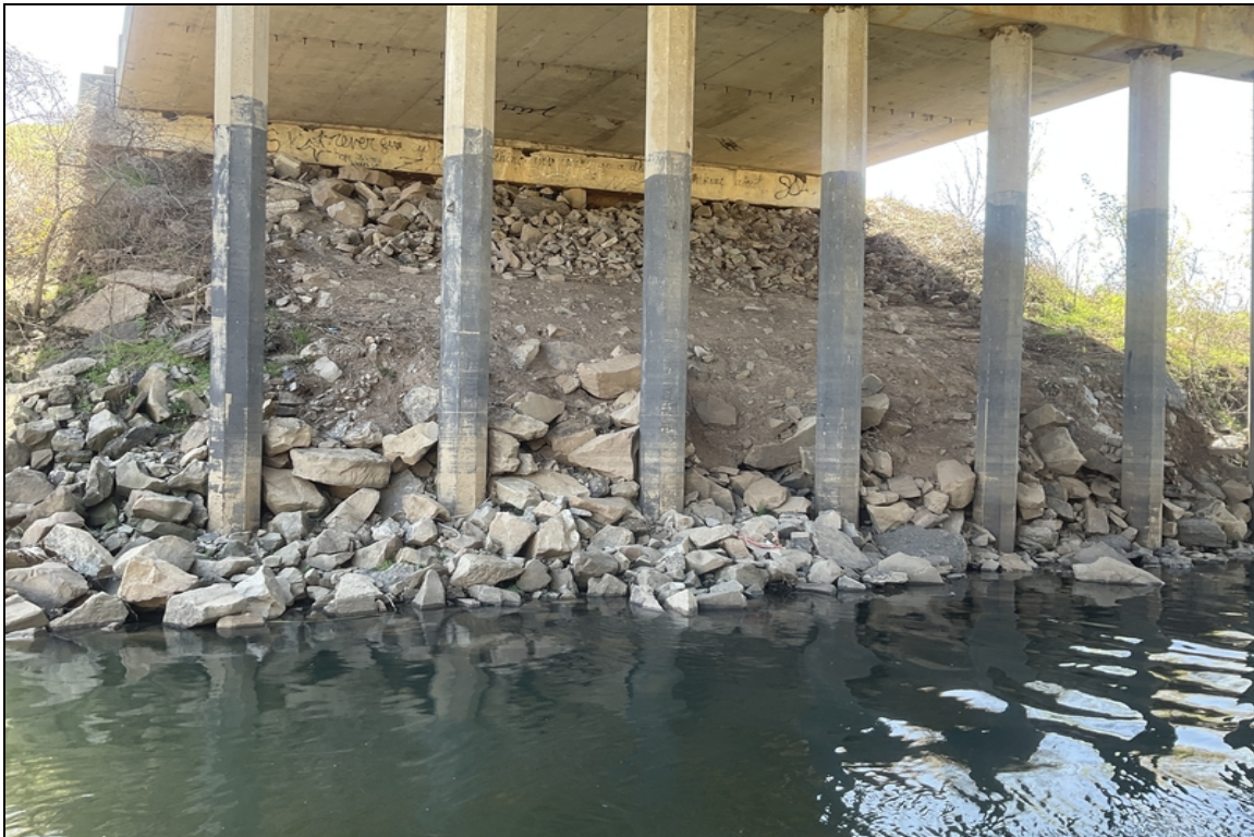
There is embankment erosion and rip rap displacement along both sides of the channel. Photo of South embankment.
