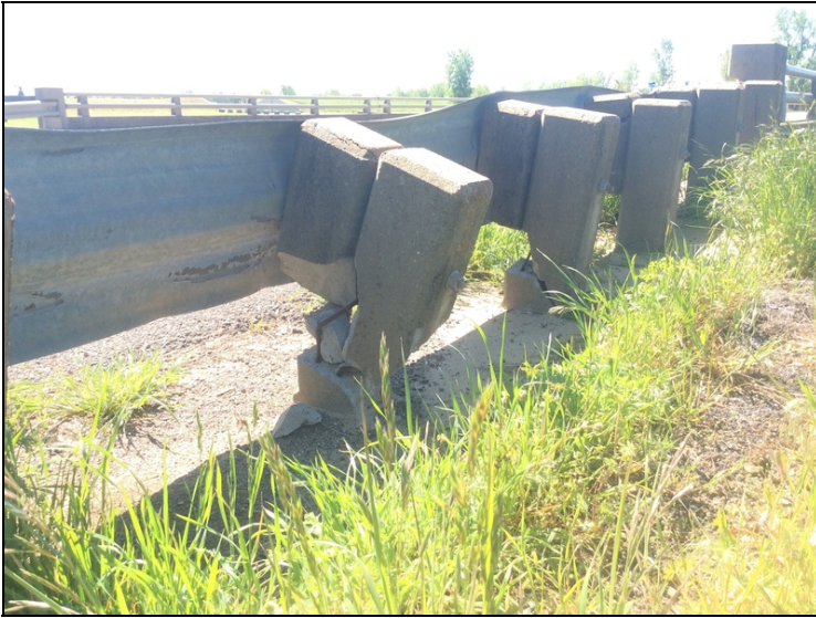
Northwest approach railing-Fractured posts.
