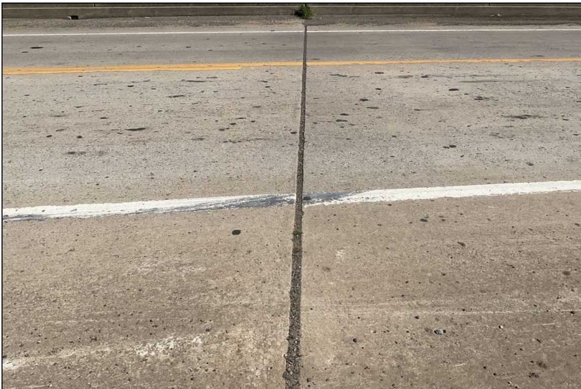
Expansion joint over Bent # 2. Debris impact.
