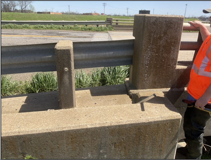
Void under the North approach gutters.
