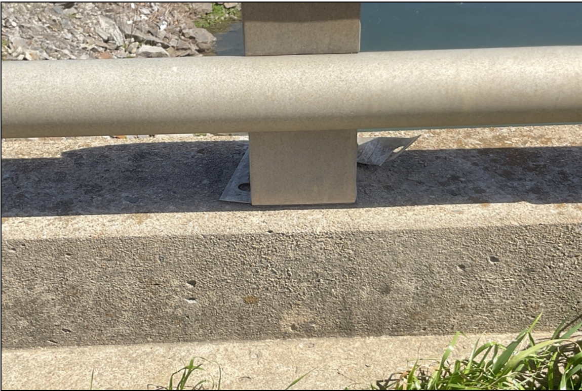
The Right bridge railing post over Bent # 3 has loose anchor bolts.
