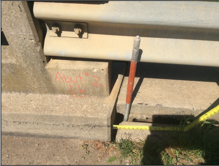
Abutment # 2, left side. Void.
