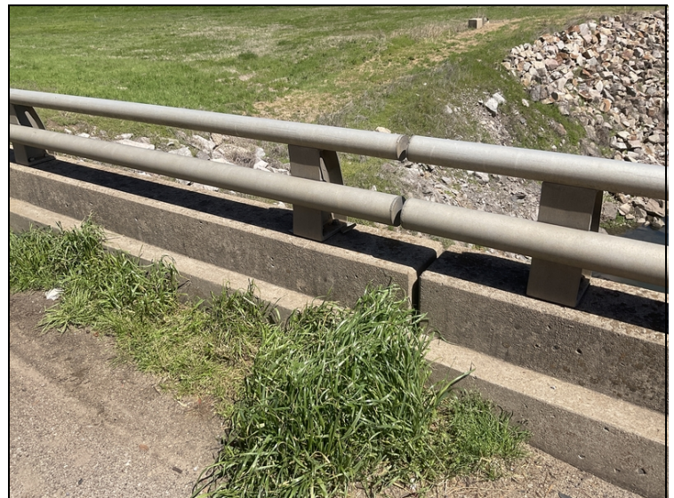
The right bridge railing post over Bent # 3 has loose anchor bolts.
