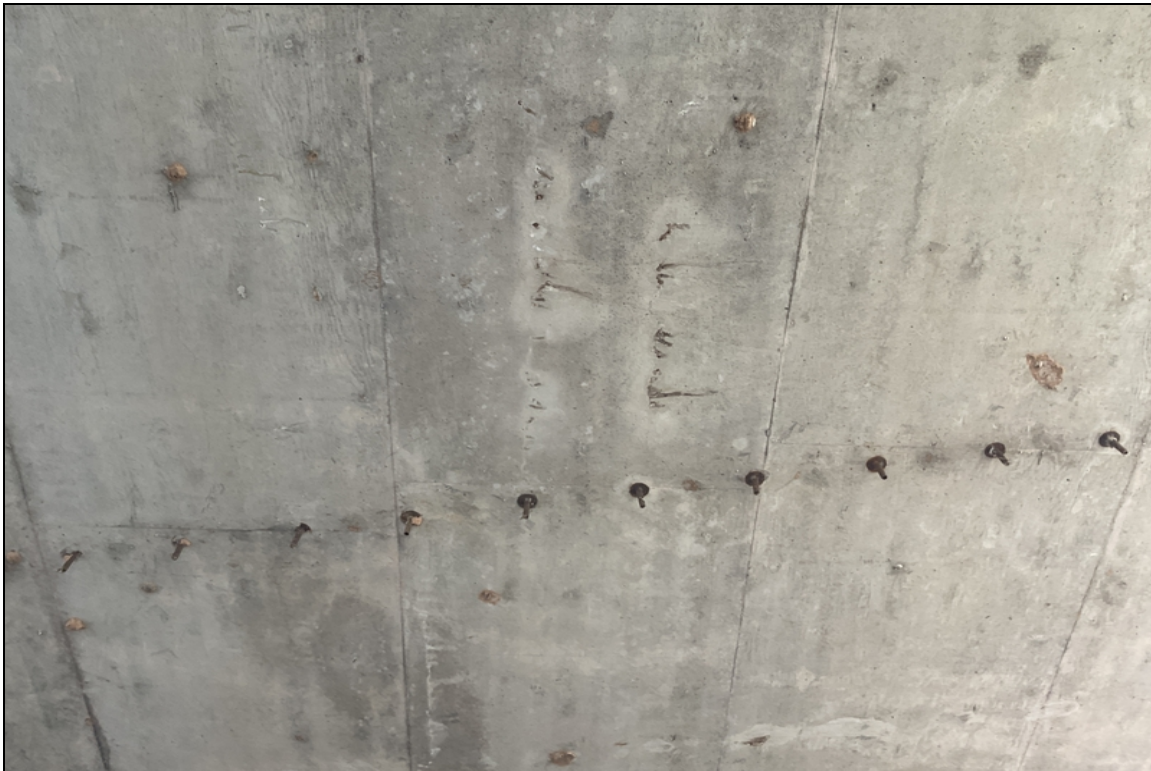
Span # 1 slab soffit with longitudinal cracks and rust stains.
