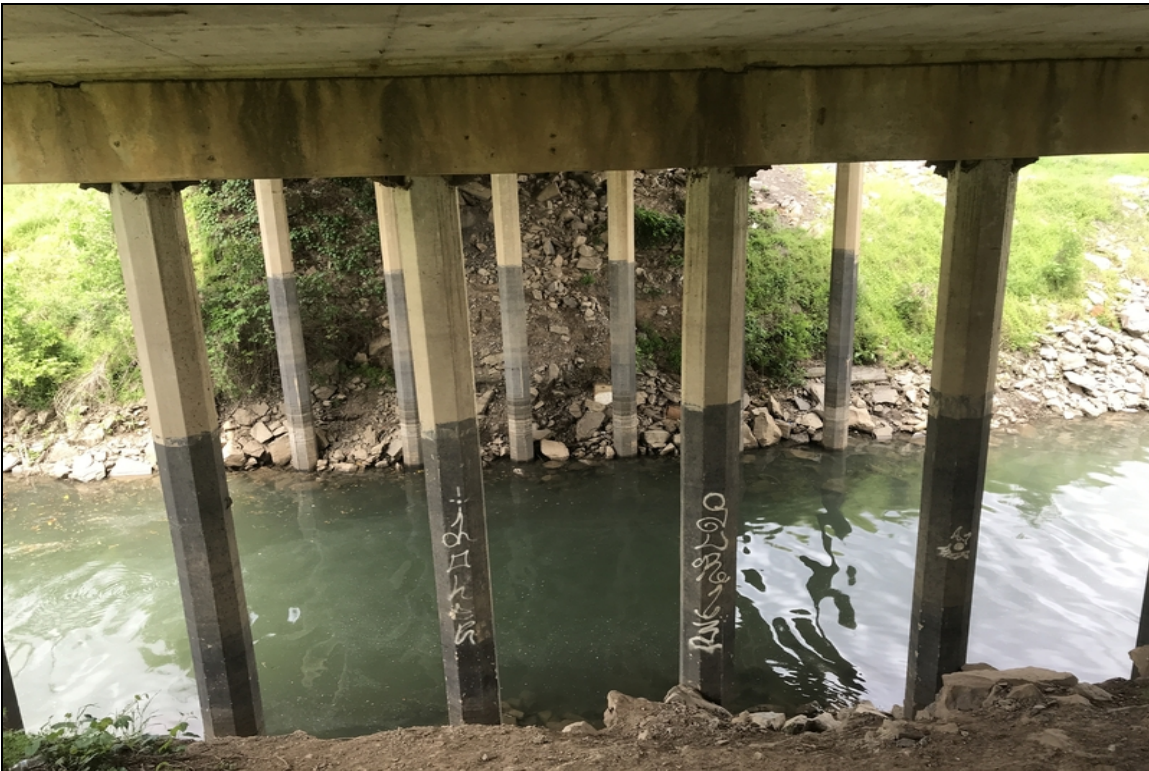
Typical concrete piles.
