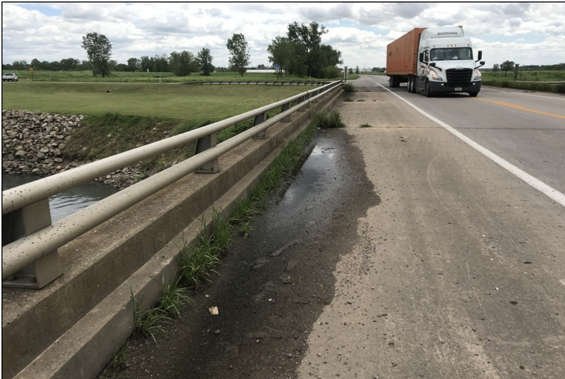
Dirt and debris accumulation in the gutters.
