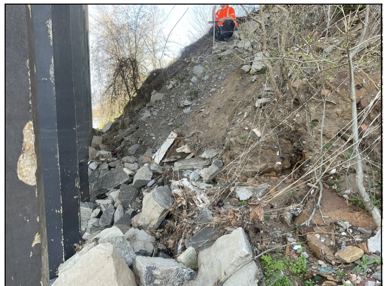
There is embankment erosion and rip rap displacement along both sides of the channel. Photo of North embankment.
