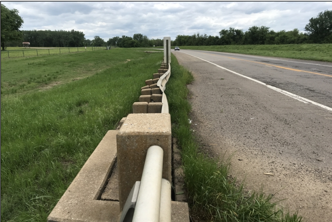
Northwest approach guardrail damage.
