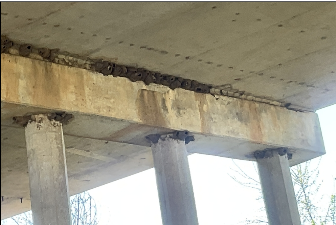
-The ahead side of Bent # 2 cap has two delaminated areas approximately 16" long adjacent to Pile # 2.
