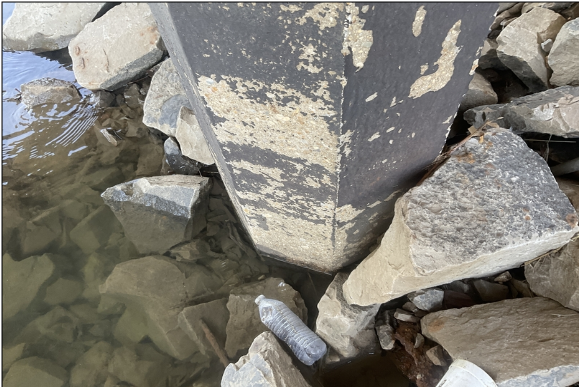
Bent # 3. Piling # 5 typical. -Minor areas with missing tar at the base of the columns.
