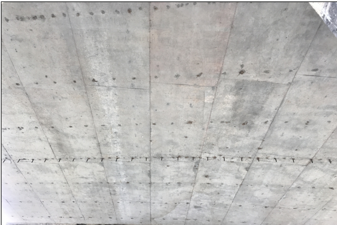
Span # 2 longitudinal cracking visible on the undersurface of the slab.
