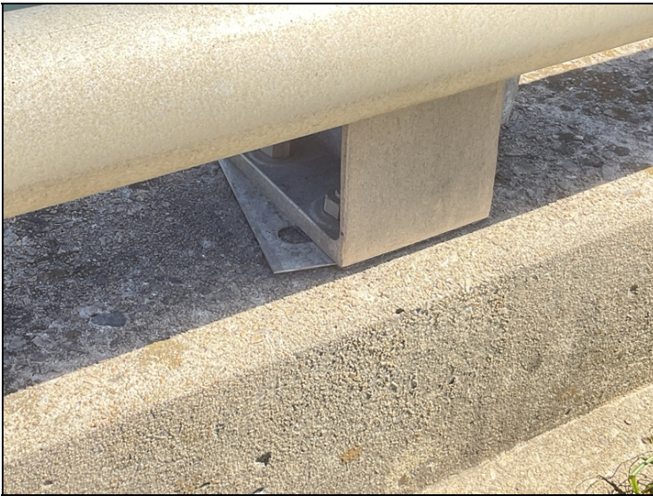
The right bridge railing post over Bent # 3 has loose anchor bolts.
