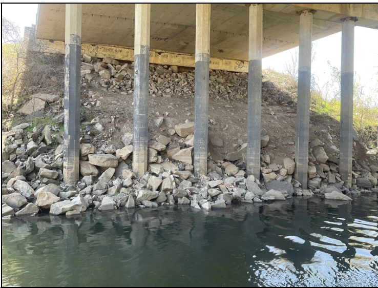
There is embankment erosion and rip rap displacement along both sides of the channel. Photo of South embankment.
