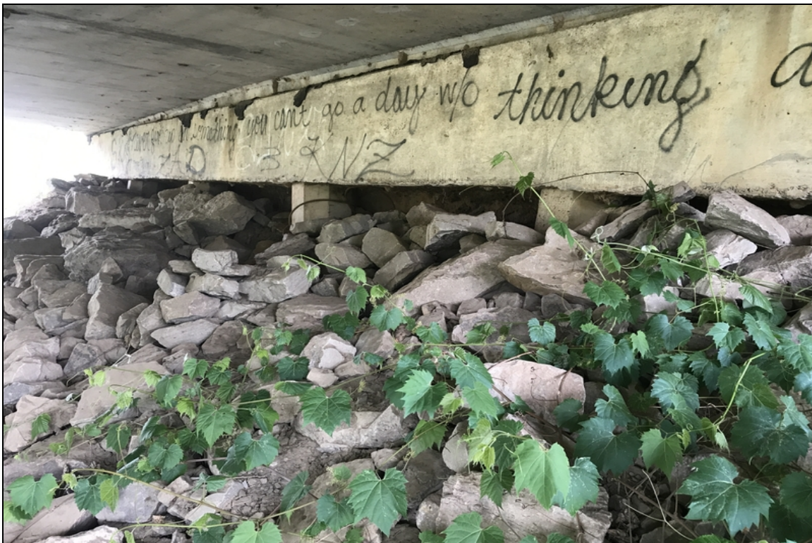
Bent # 1 approach roadway settlement.
