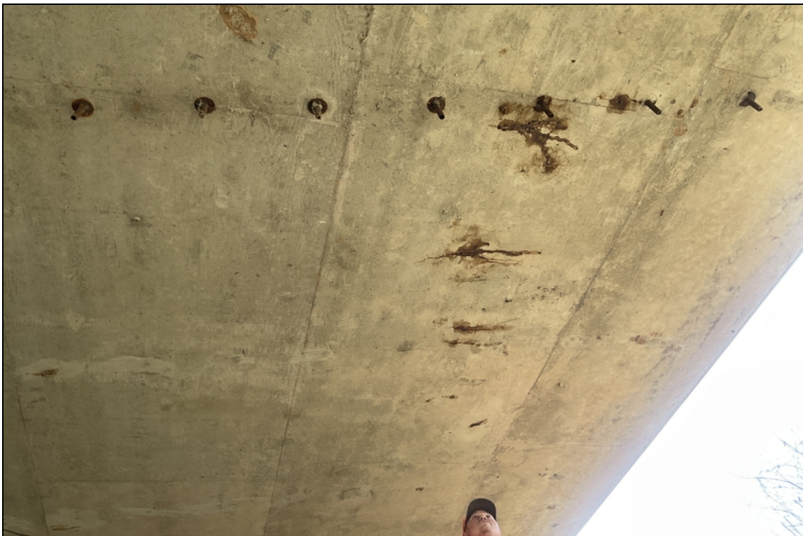
Span # 1 slab soffit with transverse cracks with rust stains.
