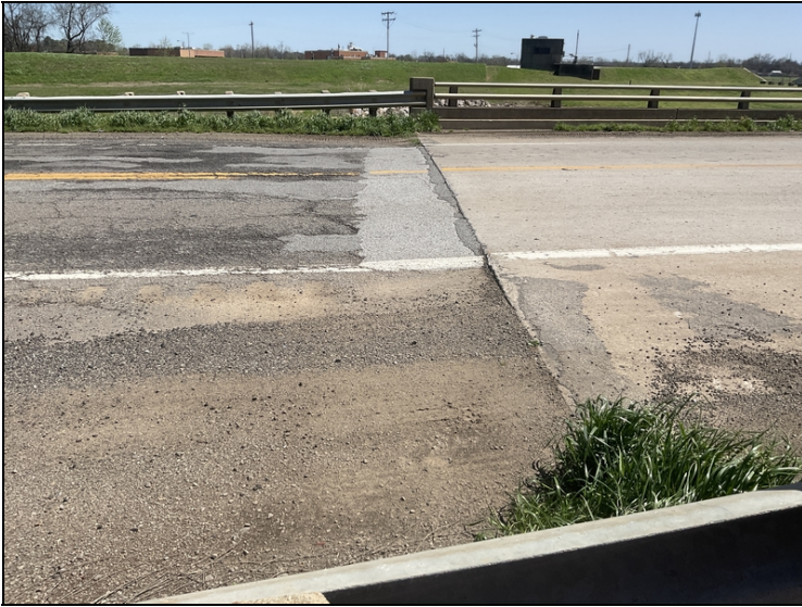
Settlement at the North approach slab adjacent to Bent # 4.
