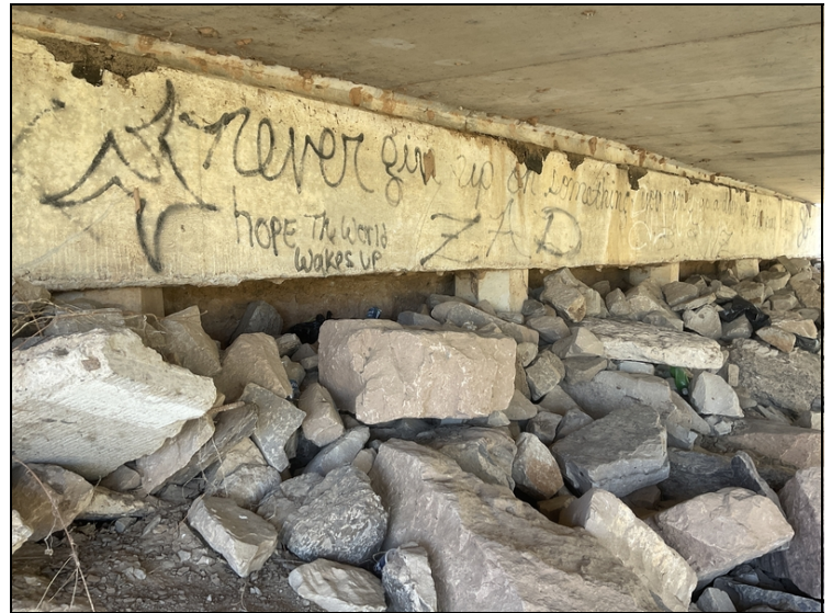
Earth settlement under the South abutment cap.
