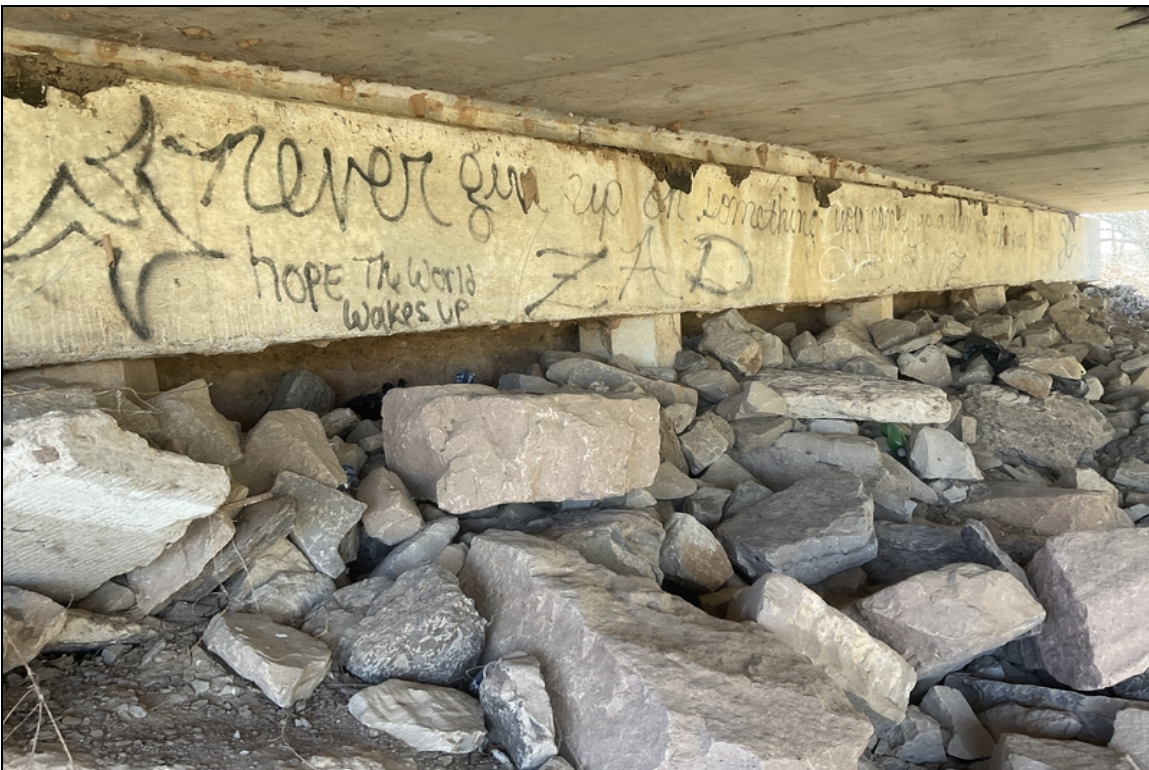
Earth settlement under the South abutment.
