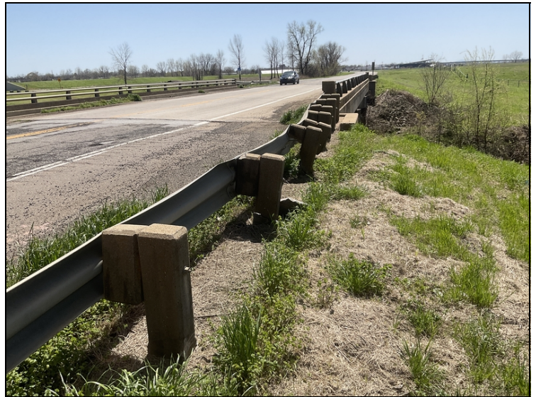
Northwest approach guardrail has collision damage.
