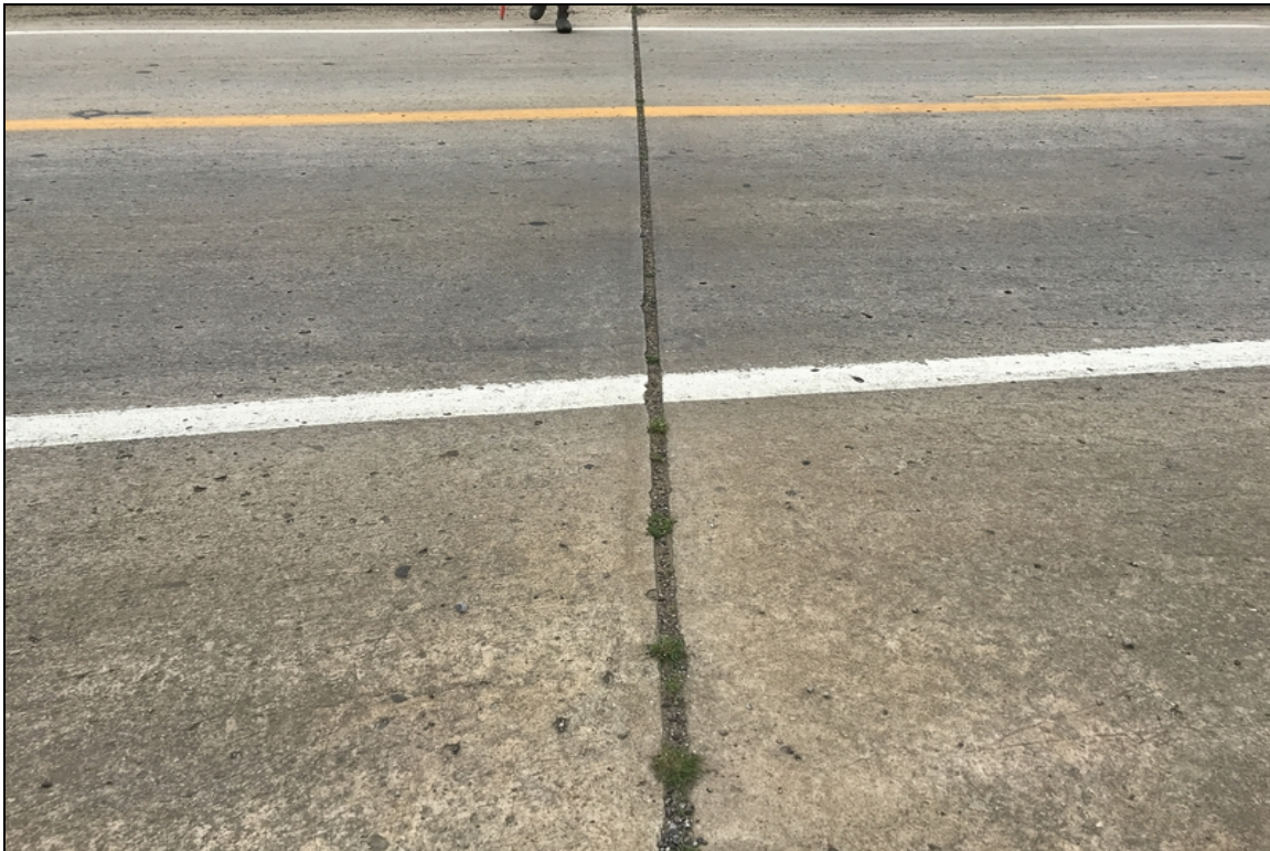
Bent # 3 debris impact in the joint seal.
