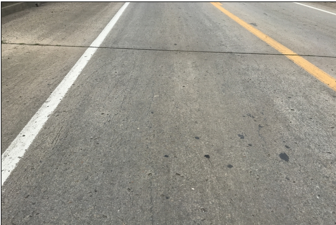
Longitudinal cracking that has been sealed in the past.
