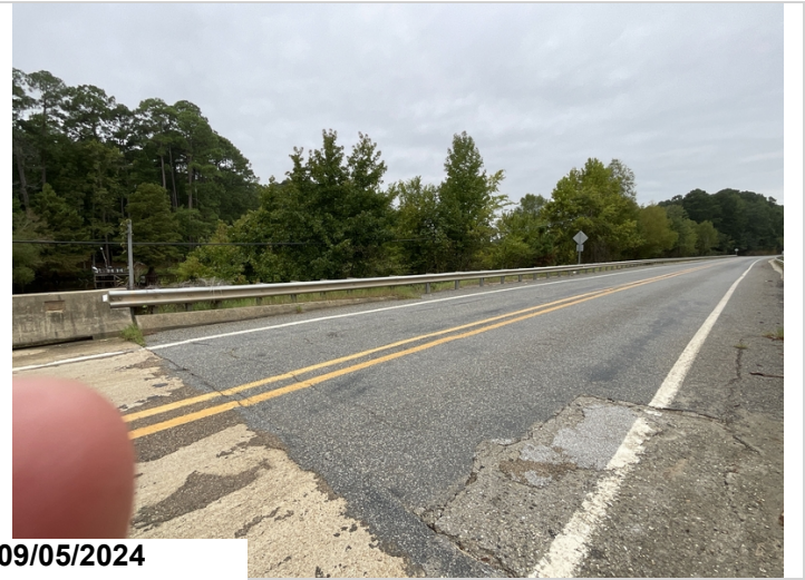
Bridge railing transition.
