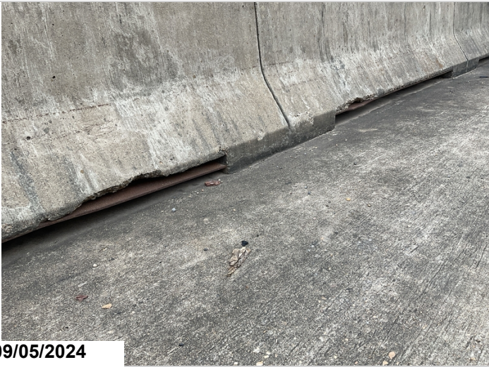
The beginning of the bridge on the left side has minor spalling. Note: The metal plate is loose on the bottom of the parapet wall.
