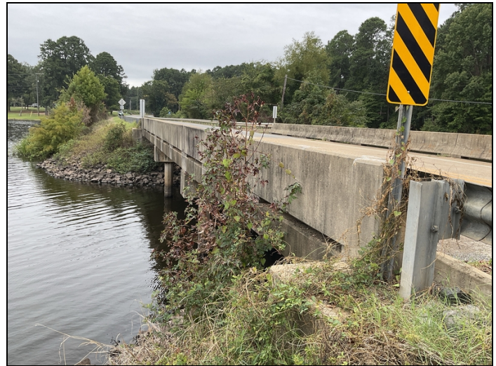
Vegetation on the left side at the beginning of the bridge is growing above the bridge.
