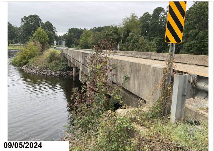
Vegetation on the left side at the beginning of the bridge is growing above the bridge.
