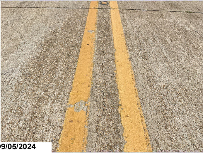
Span 1, centerline, 15' of large cracking.
