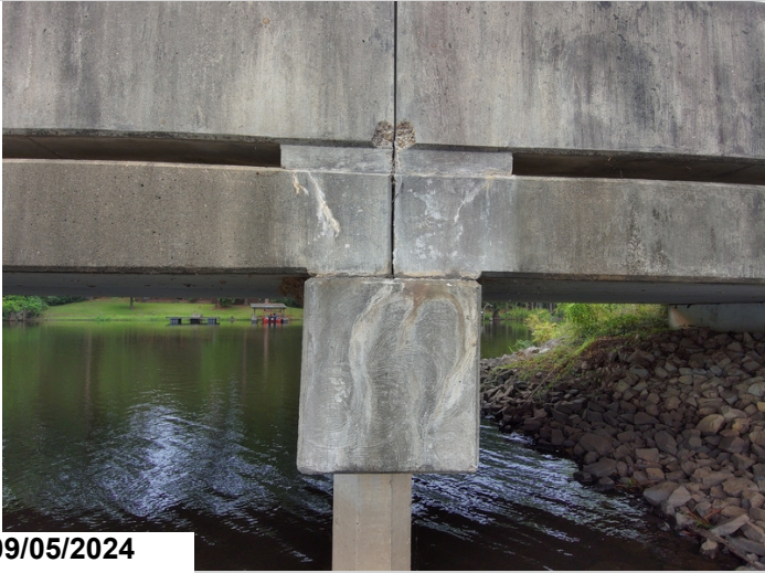
Bent 3, Right side, 2' of cracking with efflorescence, CS2.
