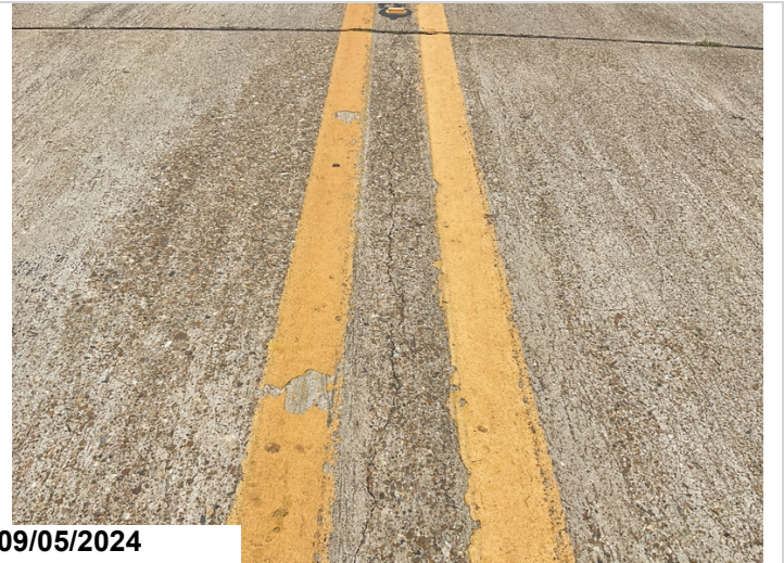
Span 1, centerline, 15' of large cracking, CS3.
