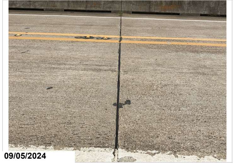
All joints have leakage and debris impaction.
