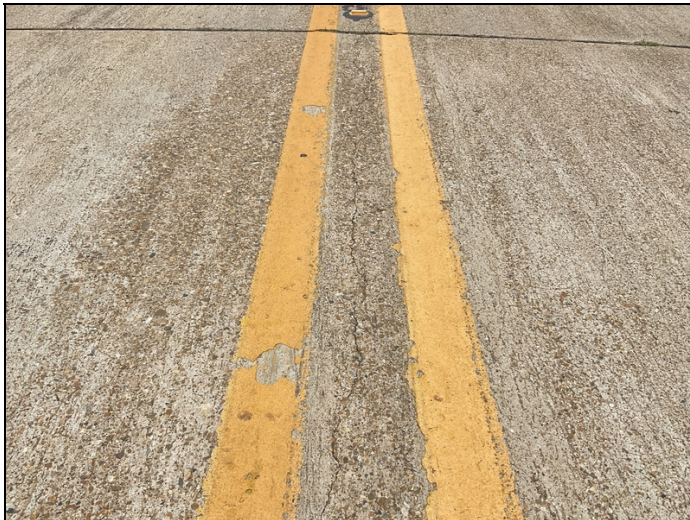
Span 1, centerline, 15' of large cracking.
