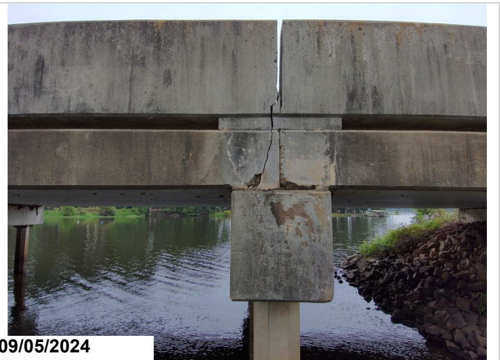
bent 3, right side, 1' of large delam, CS3
