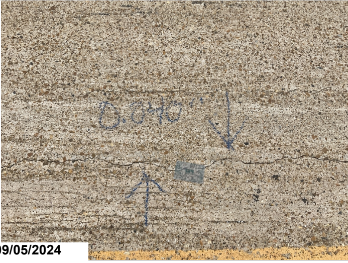
Numerous cracks in various locations of all spans, CS2.
