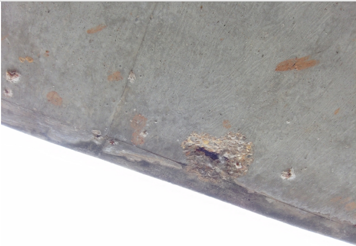
Span 1, Left side, 1' of exposed rebar, CS2.
