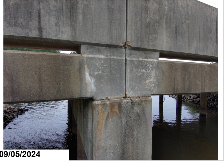
Bent 2, right side, 1' of cracking with efflorescence, CS2.
