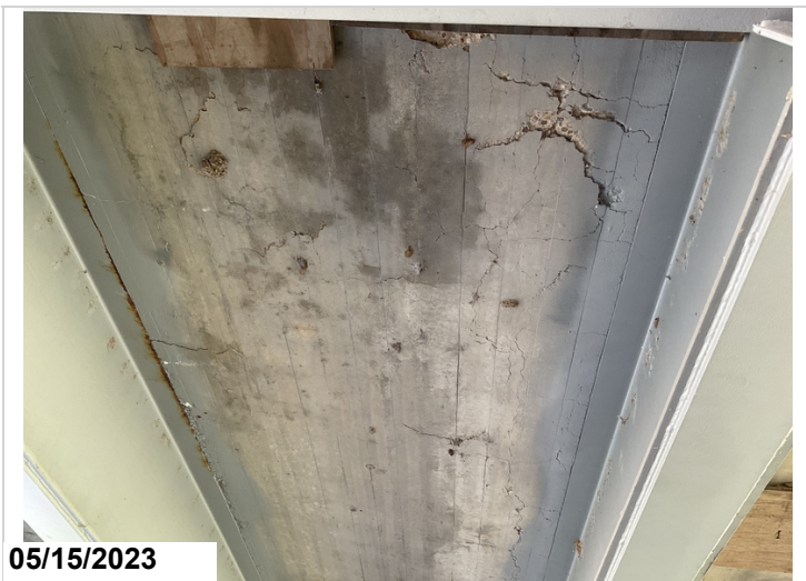
Delam span 9 bay 2
