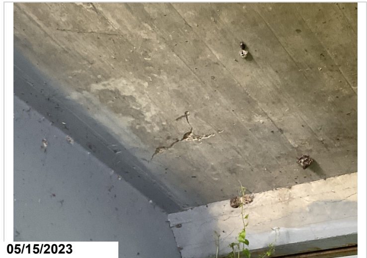
Delam span 3 bay 4
