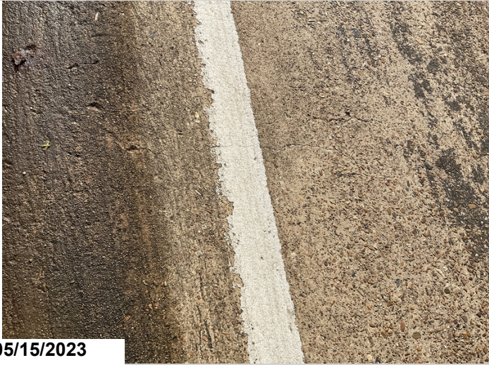
Deck cracking in various locations some sealed some not
