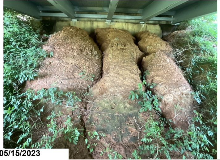
Erosion at bent 1
