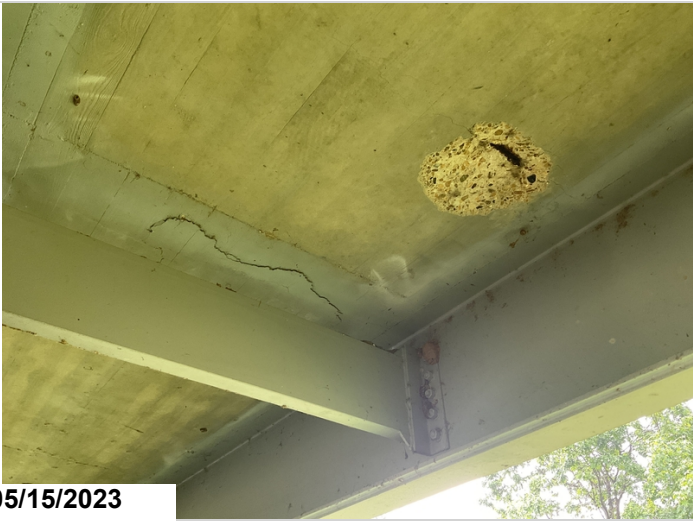
Rebar exposed and delam span 2 bay 4
