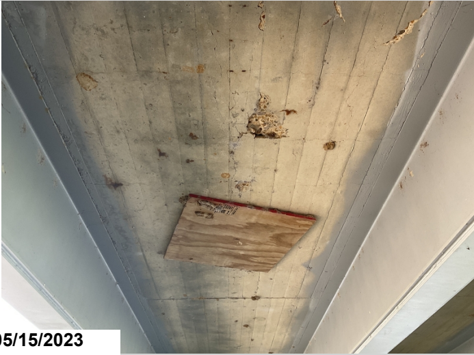
Spall and old patch span 8 bay 1
