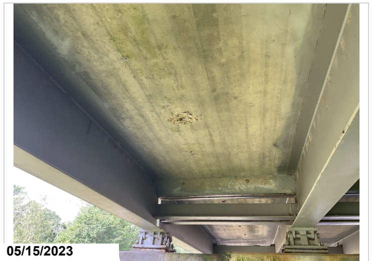
Rebar exposed span 10 bay 4
