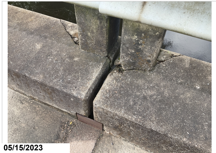
End of span 4 right side guard rail posts are cracked severely
