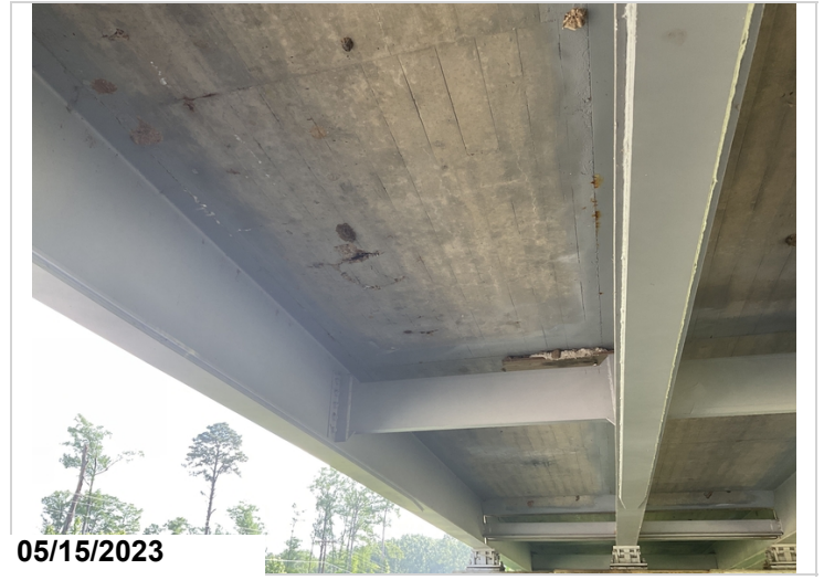
Rebar exposed span 9 bay 1
