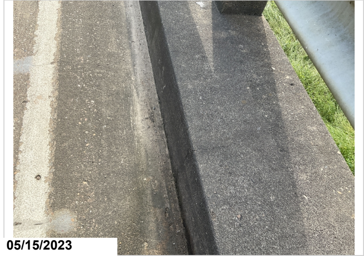
Cracking in concrete guard rail various locations
