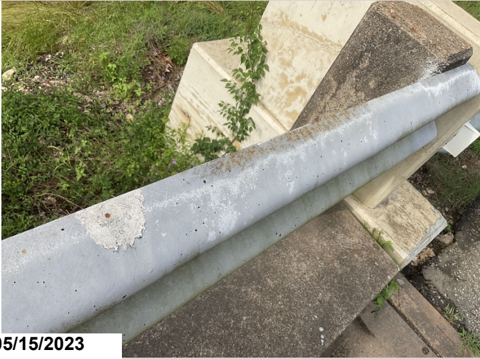
Minor amount of corrosion on guard rail in various locations
