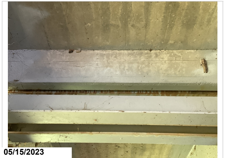
Cracking in various haunch areas no element for this
