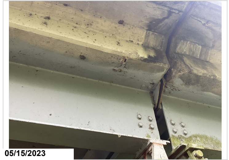
Rebar exposed span 2 left side above bent 2
