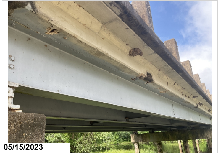
Rebar exposed span 6 left side
