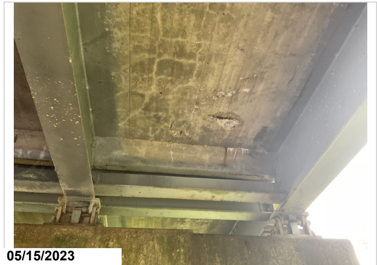
Span 5 bay 4 rebar exposed and delam
