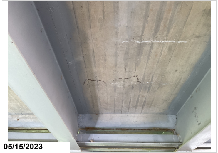
Delam span 8 bay 3
