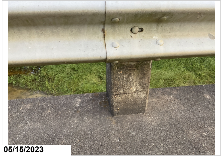
Middle of span 2 left side post has rebar exposed
