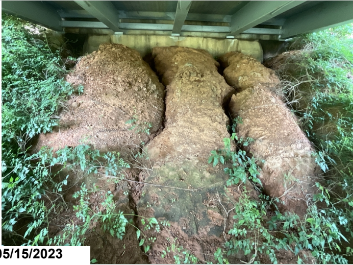
Erosion at bent 1
