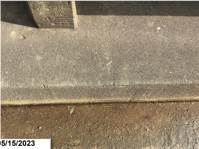
Cracking in concrete guard rail various locations
