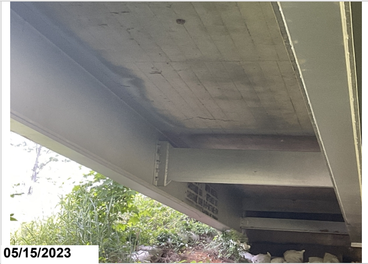
Delam span 10 bay 1
