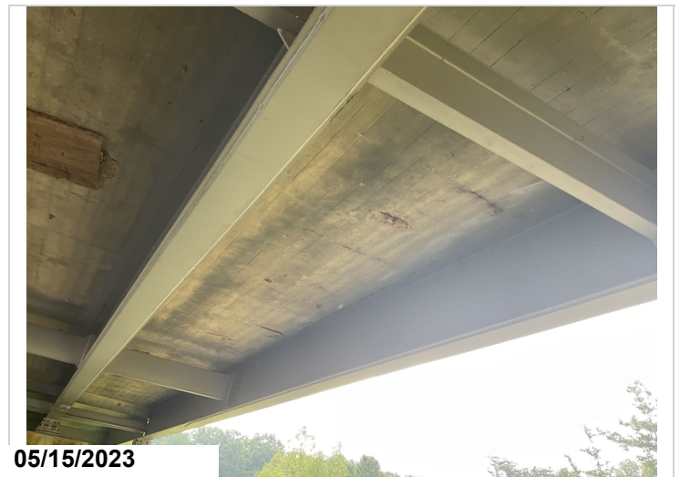
Rebar exposed and delams span 9 bays 3&4
