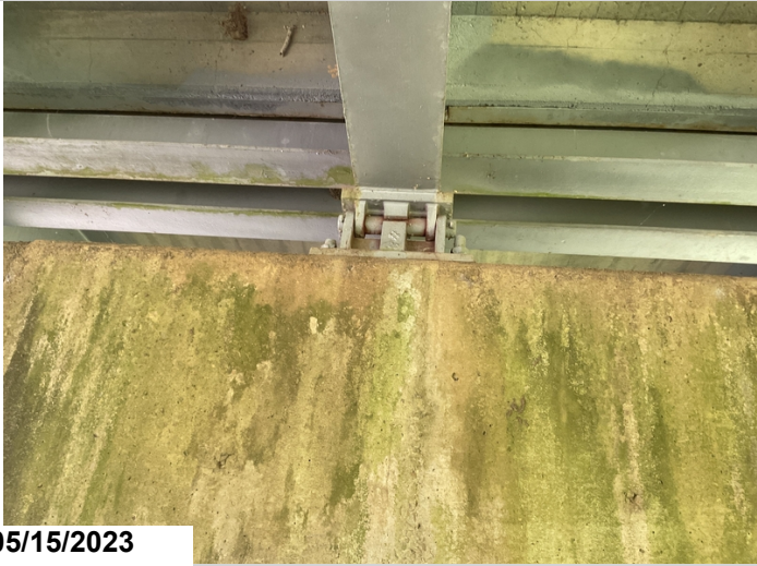
Movable bearing are beginning to corrode
