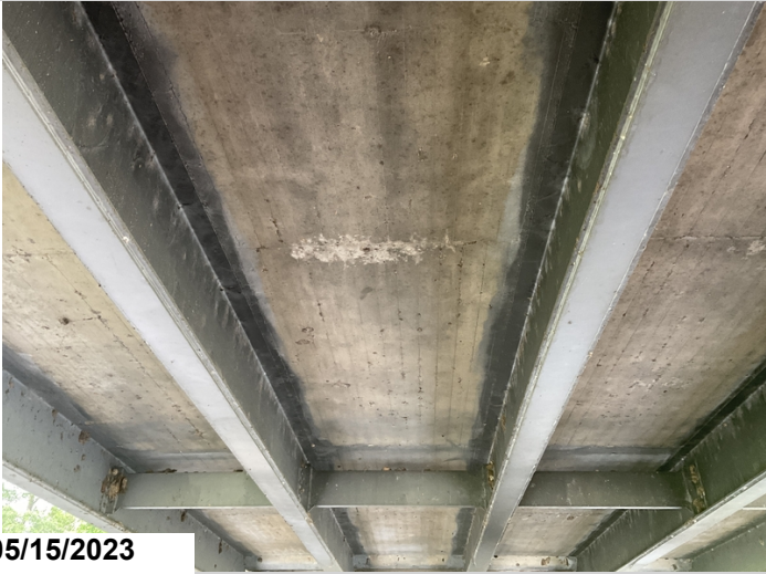
Span 5 bay 3 efflorescence
