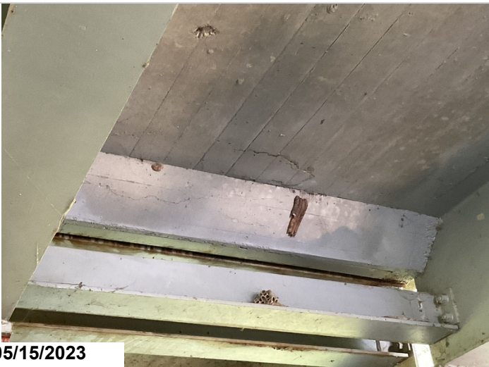
Delam span 2 bay 1
