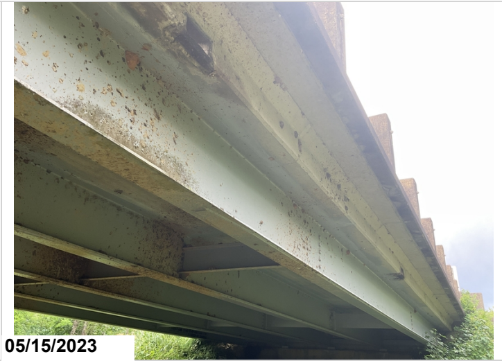
Cracking around both drain holes span 1 left side
