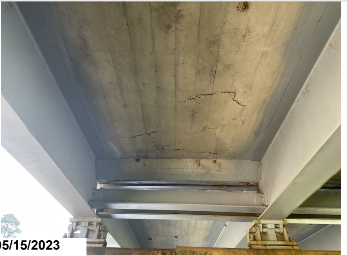
Delam span 8 bay 1
