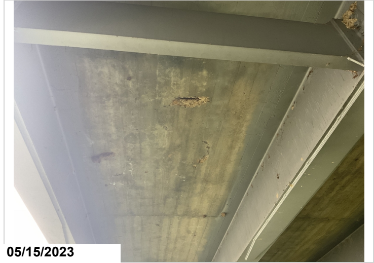
Rebar exposed and delam span 6 bay 1
