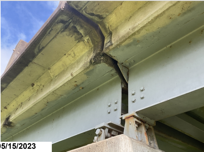
Delam above bent 7 right side
