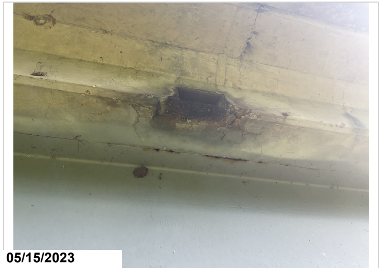
Delam right side span 2 drain hole
