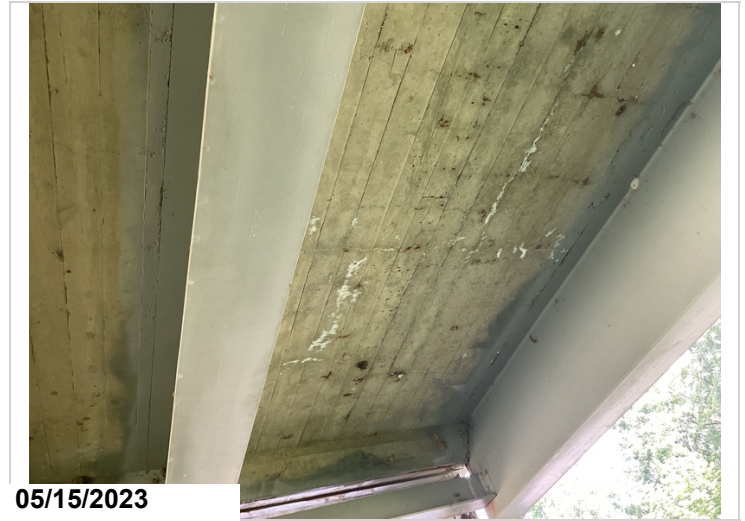
Efflorescence span 10 bay 1
