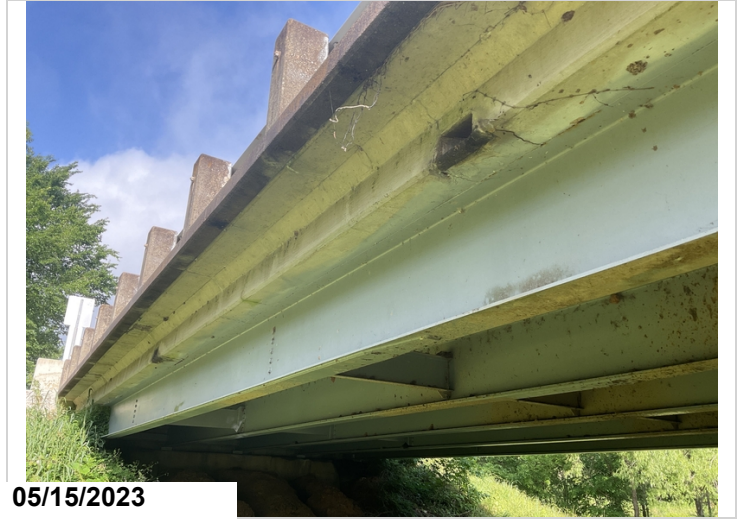
Cracking at both drain holes span 1 Rt side
