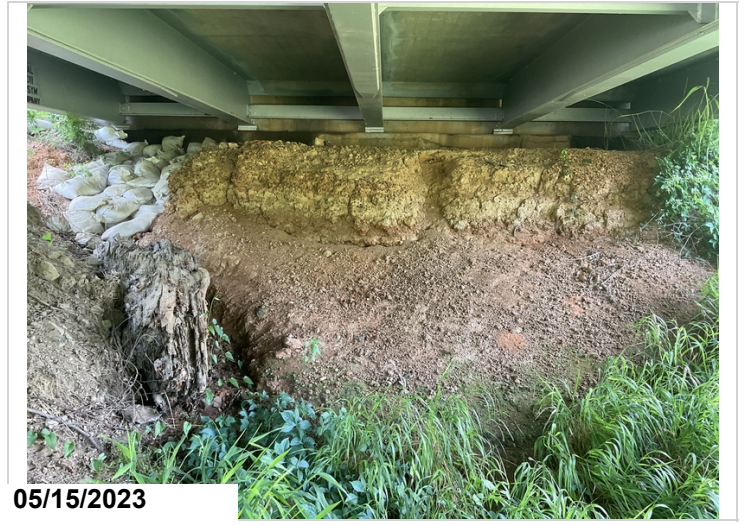
Erosion bent 11
