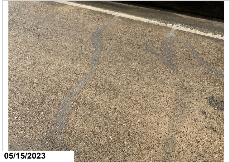
Deck cracking in various locations some sealed some not
