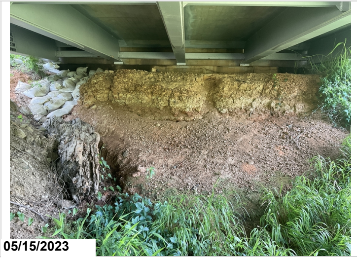
Erosion bent 11
