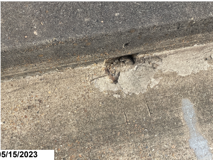
Beginning of span 7 left side drain hole has rebar exposed
