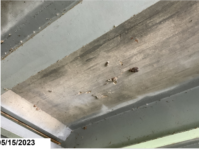
Delam span 3 bay 2
