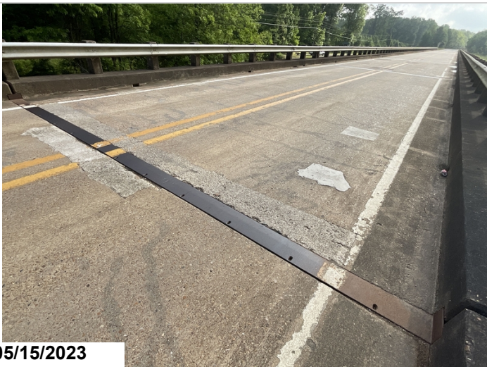
Old patches all across deck surfaces spanning all spans in various locations and sizes
