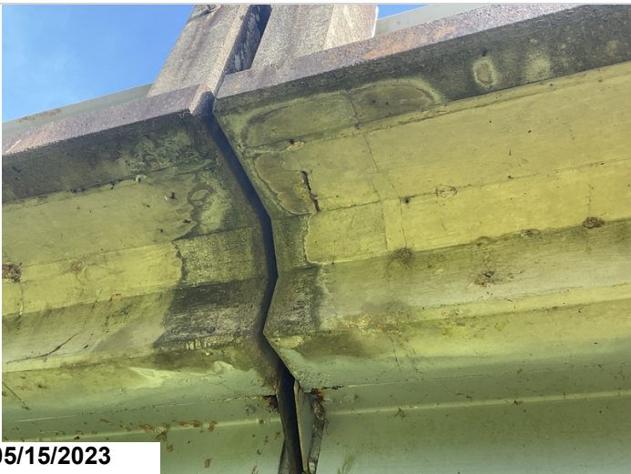
Rebar exposed above bent 2 Rt side span 2
