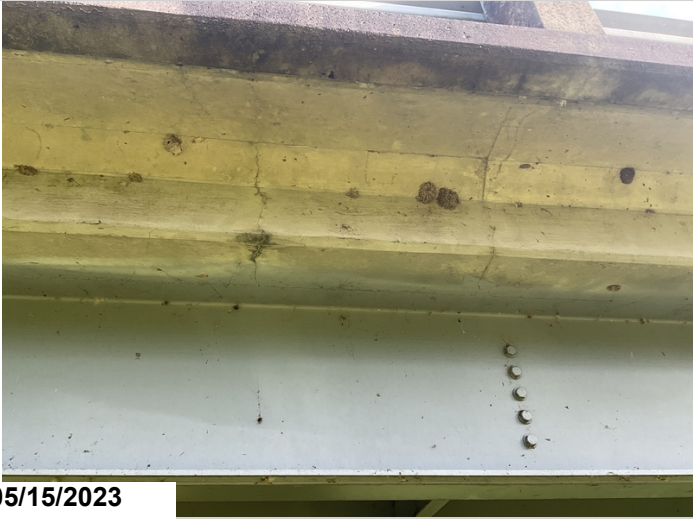
Cracking in deck various locations
