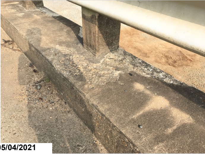
Large Delam right side curb
