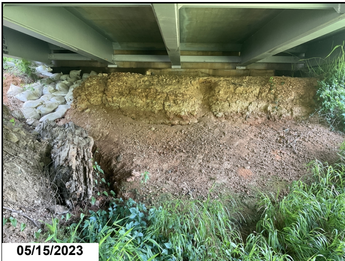
Erosion bent 11
