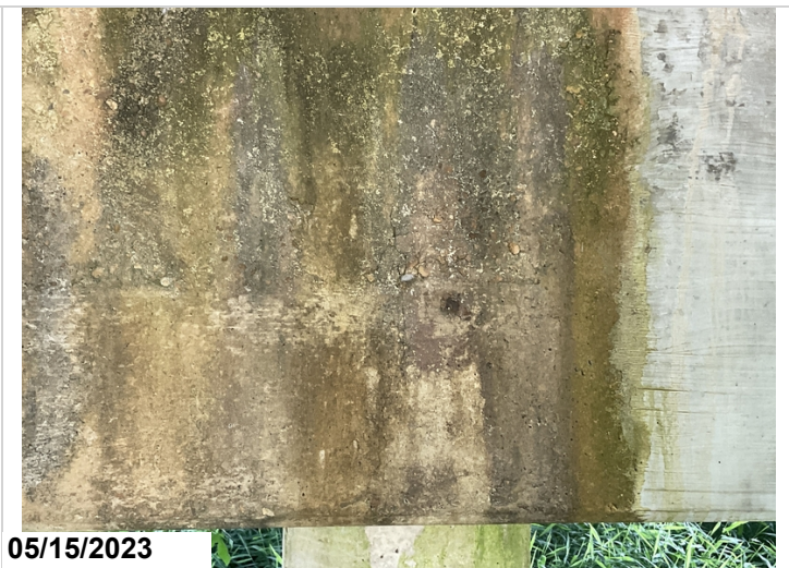
Map like cracking bent 10 span 9 side
