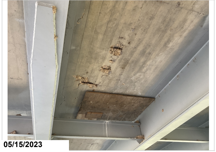
Rebar exposed span 9 bay 2
