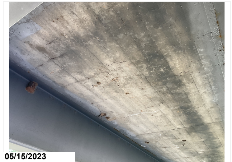
Delam span 9 bay 4
