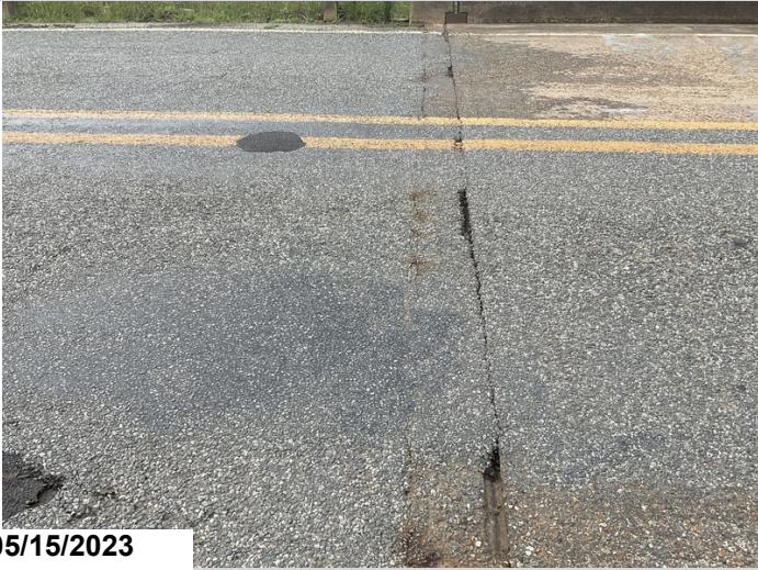
End of bridge debris impaction
