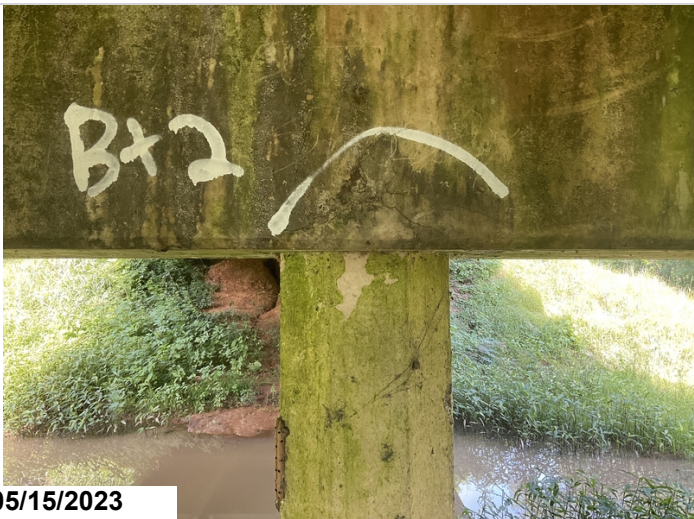
Bent 2 cap delam span 2 side
