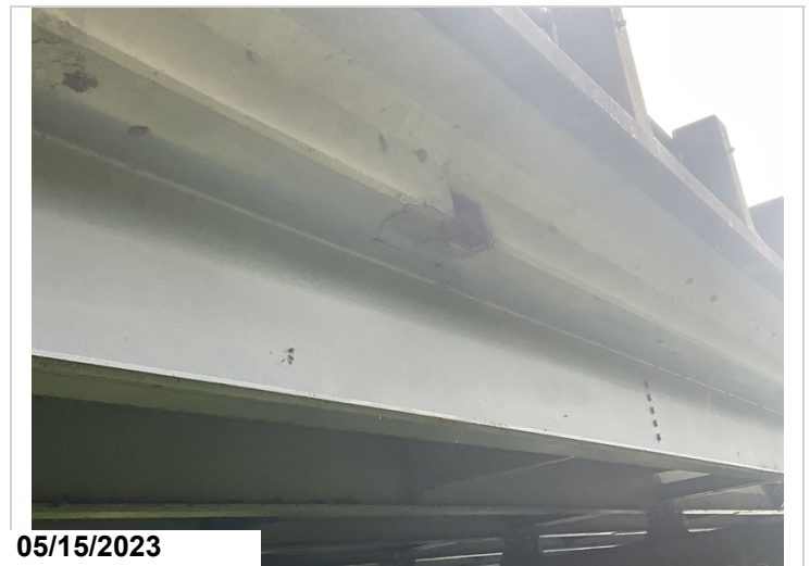
Delam span 2 Rt side by drain hole
