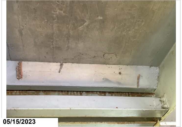
Delam span 2 bay 2
