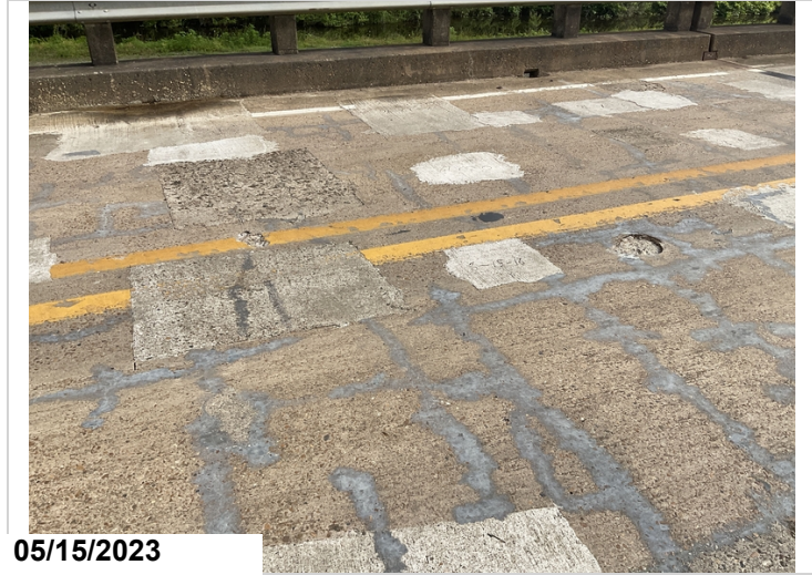
New pop out spall span 9 by yellow line
