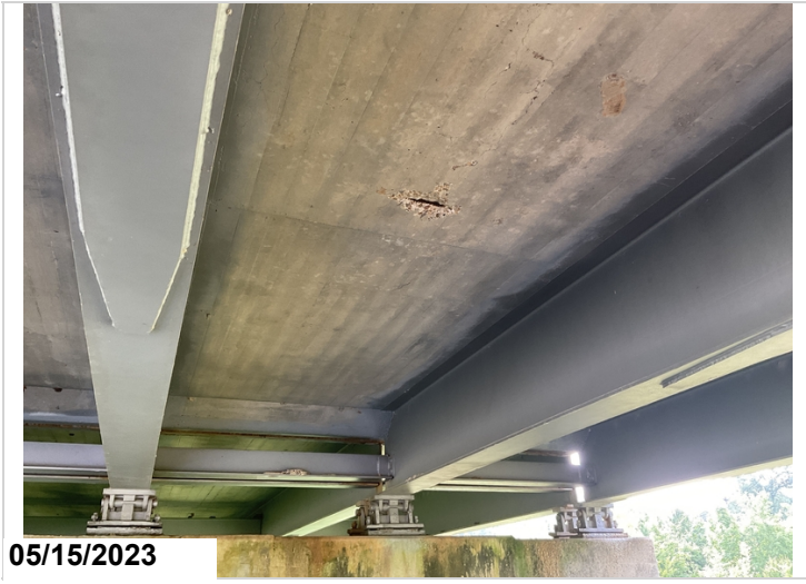
Rebar exposed span 9 bay 3
