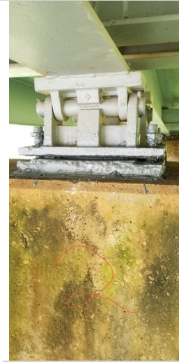
bearings at bent 10 beams 2,3,4 shims were added and painted
