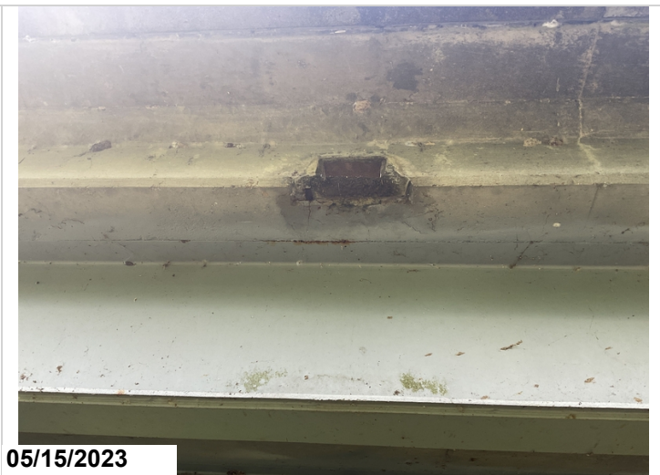
Rebar exposed left side span 2 by drain hole
