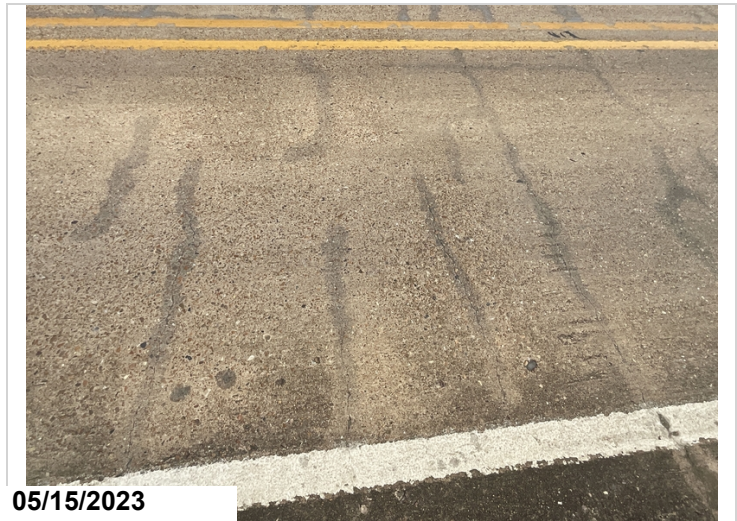
Large amounts of cracking in all spans on bridge deck in various locations some sealed some not sealed.
