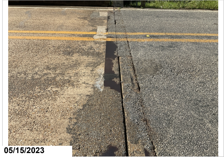
Beginning of bridge debris impaction
