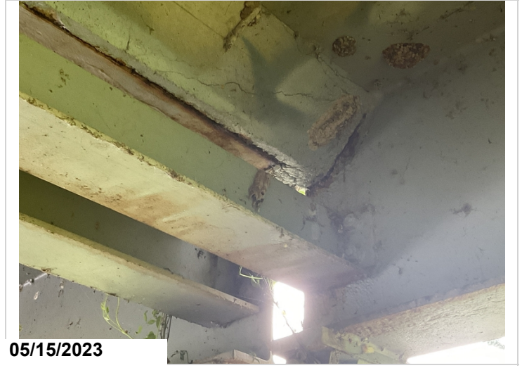
Section loss first 8 in of beam span 2 above bent 3 beam 5
