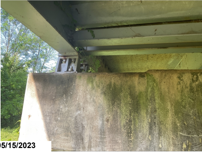
Corrosion beginning on fixed bearings various locations.
