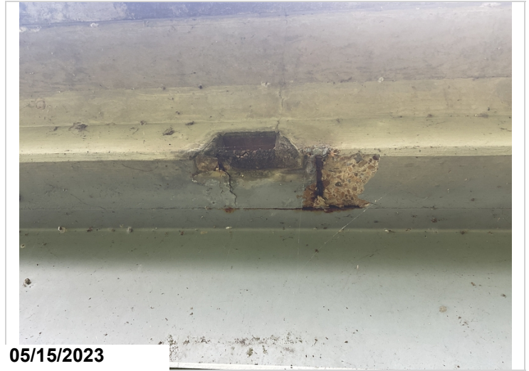
Rebar exposed span 2 left side by drain hole
