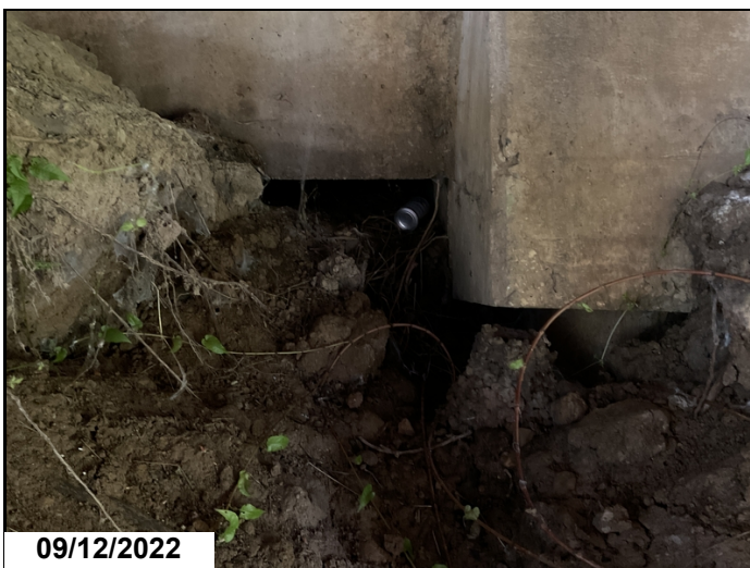
Scour hole leading under abutment 4
