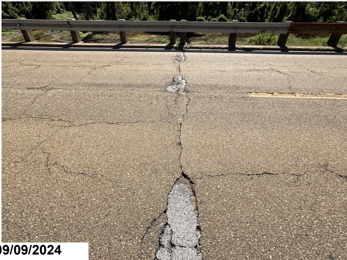
Joints are covered by an asphalt overlay.
