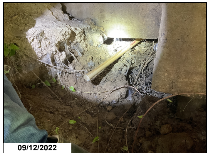
Scour hole leading under abutment 4
