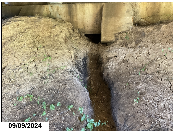
Scour hole leading under abutment 4 9/24
