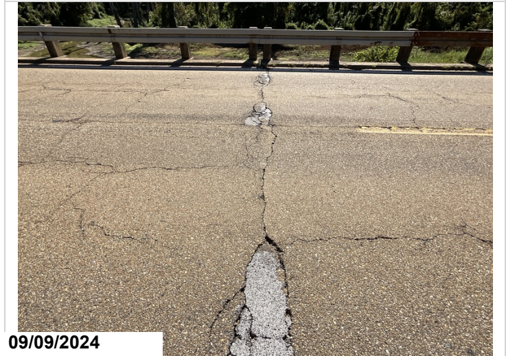
Joints are covered by an asphalt overlay, CS4.
