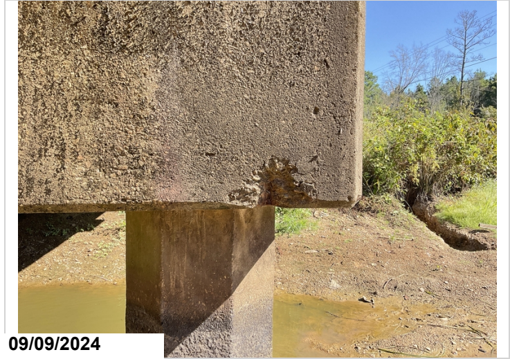
Bent 3, span 2 side, right side, 1' of exposed rebar, CS2.
