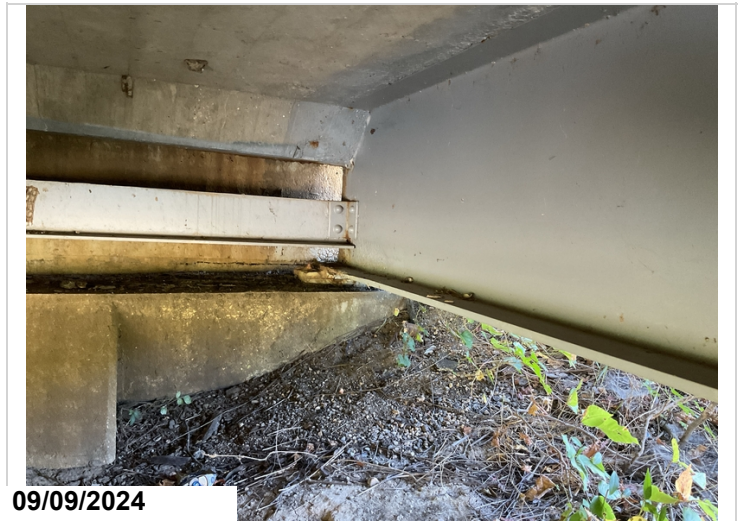
Bent 1, beam 1, left side, 1' of section loss, CS3.
