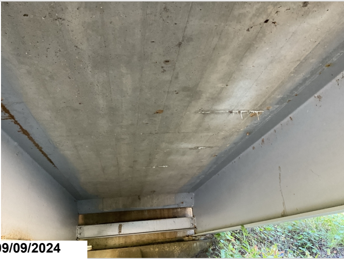
Span 1, between beams 1 & 2, 2' of cracking with efflorescence, CS2.
