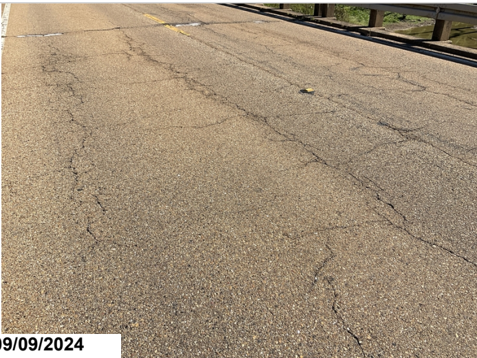
Cracking in all spans of the wearing surface, CS2.
