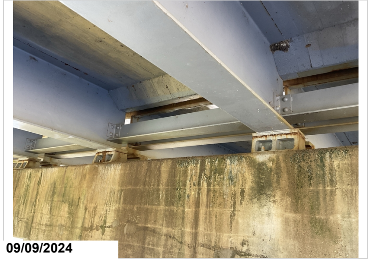
All fixed bearings have minor to moderate corrosion, CS3.
