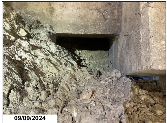
Scour hole leading under abutment 4 9/24
