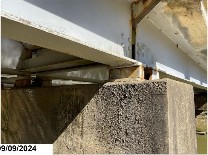
All movable bearings have minor to moderate corrosion, CS3.
