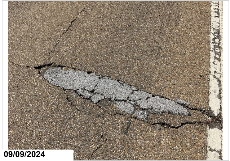
8' total of spalling in the wearing surface in various locations, CS2.
