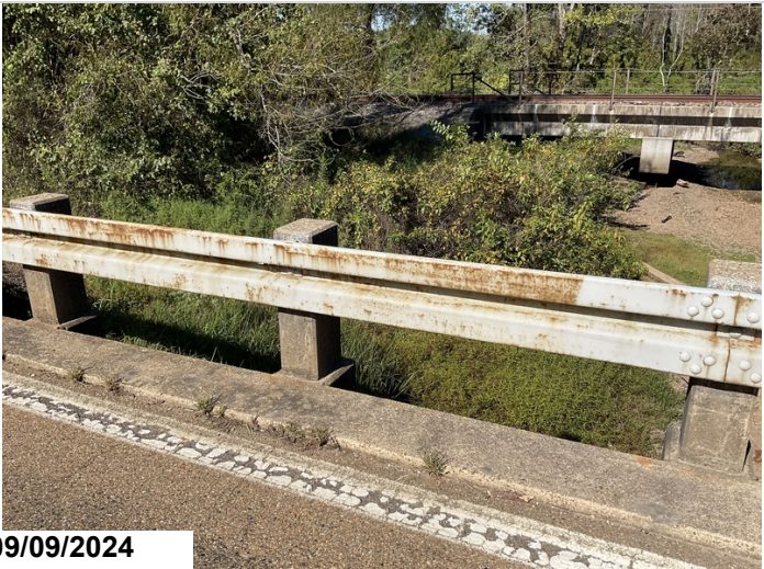
The left and right side of the metal bridge railing has corrosion, CS2.
