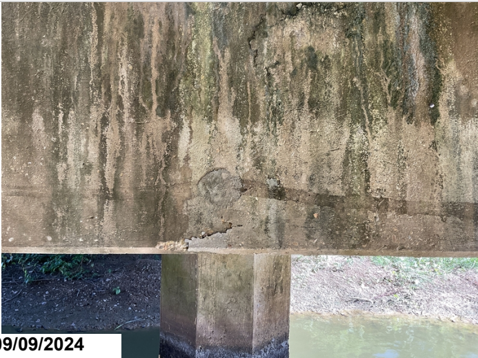
Bent 3, span 2 side, 1' of Delam, CS2.
