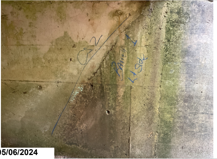
Barrel 1, Outlet end, Cracking, CS2.
