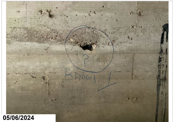
Barrel 1, Lt side spall, CS2.
