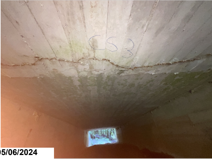
Barrel 1, Efflorescence with rust staining, CS3.
