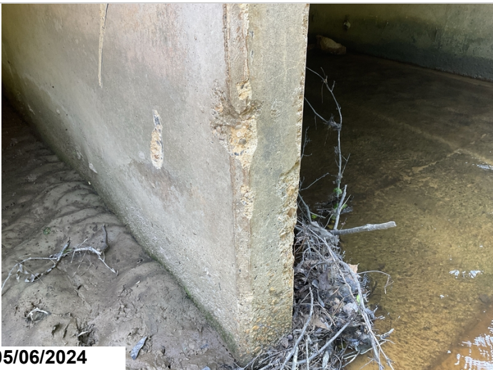
Divider wall, Inlet end, Spalling between barrels 1 & 2. CS2
