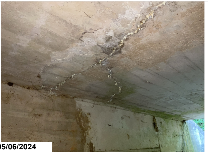
Barrel 1, Efflorescence, CS2.
