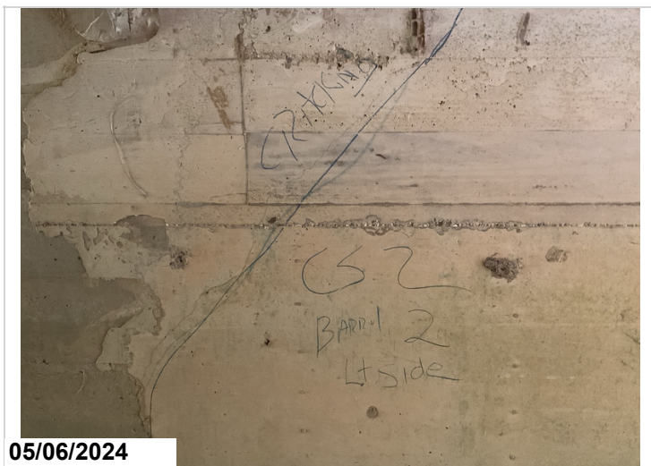
Barrel 2, Cracking, CS2.
