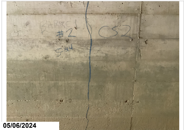
Barrel 2, Cracking, CS2.
