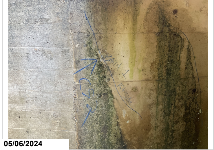
Barrel 1, Rt side, Inlet end, Cracking, CS2.
