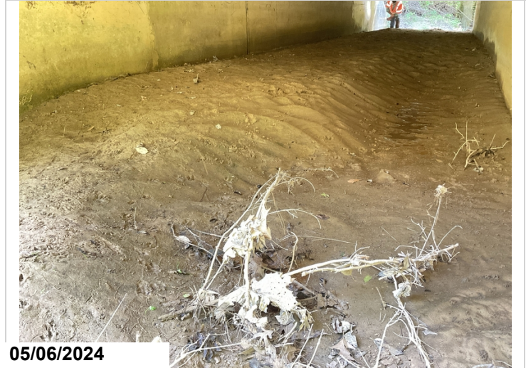
Sediment buildup throughout the entire length of barrel 1 that slightly restricts the channel flow
