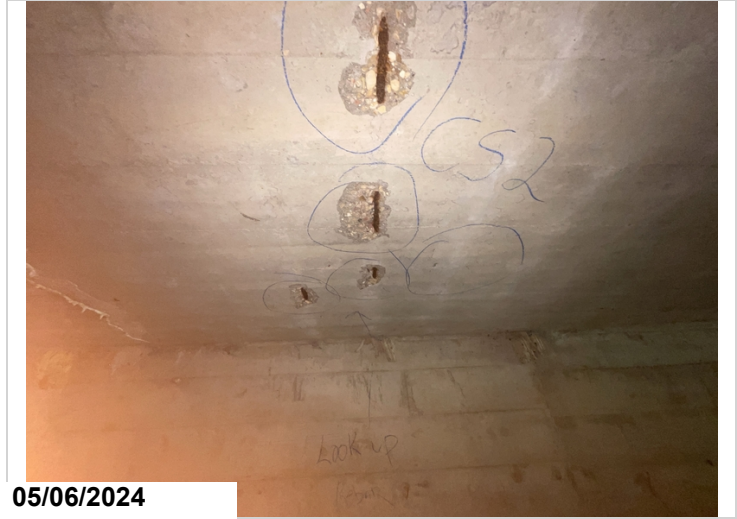
Barrel 1, Exposed rebar with no section loss and delamination, CS2.
