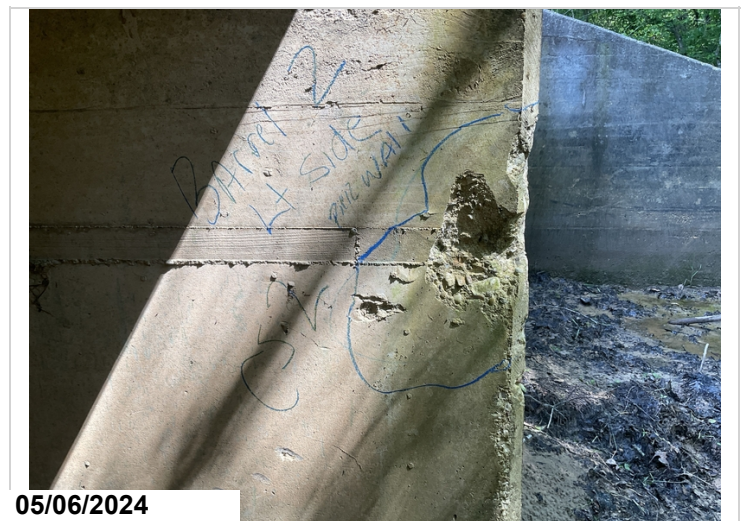
Divider wall, Outlet end, Spalling between barrels 1 & 2. CS2
