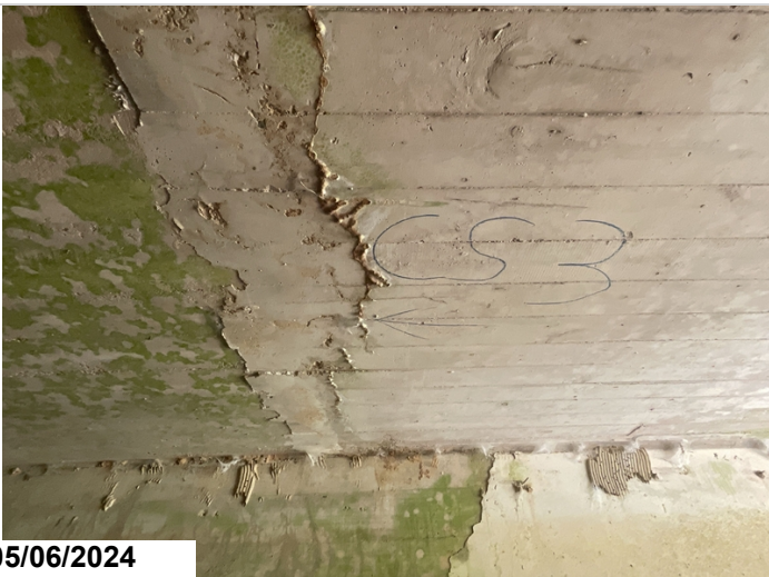
Barrel 2, Efflorescence with rust staining, CS3.
