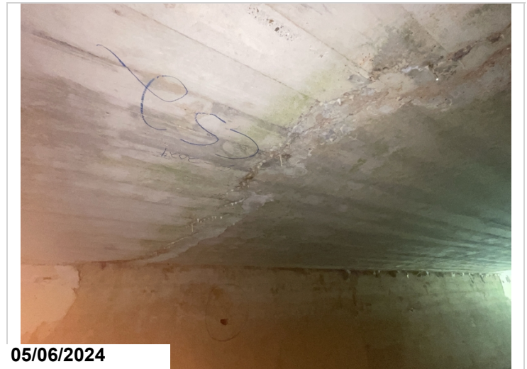
Barrel 2, Efflorescence, CS2.
