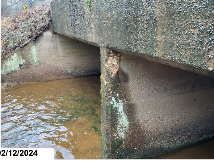
Spall at top of divider wall on outlet end. CS2
