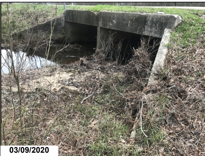
DEBRIS AND SEDIMENT AT INLET OF BOX 1
