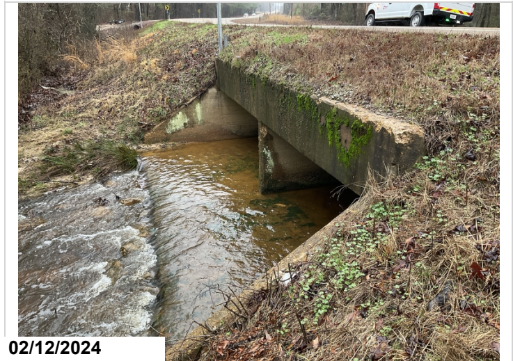
Culvert outlet end
