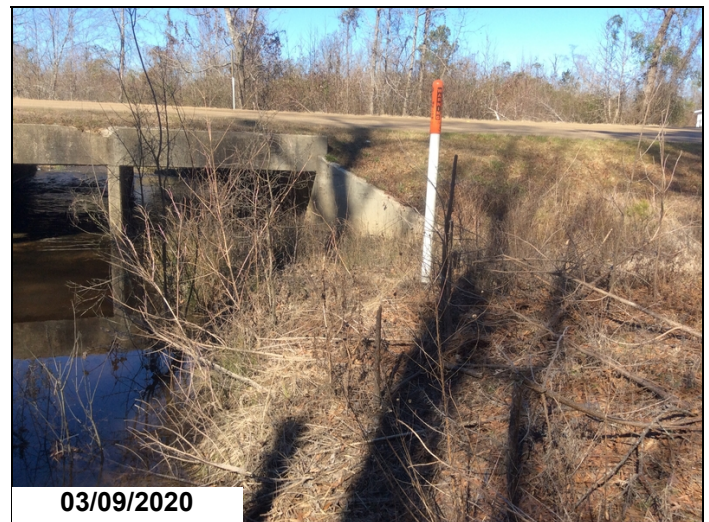
DEBRIS AND SEDIMENT AT INLET AND OUTLET ENDS OF BOX 1
