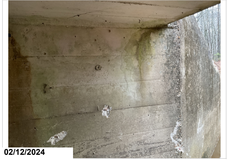
Cracking in barrel 1. CS2
