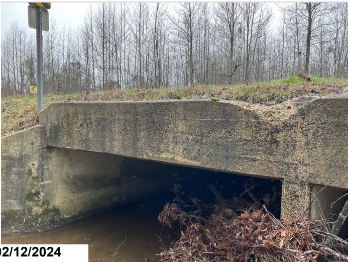
Large spalls on inlet end headwall. CS2
