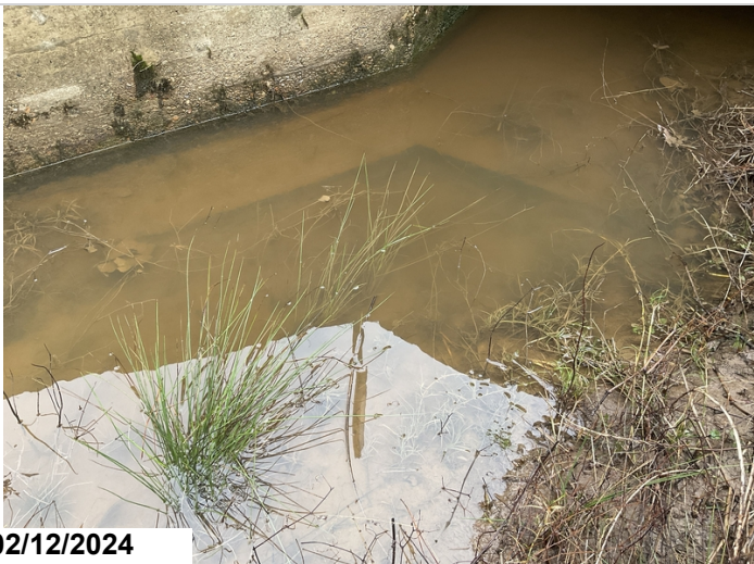
Scour around inlet end footing at both barrels 1 & 2.
