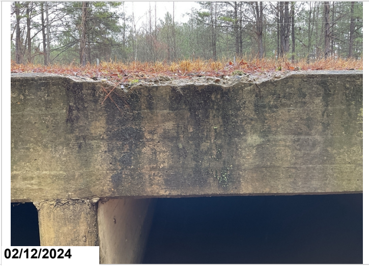
Spalling to headwall on outlet end above barrel 2. CS2
