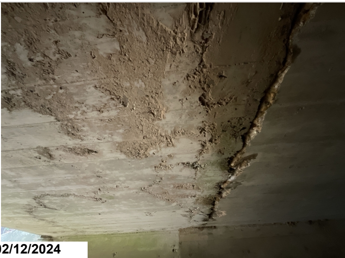
Barrel 1 add on section, honeycombing and spalling. CS2
