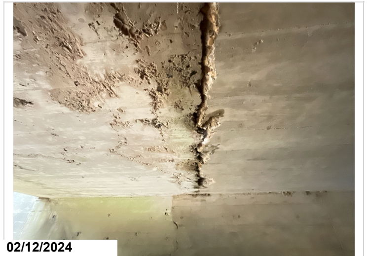
Barrel 1 add on section, honeycombing and spalling. CS2
