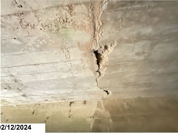
Barrel 2 spalling
