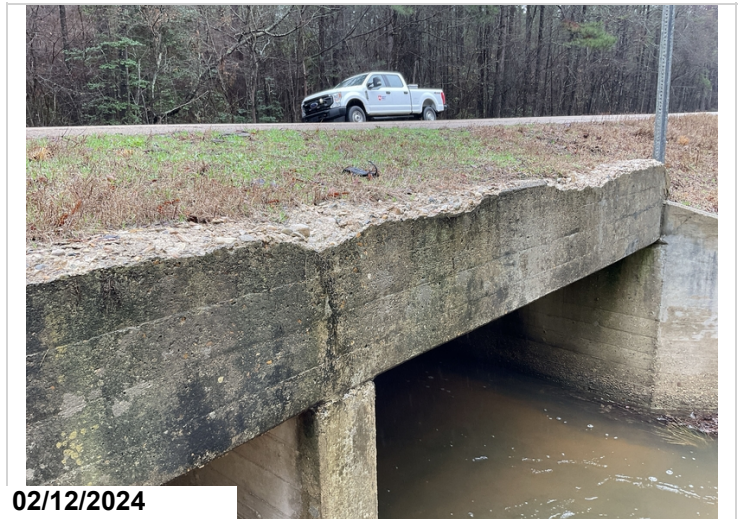
Spalling to inlet end headwall. CS2
