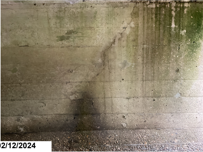
Typical cracking throughout both barrels. CS2
