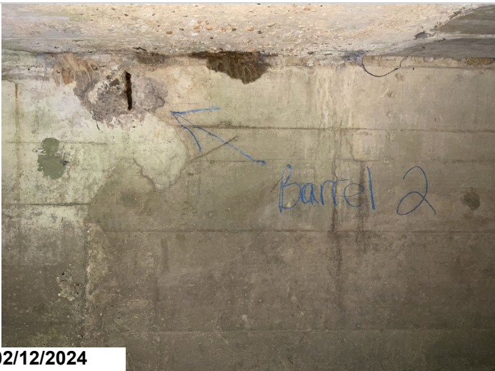
Barrel 2 exposed rebar. CS2
