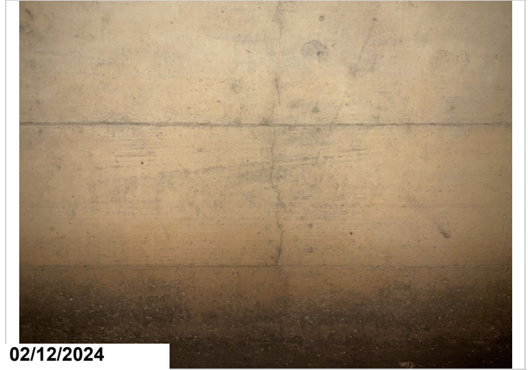
Typical cracking throughout both barrels. CS2
