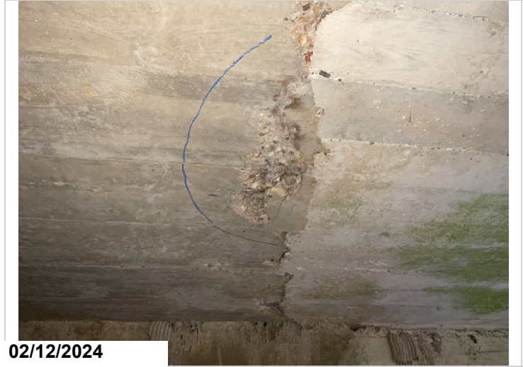
Spalling in barrel 2. CS3
