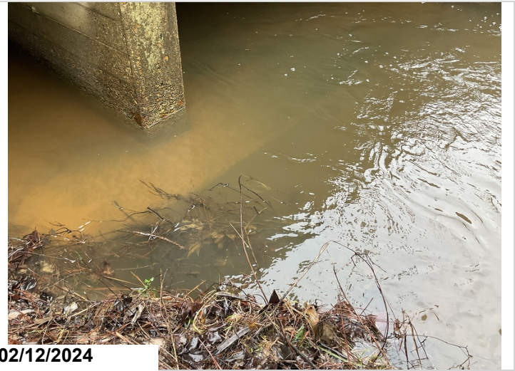
Scour around inlet end footing at both barrels 1 & 2.
