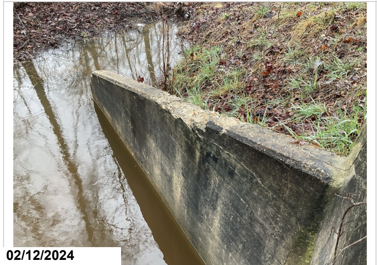
Salt damage barrel 2 LT side wingwall, approx. 3' long.
