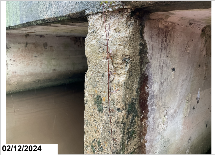
Spalling on inlet end divider wall. CS2
