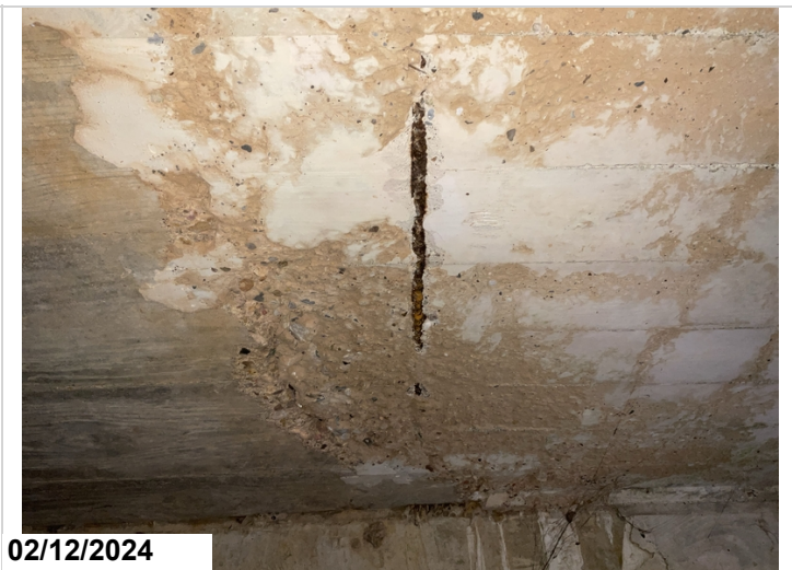
Exposed rebar to top of barrel 1 near inlet end, 2 LF no section loss CS2.
