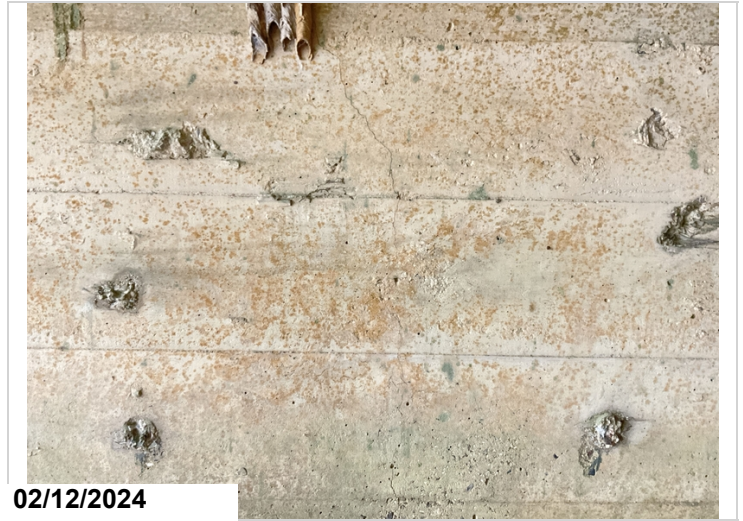
Cracking throughout both barrels 1 & 2. CS2
