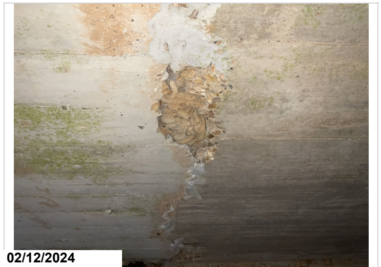
Spalling to barrel 1 ceiling, 1 LF CS2.
