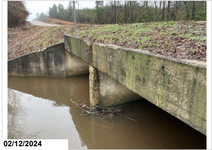
LT side upstream headwall spalling, 5 LF CS2
