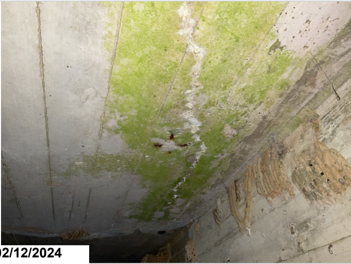
Barrel 1 efflorescence. CS2
