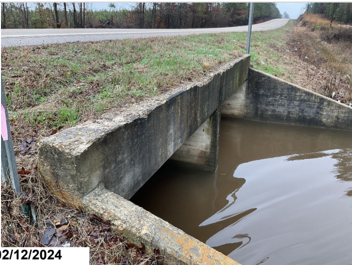
Outlet end headwall spalling, 5 LF CS2
