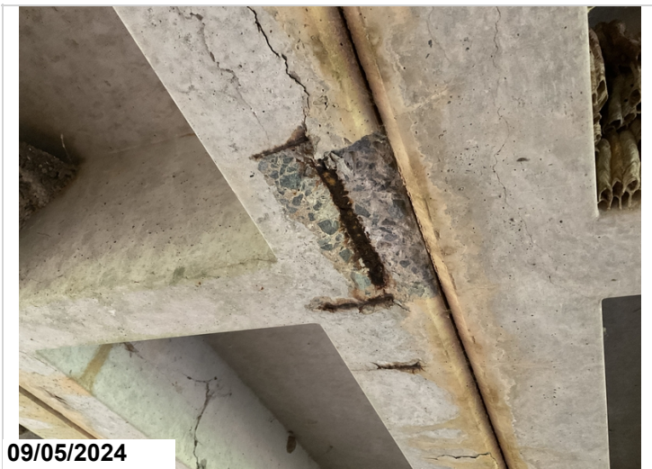
Span 2, Unit 3, Exposed rebar, CS2
