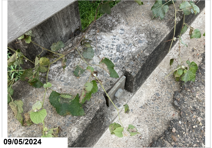
Concrete bridge railing, Both Rt and Lt sides, Spalling, CS2
