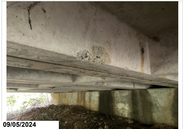
Span 1, Minor spalling, CS2
