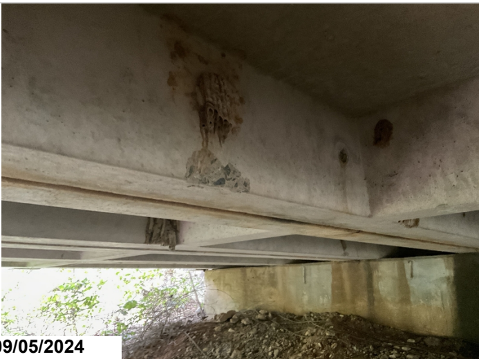
Span 1, Minor spalling, CS2
