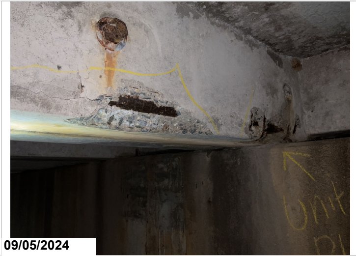
Span 3, Unit 4, Exposed rebar, CS3
