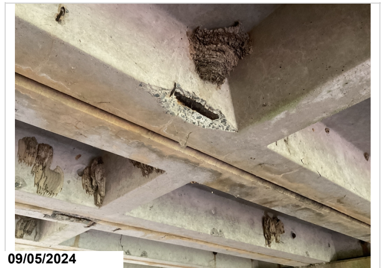
Span 2, Unit 5, Exposed rebar, CS2
