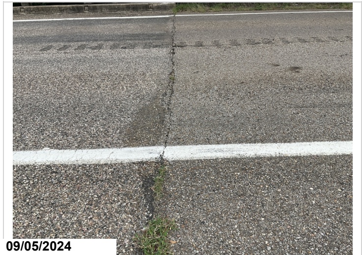
Wearing surface, Bent 4, Cracking, CS2
