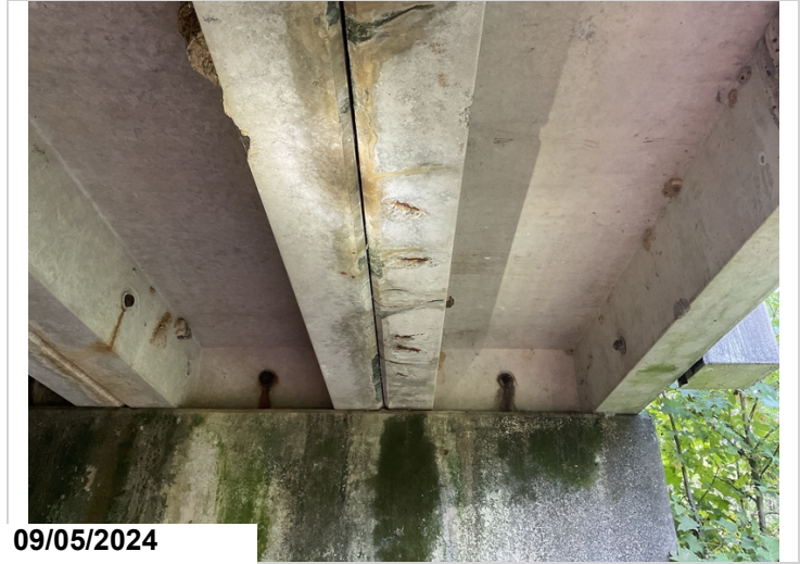
Span 2, Unit 10, Exposed rebar, CS2
