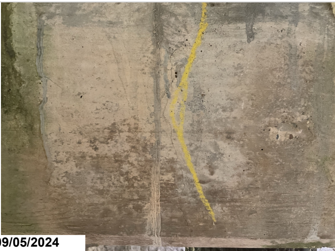
Bent 2, Looking back, Cracking, CS2
