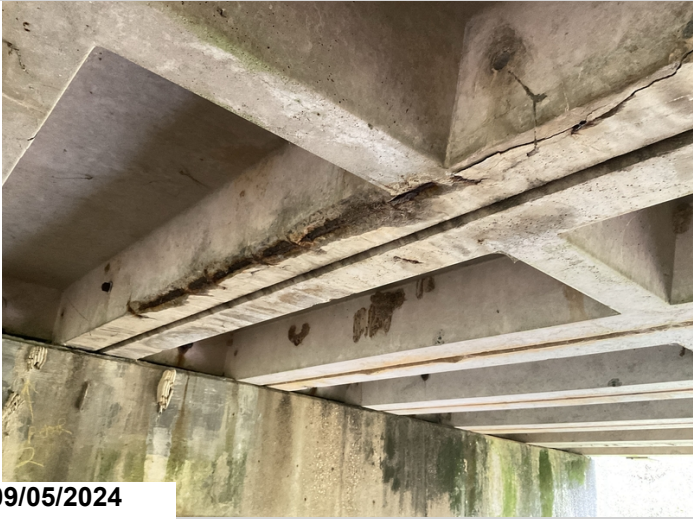
Span 2, Unit 5, Exposed rebar, CS3
