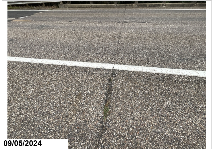
Joint filled by asphalt overlay impacting joint movement
