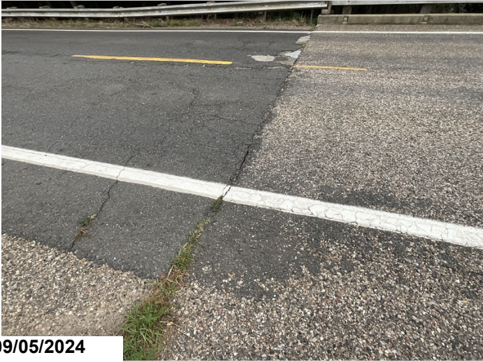
Wearing surface, Bent 1, Cracking, CS2
