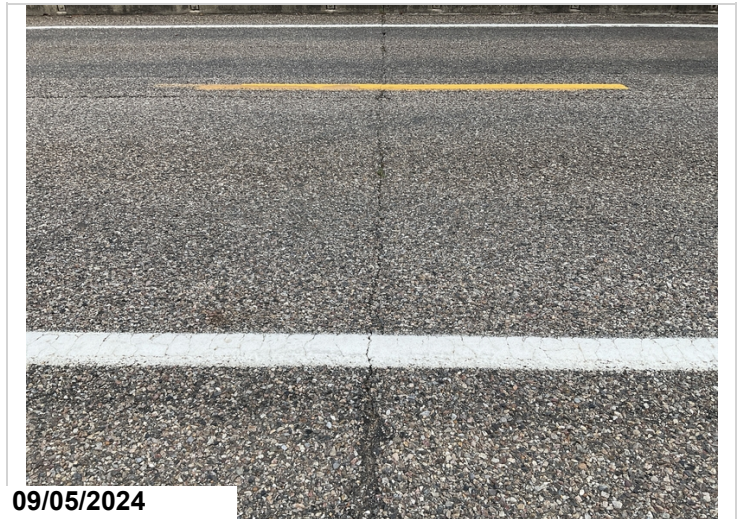
Pourable joint seal, Bent 3, Debris impaction, CS4
