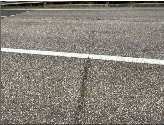
Joint filled by asphalt overlay impacting joint movement
