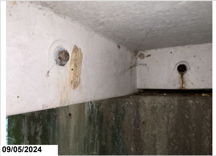
Precast units are bolted together
