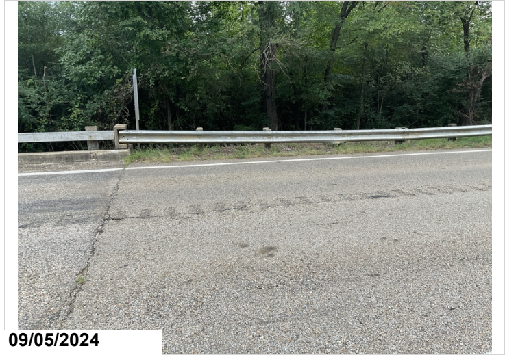
Bridge railing transition
