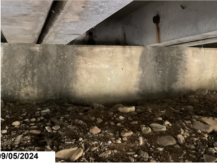
Bent 4, Looking ahead, Linear cracking under unit 5, CS2
