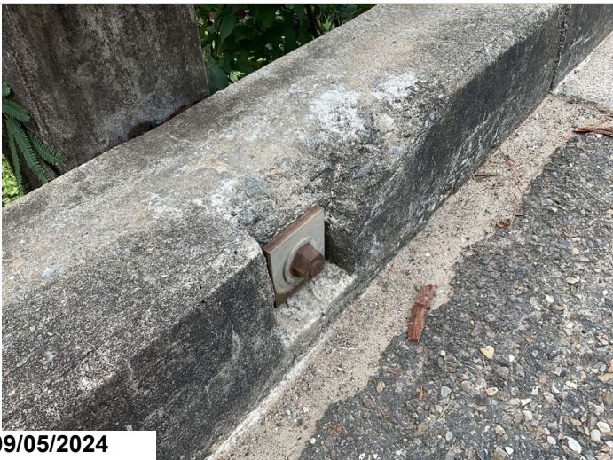
Concrete bridge railing, Both Rt and Lt sides, Spalling, CS2
