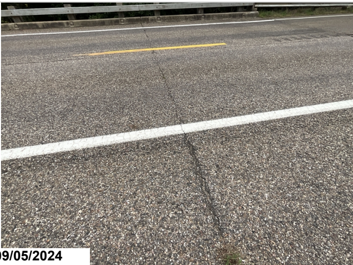
Wearing surface, Bent 3, Cracking, CS2
