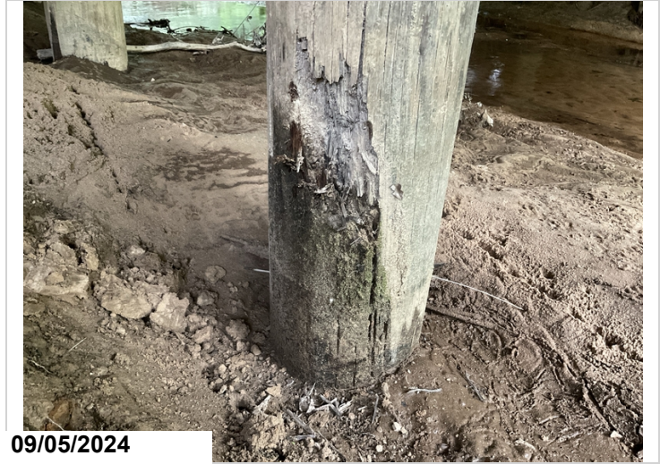
Bent 2, Pile 5, Decay, CS2
