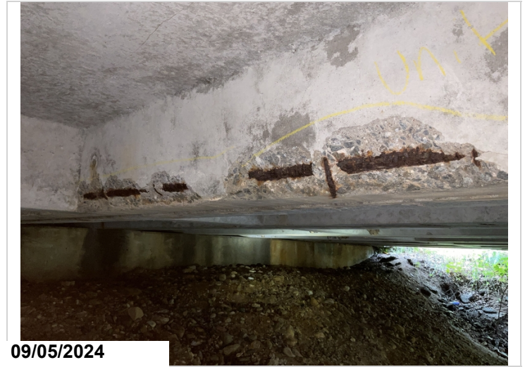
Span 3, Unit 4, Exposed rebar, CS3
