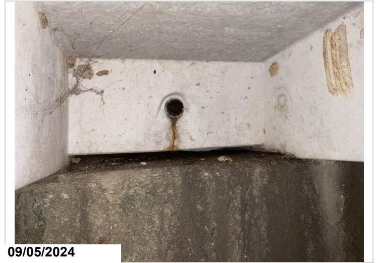
Precast units are bolted together
