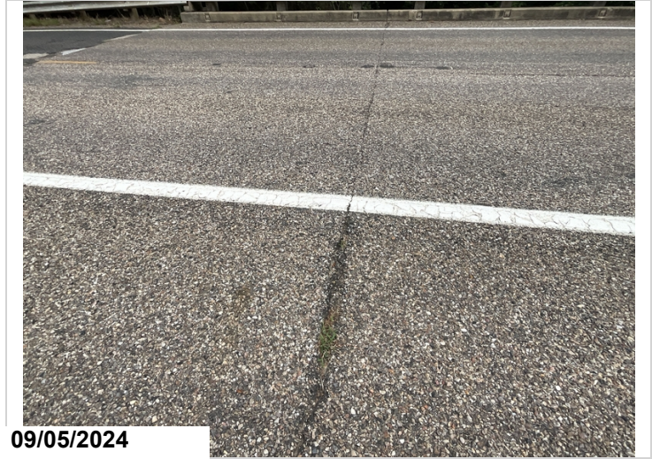
Wearing surface, Bent 2, Cracking, CS2
