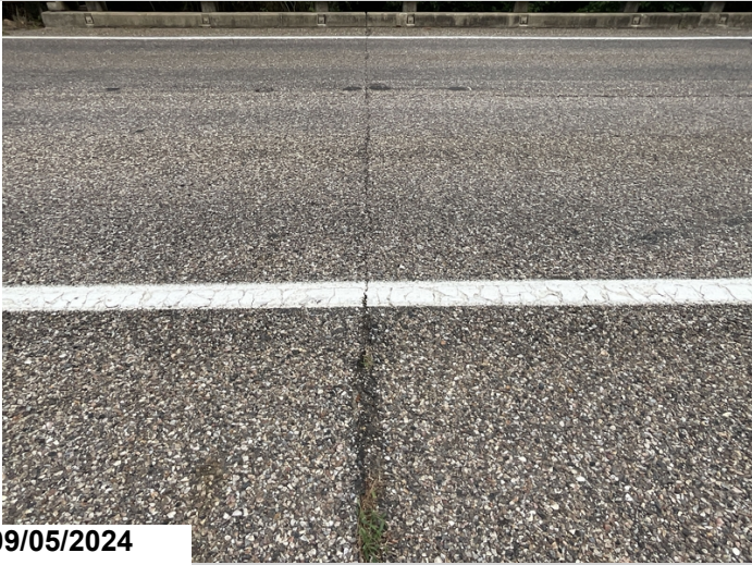
Pourable joint seal, Bent 2, Debris impaction, CS4
