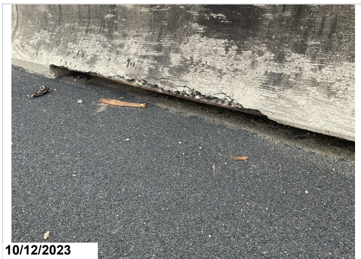
2023 small spalls in parapet wall photo taken right side span 4. Approach span
