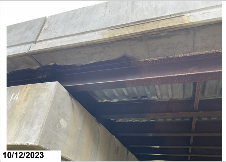
Typical painted beam ends.
