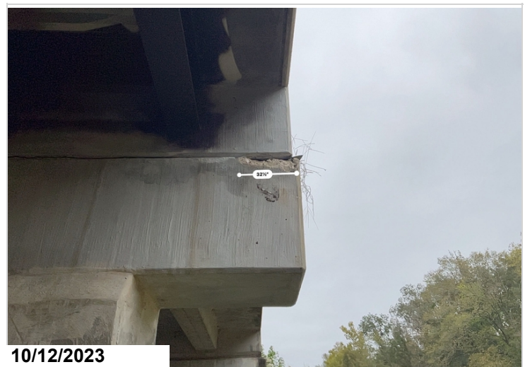
Bent 15 back, right edge, spall in the top of the cap.
