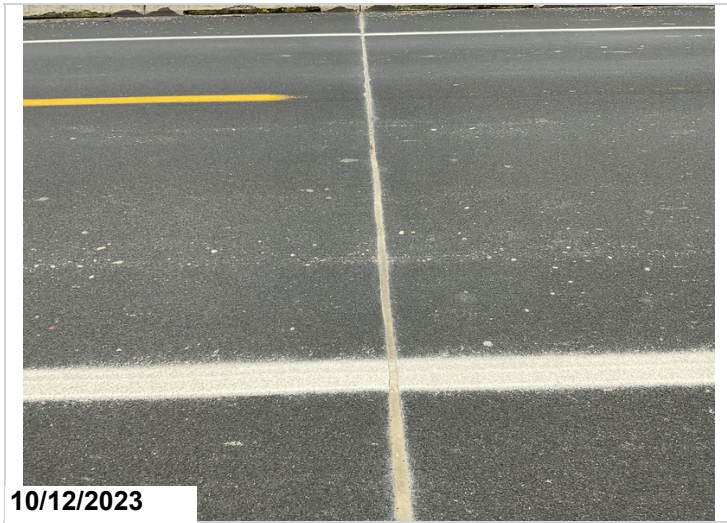
Approach span joints
