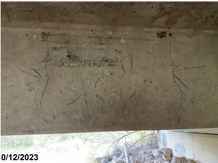
Span 17, girder 2 right side, minor cracks.
