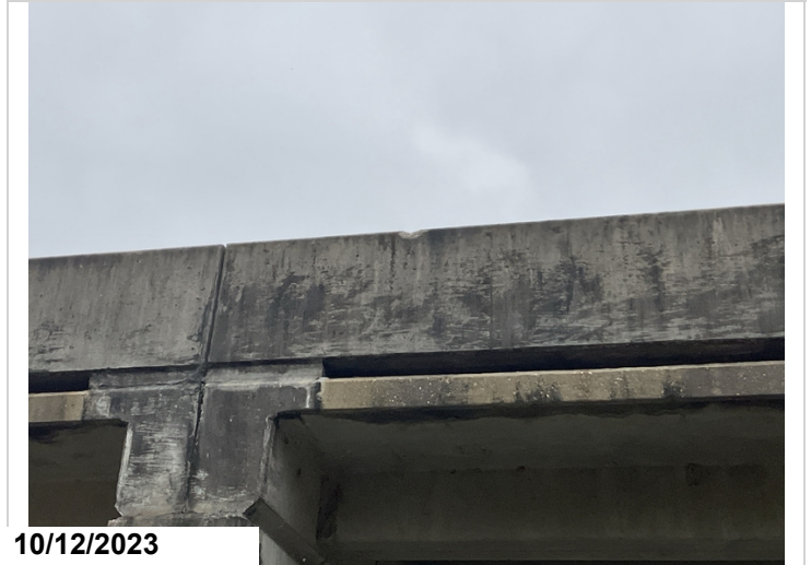
Span 3, right bridge rail, spall on the top of the rail.
