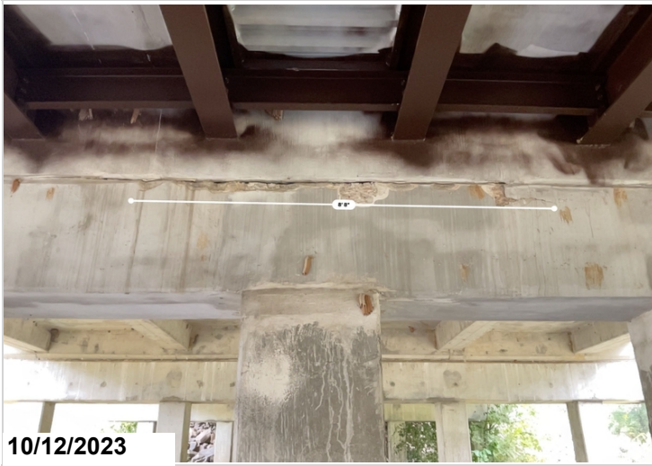
Bent 15 back, large spalls at the top of the cap above pile 3.
