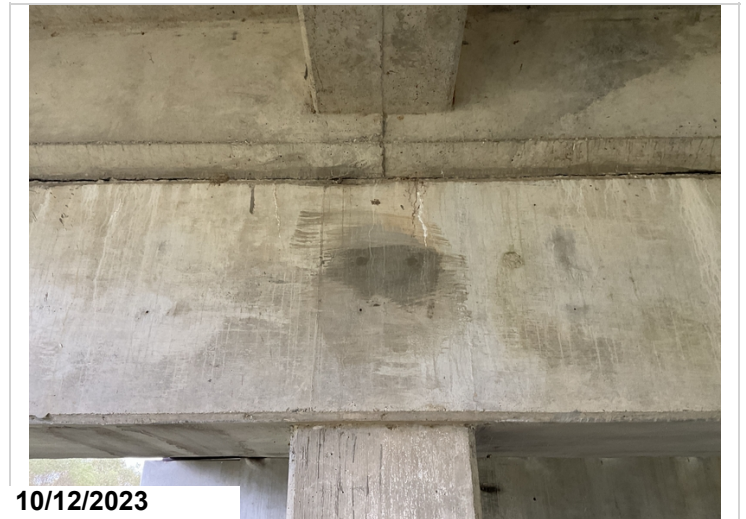
Bent 9 back, above pile 2, cracks with efflorescence in the cap.
