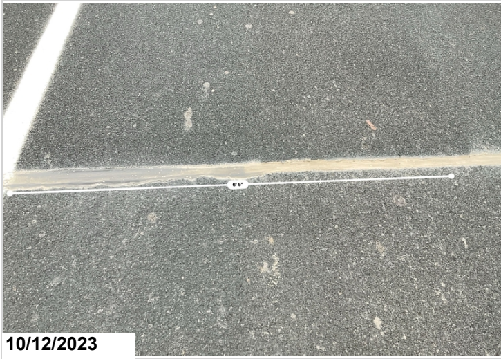
Joint coming loose from edges joint 8
