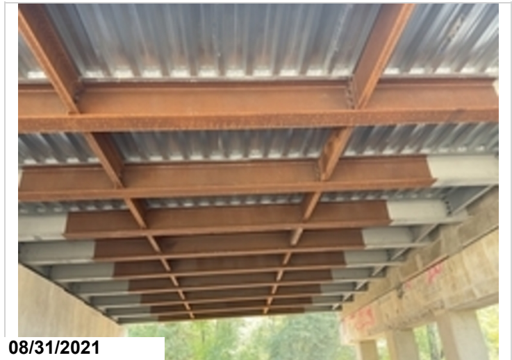
08/2021 repairs were made on job # 030458 steel beams span 9-14
