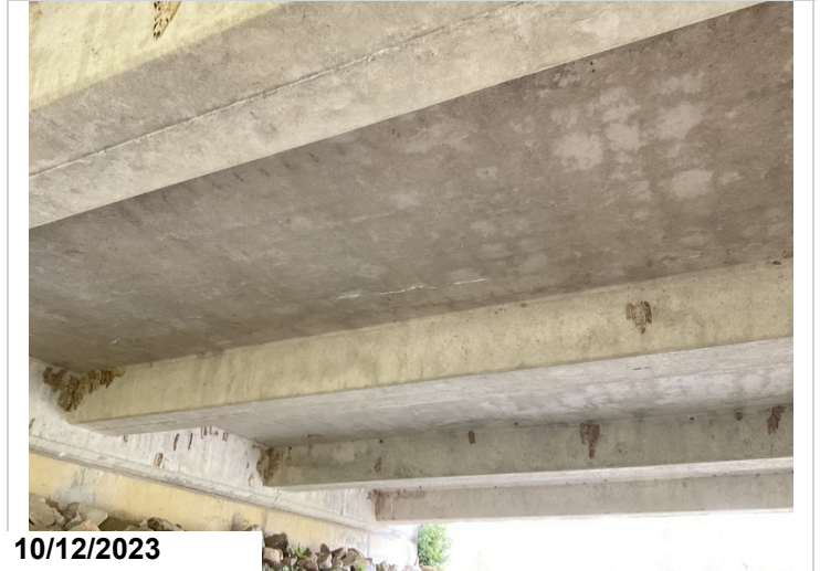
Bay 3 span 1 efflorescence
