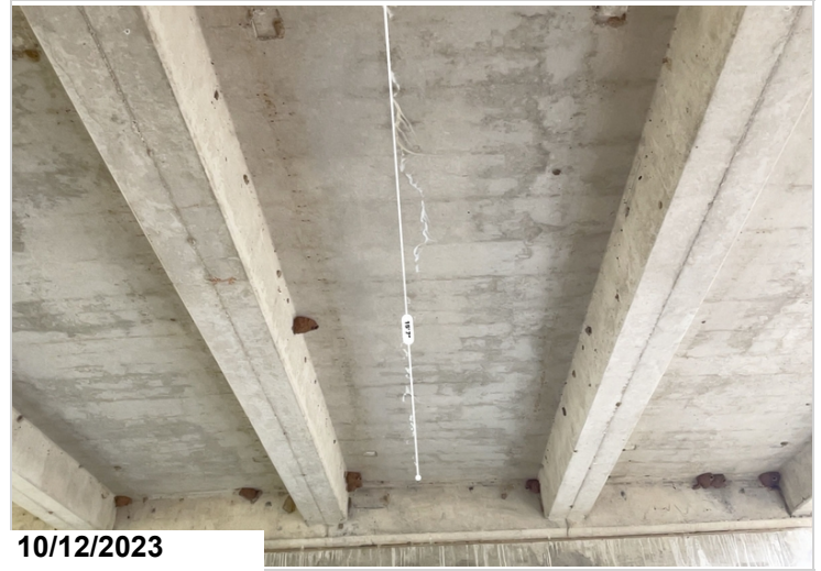
Span 5, bay 2, typical longitudinal crack with efflorescence.
