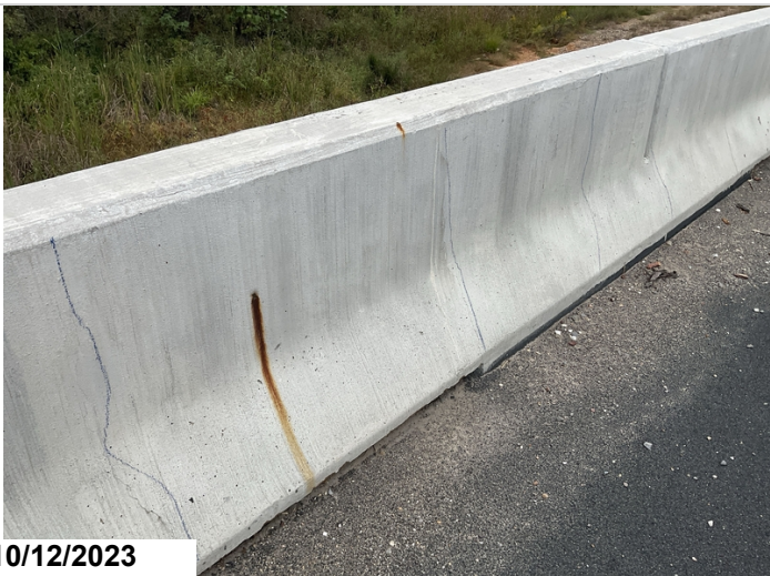
Minor cracks in parapet wall main-span
