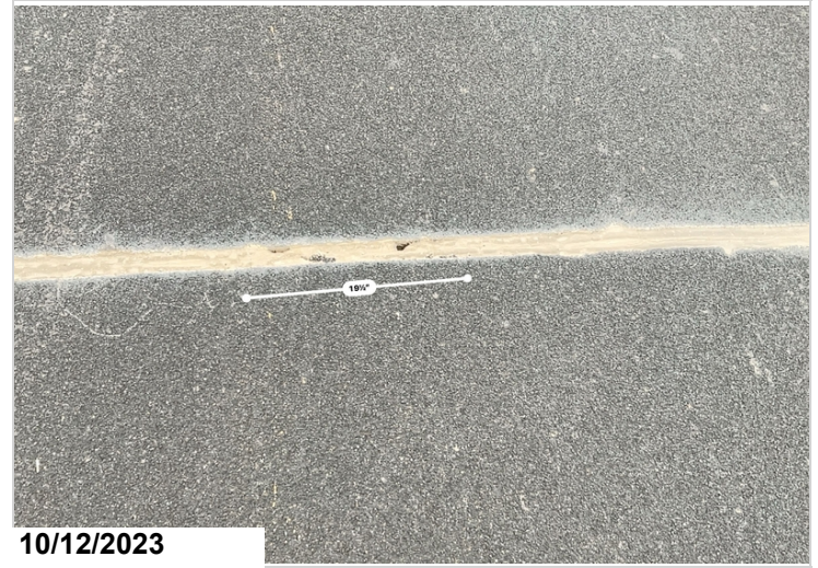
Main span joint with small hole. Joint 8
