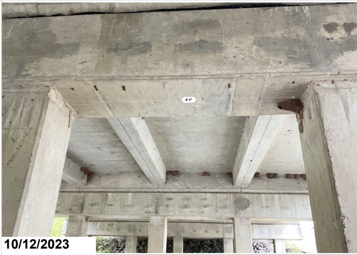
Bent 4, bottom of cap between pile 2 and 3, exposed rebar.
