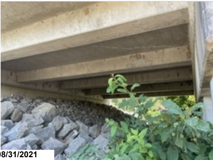
end bridge abutment with riprap on slope
