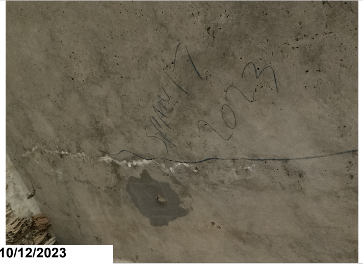
Span 17, bay 3 near bent 18, crack with efflorescence in the under surface.
