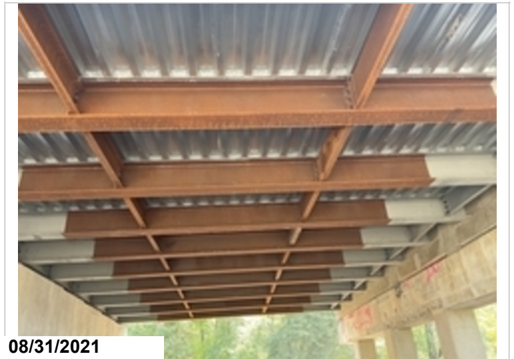
steel beams in main span
