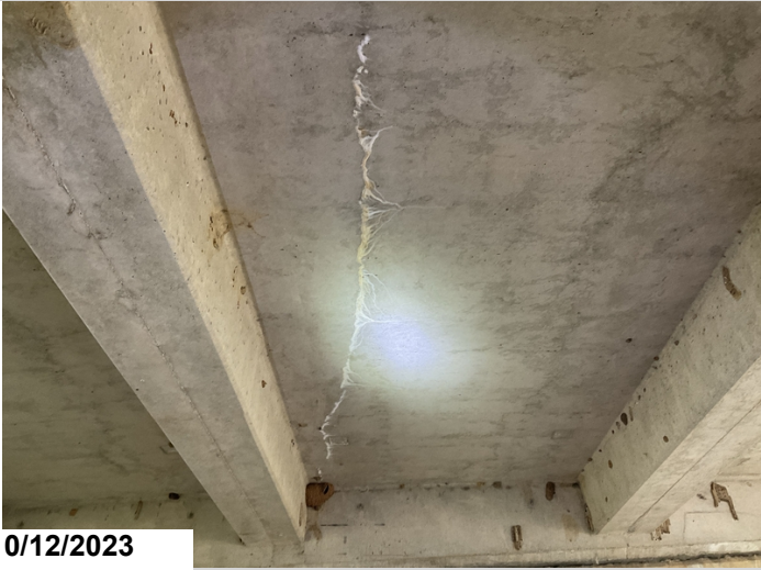
Span 16, bay 2, crack with efflorescence in the under surface.
