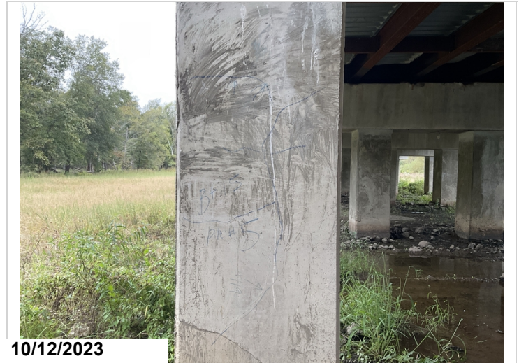
Bent 15, pile 5 ahead, cracks in the concrete encasement. Typical.
