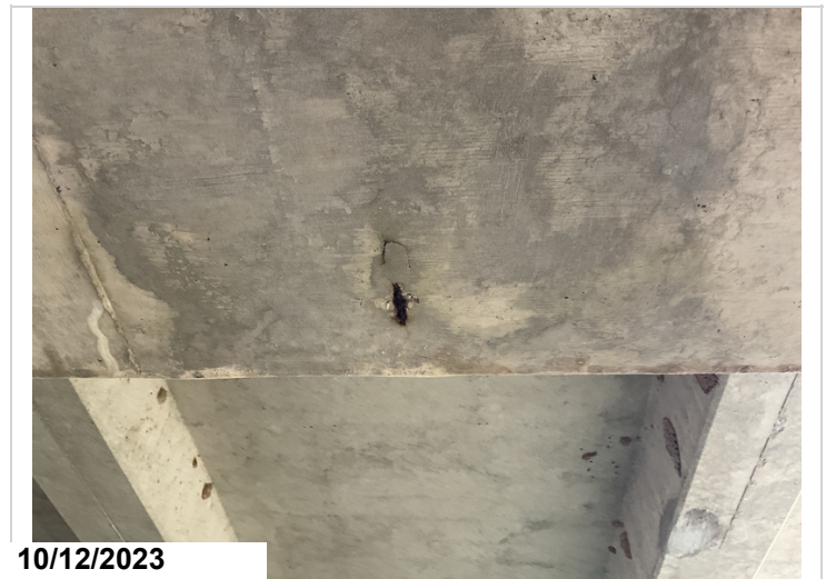
Bent 16, bottom between pile 3 and 4, exposed rebar.
