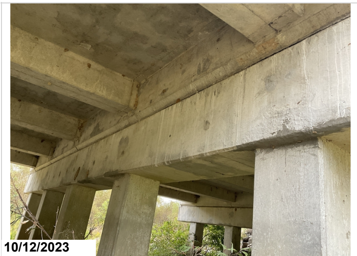
Bent 16, back side of cap, patches above pile.
