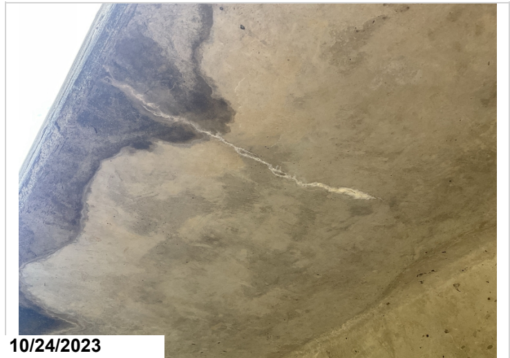
Efflorescence on bottom of deck.
