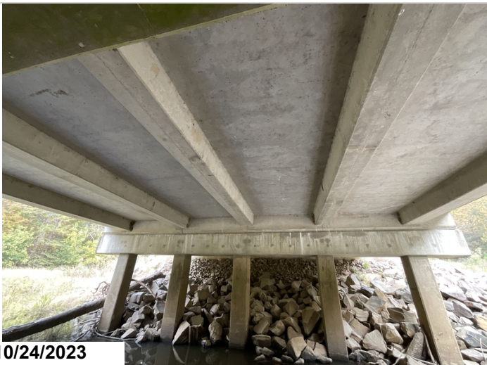
Photo taking in span 2 Superstructure in good condition. Minor cracking in concrete T Beam.
