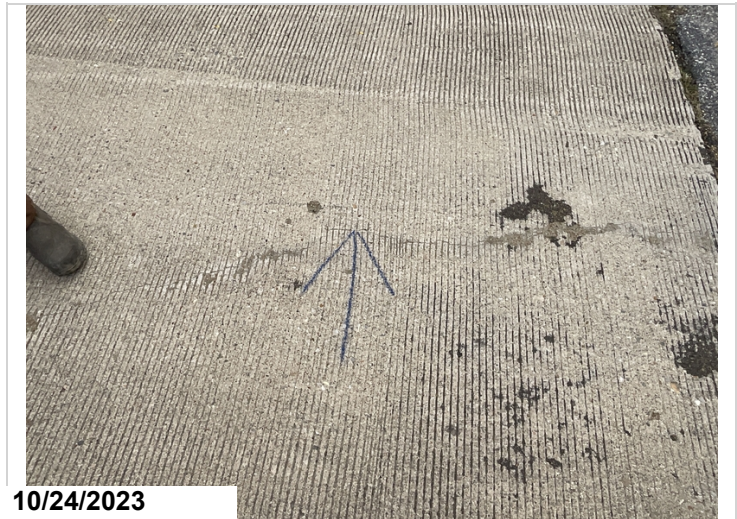
Cracks in the deck.
