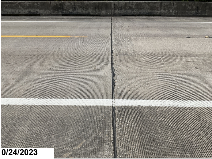
Joint seal in satisfactory condition.
