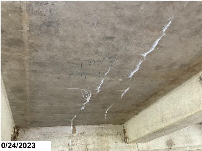
Span 3 bay 2 efflorescence with minor rusting.
