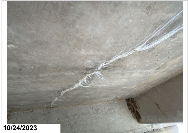
Span 3 at bay 4 efflorescence on bottom of deck.
