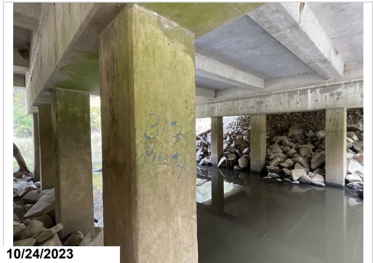
Bent 2 pile 4 concrete encasement in good condition.
