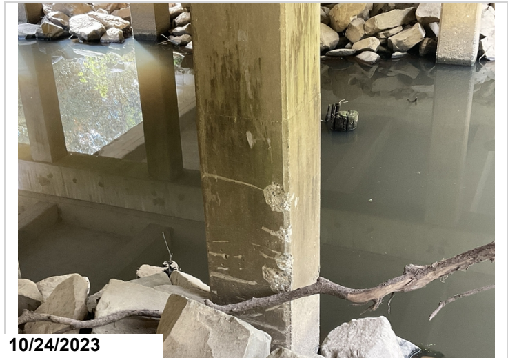
Bent 3 pile 2 minor spalling on concrete encasement.
