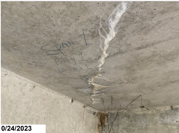
Span 1 bay 1,2,3,4 Efflorescence with rusting.
