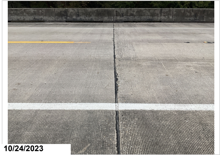
Joint condition in satisfactory condition at bent 2 and 3.
