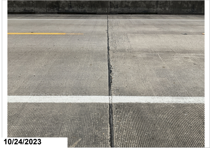
Joint seal at bent 2 & 3 are in satisfactory condition.
