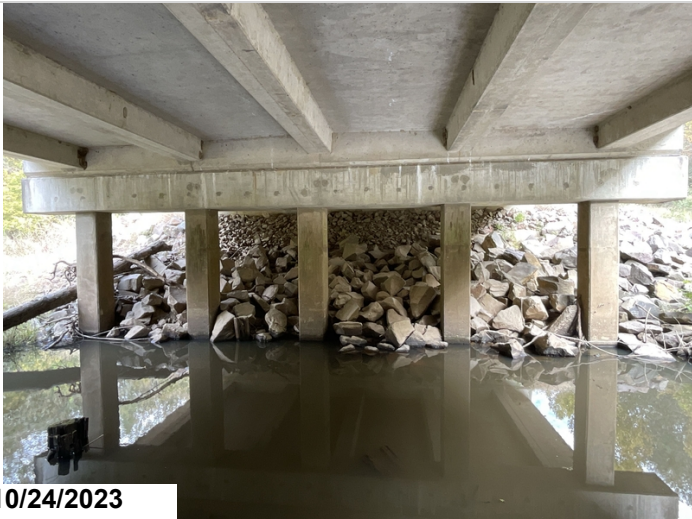
Bent 3 in very good conditions.
