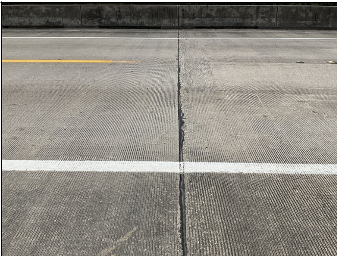
Joint seal in satisfactory condition.
