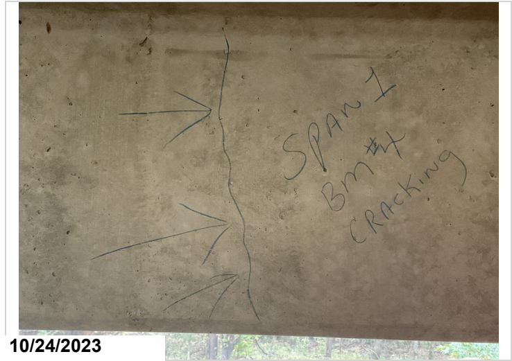
Span 1 beam 4 minor cracking in concrete.
