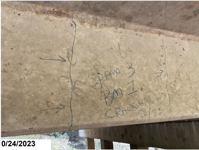
Beam 1 span 3. Minor cracking.
