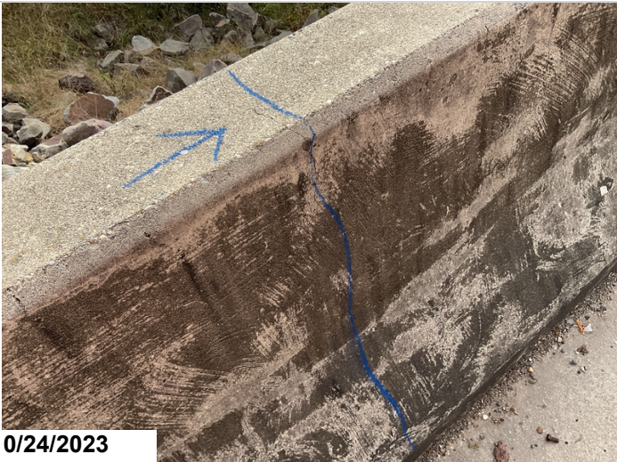
Cracking in concrete railing
