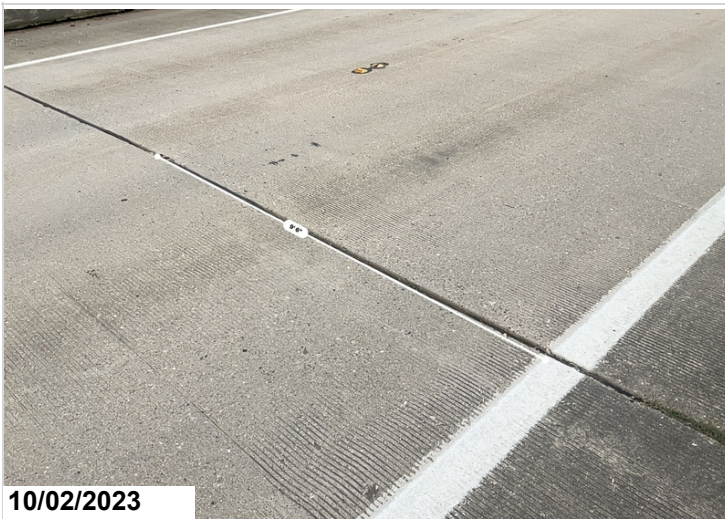
Joint 7 around 9 ft joint missing
