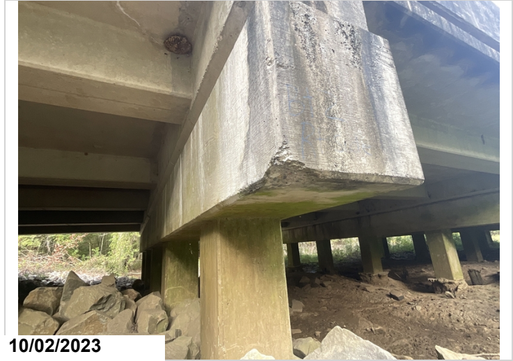
Bent 2 cap right side bottom of cap on end small spall.
