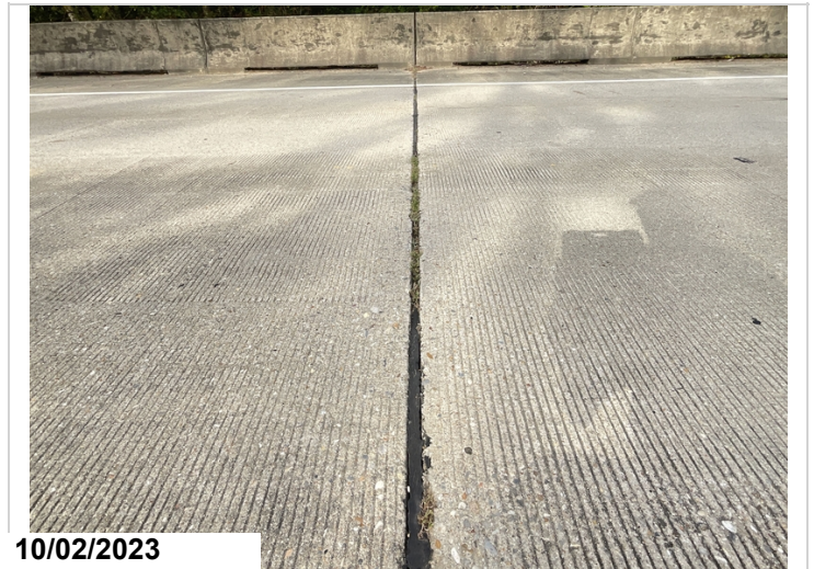
Joint 4 part of poured joint missing with grass growing in joint line
