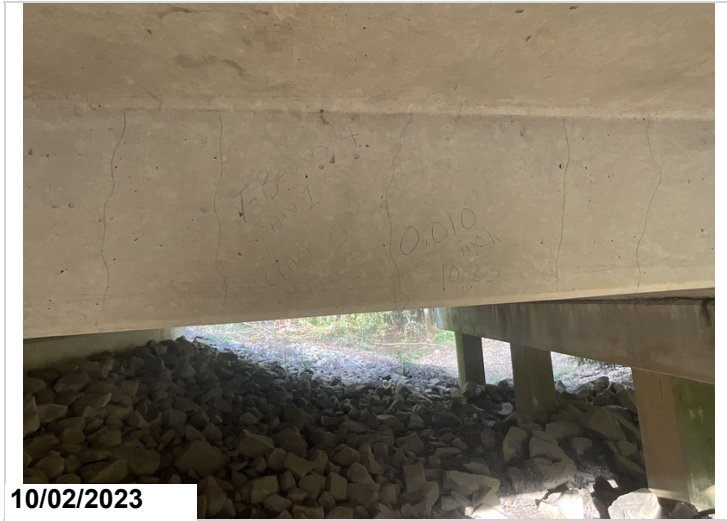
Span 1 light cracking in concrete tee beams size 0.010 photo of beam 4
