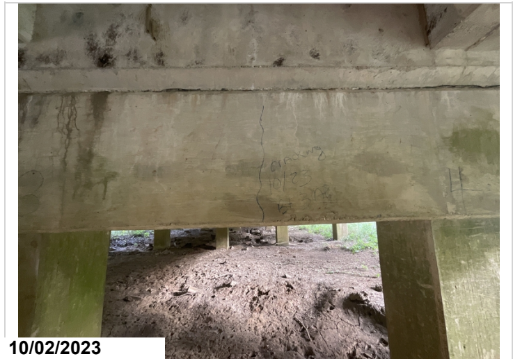
Bent 3 light cracking in cap between piles 3 and 4 span 2 side.
