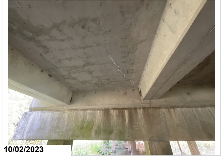
Span 5 efflorescence in bottom of deck bay 1 at bent 6 area.
