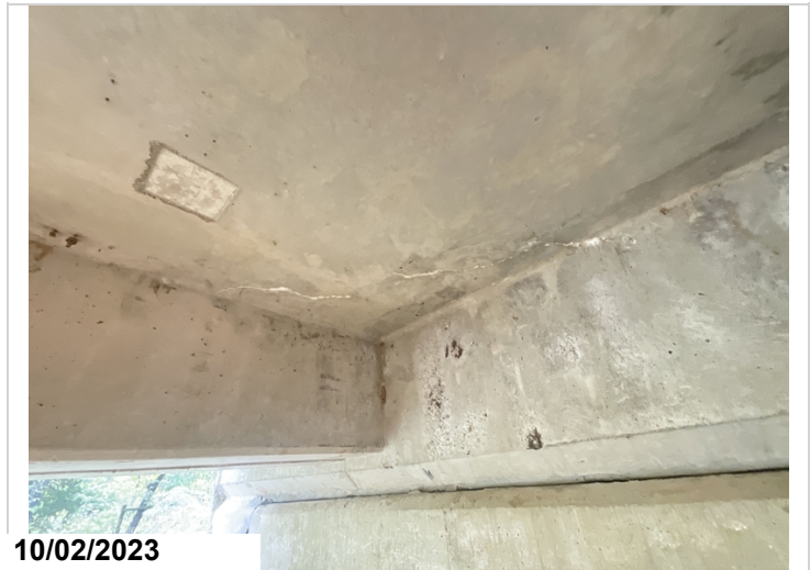
Span 1 at bent 1 bay 4 efflorescence in bottom of deck
