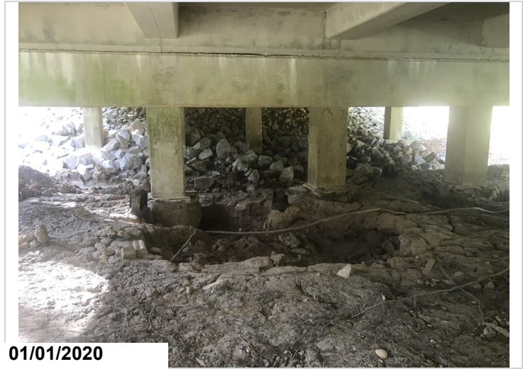
Erosion around bent #3
