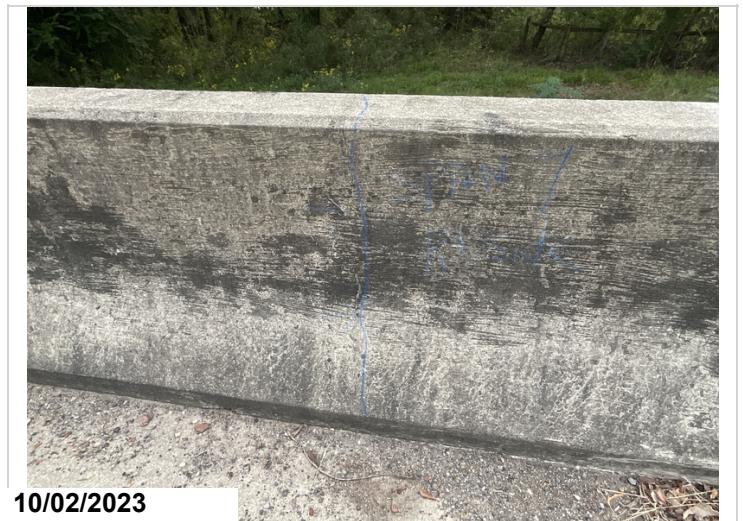
Span 1 right side cracking in parapet wall
