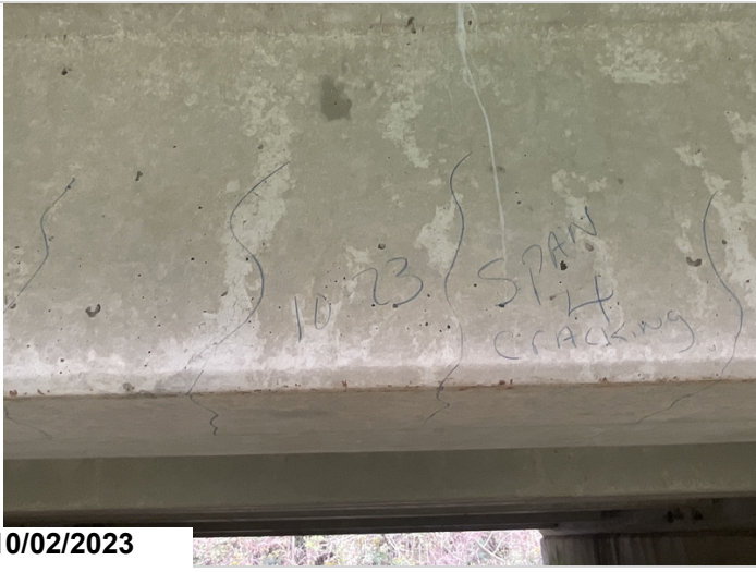
Span 4 photo taken of very light cracking in tee beams 0.010 size.
