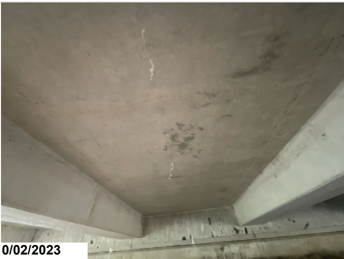
Span 1 bay 3 efflorescence in bottom of deck
