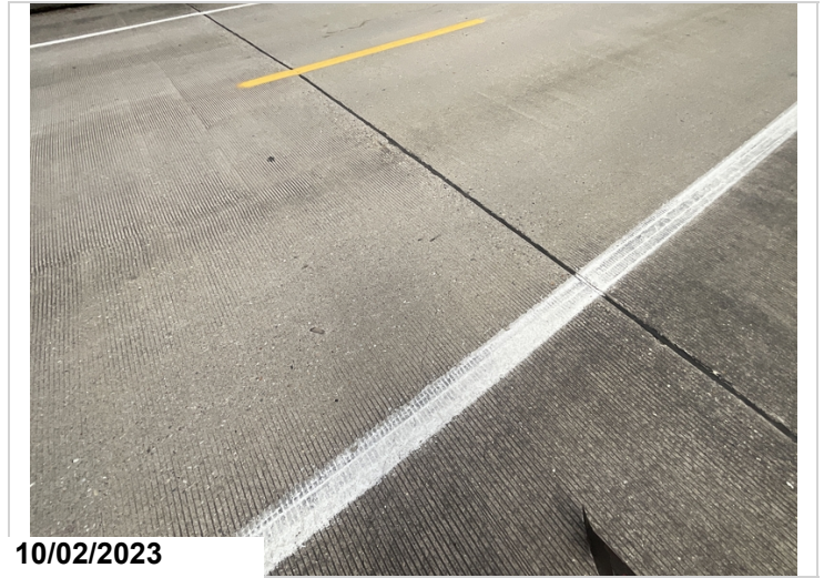
Span 7 cracking in top of deck 0.018
