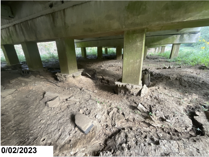
Bent 3 concrete poured around steel piles.
