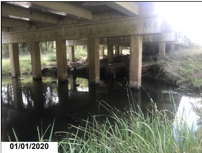
Erosion at under Span #6 7' deep hole width of bridge
