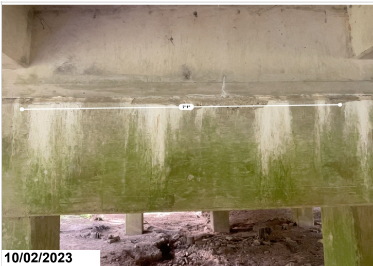
Bent 5 span 5 small spall on top of cap 7 ft long.
