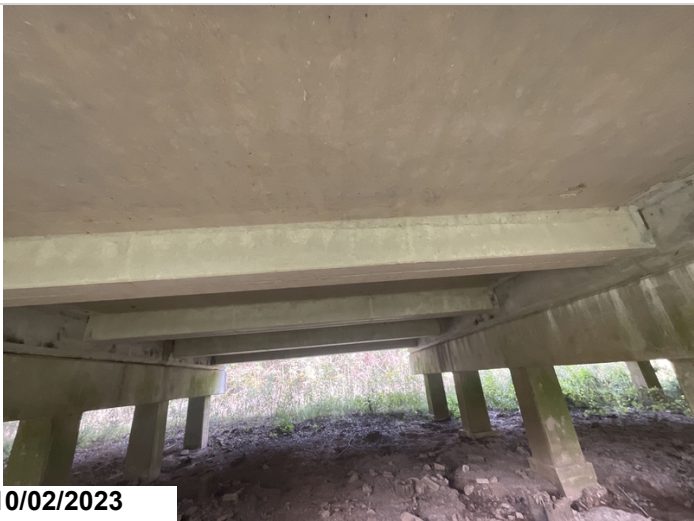
Typical photo of tee beams
