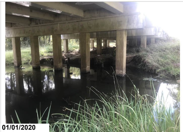
Erosion at under Span #6 7' deep hole width of bridge
