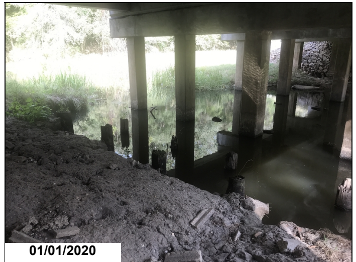
Erosion under Span #6
