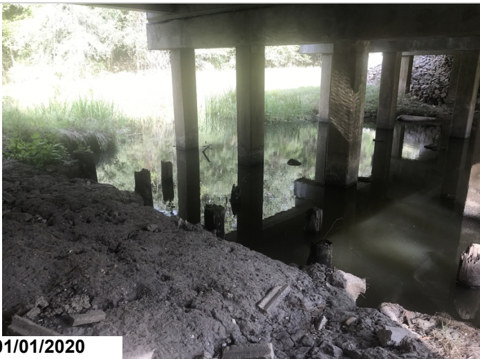
Erosion under Span #6
