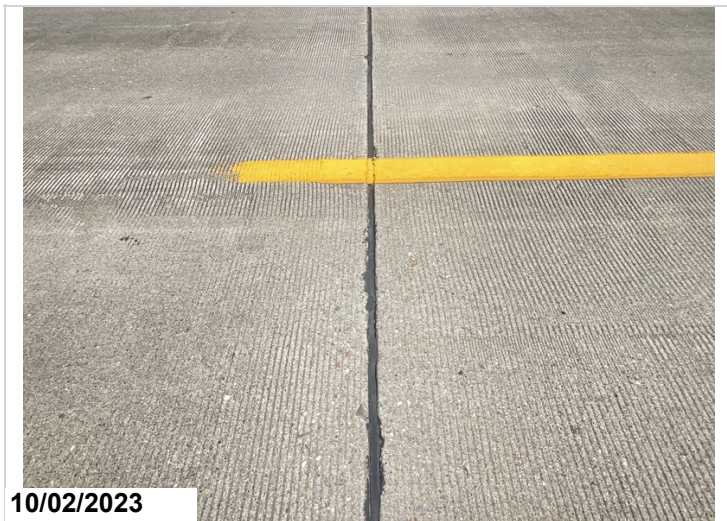
Joint material at bent 2
