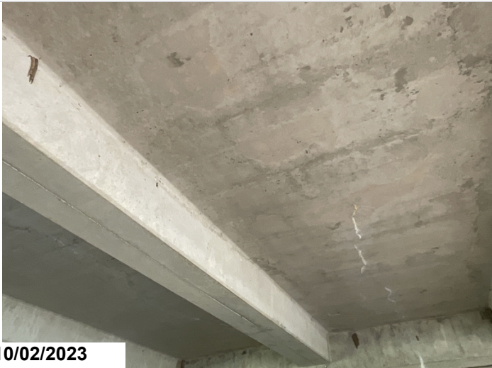
Last span bay 2 and 3 efflorescence bottom of deck
