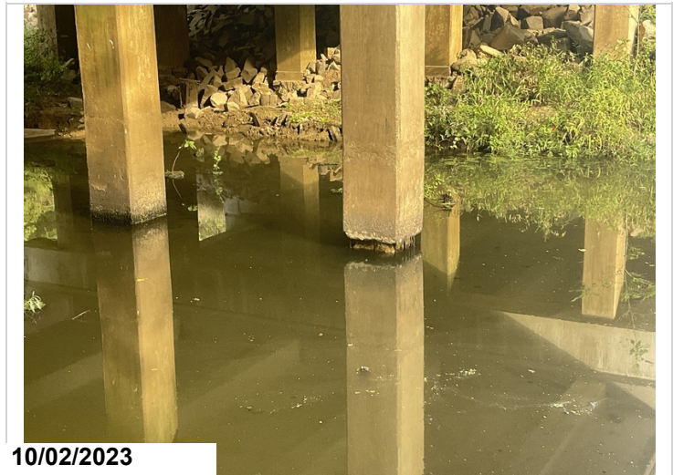
Bent 8 pile 5 concrete encasements has come apart at ground line exposure of rebar with heavy section loss to rebar. Note concrete is only encasements for steel pile
