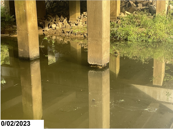
Bent 8 pile 5 concrete encasements has come apart at ground line exposure of rebar with heavy section loss to rebar. Note concrete is only encasements for steel pile
