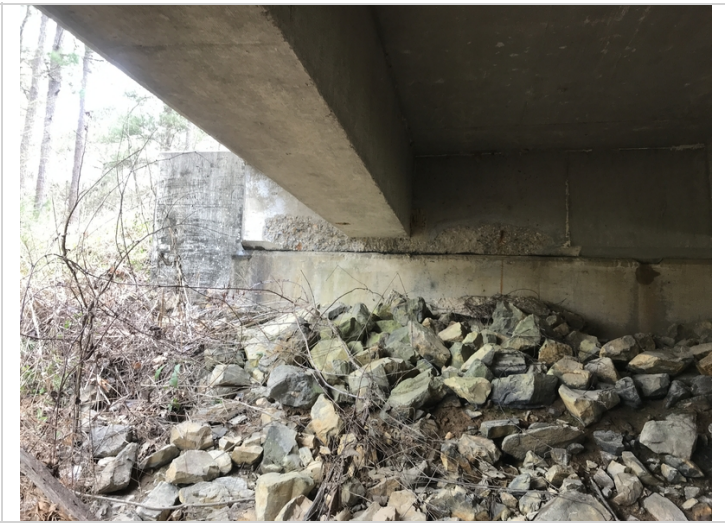
Approx. 10 ft spall on horizontal deck wall at bent 1 under beam 5...
