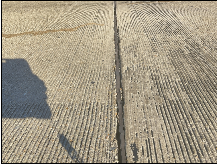
Joints need cleaned and repaired typical all joints
