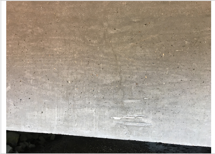
Minor cracks on concrete tee beams in various locations
