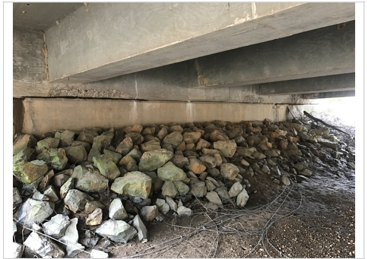
Approx. 20 ft of spalling on horizontal deck wall at bent 5.
