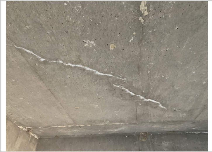
02/2022 efflorescence
