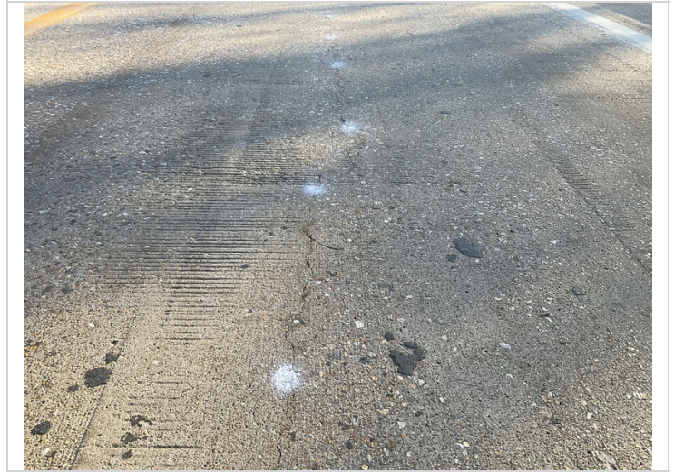
2022 cracking in deck
