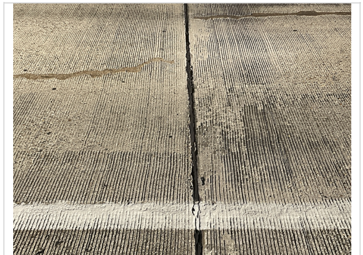
Joints need cleaned and repaired typical all joints
