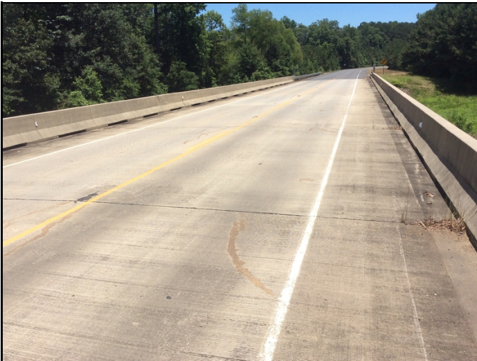
Deck cracks
