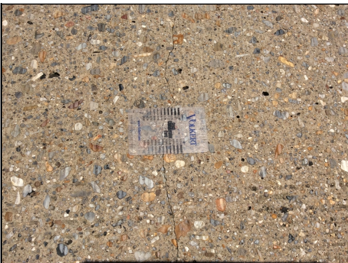
Deck cracks 0.030 size
