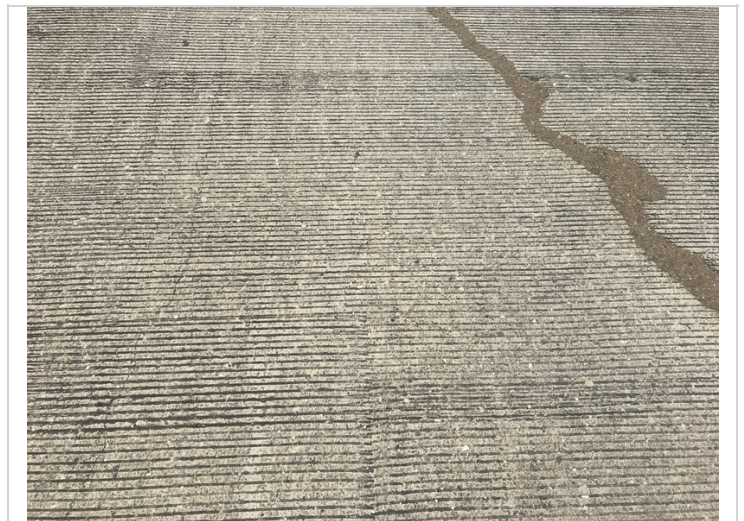
Some cracks sealed and other not sealed
