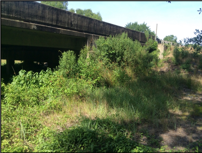
TREES AND BRUSH GROWING UNDER AND ALONG SIDES OF BRIDGE
