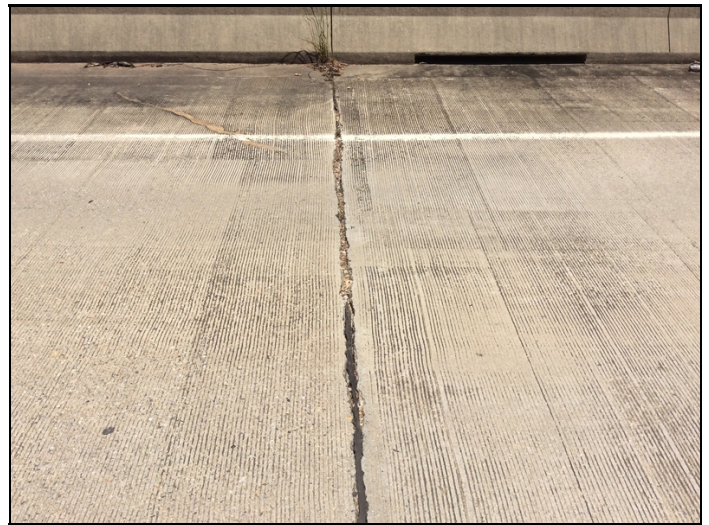
ALL JOINTS HAVE SOME AREA 'S OF MISSING MATERIAL,
