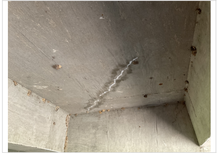
Efflorescence on underside of deck various locations
